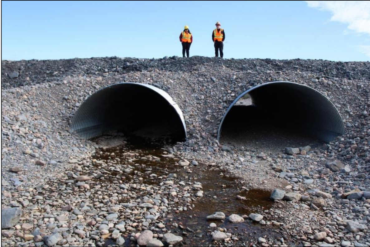
Photo 22: Culverts installed at Rascal Stream Crossing.
