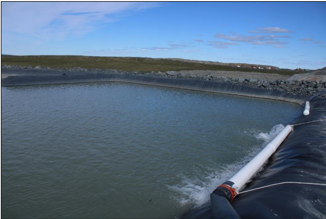
Photo 21: Lime Treatment being applied to sedimentation Ponds.
