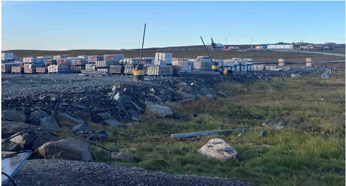
G-17: Laydown, looking S towards airstrip
