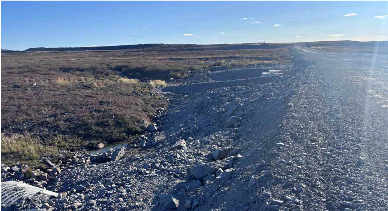
G-29: South side road rockfill, looking SW
