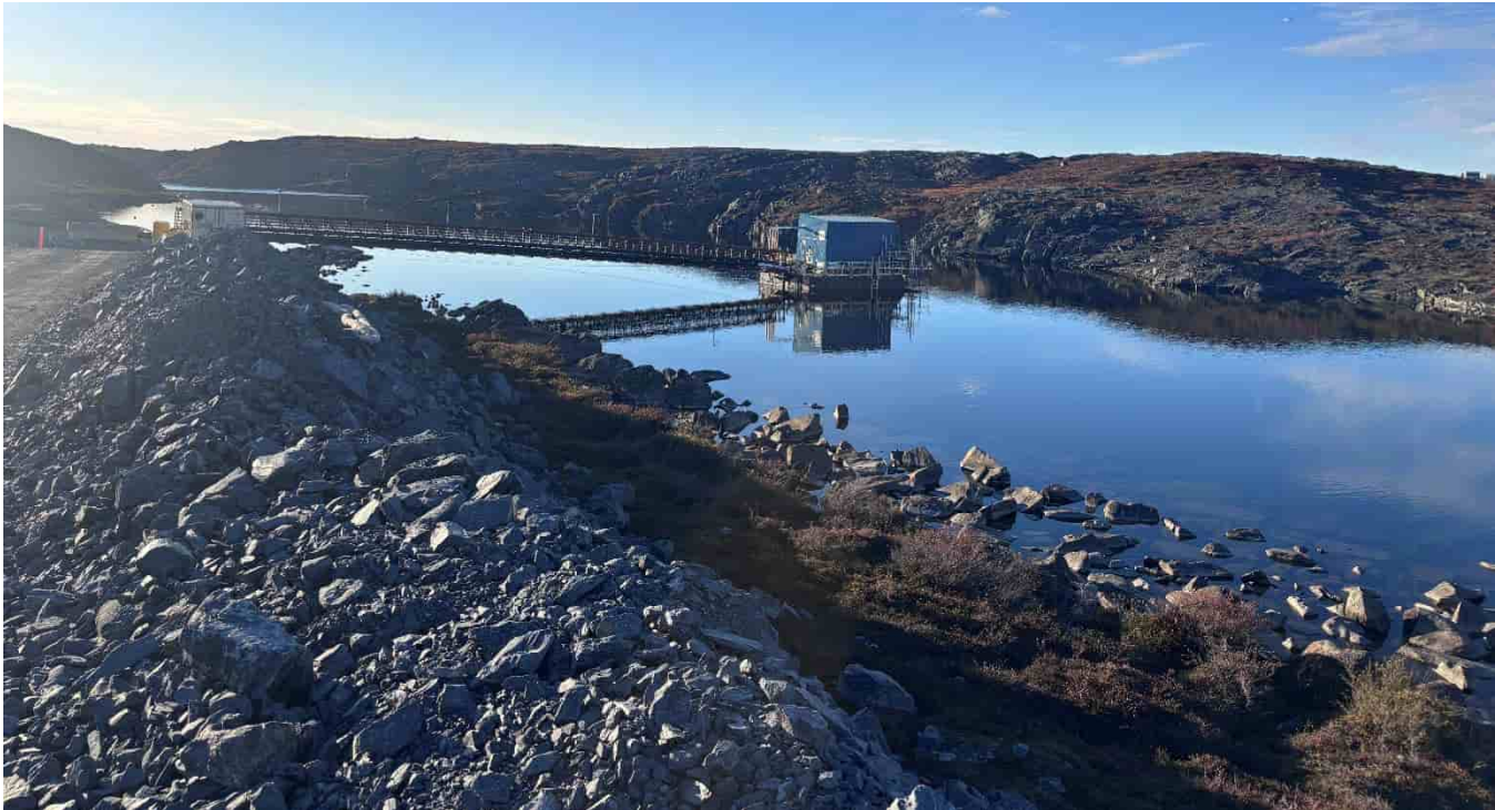
G-175: Barge access dock and pad slope above lake
