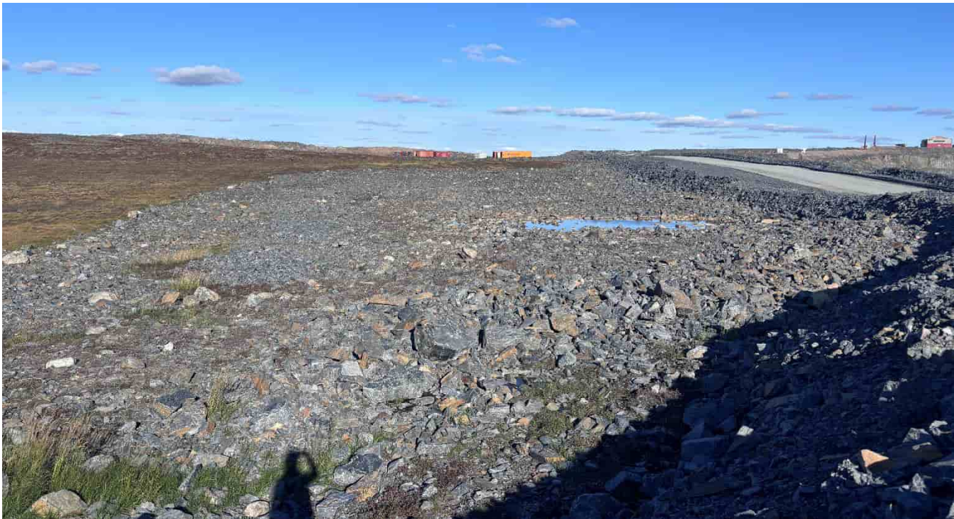
G-167: Acces road, looking NE
