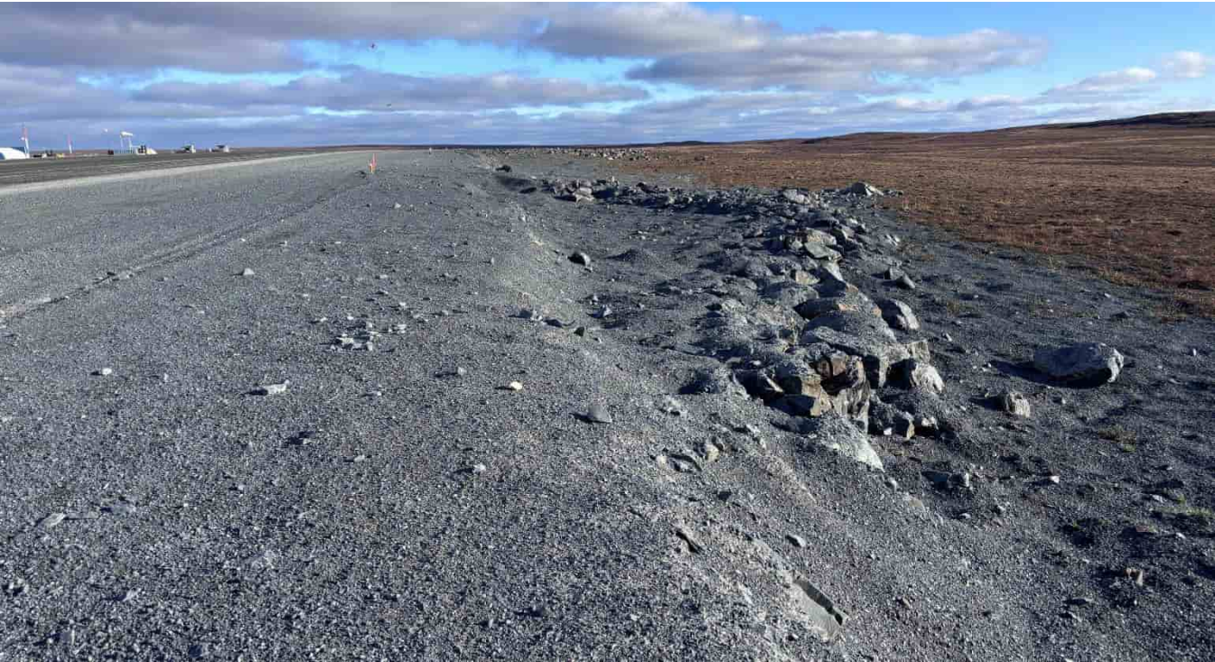
G-52: SW runway rockfill, looking SE – Undefined edge in area
