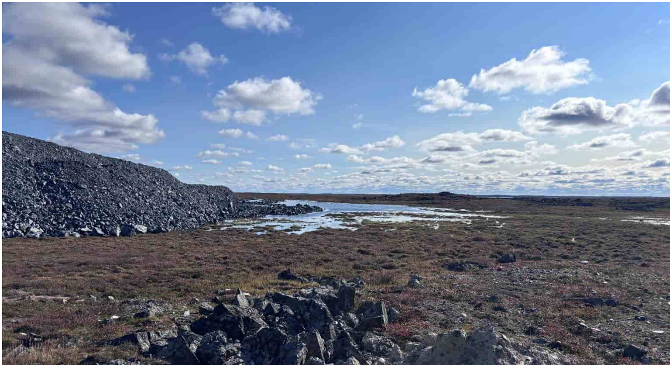
G-144: Waste rock dump in pond, as seen from diversion – Steeper slopes into ponded area
