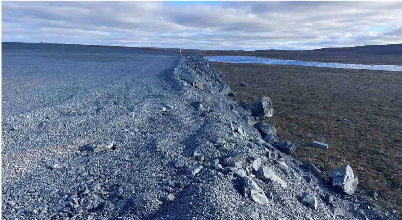
G-32: SW slope of SW airstrip apron, looking SE
