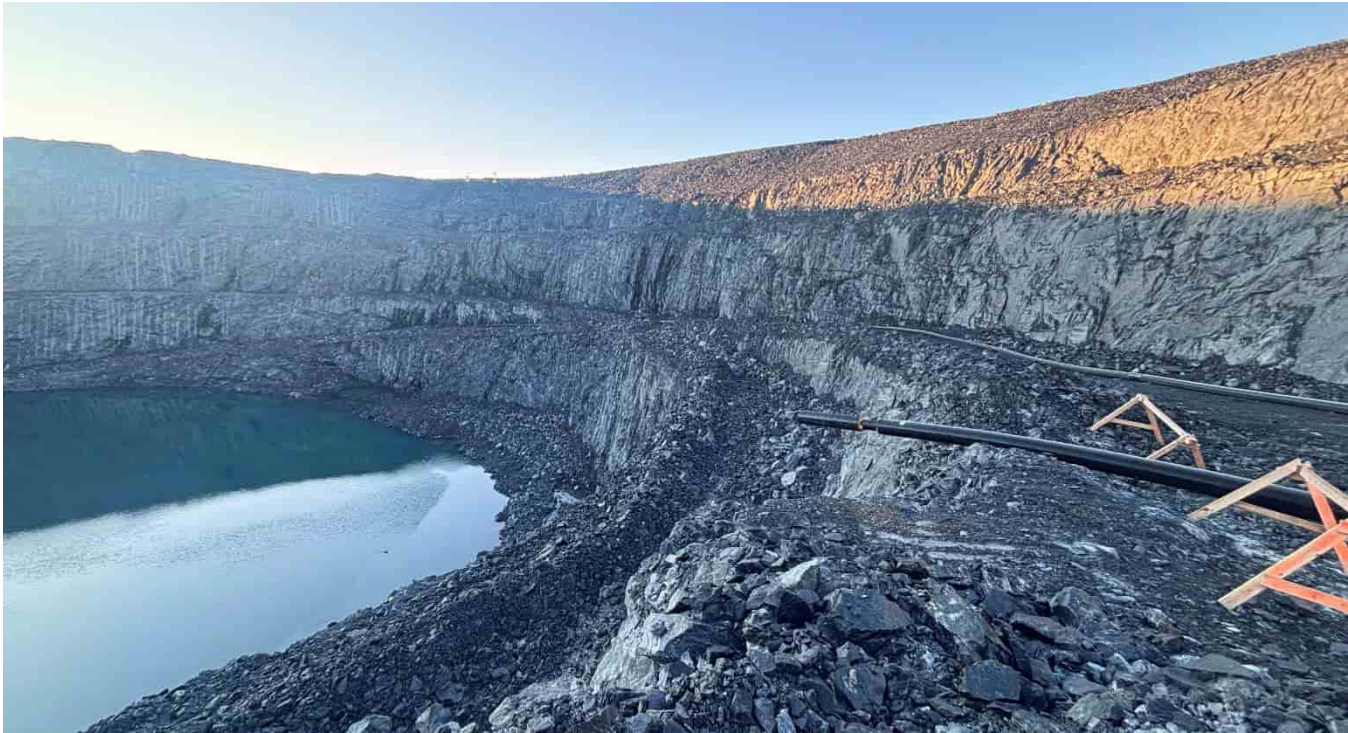
G-112: Western wall, looking S + tailings pipeline in place
