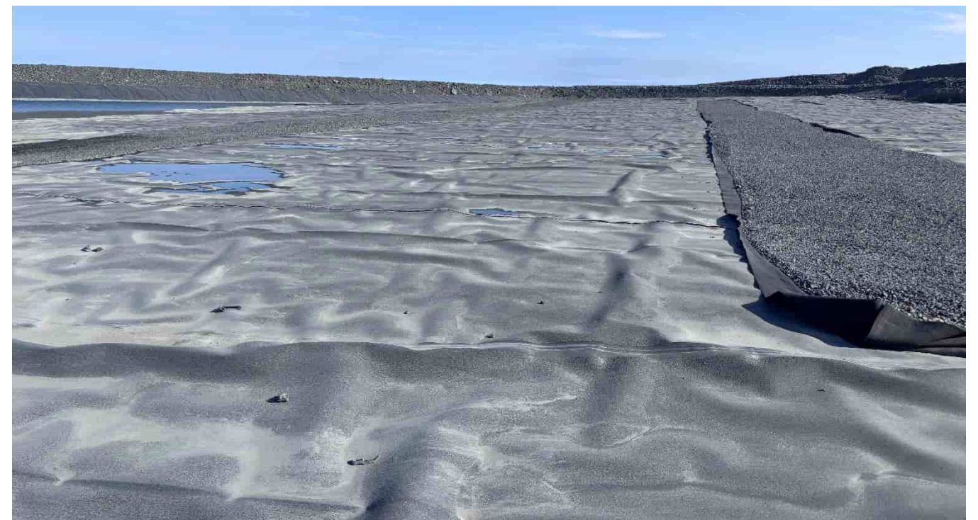
G-235: Typical liner surface conditions, looking NE
