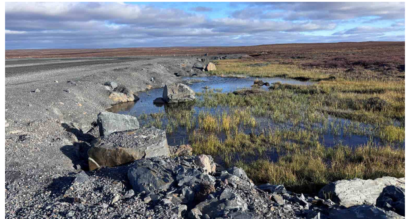
G-56: Ponding at SE end of runway, looking SE
