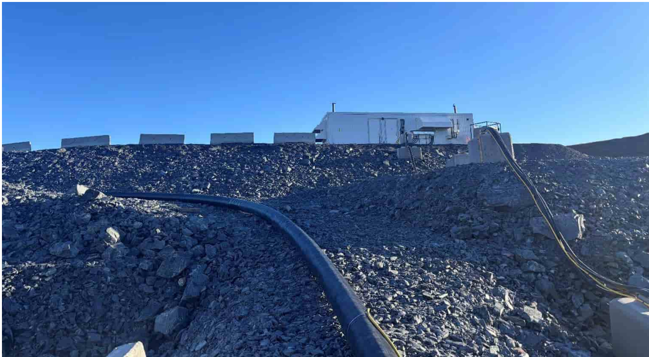
G-176: Slope above barge access road and pipeline, looking S
