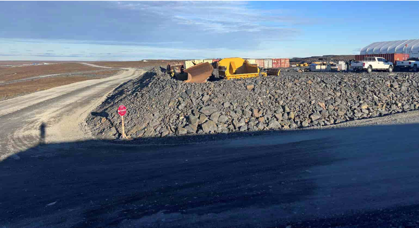
G-185: Junction between All-Weather Road and operations area access road, looking E
