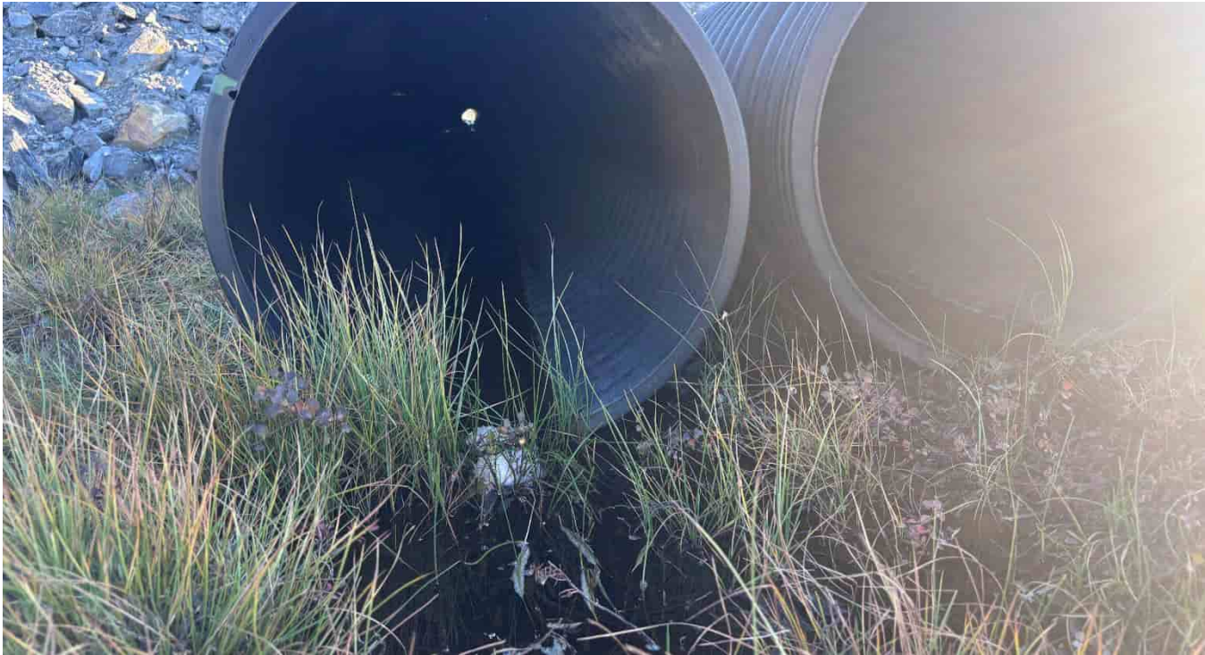
G-90A: Downstream (N) end of western culverts
