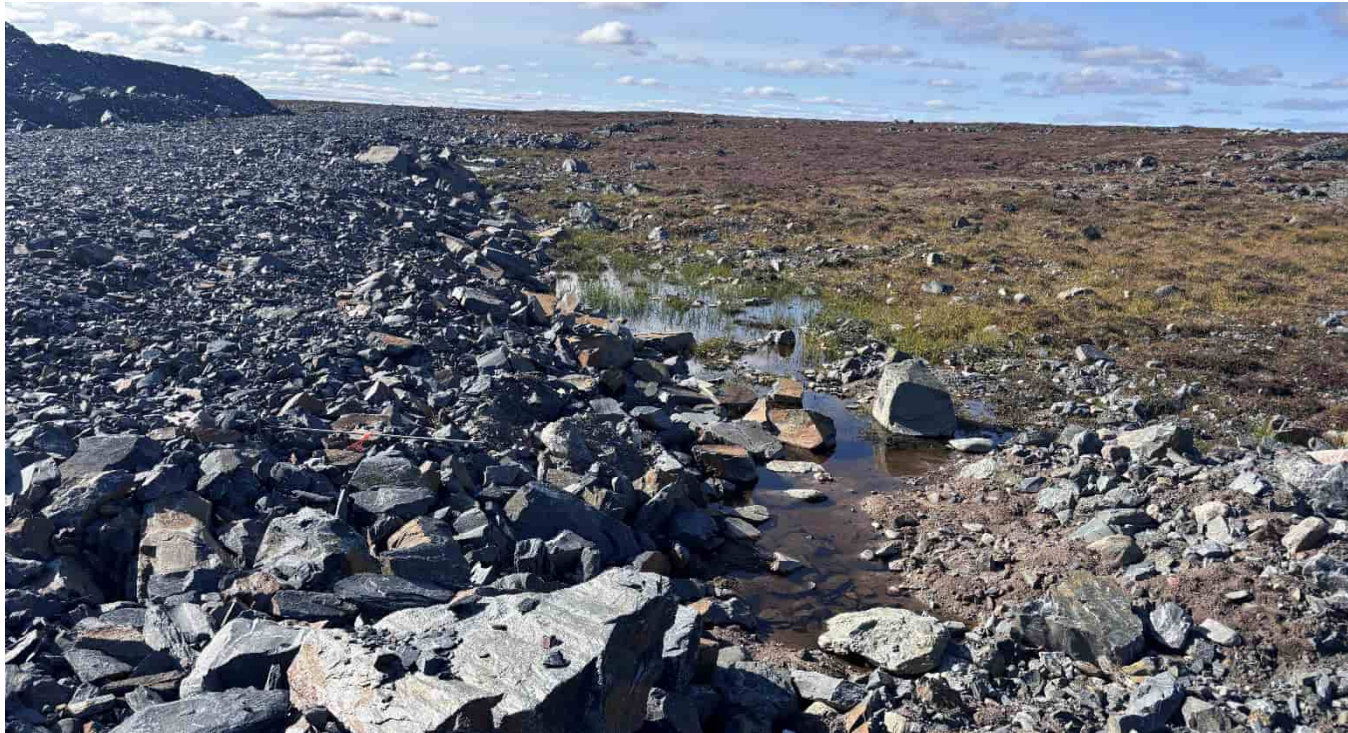
G-142: Ponding water beside diversion, looking SW – thin rockfill placements in area
