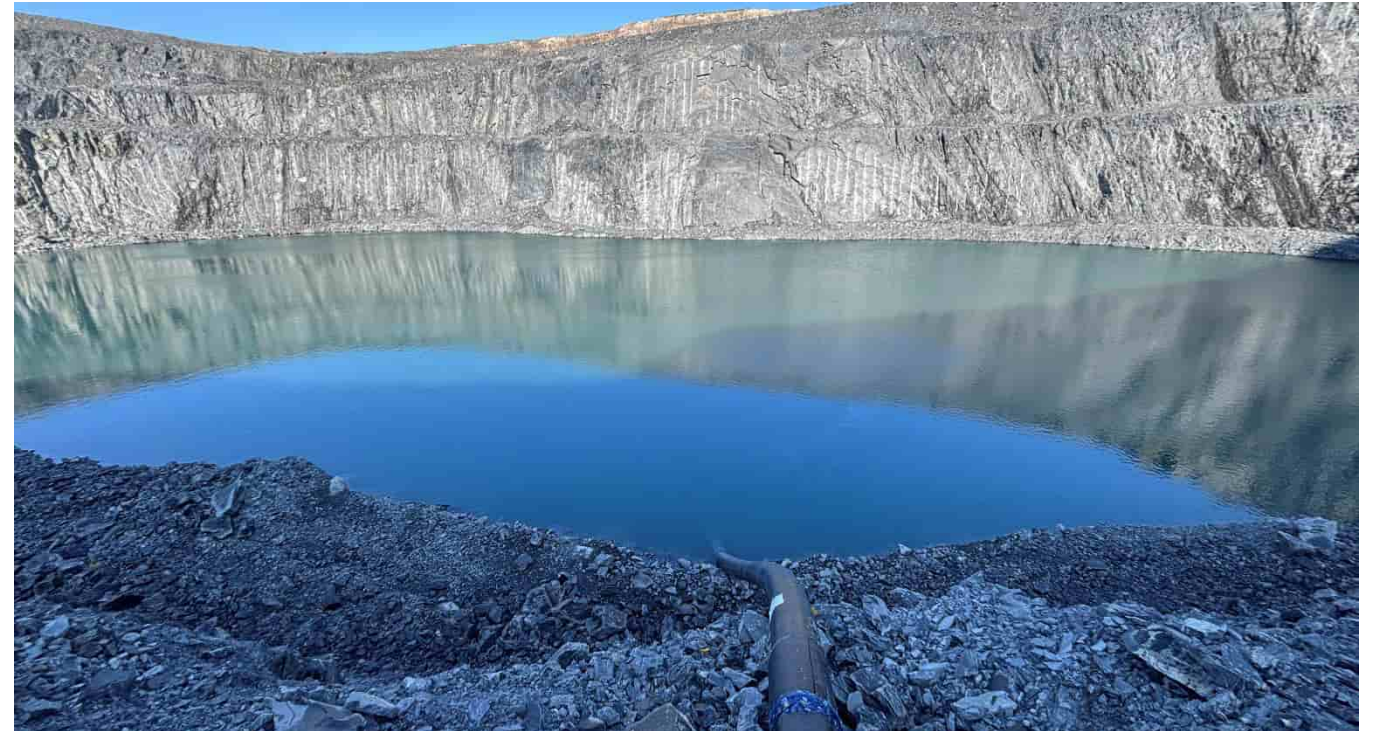
G-124: Tailings deposition pipeline entrance into pond, looking N
