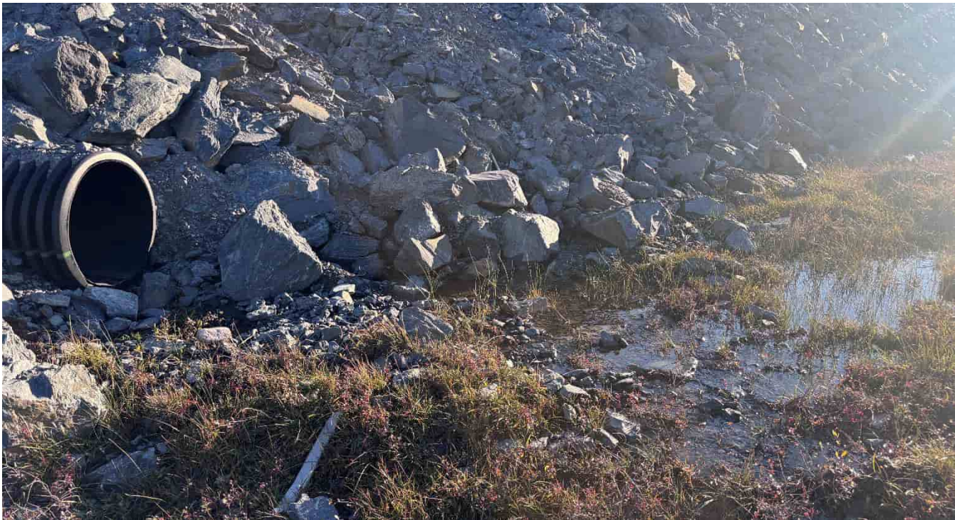
G-91: Downstream (N) end of eastern culvert
