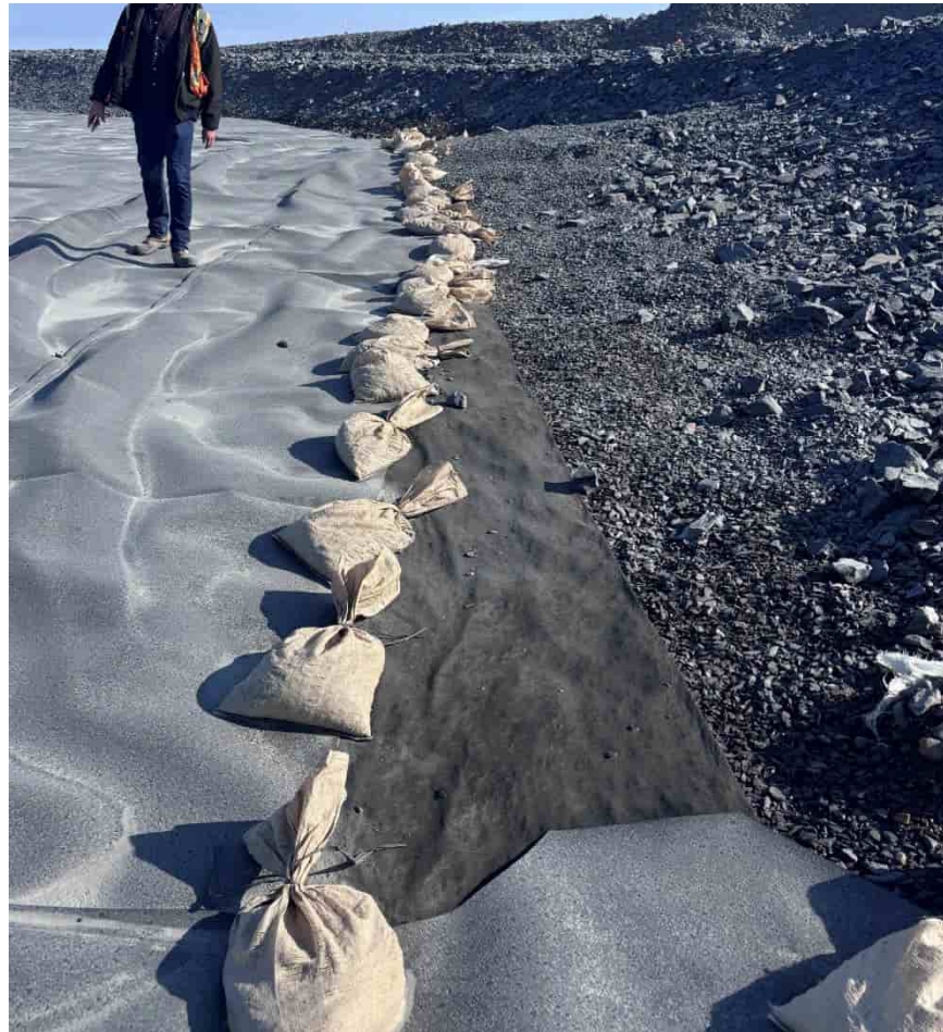
G-233: Typical S edge of liner condition, looking E – liner daylighting / laid ont tundra at this edge
