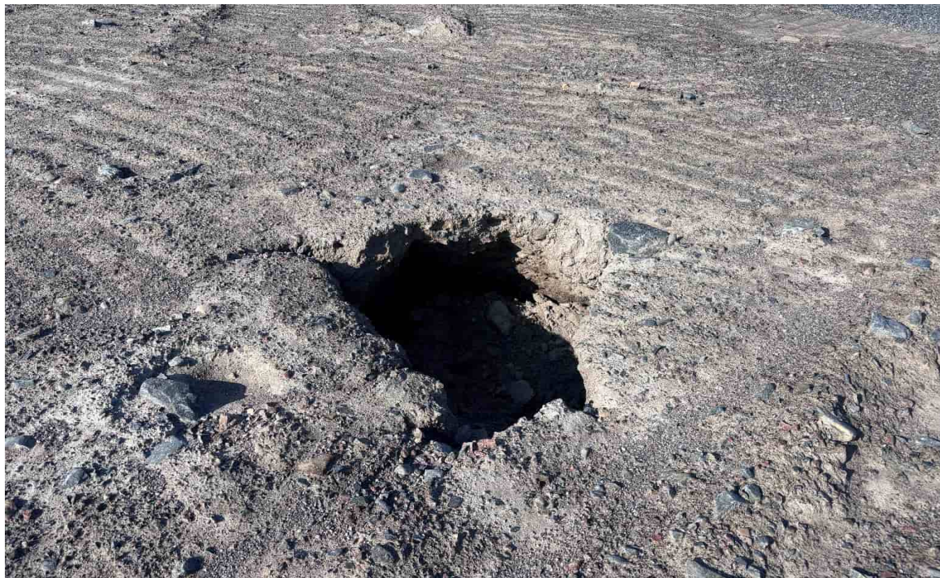
G-131: Example of the sinkhole in eastern side of the overburden stockpile
