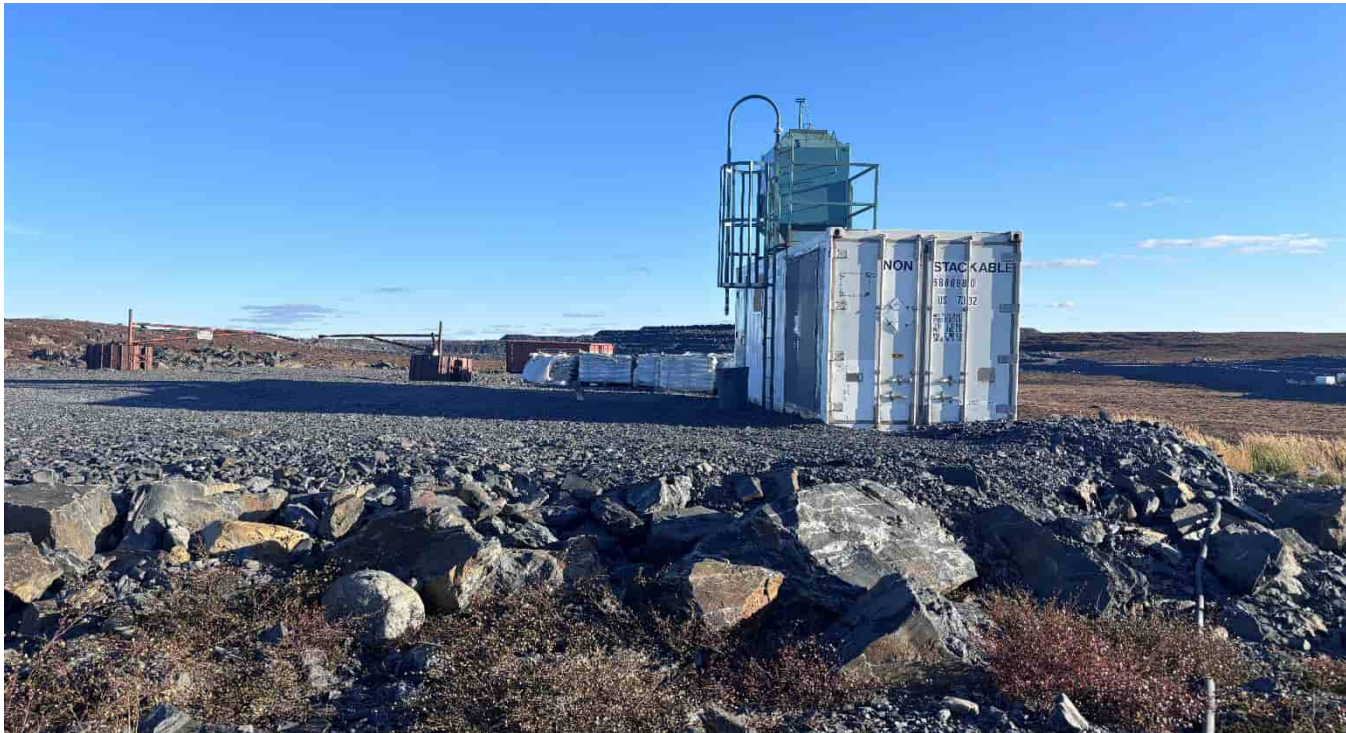
G-106: Old explosive storage pad, looking S
