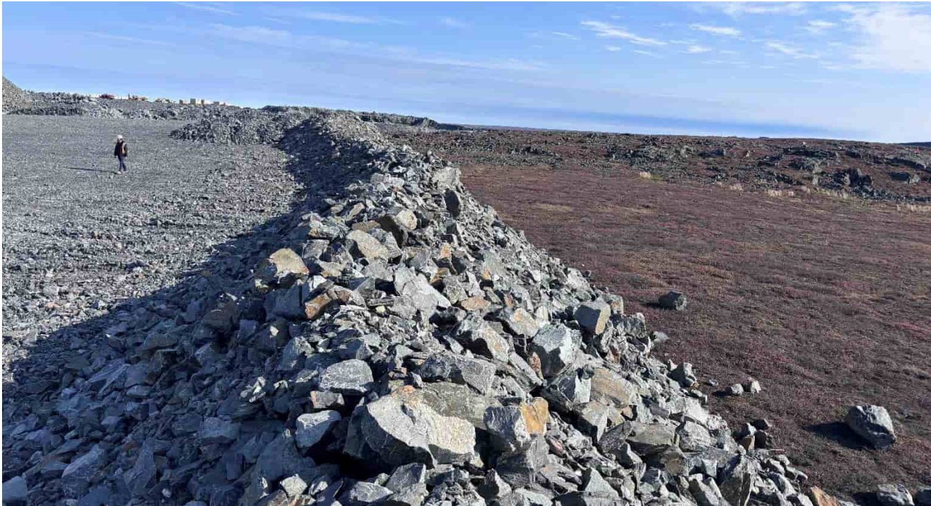
G-224: Edge of S side of pad, looking E
