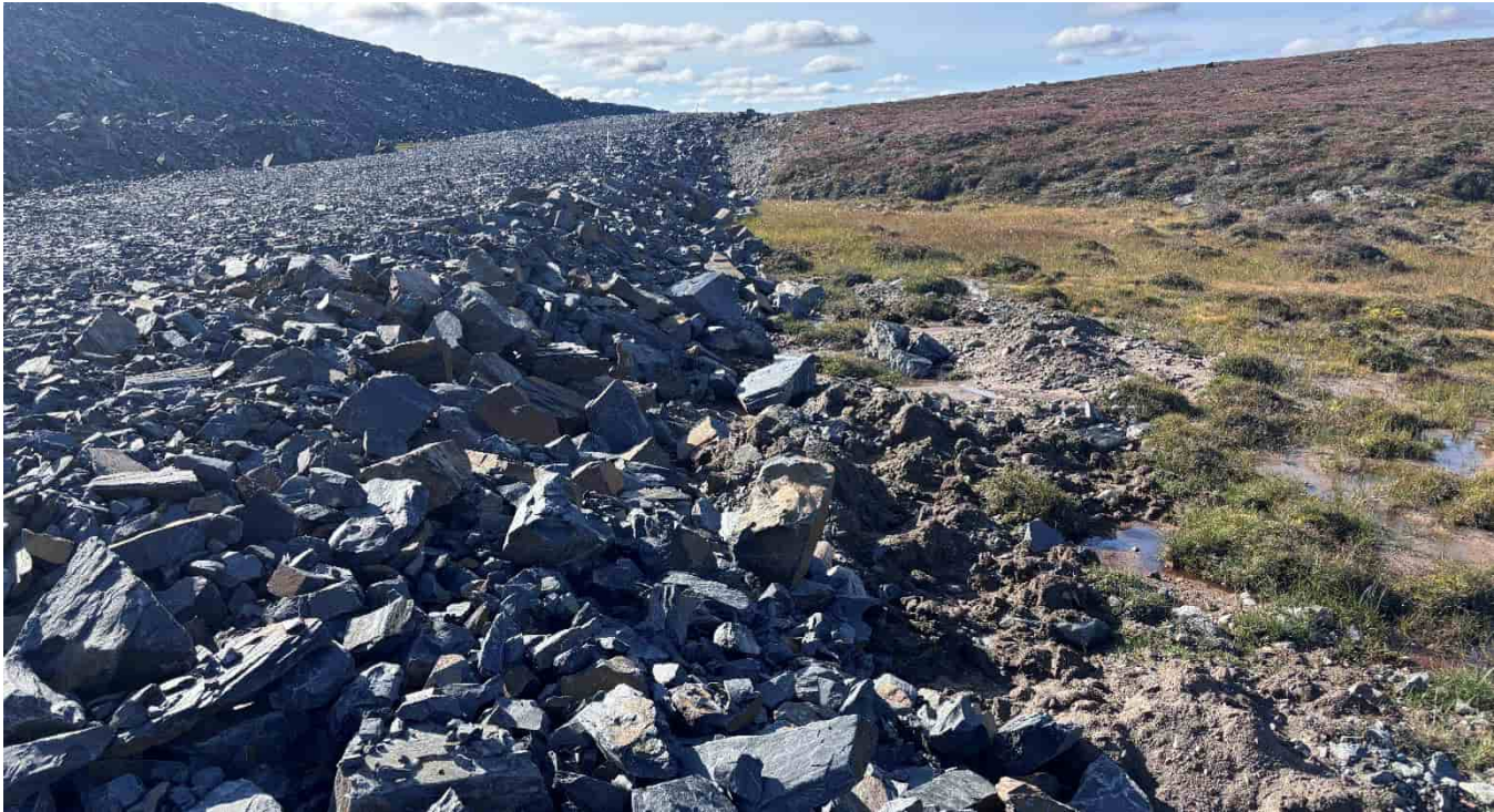
G-139: Beginning of diversion, looking SW – some ponding water
