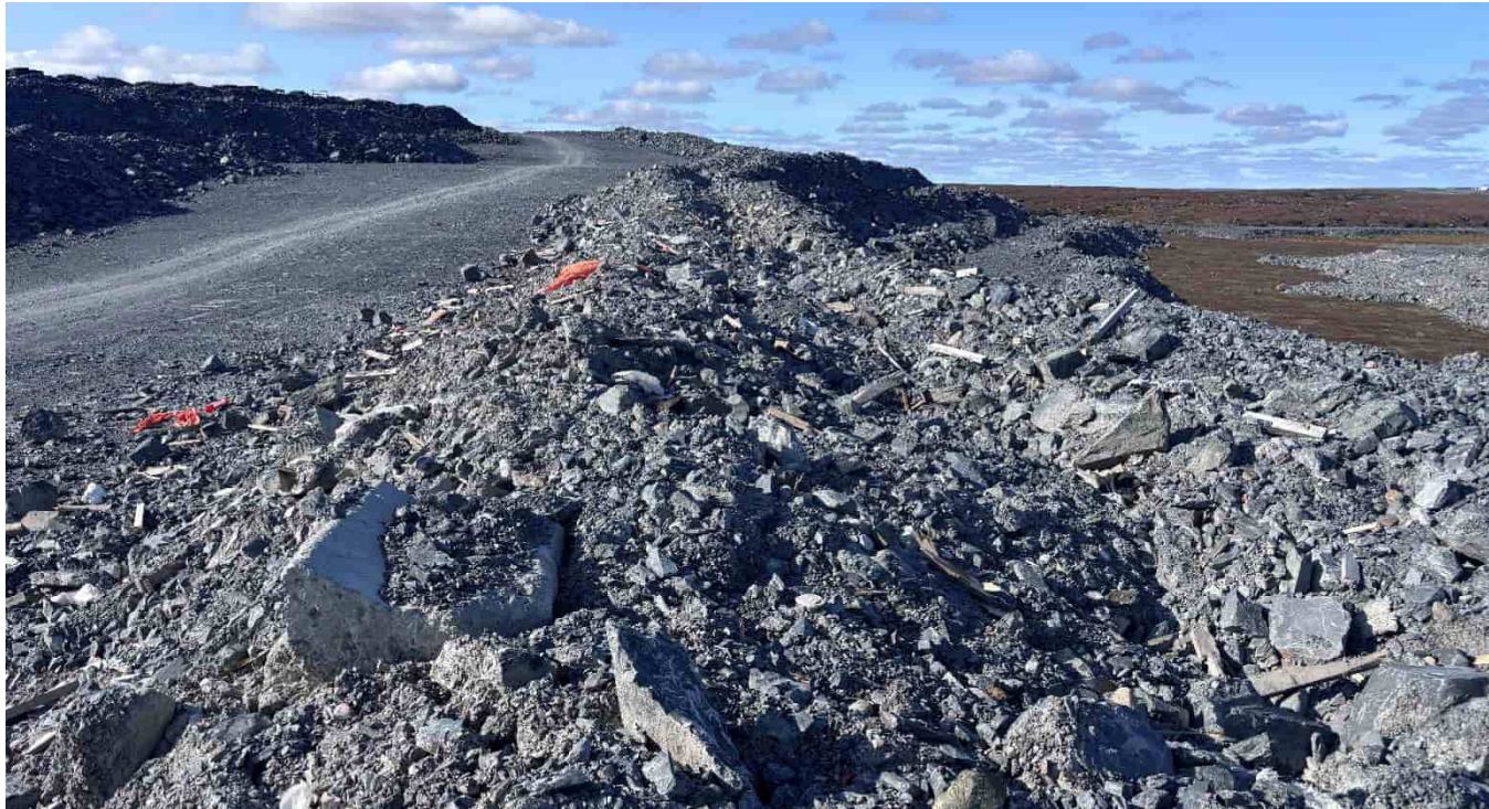
G-134: Entrance road to Echo WRSA, looking SW – Garbage in upper windrow
