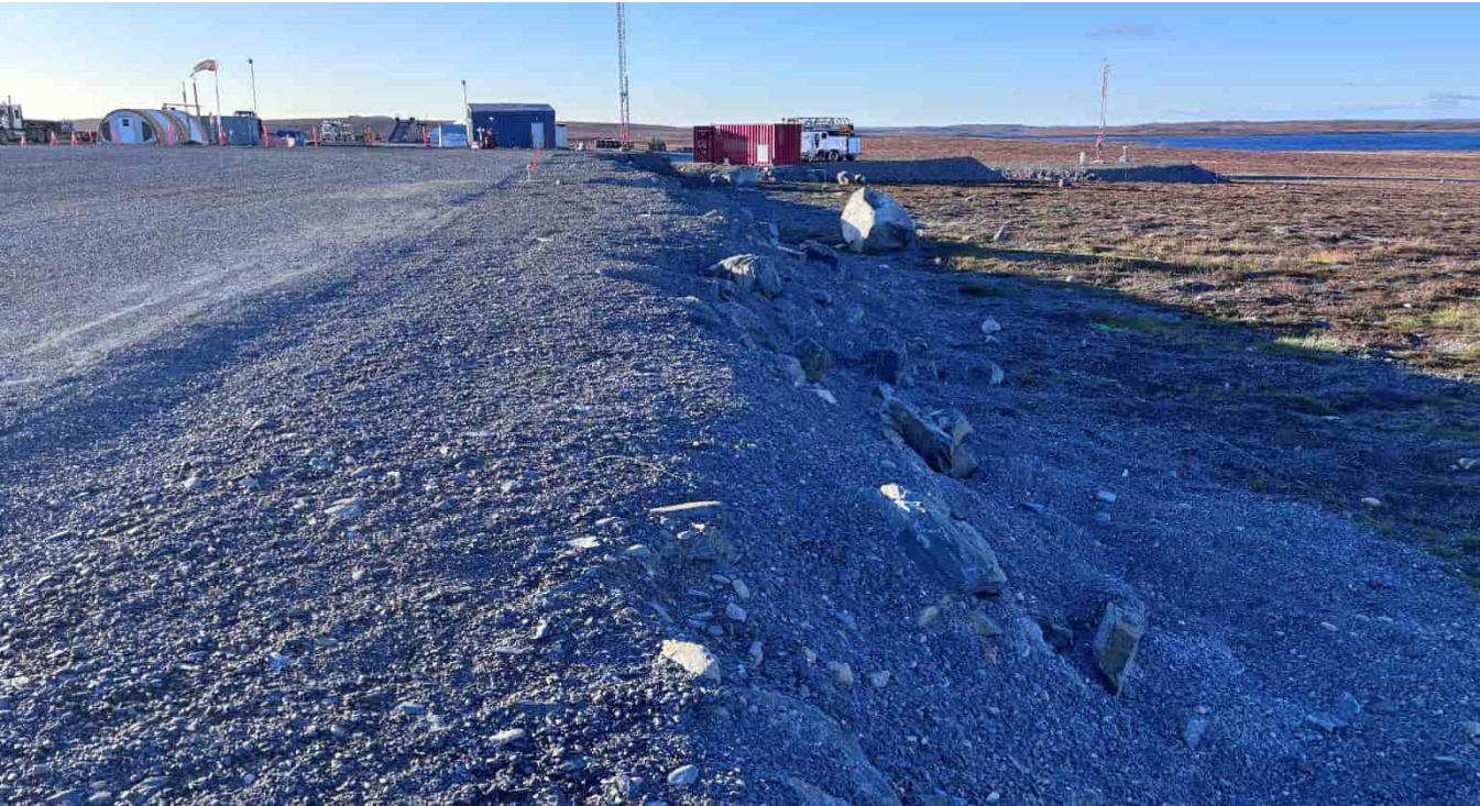
G-68: Slopes of NE apron south of laydown area
