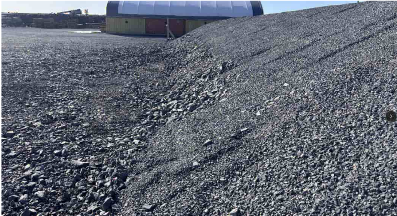
G-216: Tote Storage Facility: Toe of the eastern berm
