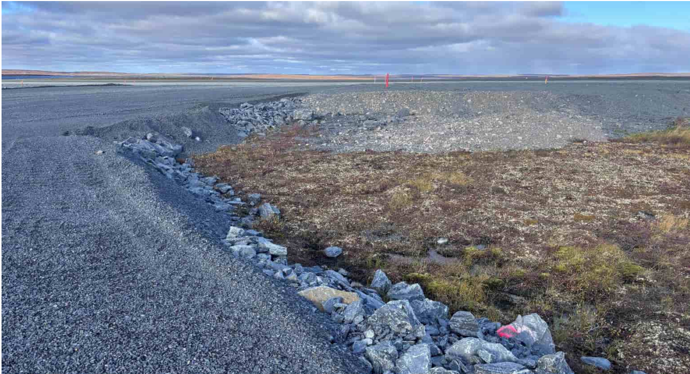
G-40: Looking NE towards runway from SW apron
