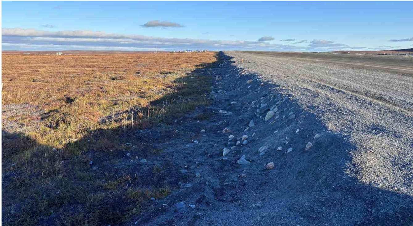
G-75: Typical runway slope, looking SE
