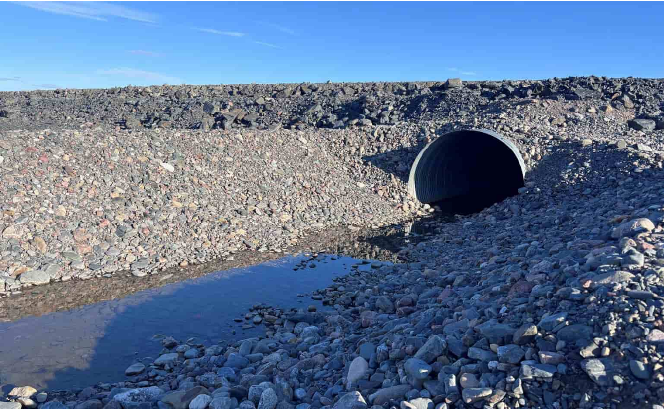
G-27: Downstream (N) side of eastern culvert
