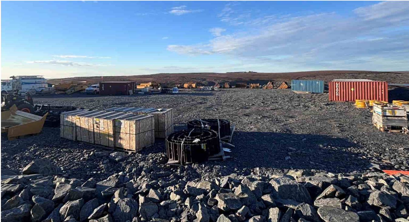
G-193: Laydown area N of Sandvik
