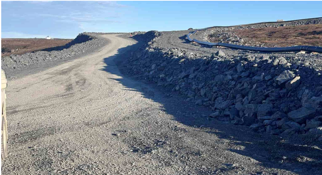
G-182: Barge area access road, looking SE
