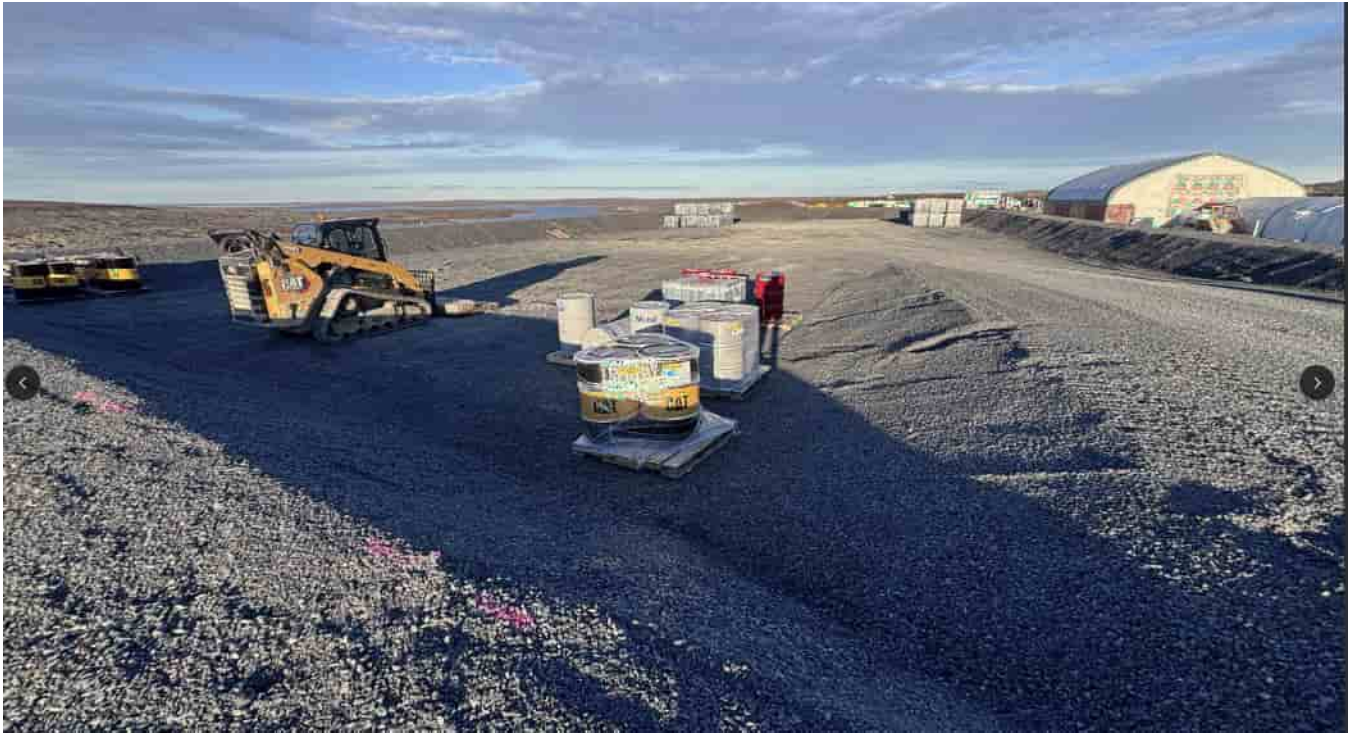
G-217: Tote Storage Facility, looking E
