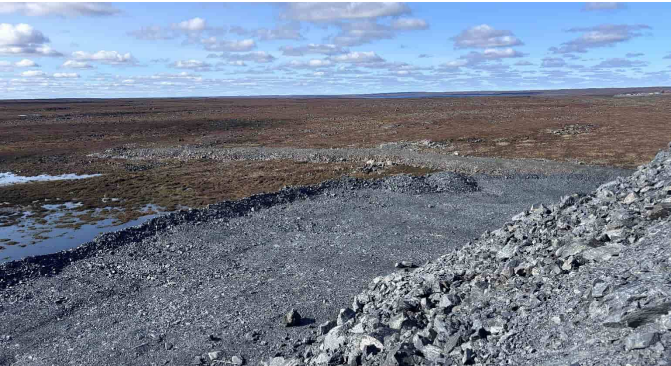
G-137: Looking SW towards Echo Diversion from waste rock storage area - ponding water on SSW end
