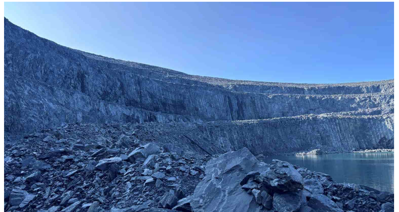
G-125: Southern wall and tailings pipeline, looking W
