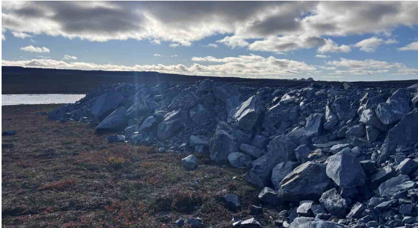
G-39: SE rockfill of SW apron, looking SW – Some larger boulders notes near edges
