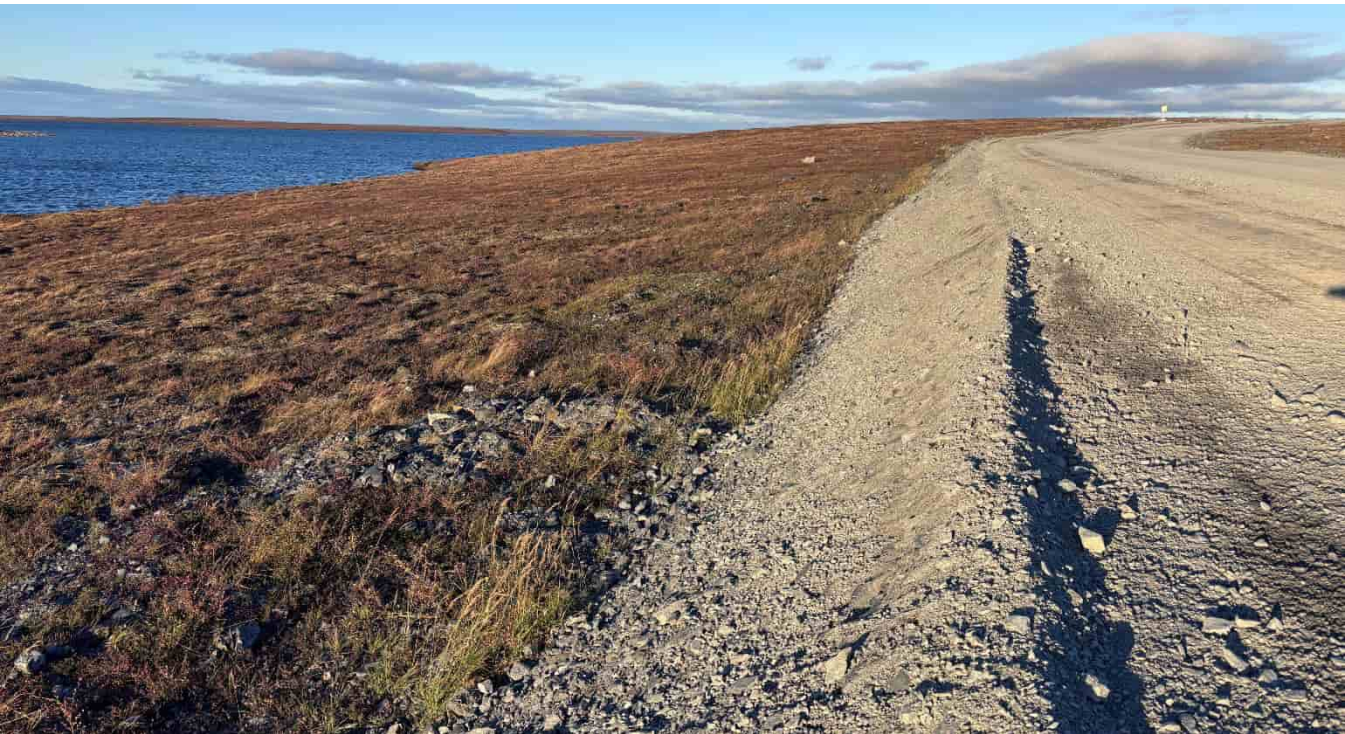
G-86: Typical rockfill of All-Weather Road beside airstrip
