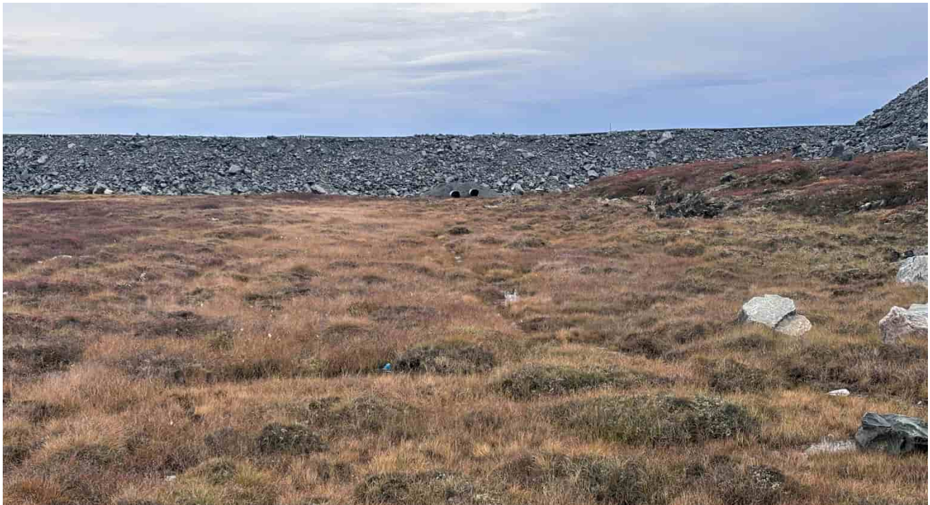
G-206: Tundra, looking SE towards tailings pipeline road rockfill and culverts
