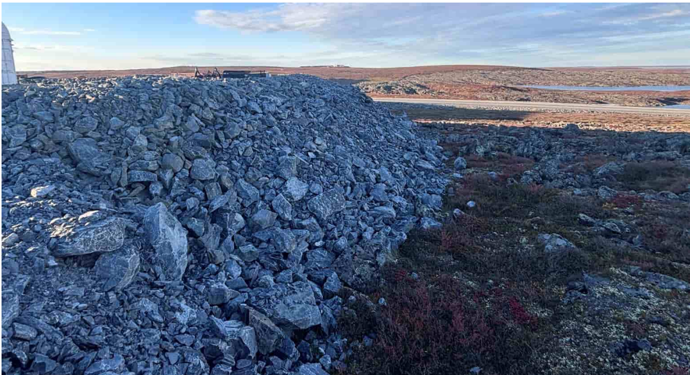
G-195: Pad slope beside Sandvik, looking N
