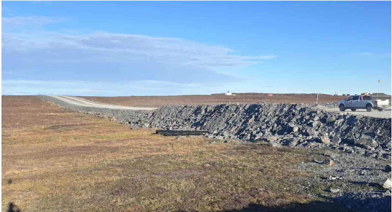
G-89: N rockfill of All-Weather Road looking towards echo crossing culverts
