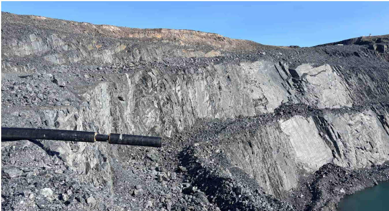
G-121: Tailings deposition pipeline end, looking NE
