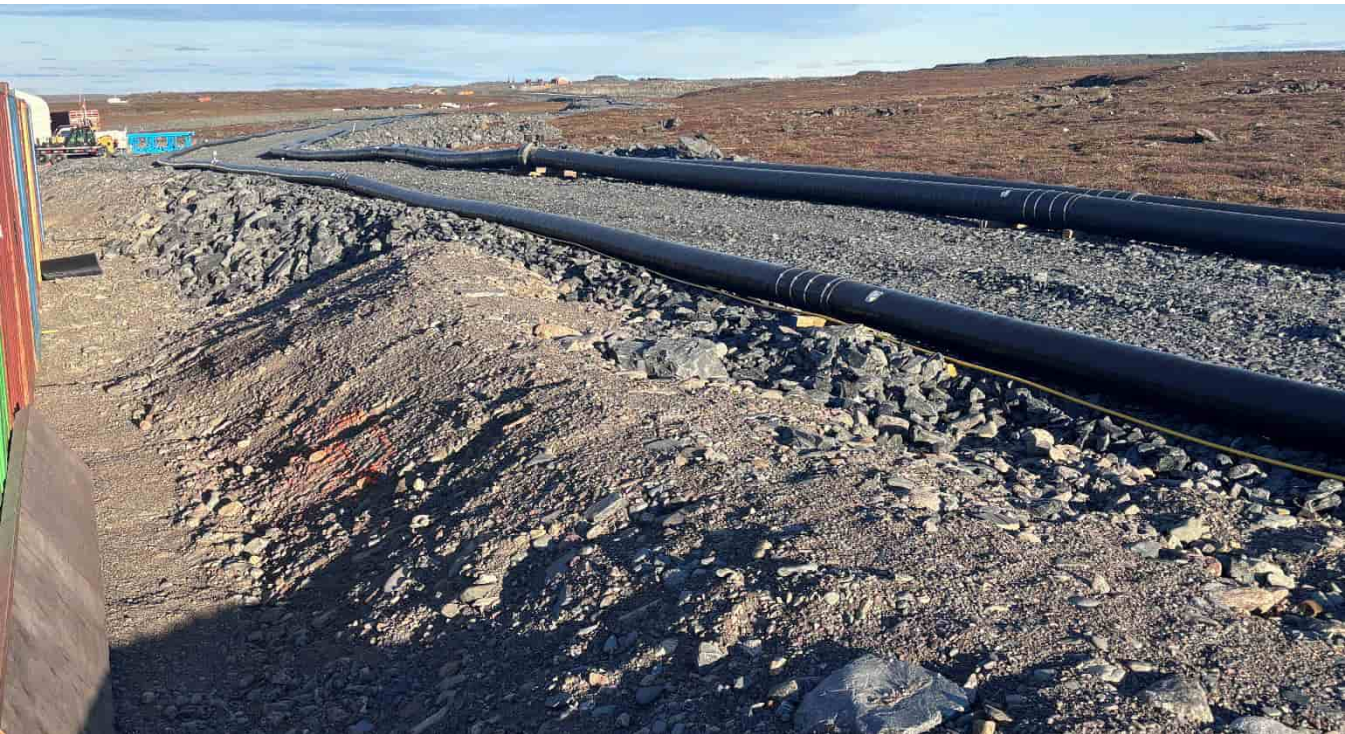
G-191: Berm between laydown area and tailings pipeline, looking E
