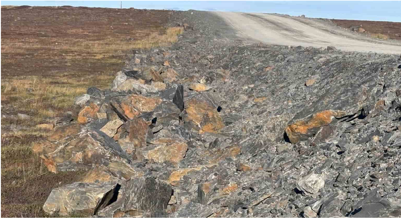
G-93: All-Weather Road N rockfill, looking E
