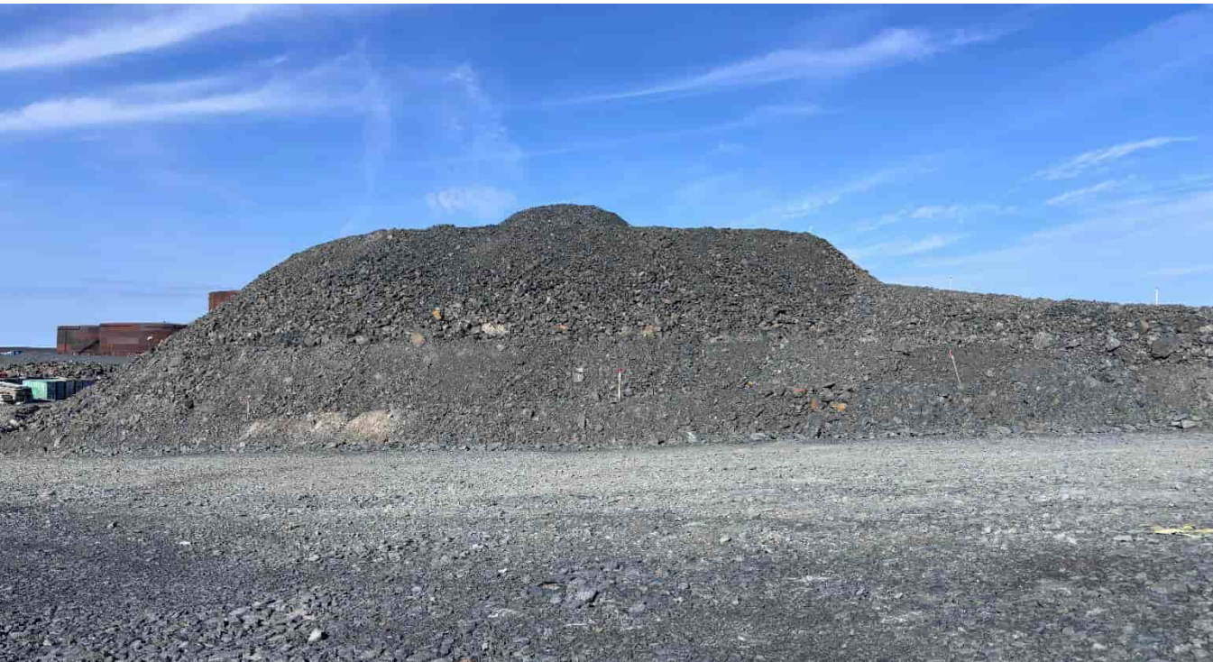
G-222: ROM stockpile slopes
