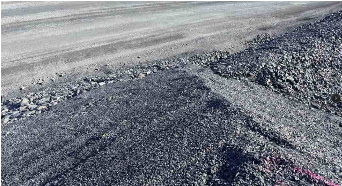
G-215: Tote Storage Facility: Northern berm, looking N form the berm crest
