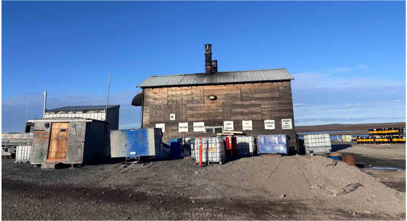
G-7: Incinerator, looking NE
