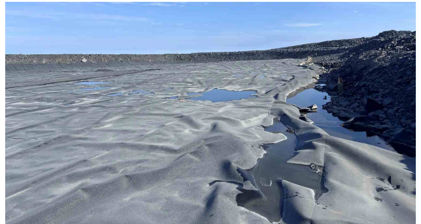
G-234: Ponding water at S edge of pond, looking E – Note varying crest of liner
