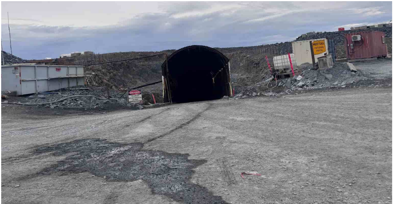
G-202: Underground portal, looking SW
