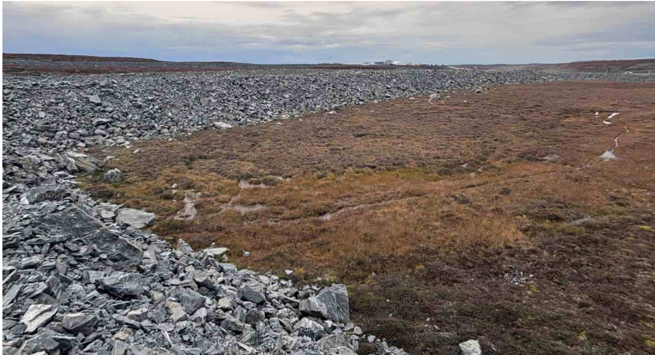
G-172: Tire pad and road rockfill, facing W – minor ephemeral stream flow
