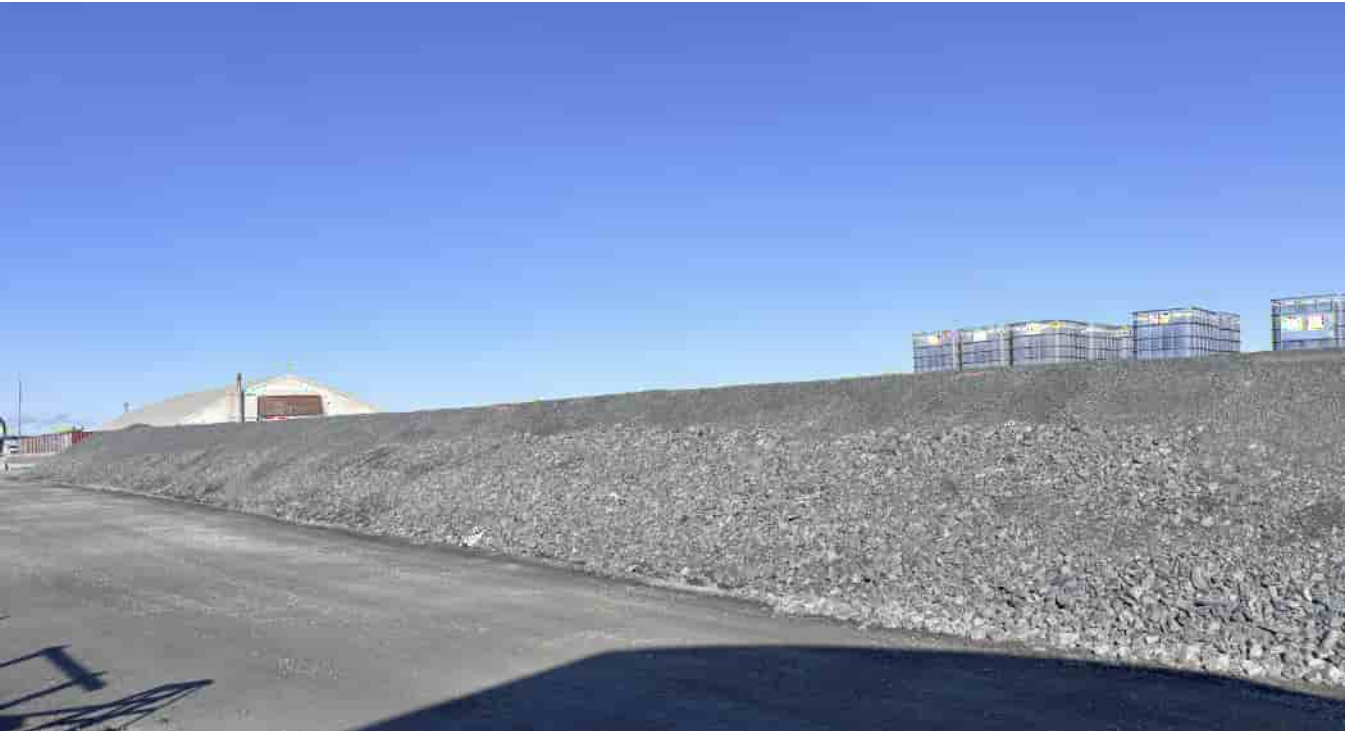
G-209: Tote Storage Facility: Southern berm
