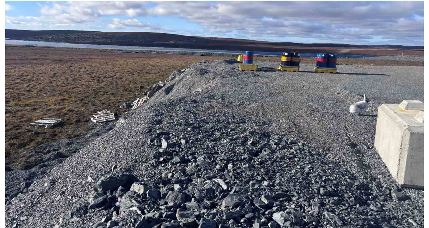
G-33: Slope of SW apron, looking NW
