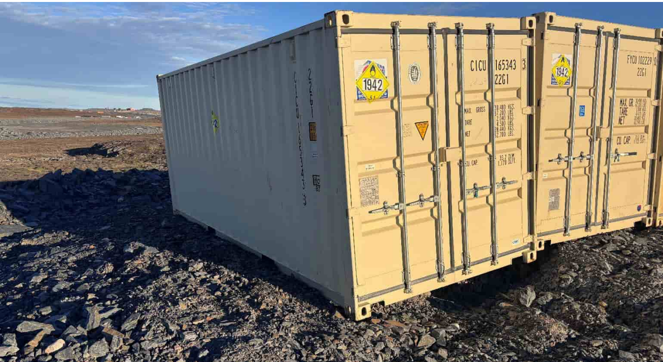
G-199: Differential settlement of northernmost seacan in Sandvik laydown area
