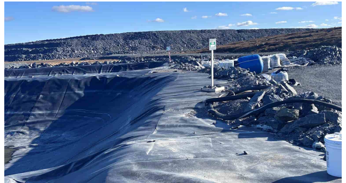
G-155: Coarse over-liner material
