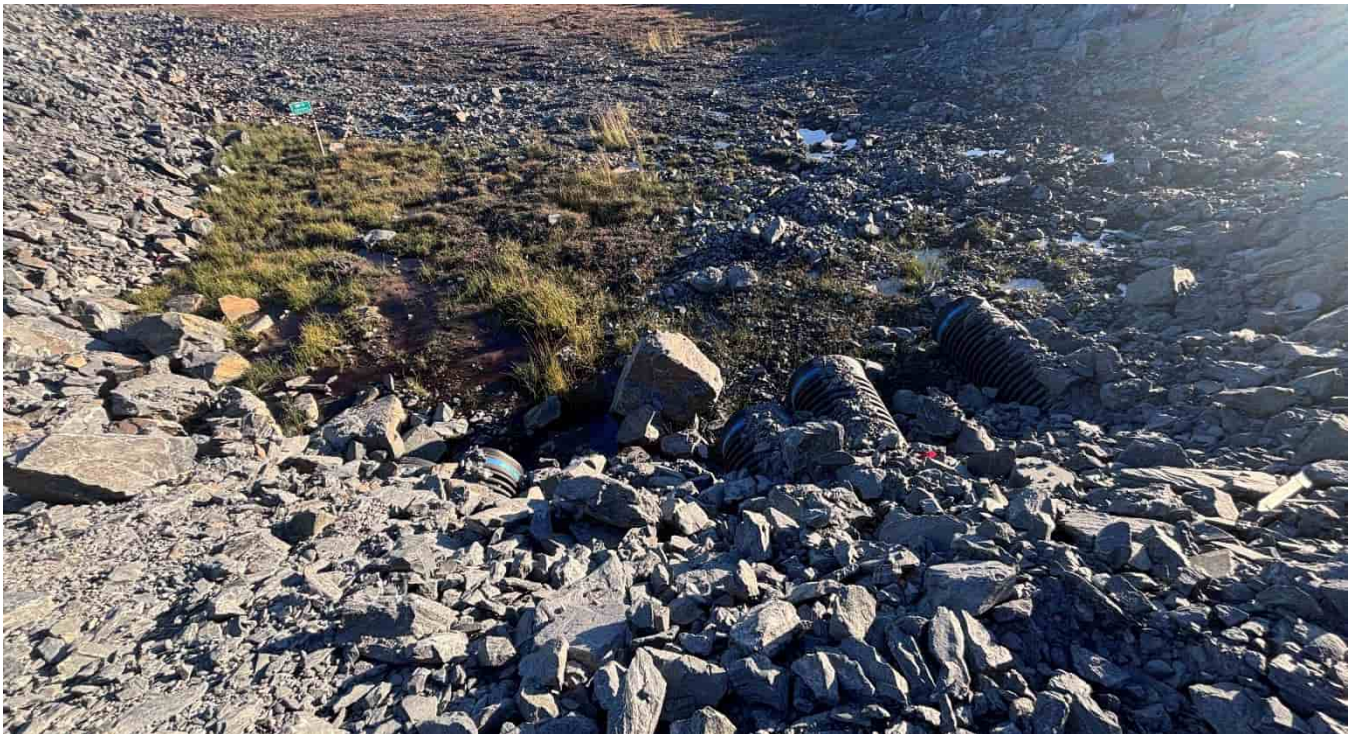
G-95: Upstream (S) end of western culverts
