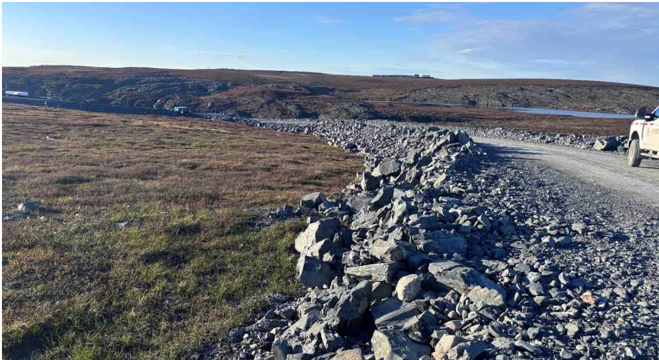
G-98: W rockfill of barge area access road, looking NW
