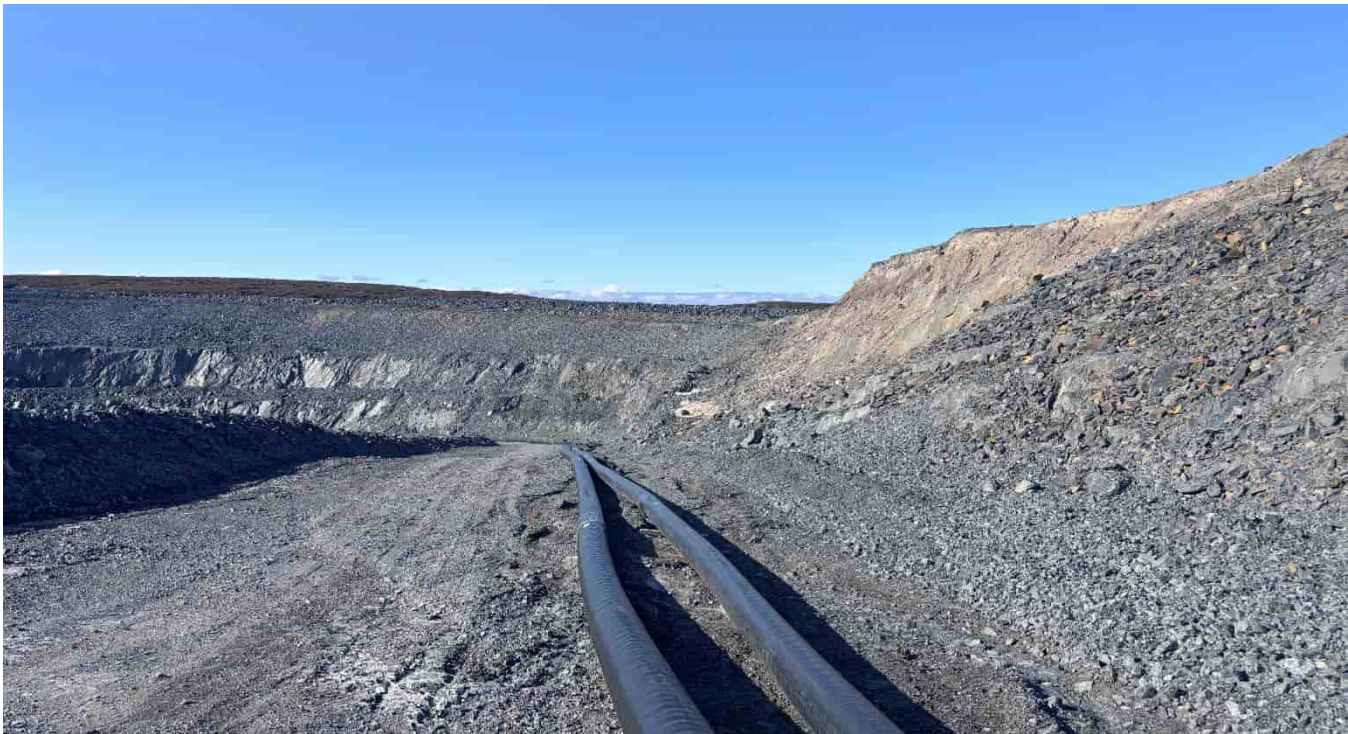
G-114: Tailings pipeline at entrance to Echo TF
