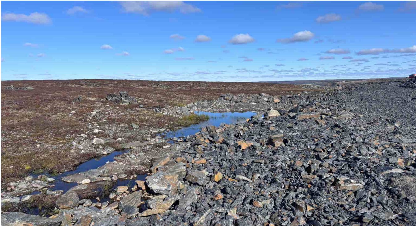
G-143: Ponding water beside diversion, looking N – undefined edge of diversion slope
