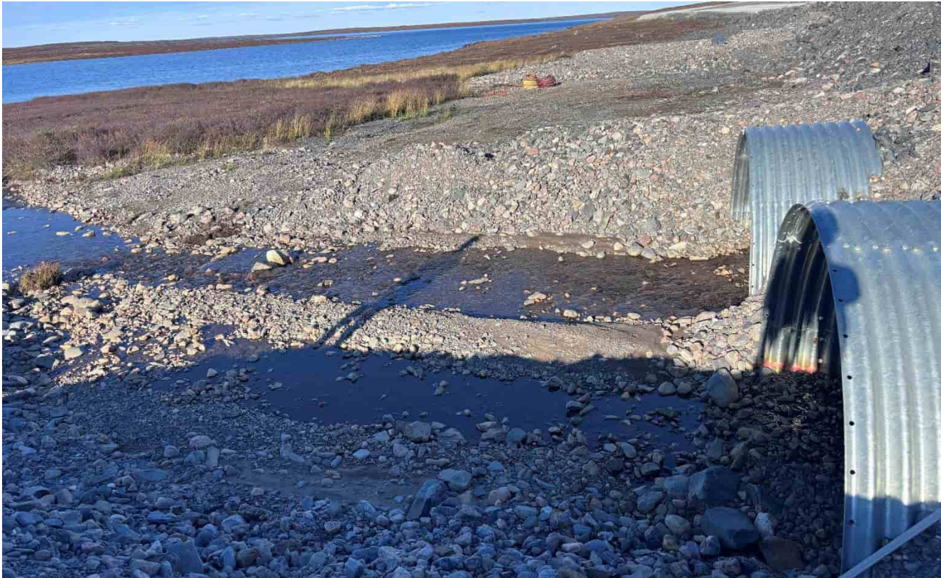
G-26: Downstream (N) side of twin culverts, looking E
