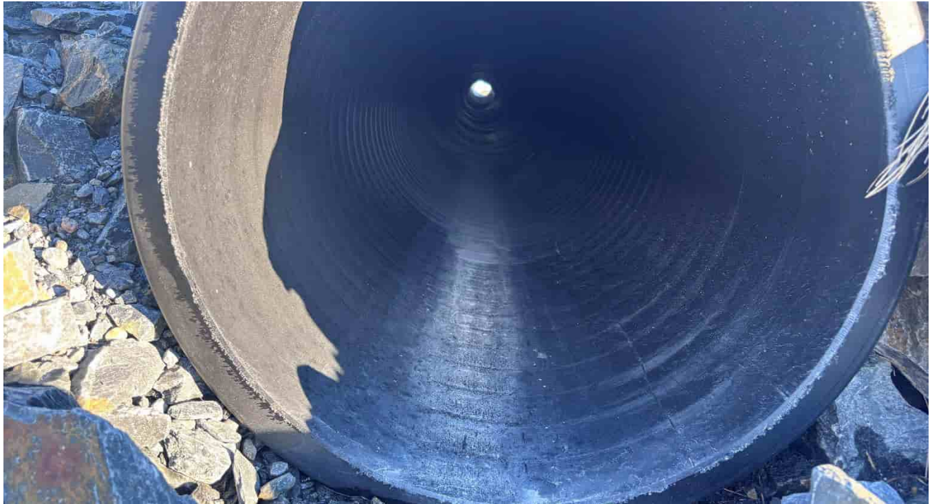
G-92: Downstream (N) end of dry culvert
