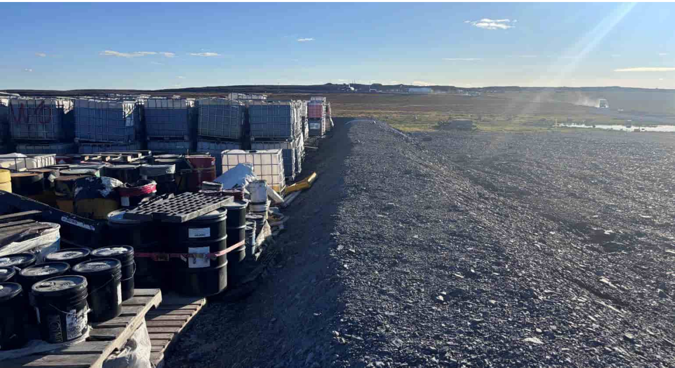
G-12: Exploration camp tote storage and berm
