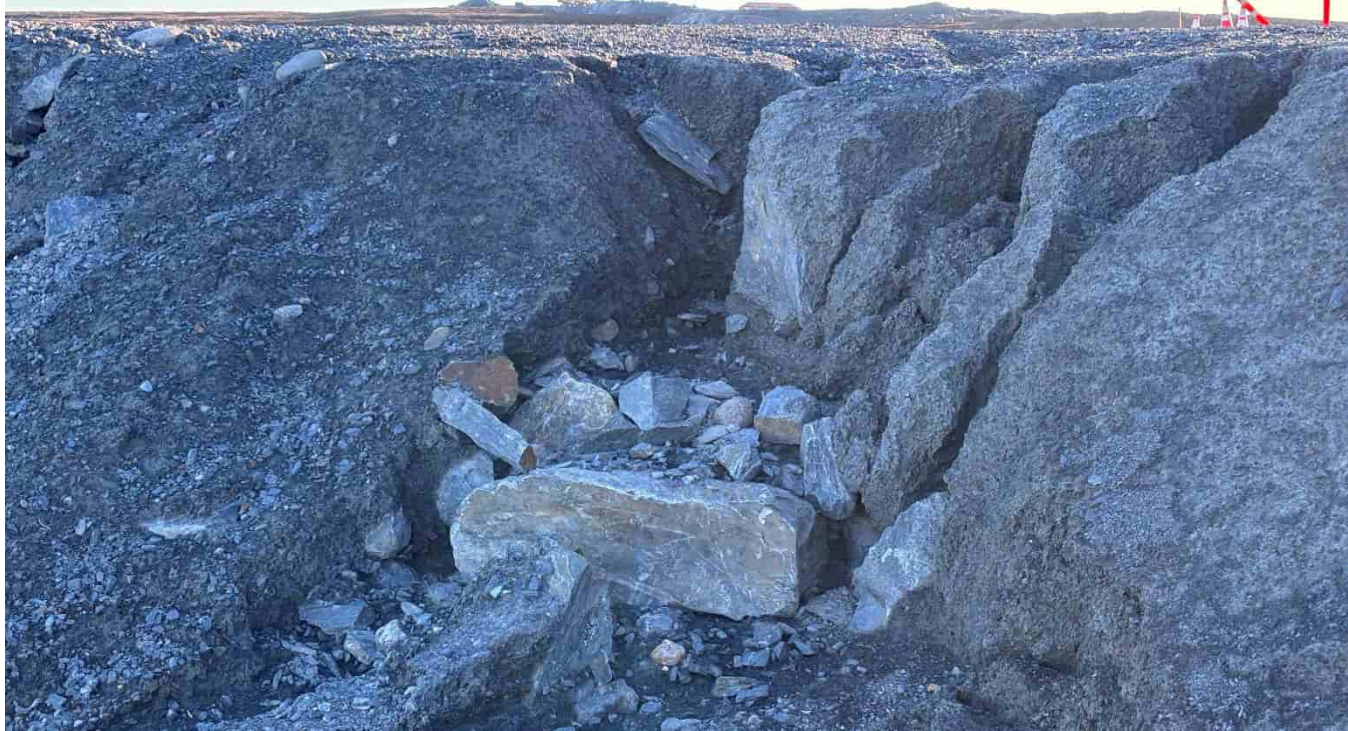
G-71: Erosion pathway on NE apron
