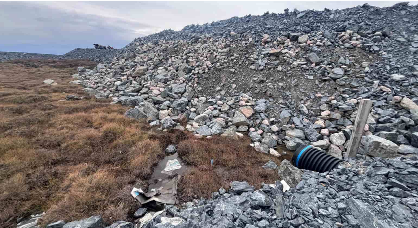
G-205: Road rockfill – culvert inlet behind pad (outlet in pad rockfill)
