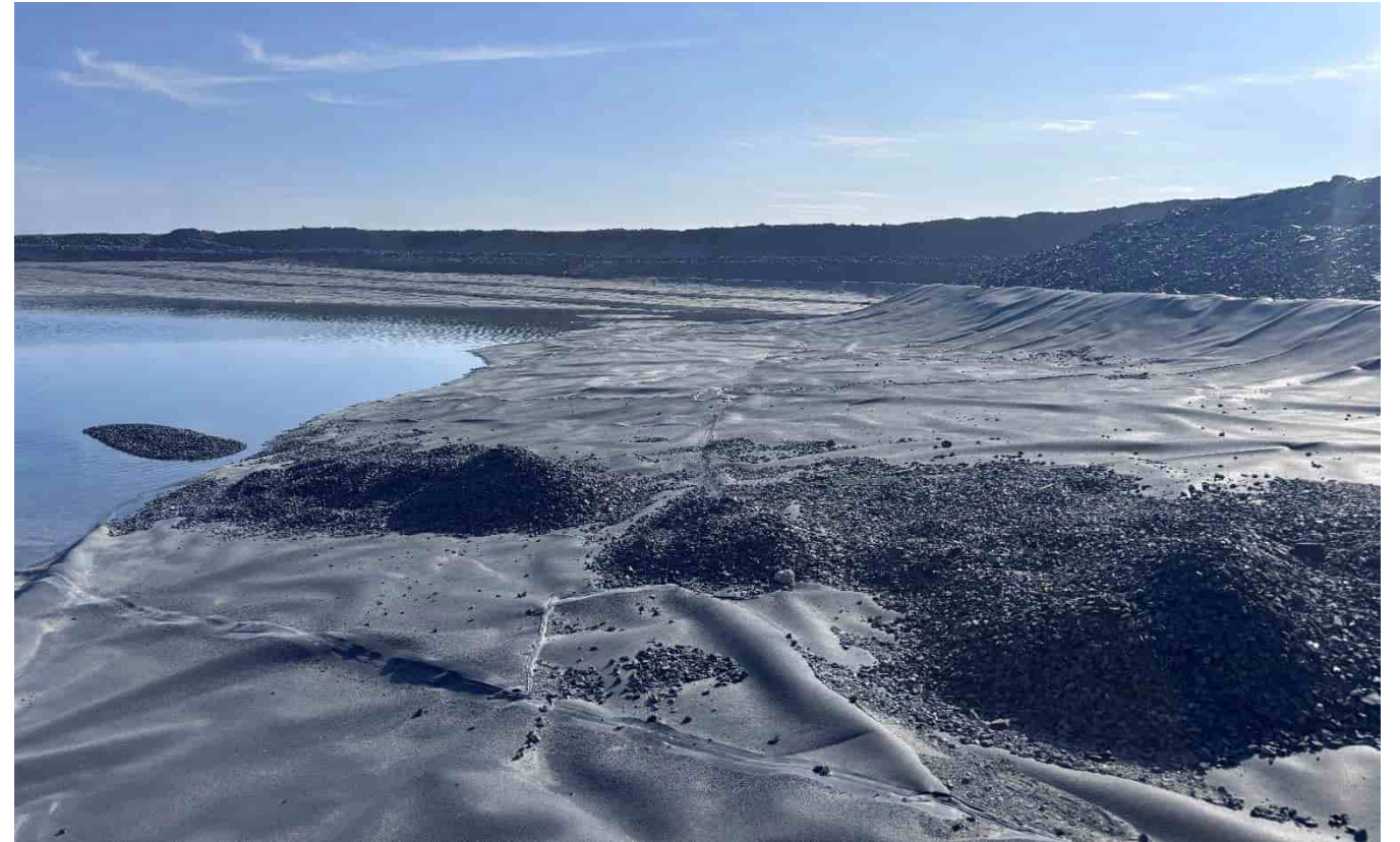
G-237: Rock material directly on liner, looking SE
