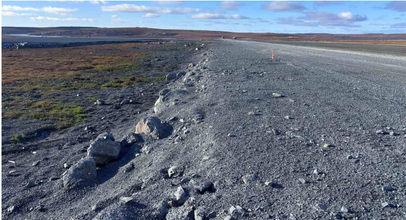
G-51: SW runway rockfill, looking NW
