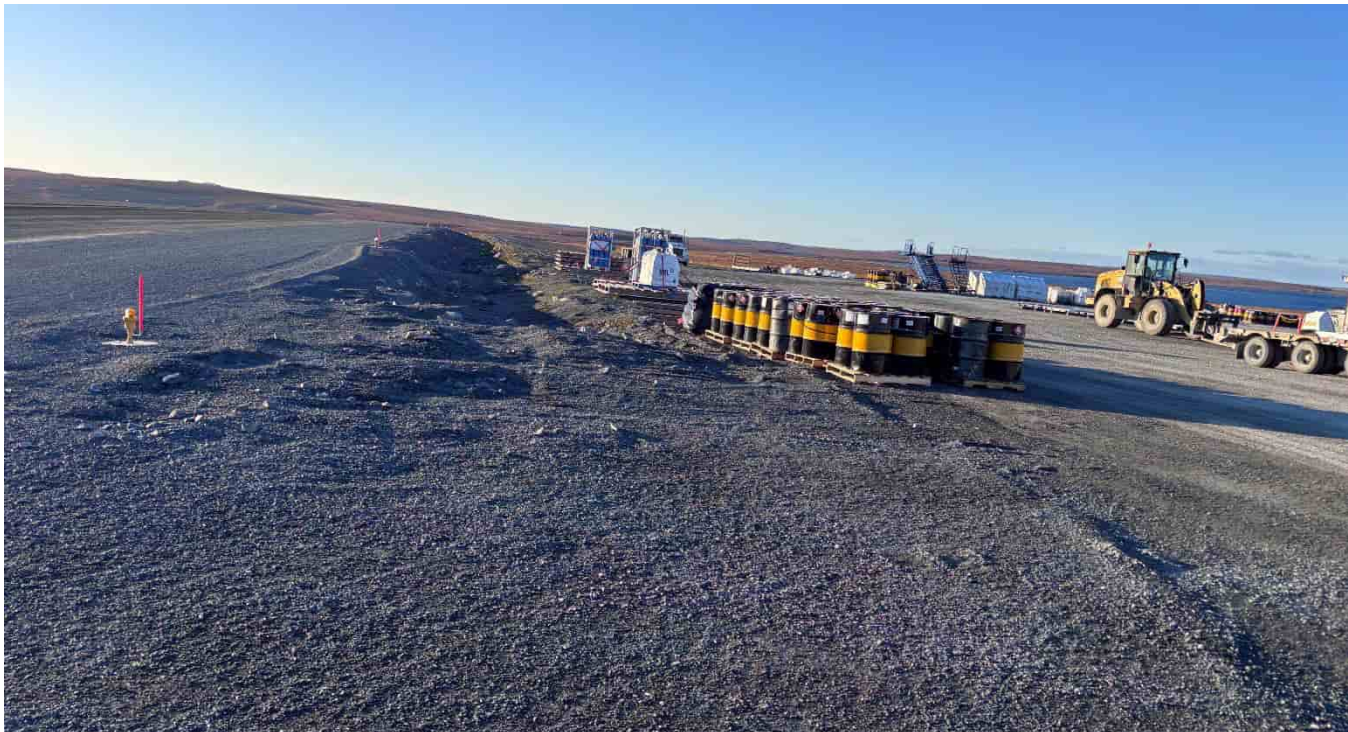
G-73: Airstrip laydown area and runway, looking NW
