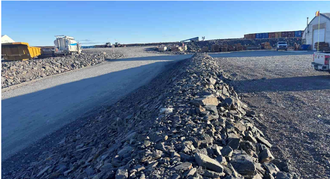
G-184: Parking pad slope above operations area access road, looking S
