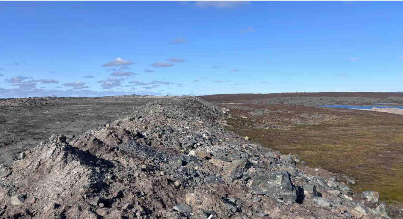
G-127: Echo overburden stockpile – eastern slope, looking N
