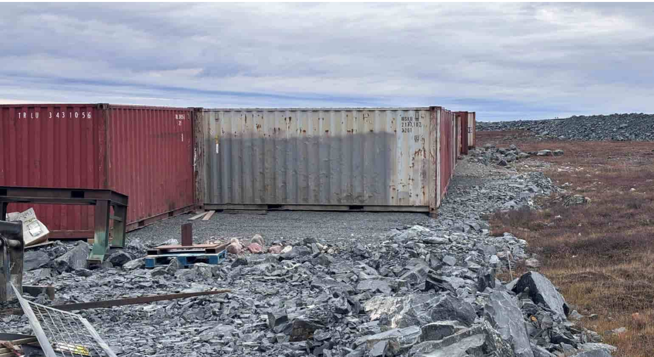
G-207: Maintenance warehouse laydown – pad daylighting into tundra / slope
