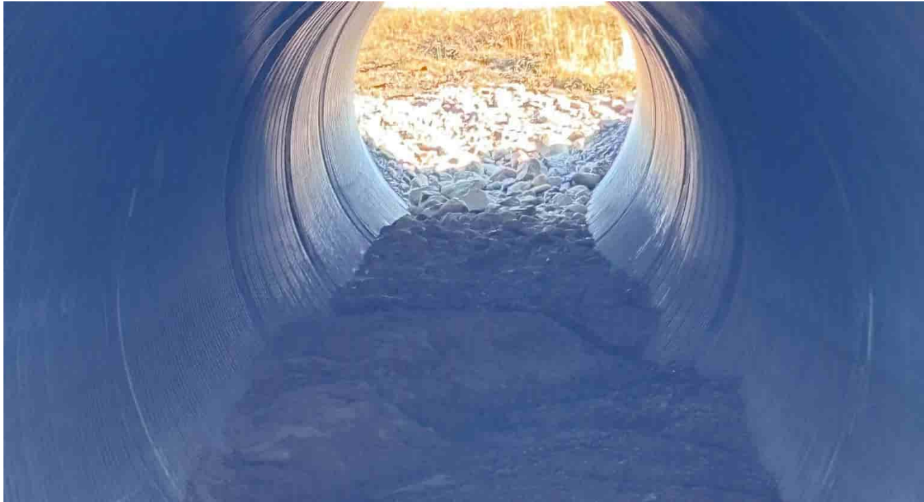
G-28: Interior of eastern culvert, looking upstream
