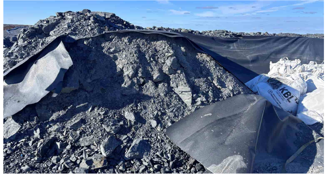
G-161: Inconsistent liner and damage to northernmost pond - low potential containment volume in area
