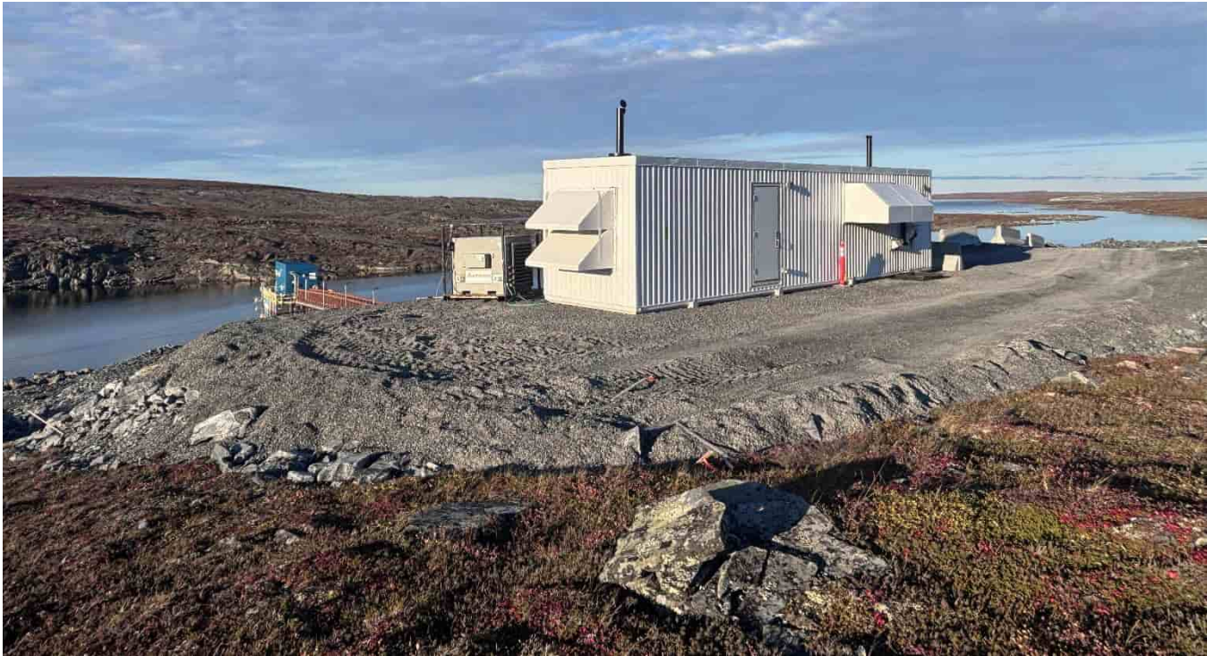
G-179: Highest pad above barge access road – pad approximately daylighting into slope
