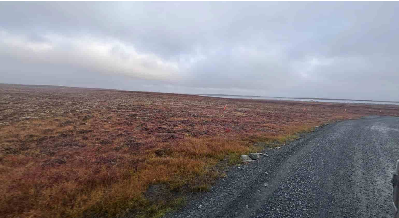
G-24: Tundra N of airstrip access road – Note thickness of road rockfill
