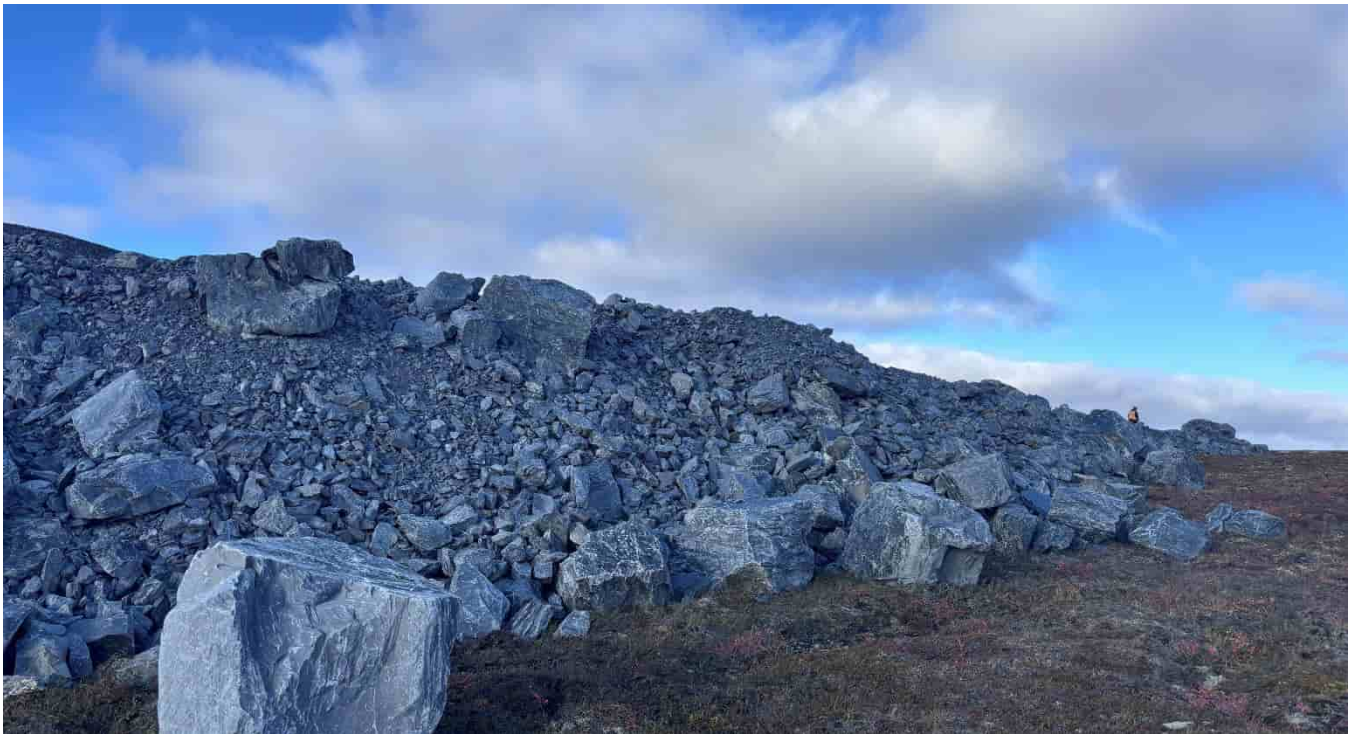
G-38: SW apron, looking NE
