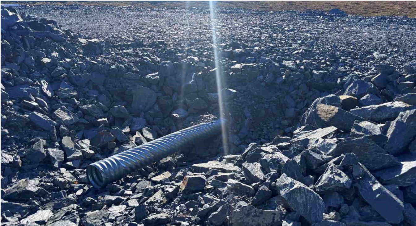
G-157: Culvert underneath pad
