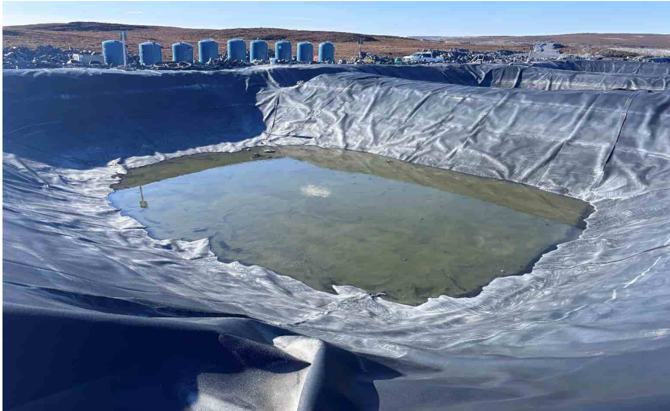
G-150: Treatment pond cell
