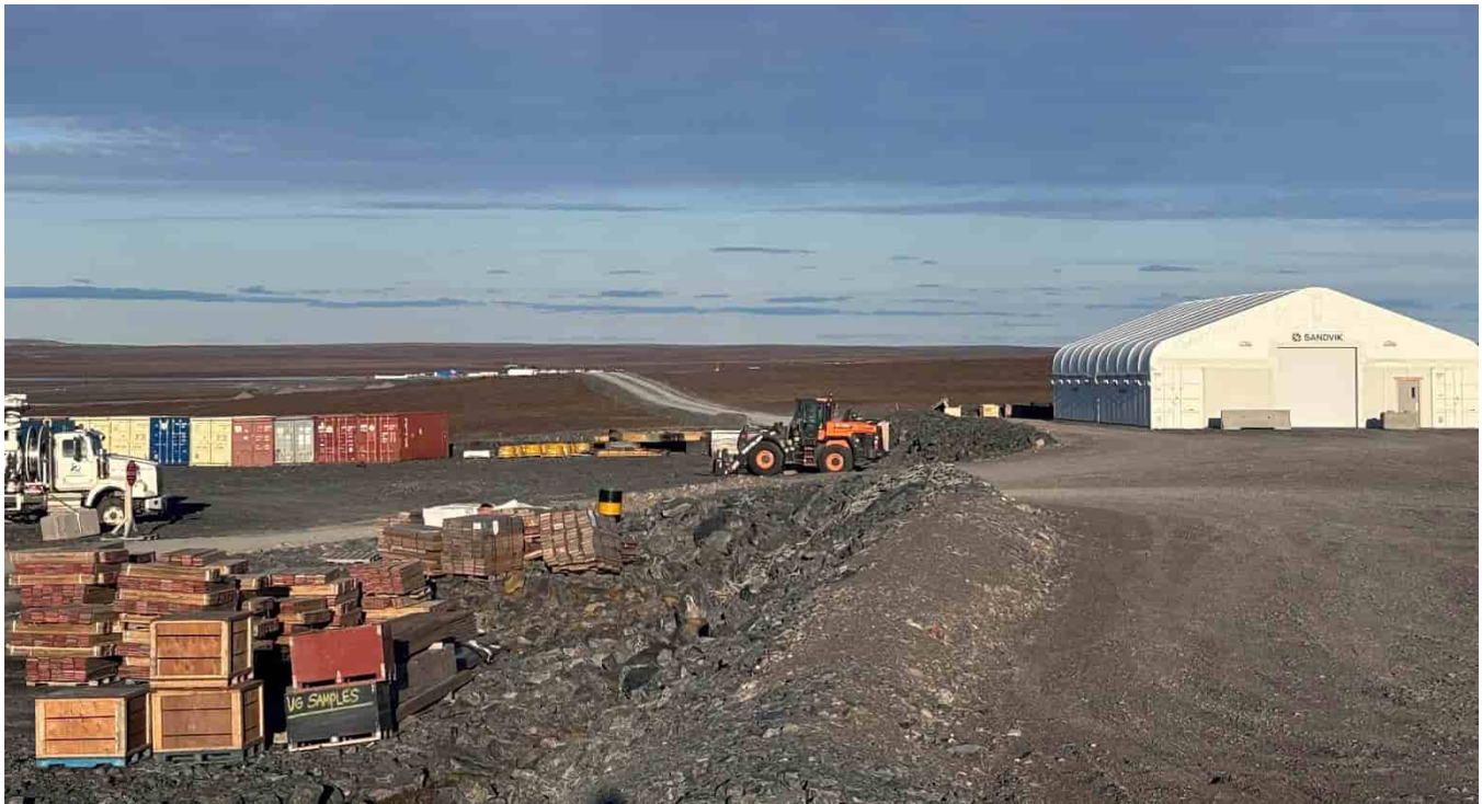
G-190: Laydown area and Sandvik, looking E
