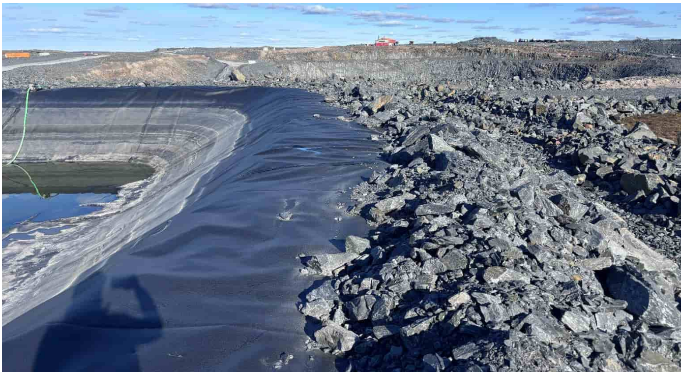
G-154: Coarse over-liner material
