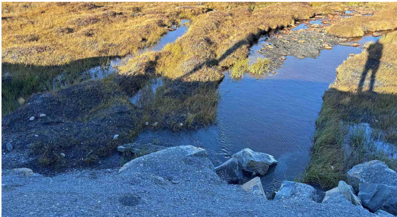
G-61: Culvert under SE end of runway
