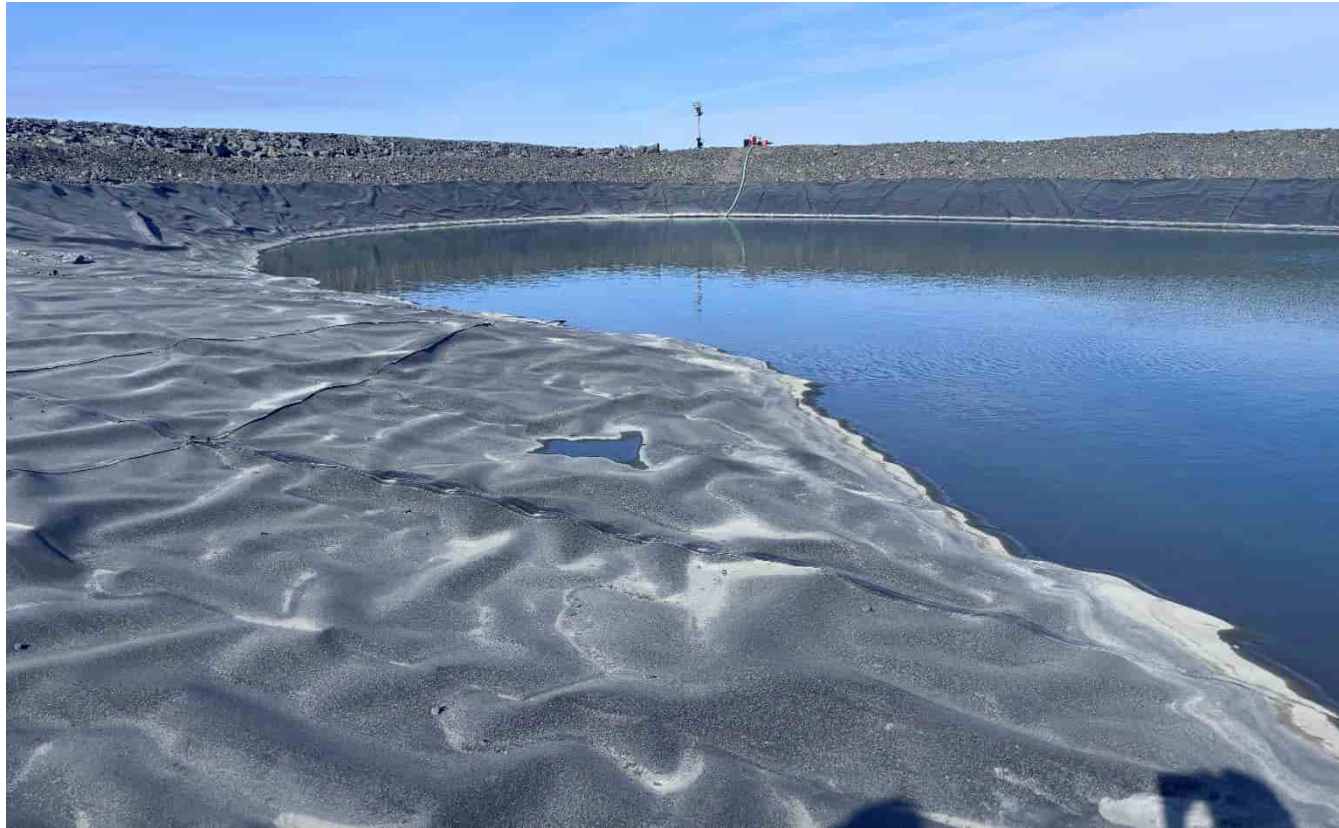
G-236: Edge of main Camp Pad pond at the time of the inspection, looking NW
