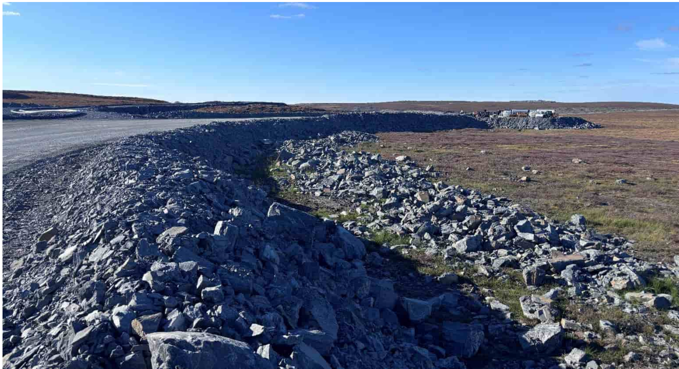
G-166: Road beside water treatment plant, looking NW
