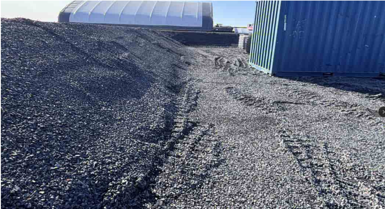
G-213: Tote Storage Facility: Toe of the eastern berm, looking E
