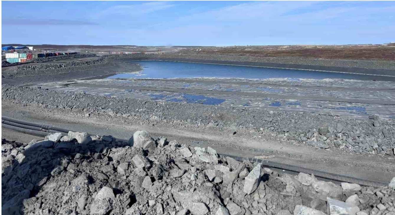
G-229: Contact water pond, looking NW
