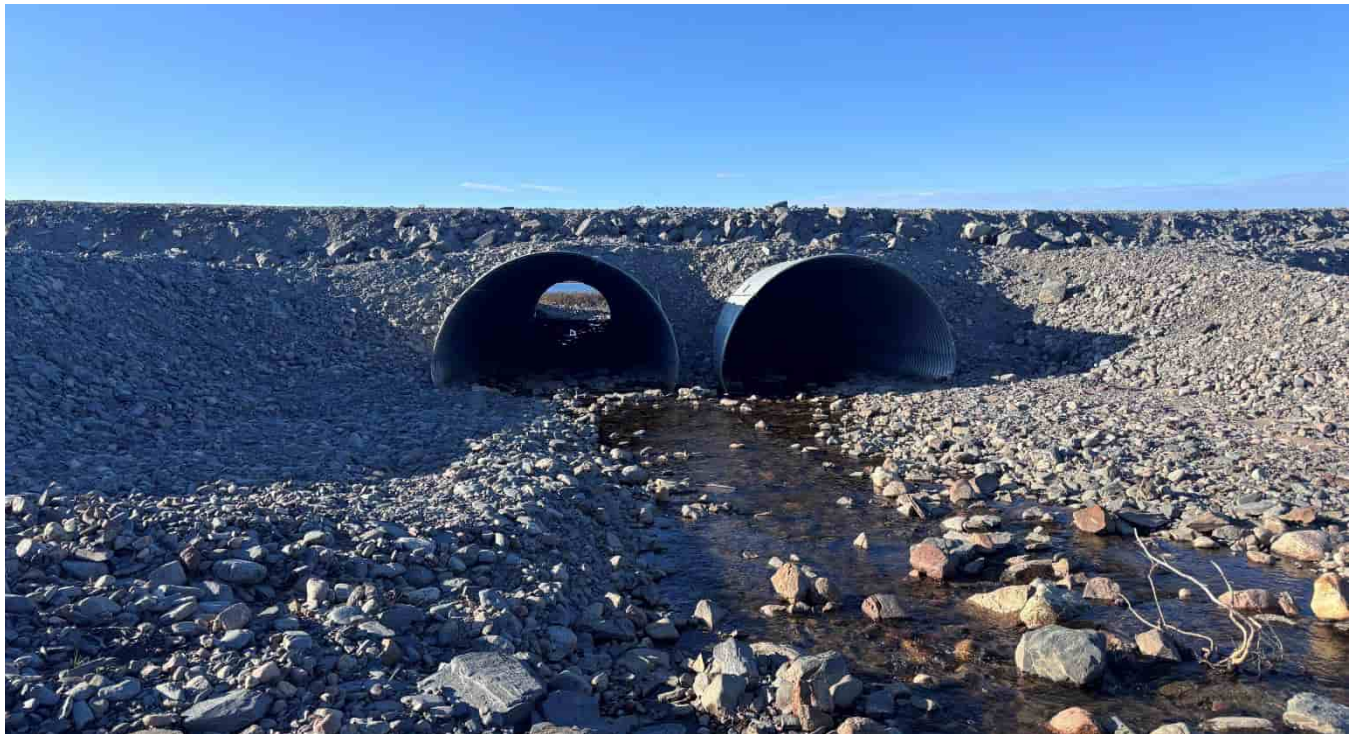
G-30: Upstream (S) side of twin culverts
