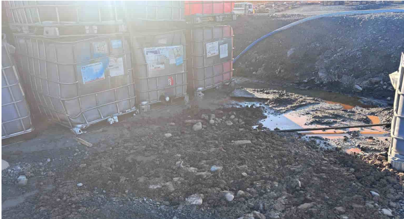
G-13: Tote storage area and berm
