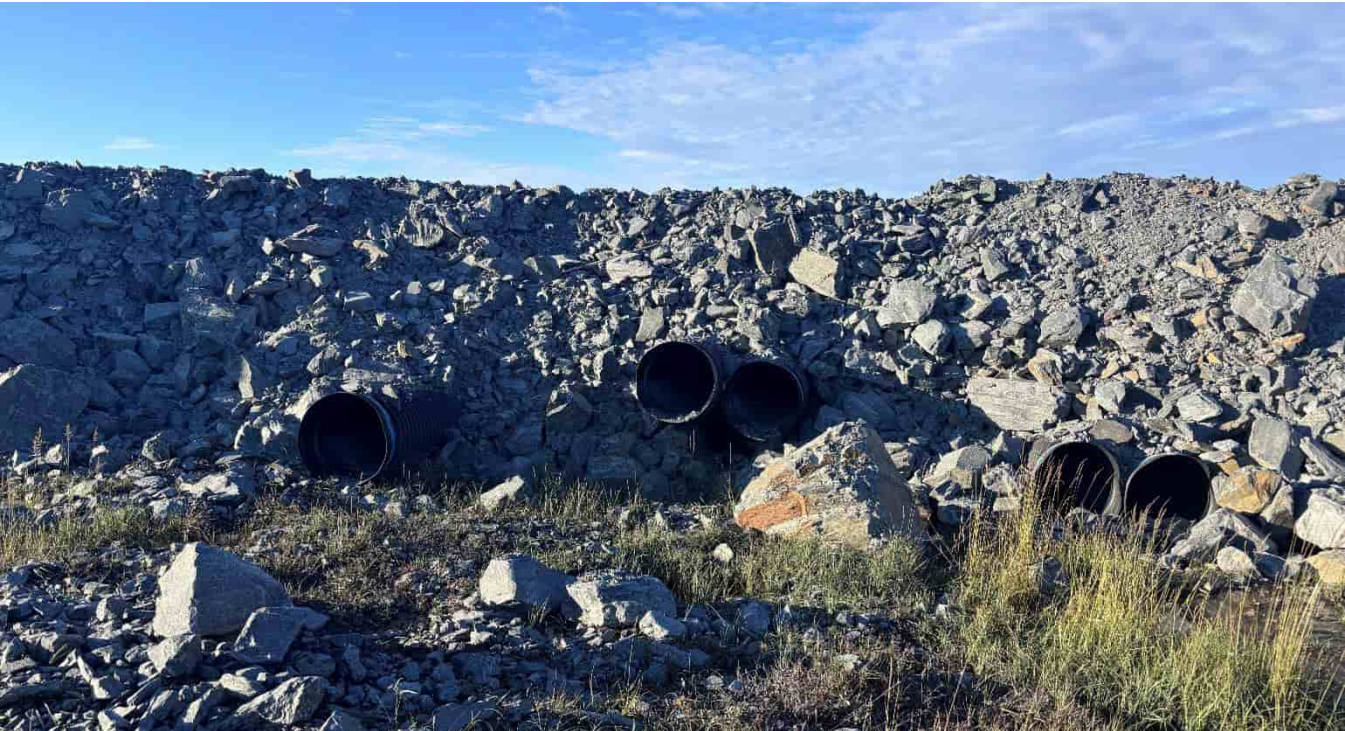
G-97: Upstream (S) side of western culverts – Two culverts raised approximately 0.5m from the toe rockfill
