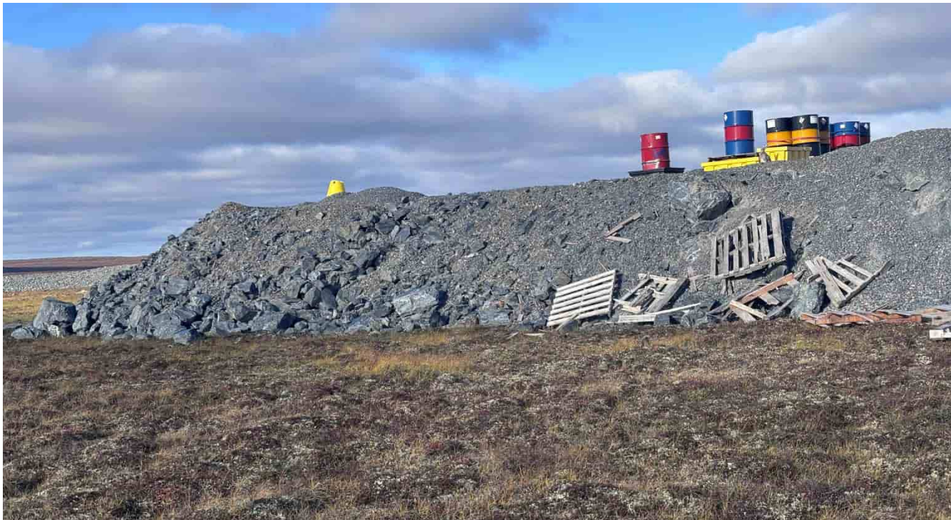
G-34: SW apron at W corner
