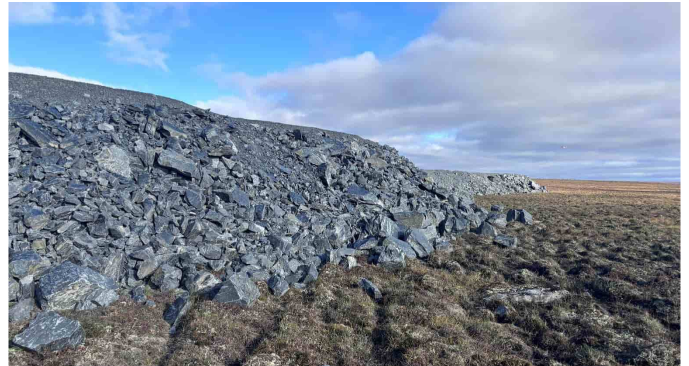
G-35: Slope face of SW apron
