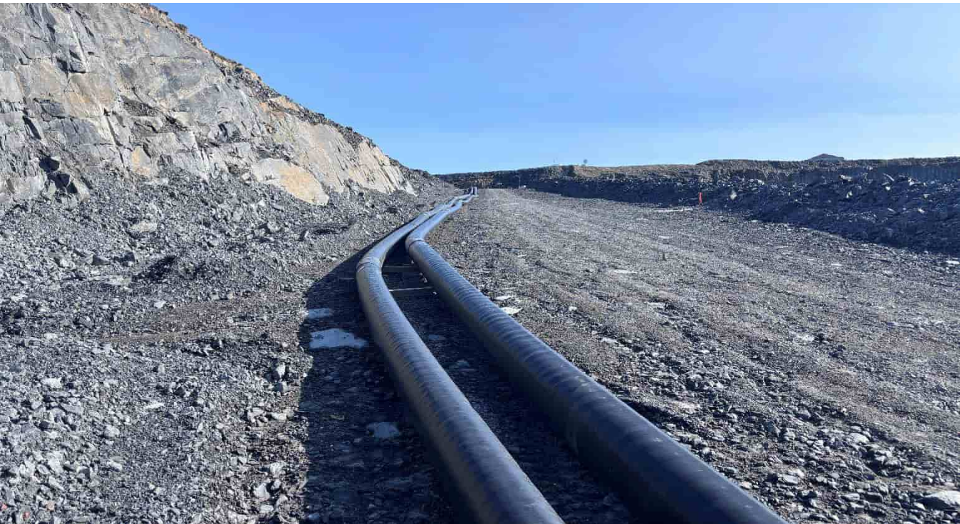
G-118: tailings pipeline, looking E
