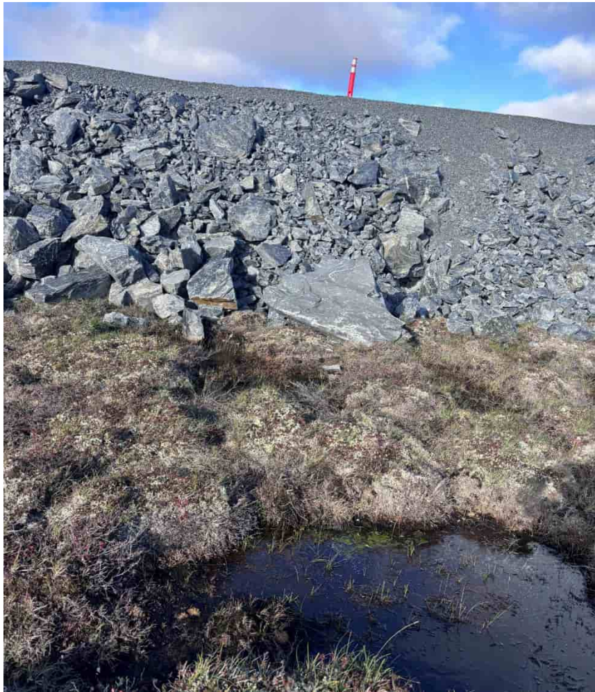
G-36: Below SW apron toe, looking NE
