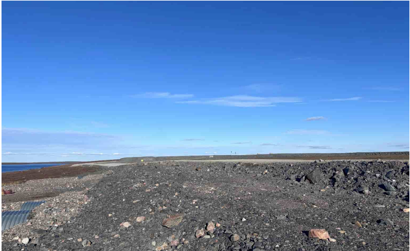
G-25: North side of road rockfill above twin culverts, looking E
