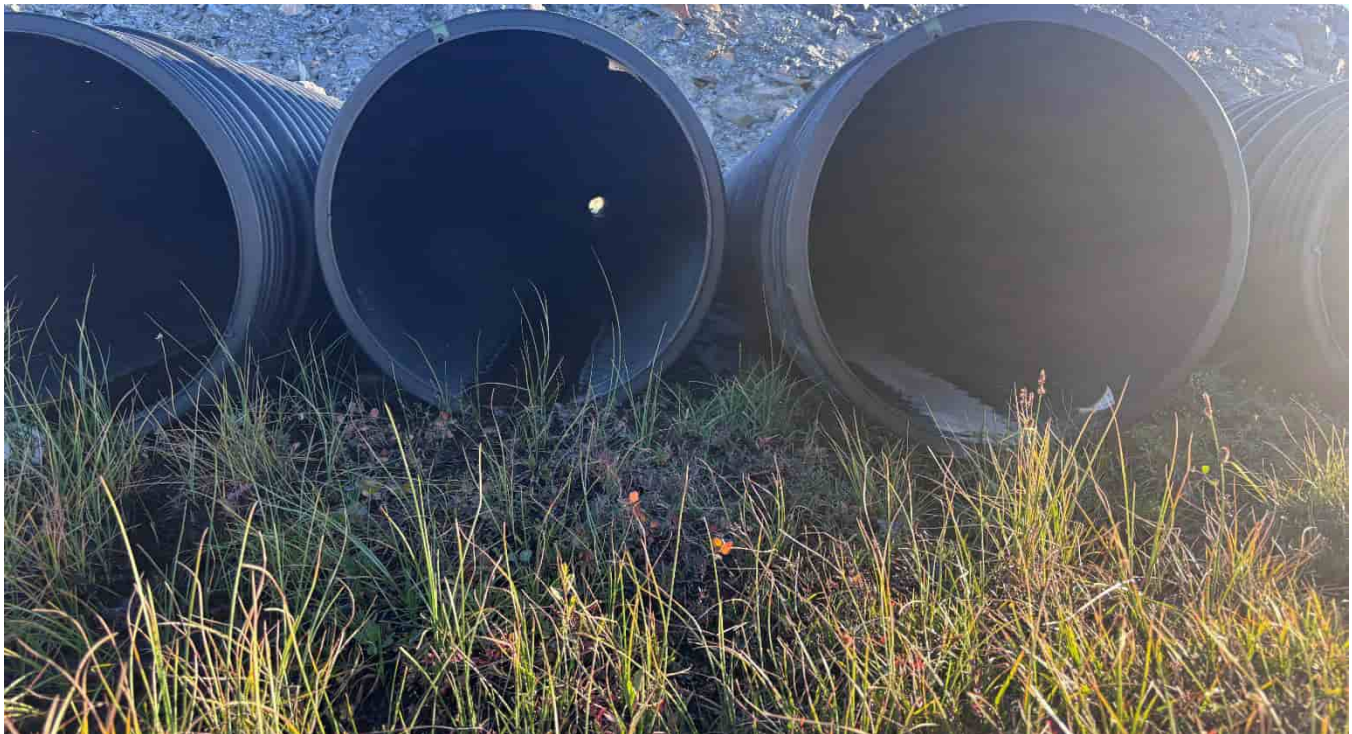
G-90B: Downstream (N) end of western culverts
