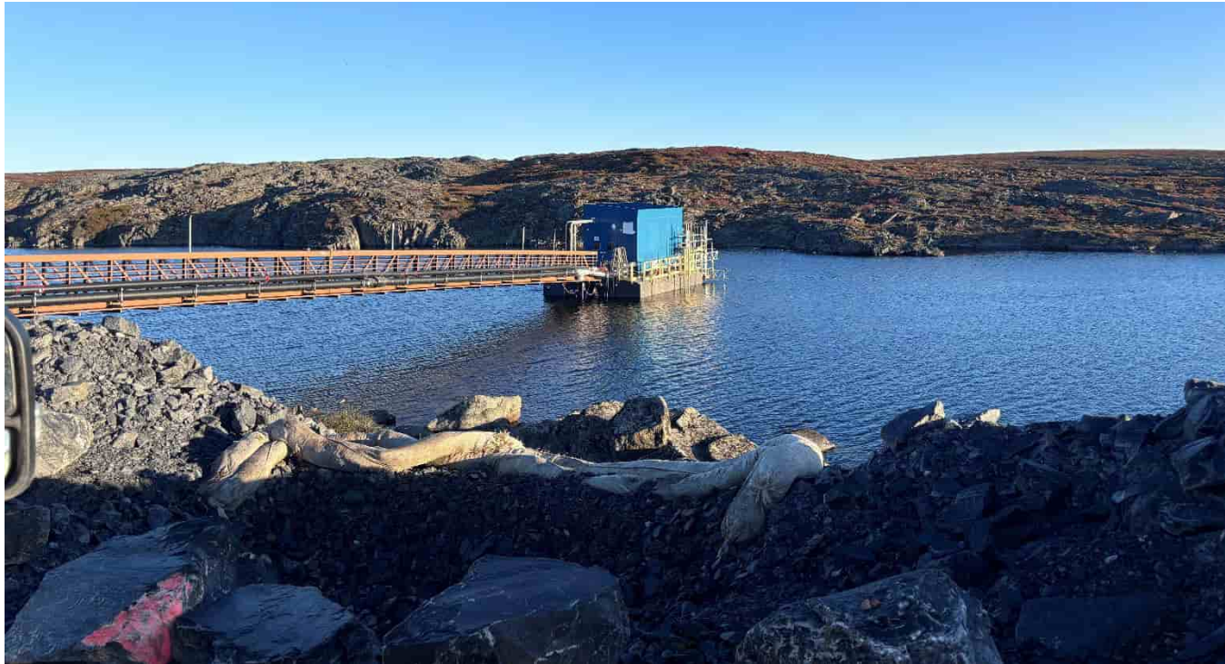
G-174: Barge access dock, facing NW
