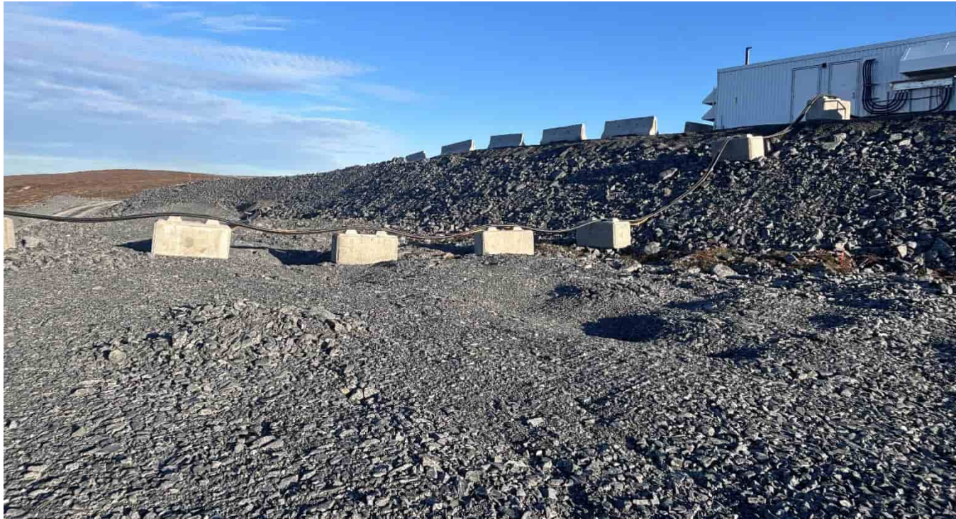
G-178: Middle pad above barge access road, looking SE
