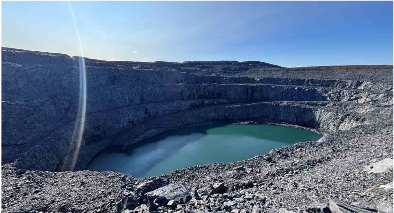
G-115: Overall view of Echo TF
