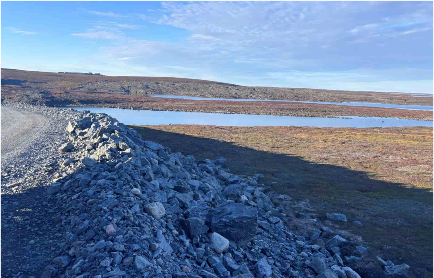
G-100: E rockfill of access road to Goose barge area, looking N
