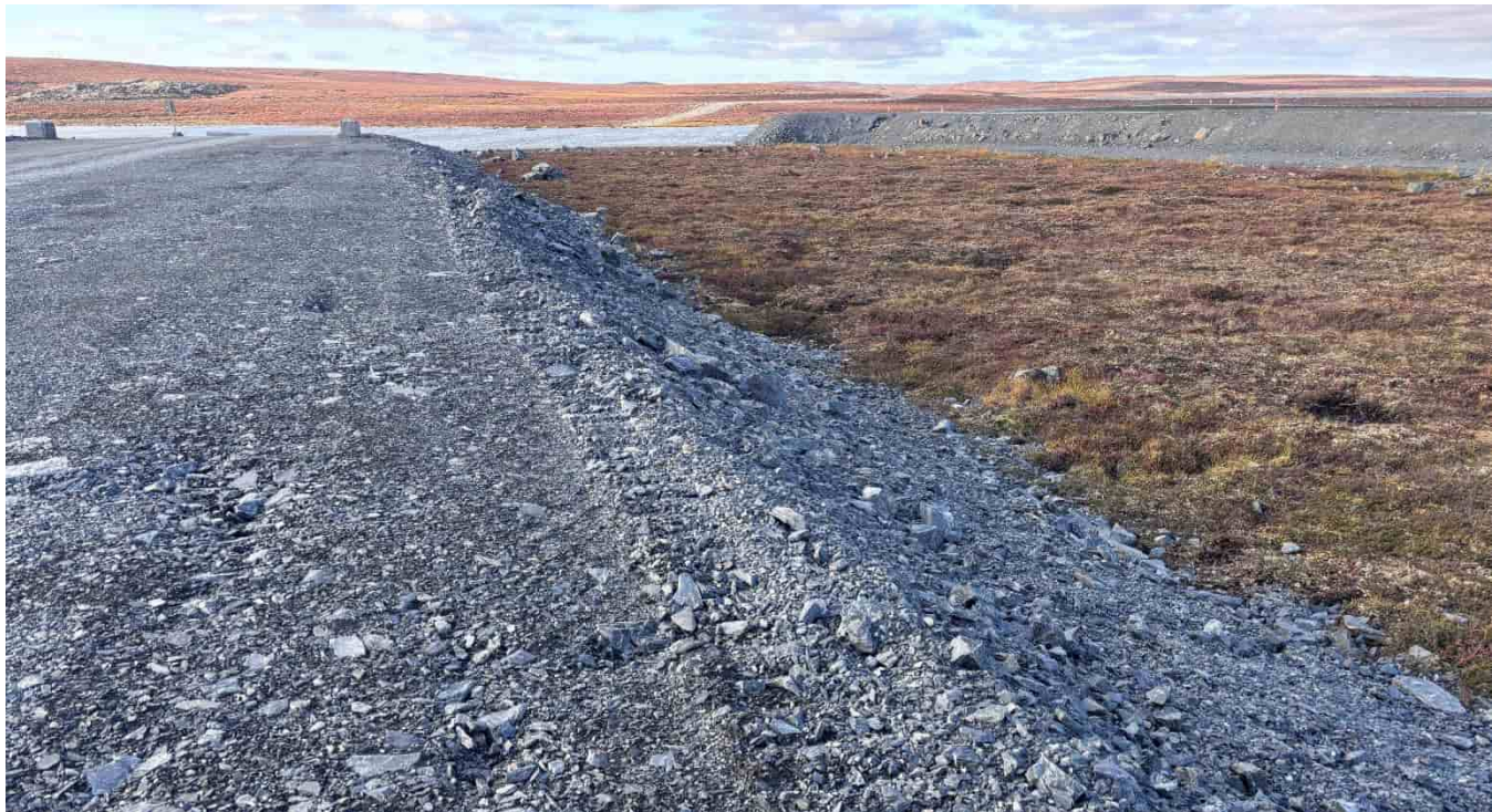
G-45: Airstrip runway access road rockfill, looking NW
