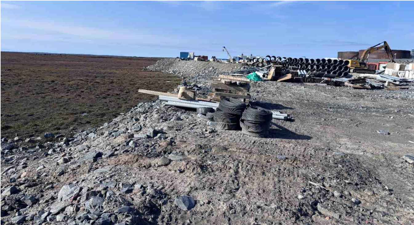
G-220: Edge of ROM area, looking W towards main plant
