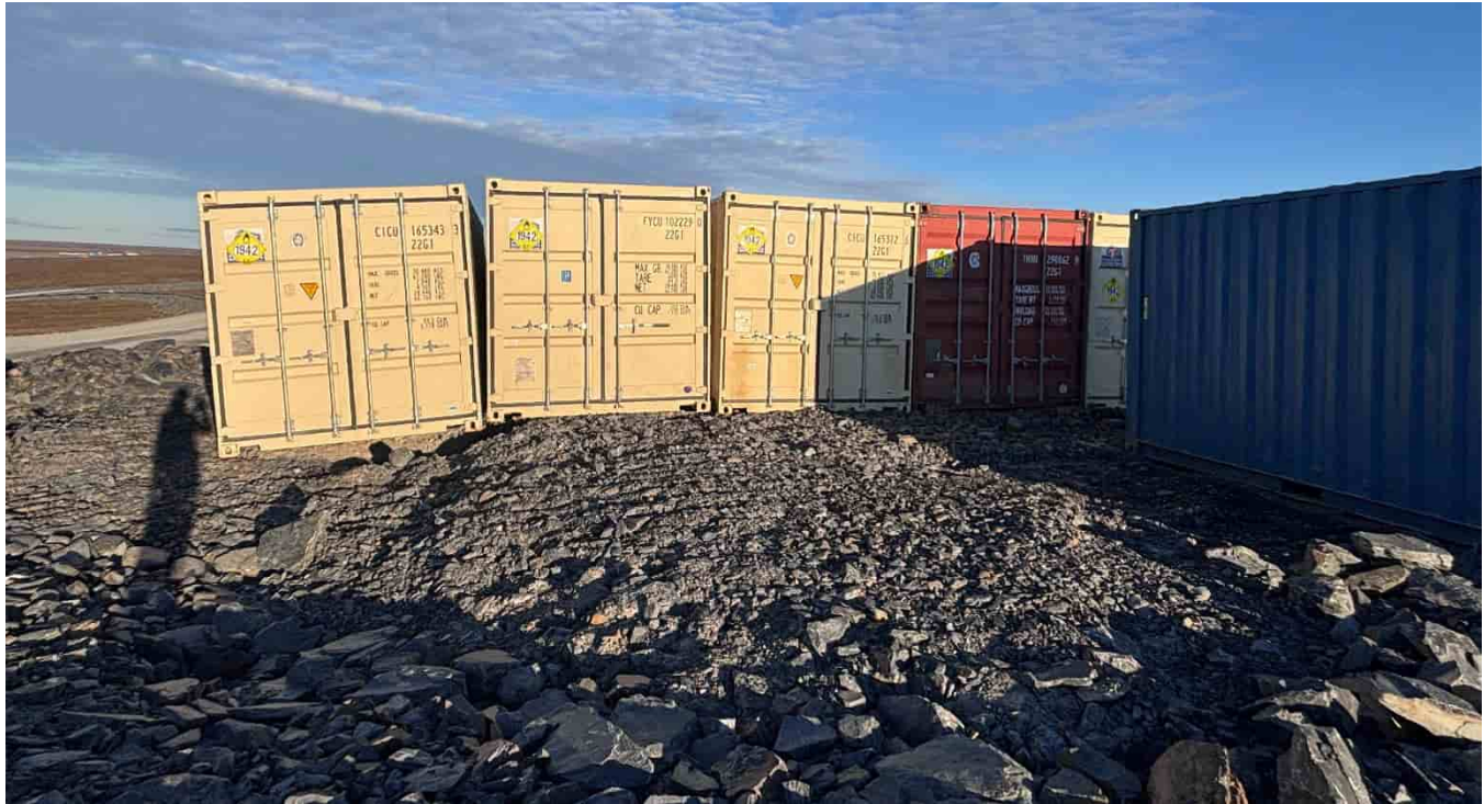
G-200: Differential settlement of seacan, looking E
