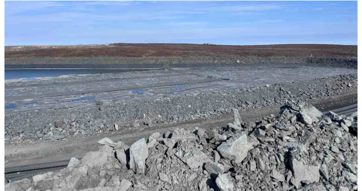
G-230: Contact water pond, looking NE
