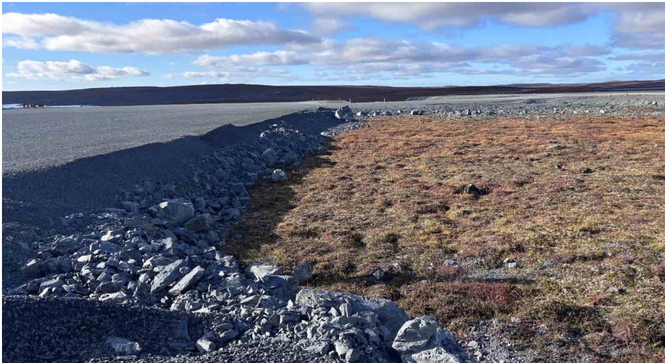
G-41: Airstrip rockfill, looking NW
