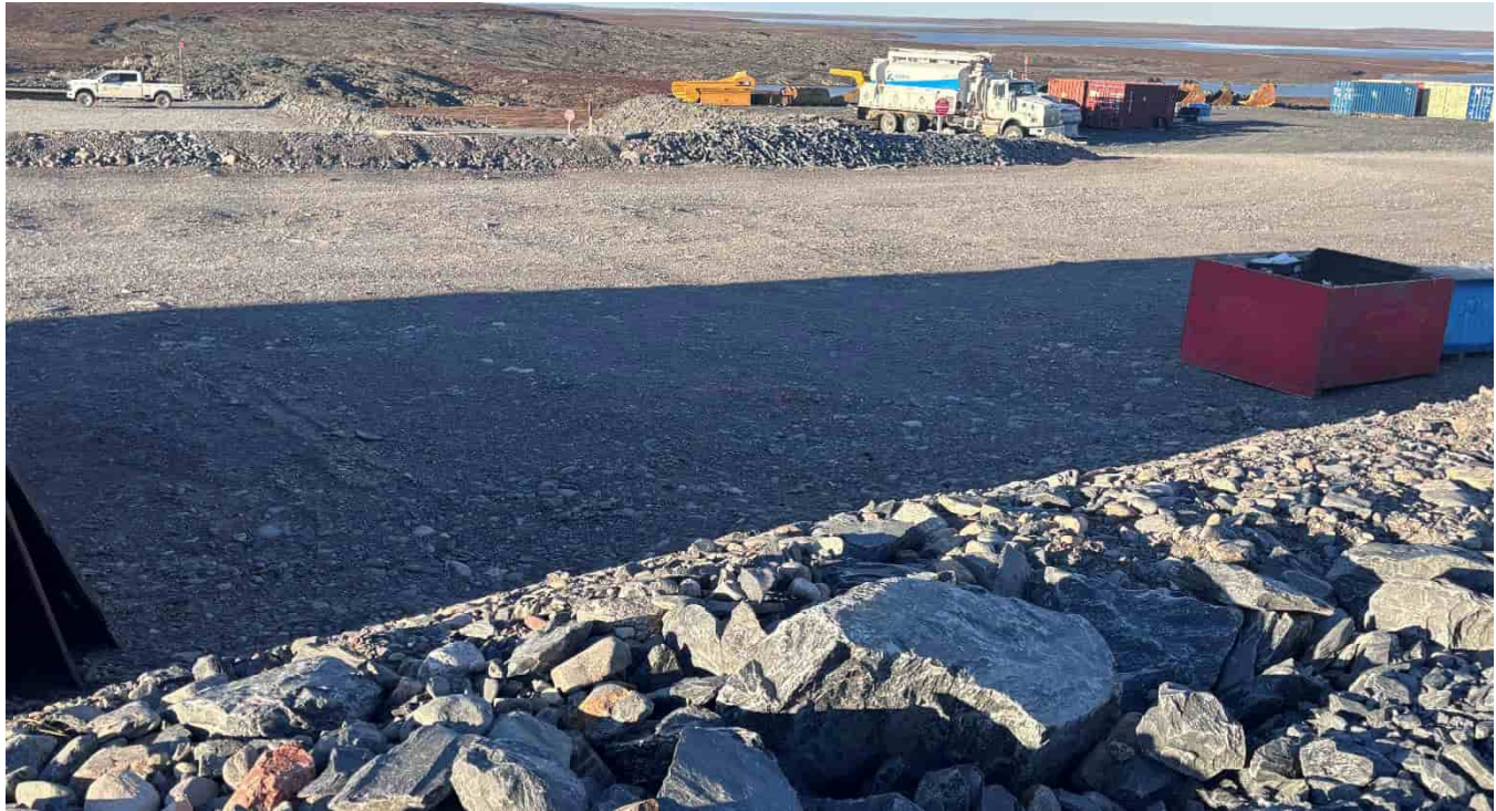
G-192: Tailings pipeline road rockfill above laydown, looking N
