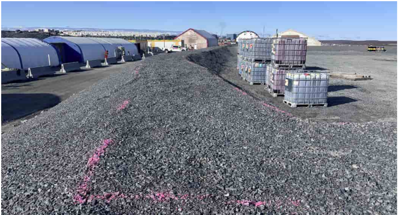
G-210: Tote Storage Facility: Crest of the southern berm, looking NW
