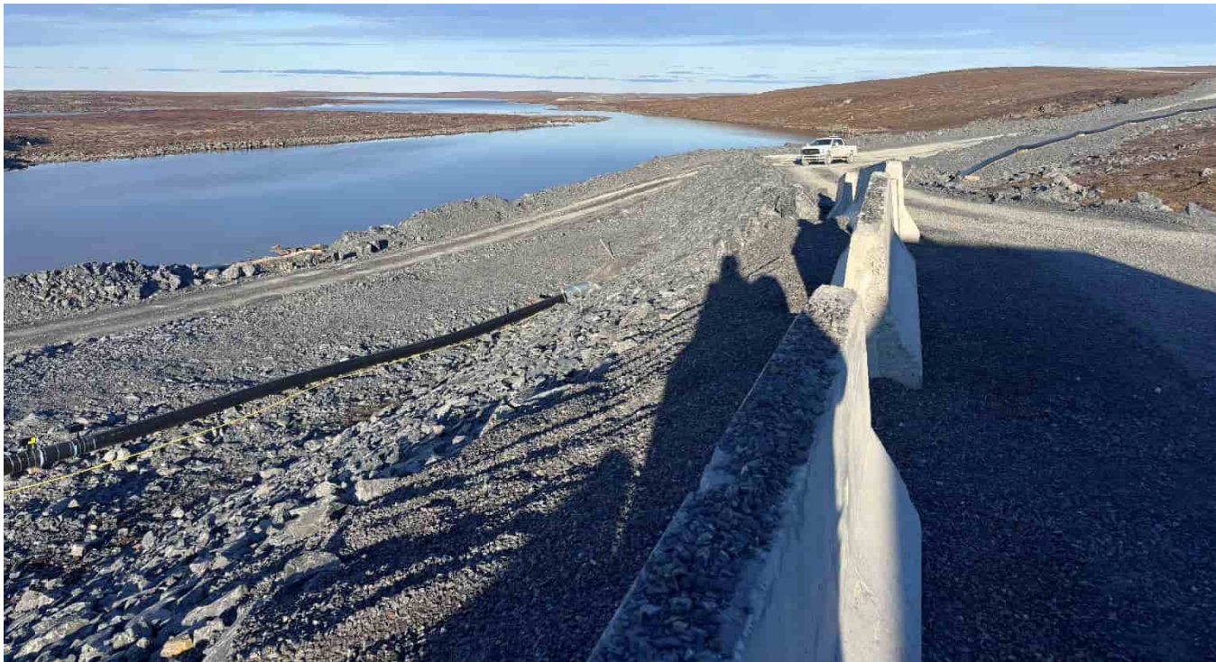
G-180: Access road to highest pad and trailer
