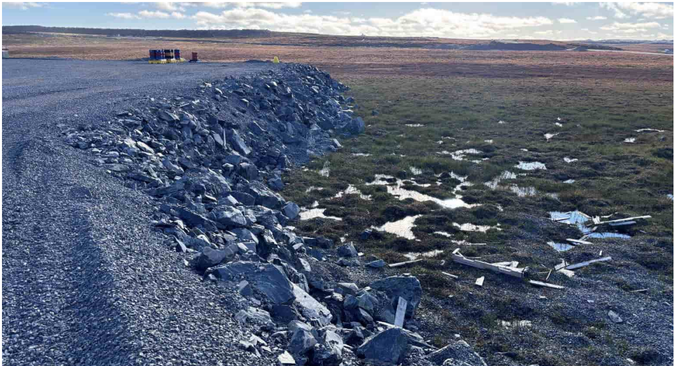
G-49: SW apron, looking SW.
