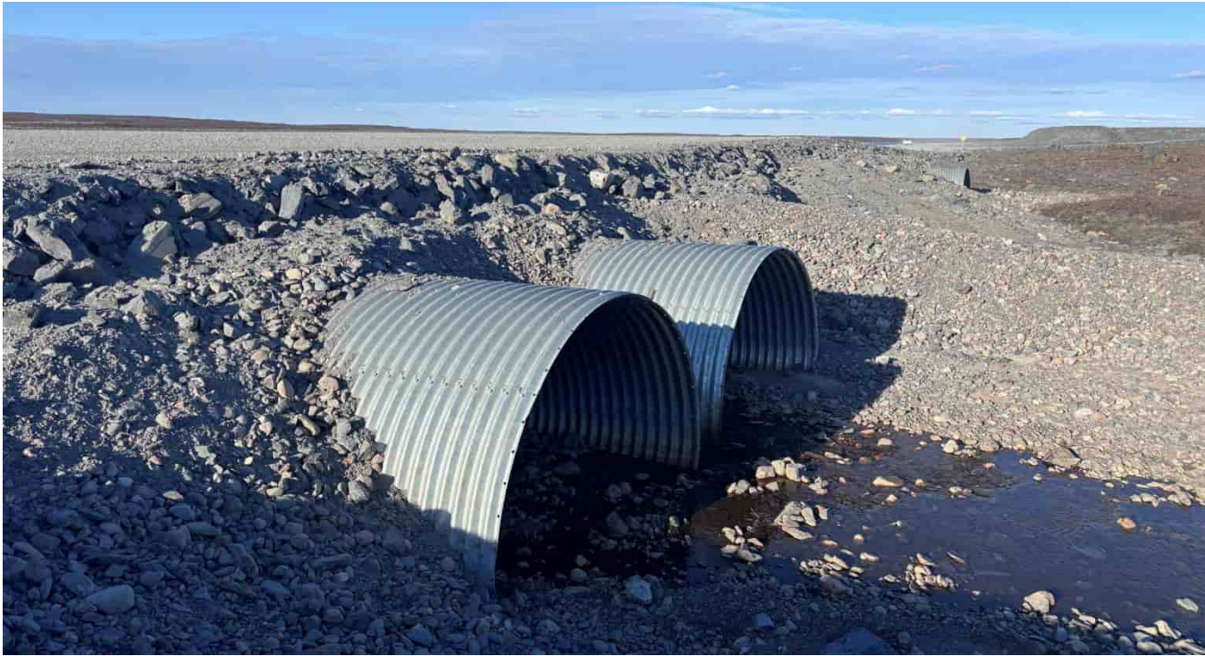
G-31: Upstream (S) side of twin culverts, looking NE
