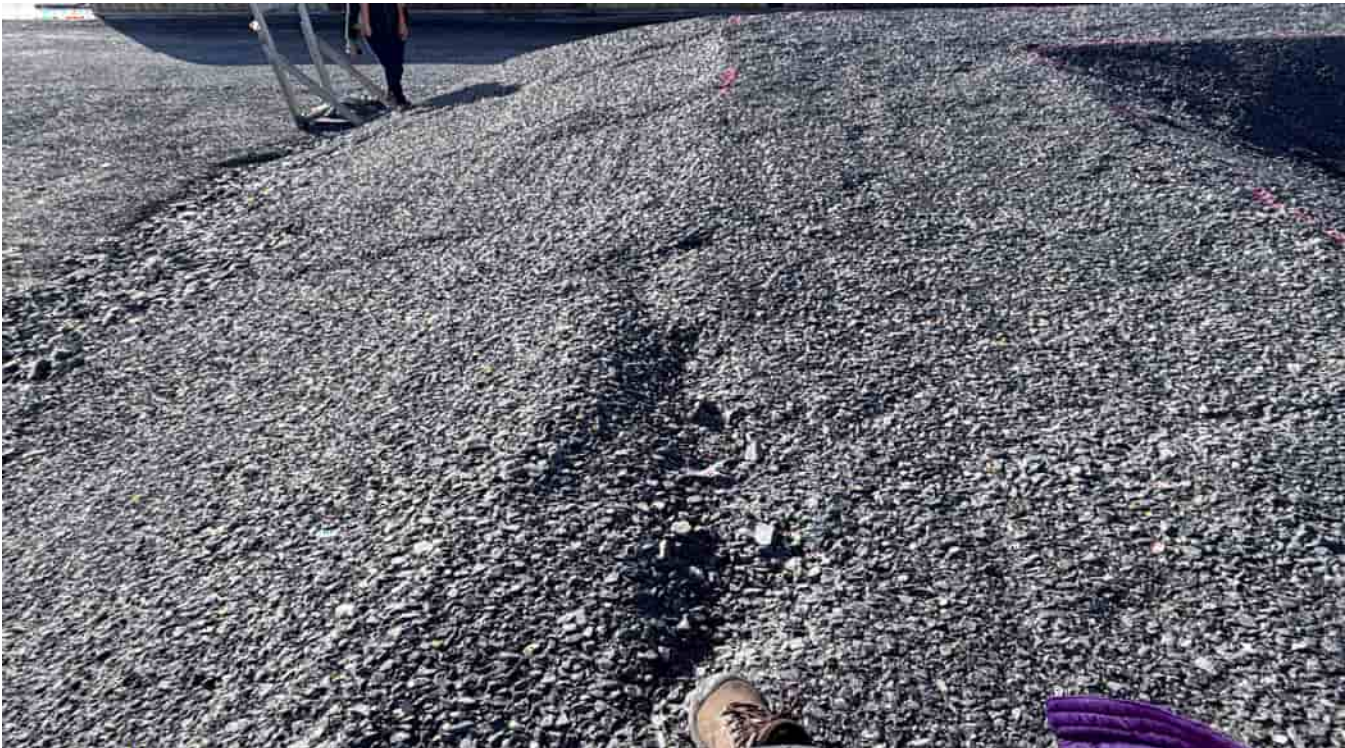
G-211: Tote Storage Facility: SE corner
