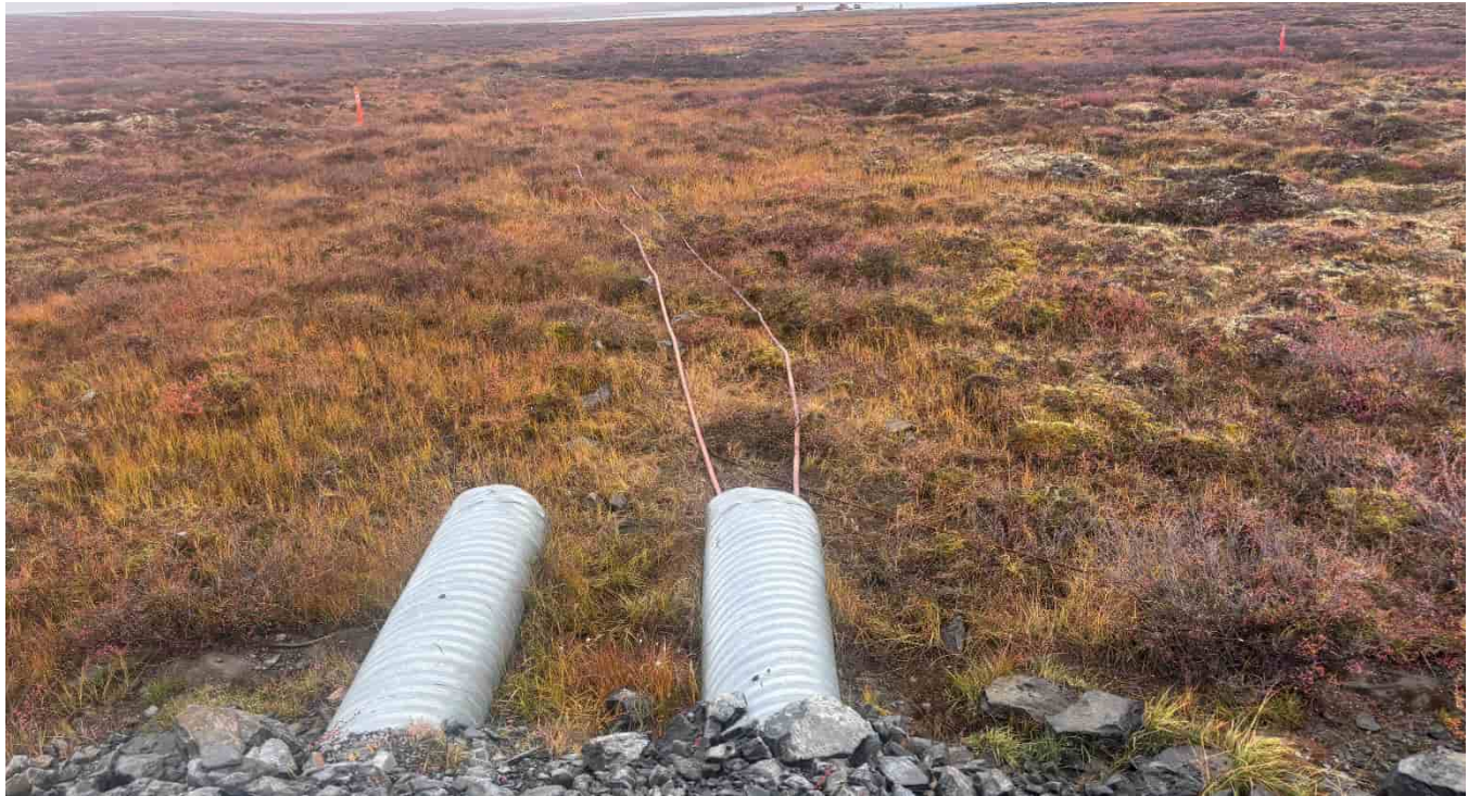
G-21: Culverts under the airstrip access road, looking N
