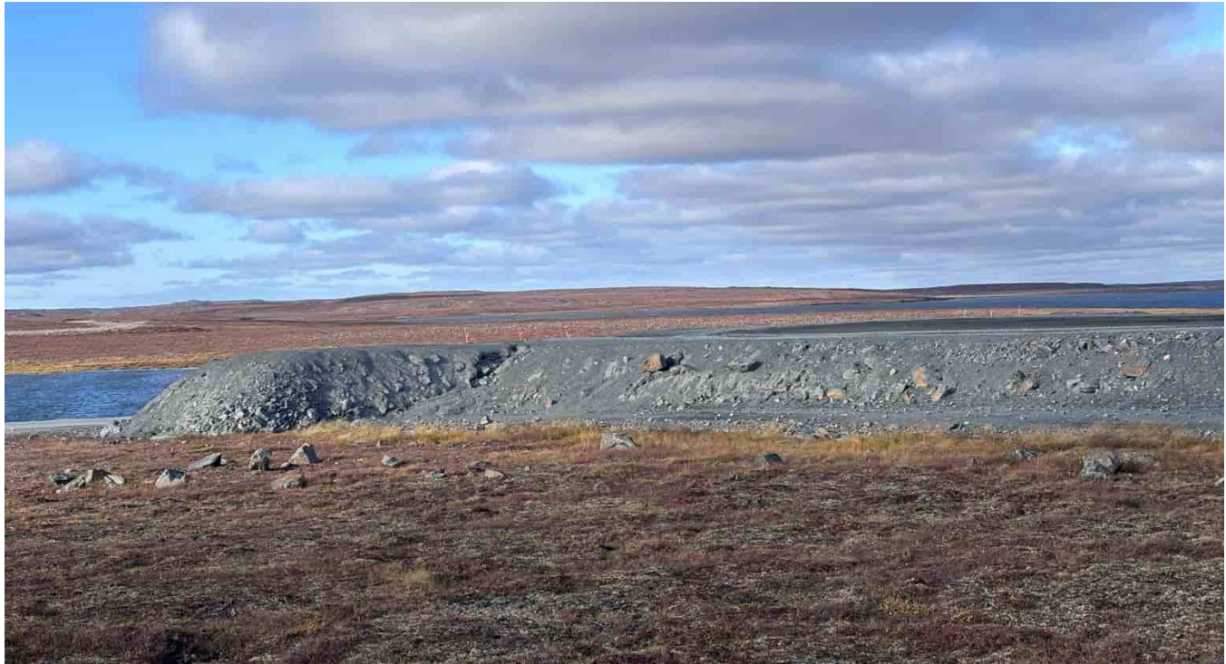
G-47: Airstrip rockfills at NW end of runway
