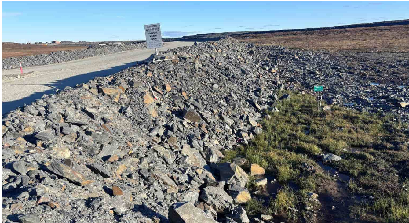
G-96: Echo Pit Haul Road W rockfill
