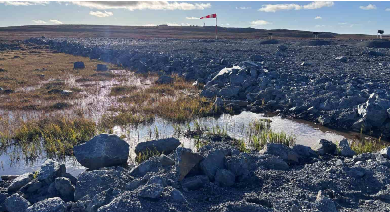
G-54: Ponding water at SE end of airstrip
