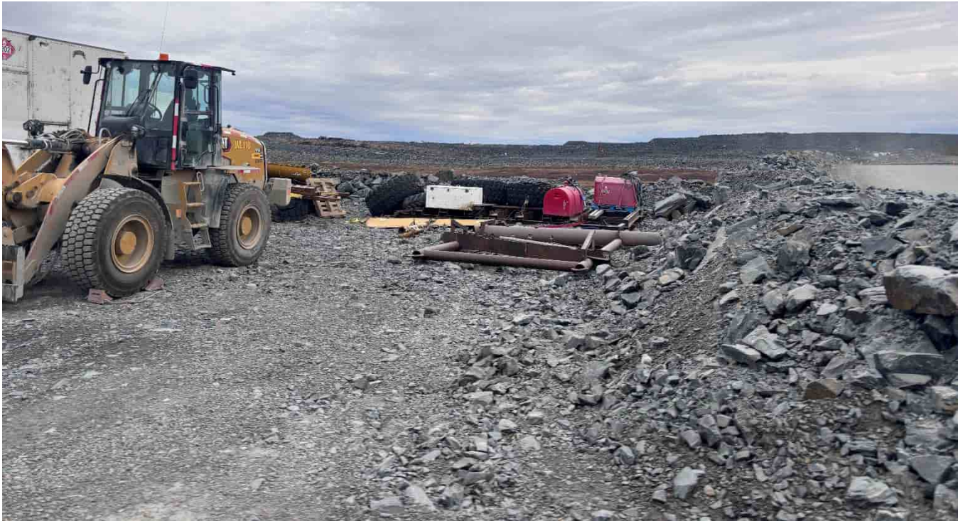
G-169: Laydown area and Echo Pit Haul Road, facing S
