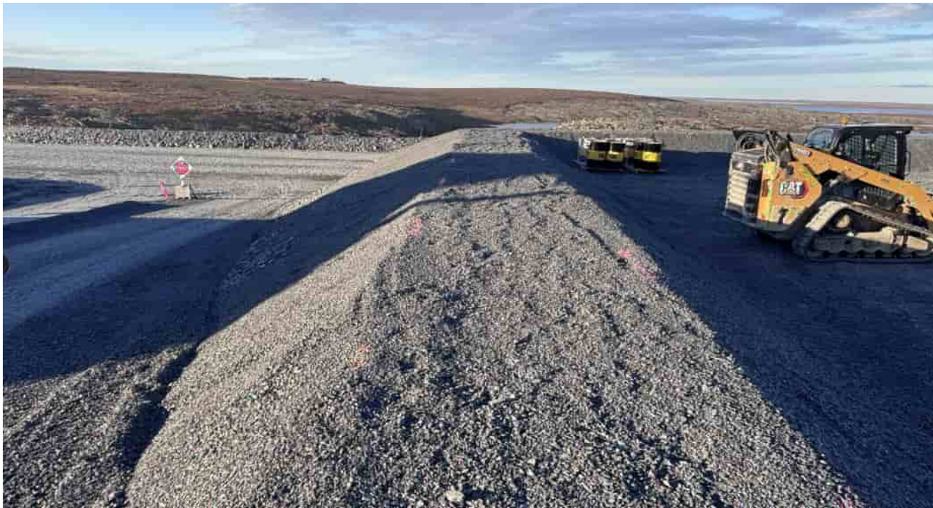
G-218: Tote Storage Facility: Western berm, looking N
