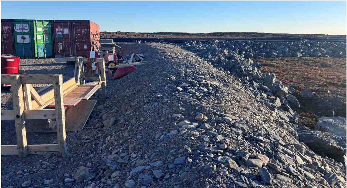
G-188: Berm beside laydown pad, looking S
