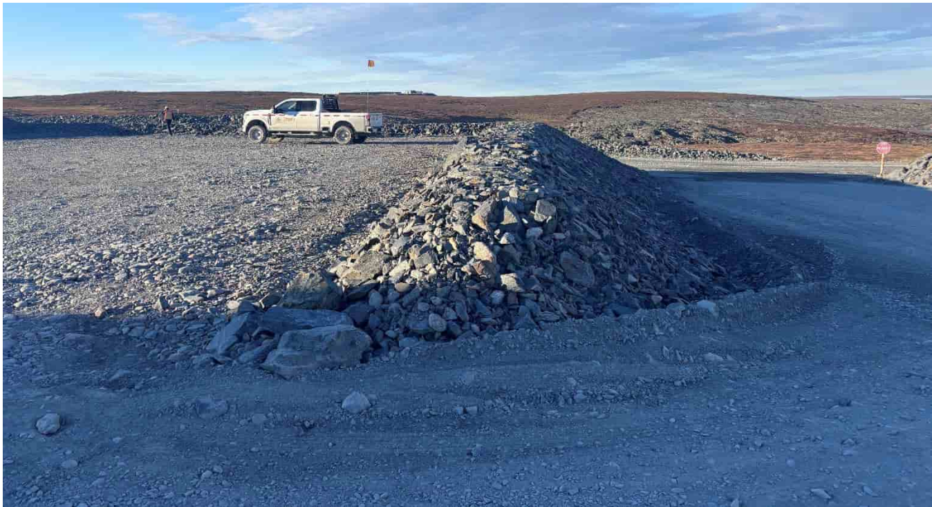
G-186: Parking pad slope above access road, looking N
