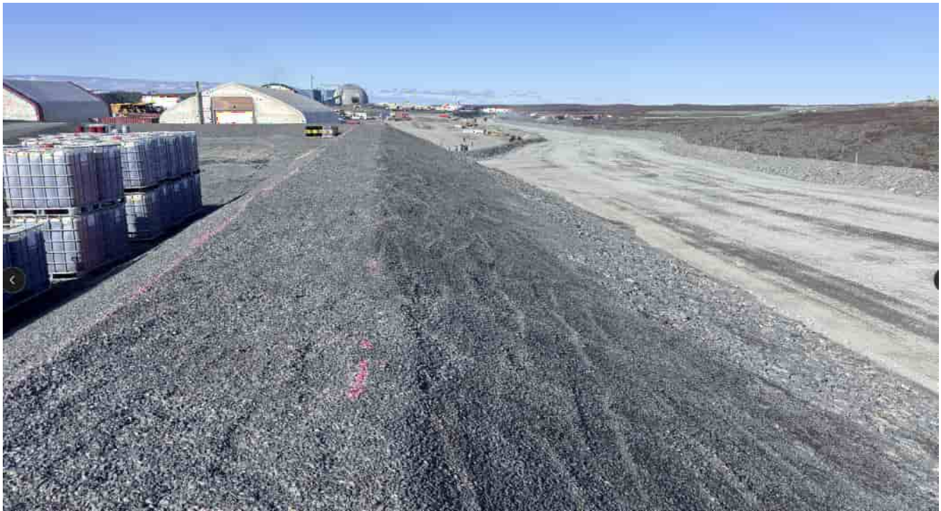
G-214: Tote Storage Facility: Crest and side of the northern berm, looking NW
