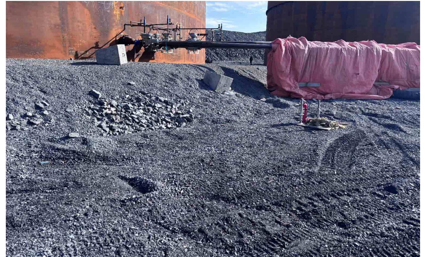
G-370: Slope beside western tanks, looking E
