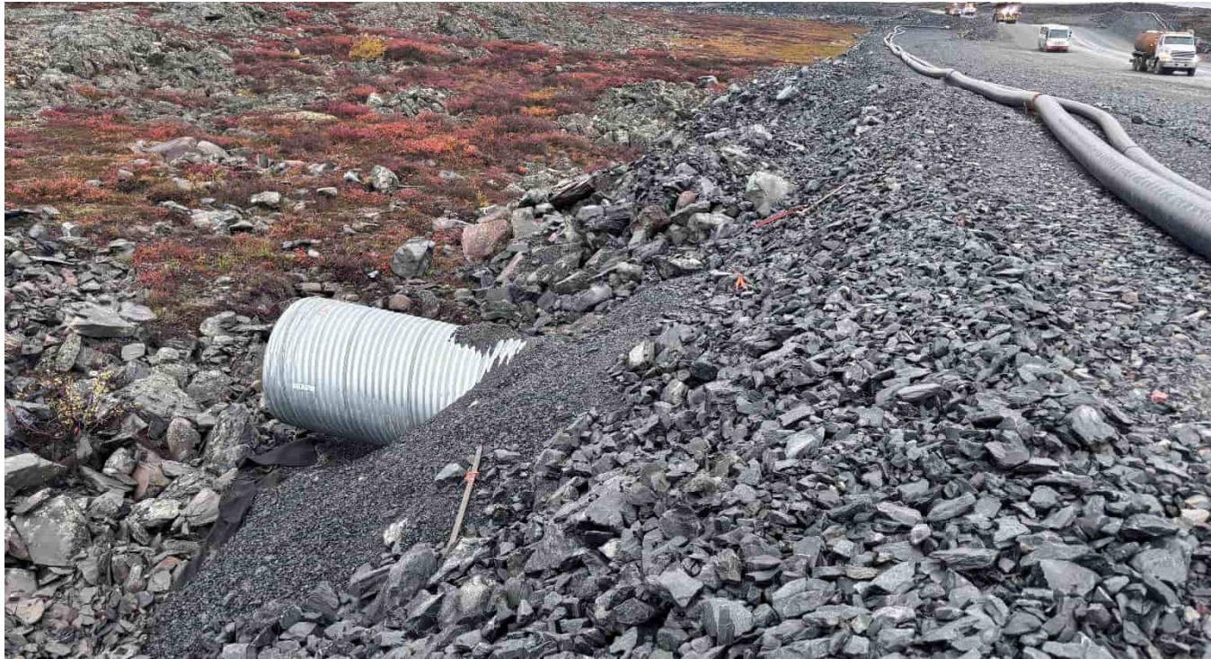
G-391: Northern culvert inlet, facing NW
