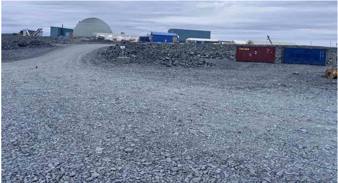
G-384: View towards main plant from laydown area, looking S
