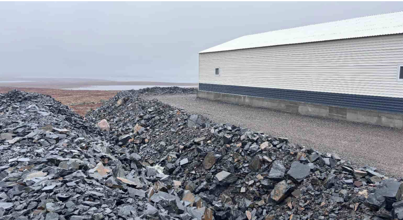
G-432: Berms between emulsion plant and laydown pads, looking E
