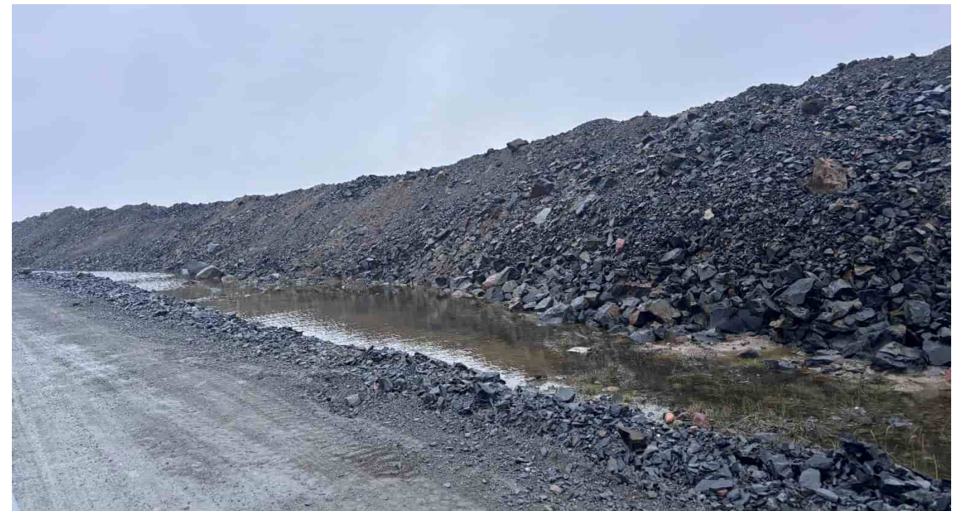
G-405: Ponding between road and N slope of stockpile pad, looking E
