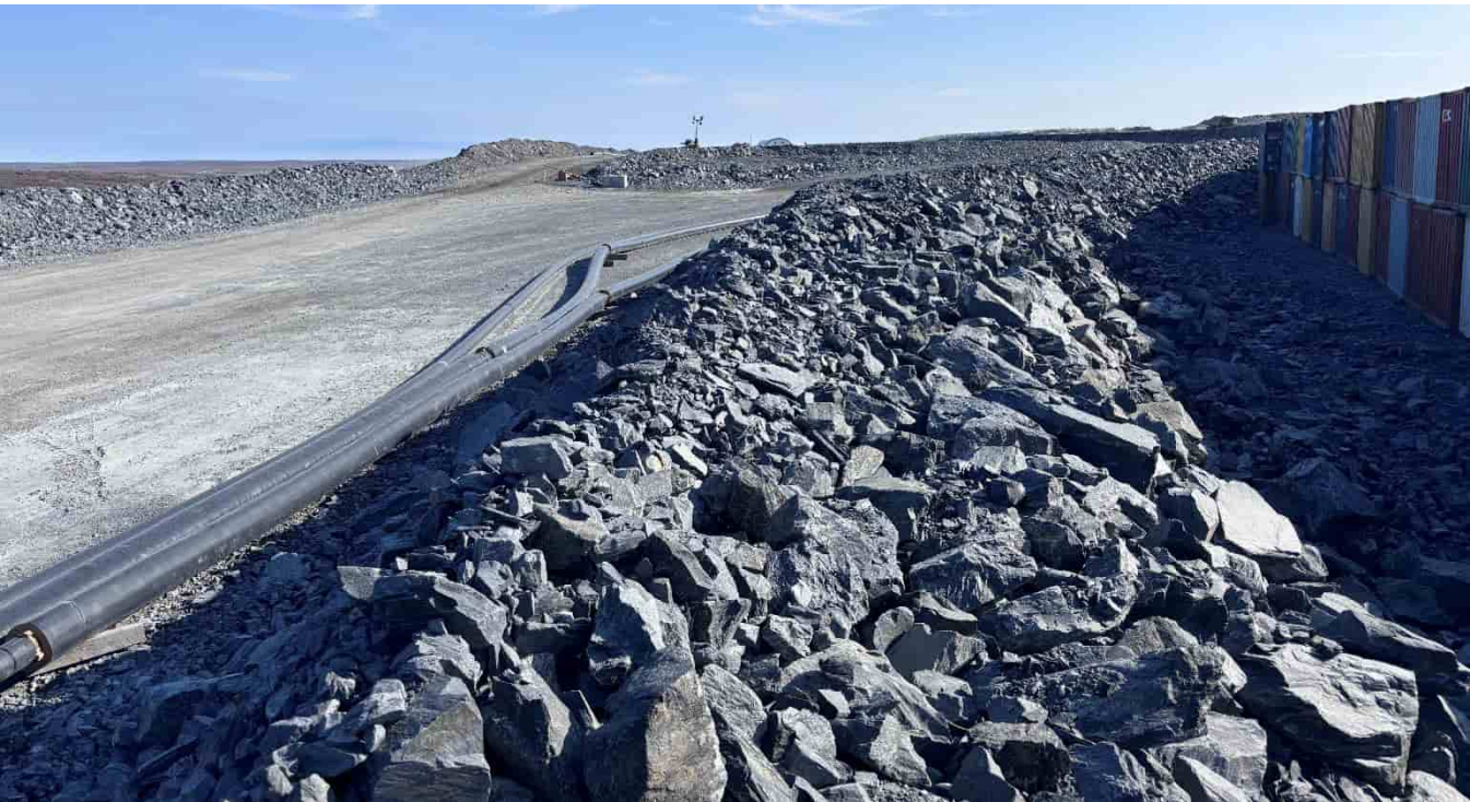
G-247: Berm between tailings pipeline road and seacan laydown area, looking E
