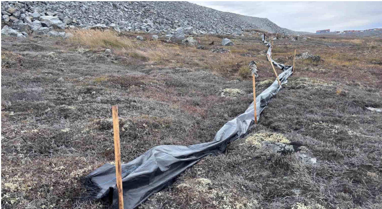
G-254: Silt fencing on N side of road – Looking W
