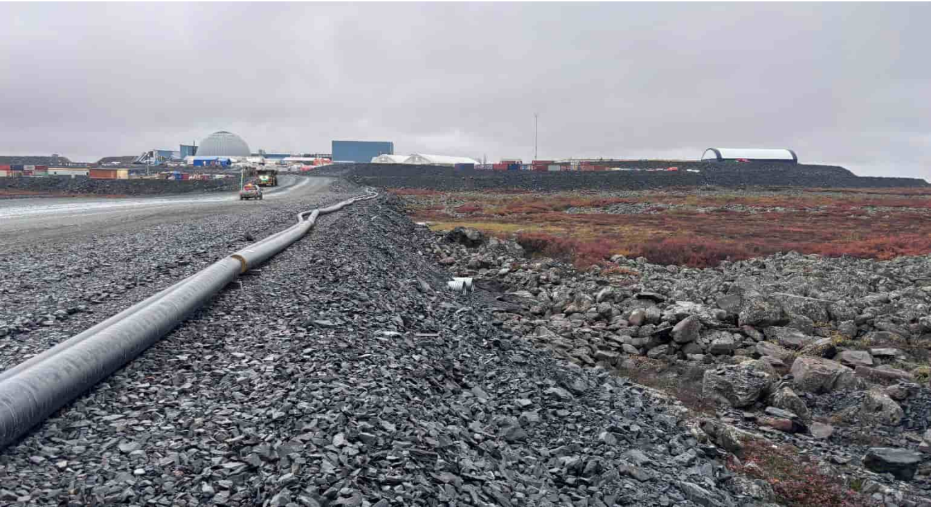
G-392: View towards twin culverts inlet, looking S along road rockfill
