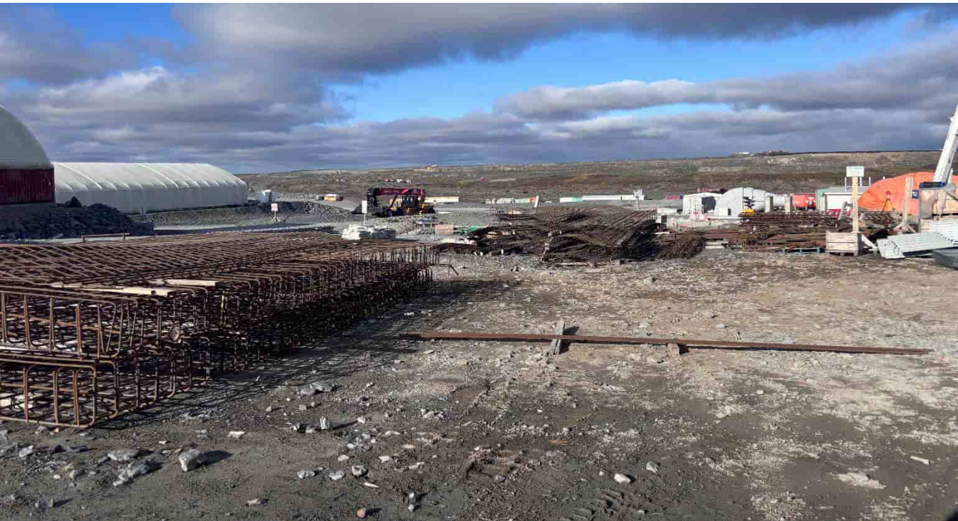
G-307: Rebar laydown N of pipefitters building
