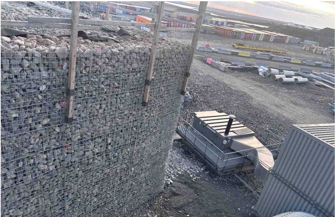
G-318: MSE wall E corner, looking N
