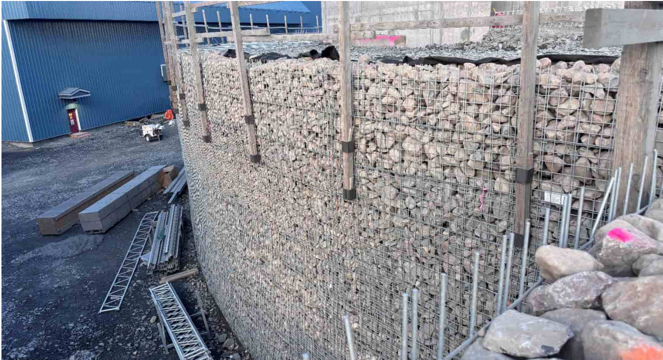
G-314: MSE wall SE side, looking S
