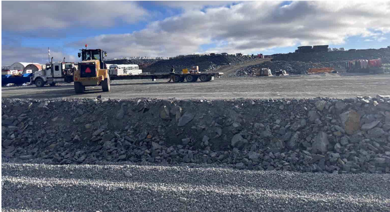
G-240: Underground laydown area as seen from All-Weather Road
