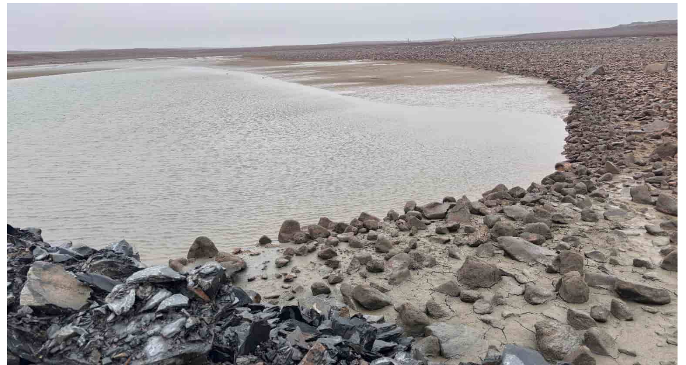
G-451: Pond dewatering waterline, looking NW
