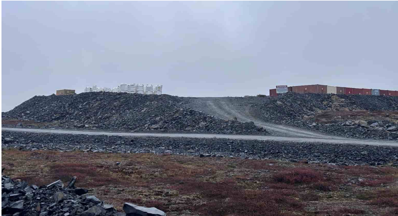
G-410: Explosives storage area, looking NE from rock storage area
