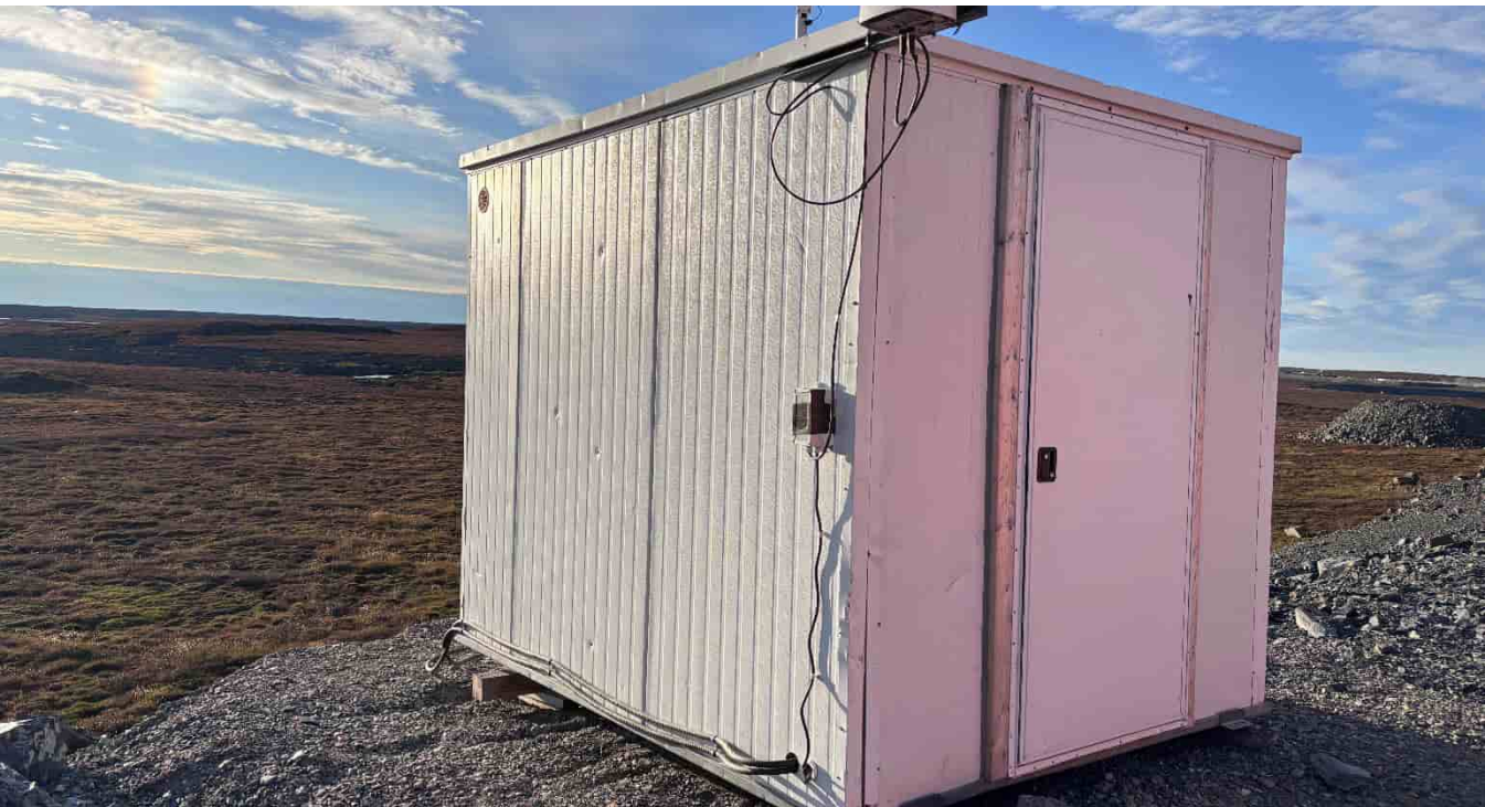
G-272: Storage container close to western pad edge, looking NW – settlement noted in area
