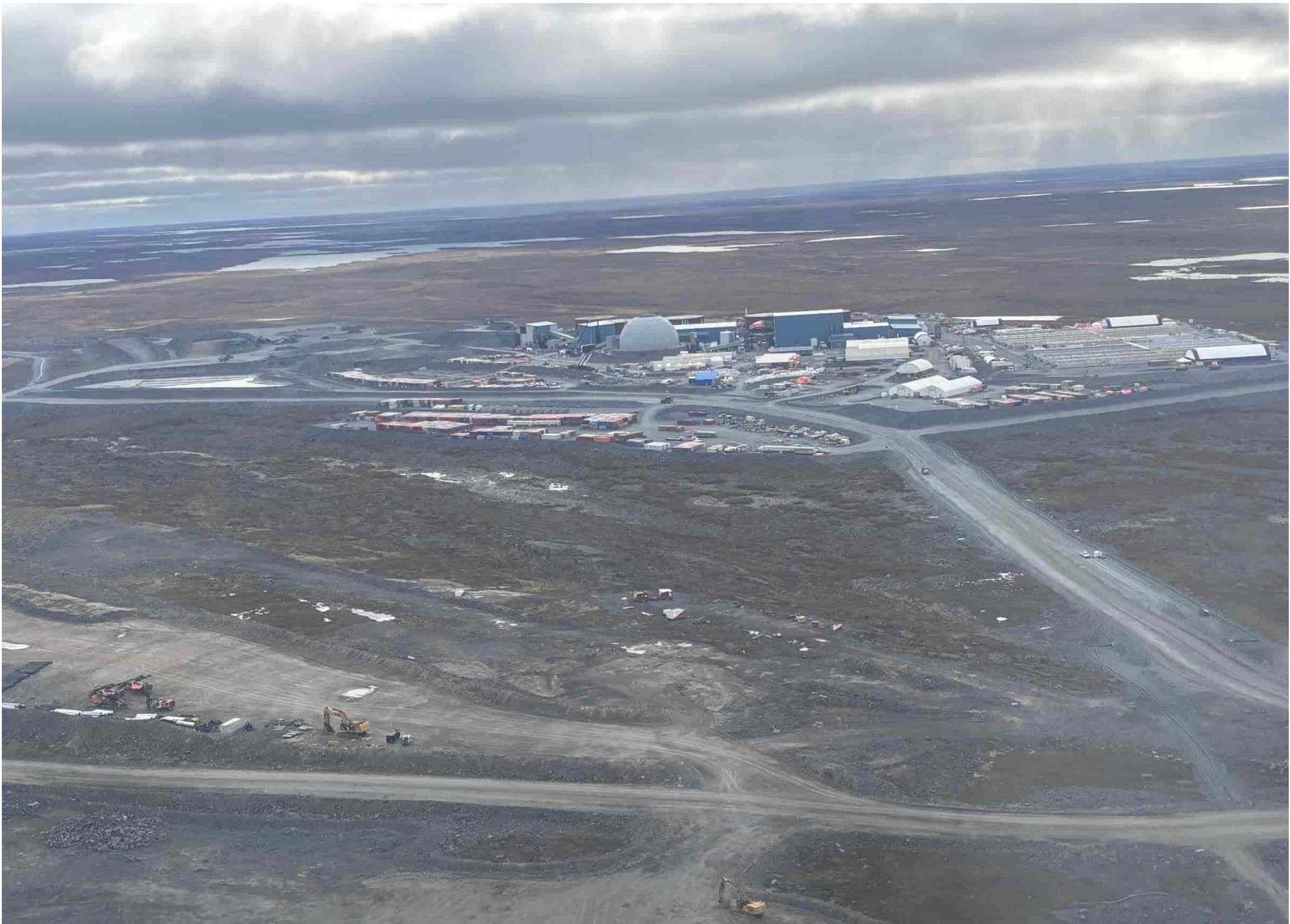
Heli Photo 8: Umwelt overburden stockpile and main plant area, looking S
