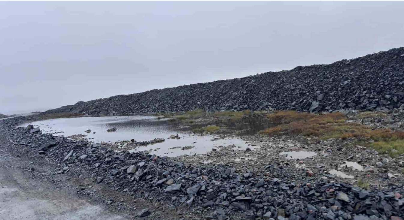
G-419: Ponding at toe of southern pad slope, looking NW
