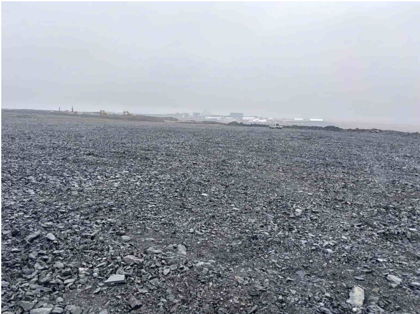
G-422: Typical rock storage area surface conditions, looking S
