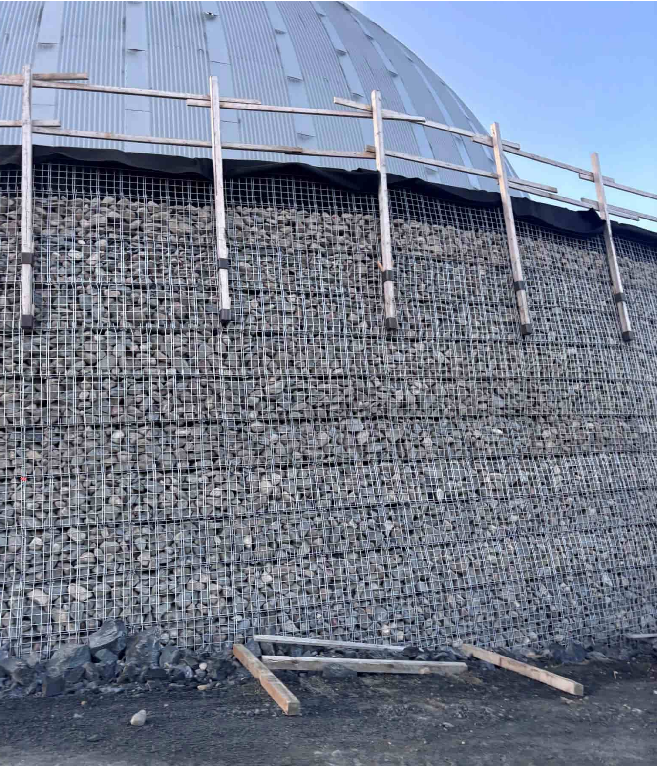
G-312: Typical MSE wall construction
