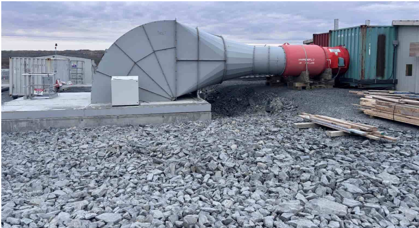
G-302: Vent raise, looking NE
