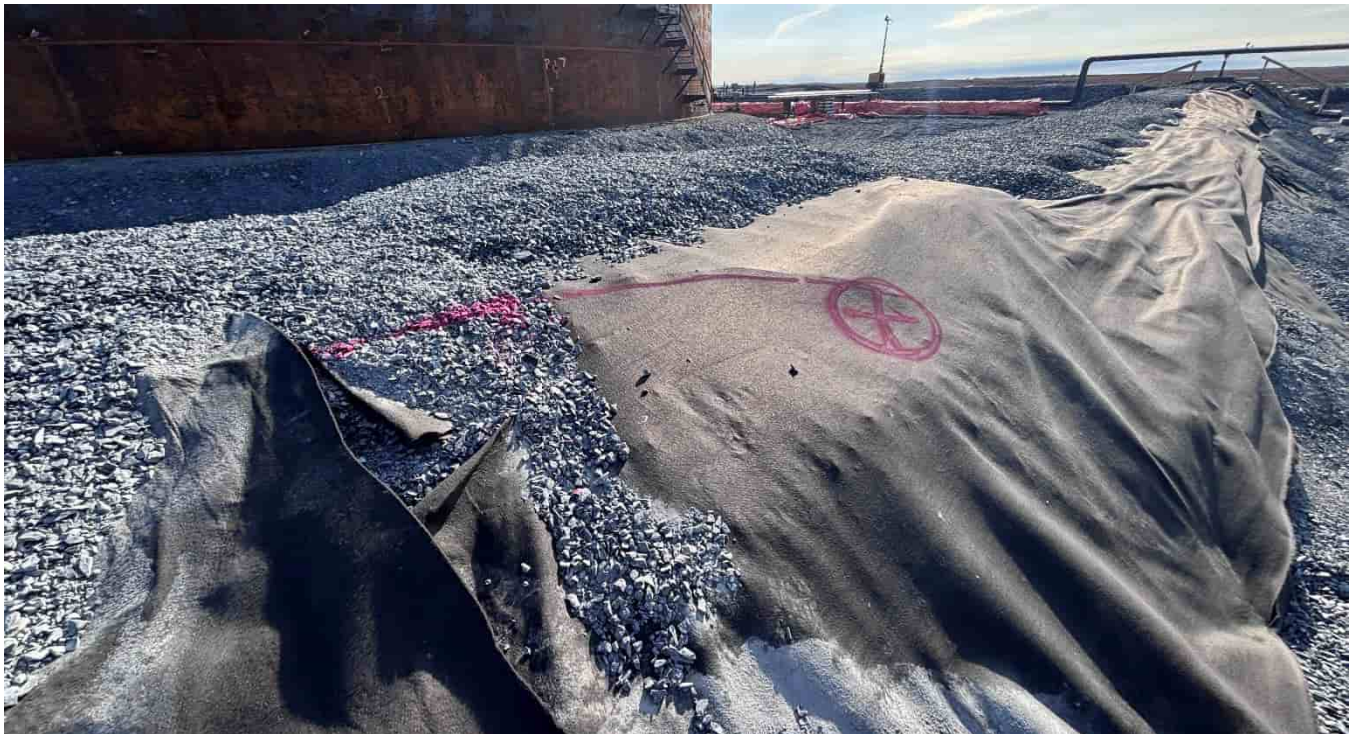
G-360: A berm between central tanks, looking S – the mark indicates the edge of the liner approximately at the elevation governing the containment volume – areas revisited with site staff during visit
