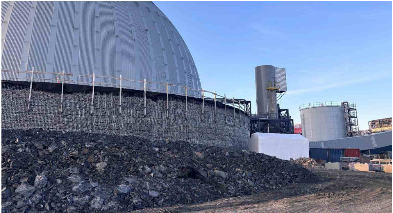
G-311: Ore dome MSE wall, looking SW
