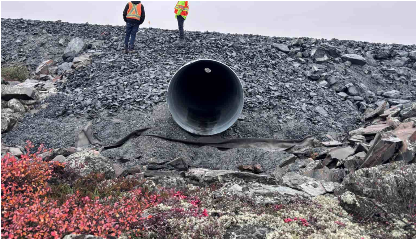
G-397: Northern culvert outlet
