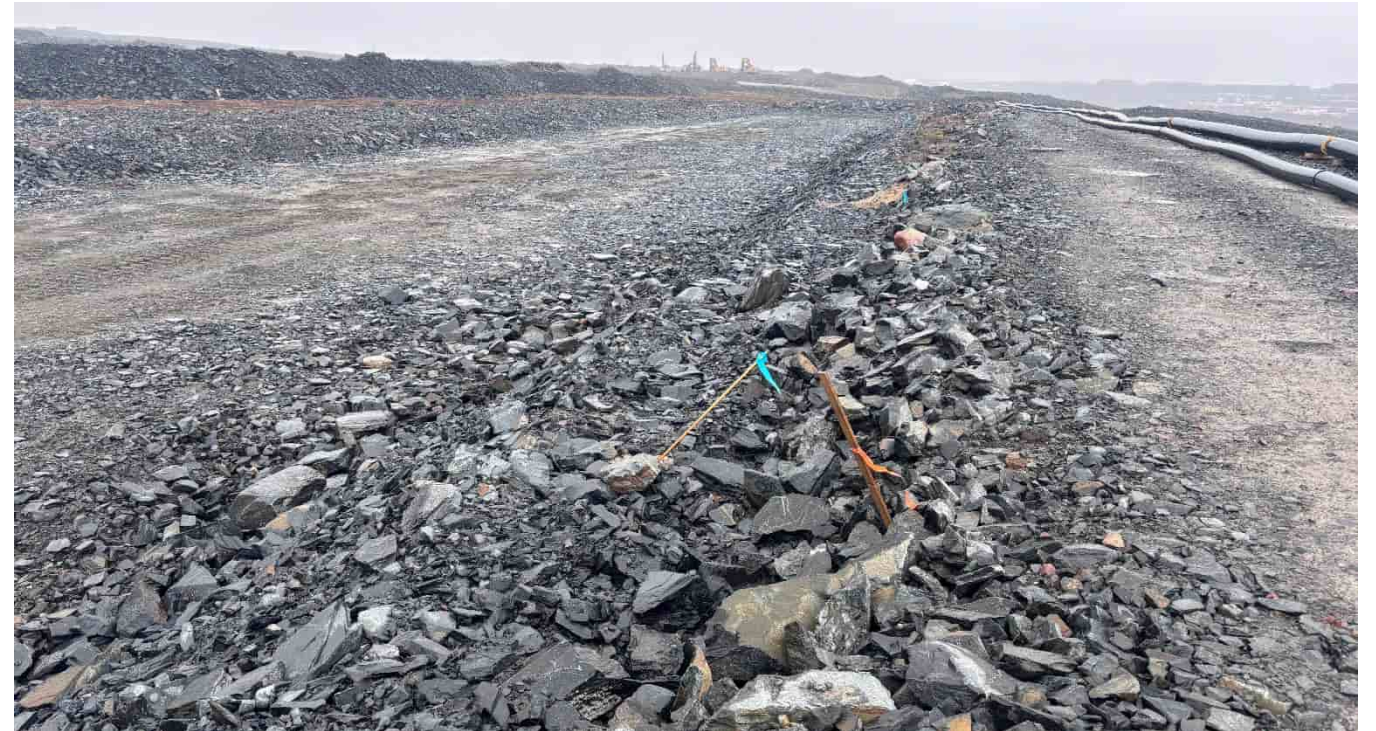
G-459: Western edge of spillway, looking SE
