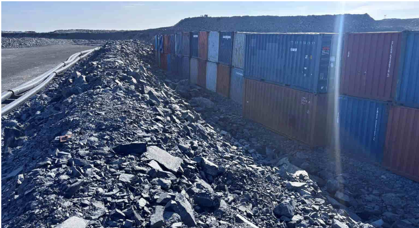
G-290: Berm between tailings pipeline road and seacan laydown area, looking SE
