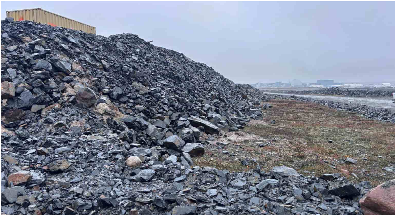
G-424B: Slope below explosives storage area, looking S
