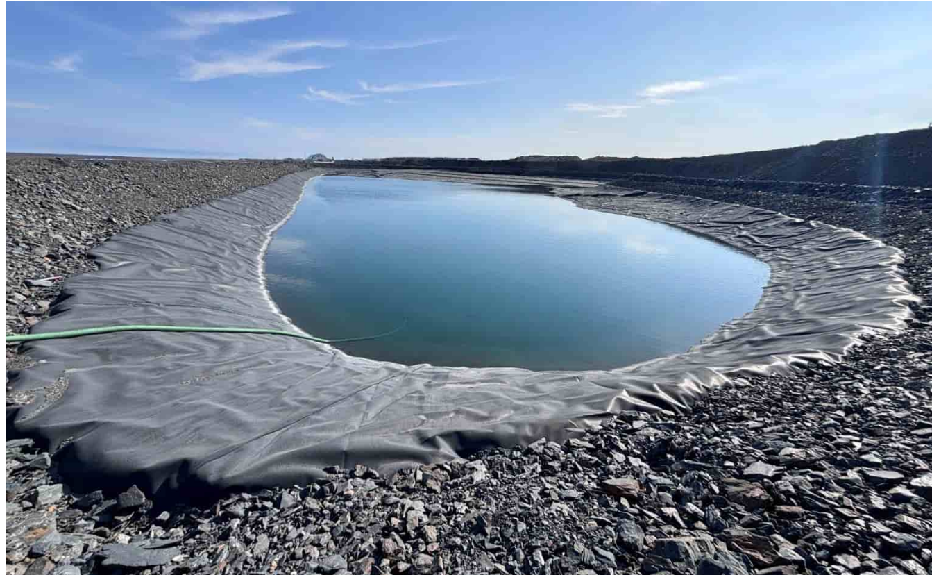
G-239A: Overall pond view from NW corner
