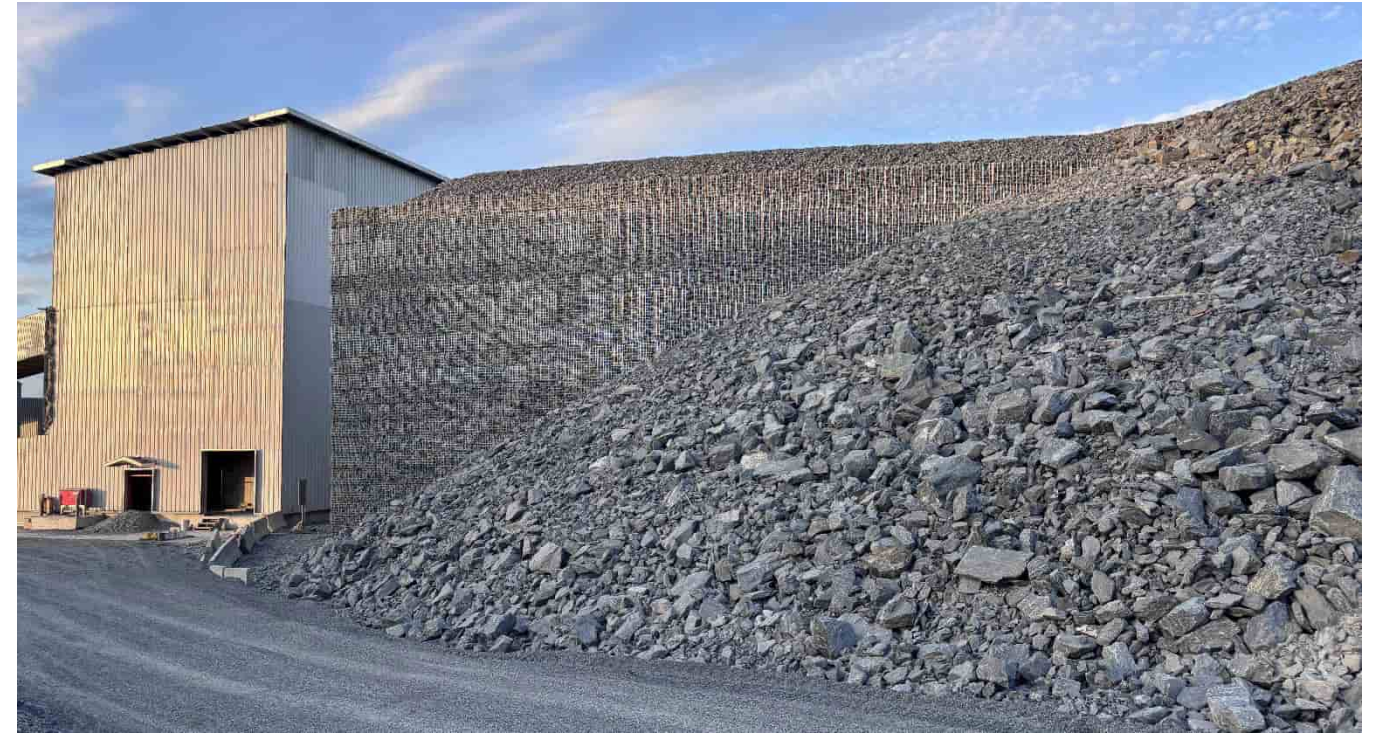
G-322: MSE wall and slope, looking N
