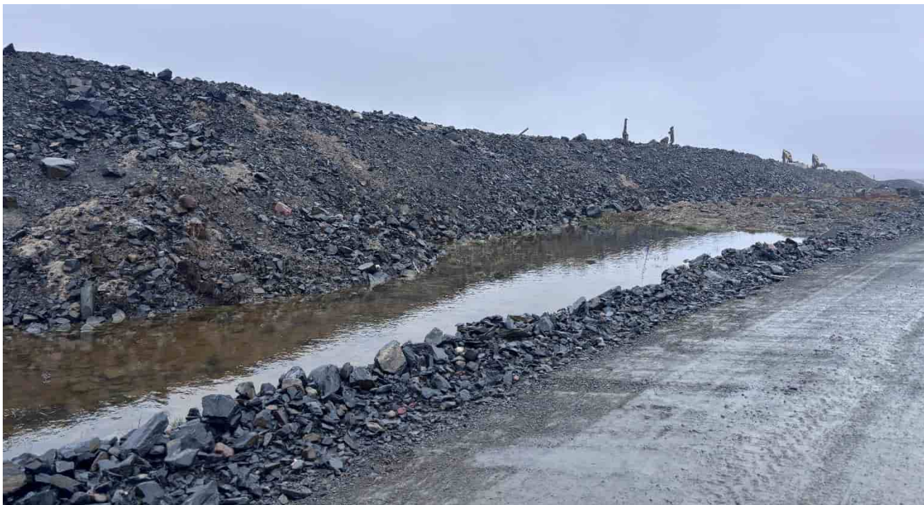
G-404: Ponding between road and N slope of stockpile pad, looking W
