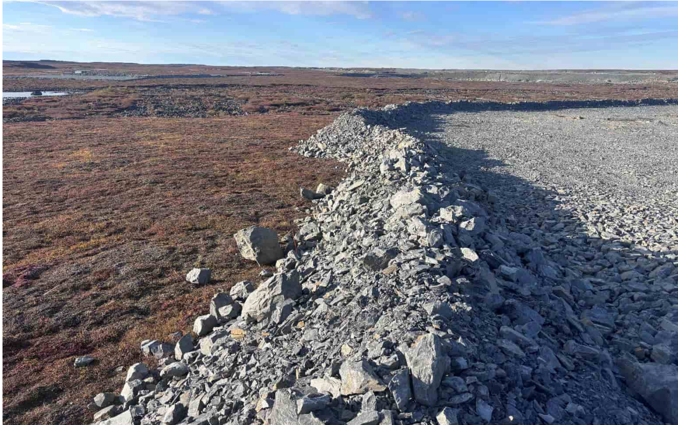
G-262: Camp pad W slope, looking N
