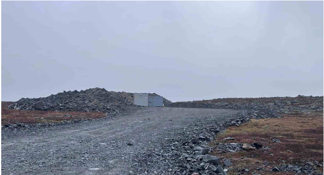
G-425: Access road, looking S
