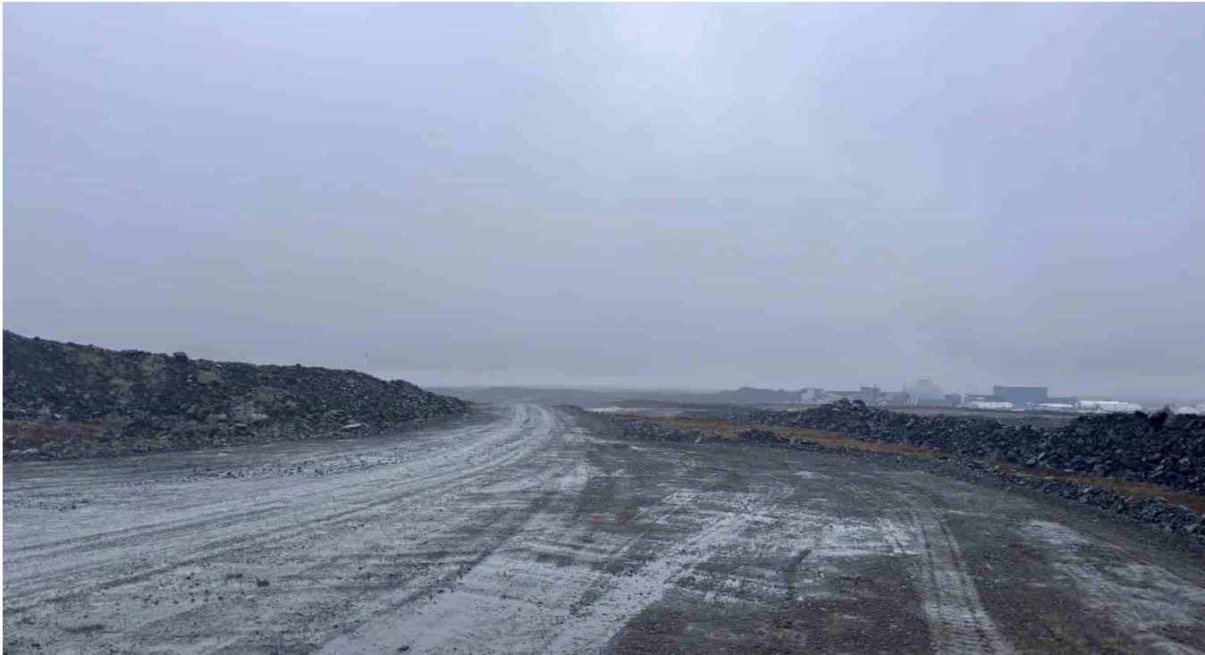
G-423B: Explosives area access road, looking S
