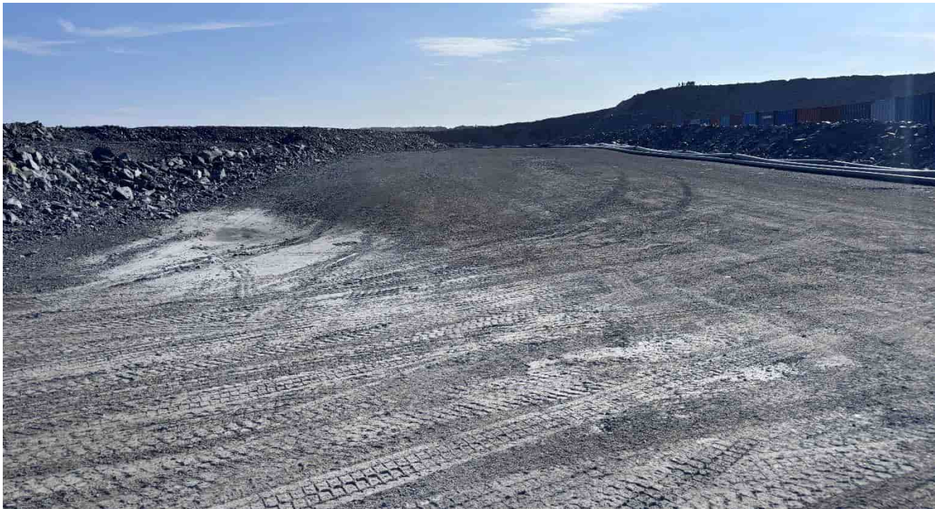
G-246: Laydown area and tailings pipeline W of contact water pond
