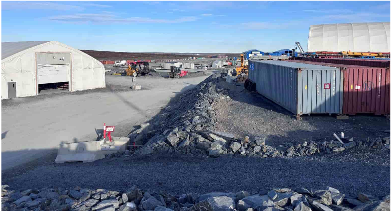
G-258: View towards site services area from camp pad, looking E
