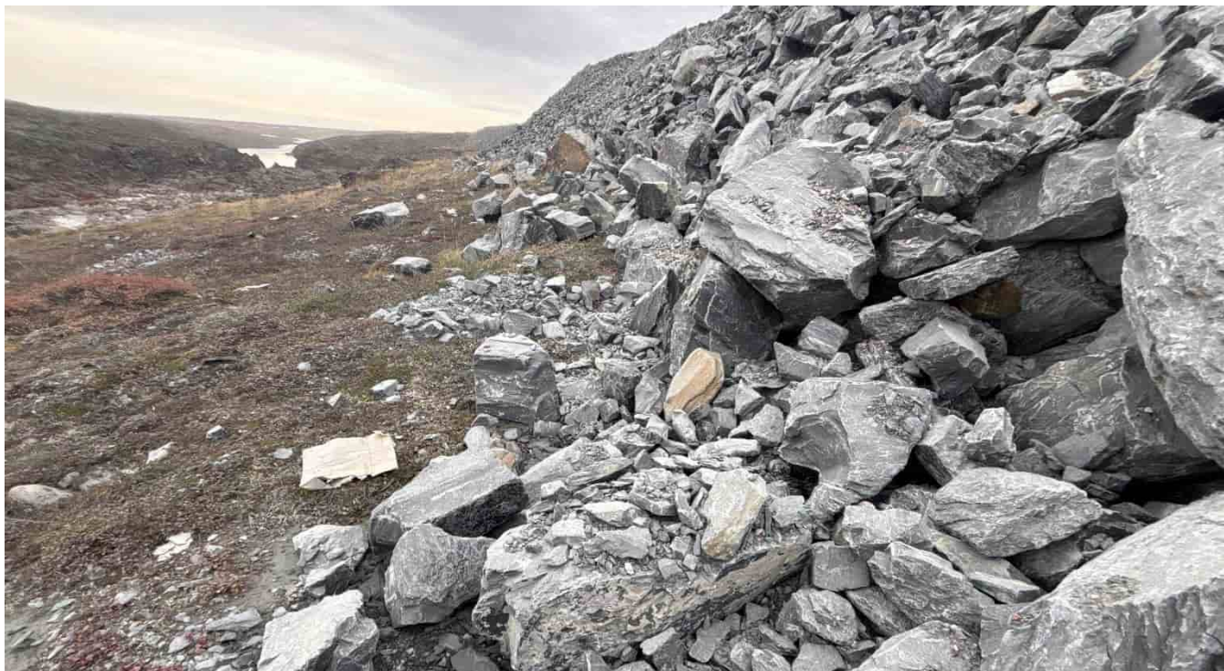
G-250: Downstream slope of All-Weather Road N rockfill
