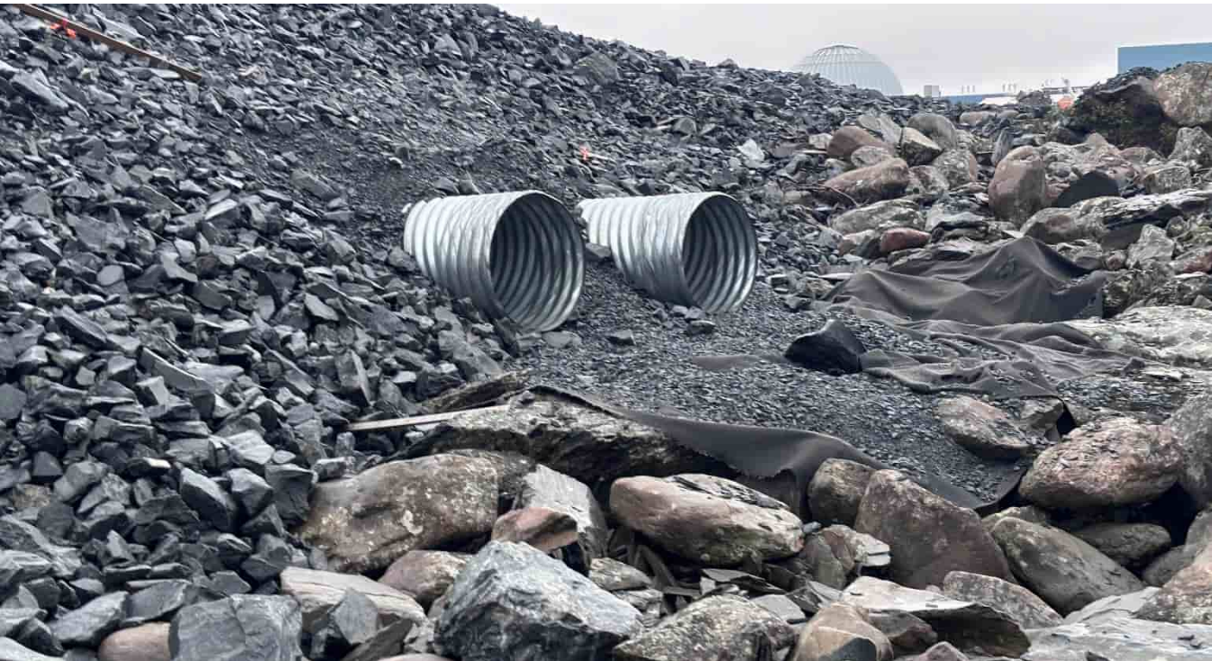
G-394: Twin (southern) culverts inlet
