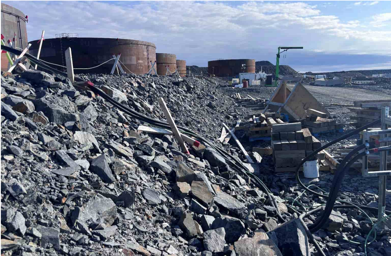
G-382: Laydown area S of tank farm, looking E from fuel transfer / refueling
