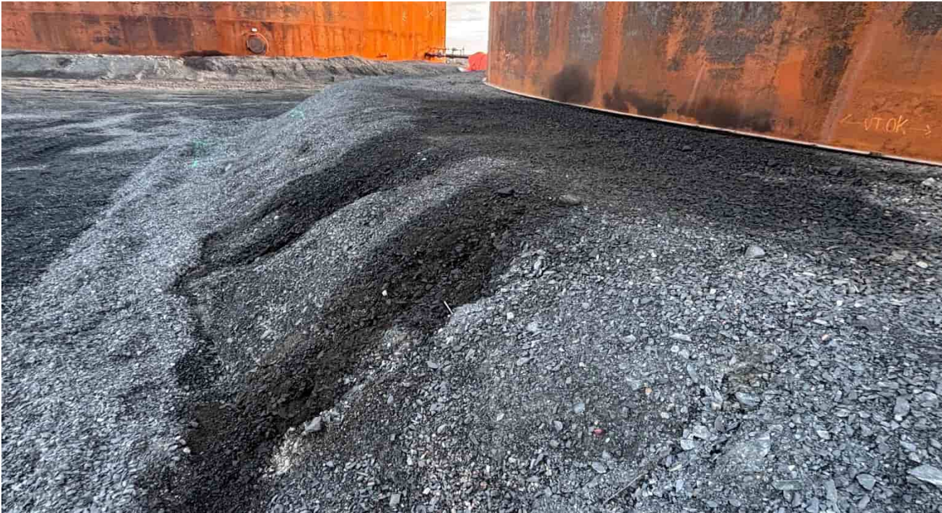
G-331: Tank pedestal slope
