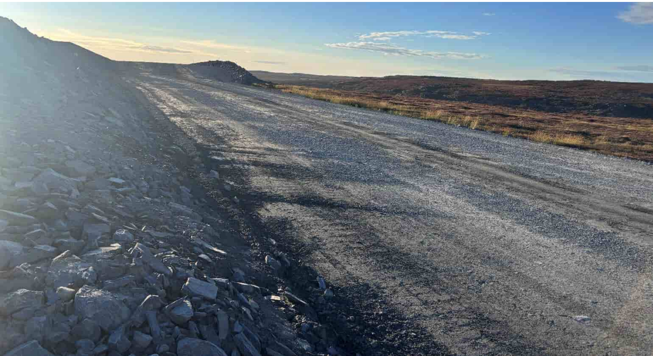
G-243: All-Weather Road slope below Sandvik laydown, looking W
