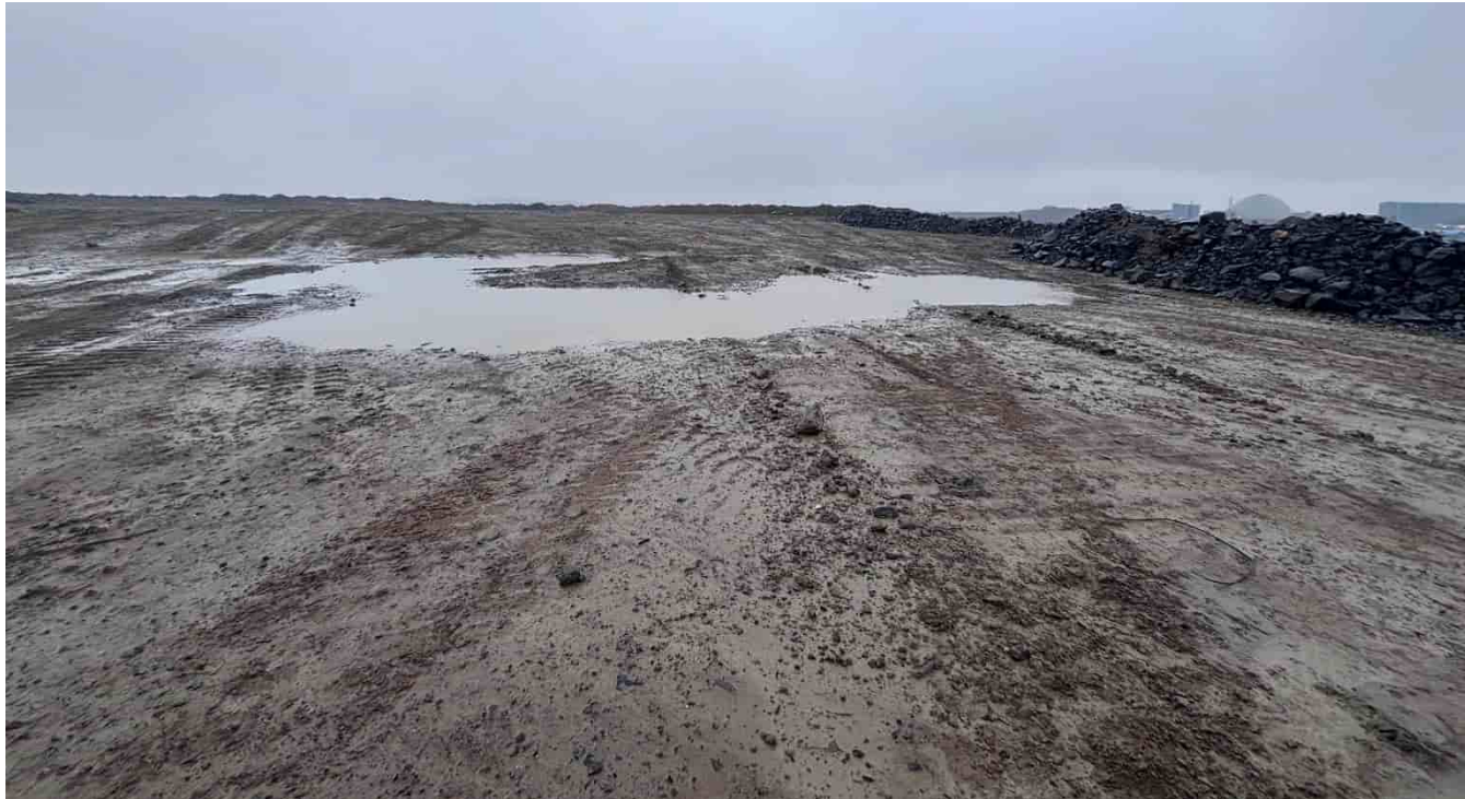
G-402: Ponding on overburden stockpile surface, looking S
