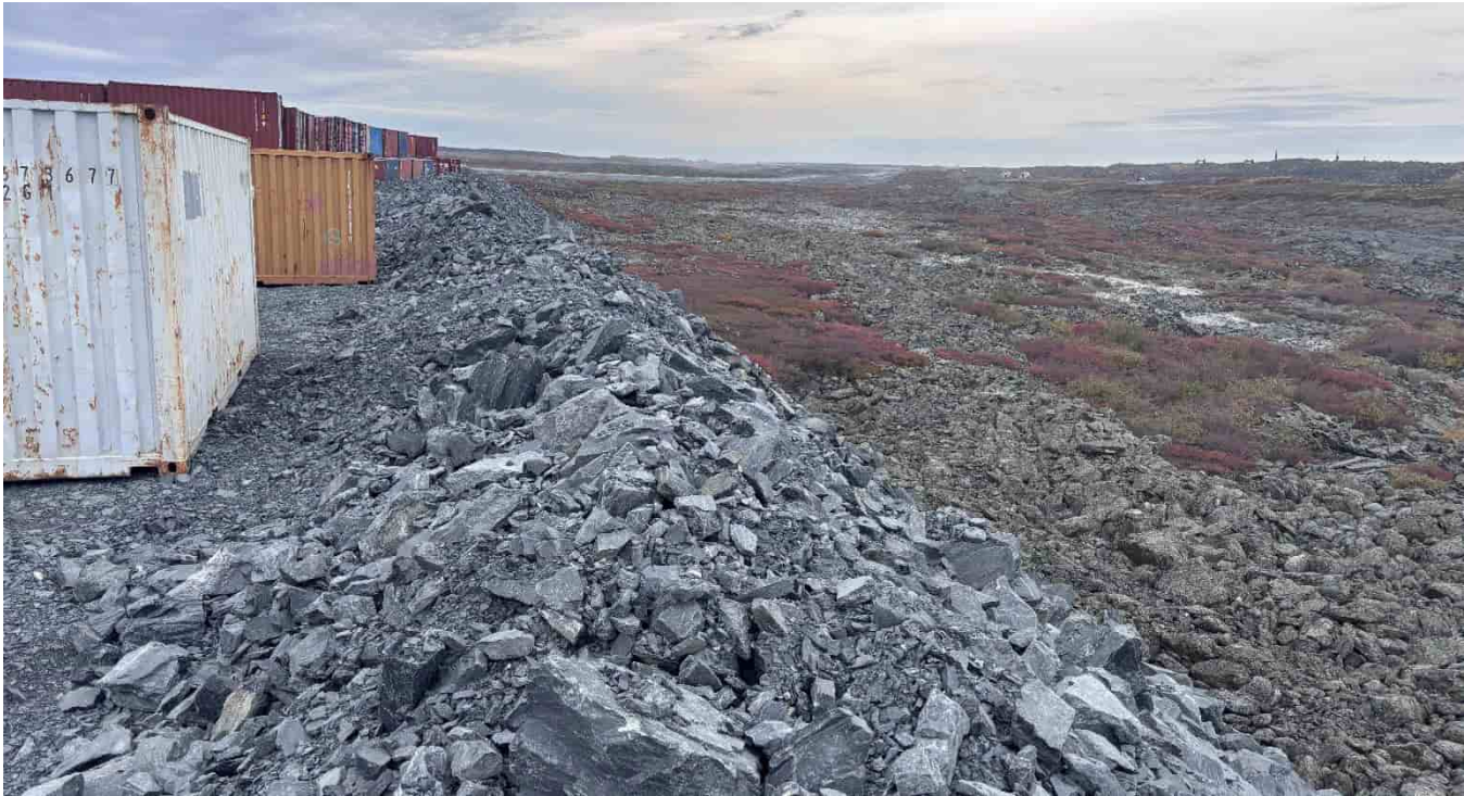
G-385: Laydown area NE pad slope, looking NW
