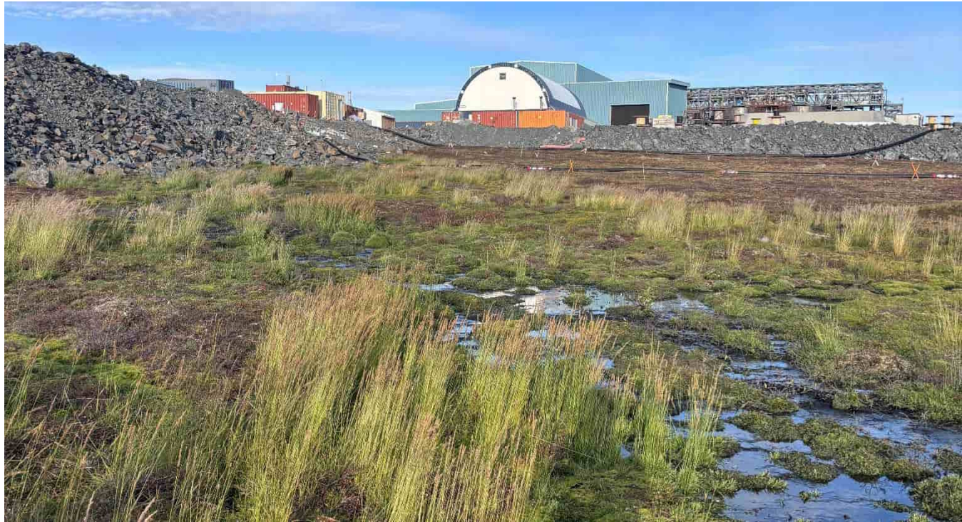
G-265: S edge of camp pad, looking E – downstream of post (grey water) treatment discharge
