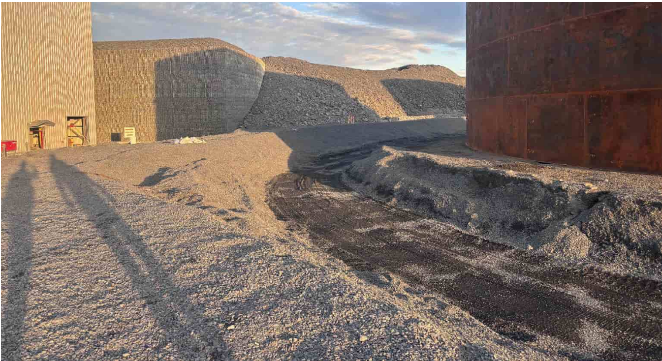
G-333: View E towards crusher MSE wall from tank farm
