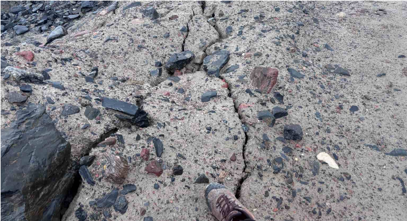
G-399: Example of settlement cracks (expected) in overburden stockpile surface
