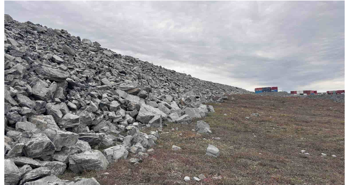
G-249: All-Weather Road N rockfill, looking W
