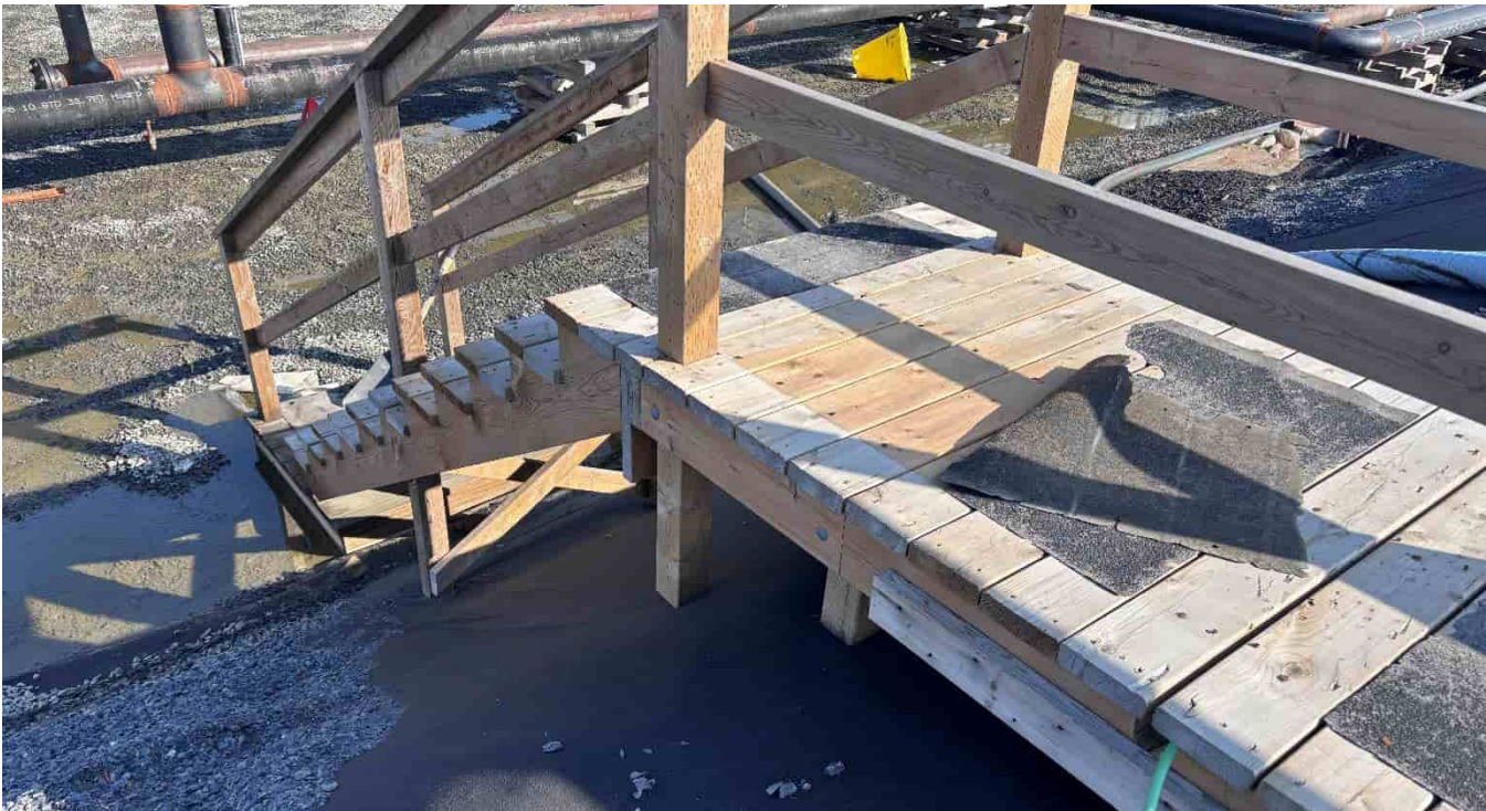
G-353: Stairs over southern berm, looking N. Stairs installed on top of the exposed geotextile.
