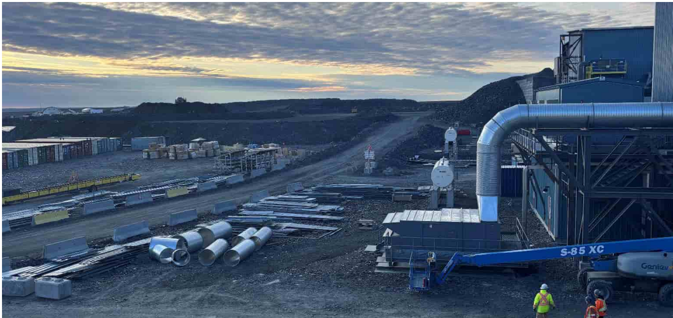
G-319: View SE towards crusher from MSE wall
