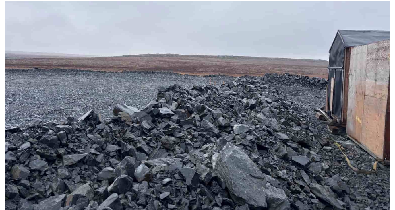
G-447: Pad and berm around future SWP Dam area
