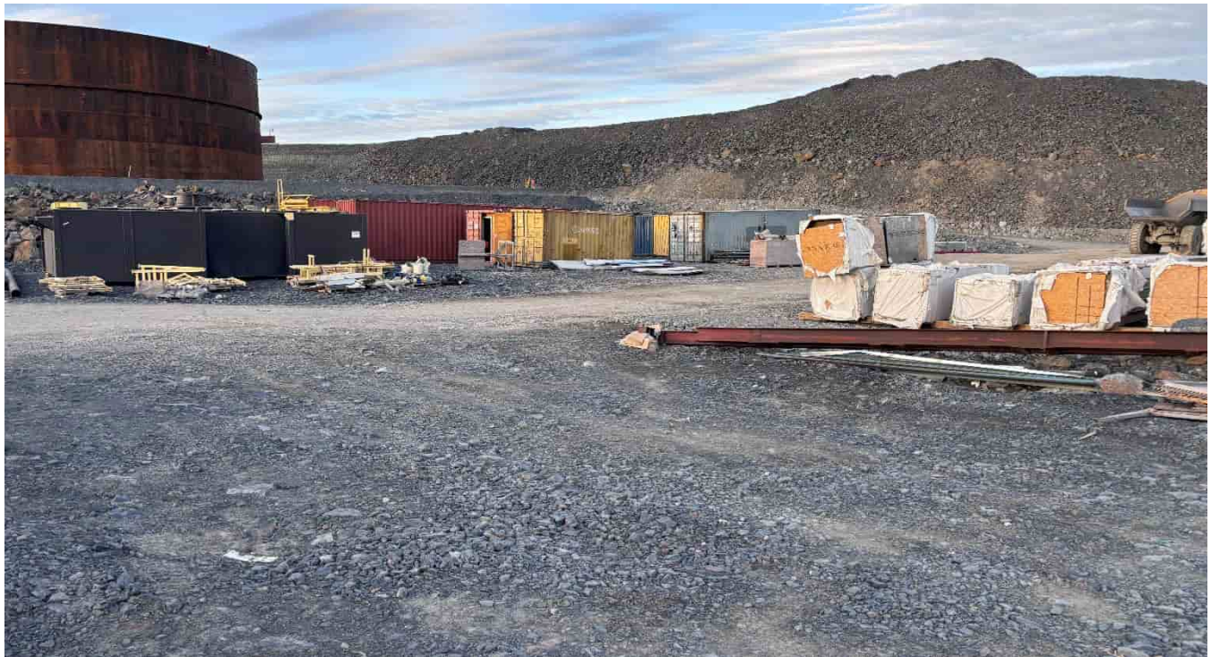
G-286: Looking NE from laydown area towards tank farm and ROM stockpile
