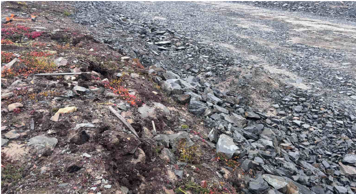
G-456: Southern end of spillway, looking N
