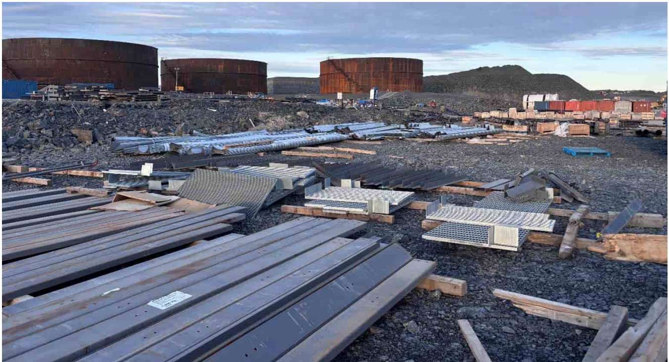
G-282: Laydown area, looking NE
