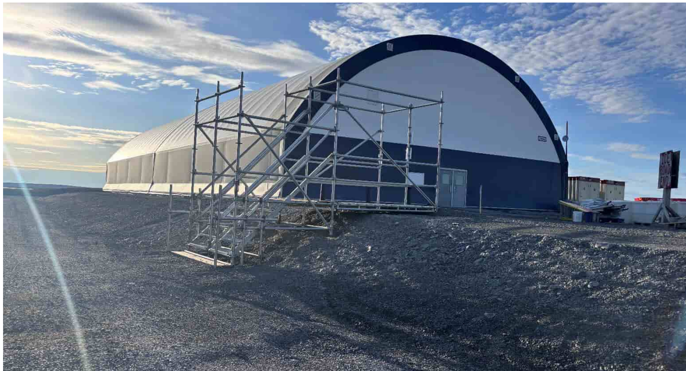
G-267: Berm at N end of camp pad, looking W
