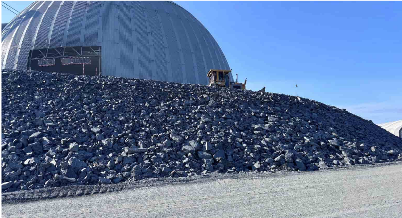
G-296: Typical slope below ore dome
