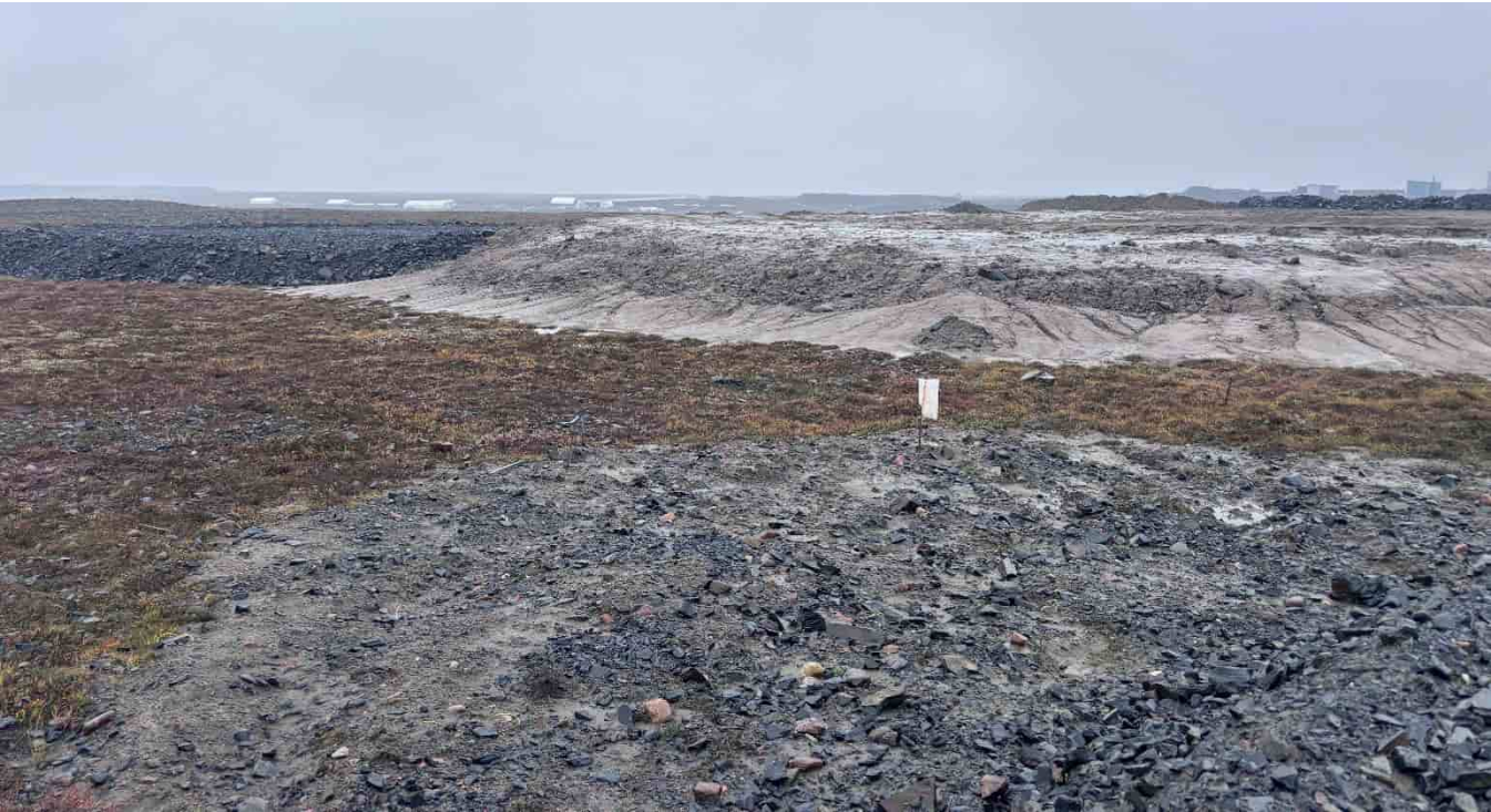
G-407: Overburden stockpile, looking S from road – some erosion from surface water noted on slopes
