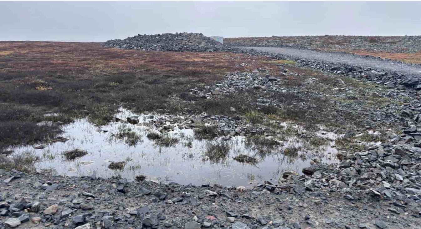
G-426: Emulsion plant access road, looking S
