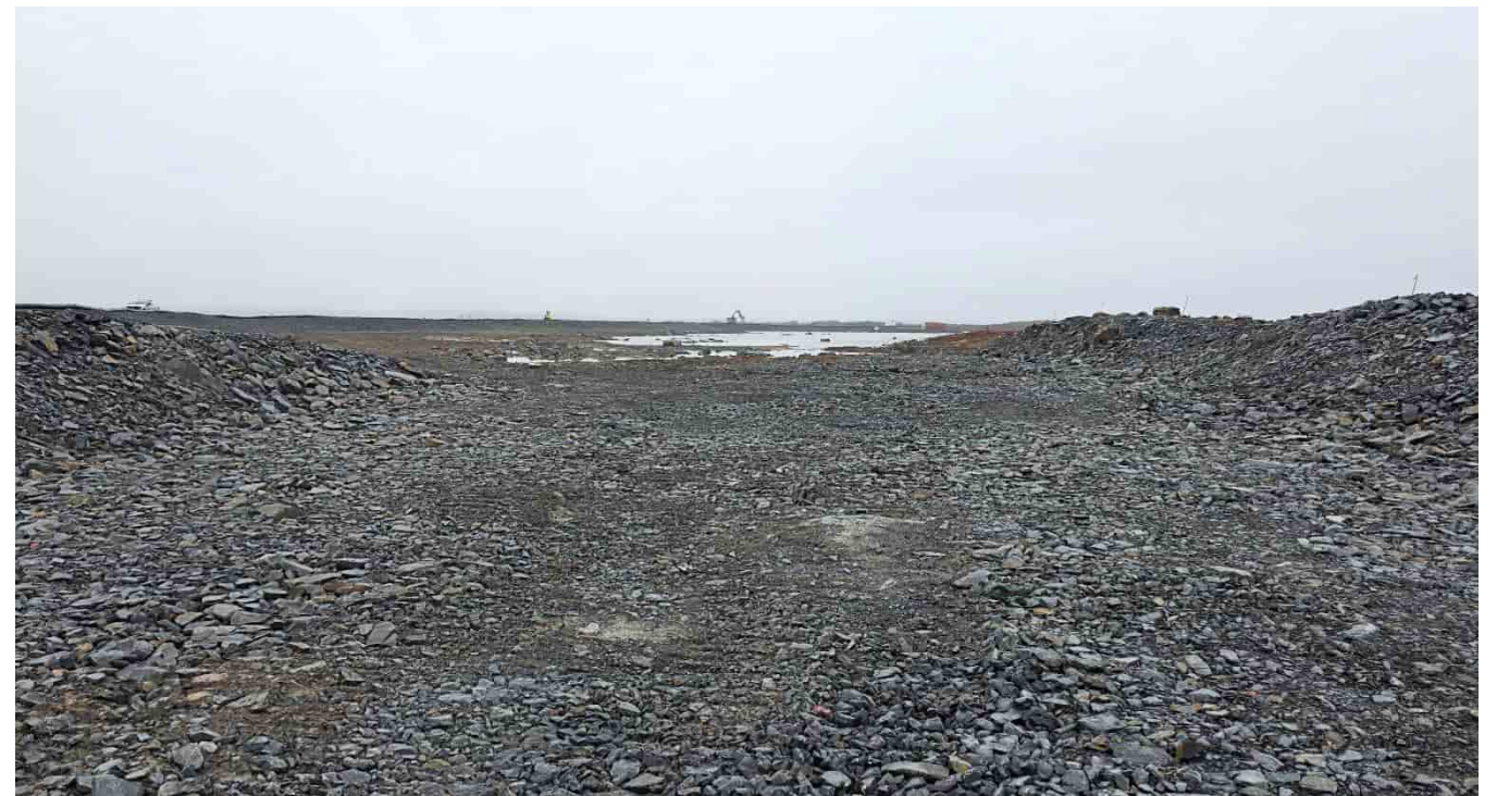
G-461: Upstream (NW) end up spillway, looking NW
