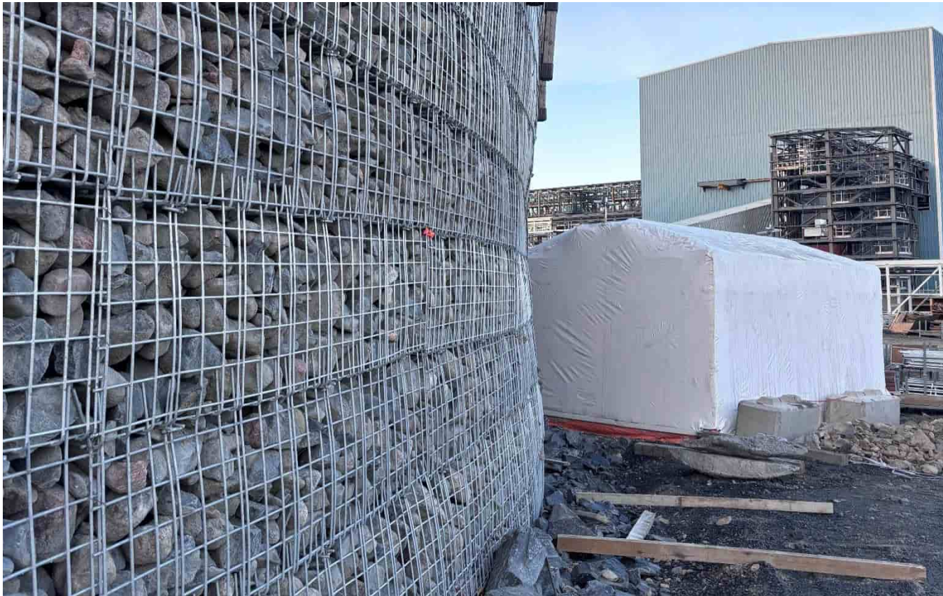
G-320: Typical MSE wall construction
