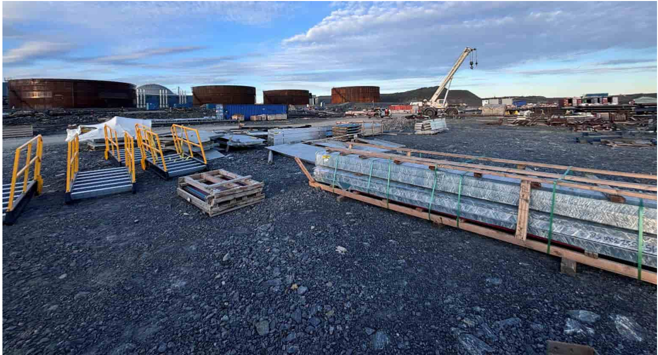
G-280: Laydown S of tank farm, looking NE
