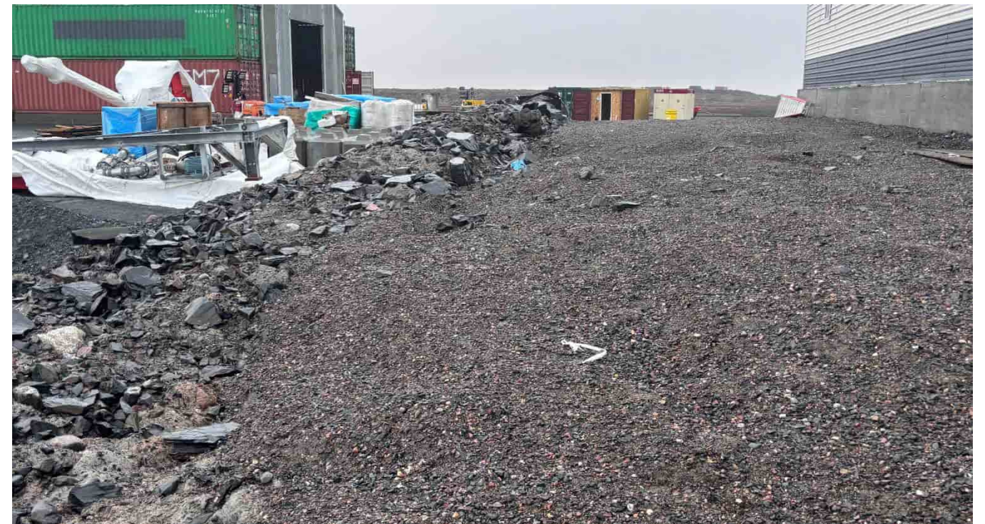
G-436: Emulsion plant berm, looking W
