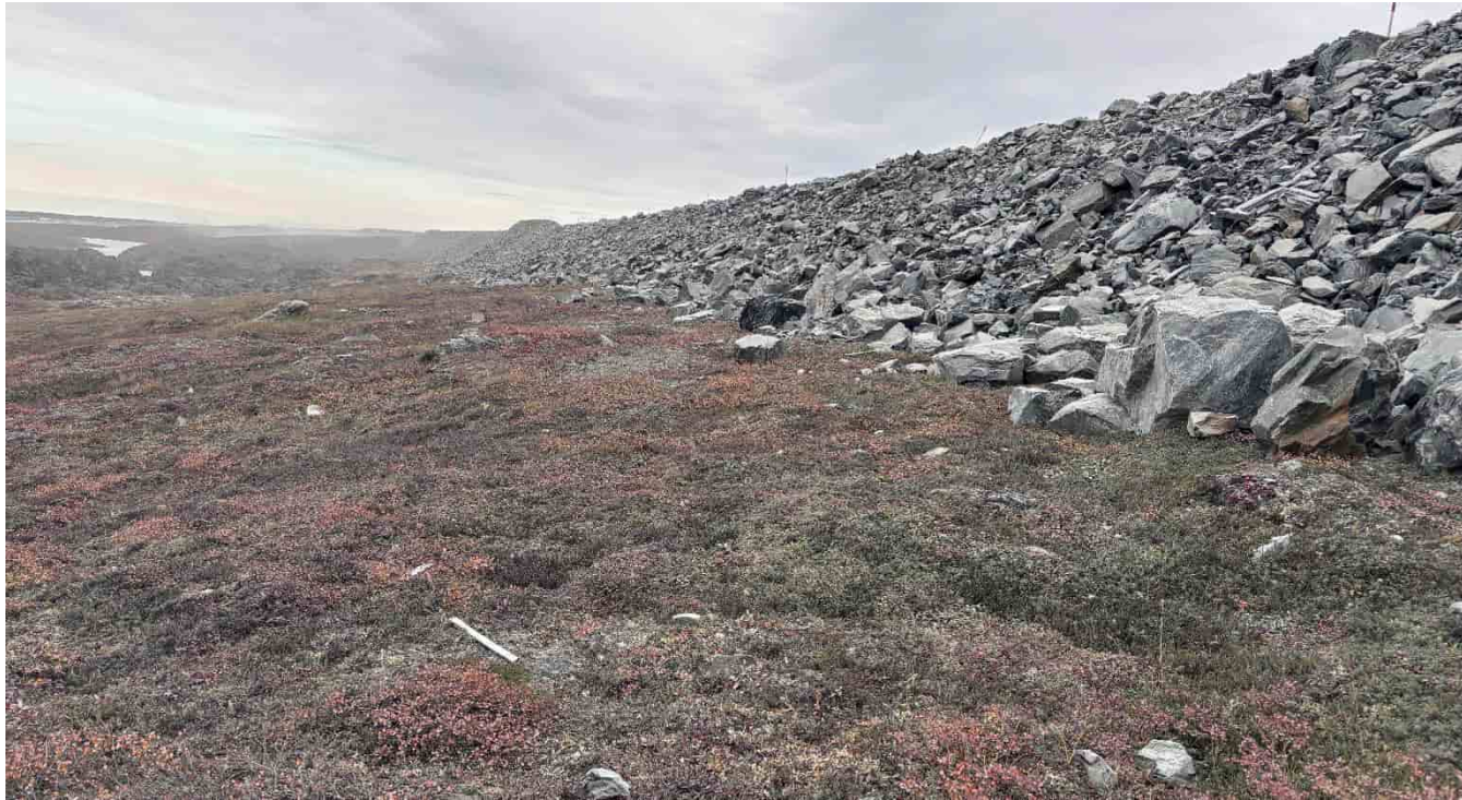
G-248: All-Weather Road N rockfill, looking E
