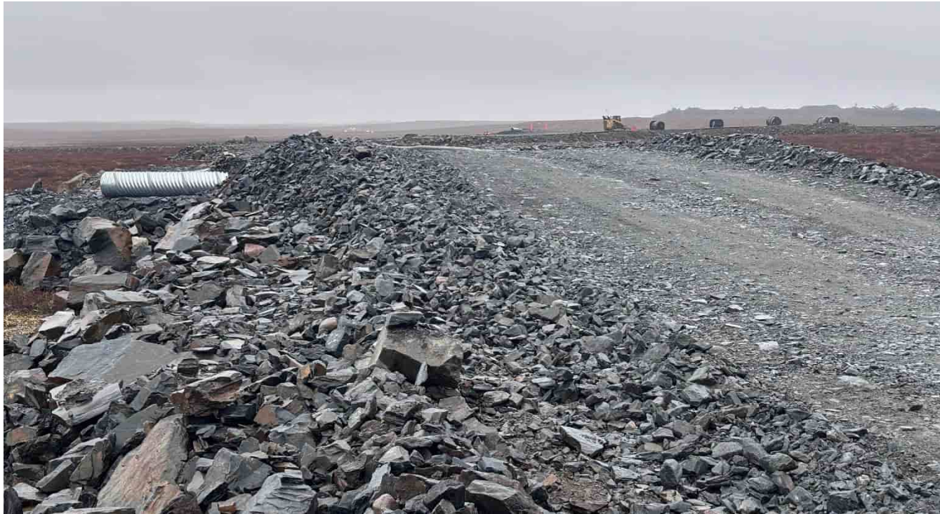
G-444: Culvert under SWP Dam Access Road, looking NW
