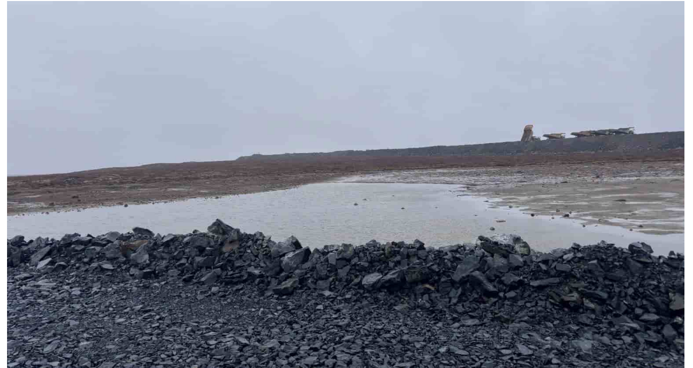
G-449: Northeastern pond (Round Pond) dewatering, looking N
