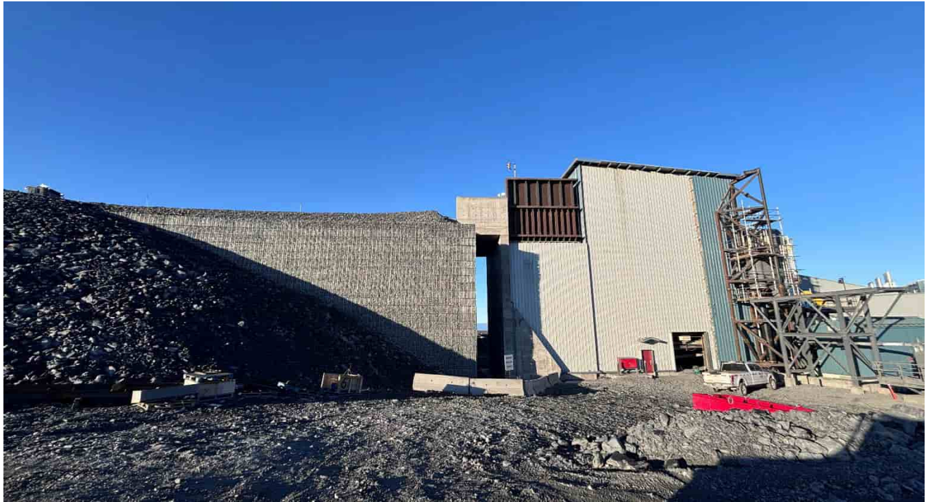
G-325: MSE wall eastern side and crusher, looking W
