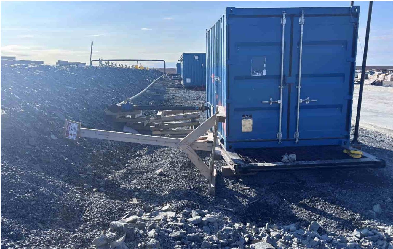
G-376: Looking S along toe of berm between fuel transfer / refueling and tank farm
