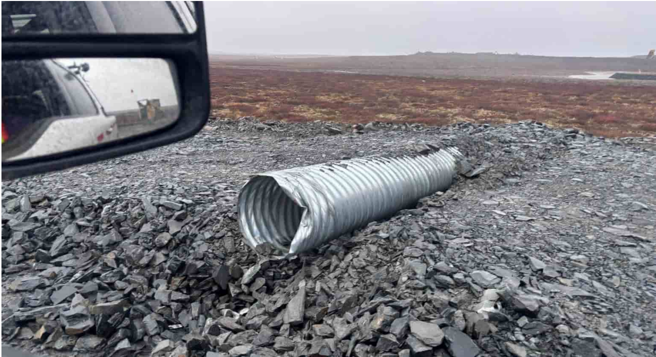
G-441: Exposed culvert, looking N (noting location for consideration when advancing Phase w of SWP)
