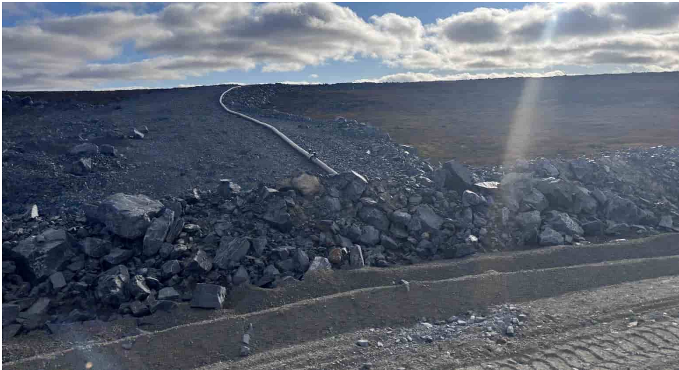
G-242: Pipeline crossing under road, looking S
