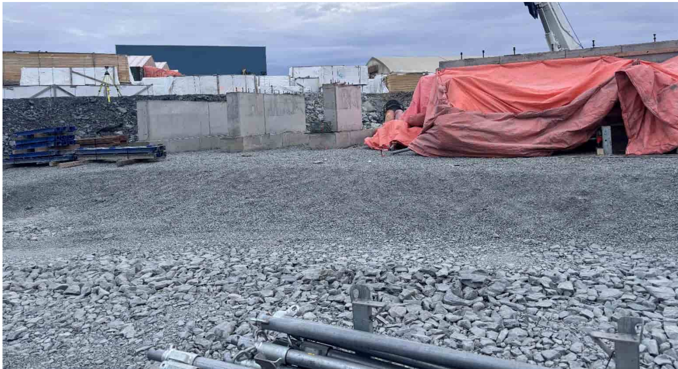
G-303: Laydown area beside vent raise
