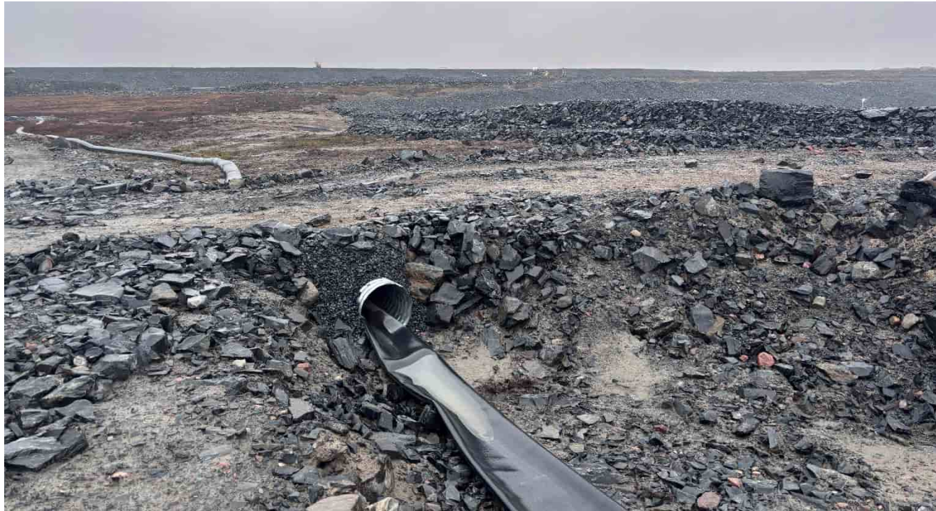
G-448: Culvert under access road to Umwelt Pit from SWP Access Road, looking NE
