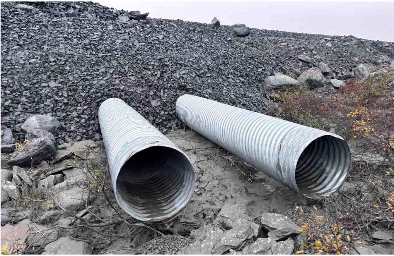
G-396: Twin culverts outlet
