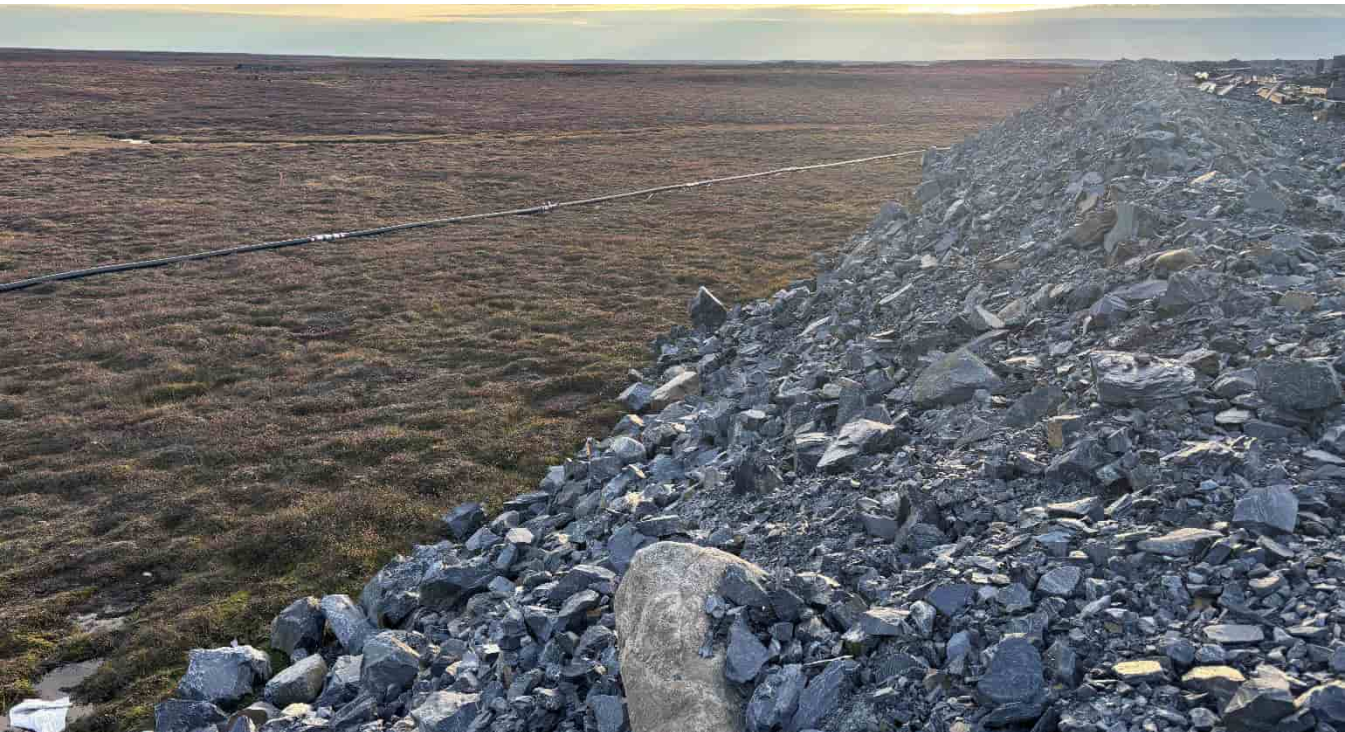
G-283: Southern pad slope, looking W – pipeline on tundra beyond toe
