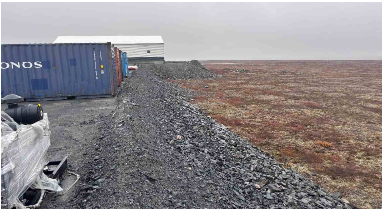
G-435: Eastern pad slope, looking N
