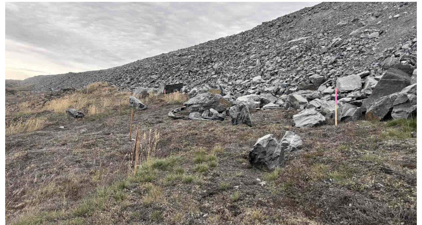
G-251: Downstream slope of All-weather road. Area marked where some drainage through rockfill or slope relaxations and some coarser material roll out previously noted
