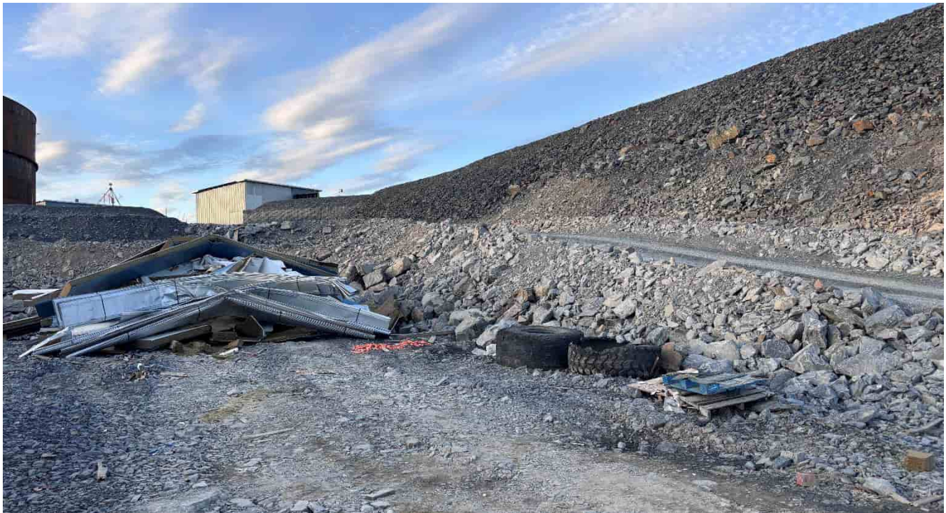
G-329: MSE wall and approach road, looking N from laydown area
