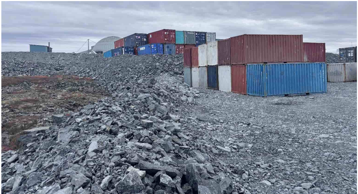
G-386: Laydown area SE pad slope, looking SW
