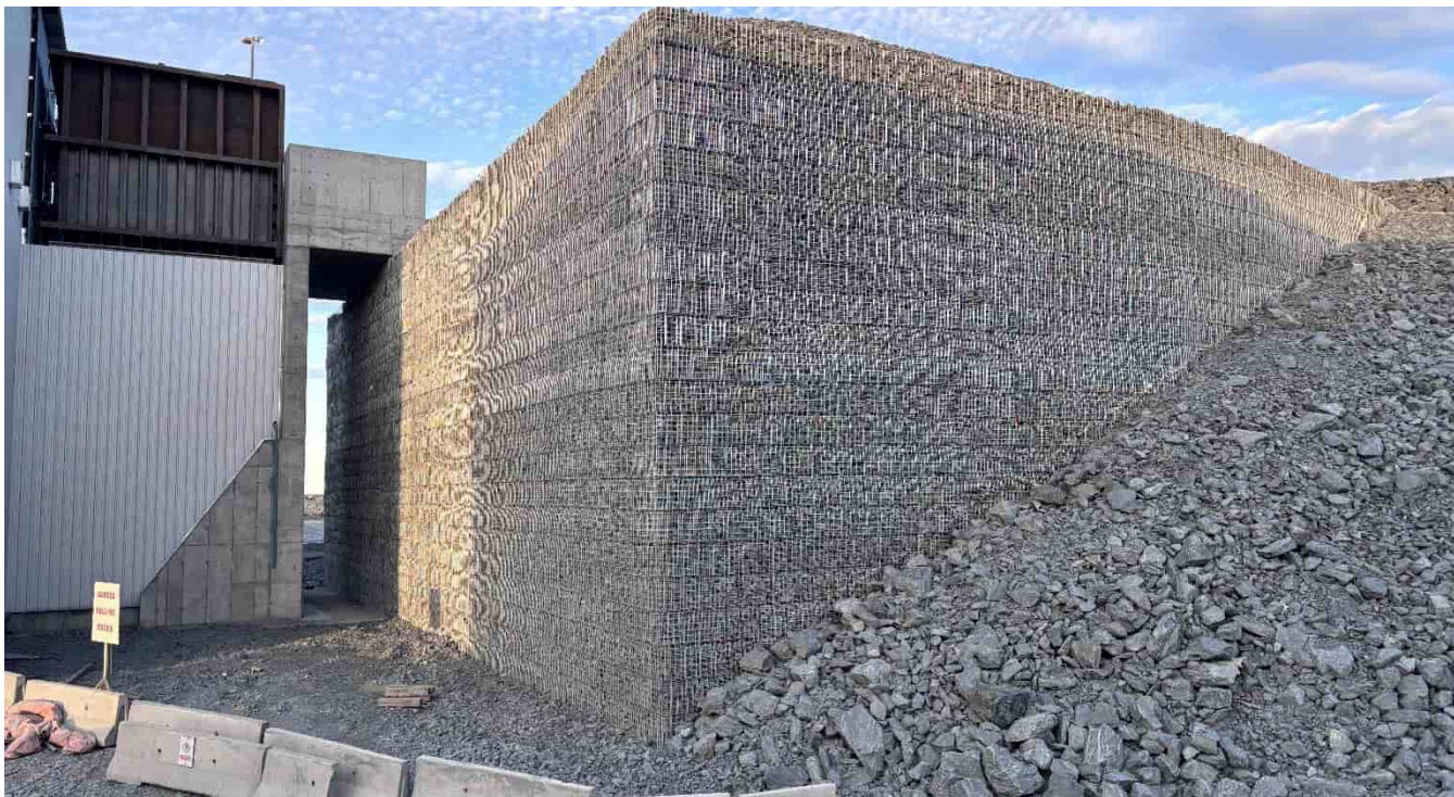
G-323: MSE wall W corner, looking E
