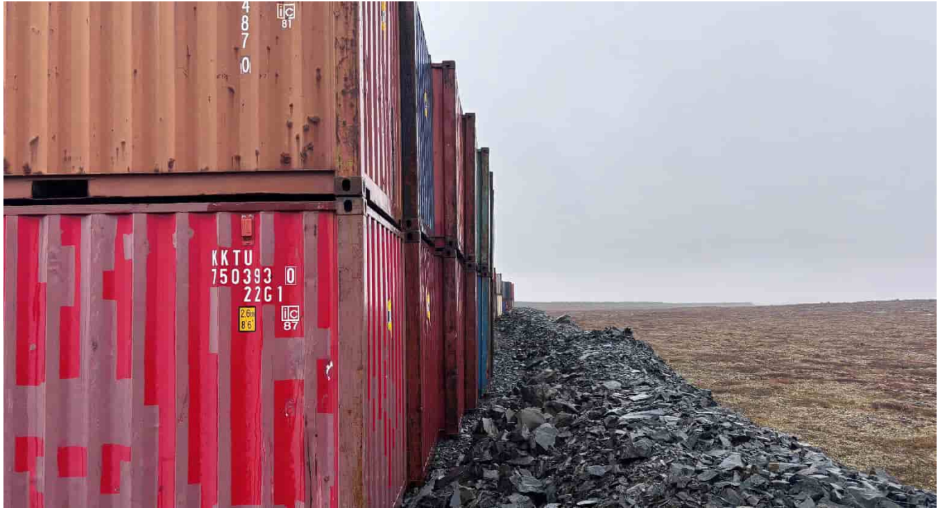
G-429: Northern slope of laydown pad, looking W
