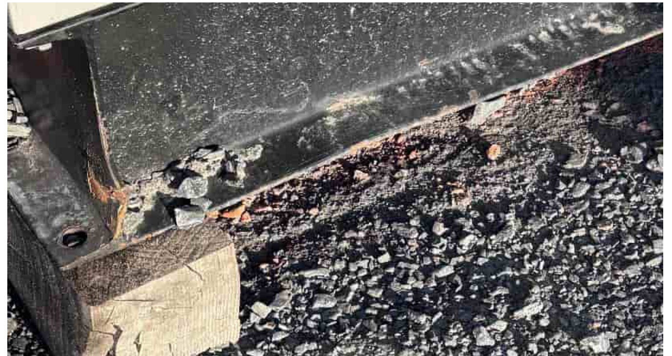
G-268: Camp pad, example support below ancillary structures (beyond main camp trailers / accommodation). Watch for planning maintenance
