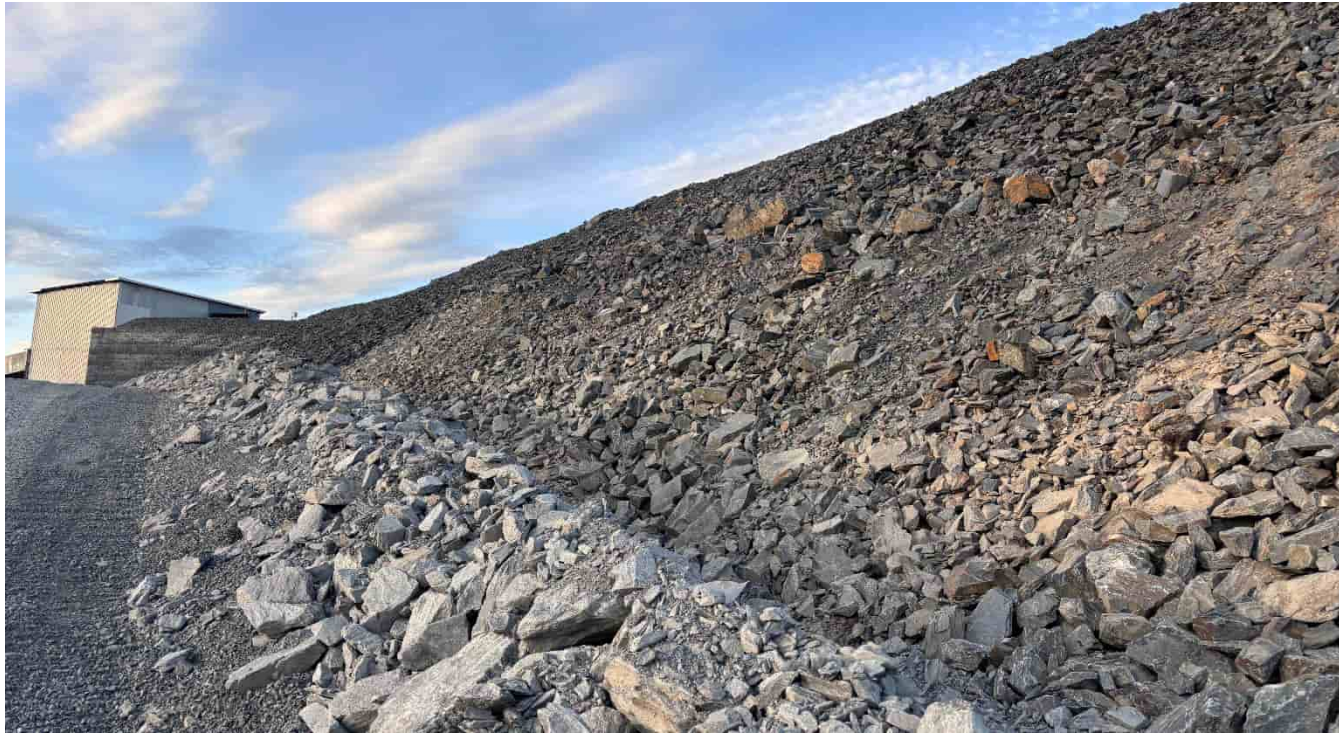
G-321: Slope approaching MSE wall, looking N
