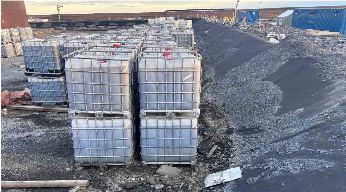
G-347: Tote storage area and western berm, exposed geotextile
