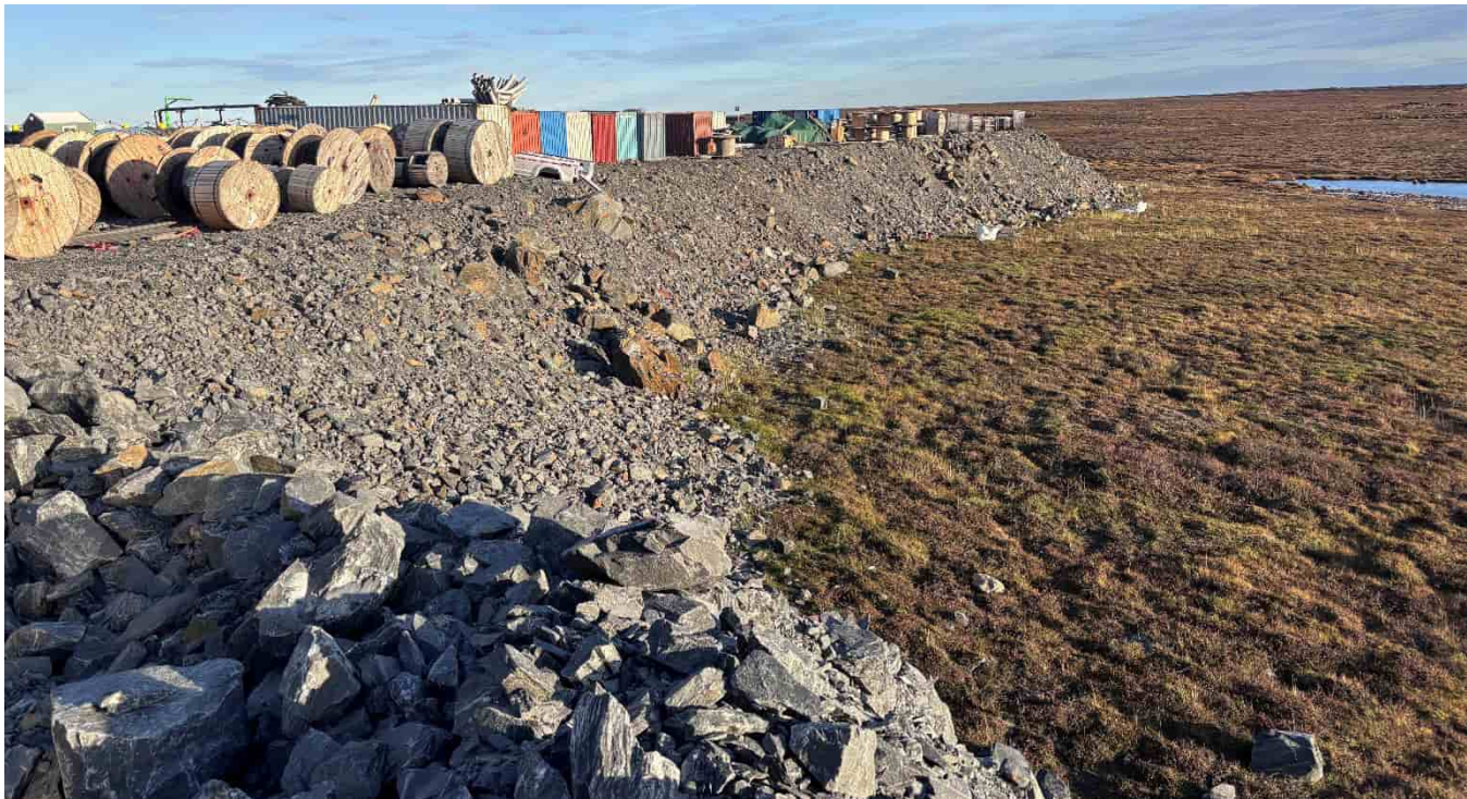
G-278: Pad slope beside laydown on western pad edge
