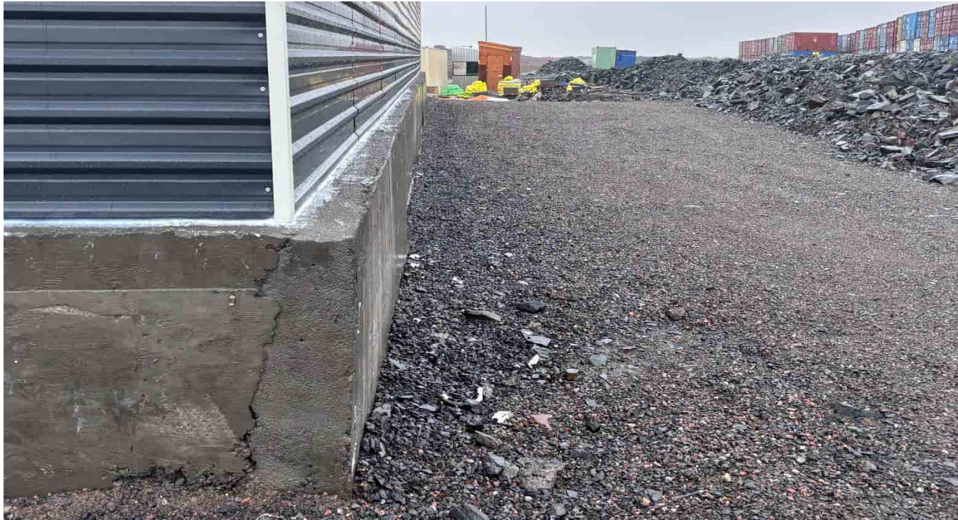
G-437: Building foundation, looking W
