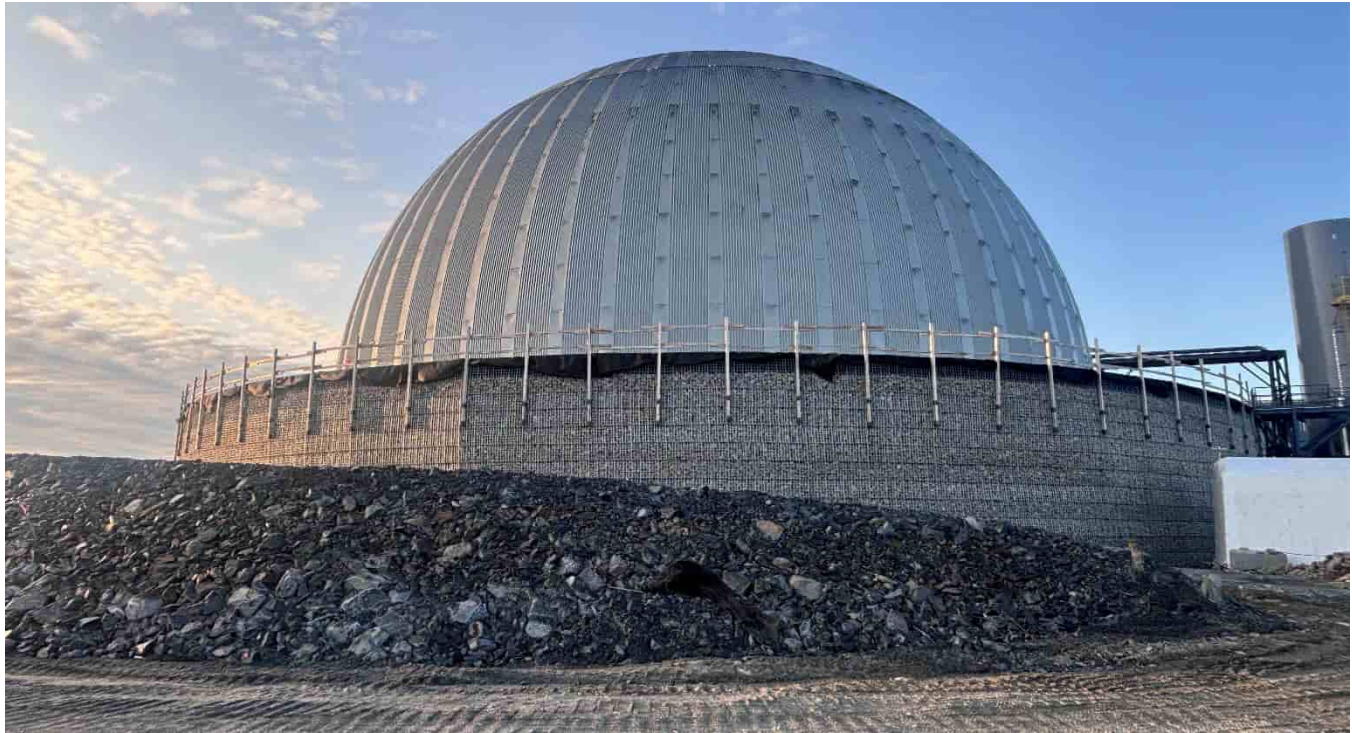
G-310: Ore dome MSE wall, looking S
