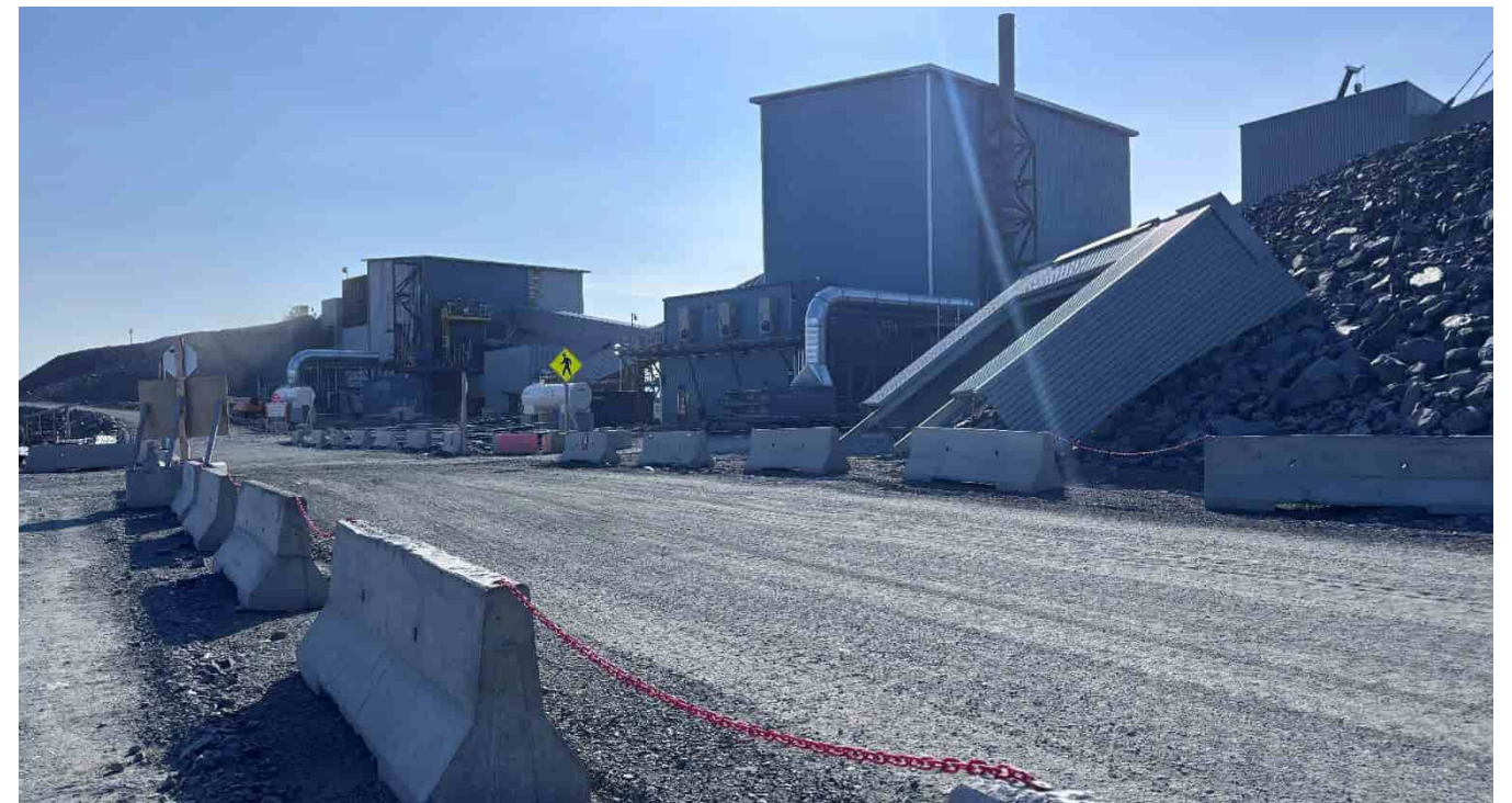
G-295: View towards crusher from road, looking S – area under construction at time of inspection
