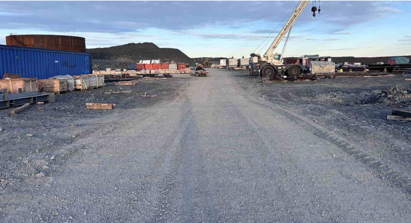
G-281: Laydown area and road S of tank farm, looking E
