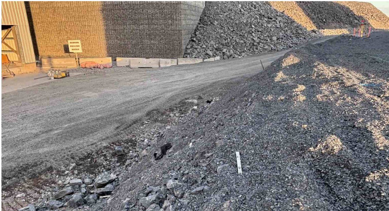
G-332: Slope across from crusher MSE wall
