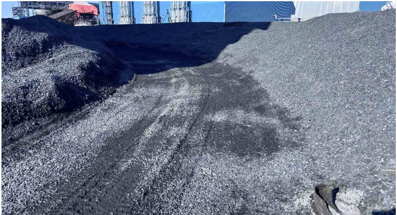
G-367: Tank farm access road, looking NW
