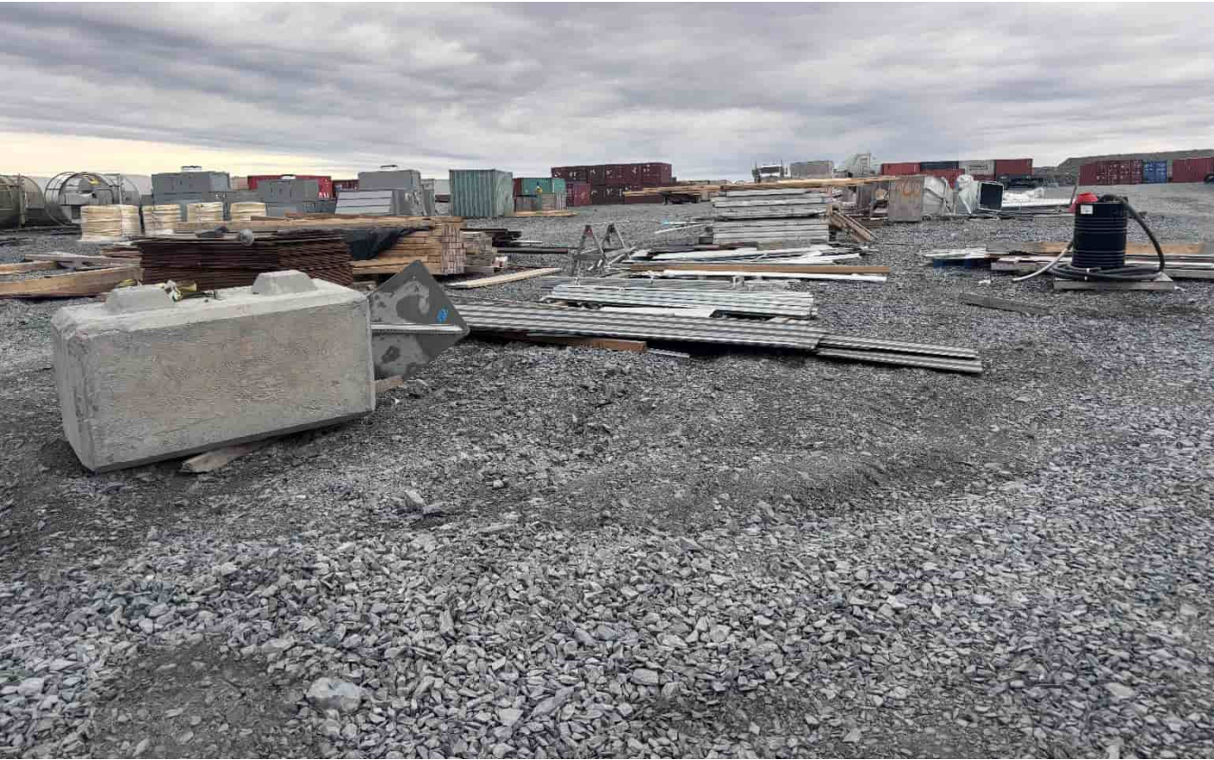
G-389: Laydown area, looking SE
