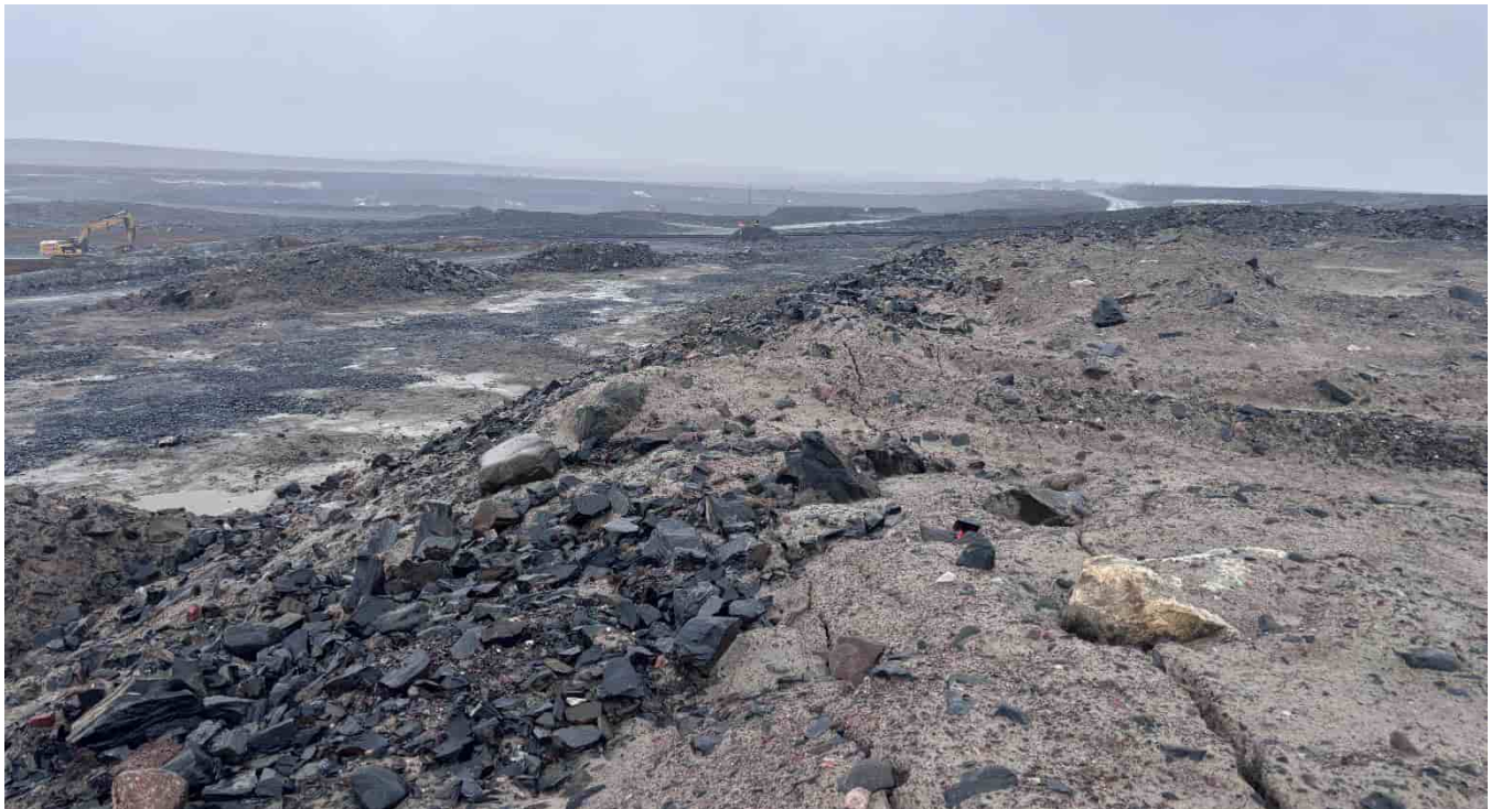
G-400: Stockpile, looking N – cracking closer to top crest near slopes
