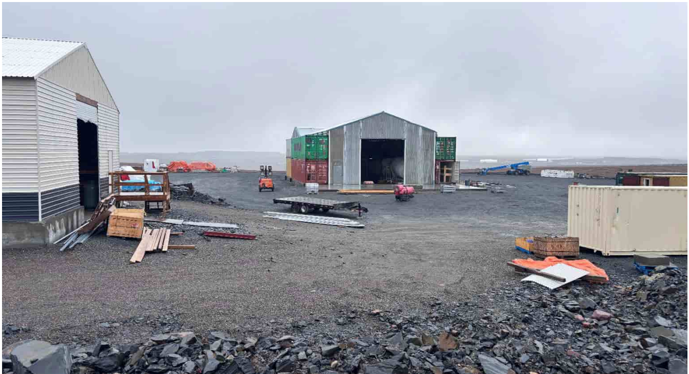
G-431: Emulsion plant general view, looking S
