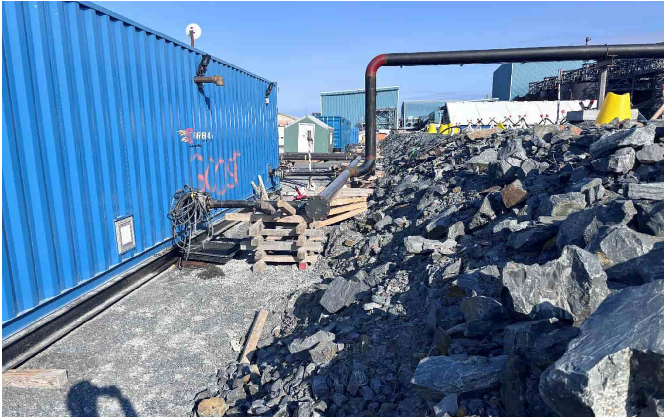
G-383: Looking N along toe of berm between fuel transfer / refueling and tank farm
