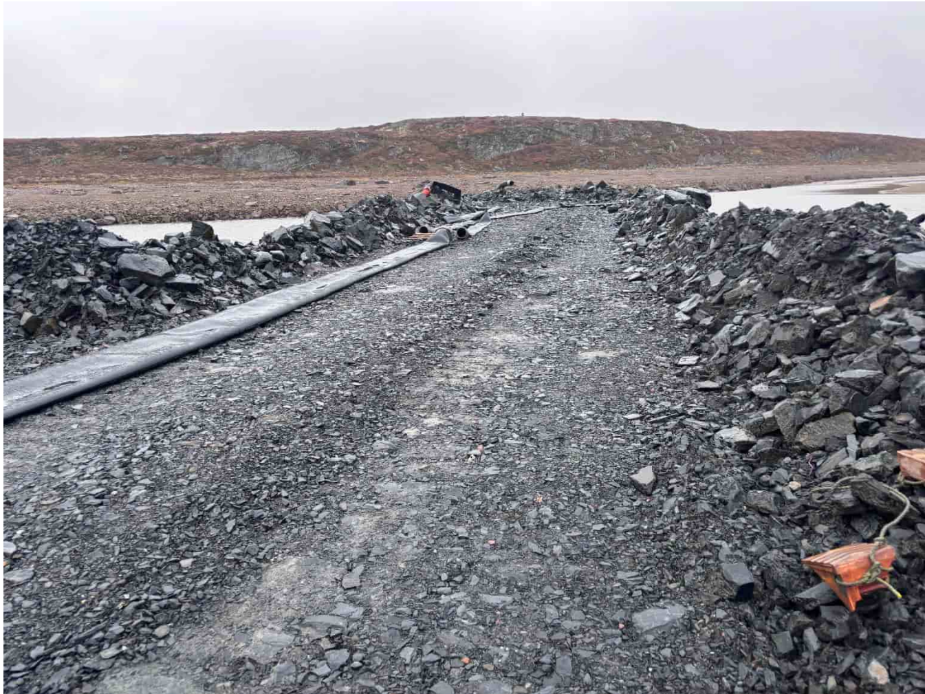
G-452: Northeast pond (Round Pond) access road, looking W
