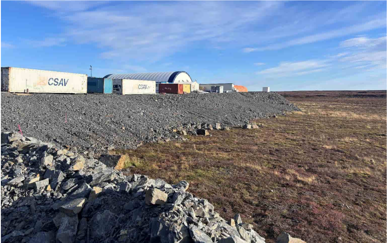
G-263: Camp pad W slope, looking SE
