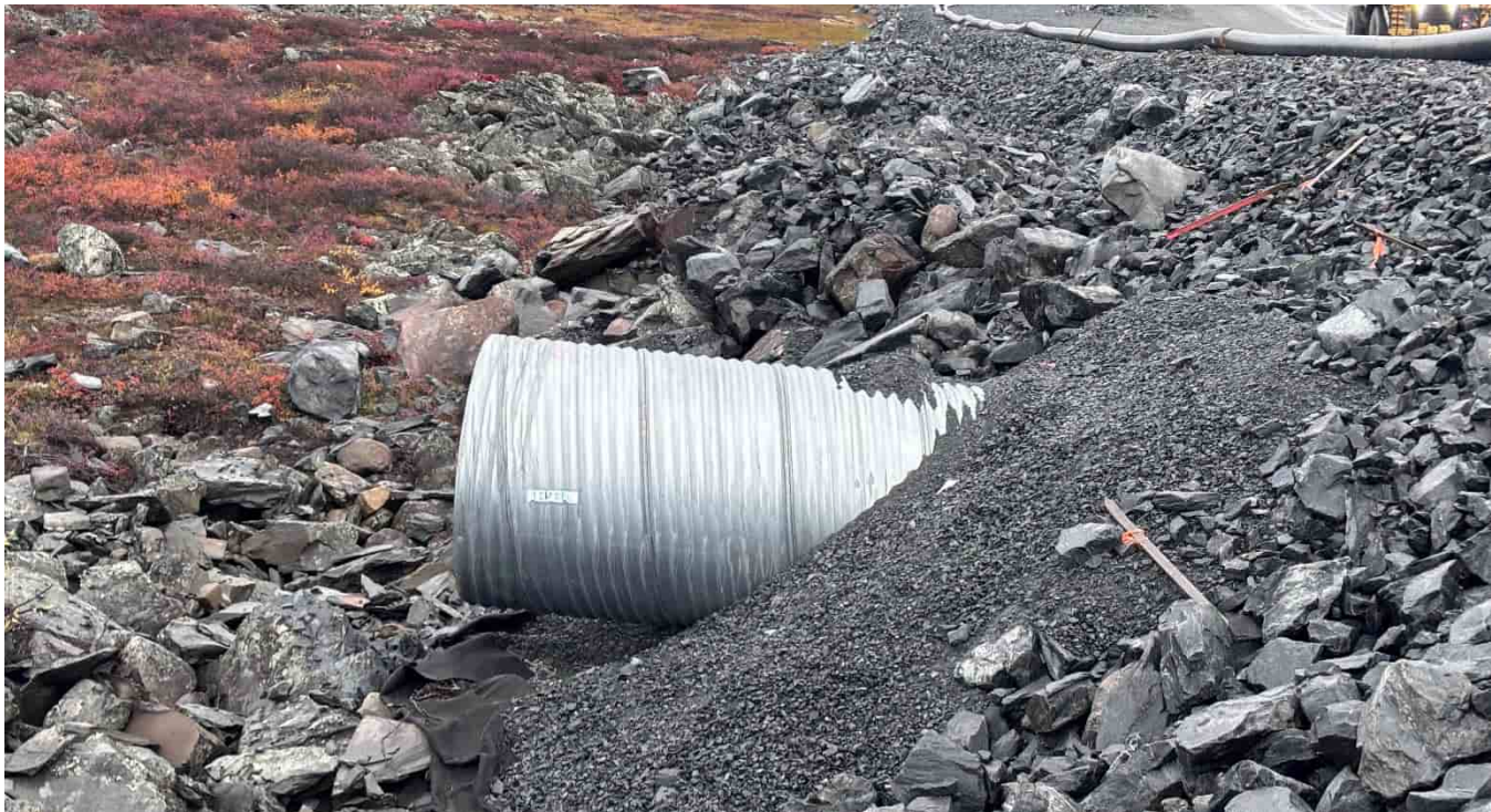
G-393: Northern culvert inlet, looking N
