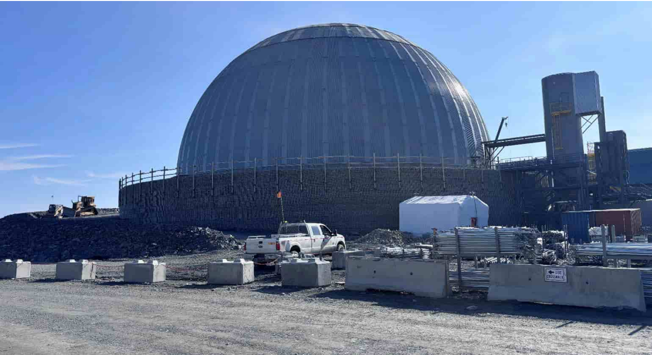
G-297: View towards ore dome from road, looking SE
