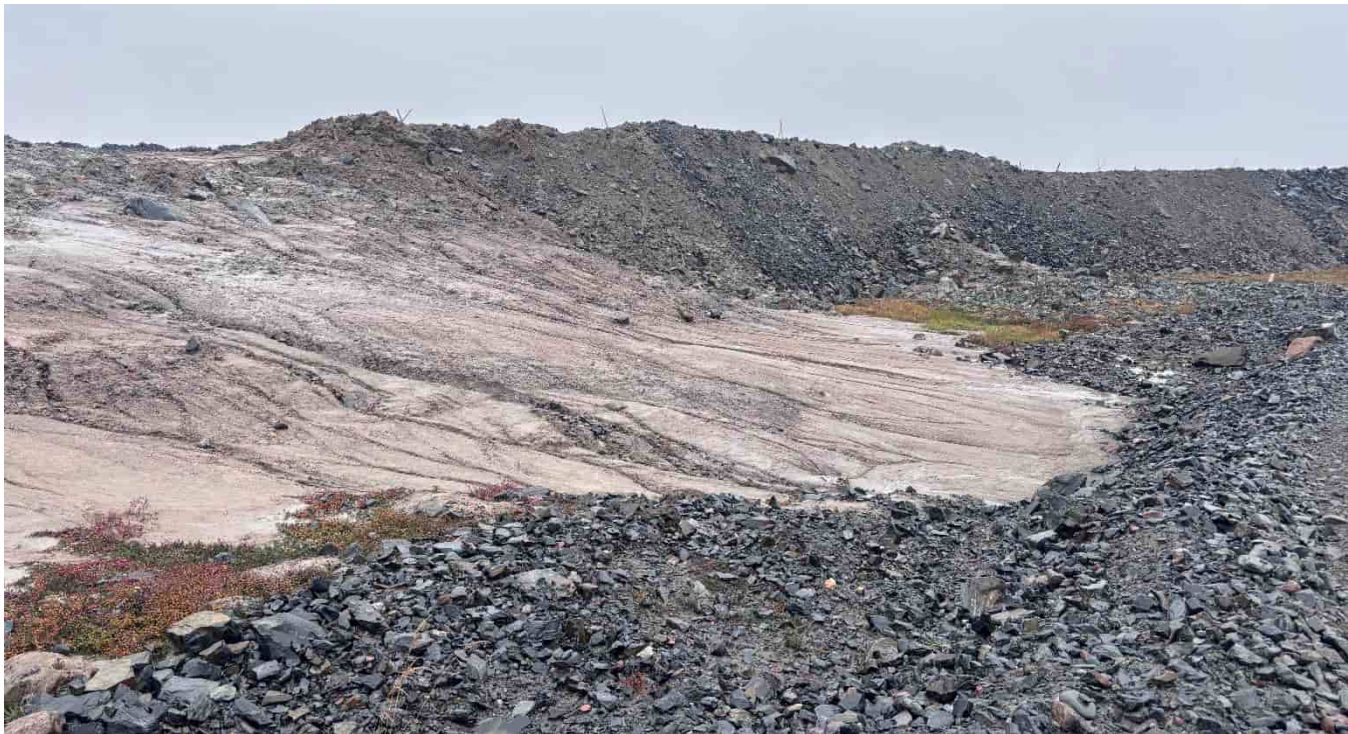
G-408: Stockpile beside road corner and northern pad slope thaw and erosion of overburden material (expected with this type of material when left exposes)
