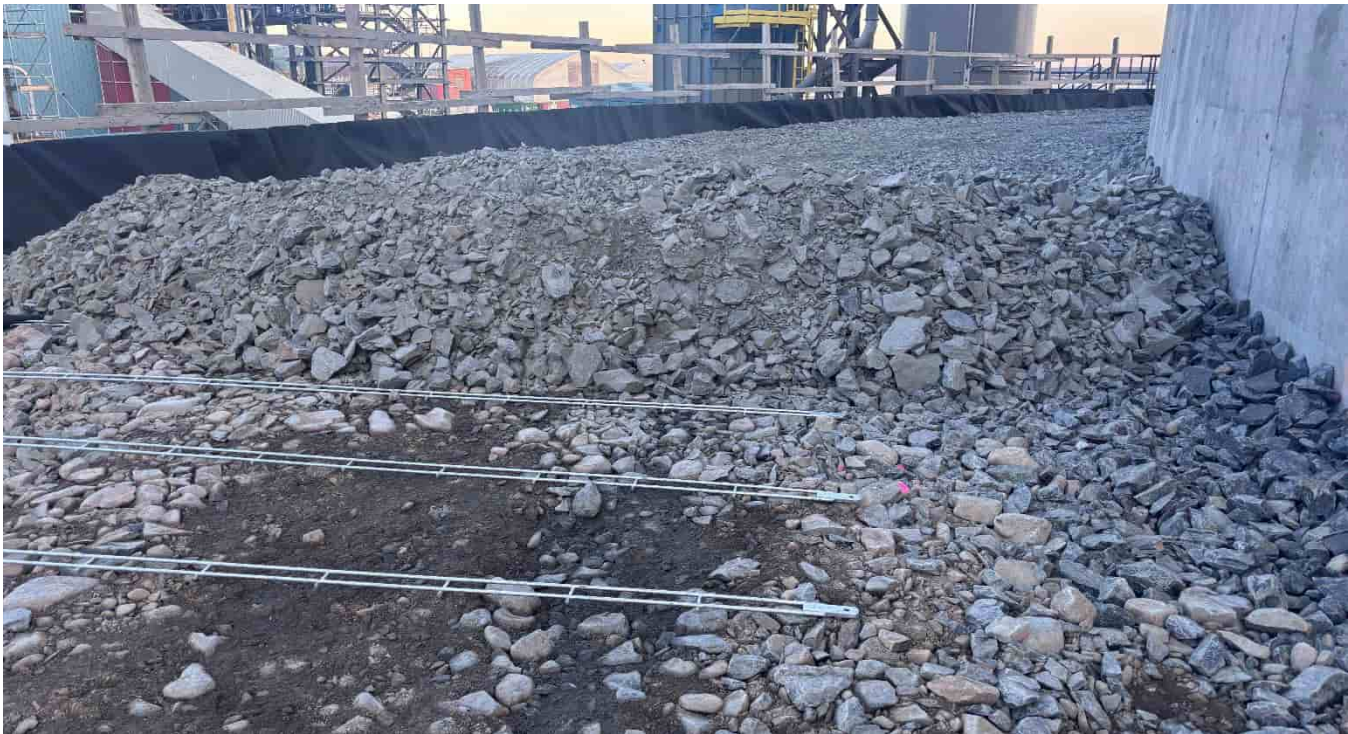
G-316: MSE wall reinforcing example – construction in porogress
