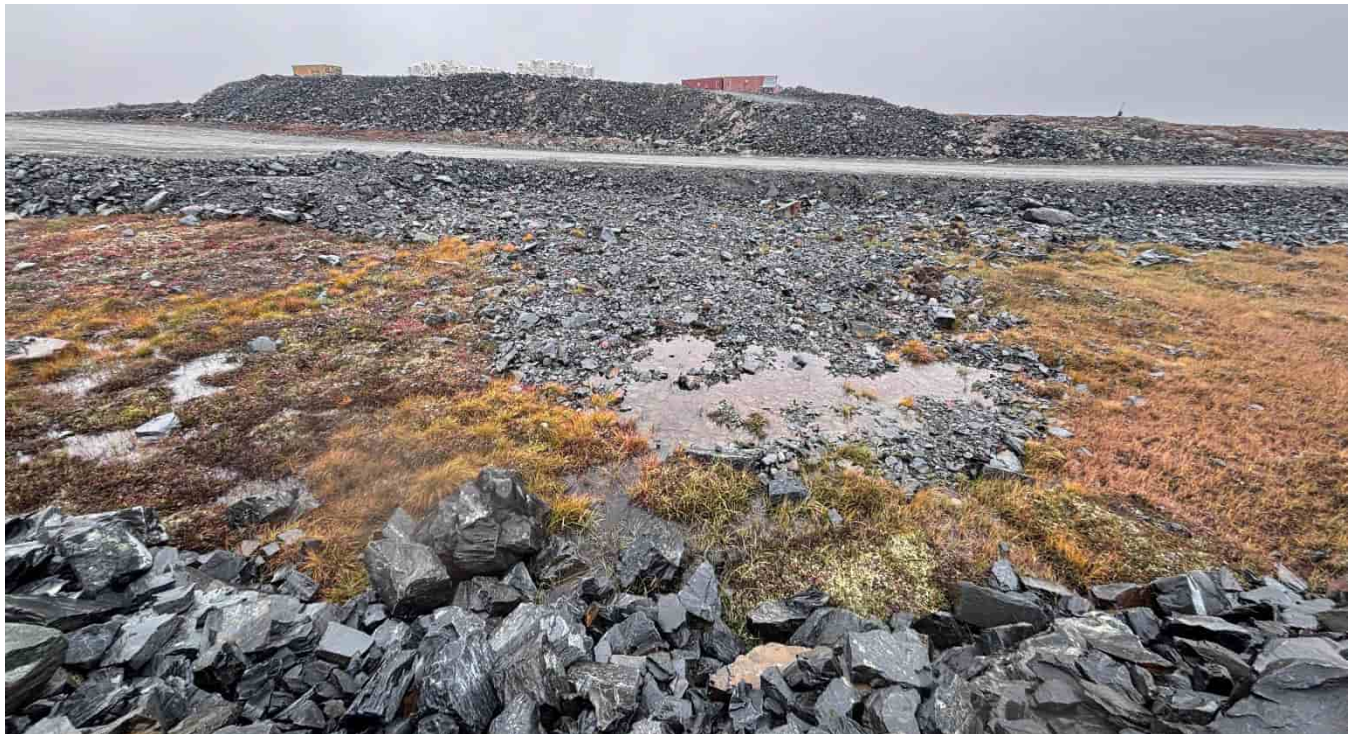
G-412: Toe of rock storage area eastern slope, looking E
