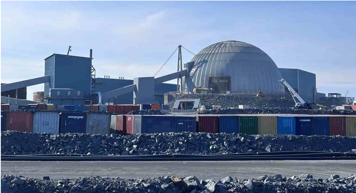
G-289: Overall view towards ore dome and plant area from the berm between the All-Weather Road and contact water pond
