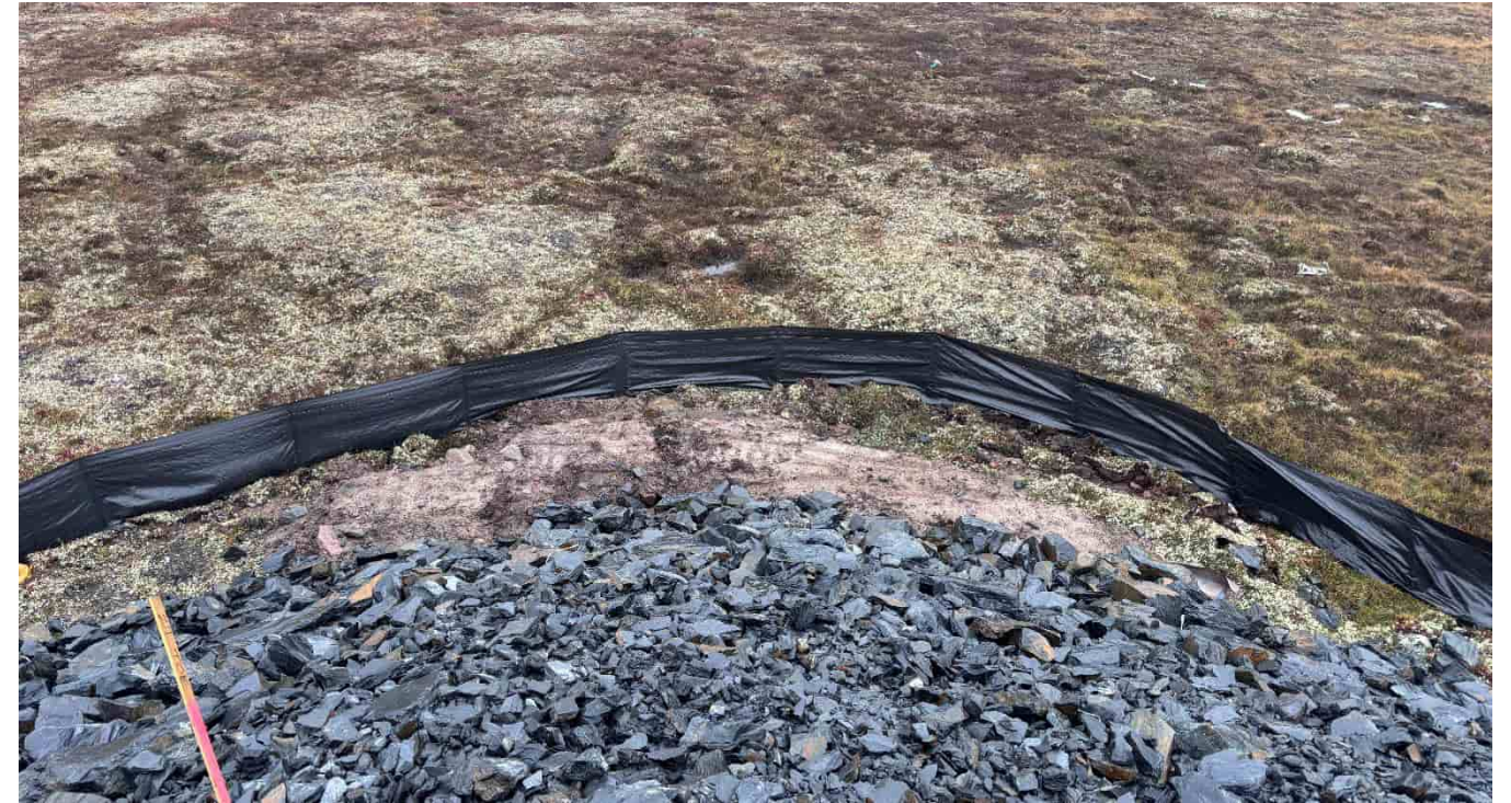
G-434: Silt fencing at SE corner of pad
