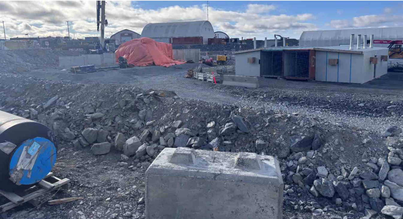
G-305: Looking S towards scaffolders and ironworkers area
