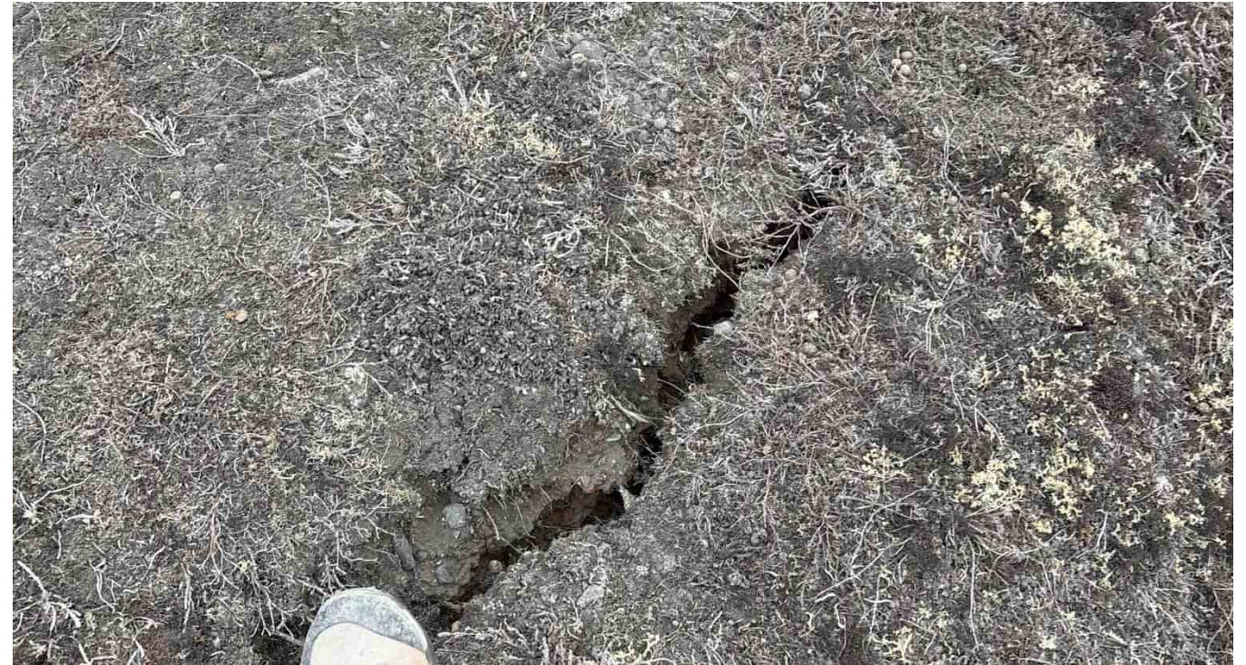
G-253: Tundra near toe of rock fill – settlement to be expected near toes
