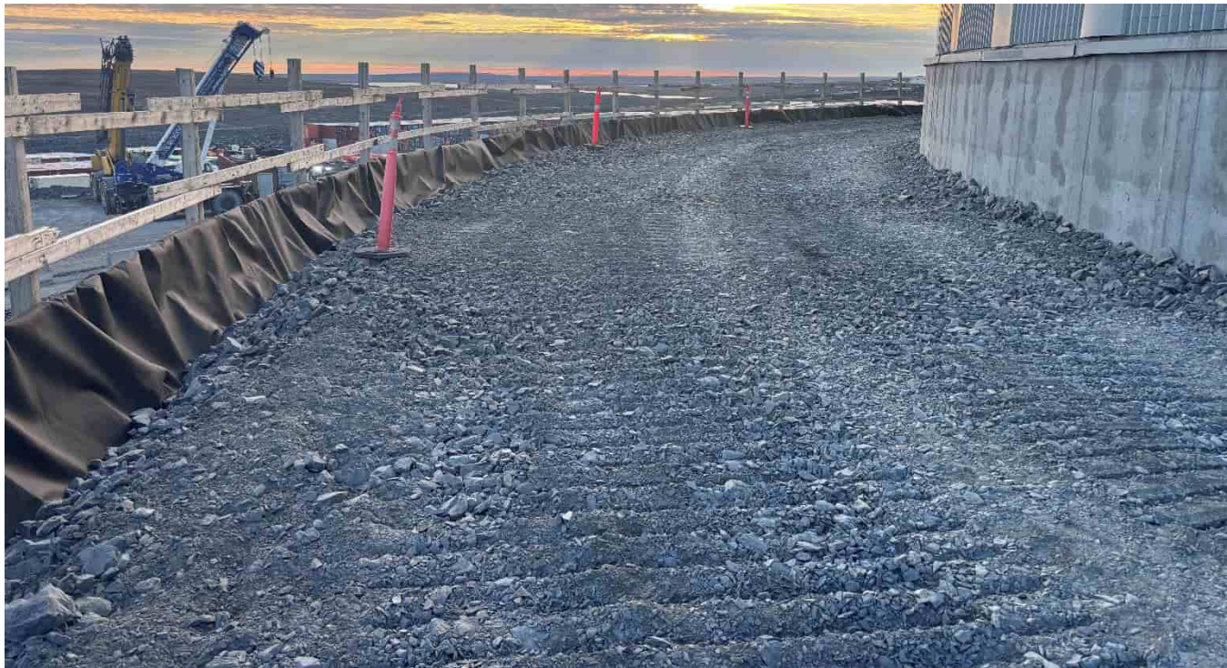
G-315: Typical MSE wall finished construction – construction in progress
