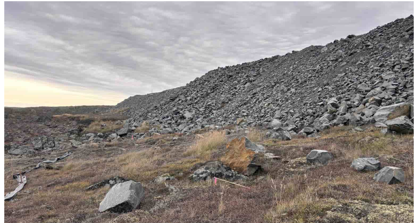
G-255: Road rockfill, looking E – Historic silt fencing at toe
