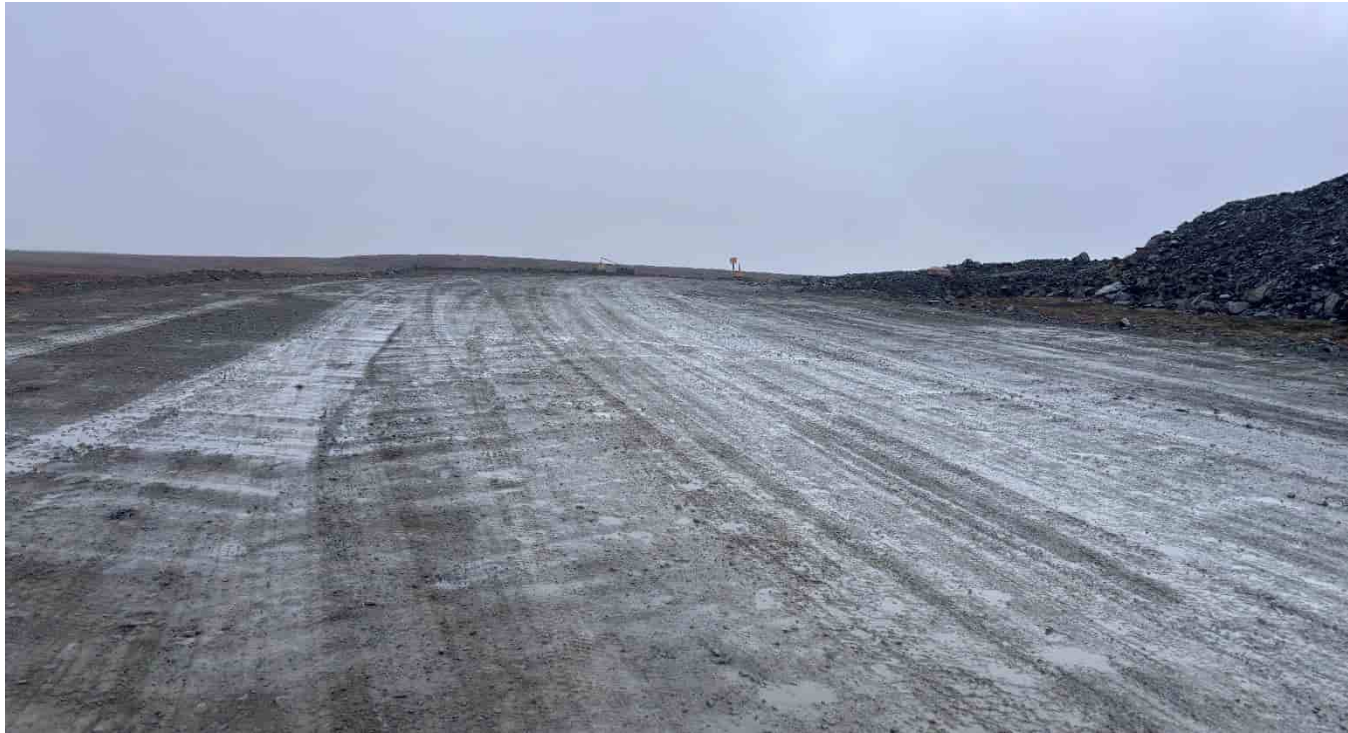
G-423A: Explosives area access road, looking N
