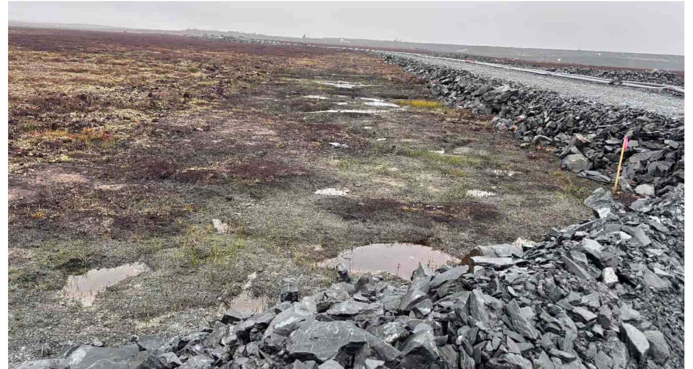
G-445: SWP Dam Access Road
