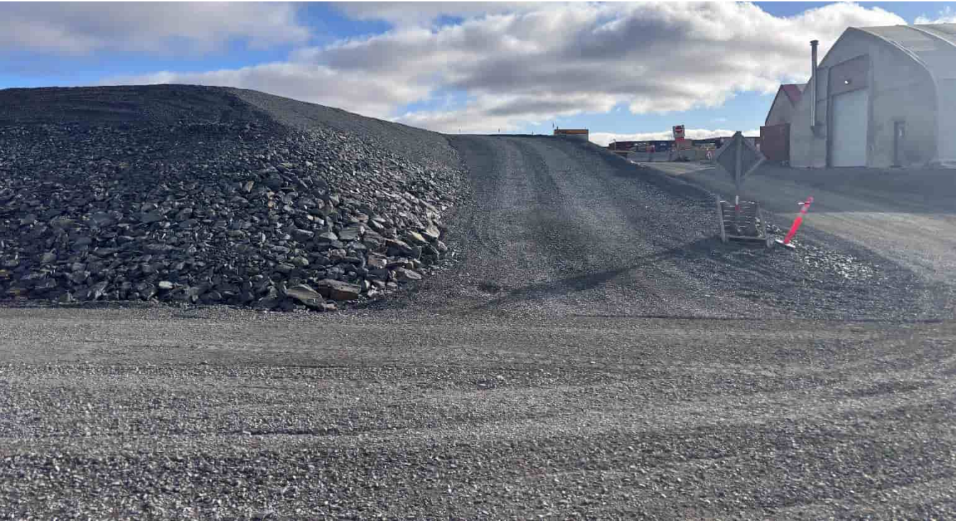
G-241: Entrance to tote storage and operations area – Looking S from All-Weather Road
