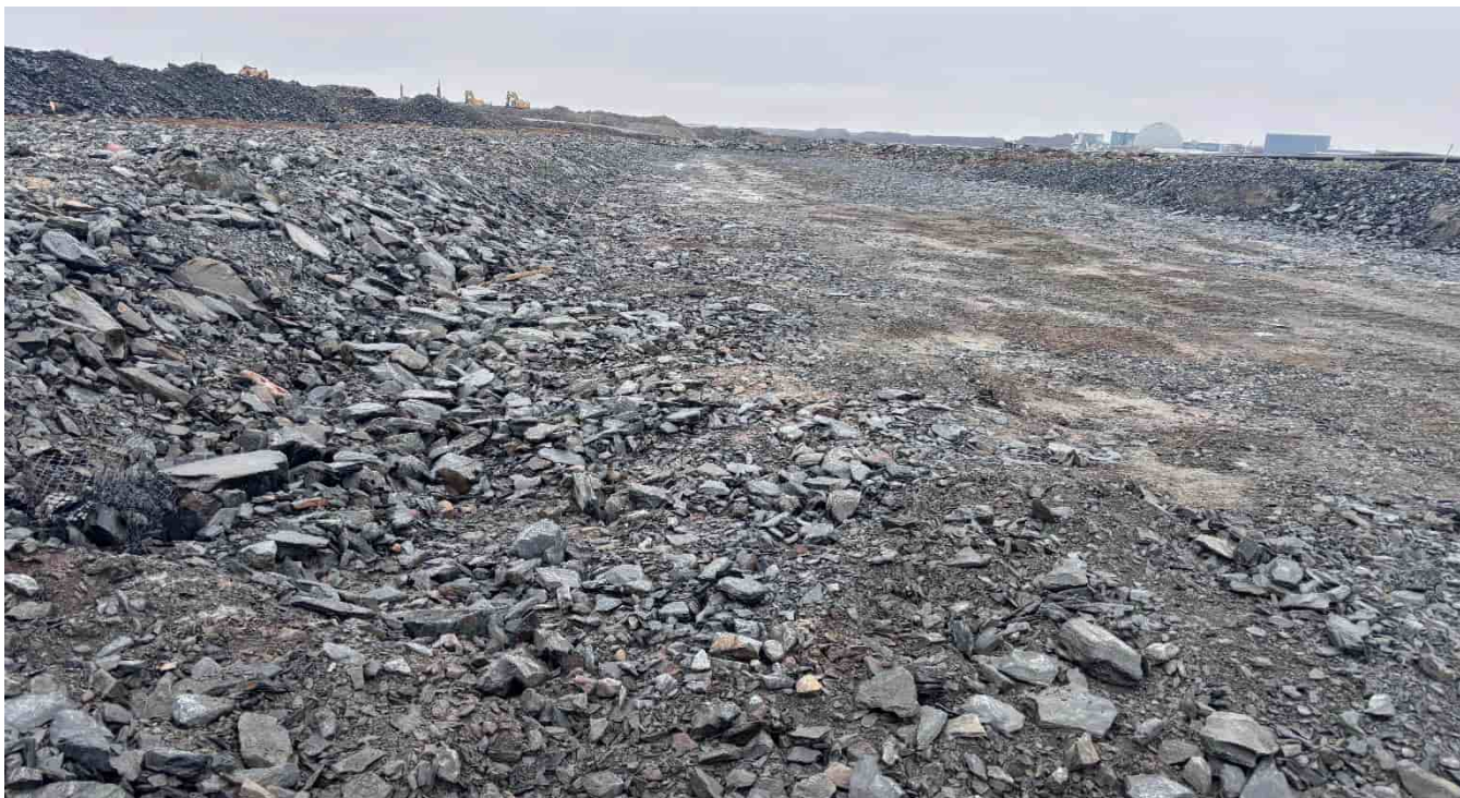
G-460: Spillway, looking SE
