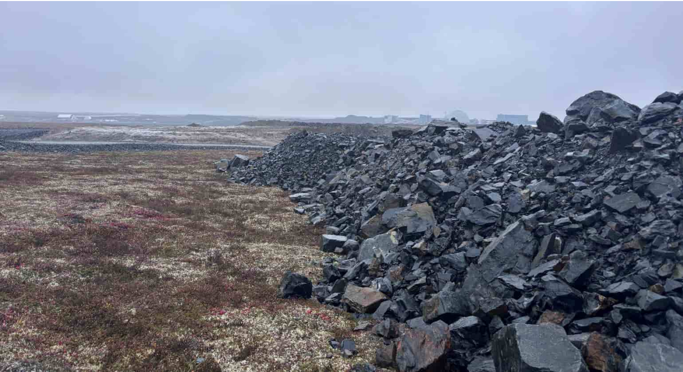
G-411: Eastern pad slope, facing S
