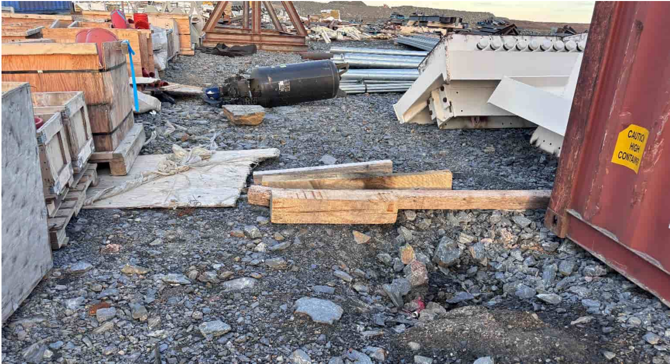
G-285: Settlement of laydown area near edge of seacan
