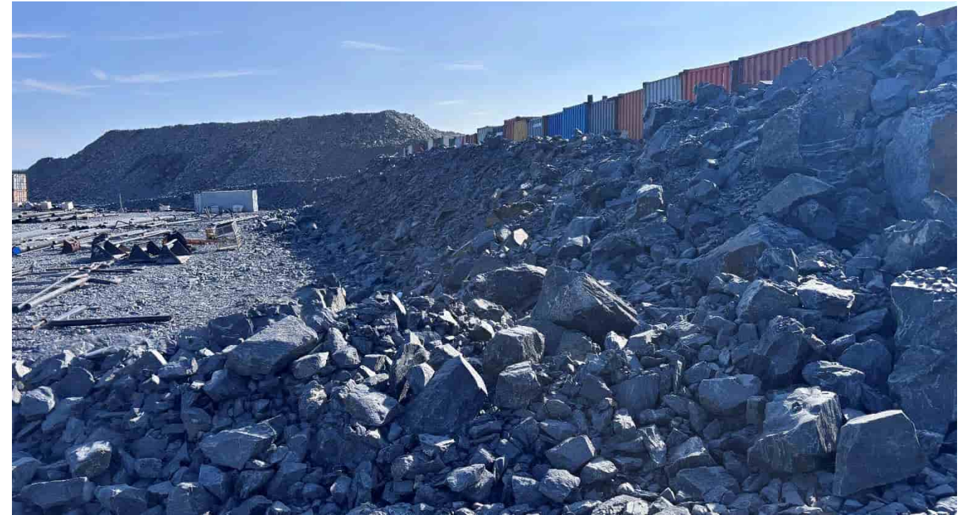
G-293: Laydown area berm, looking SE
