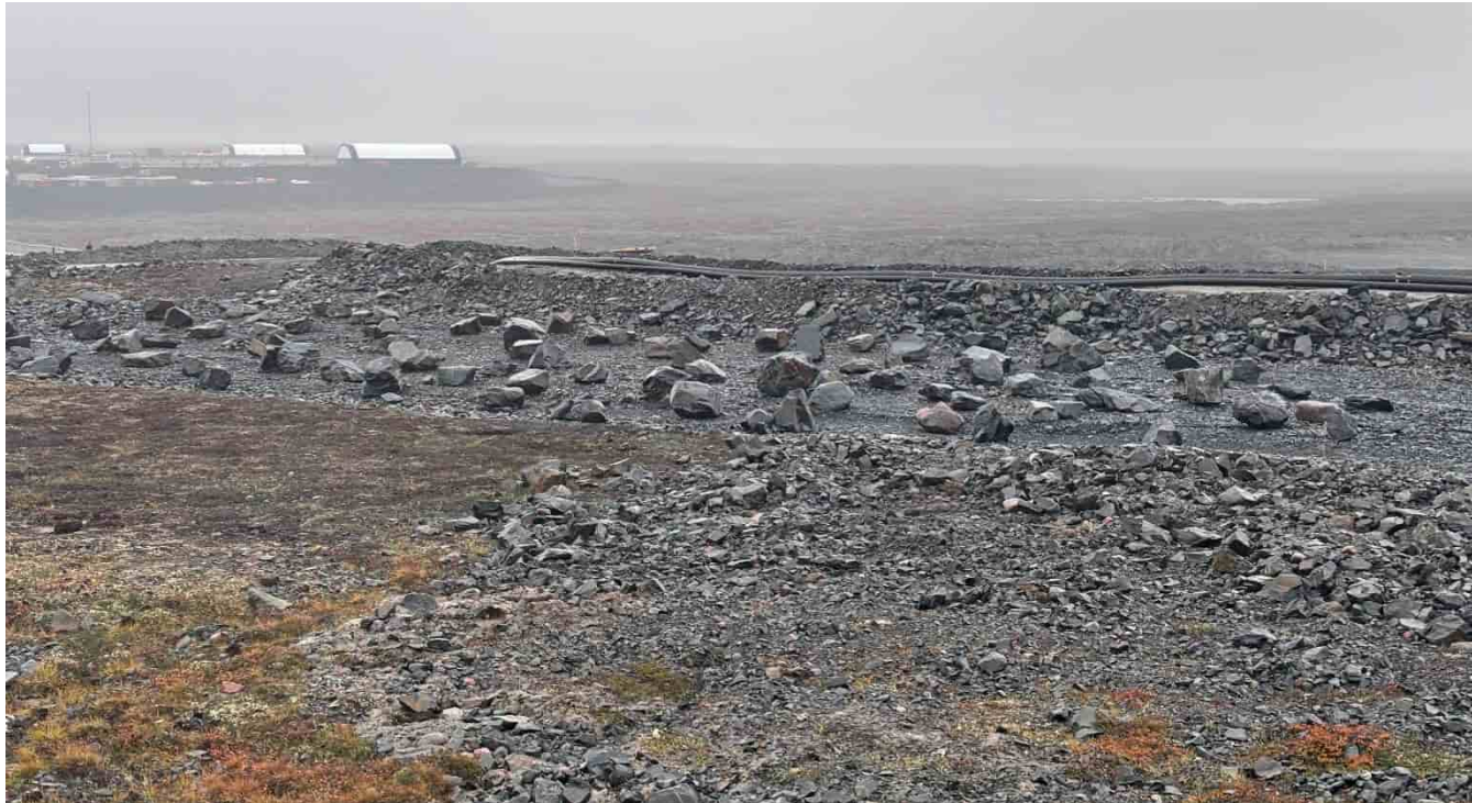
G-458: Looking W towards downstream (SE) end of spillway
