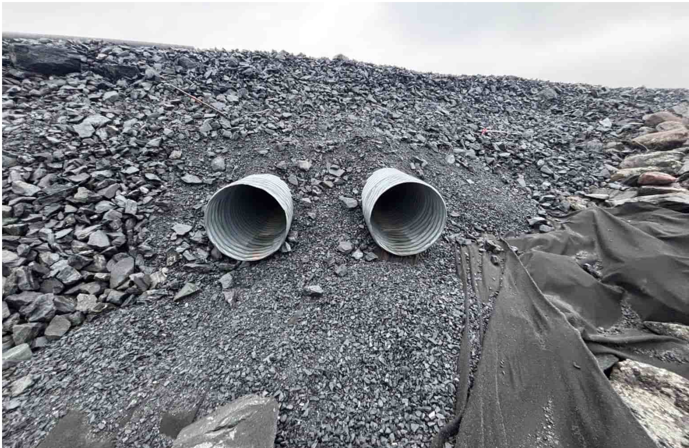
G-395: Twin culverts inlet
