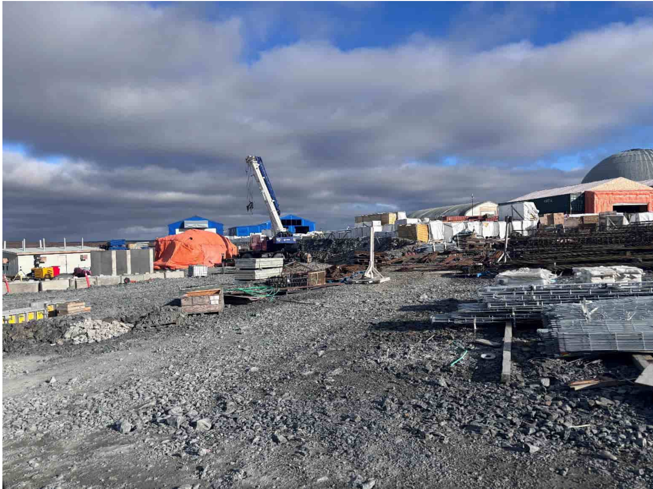
G-308: Laydown area beside site services, looking E
