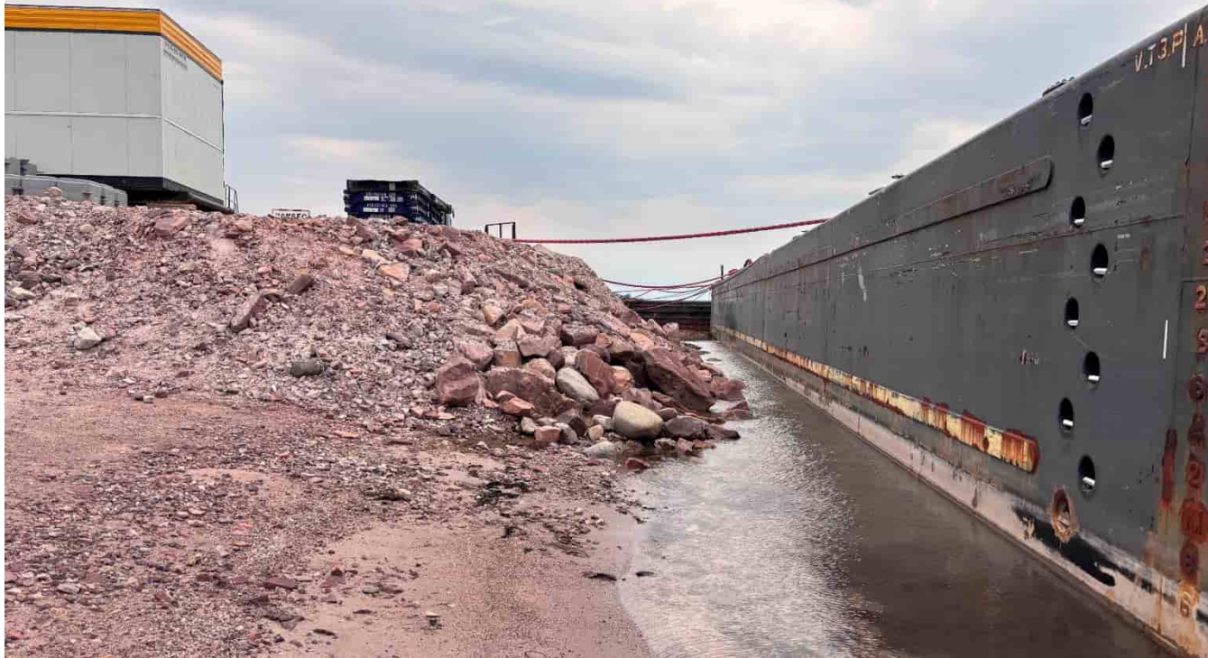
M-21: Barge access and tie off
