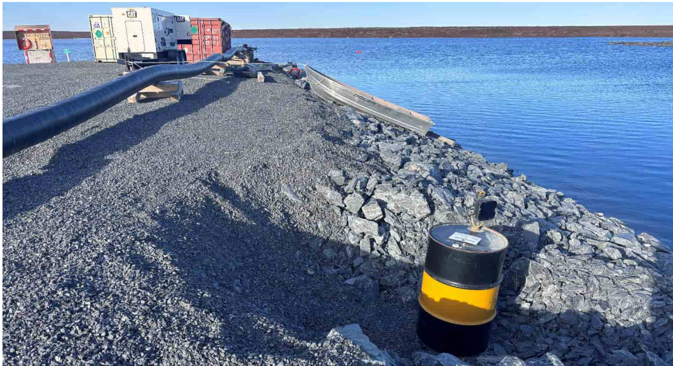
G-477: Reclaim Pipeline access road and pad
