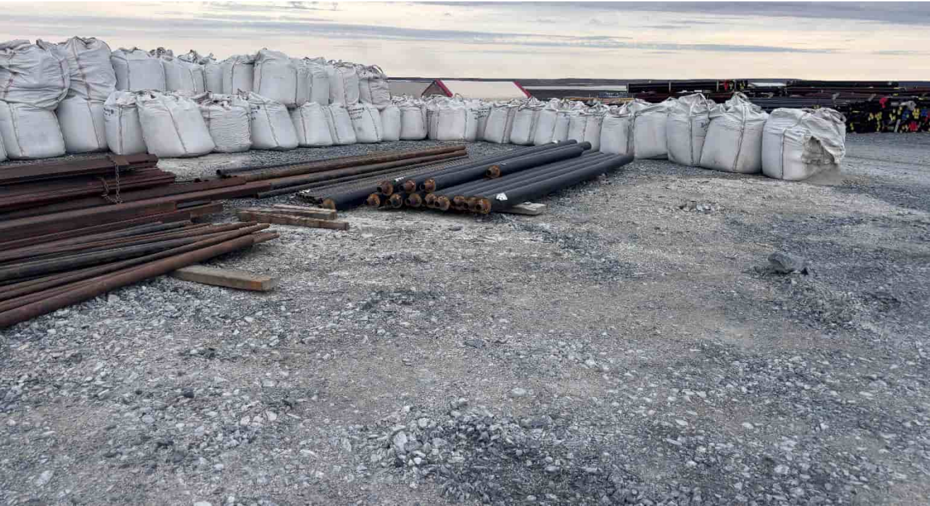
G-512: Cement and pipe laydown
