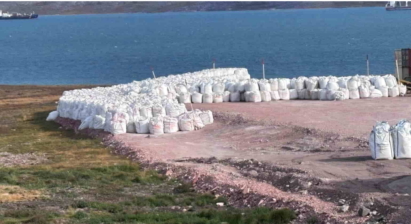
M-8: Cemented rockfill laydown at N side of pad. Temporary bag placement close to pad slope
