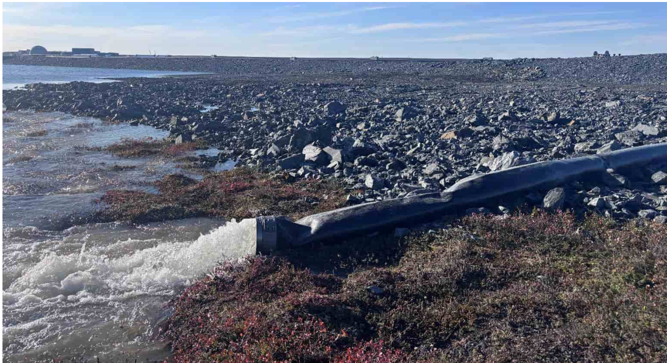
G-464: Discharge into N side of primary pond at unfavourable locations (in terms of increased potential for thermal degradation within pond footprint), looking SW (this was corrected / moved)
