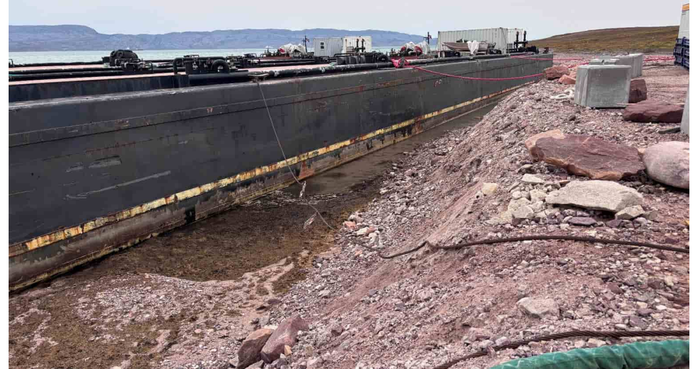
M-22: Shoreline pad slope above water
