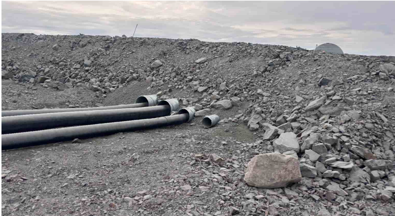
G-507: Tailings pipeline crossing under ROM stockpile western access road, looking SW
