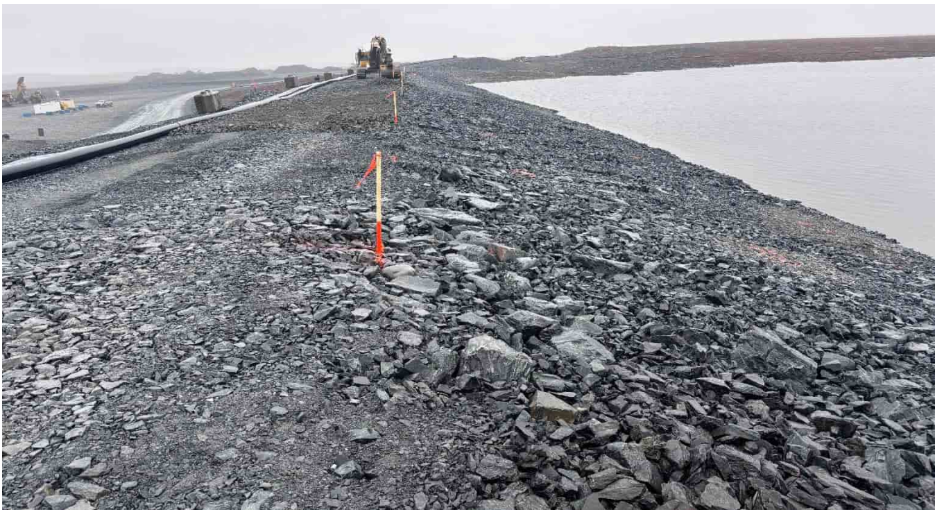
G-480: Upstream crest of dam, looking N
