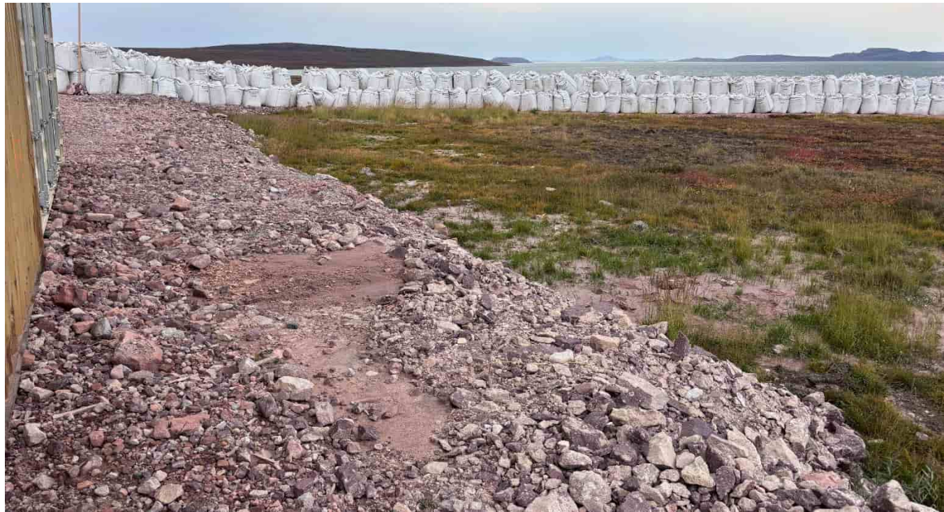
M-28: Pad slope, looking NW towards temporary cement bag storage / laydown
