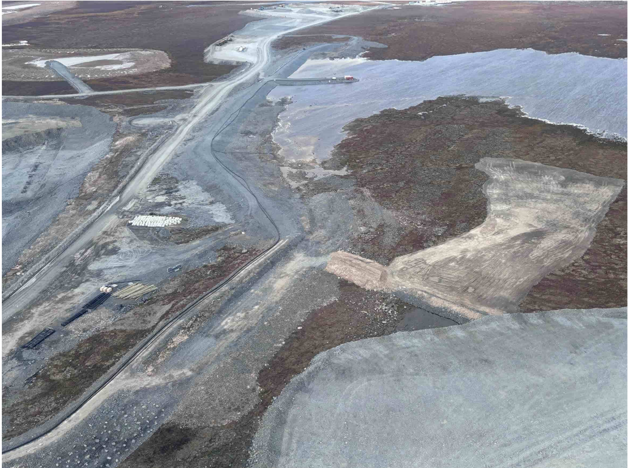
Heli Photo 5: Primary Pond, dam, and spillway, looking NW
