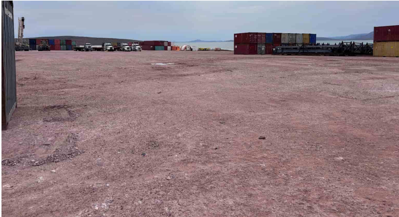
M-13: Laydown area surface conditions, looking N
