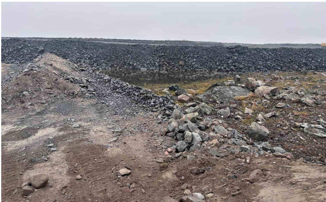
G-487: Ponding water beside overburden fill at Umwelt WRSA. The ponded water was filled to minimize future ponding in area.
