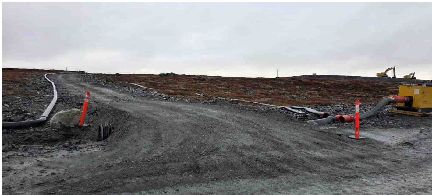
G-506: Culvert under northern access road to Primary Pond, looking E from the All-Season Road
