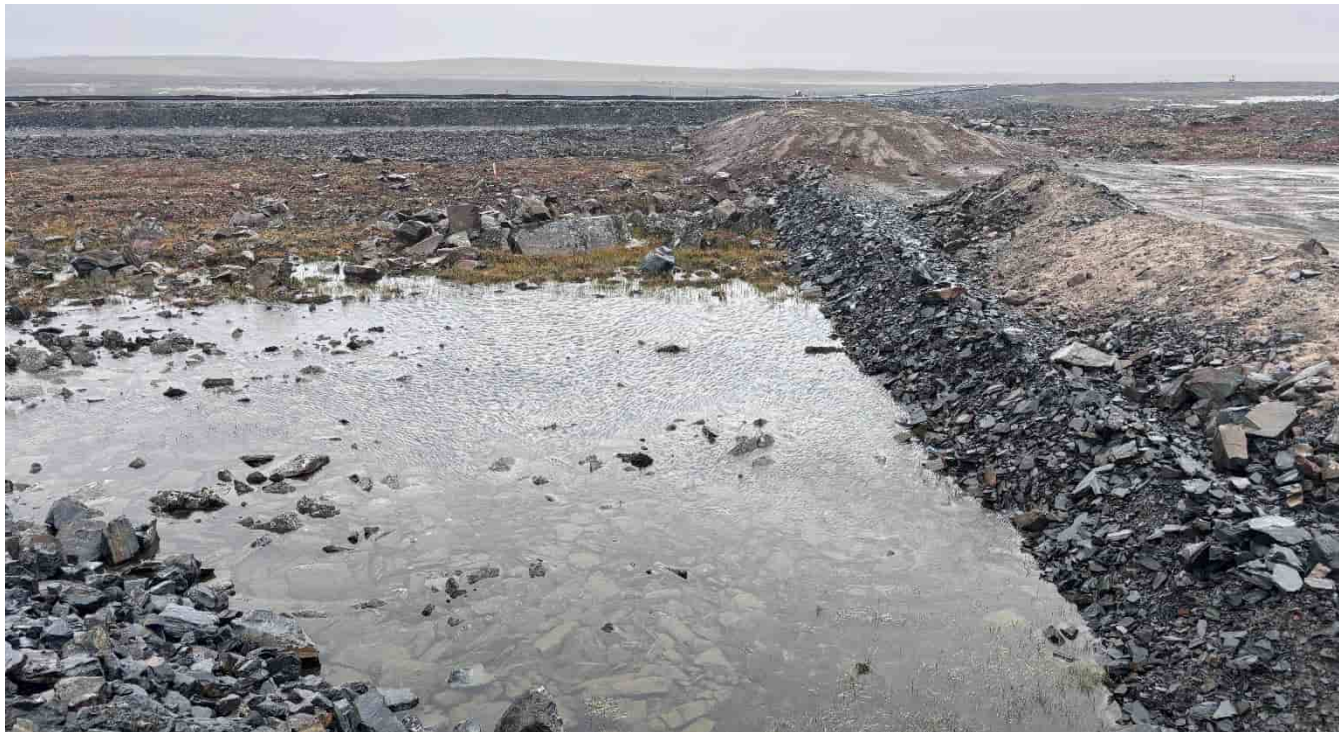
G-490: Ponding south of overburden fill
