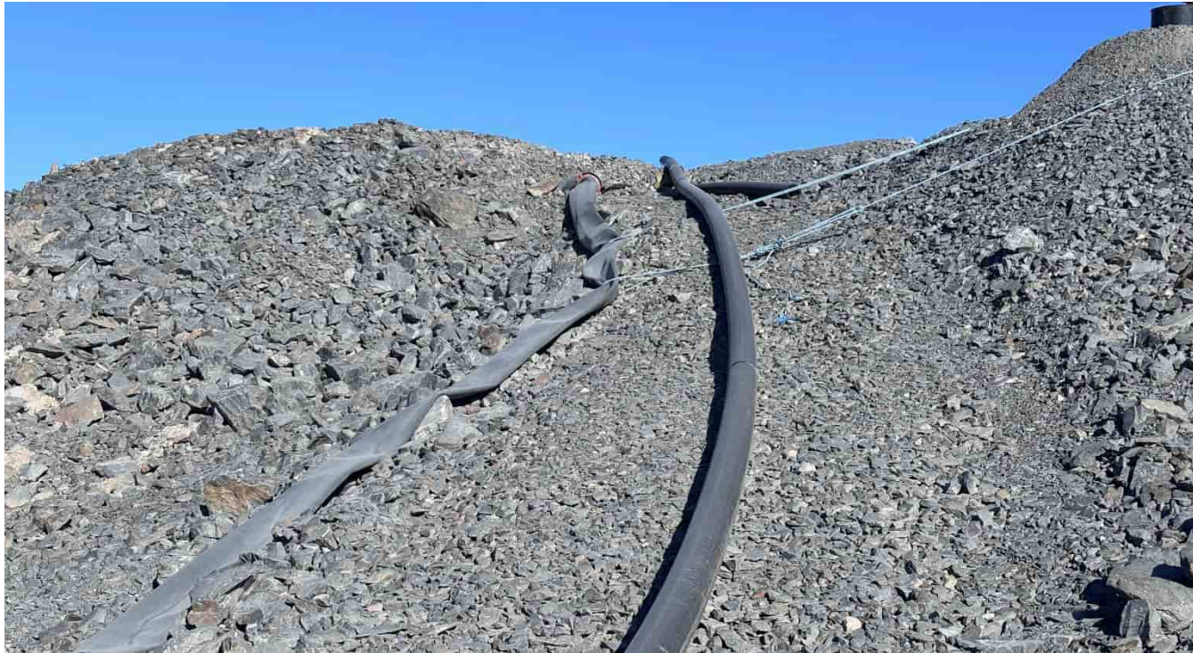
G-473: Unused pipes on downstream slope
