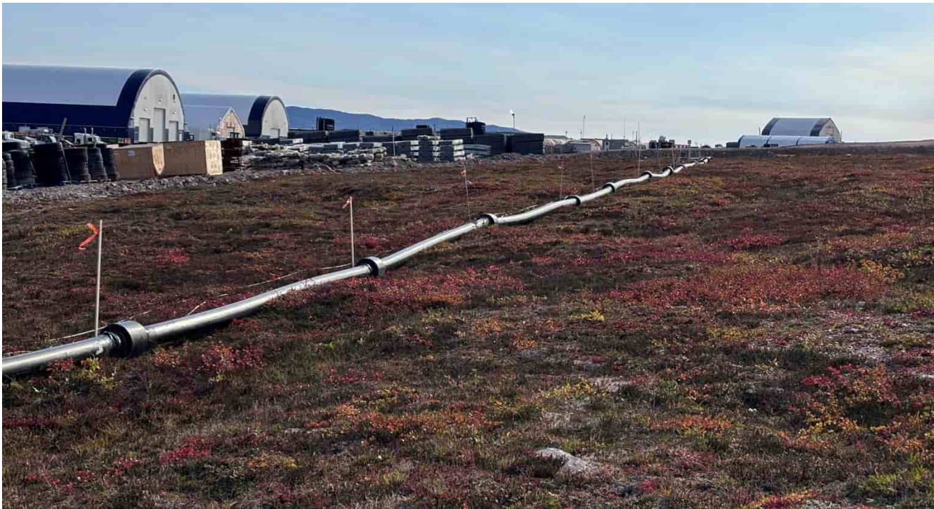
M-4: Freight storage area buildings, looking SE. Note pipe is installed on the exposed tundra
