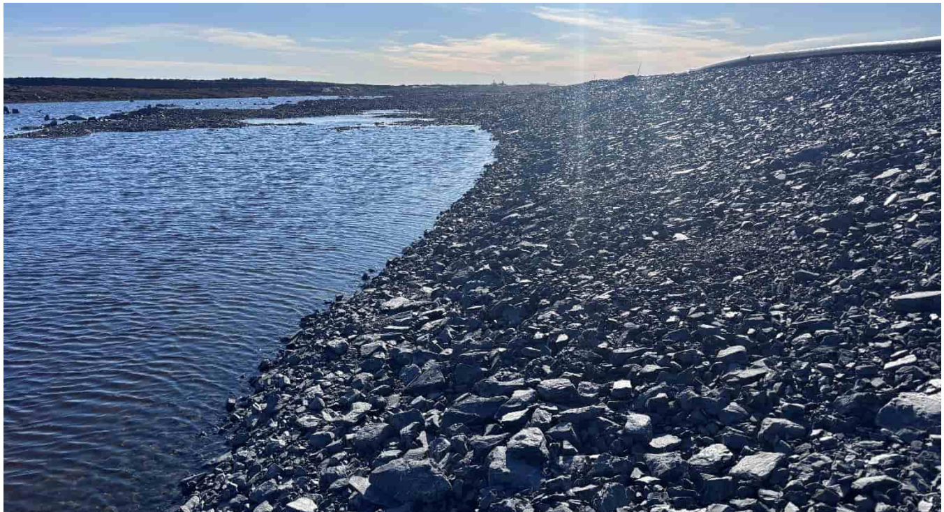
G-467: Upstream side of dam, looking SE
