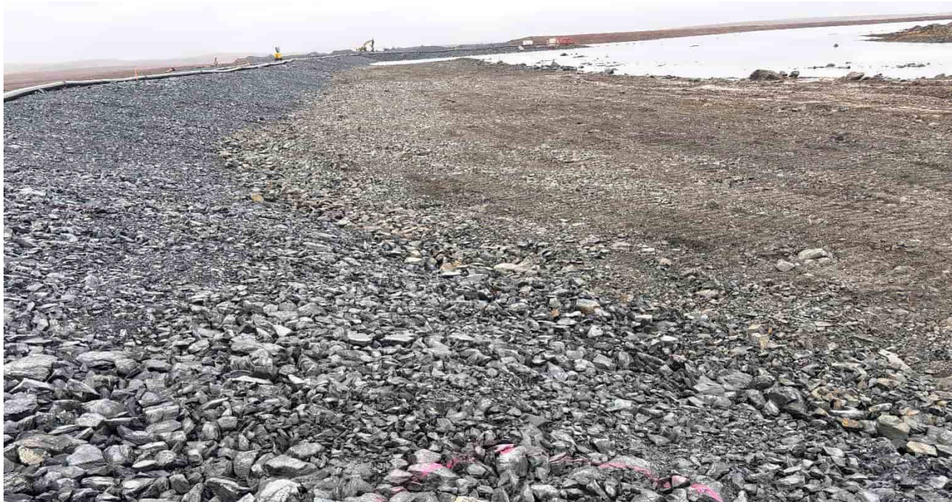
G-485: Southern end of dam and upstream thermal protection barrier, looking NW
