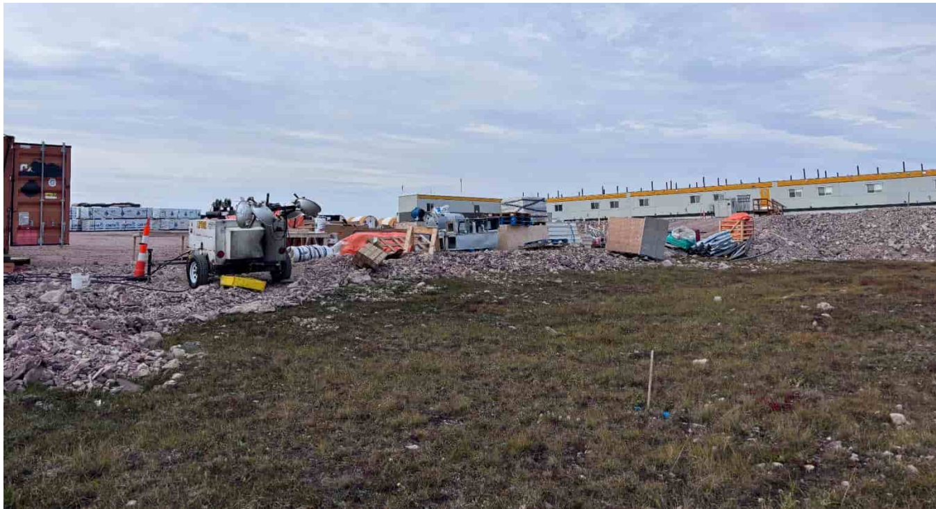
M-47: Laydown area beside pad slope at SE corner of pad
