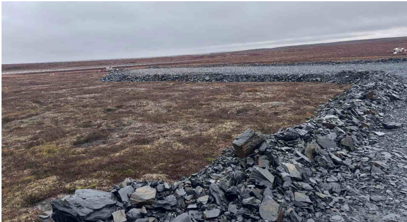
G-498: Access road typical rockfill
