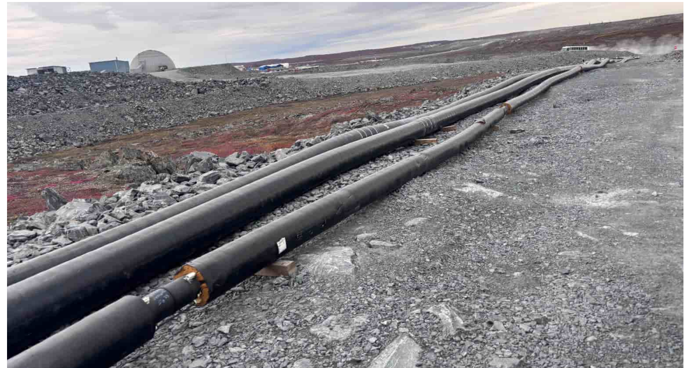
G-510: Typical tailings pipeline corridor layout, looking NW
