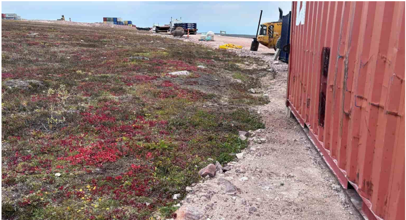
M-19: Shoreline pad – seacan near edge of thin pad
