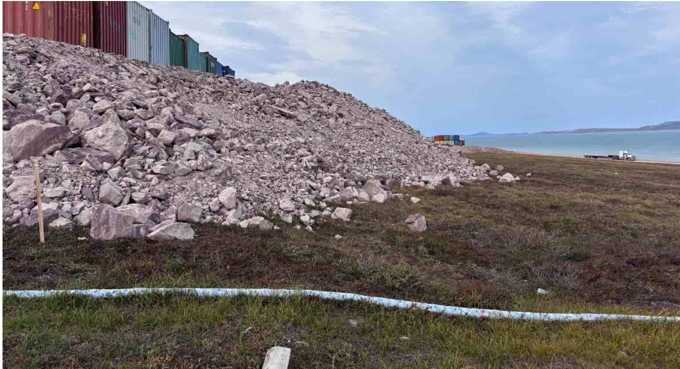
M-52: Camp pad extension, looking NW
