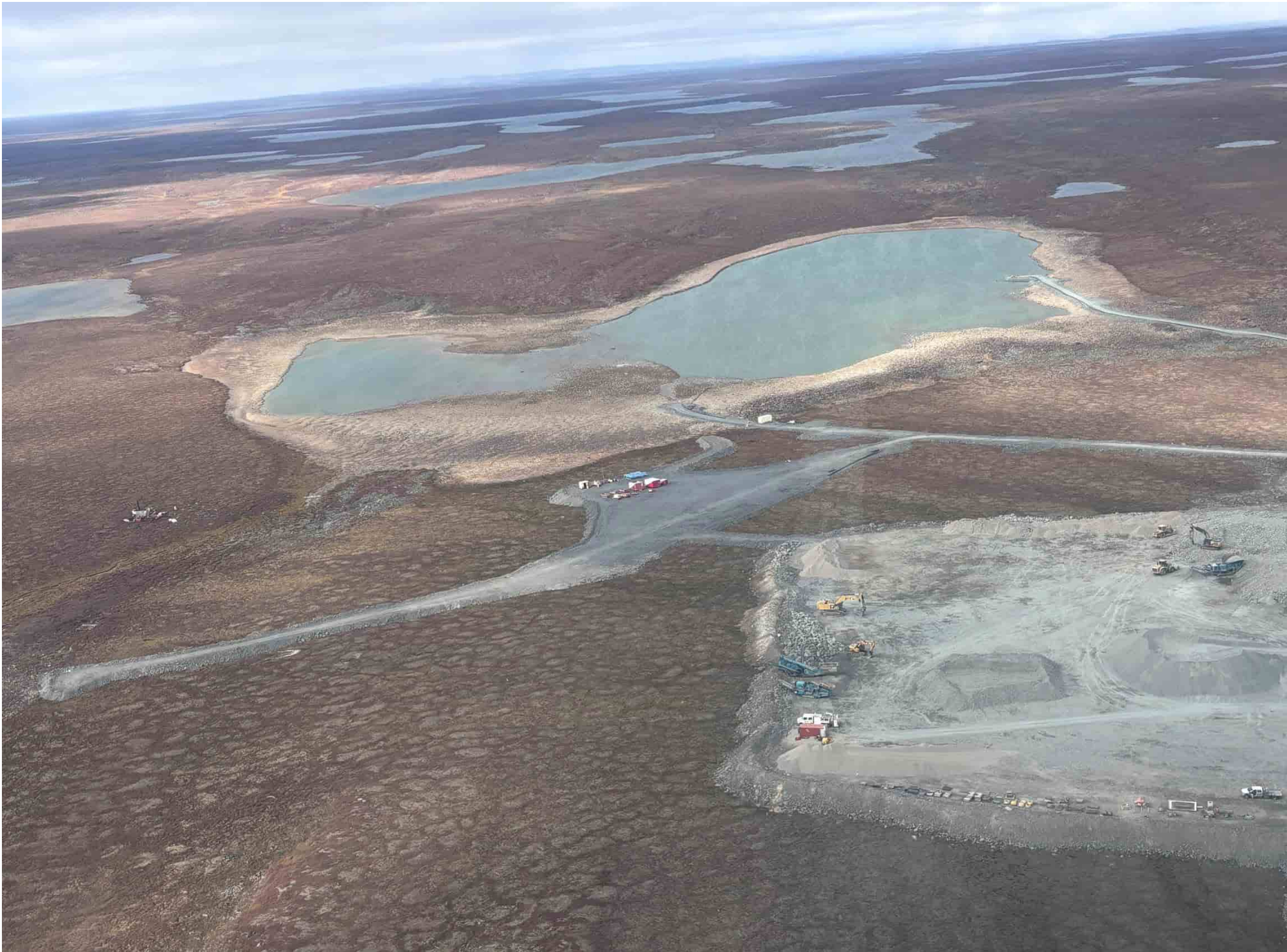
Heli Photo: Llama Lake and crusher pad, looking N – lake dewatering in progress
