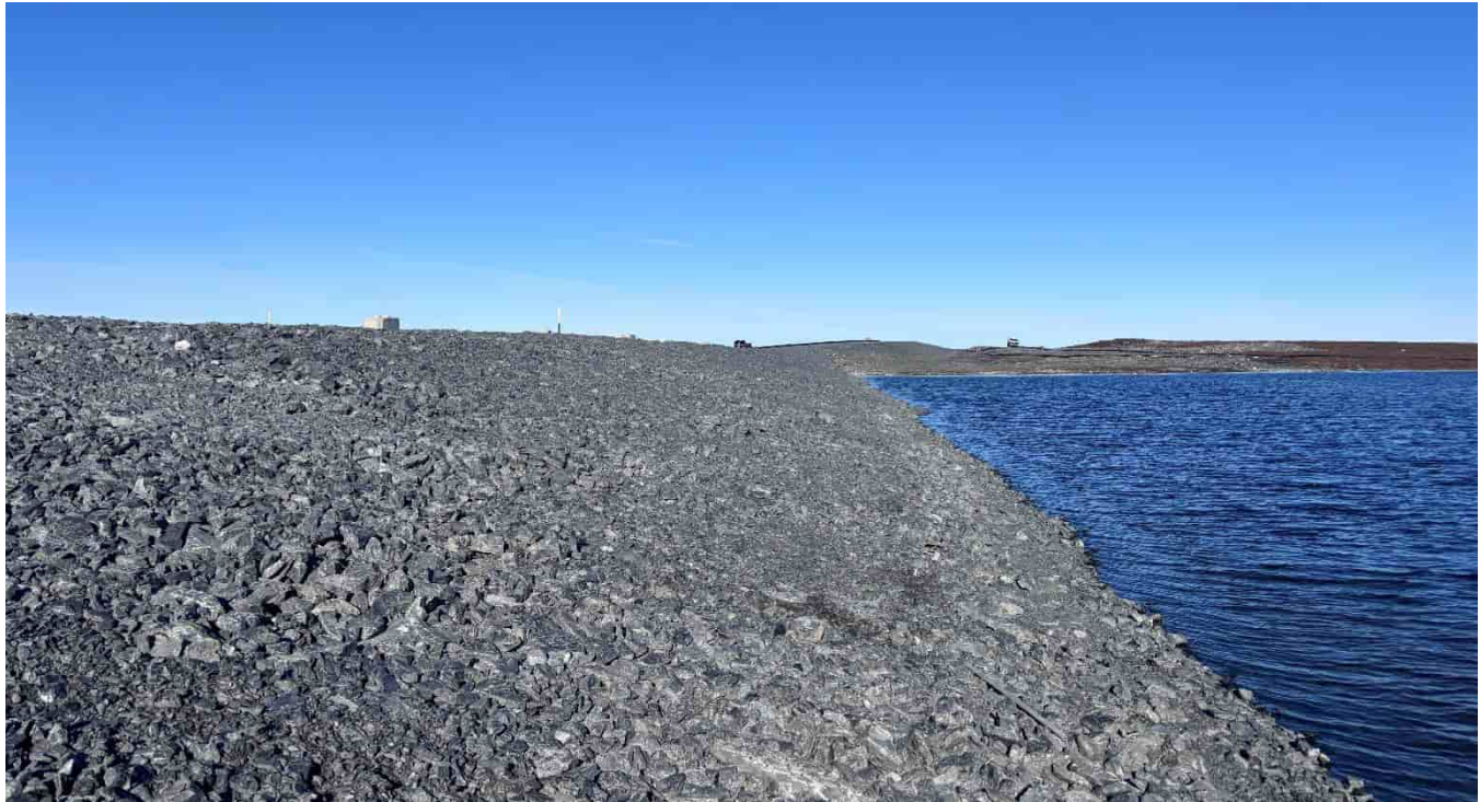
G-466: Upstream side of dam, looking NW
