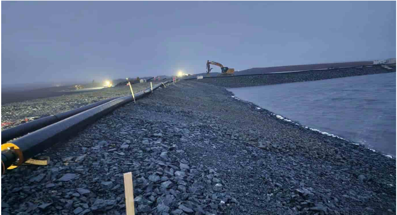
G-468: Upstream crest and upstream slope of the dam, looking NW
