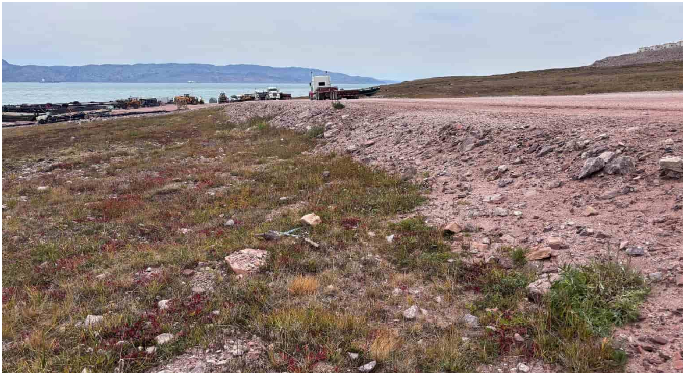
M-23: Shoreline pad access road embankment
