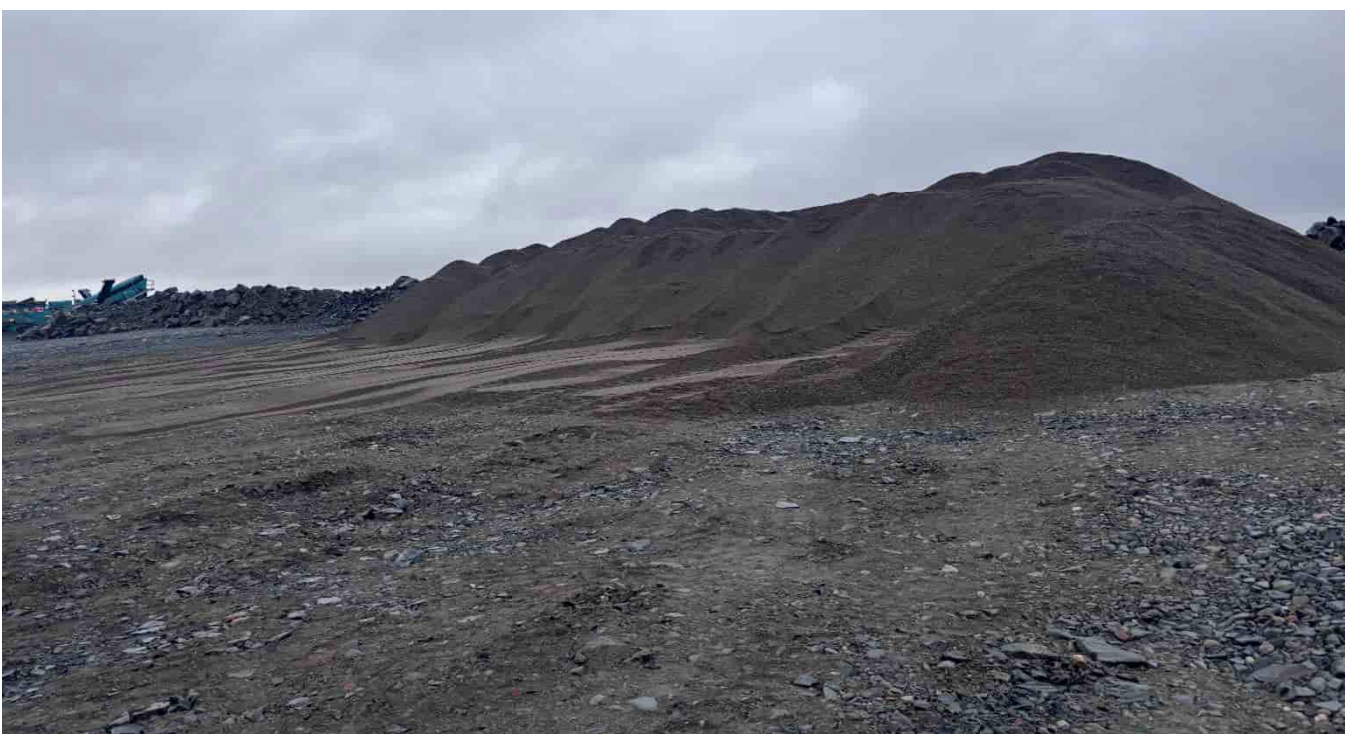
G-499: Overburden stockpile in Llama crusher pad
