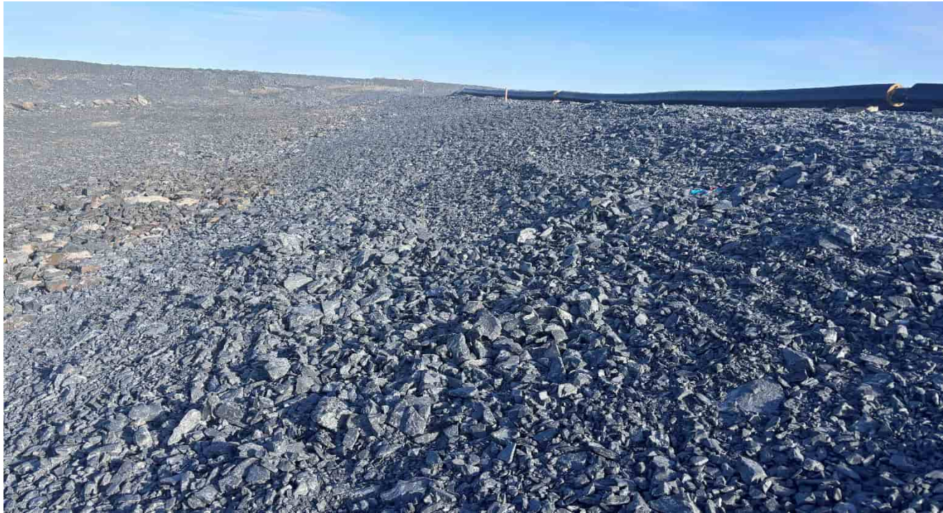
G-476: Upstream dam slope and thermal protection barrier, looking SE from southern end of pond
