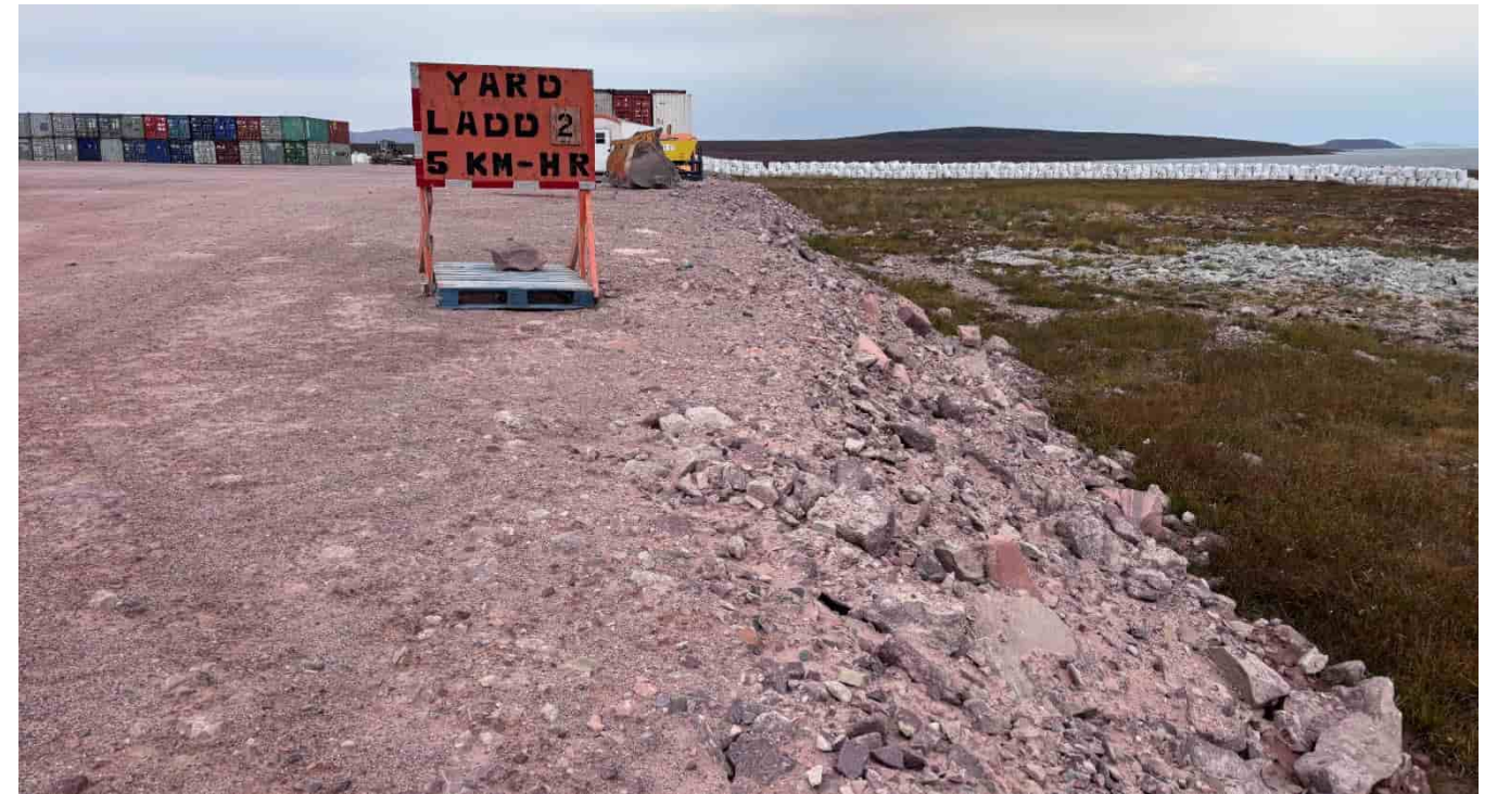
M-24: Northeastern freight storage pad slope
