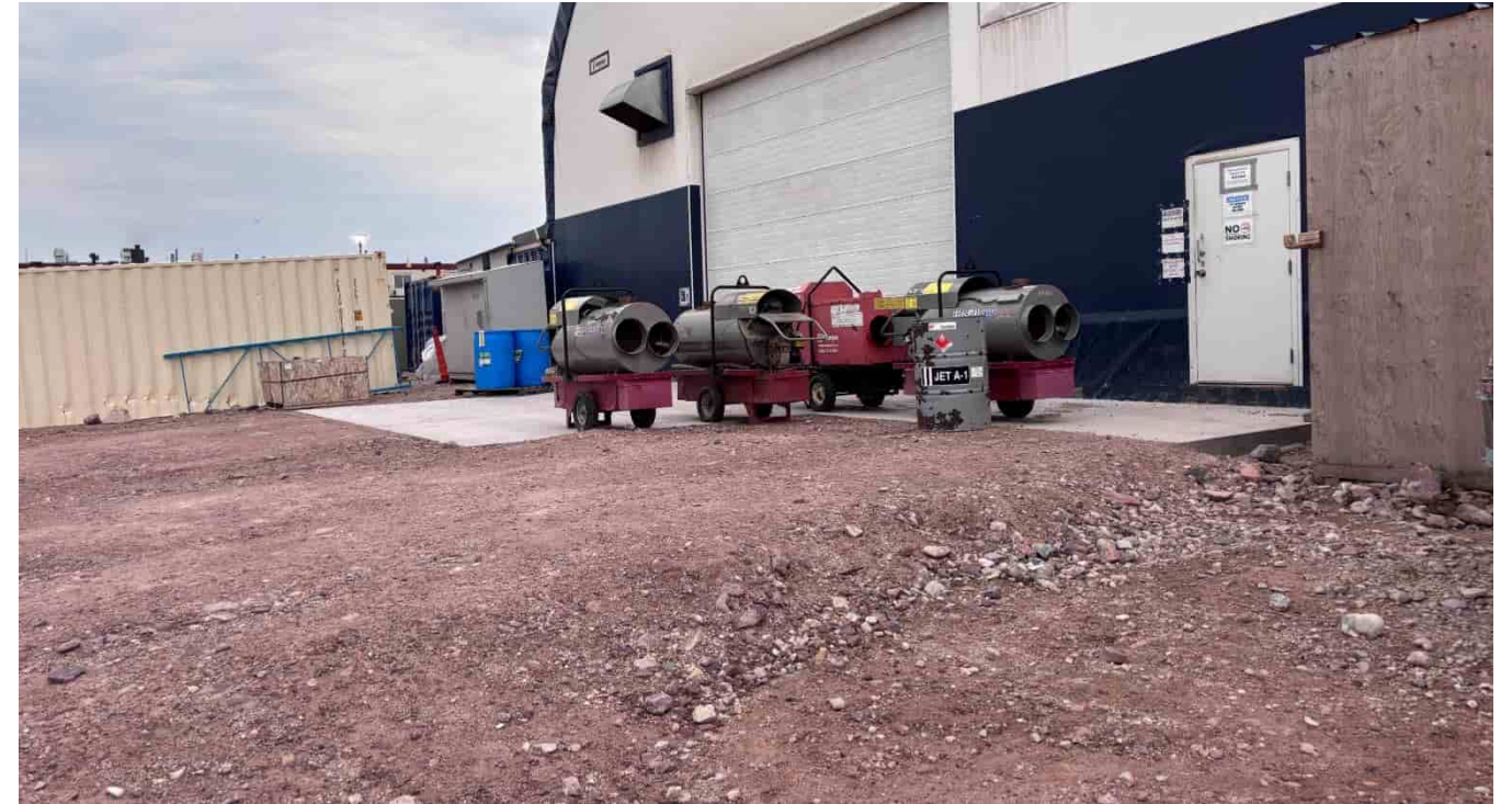
M-37: Maintenance shop area - Entrance to building and concrete pad
