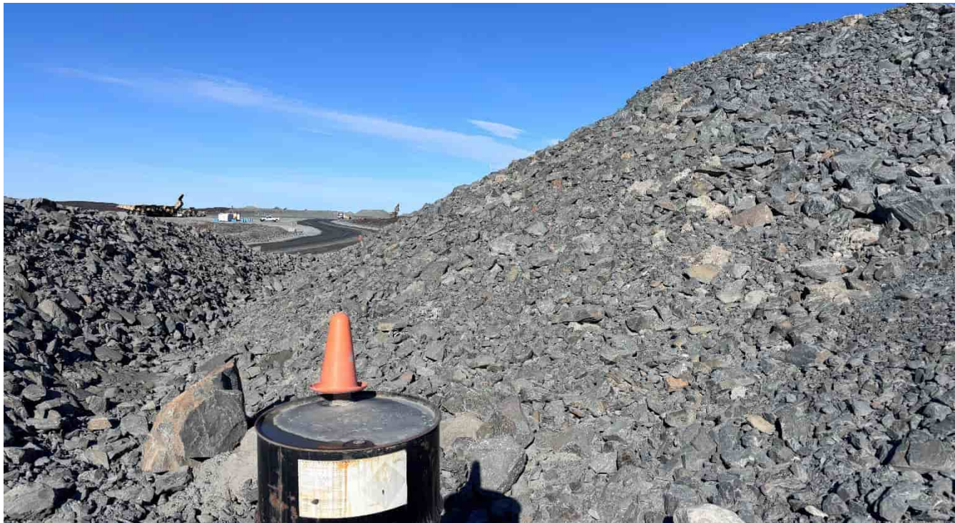
G-474: Downstream slope, looking NW
