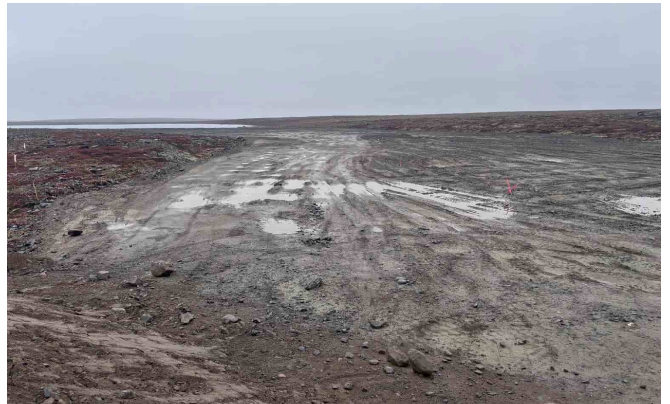
G-486: Overburden fill S of pond, looking N
