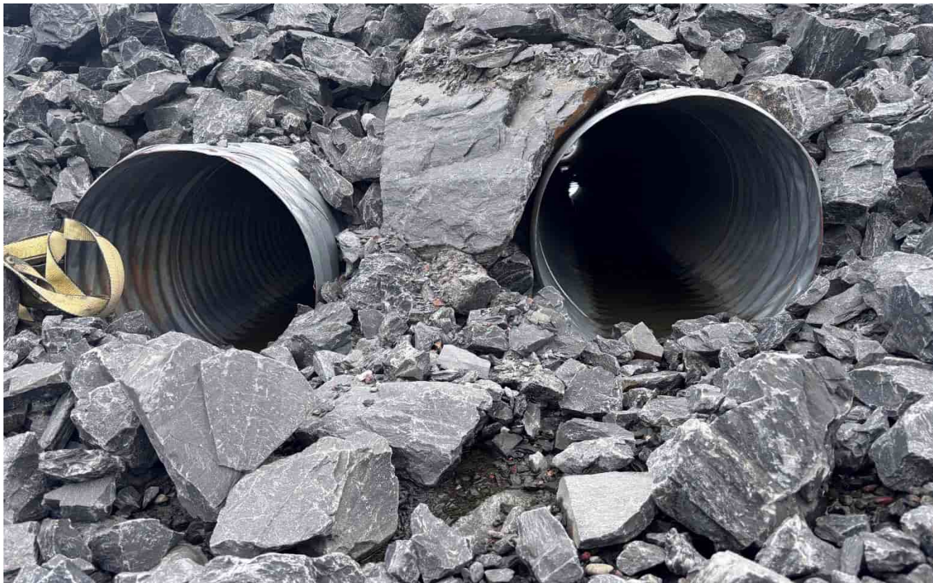
G-525: Eastern and central culvert outlets
