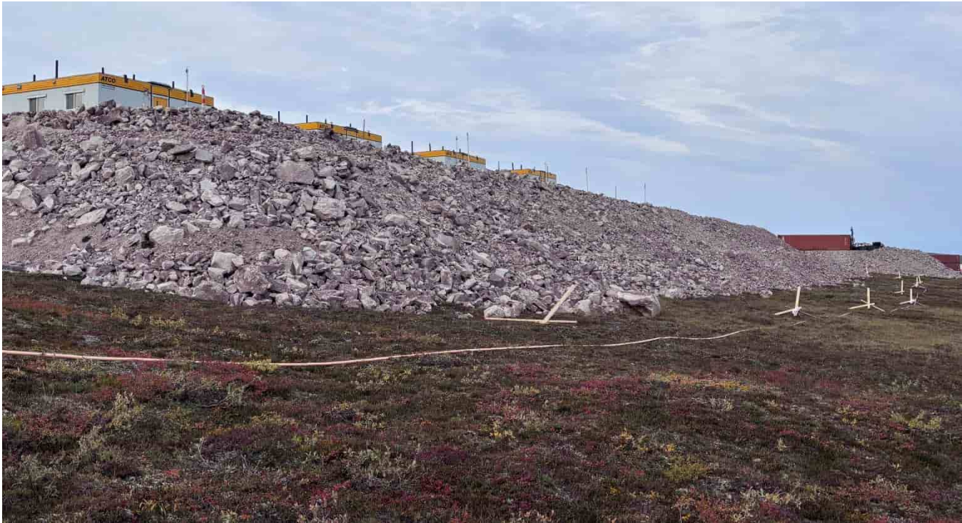
M-49: Eastern pad slope, looking NW
