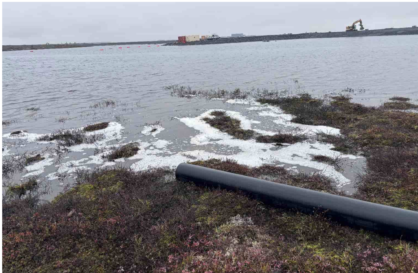
G-482: Pipe discharge into pond, looking S
