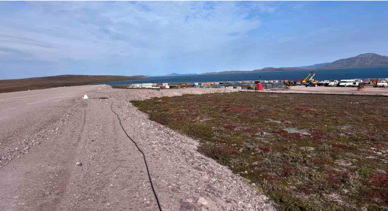
M-70: Airstrip embankment, looking NW
