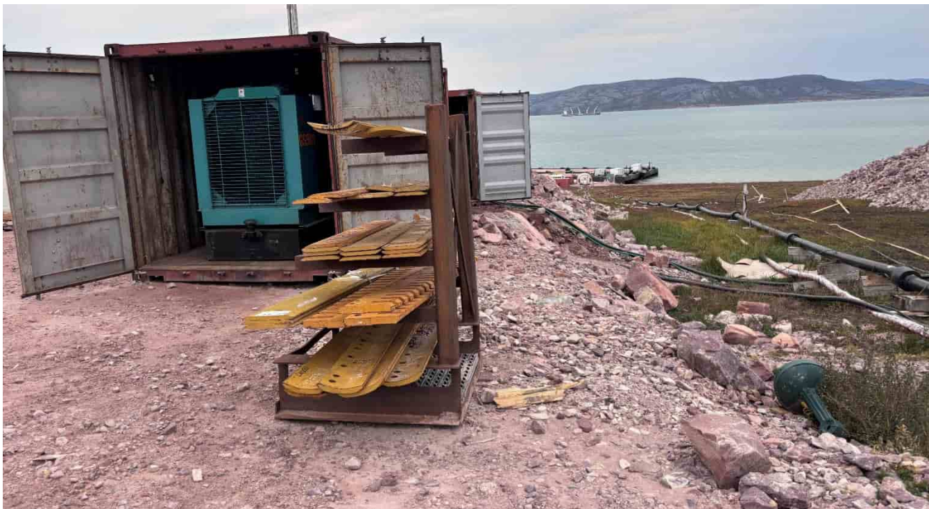
M-38: Edge of pad, looking NE – Note eroding pad slope
