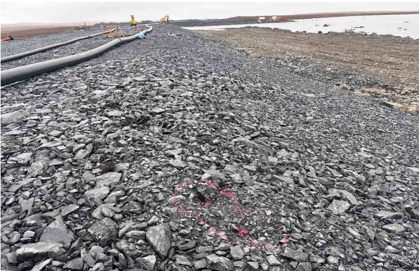
G-483: Dam crest southern end, looking N
