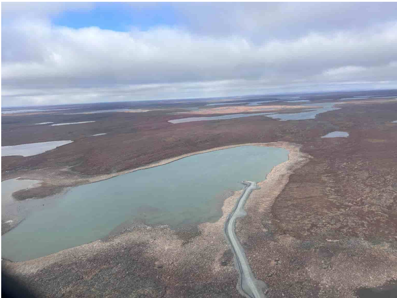
Heli Photo 7: Llama Lake northern access road, looking N
