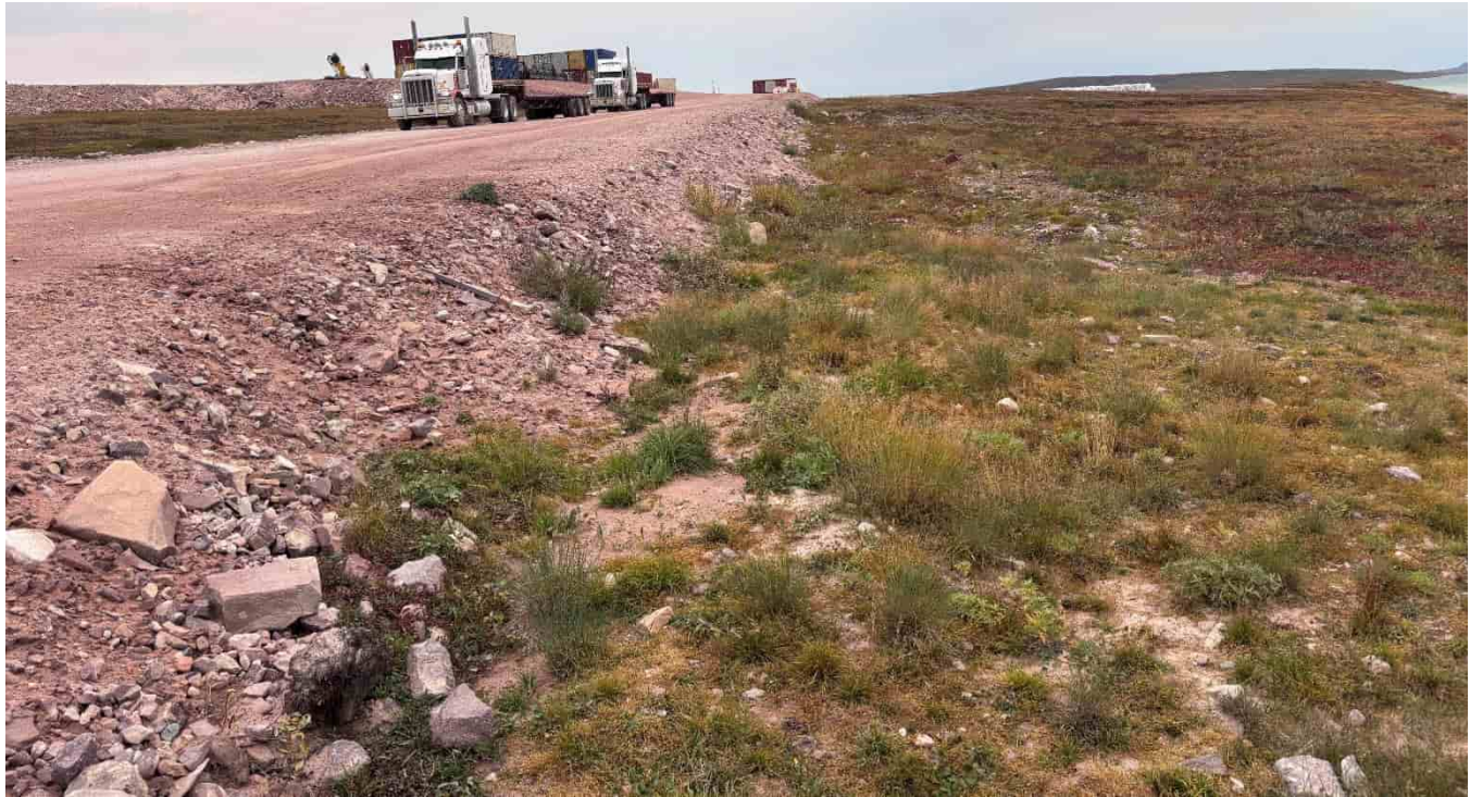
M-17: Shoreline pad access road embankment, looking NW
