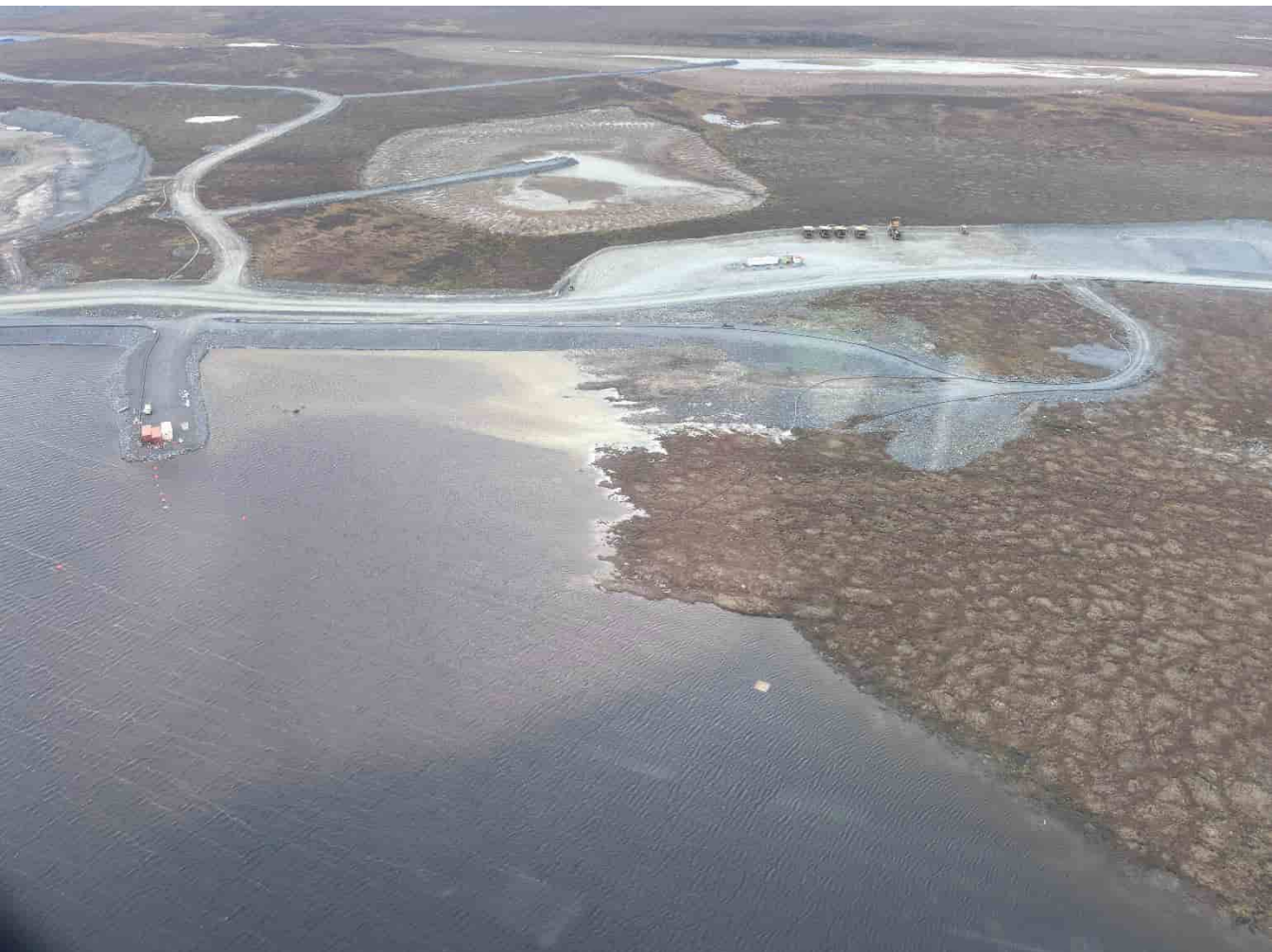
Heli Photo 4: Northern end of dam and pond, looking SW
