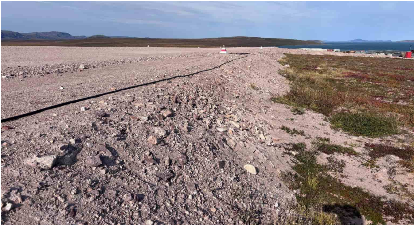
M-67: Airstrip embankment, looking NW
