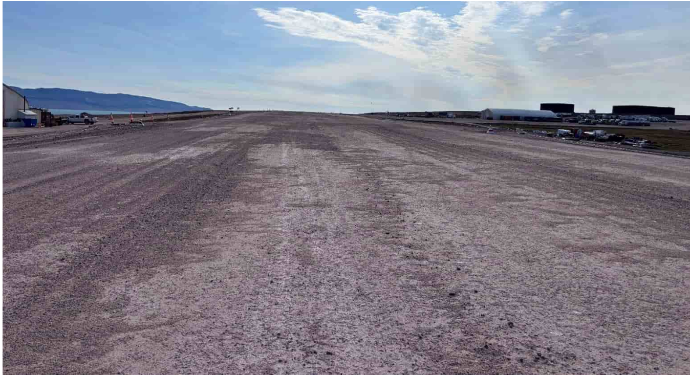
M-69: Airstrip surface conditions, looking SE
