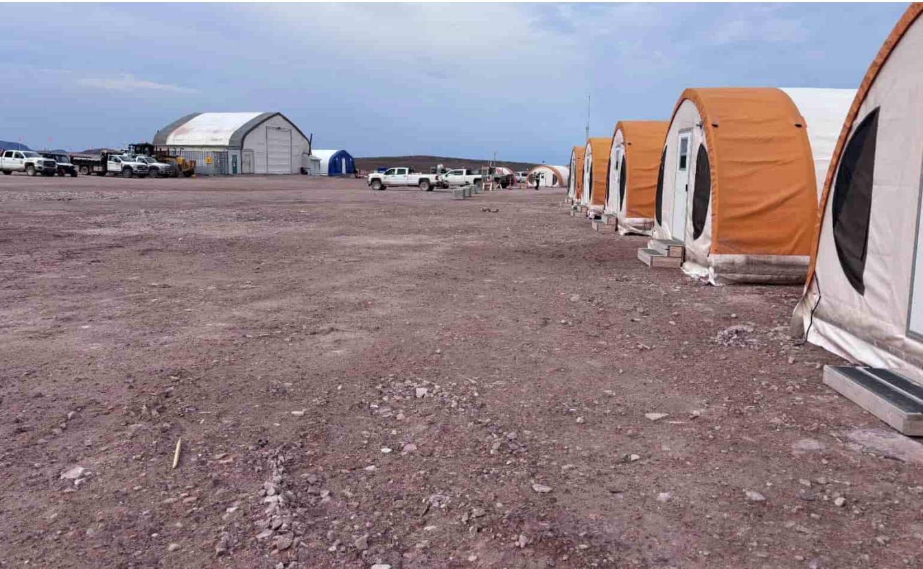
M-64: Camp pad housing and surface conditions, looking NW
