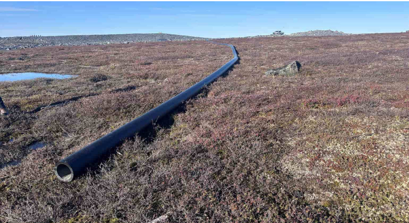
G-465: Pipe end at N side of Primary Pond
