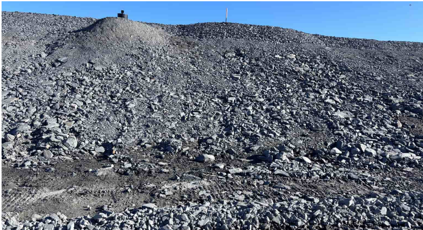
G-471: Downstream side typical dam slope, looking NE from All-Season Road
