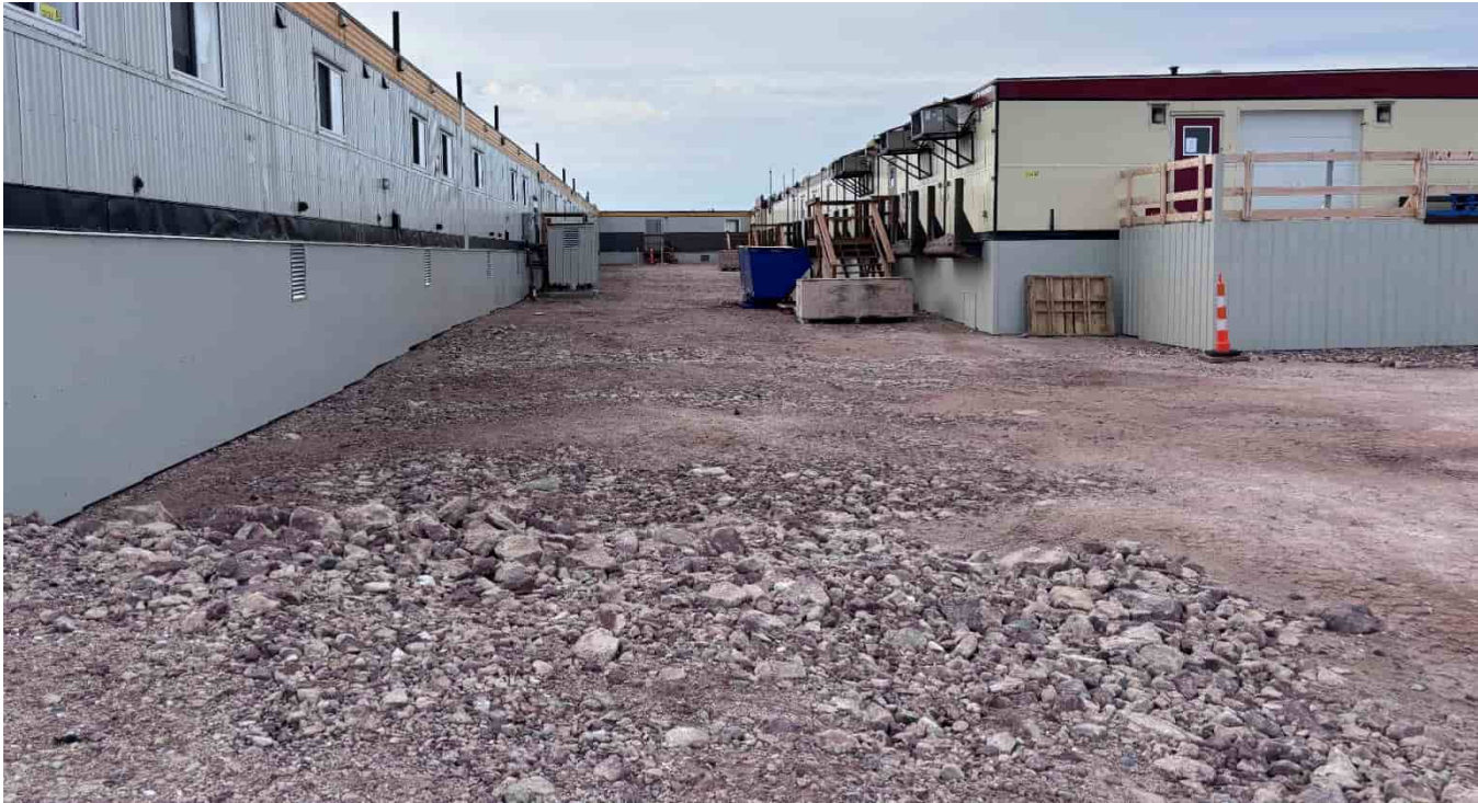
M-60: Camp pad surface conditions
