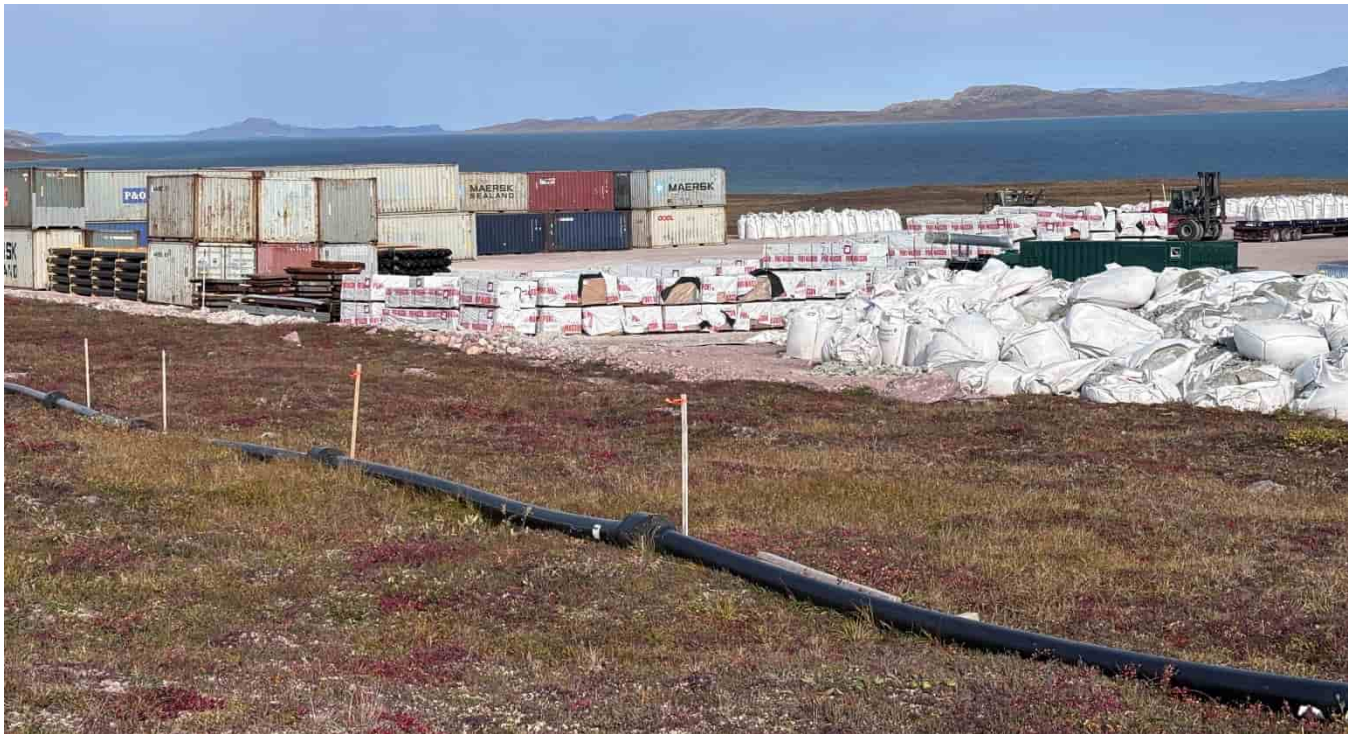
M-3: General laydown area, looking N from toe of airstrip embankment. Note pipe installed on the exposed tundra
