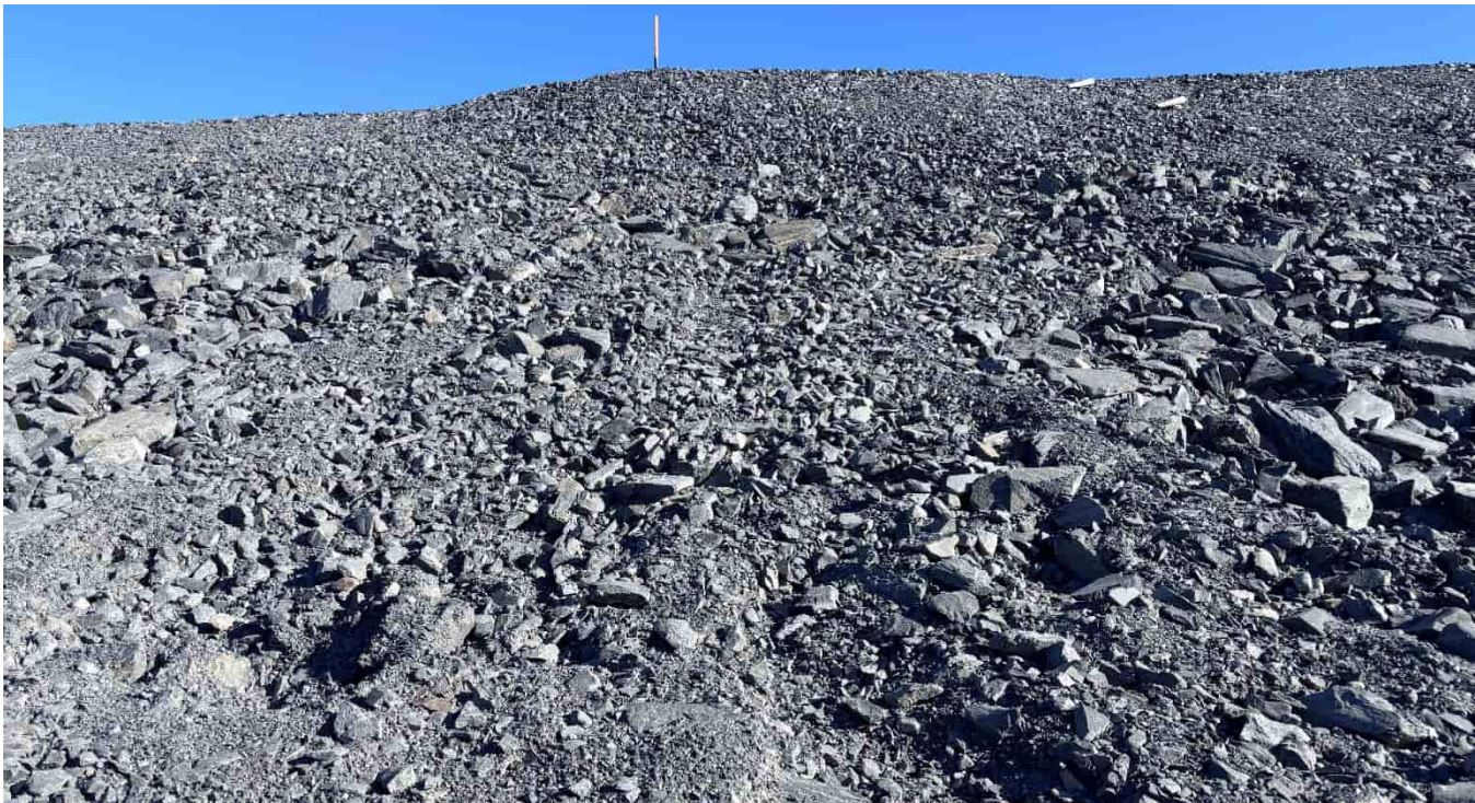
G-472: Downstream dam slope, looking towards crest at Reclaim Pipeline Access Road junction.
