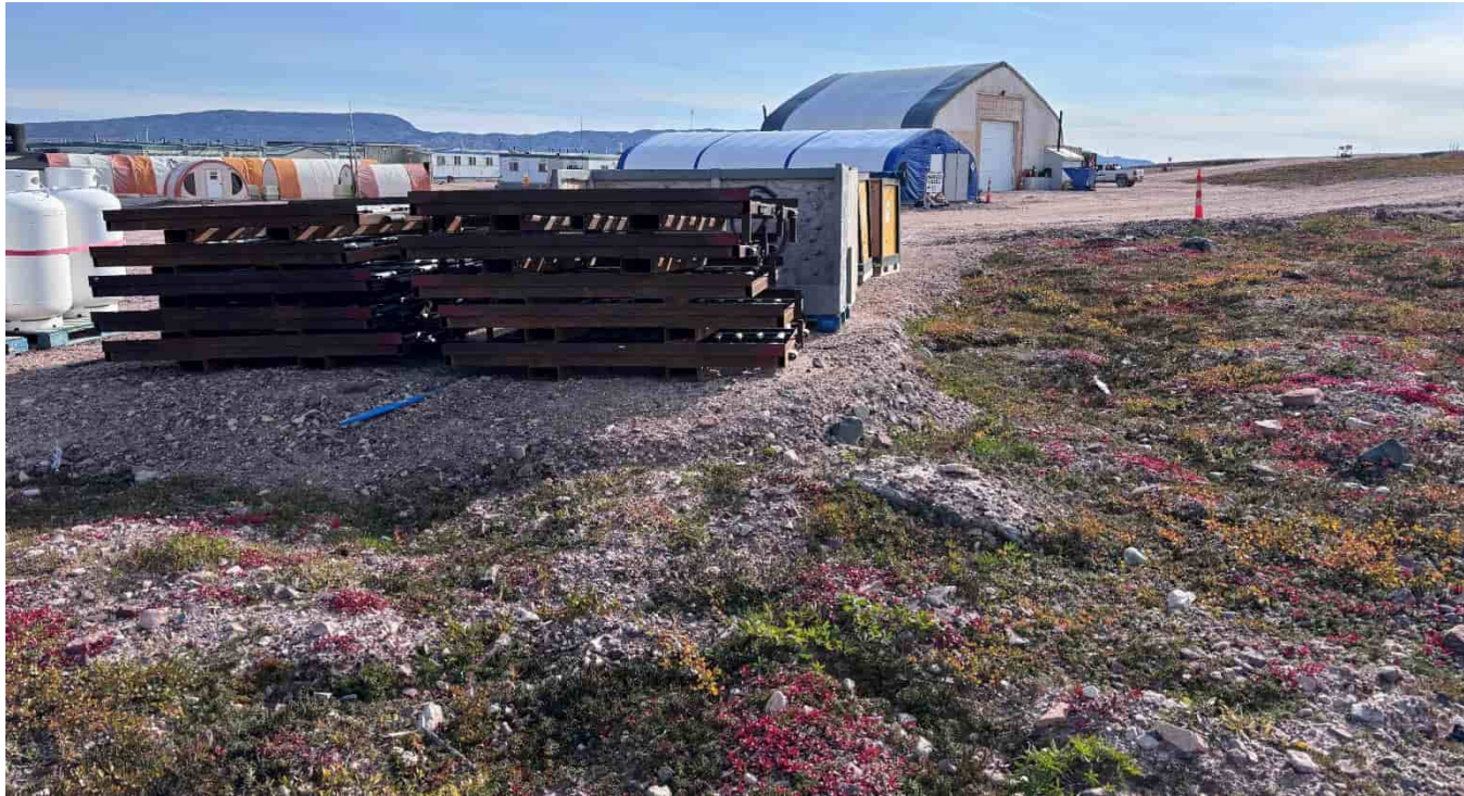
M-65: Pad between airstrip and camp pad – Note thickness of pad
