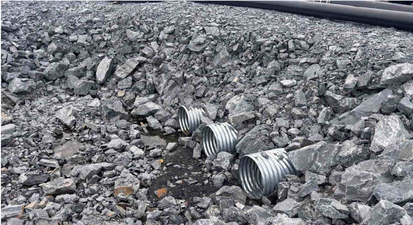
G-520: Culvert inlets (S side) under tailings corridor
