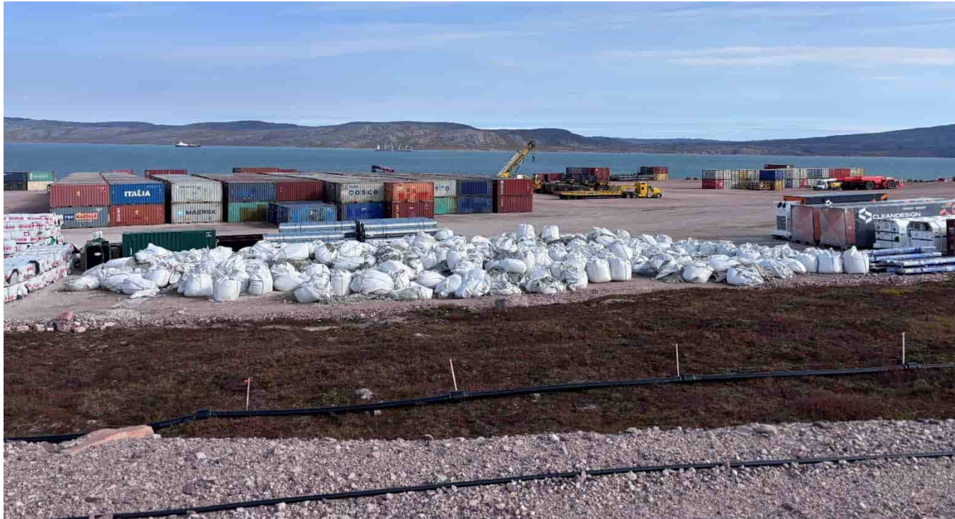
M-9: General laydown area, looking E from airstrip. Pipe placed on the exposed tundra
