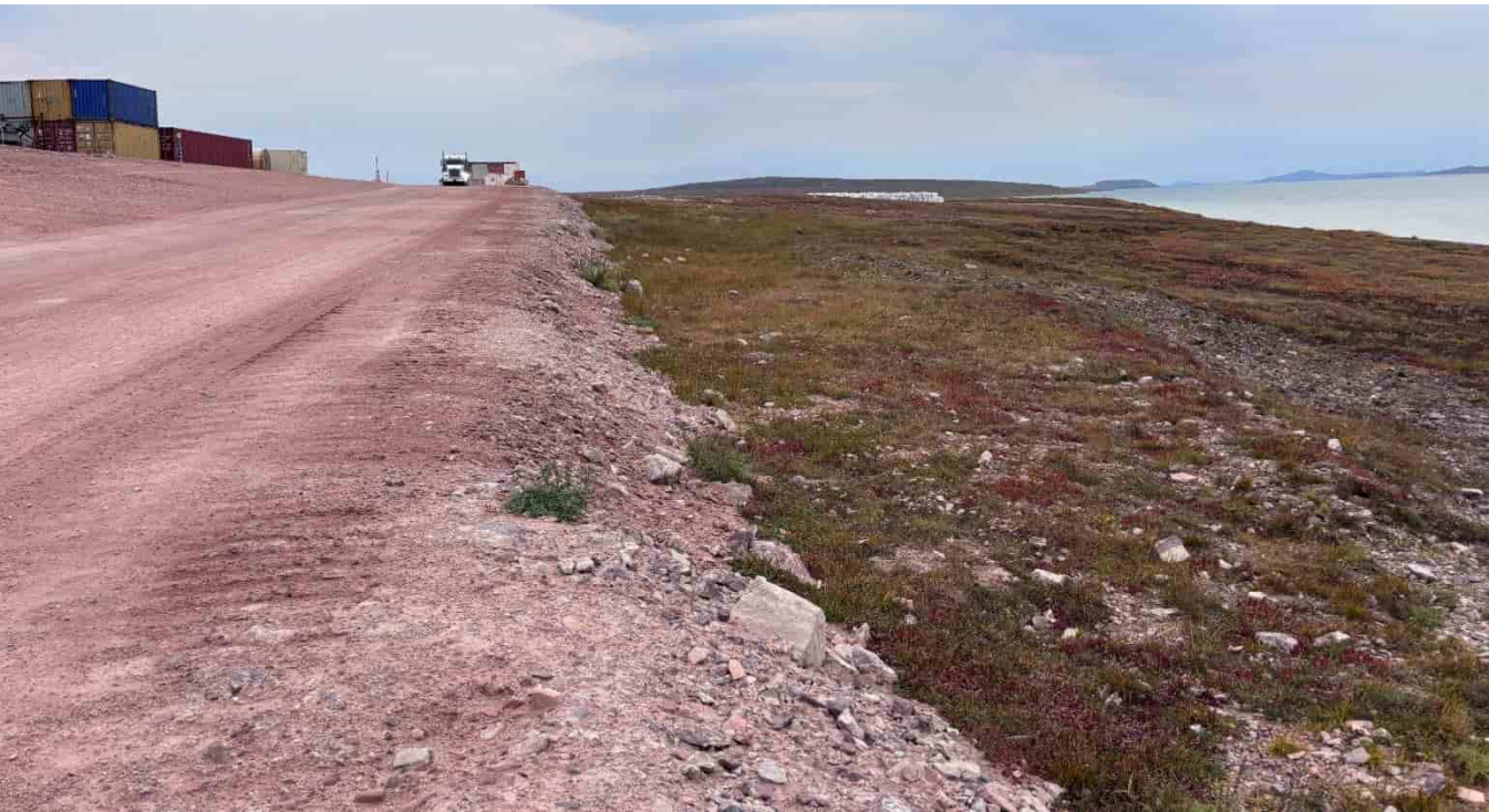
M-16: Shoreline pad access road embankment, looking NW
