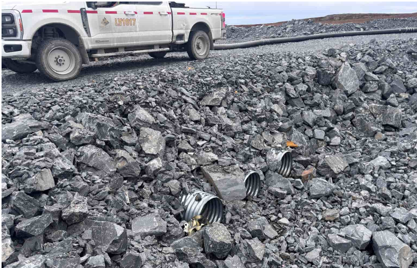
G-523: Triple culvert outlets (N side) under tailings pipeline corridor
