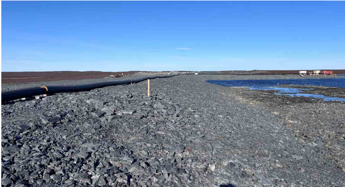
G-469: Crest of dam on upstream side, looking NW
