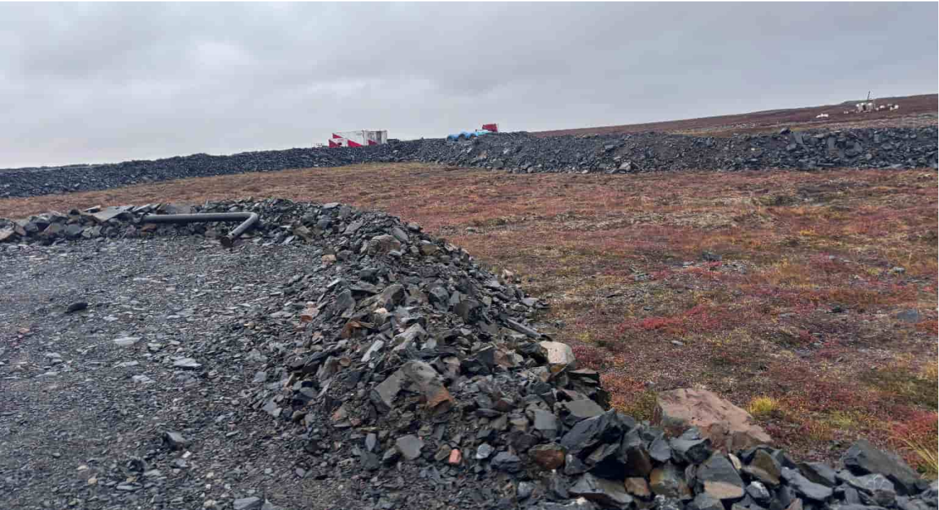
G-504: Pad slopes beside access road, looking S
