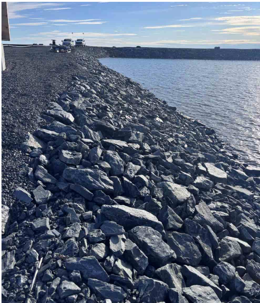
G-479: Reclaim Pipeline Access Road NW slope, looking SW
