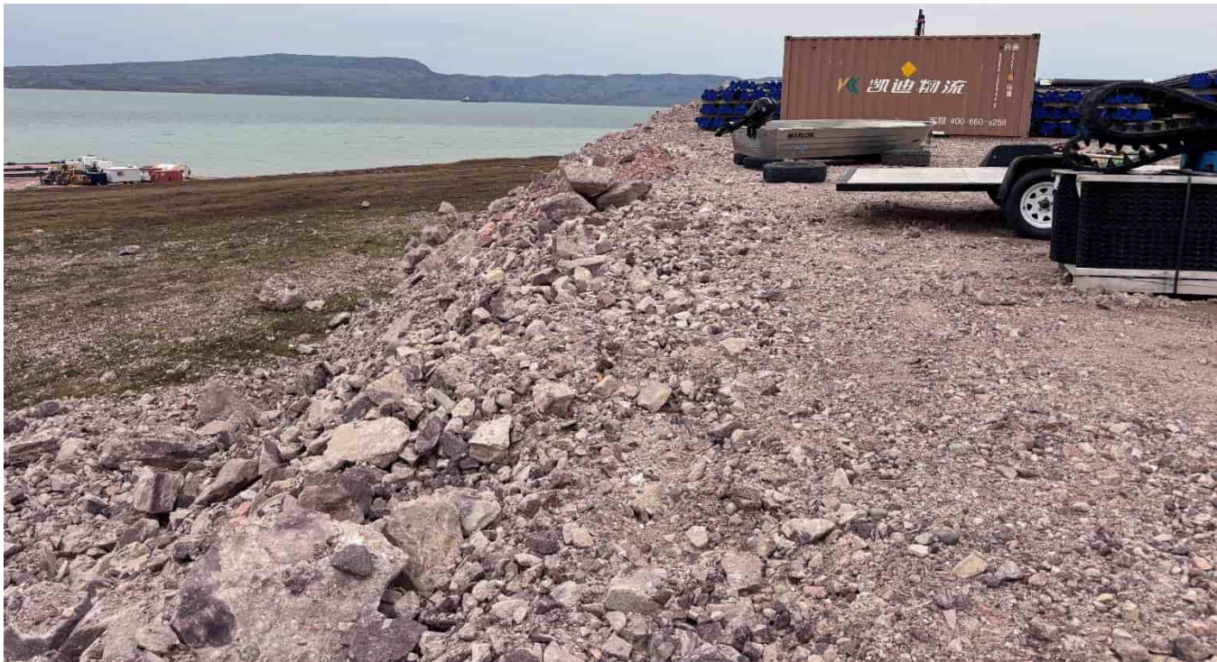
M-11: Eastern pad slope, looking SE
