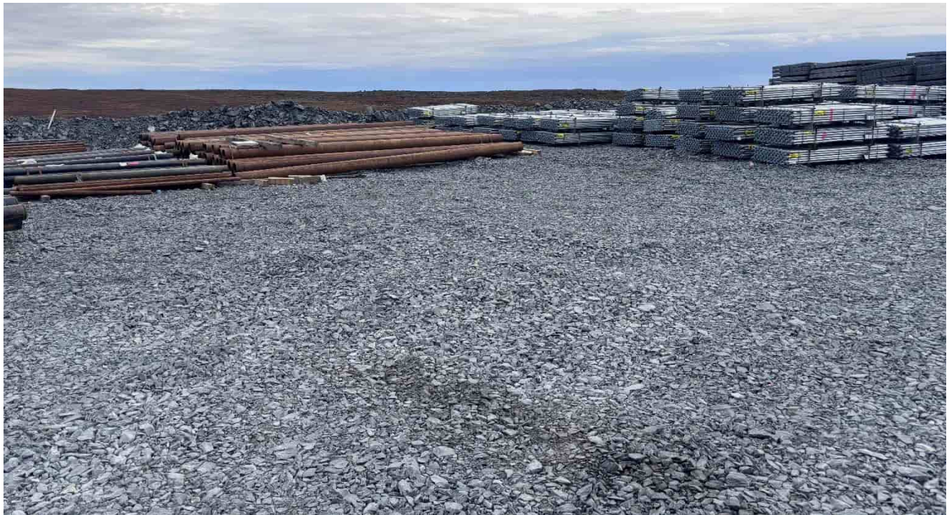
G-513: Pipe laydown beside tailings corridor
