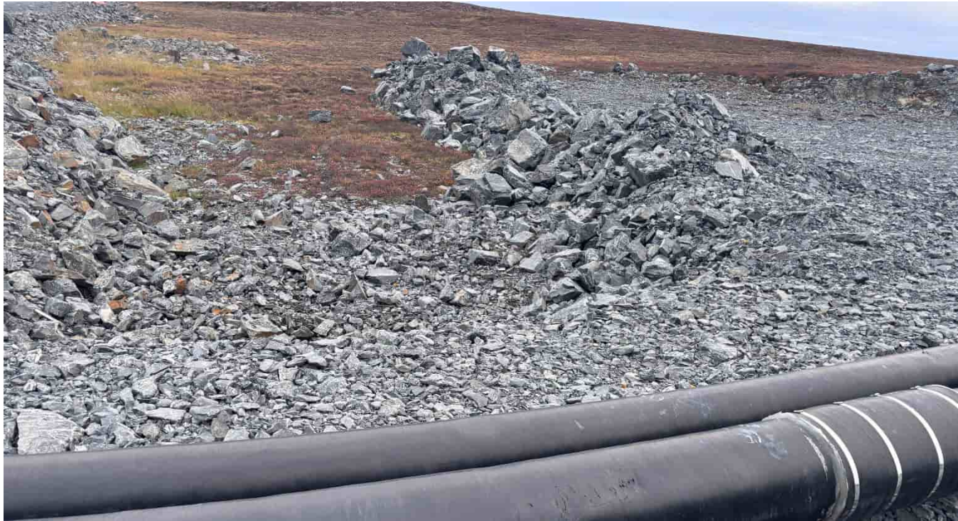
G-519: Pad on S side of tailings pipeline corridor beside Echo Pit Haul Road, looking S
