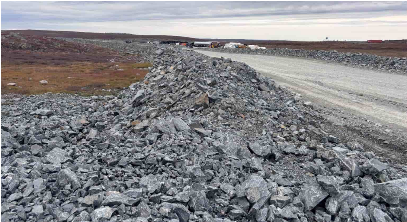
G-522: Echo Pit Haul Road rockfill, looking N from tailings corridor
