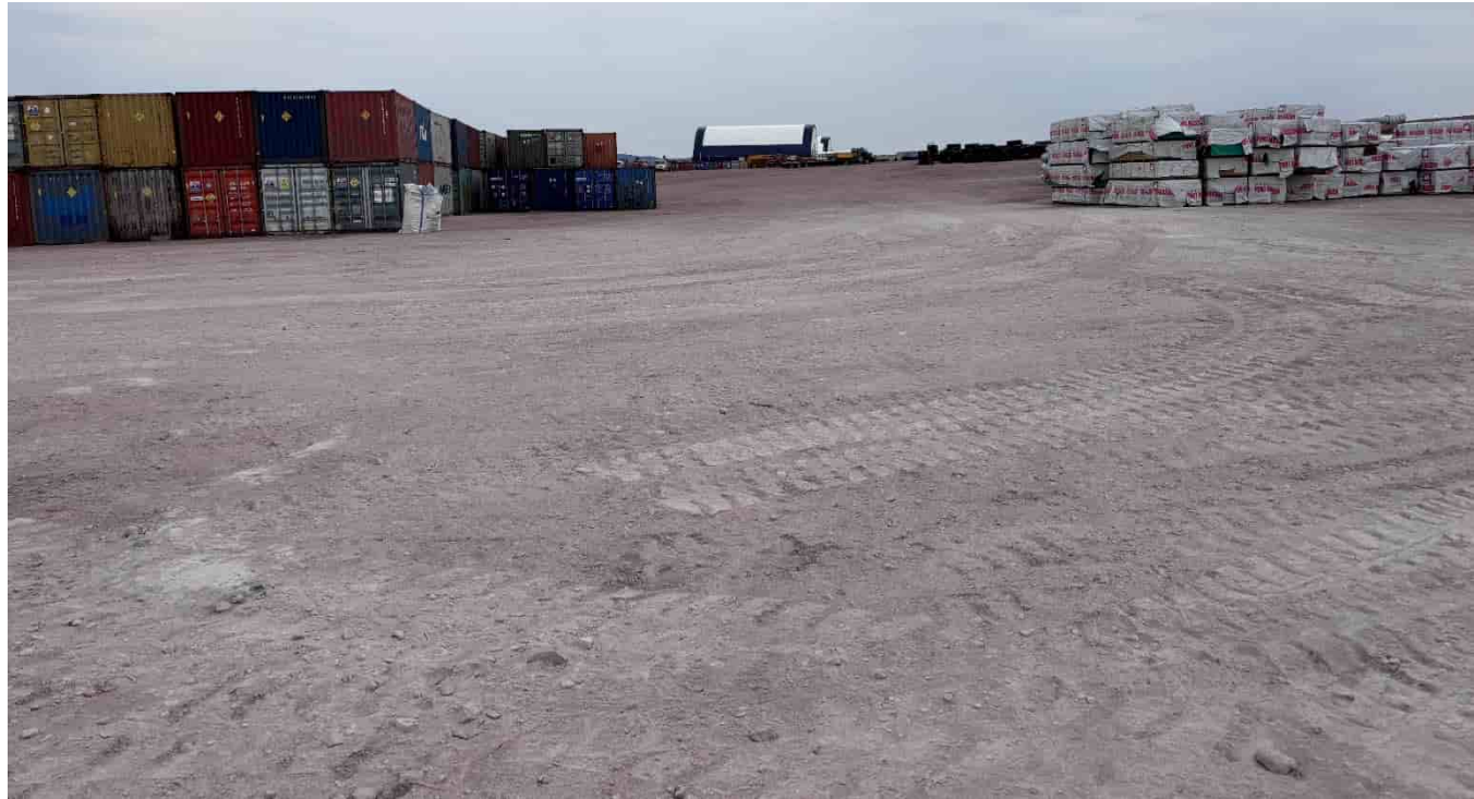
M-33: General view of pad, looking SE
