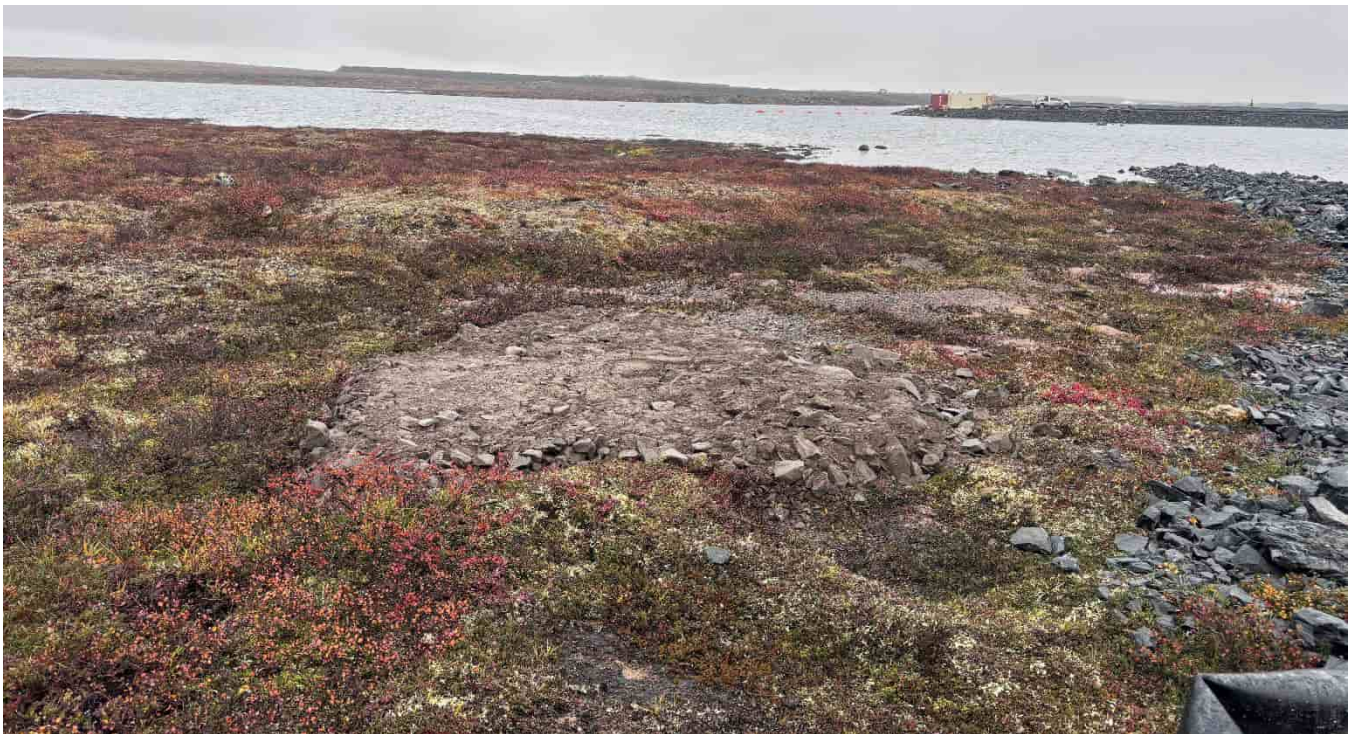
G-481: Discharge point the N of Primary Pond : Note that the disturbed area was backfilled with the low permeability material and the discharge point was moved while SRK was on site.
