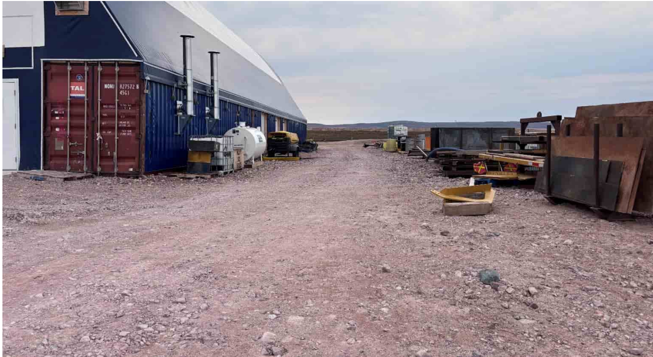
M-36: Maintenance shop area - Laydown beside building, SW
