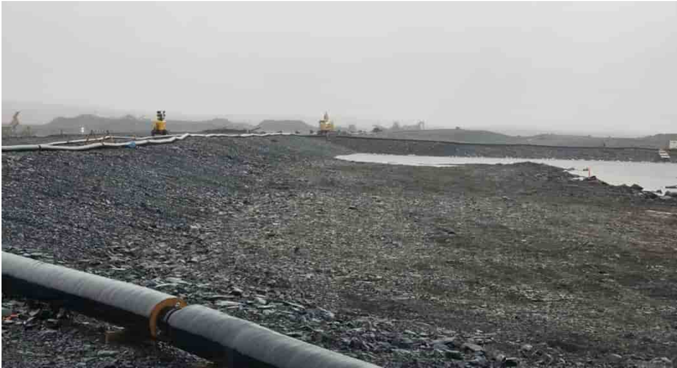
G-470: Upstream thermal protection barrier and upstream slope of the dam: southern end of pond
