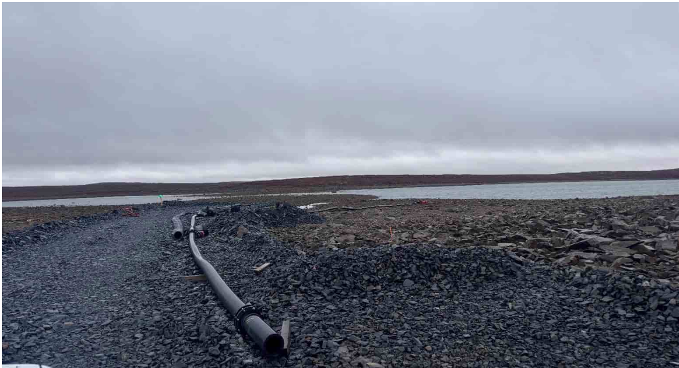
G-502: Unconnected pipeline to Llama Lake, looking W
