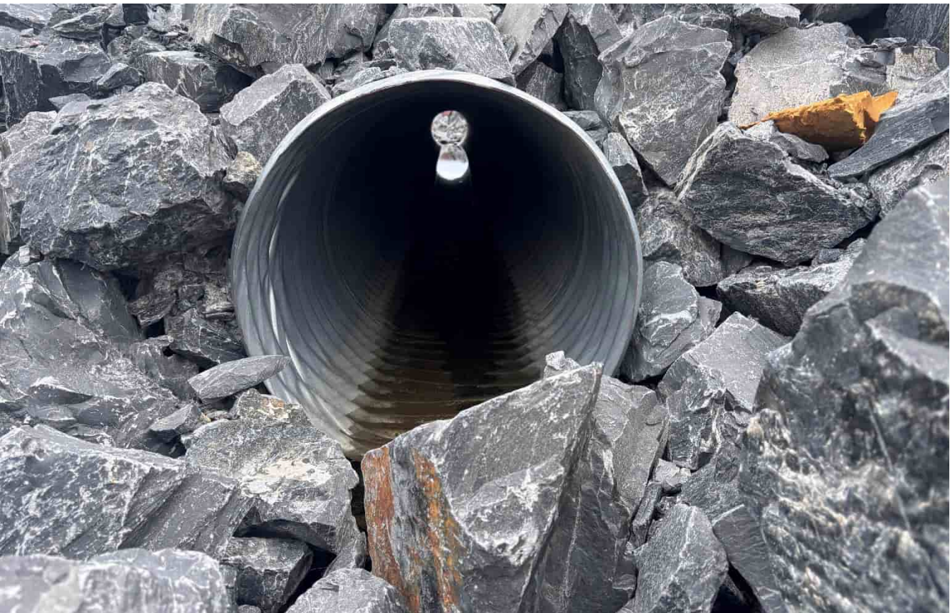
G-524: Western culvert outlet
