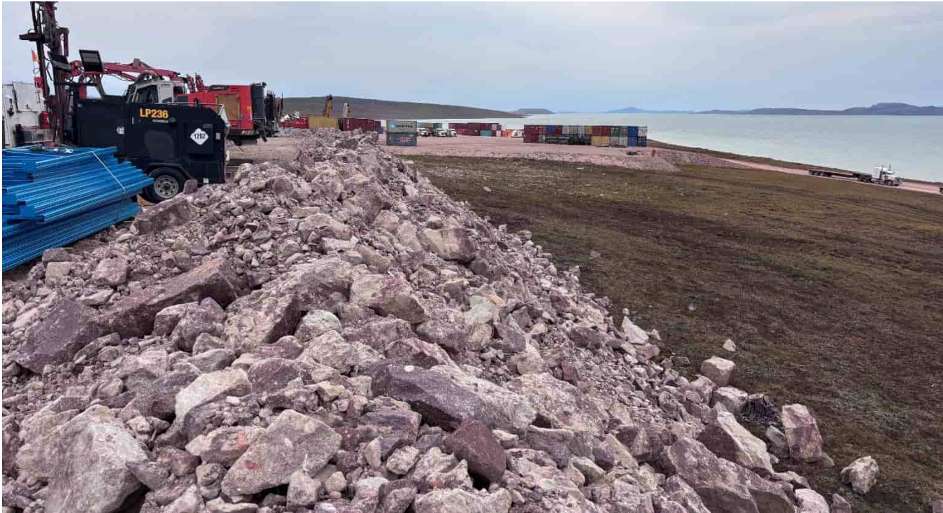
M-10: Eastern pad slope, looking N
