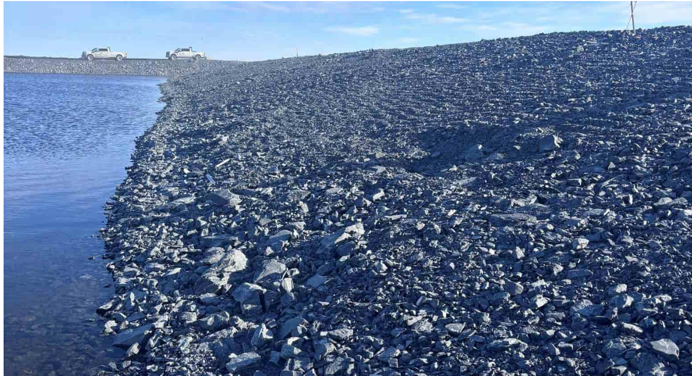
G-475: Upstream dam toe of slope, looking SE towards Reclaim Pipeline Access Road. The “depression” areas were inspected, surveyed and backfilled with the engineering fill.
