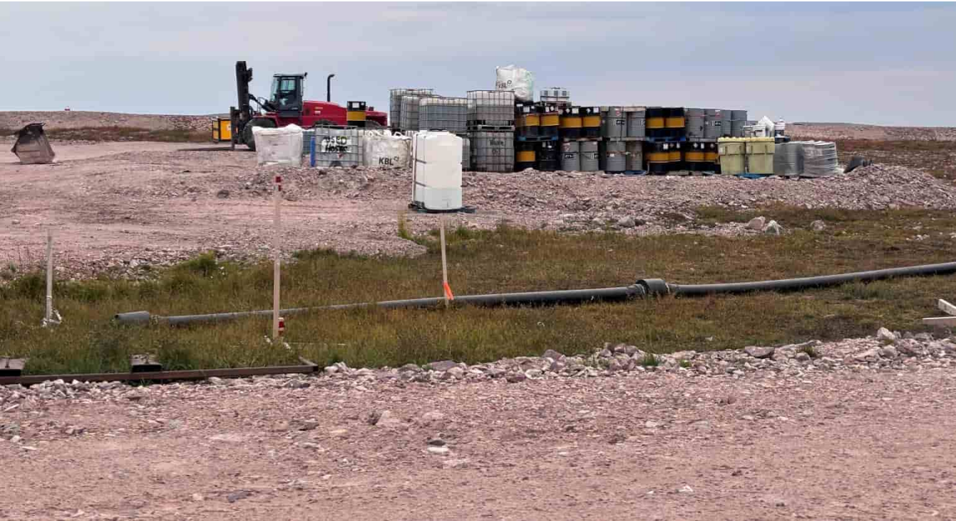
M-41: Temporary fuel storage, looking W
