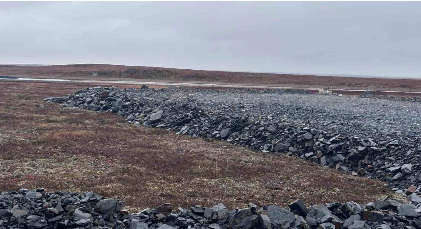
G-497: Pad S of Llama crusher pad, looking SW
