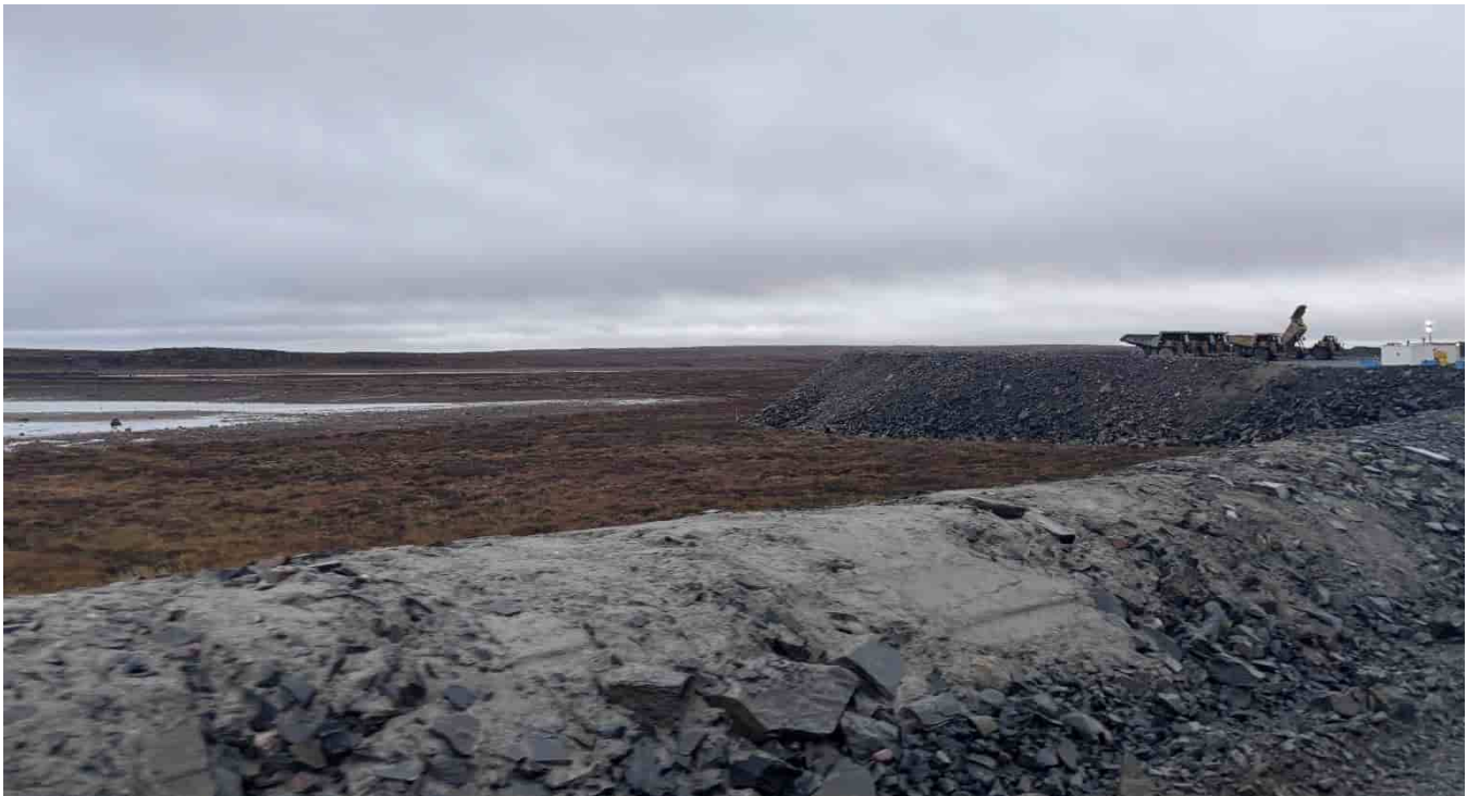
G-495: Truck laydown pad slope, looking W
