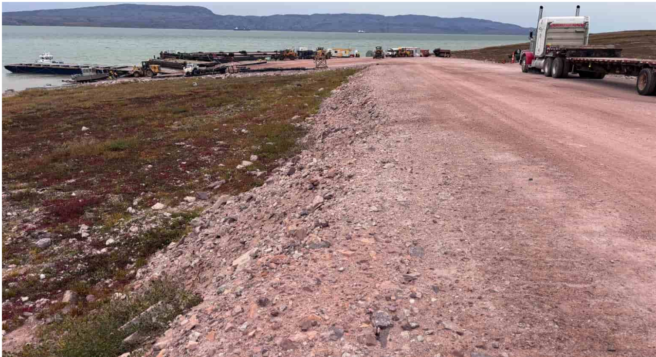
M-15: Shoreline pad access road embankment, looking SE
