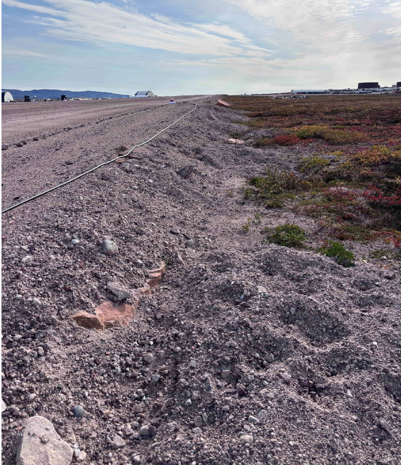
M-86: Undefined edge of airstrip embankment, looking SE
