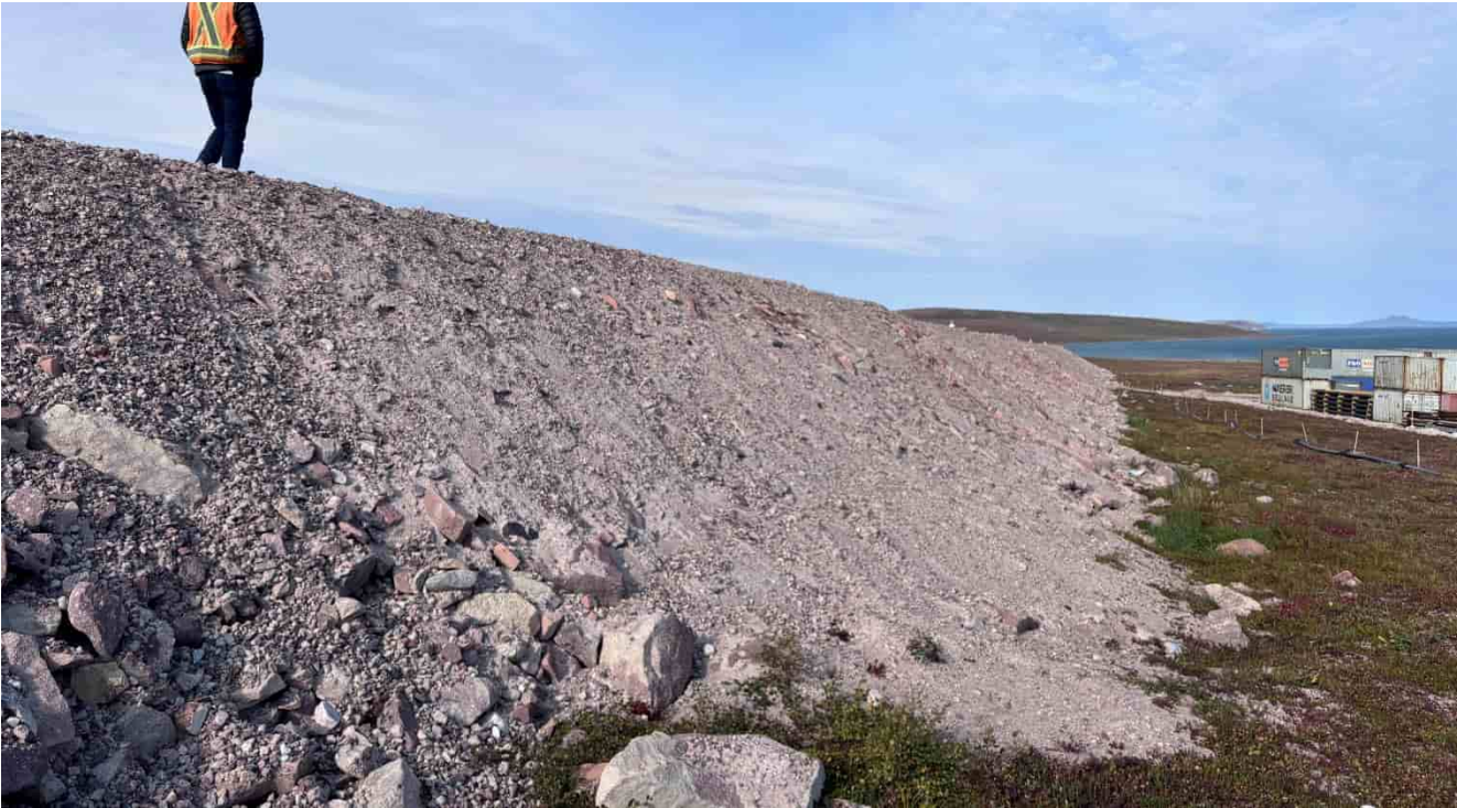
M-76: Eastern airstrip embankment
