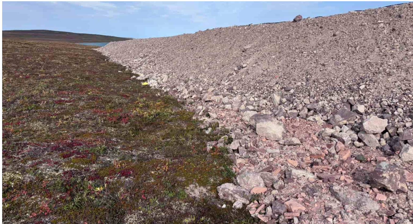
M-85: Western airstrip embankment, looking NW
