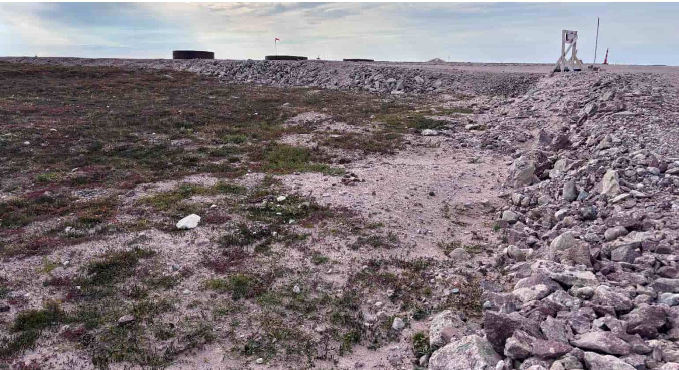
M-95: Airstrip junction with camp pad access road
