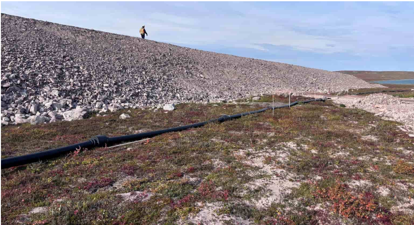
M-78: Eastern airstrip embankment beside N end of freight storage pad
