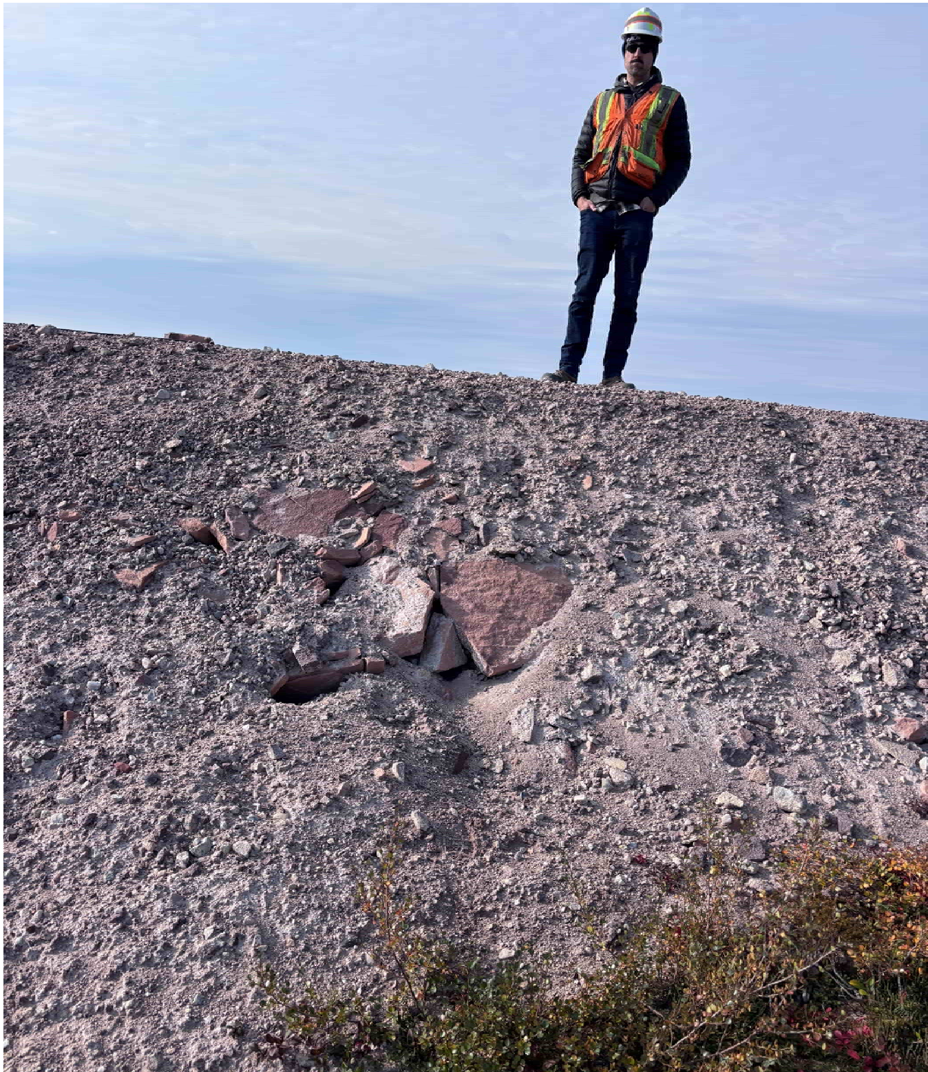
M-73: Eastern airstrip embankment
