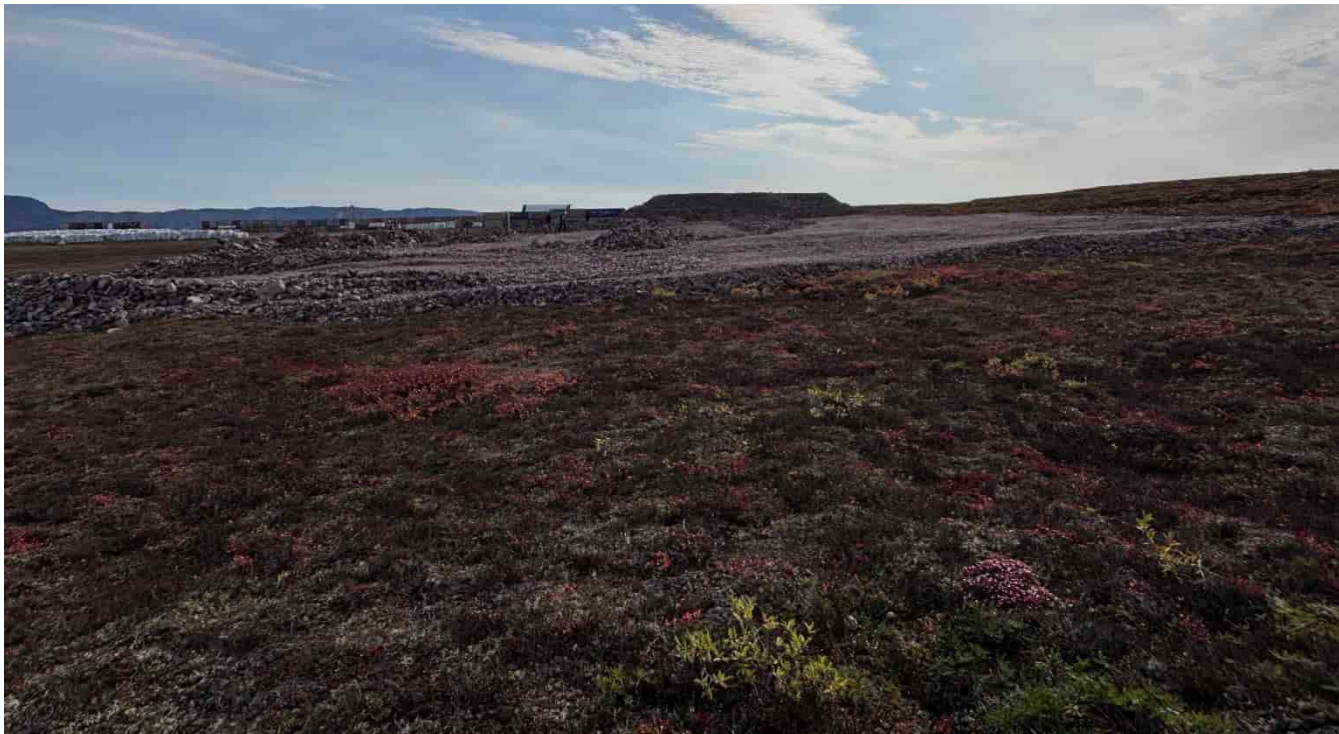
M-84: Airstrip extension, looking SE
