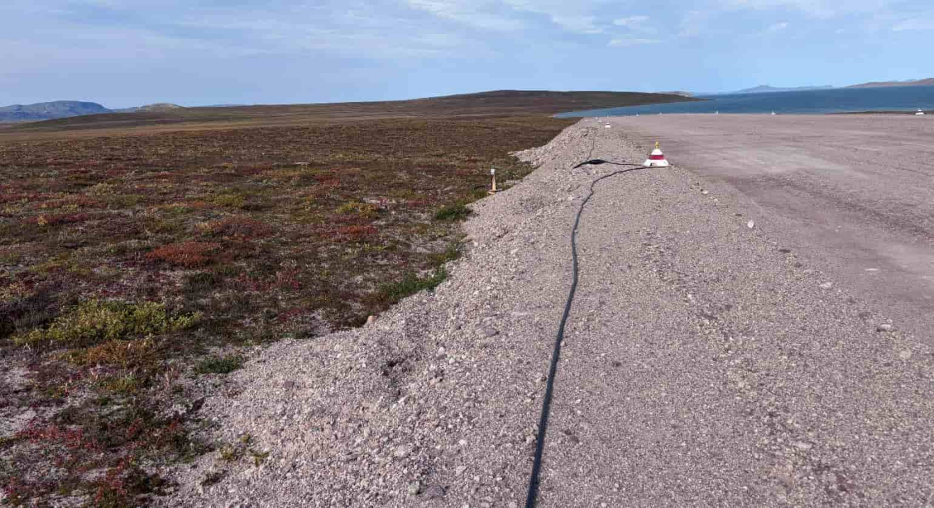
M-87: Western airstrip embankment, looking NW
