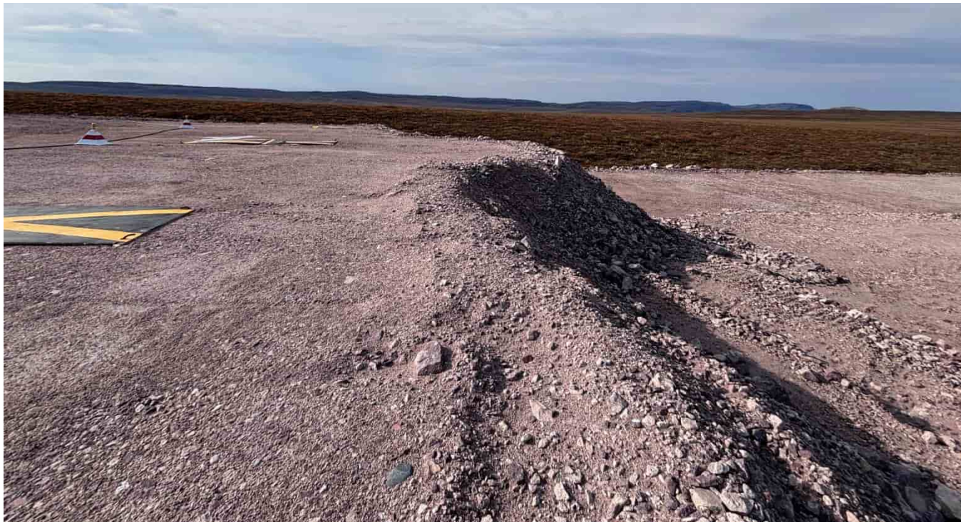
M-81: Slope between airstrip and extension, looking W
