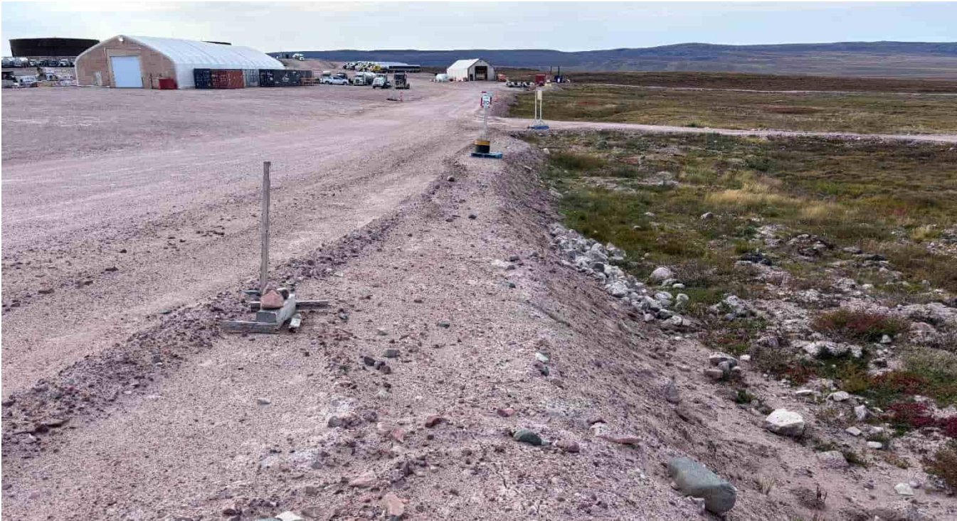
M-93: Road to tank farm
