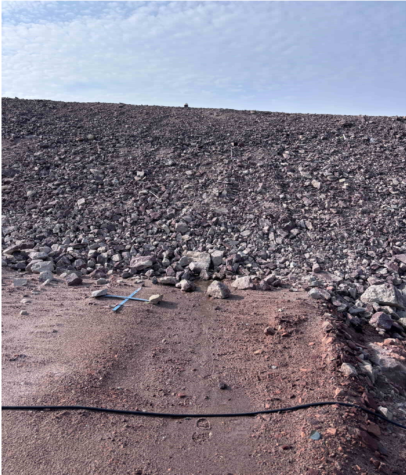
M-79: Eastern airstrip embankment tie-in to freight storage pad
