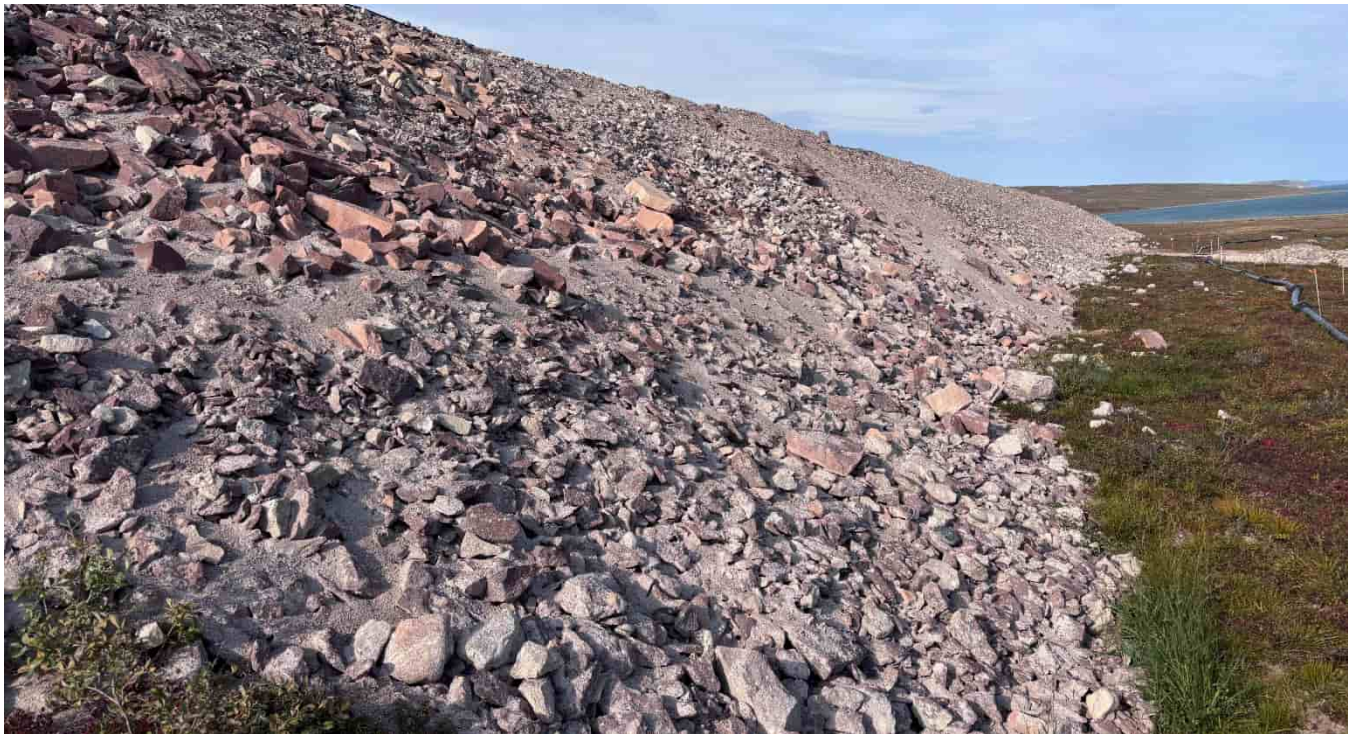
M-77: Typical embankment conditions
