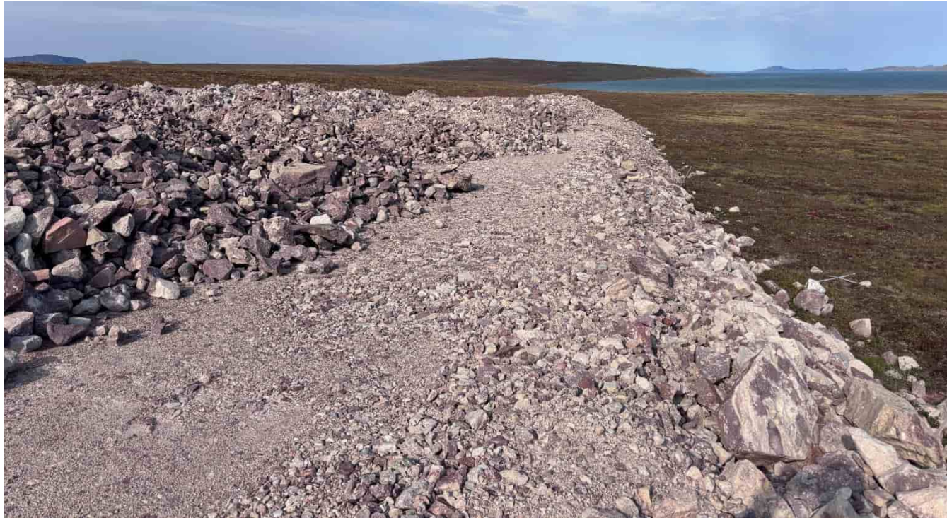
M-82: Airstrip extension placed in lifts
