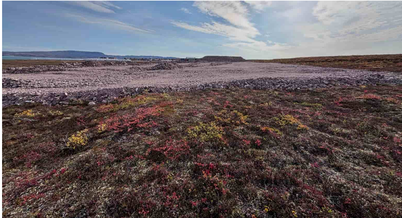
M-83: Airstrip extension, looking SE
