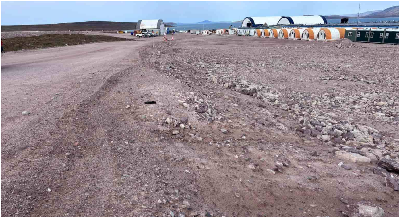
M-94: Access road to camp pad
