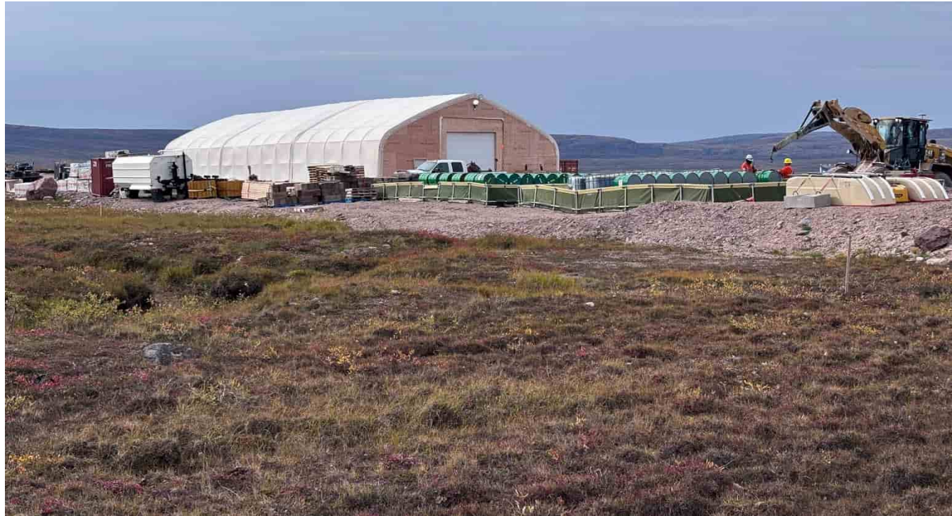
M-127: Pad between airstrip and tank farm, looking W
