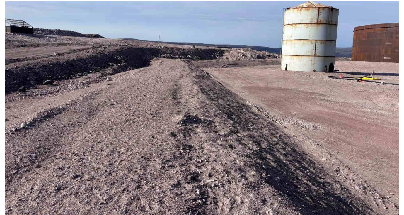
M-138: Tank farm southeastern berm, looking SW
