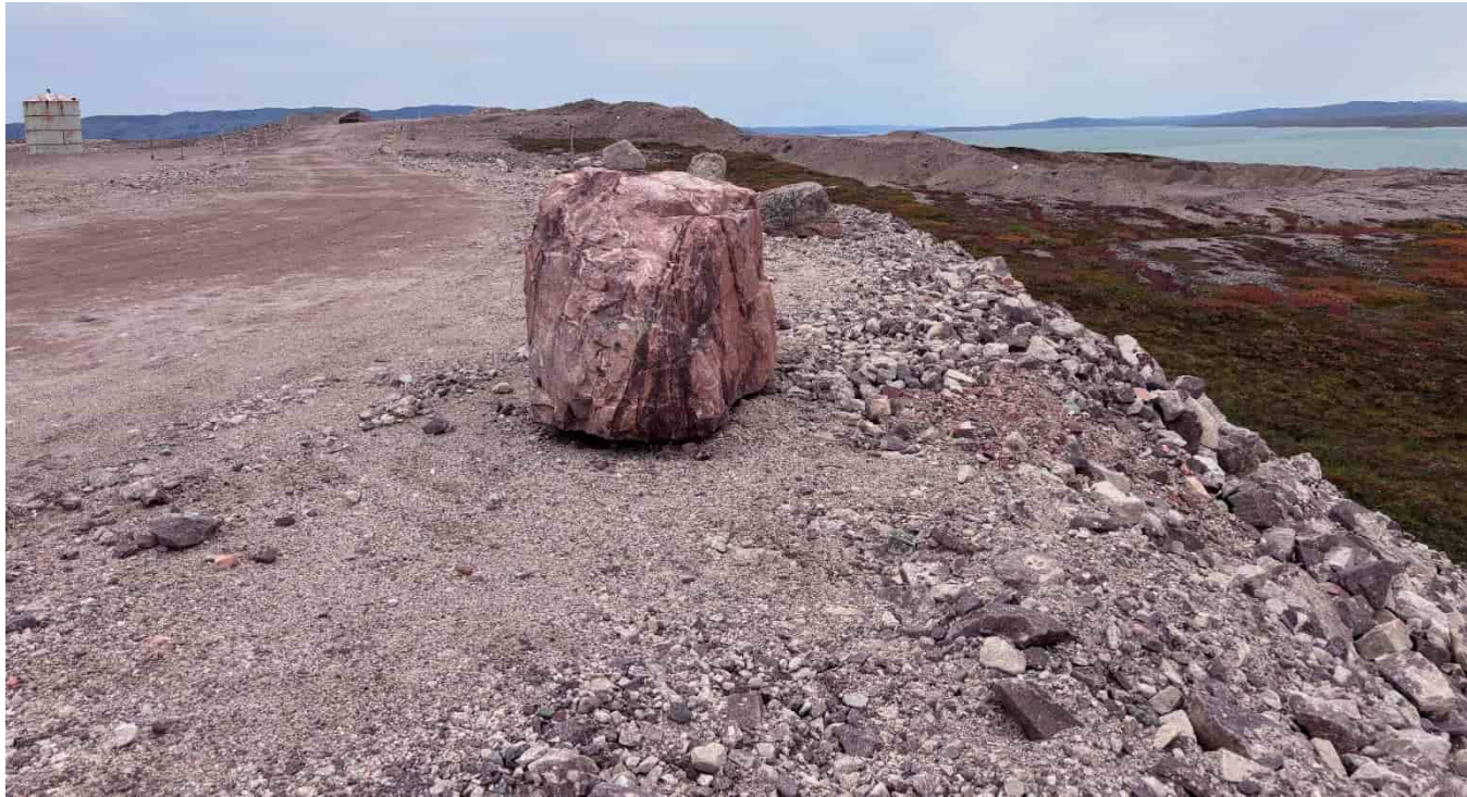
M-157: Access road for the fuel trucks at the SW corner of the tank farm, looking SE
