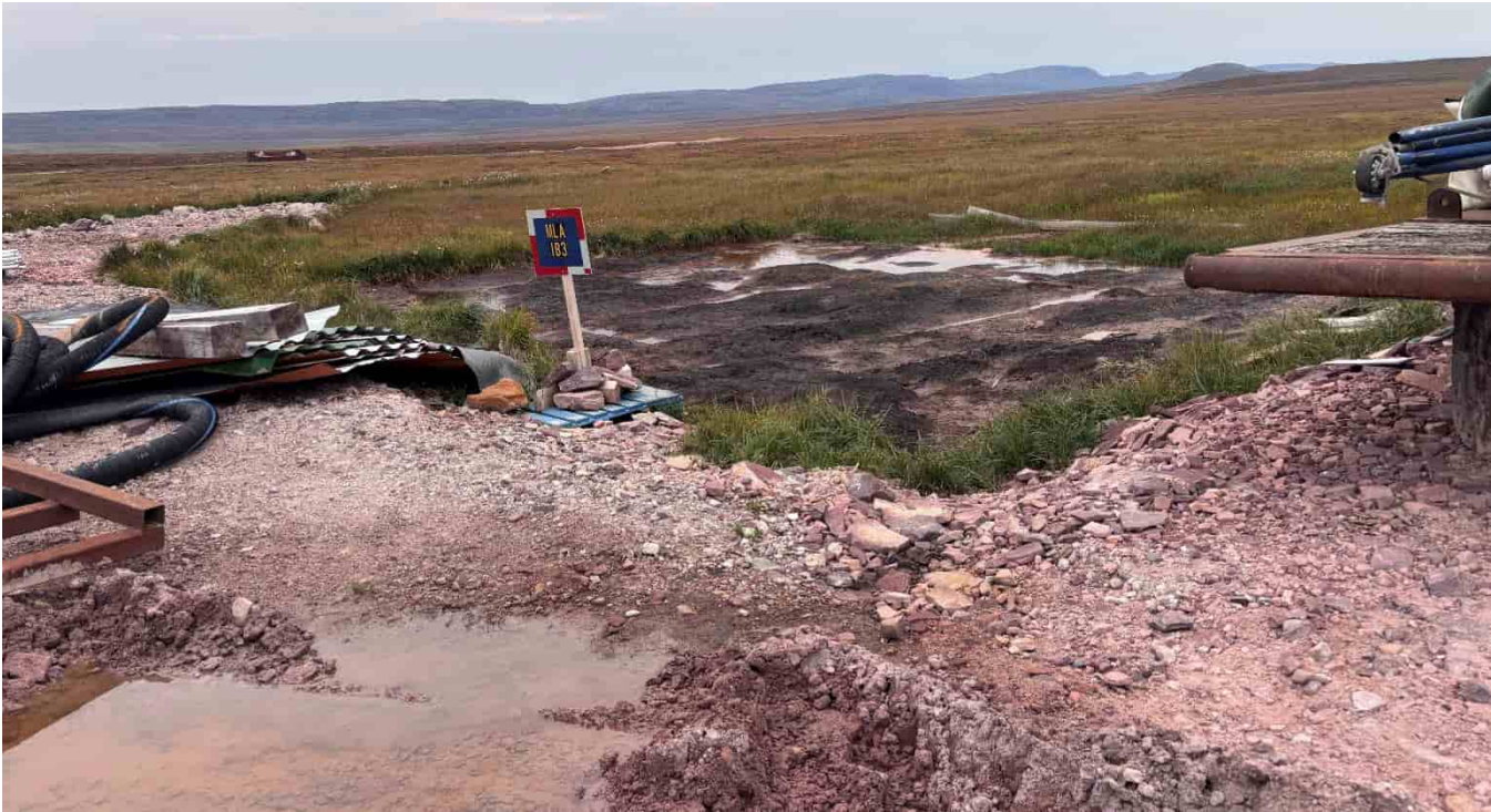
M-123: Ponding in laydown area
