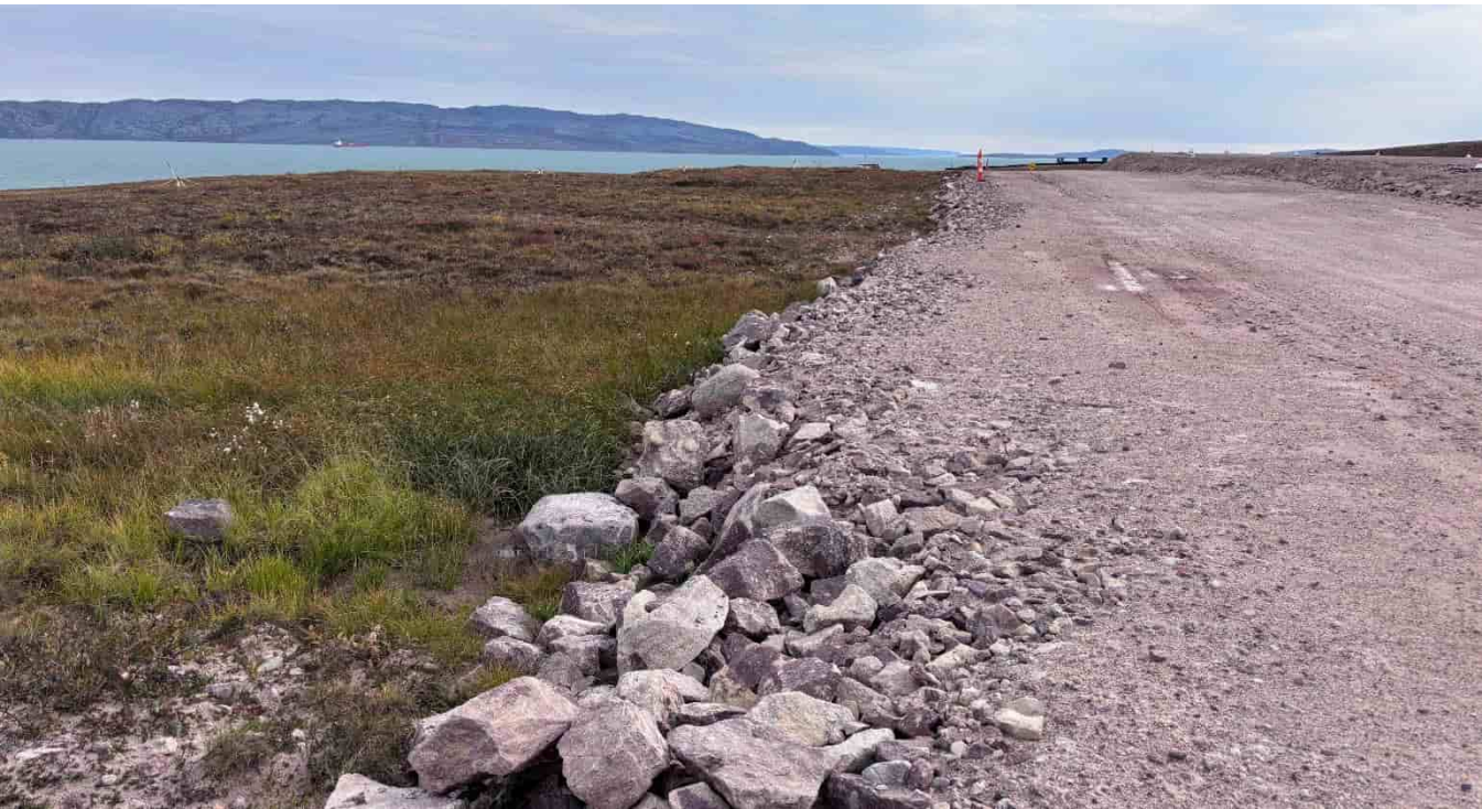
M-112: Access road embankment, looking SE
