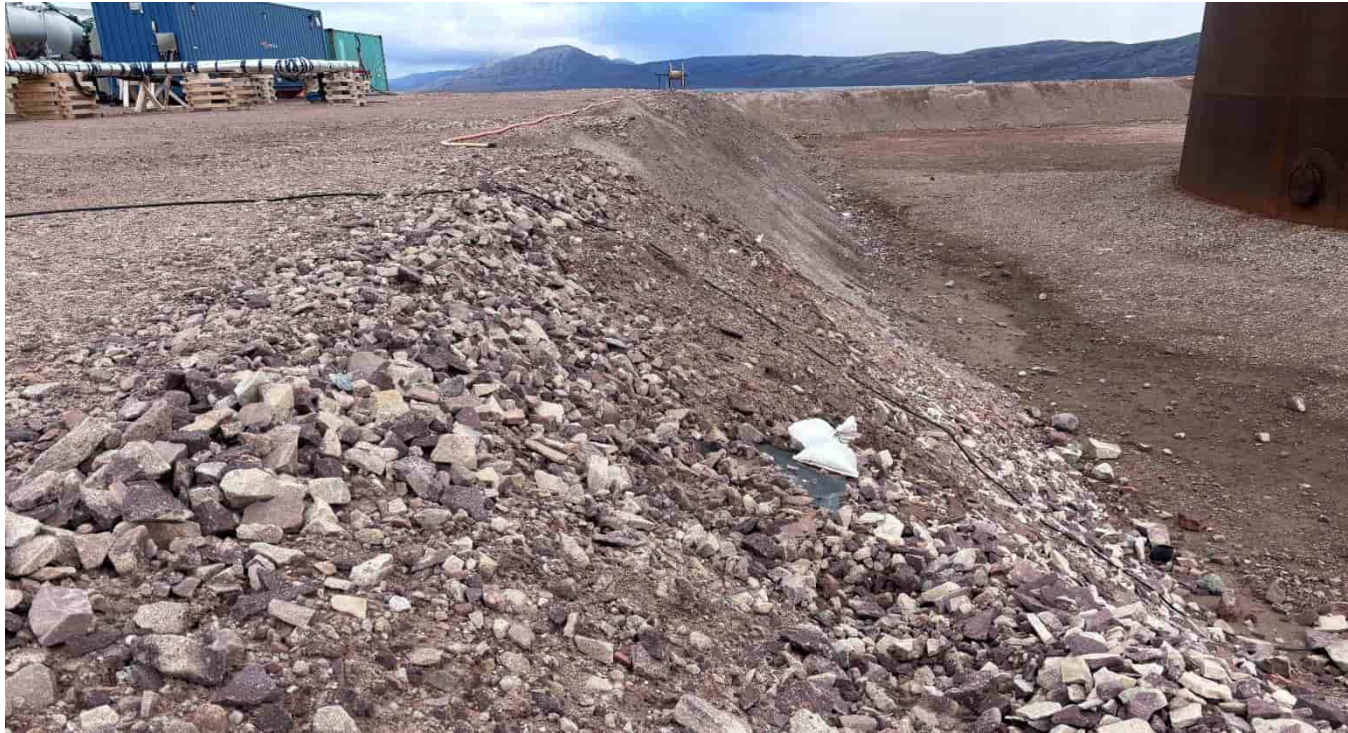
M-181: Pad slope between fireball and tank farm, looking N
