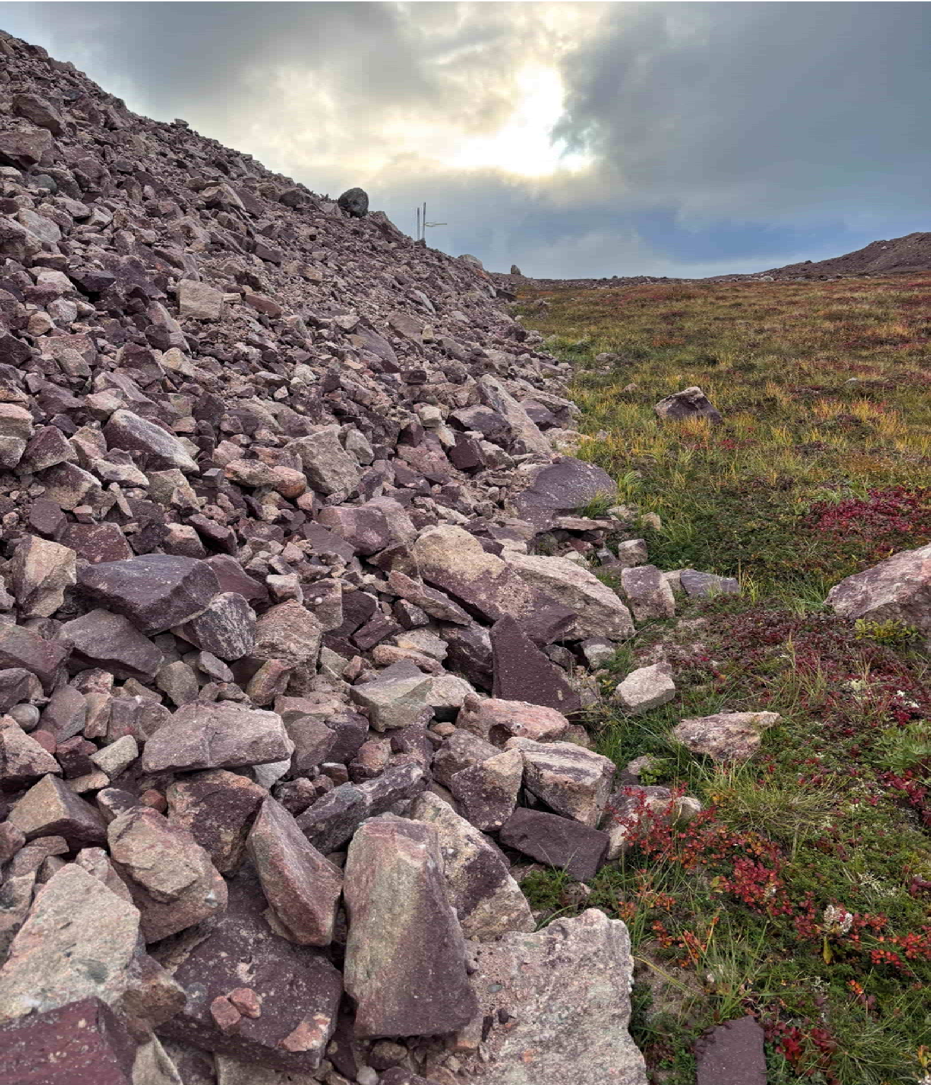
M-166: Toe of road embankment S of tank farm, looking E
