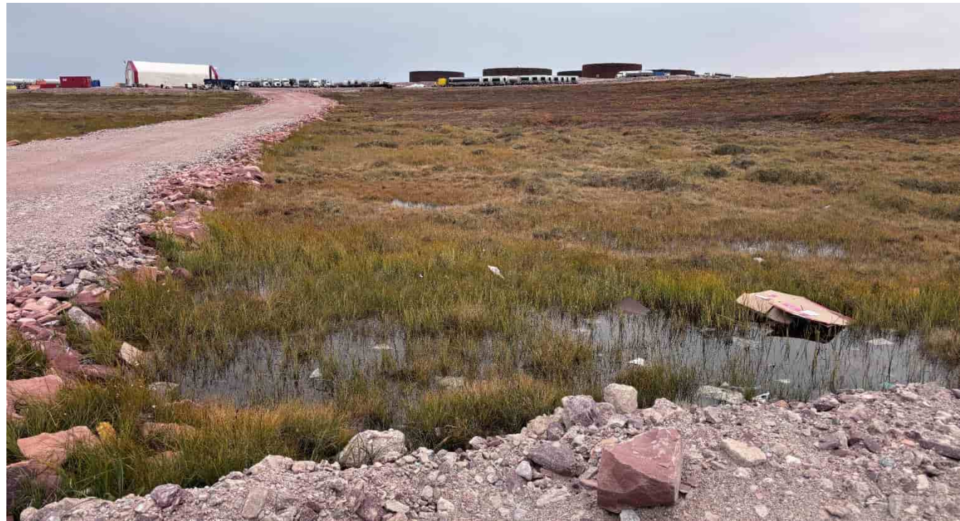
M-129: Ponding beside former explosives storage access road, looking SE
