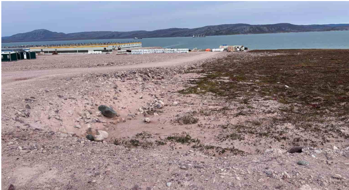
M-115: Camp pad laydown access road viewed from airstrip
