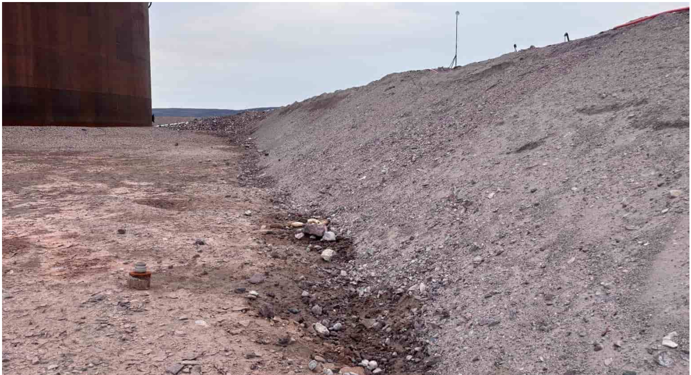
M-147: Toe of western berm, looking S
