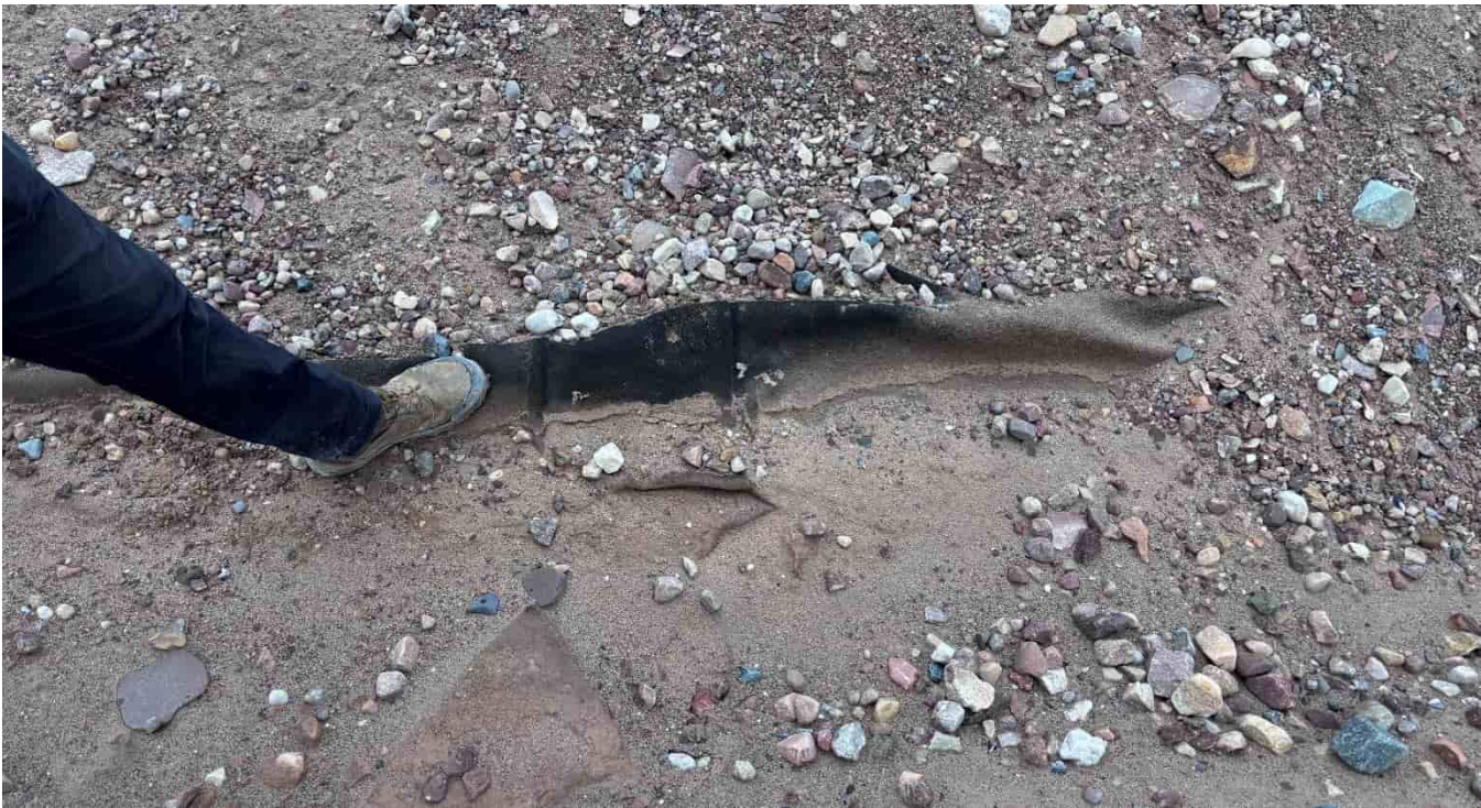
M-184: Exposed liner on slope between fireball and tank farm
