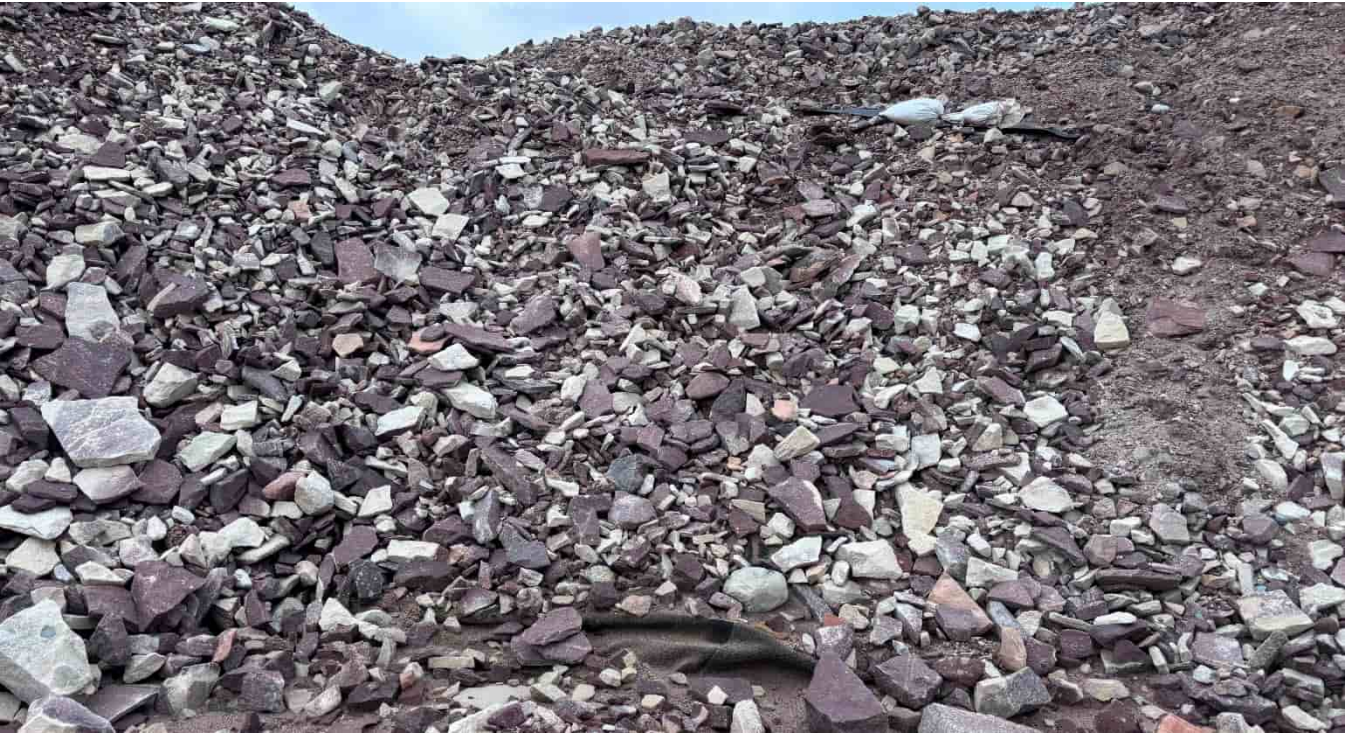
M-182: Exposed liner on slope between fireball and tank farm
