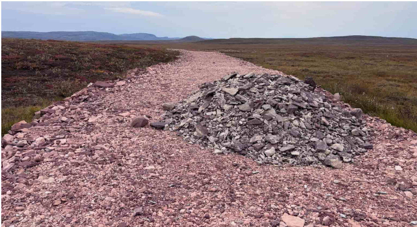
M-132: Rock pile on road
