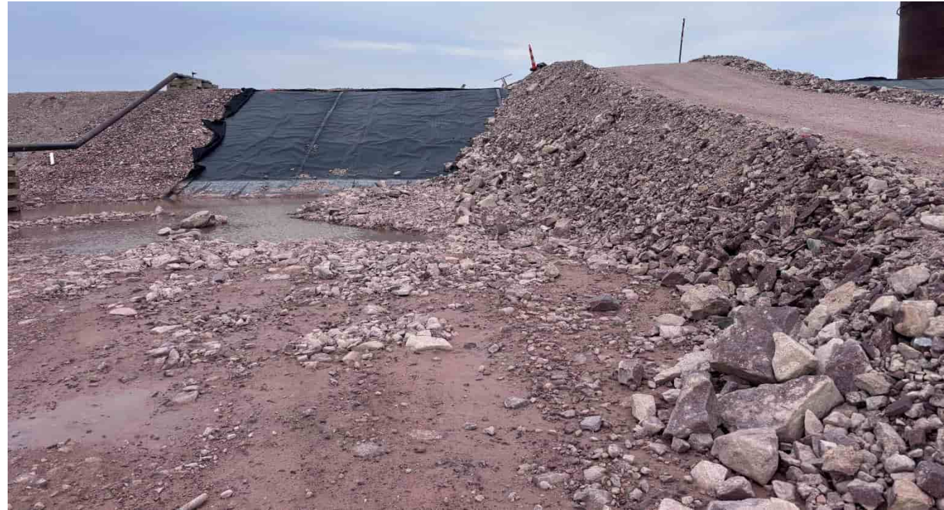
M-142: Northern embankment of entrance to tank farm
