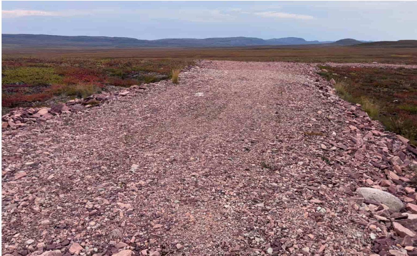
M-134: Northern end of former explosives storage access road
