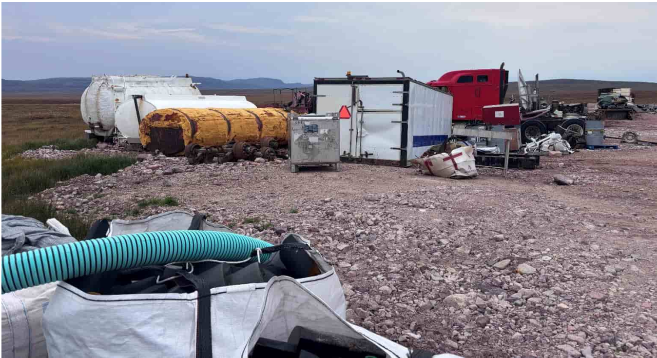
M-121: Laydown, looking NW
