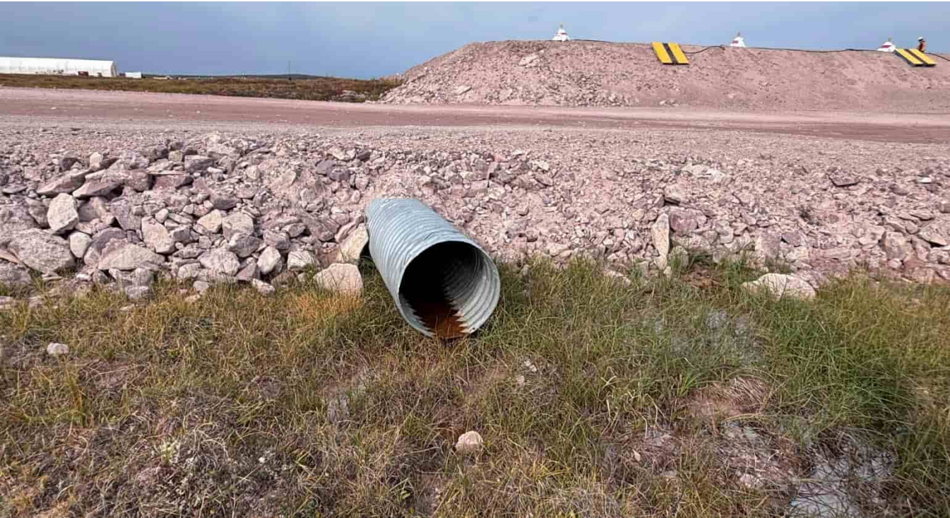
M-110: Culvert outlet under airstrip access road, beside SE end of airstrip
