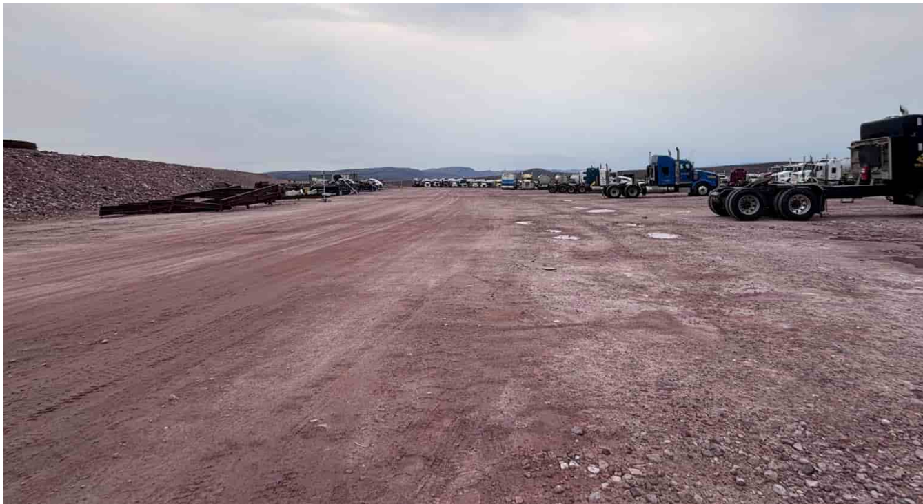
M-139: Truck laydown typical surface conditions
