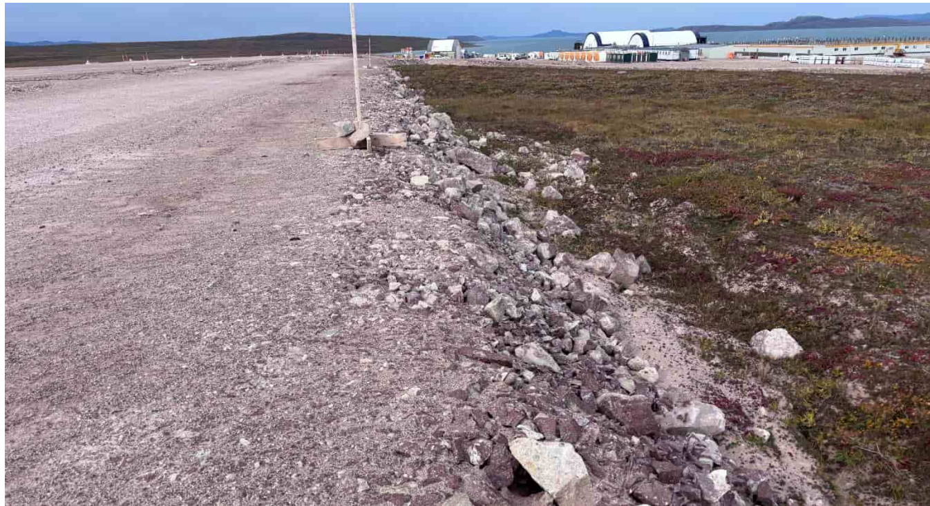
M-113: Access road embankment, looking NW
