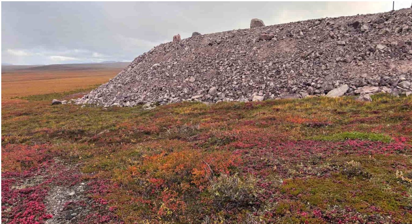
M-165: Tank farm pad NW corner, looking NE
