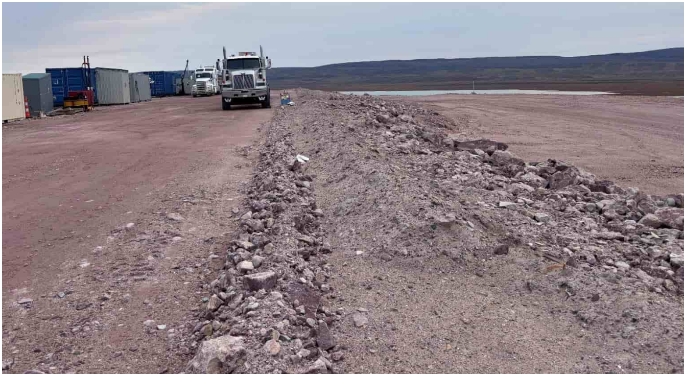
M-151: Berm at edge of fireball pad, looking S
