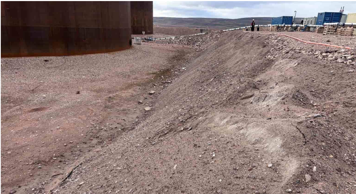
M-180: Erosion of slope below fireball
