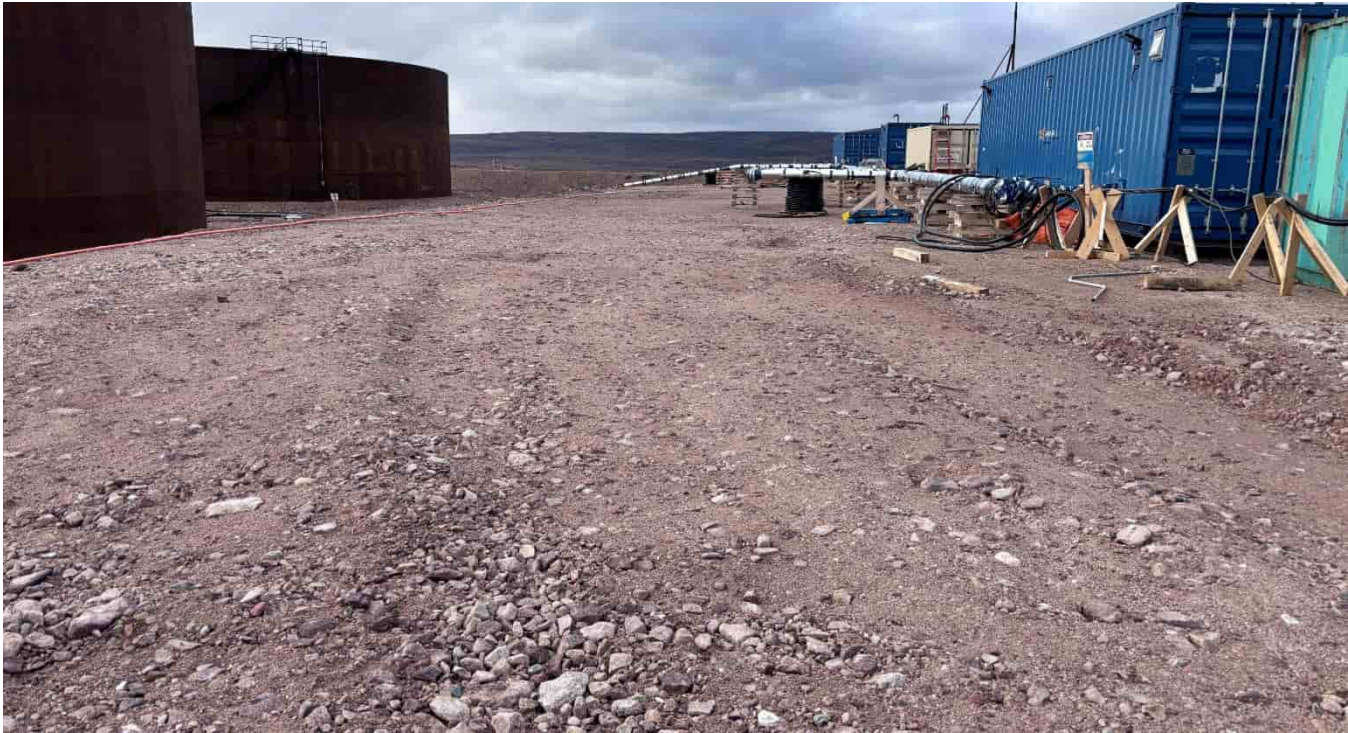
M-178: Pad between fireball and tank farm, looking SW
