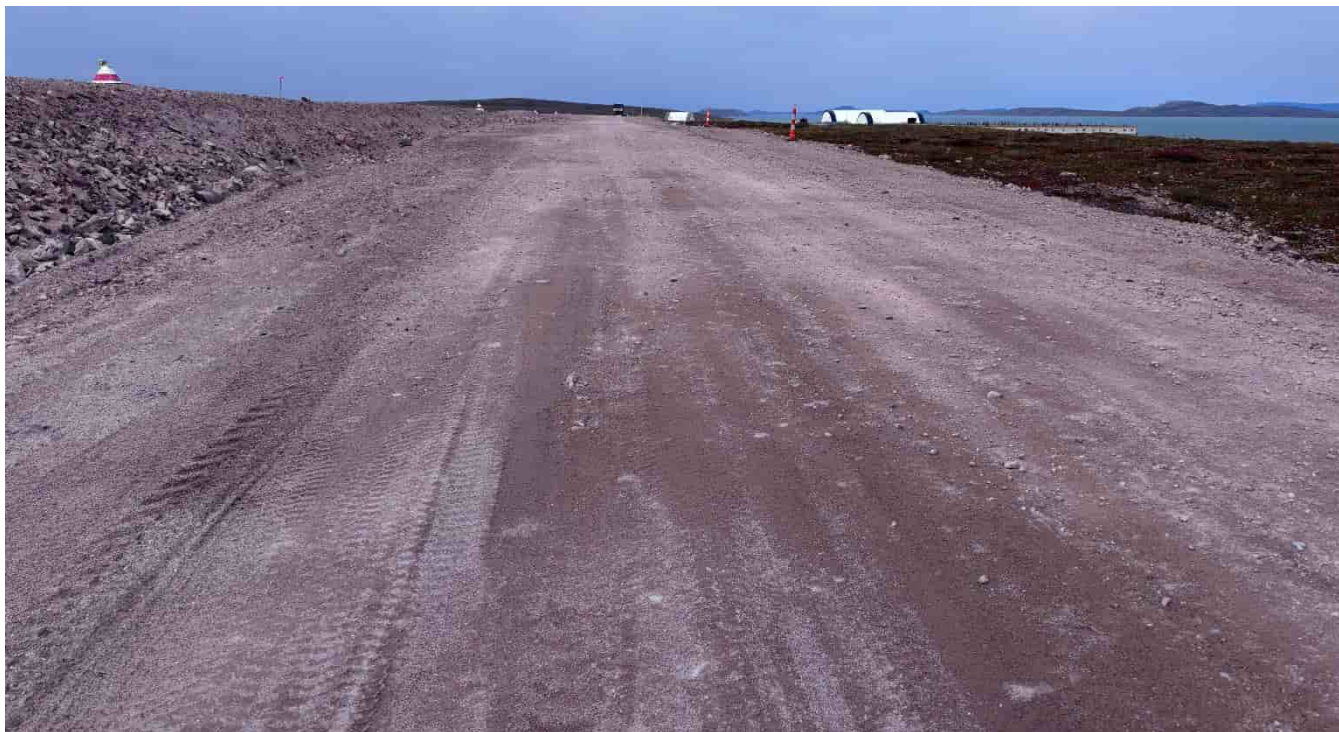
M-108: Airstrip and camp pad access road
