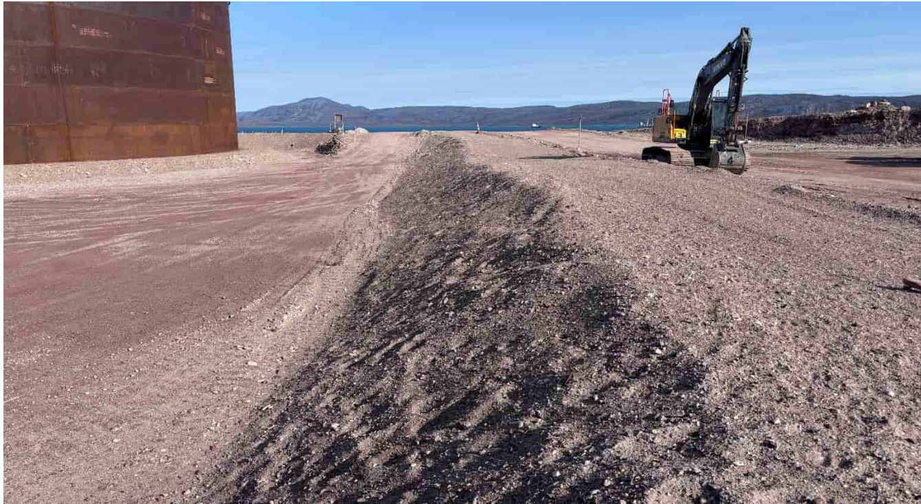
M-137: Tank farm eastern berm, looking N
