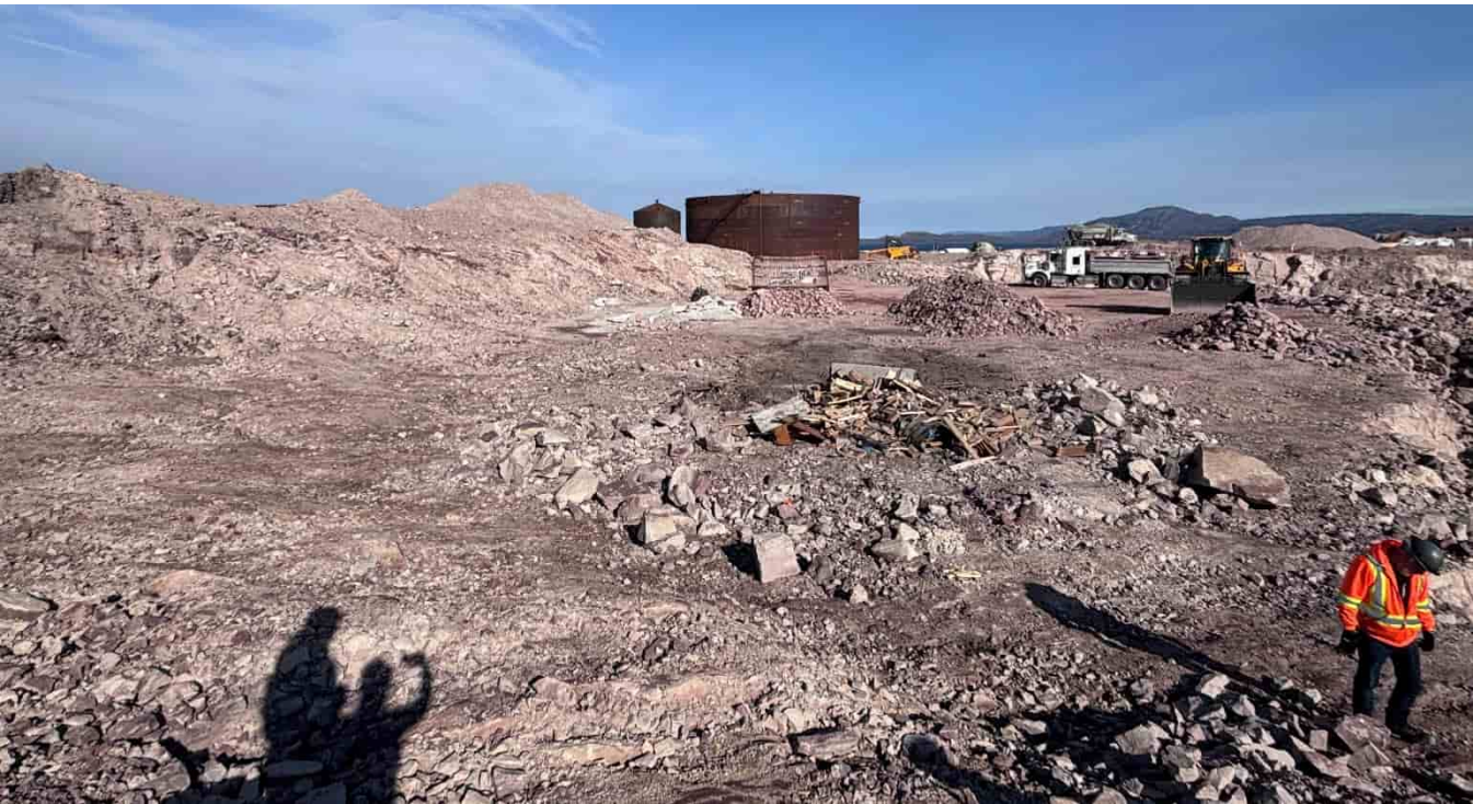
M-208: Looking NW
