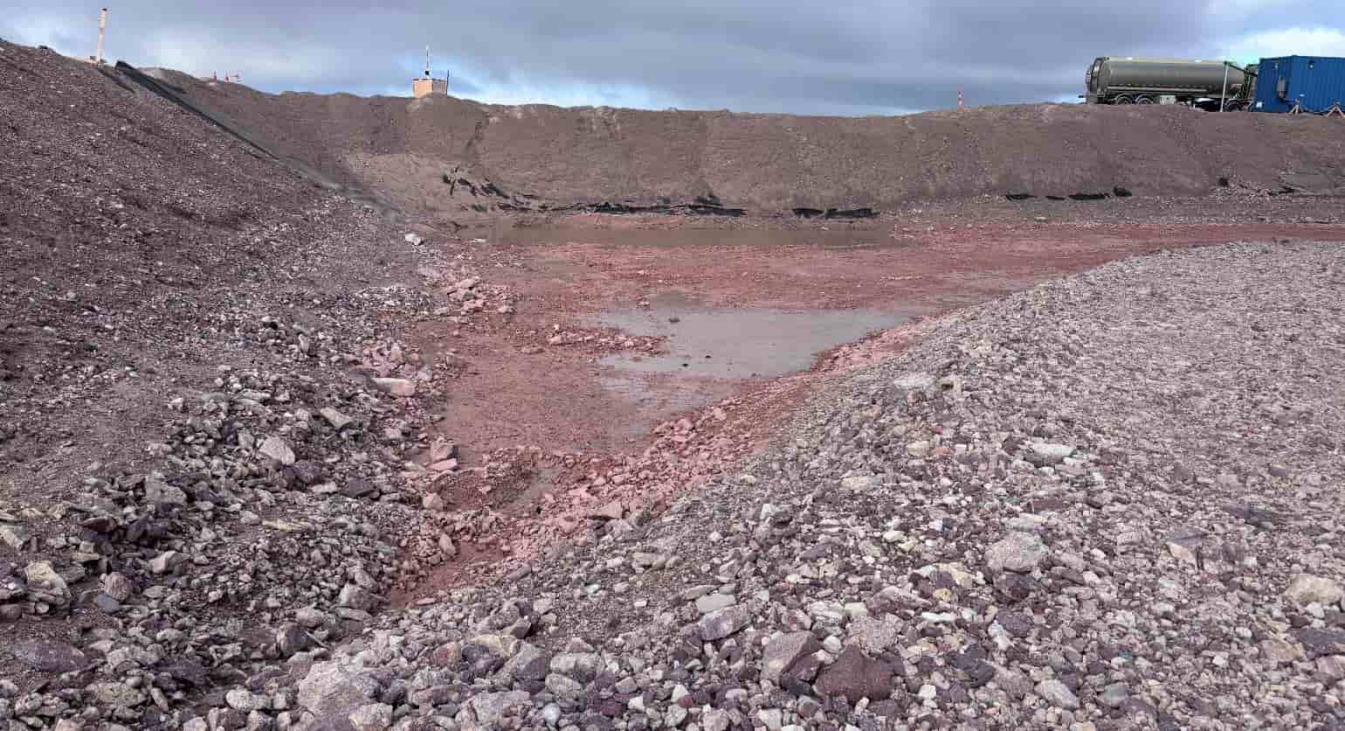
M-202: Ponding water at SW corner of tank farm, looking W
