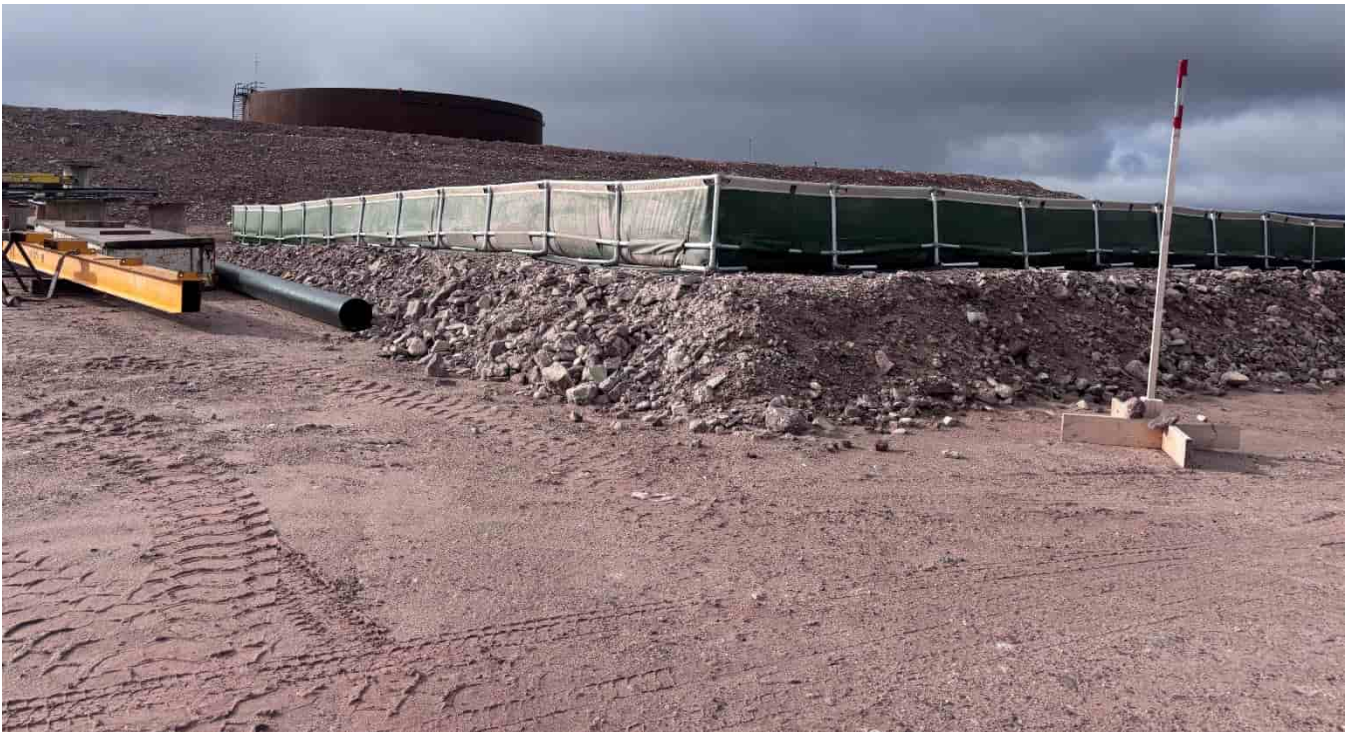
M-204: Ponds north of tank farm, looking SW
