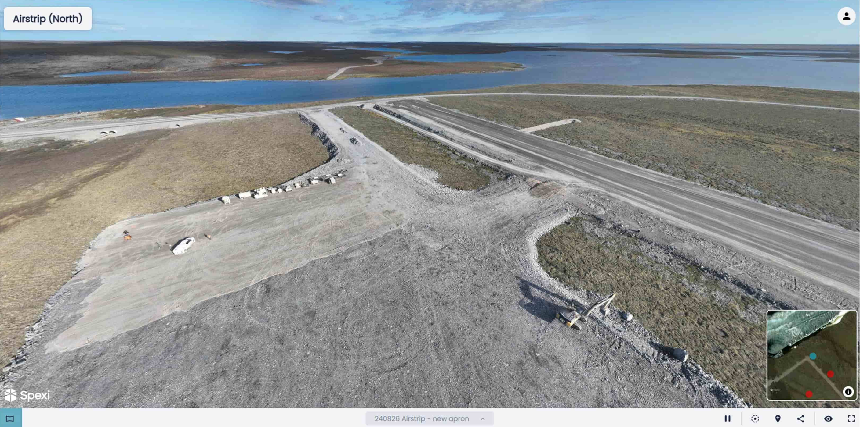
Figure 16 - Aerial image of Goose Airstrip: SW apron construction, looking N
