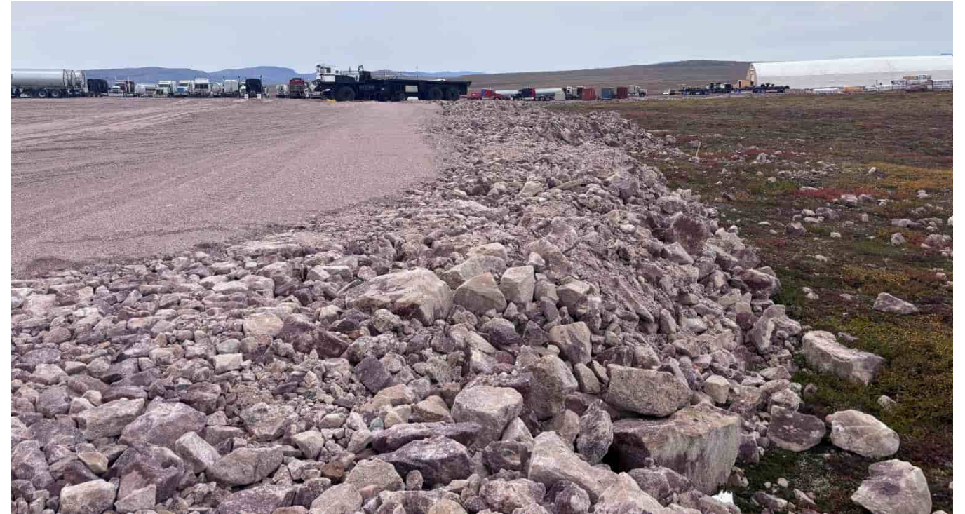
M-228: Edge of truck laydown pad, looking NW
