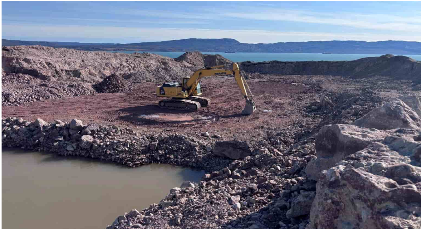
M-211: Quarry, looking E
