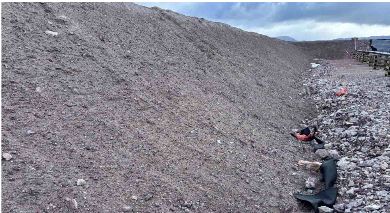
M-187: Exposed liner beneath fill at toe of northern berm, looking E
