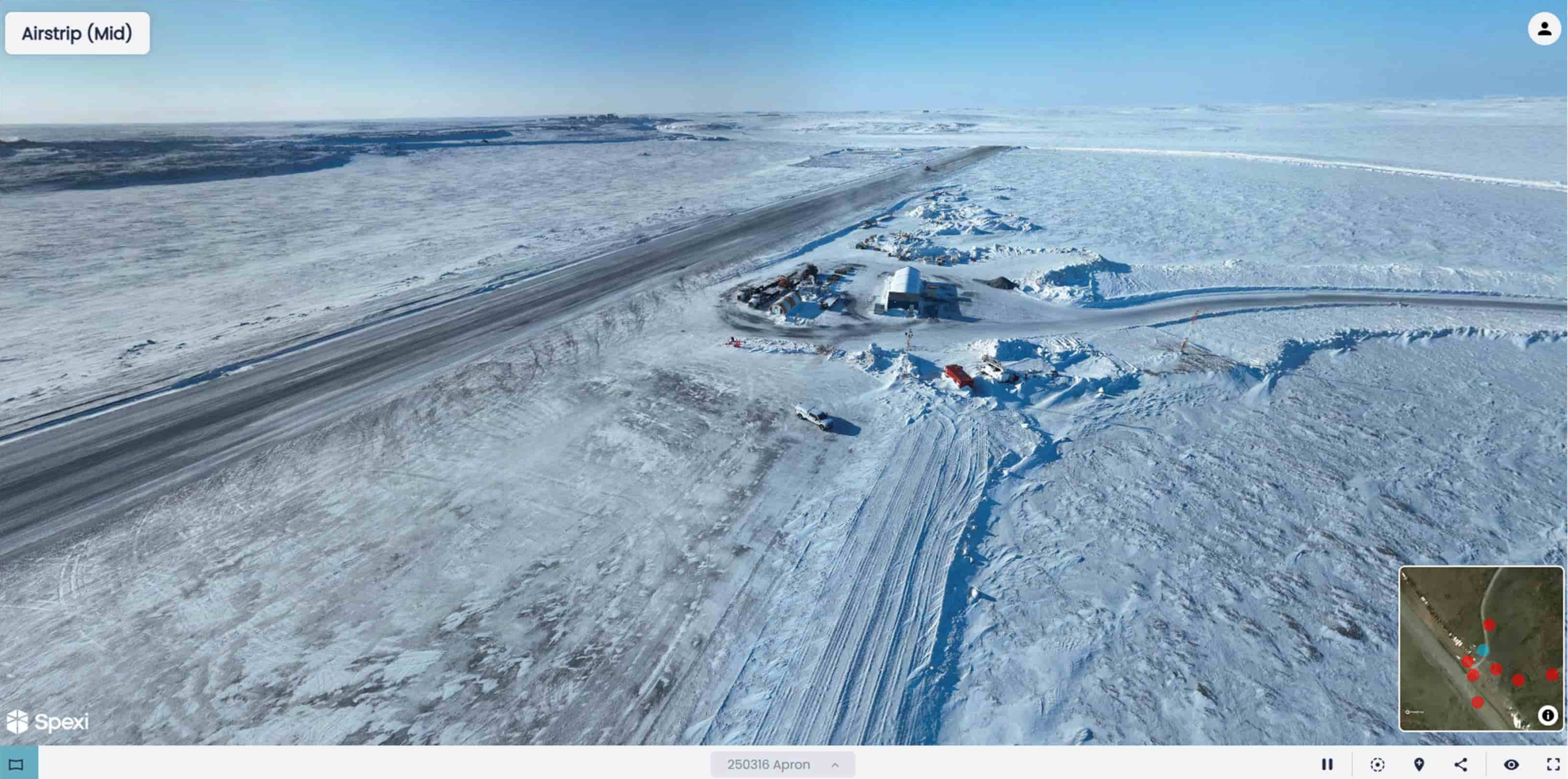
Figure 23 - Aerial image of Goose Airstrip: Looking towards the NW end of the Airstrip
