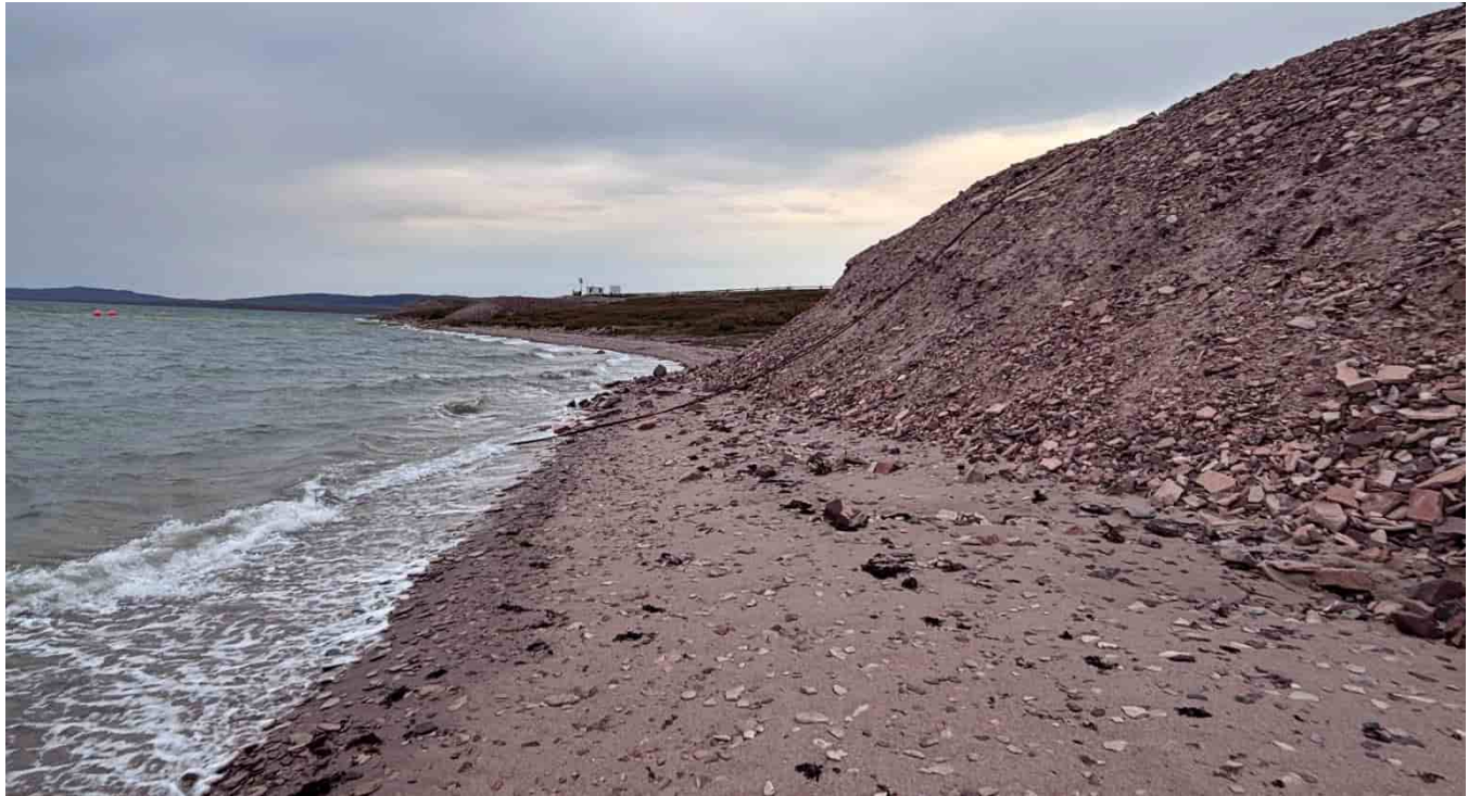
M-241: North pad slope along shoreline – Note oversteepened slope
