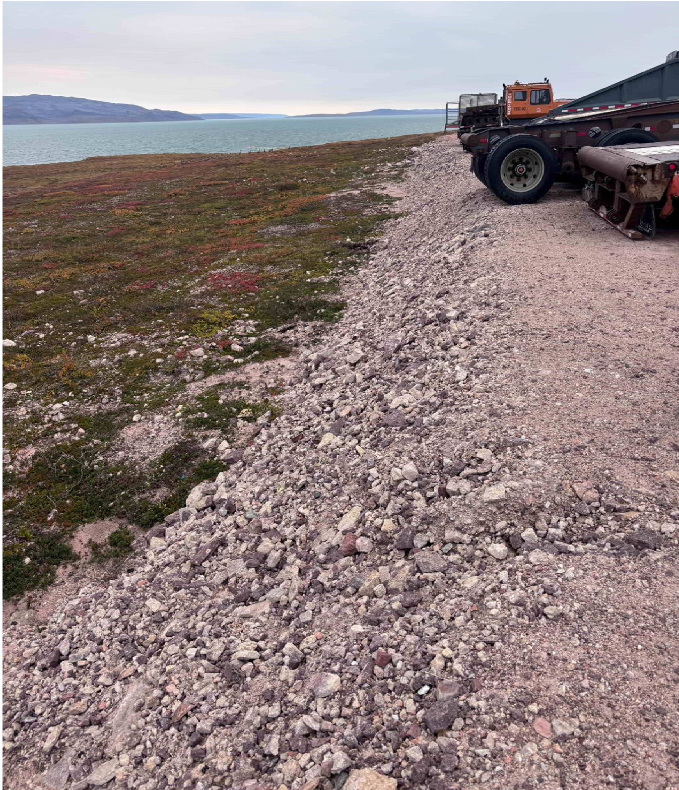
M-231: Truck parking at edge of pad beside fuel offload access road
