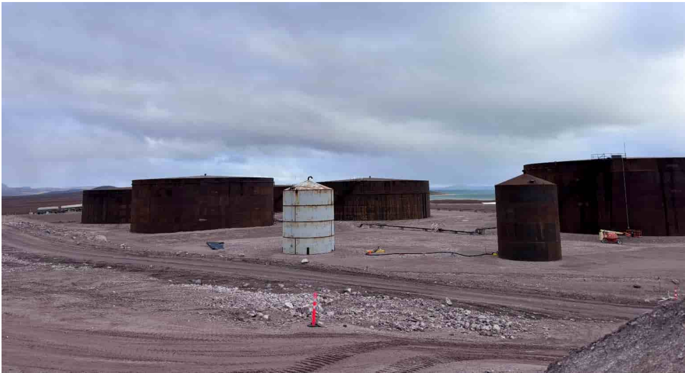
M-224: Tank farm viewed from quarry
