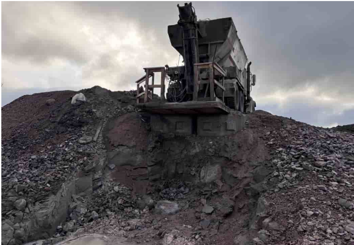
M-215: Batch plant east to the quarry. Note the deck doesn't have support
