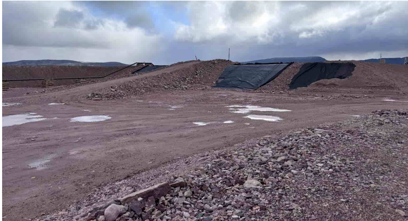
M-198: Entrance road to tank farm, looking NE
