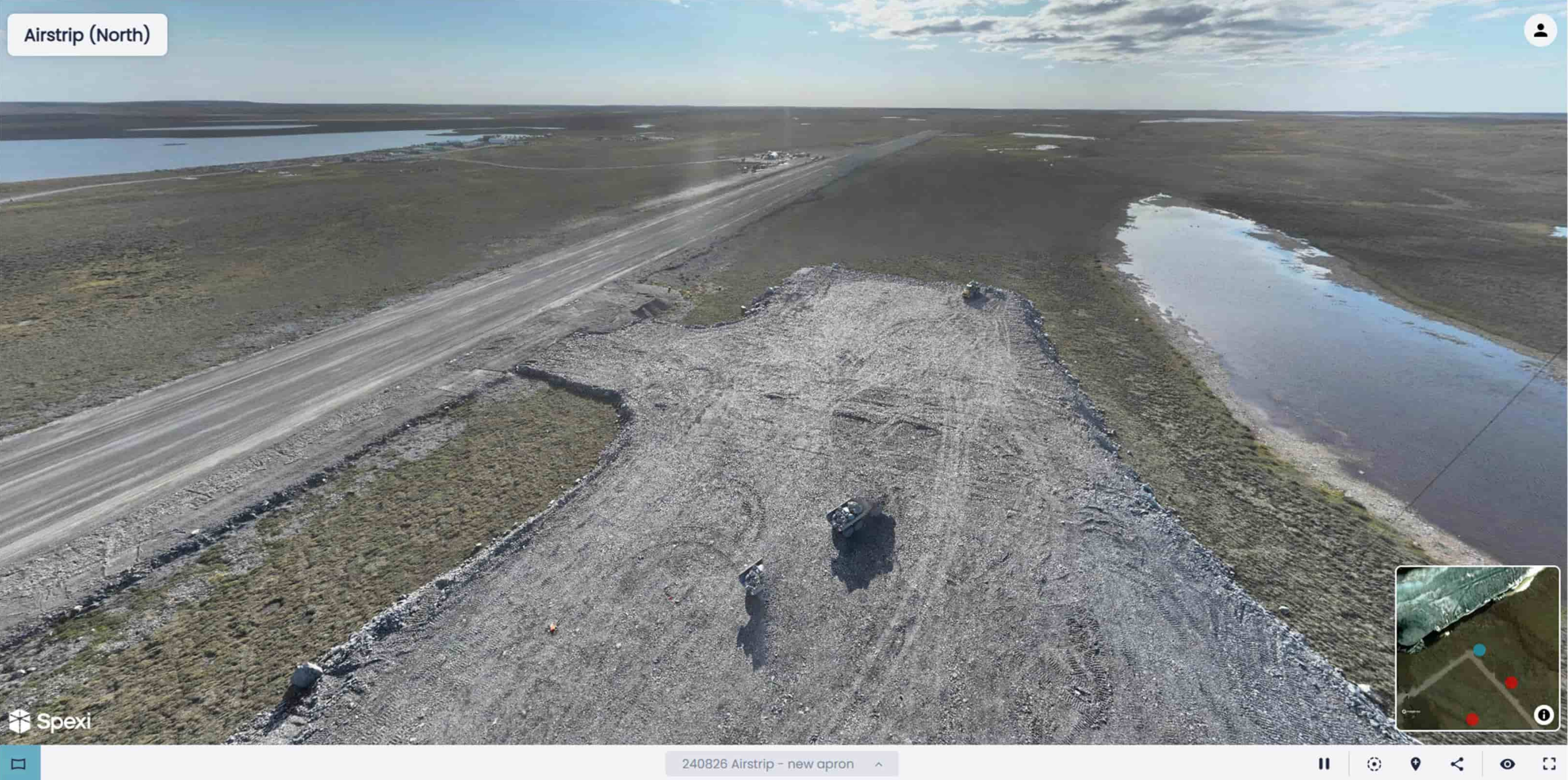
Figure 17 - Aerial image of Goose Airstrip: SW apron construction, looking SE
