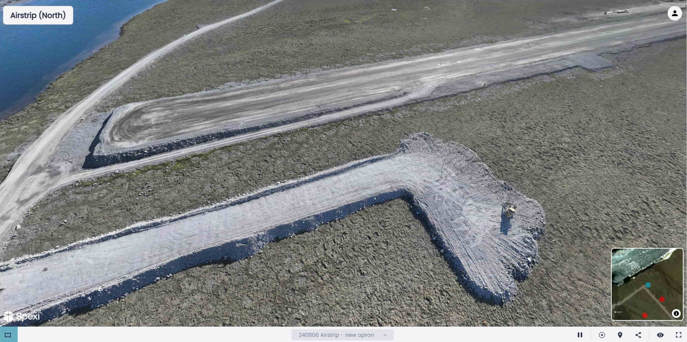
Figure 14 - Aerial image of Goose Airstrip: SW apron construction
