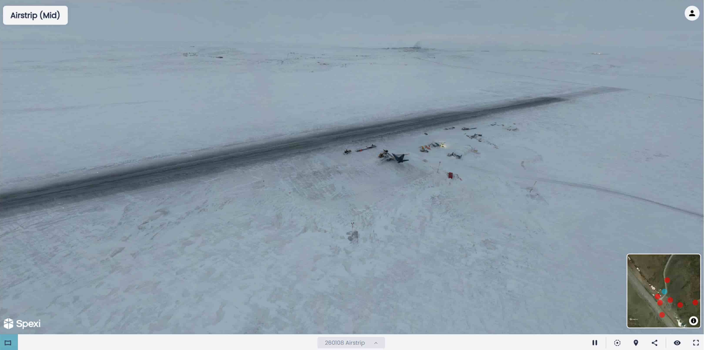
Figure 32 - Aerial image of Goose Airstrip: Looking W at the NW side of the Airstrip
