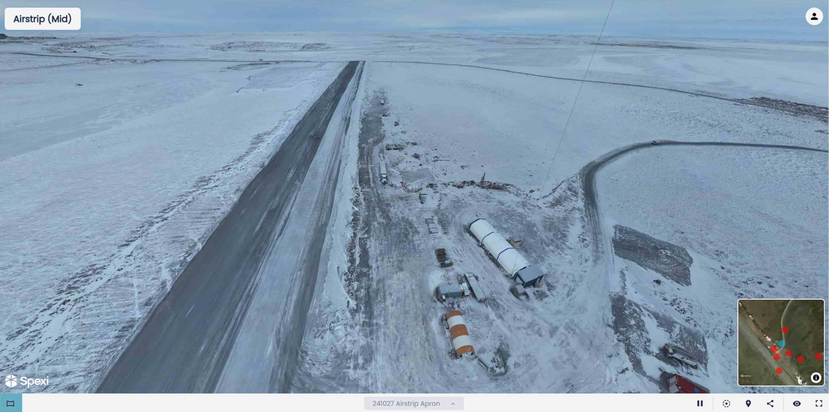
Figure 20 - Aerial image of Goose Airstrip: Looking NW from center of Airstrip
