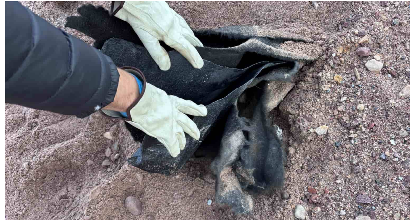
M-192: Damaged liner on eastern berm
