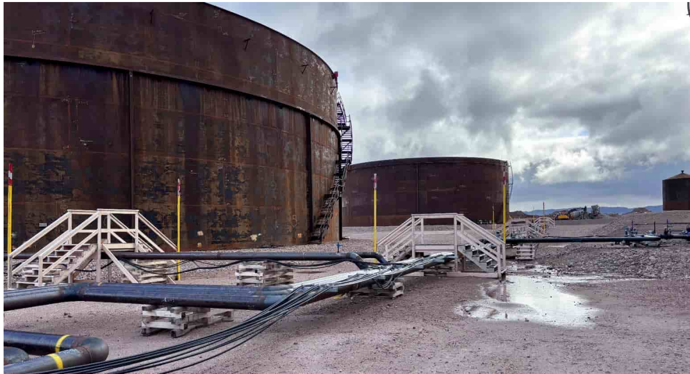
M-200: Typical piping layout and surface conditions – Note ponding water
