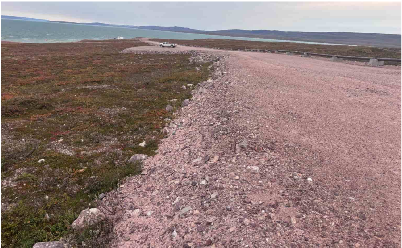
M-236: Typical road embankment, looking S
