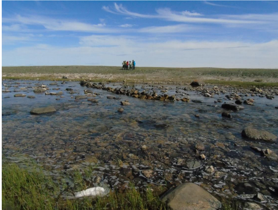
Photo 7.3-2 Directional Weir (Kugluktuk HTO students in background) for migrating Arctic char in Nulahugyuk Creek, June 24, 2015.
