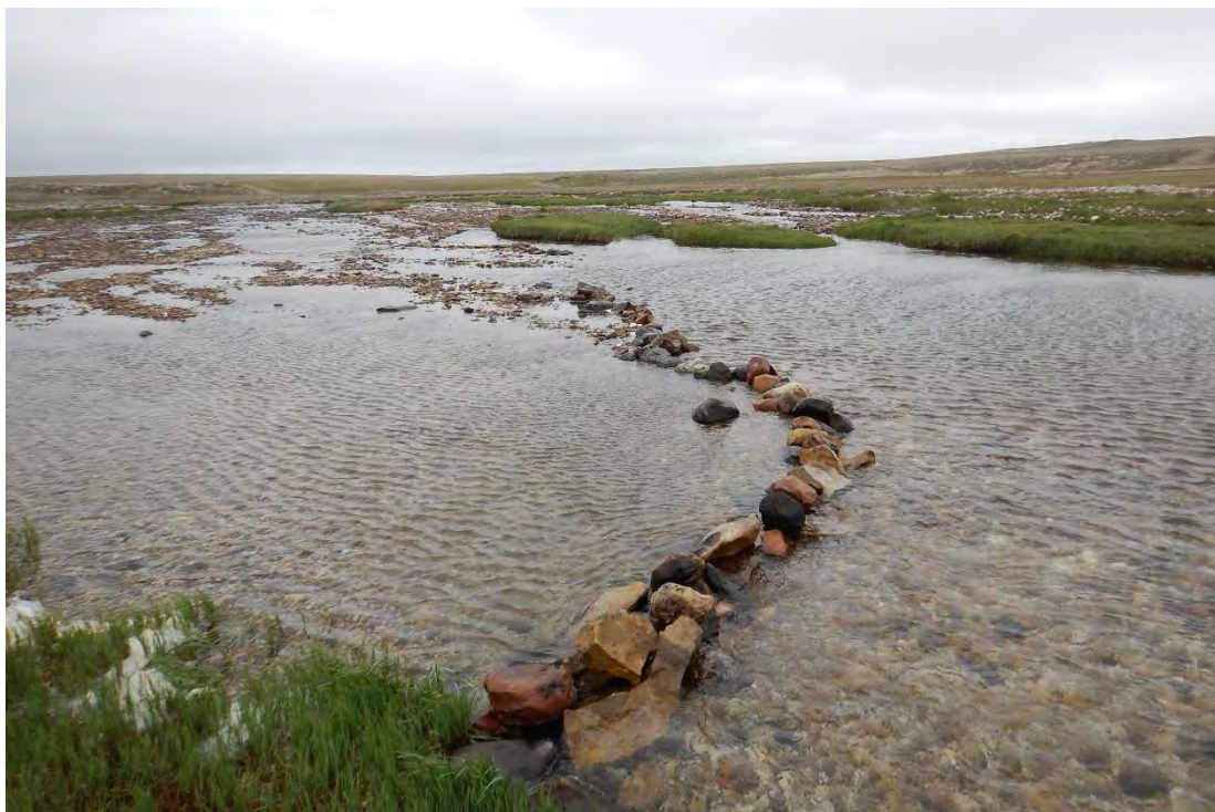
Photo 3-9: 2012 Project 5, Showing Repaired Directional Weir Near Right Downstream Bank, 15 July 2016
