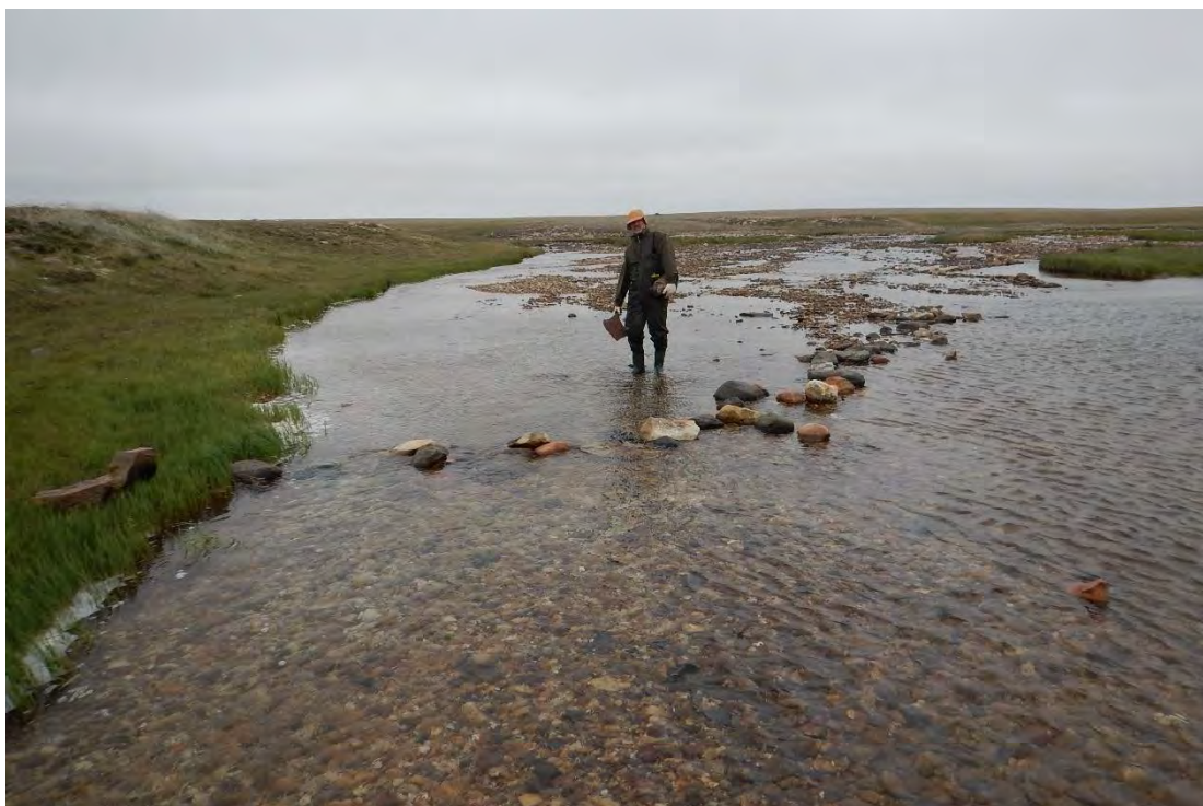
Photo 3-8: 2012 Project 5, Showing Failed Directional Weir Near Right Downstream Bank, 15 July 2016
