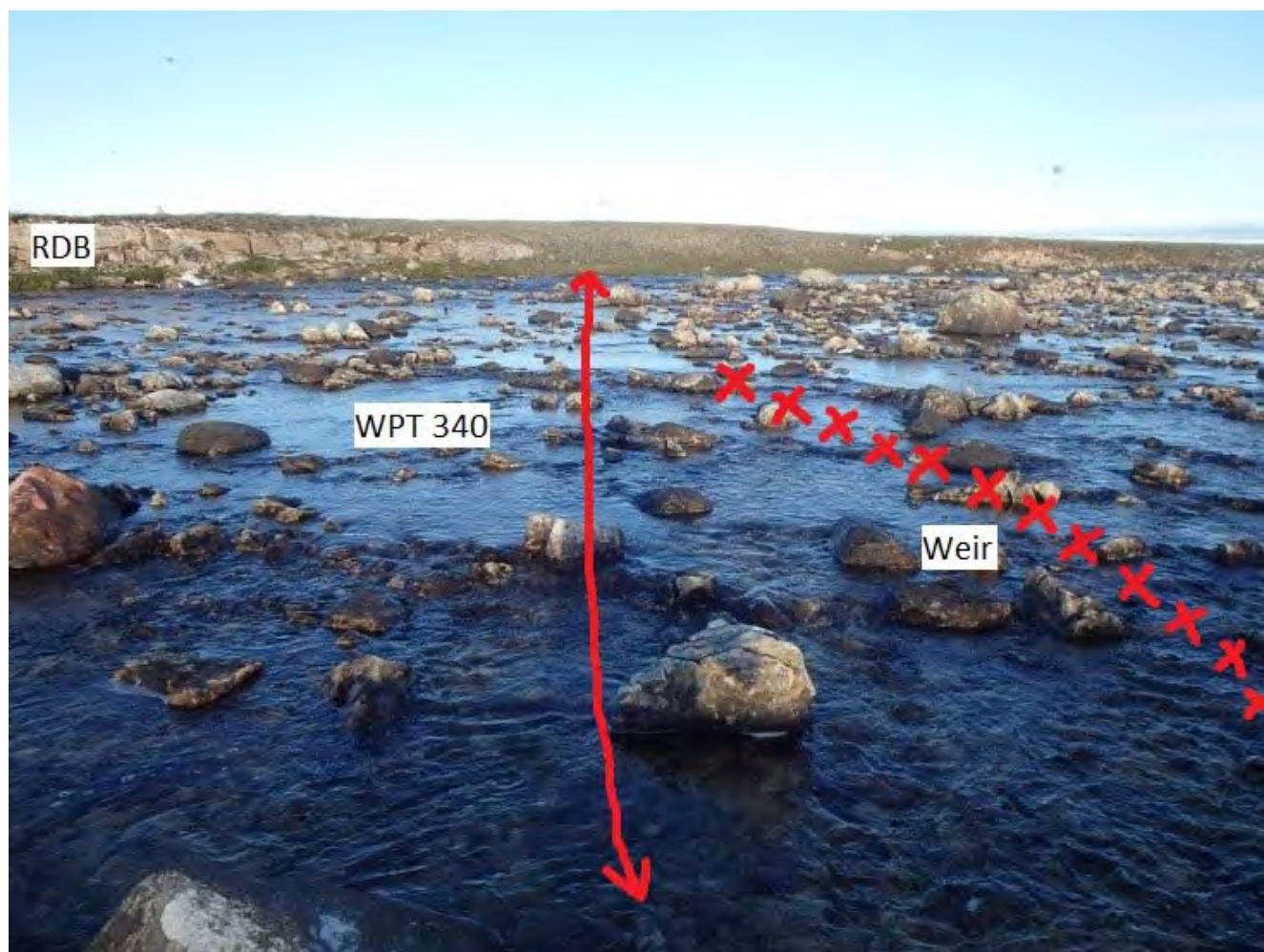
Photo C30: Looking upstream towards proposed Low-Flow Channel Site 9 showing where channel and directional weir should be constructed.
