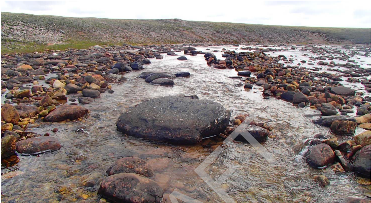
Photo 55: Upstream view from the centre of the low-flow channel constructed at Site 11. The photograph shows large boulders left within channel to act as cover for migratory fish. 20 July 2016.
