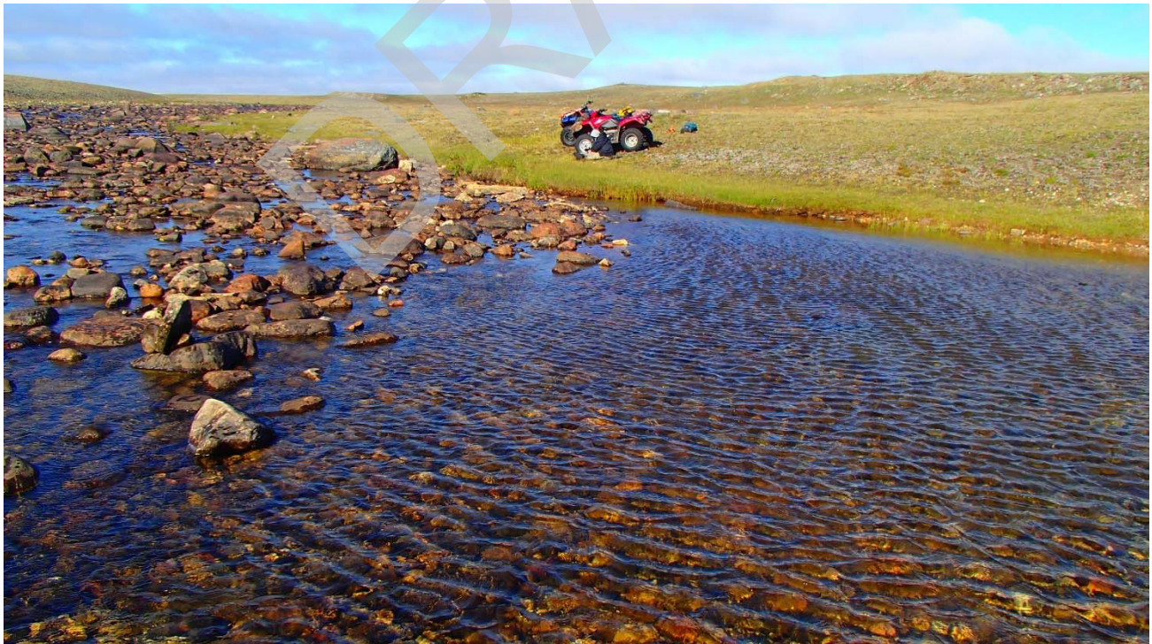
Photo 40: Upstream view from the pool located along the LDB at the downstream extent of Site 7 prior to remediation. Note the absence of an unobstructed path for fish along the LDB. 24 July 2016.
