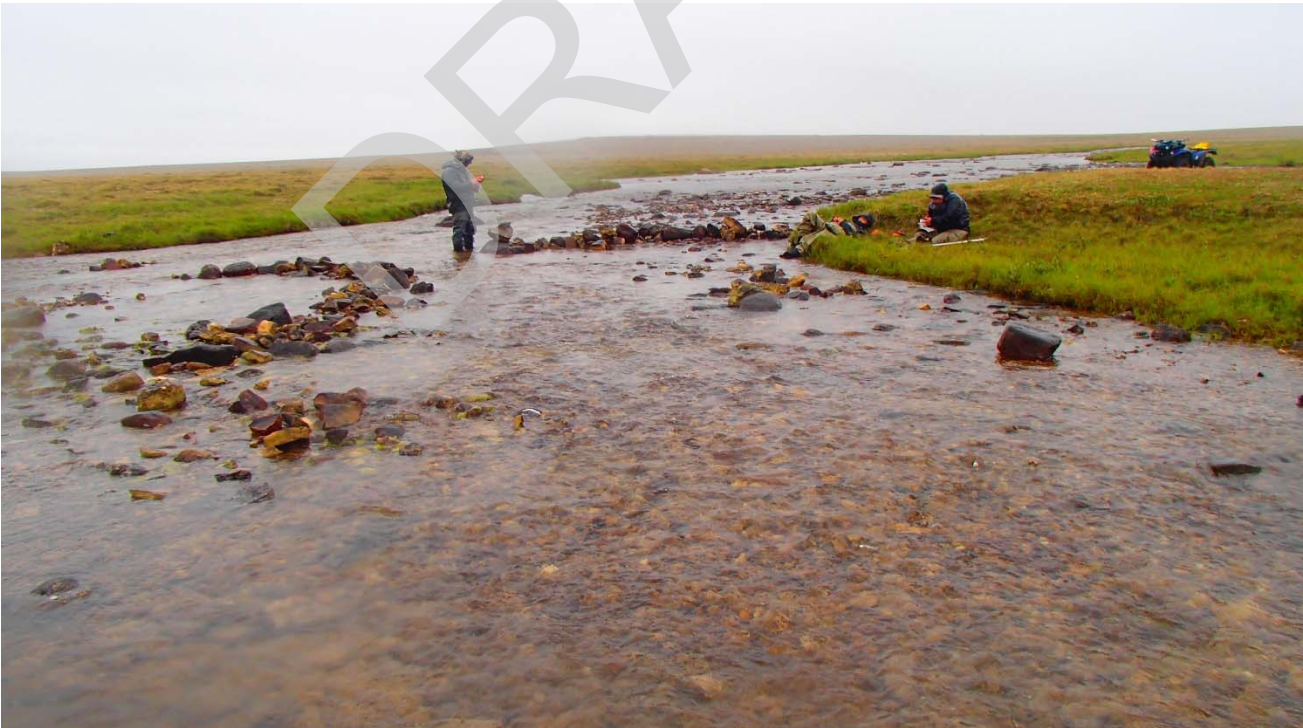
Photo 52: Upstream view of low-flow channel C and weir A constructed at Site 10. The channel provides passage toward the thalweg and the weir directs fish towards the RDB. 22 July 2016.
