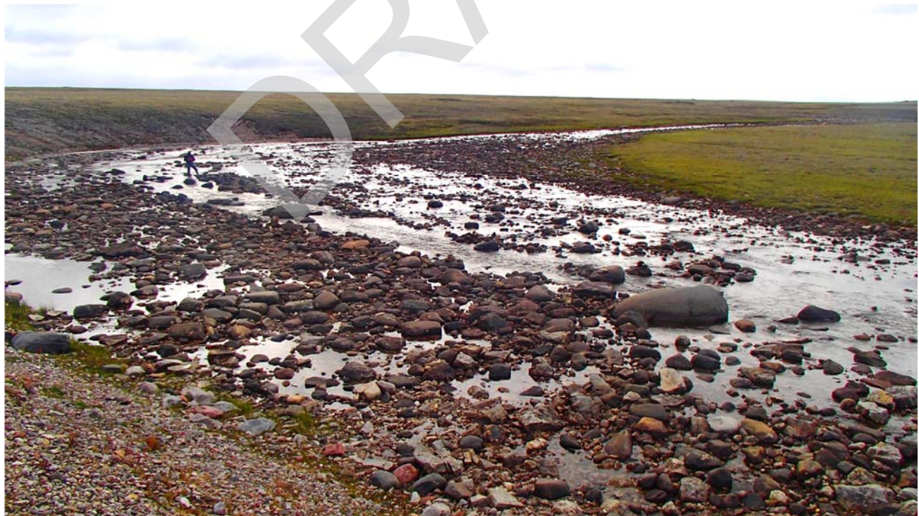
Photo 54: Upstream view from above the RDB of the low-flow channel constructed at Site 11. The low-flow channel provides an unobstructed path for fish through the centre of creek. 20 July 2016.
