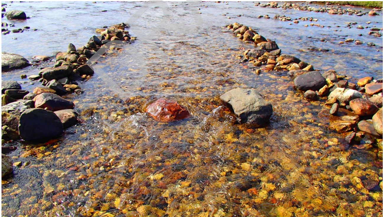
Photo 32: Upstream view of low-flow channel B constructed at Site 4, showing boulders placed within the channel to provide cover for migratory fish. 19 July 2016.
