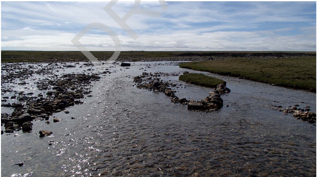
Photo 14: Facing upstream at the upper extent of Site 1 post-remediation. Note the opening along the LDB boundary to allow for fish passage in either direction around the island. 18 July 2016.
