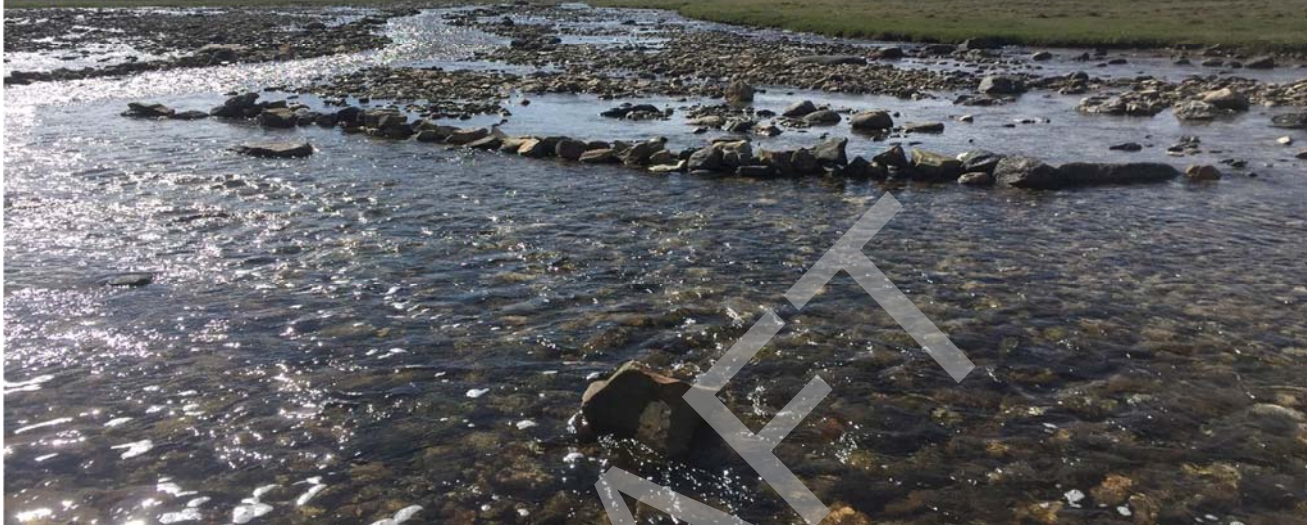
Photo 15 Upstream view of directional weir A at Site 1, guiding fish away from the area of exposed stream bed. 18 July 2016.
