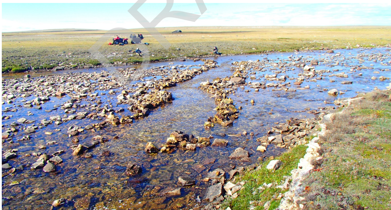
Photo 4-22: Downstream view from above the RDB of the low-flow channel constructed at Site 8. 23 July 2016.
