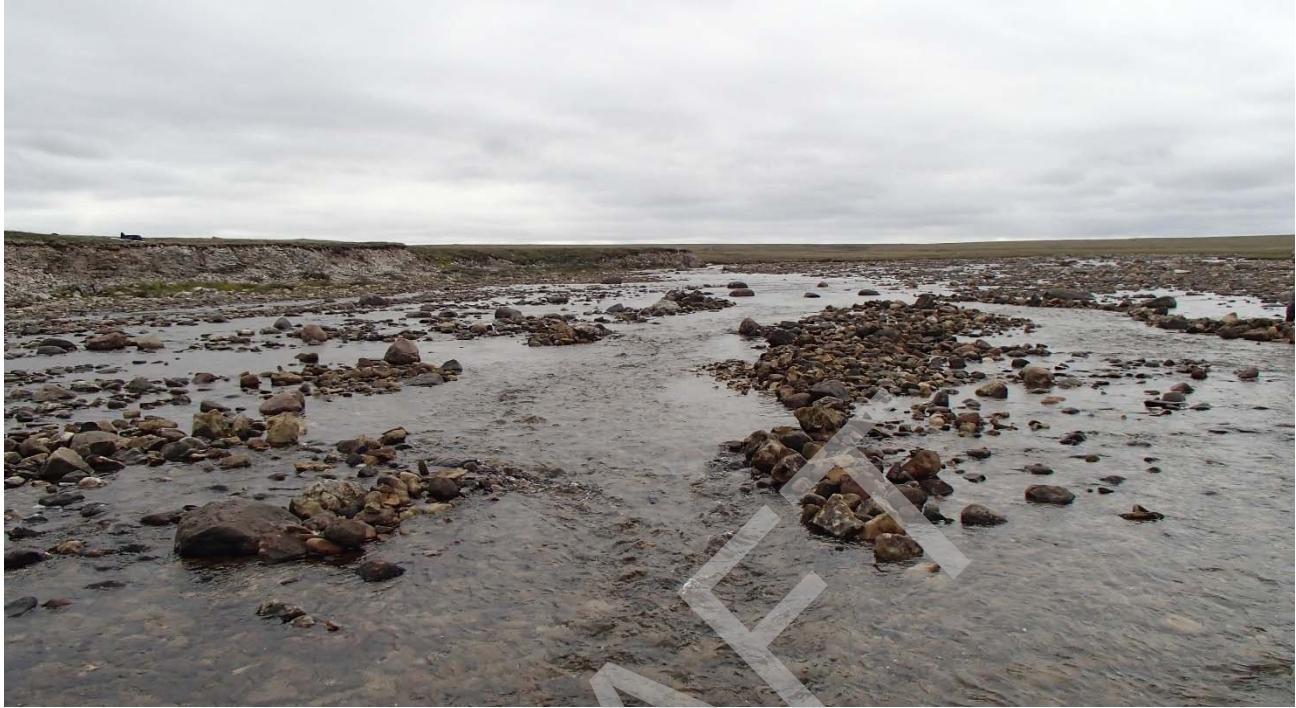
Photo 19: Upstream view of low- flow channel B, including portions of low-flow channel A, constructed at Site 2. 18 July 2016.
