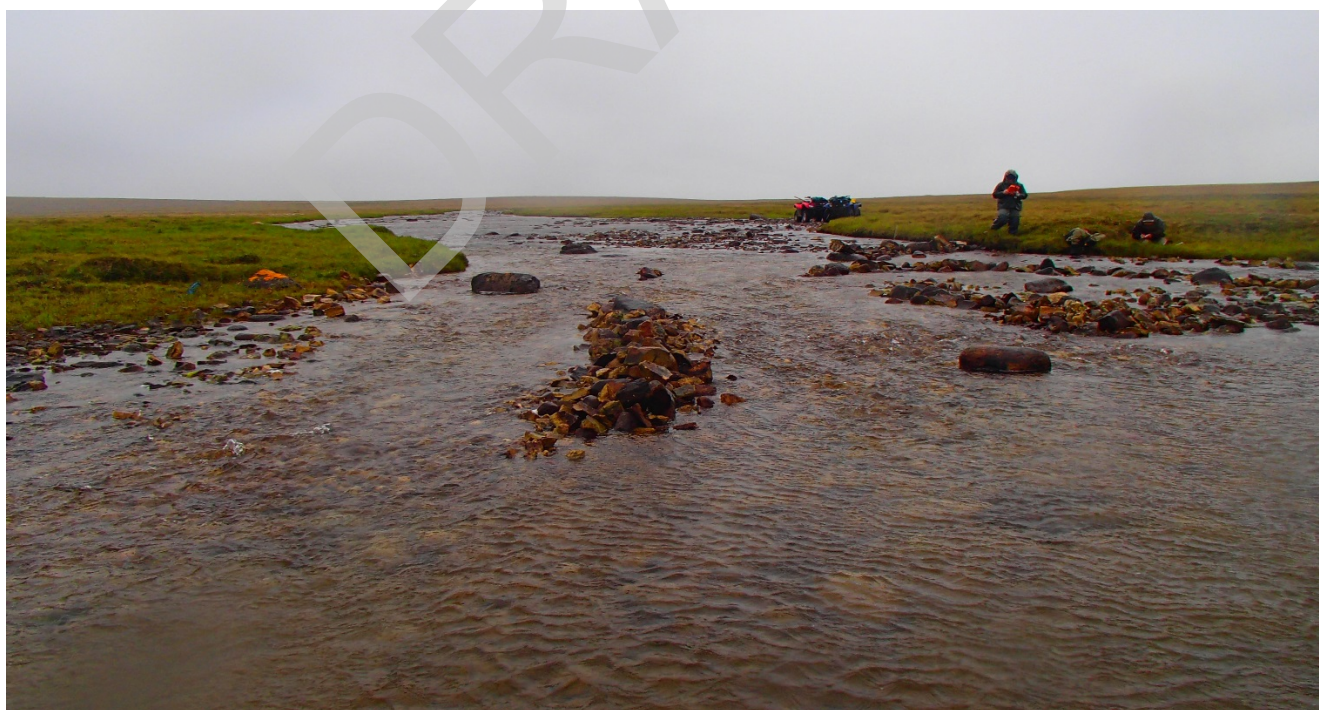
Photo 4-24: Upstream view of low-flow channel A and B constructed at Site 10. Note that the channel provides fish passage beyond the pond (in foreground). 22 July 2016.
