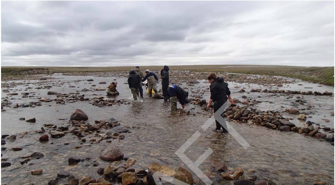
Photo 7: Local students assisting in the construction of a low-flow channel at Site 2. 18 July 2016.
