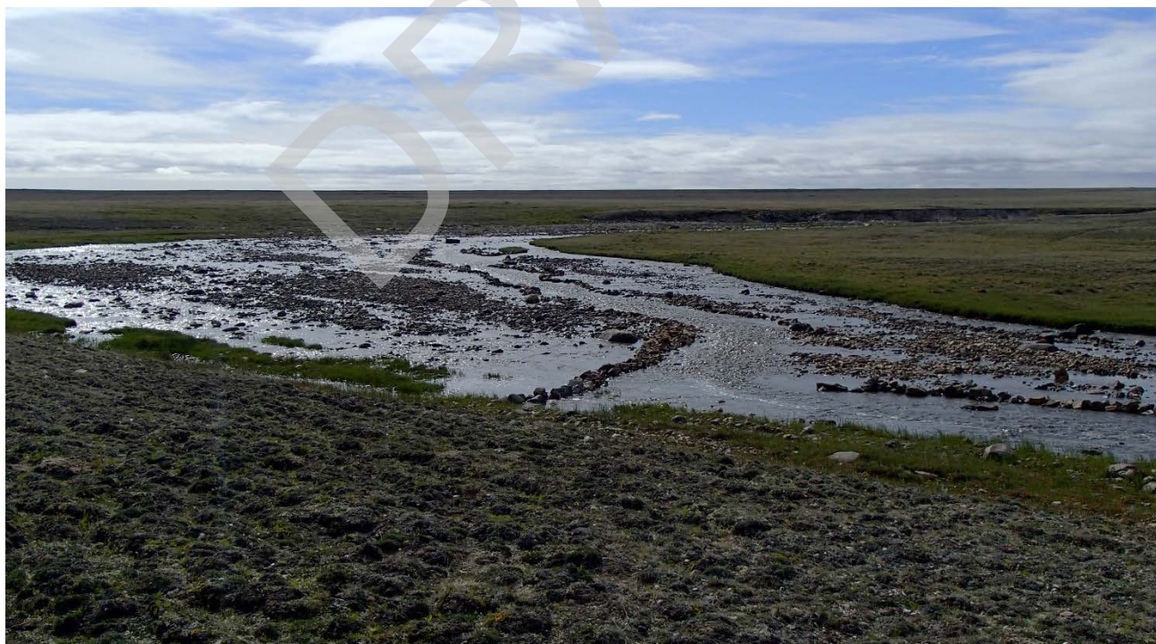
Photo 4-6: Upstream view from elevated RDB showing low-flow channel and weirs constructed during remediation at Site 1. 18 July 2016.
