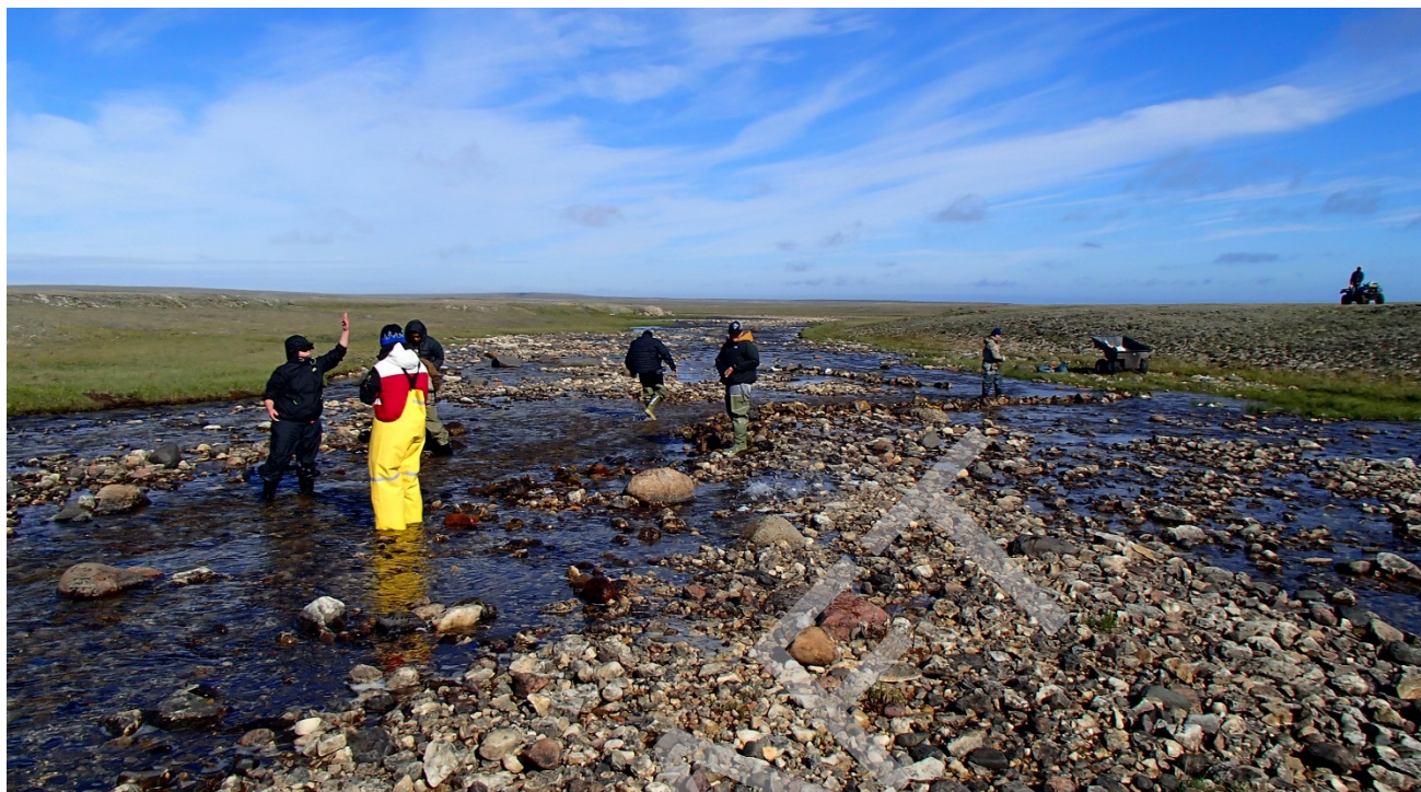
Photo 4-3: Local student and field assistants constructing the low-flow channel at Site 1. 18 July 2016.
