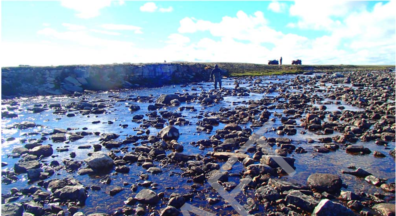
Photo 47: Upstream view from the downstream extent of Site 9 prior to remediation. Note the absence of an obvious migratory route connecting to flows along the RDB. 23 July 2016.
