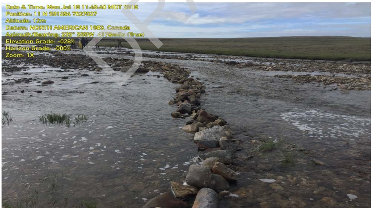
Photo 16: Directional weir B as viewed from the RDB at Site 1, guiding fish away from potential barriers further upstream. 18 July 2016.
