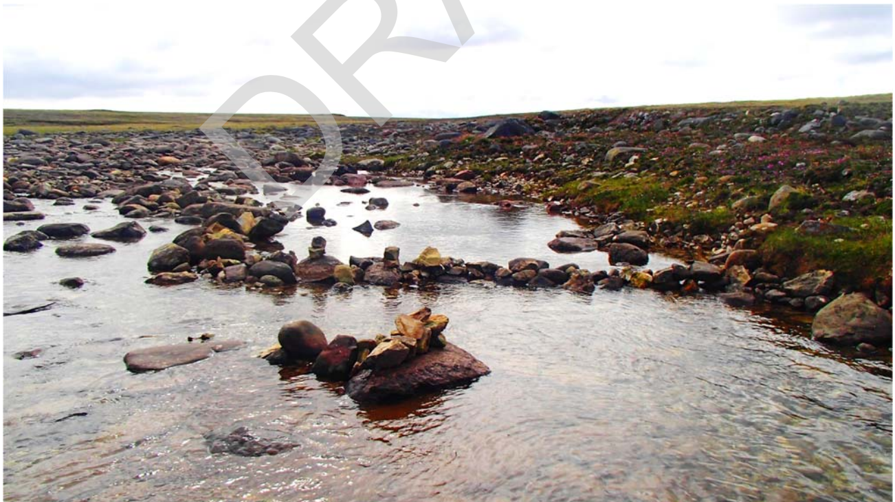
Photo 36: Upstream view of the directional weir at Site 5 to direct fish away from dry sections of the LDB. 20 July 2016.
