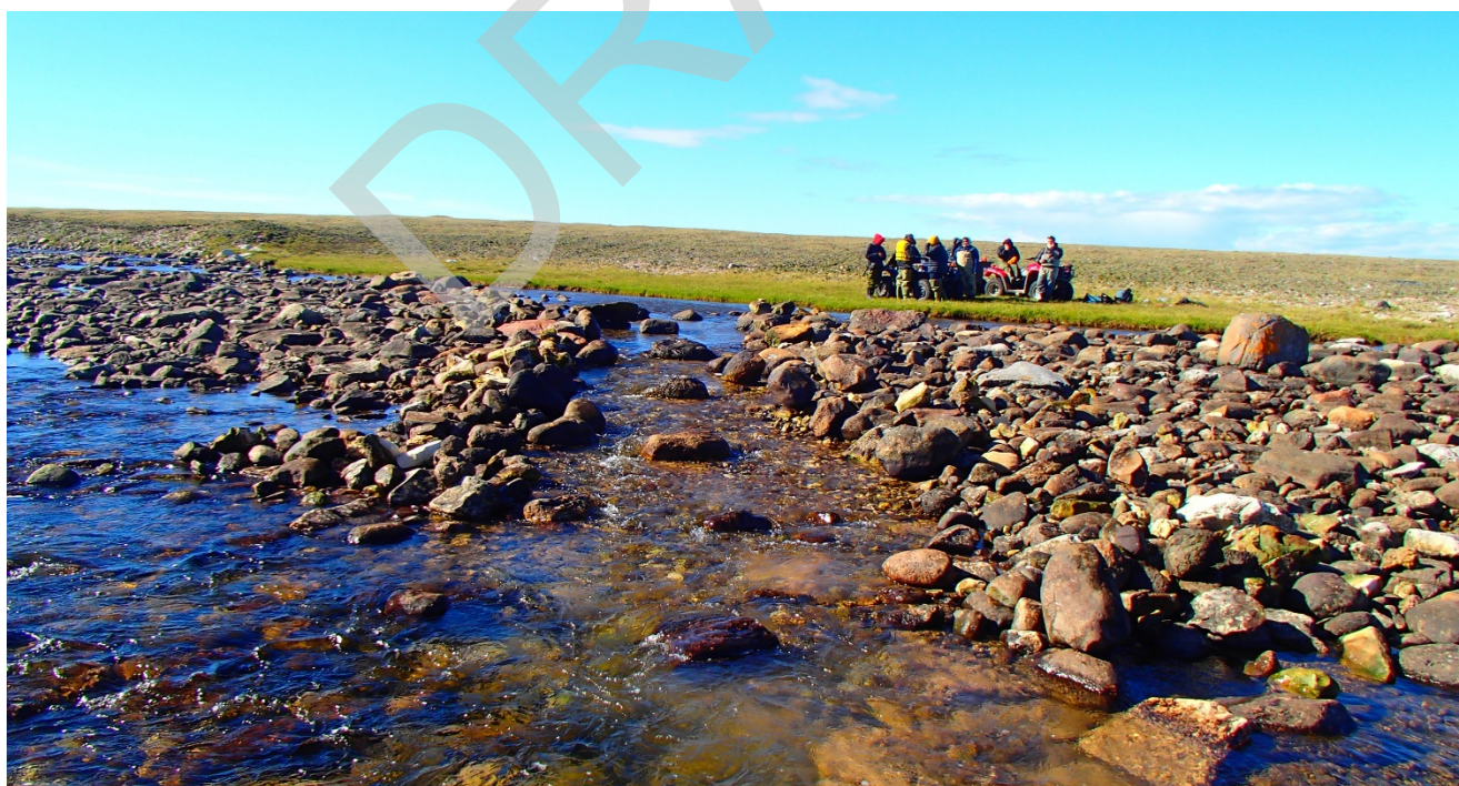
Photo 4-20: Upstream view of the low-flow channel constructed at Site 8. Note the large boulders left in the low-flow channel to act as velocity breaks and cover for fish. 23 July 2016.
