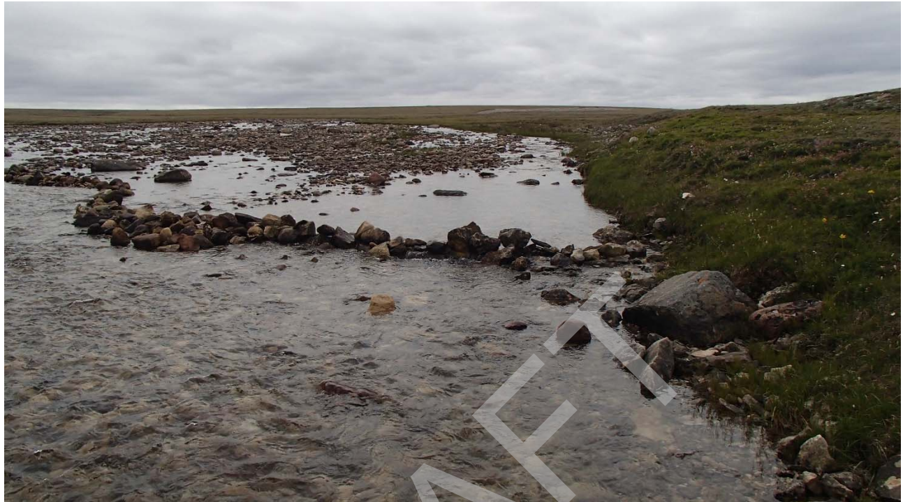
Photo 21: Upstream view of weir A constructed at Site 2 to direct fish passage away from the LDB where flows diminish further upstream. 18 July 2016.
