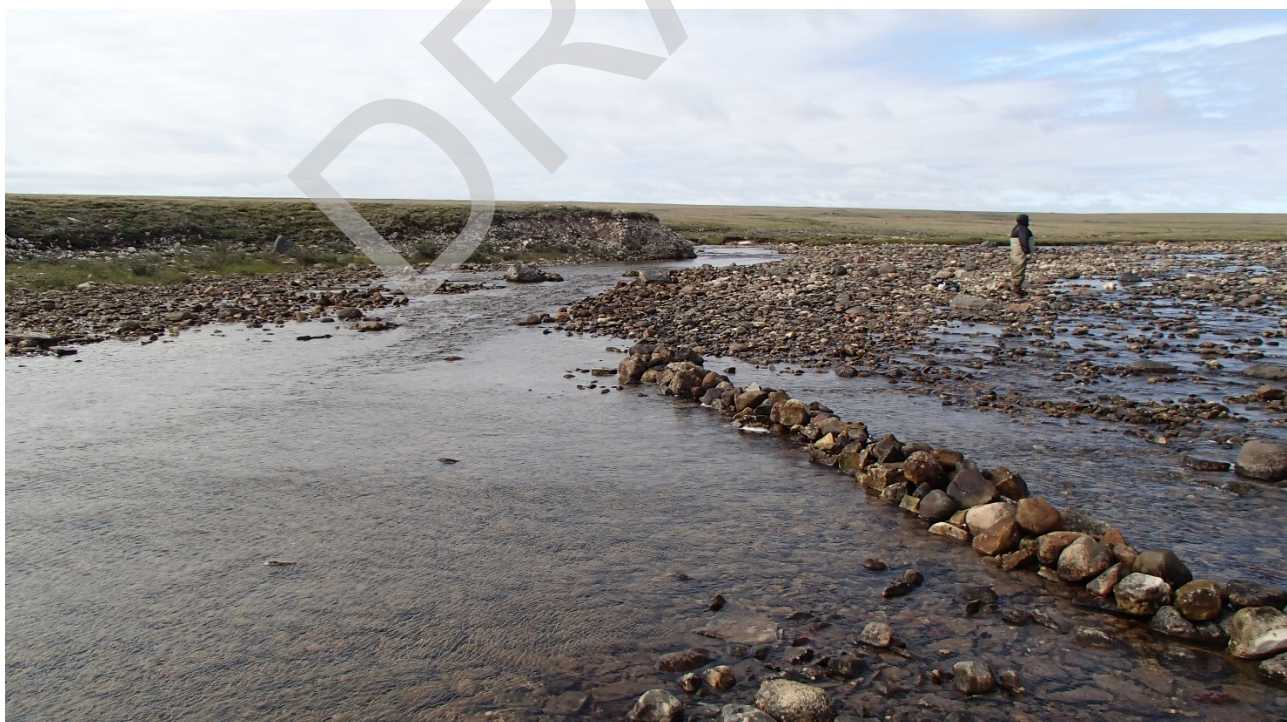
Photo 4-10: Upstream view of low-flow channel A and Weir A at Site 3 post-remediation. Note the directional weir facilitating fish passage towards the channel and away from problem area. 19 July 2016.
