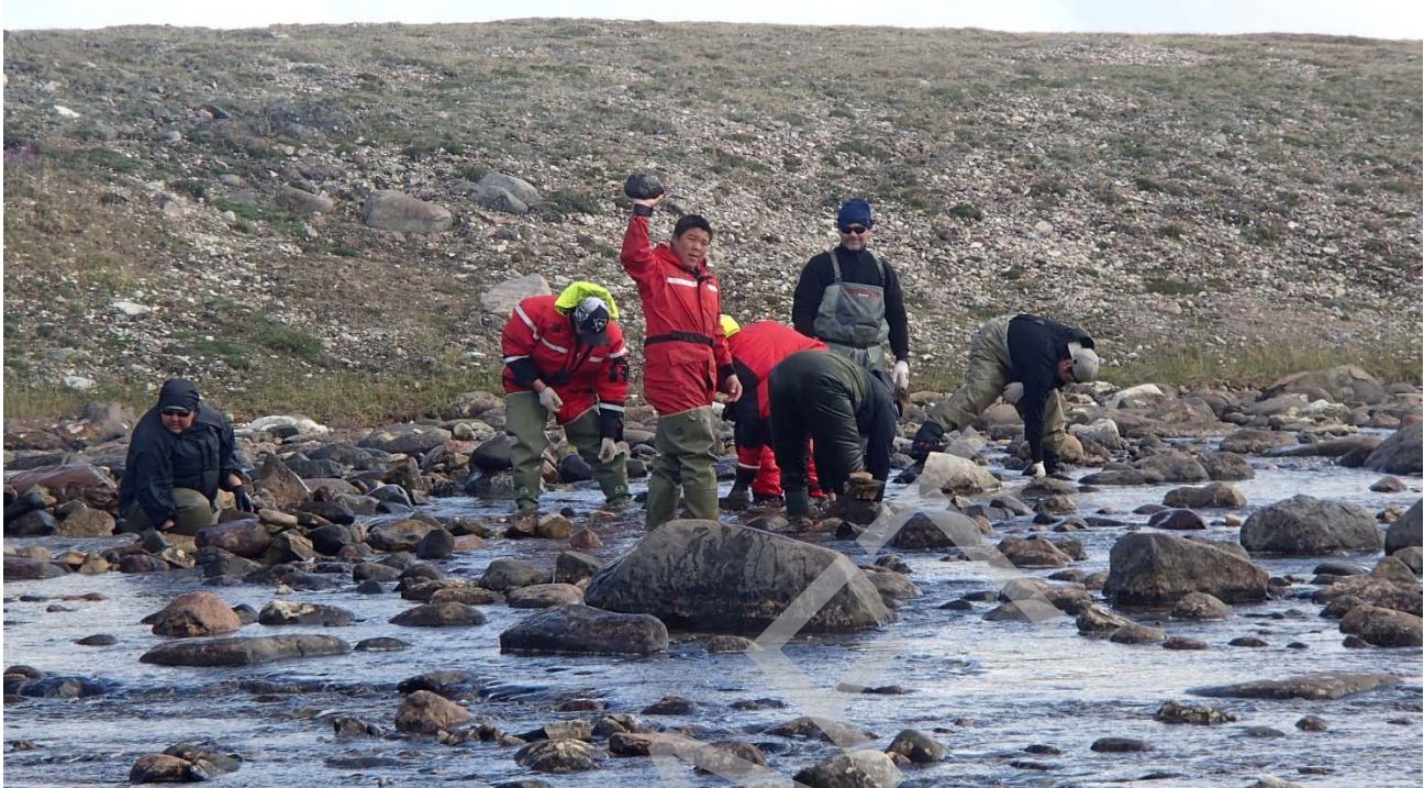
Photo 9: Local students assisting in the construction of a low-flow channel at Site 11. 20 July 2016.
