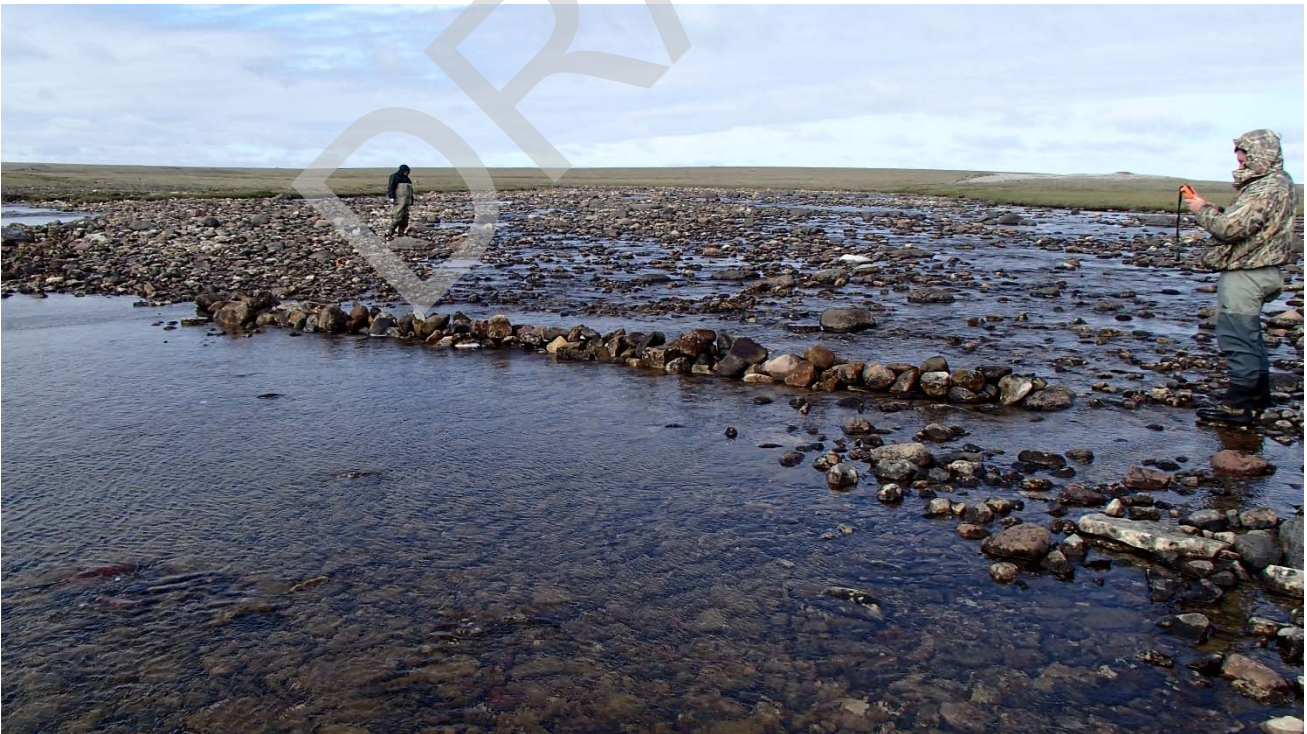
Photo 26: Upstream view of weir A constructed at Site 3 to deter fish migration along the LDB where stranding is likely. 19 July 2016
