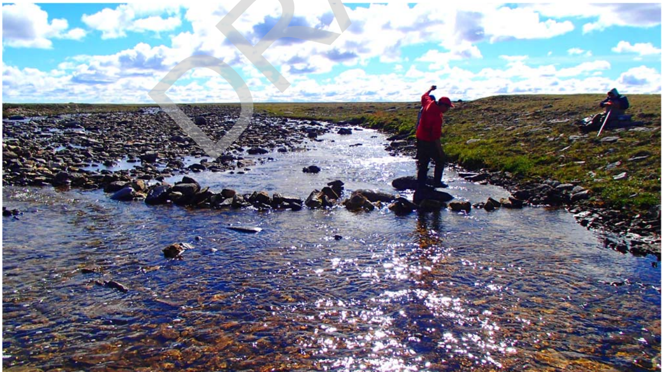
Photo 50: Upstream view from the downstream extent of Site 9 post-remediation. Photograph shows the directional weir constructed to deter passage along the LDB and to direct migration towards the low-flow channel. 23 July 2016.
