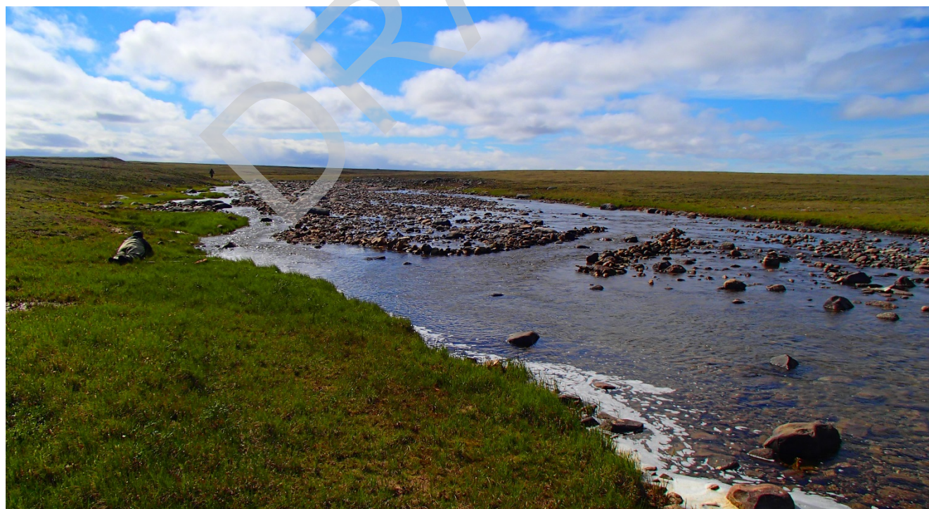
Photo 4-12: Upstream view of low-flow channels A and B constructed at Site 4. 19 July 2016.
