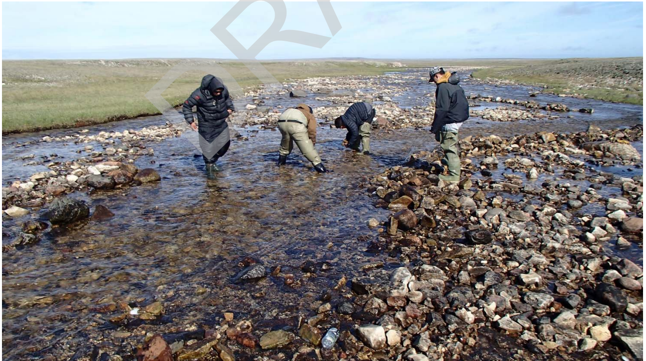
Photo 6: Local students assisting in the construction of a low-flow channel at Site 1. 18 July 2016.
