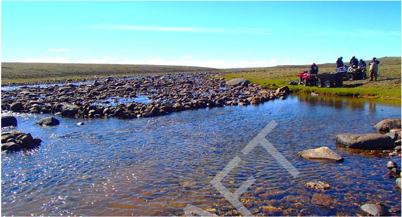
Photo 43: Upstream view from the pool along the LDB at the downstream extent of Site 7 post- remediation. Note weir A directing migratory passage towards the low-flow channels and away from the problem area along the LDB. 24 July 2016.
