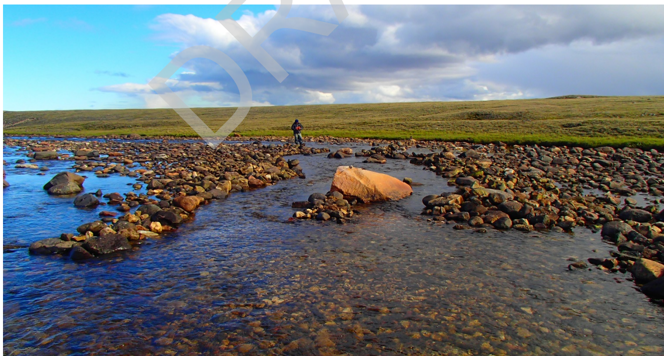
Photo 4-28: Downstream view of the low-flow channel constructed at Site 12 post-remediation, note that the channel provides fish passage across the creek. 21 July 2016.
