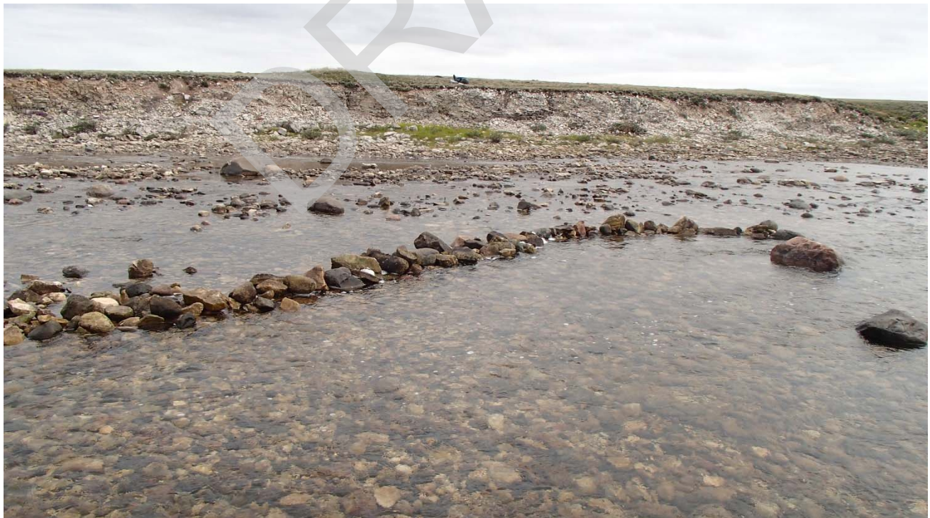
Photo 22: Directional weir B at the upstream extent of low-flow channel B at Site 2, constructed to direct flows towards the low-flow channel. 18 July 2016.
