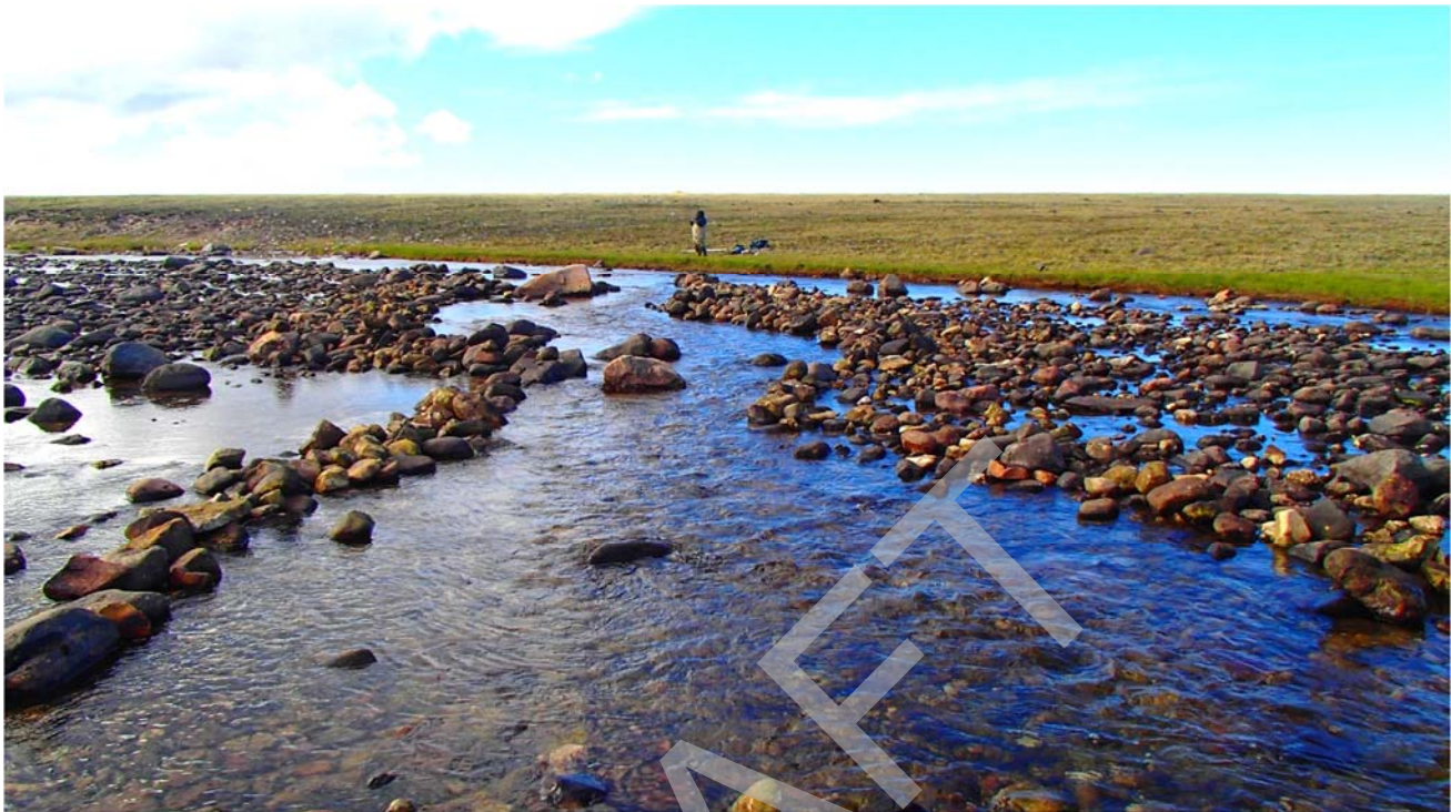
Photo 57: Upstream view of the low-flow channel constructed at Site 12, connecting suitable habitats to the LDB. Note the large boulders left within the channel to act as cover for migratory fish. 21 July 2016.
