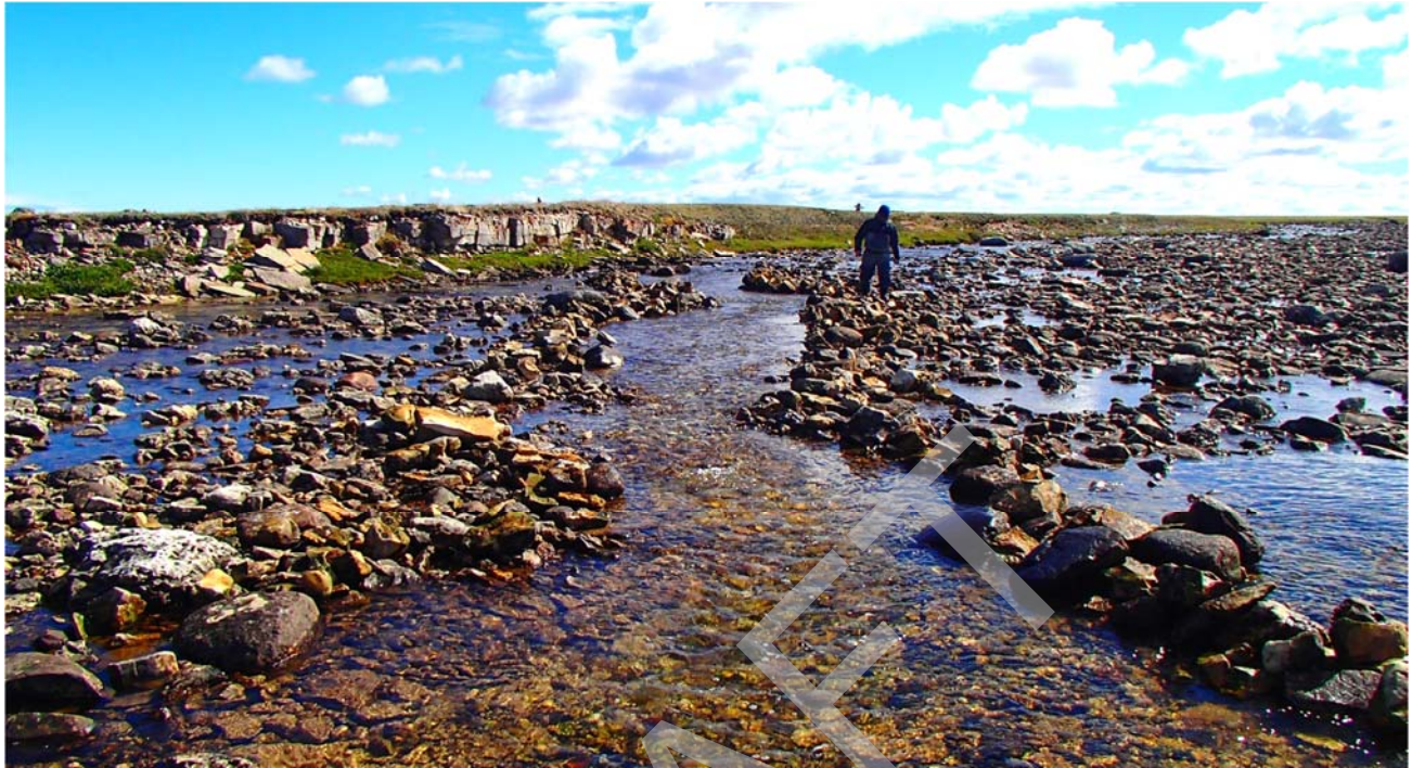
Photo 49: Upstream view of the low-flow channel constructed at Site 9, which created a clear route towards flows along the RDB. 23 July 2016.
