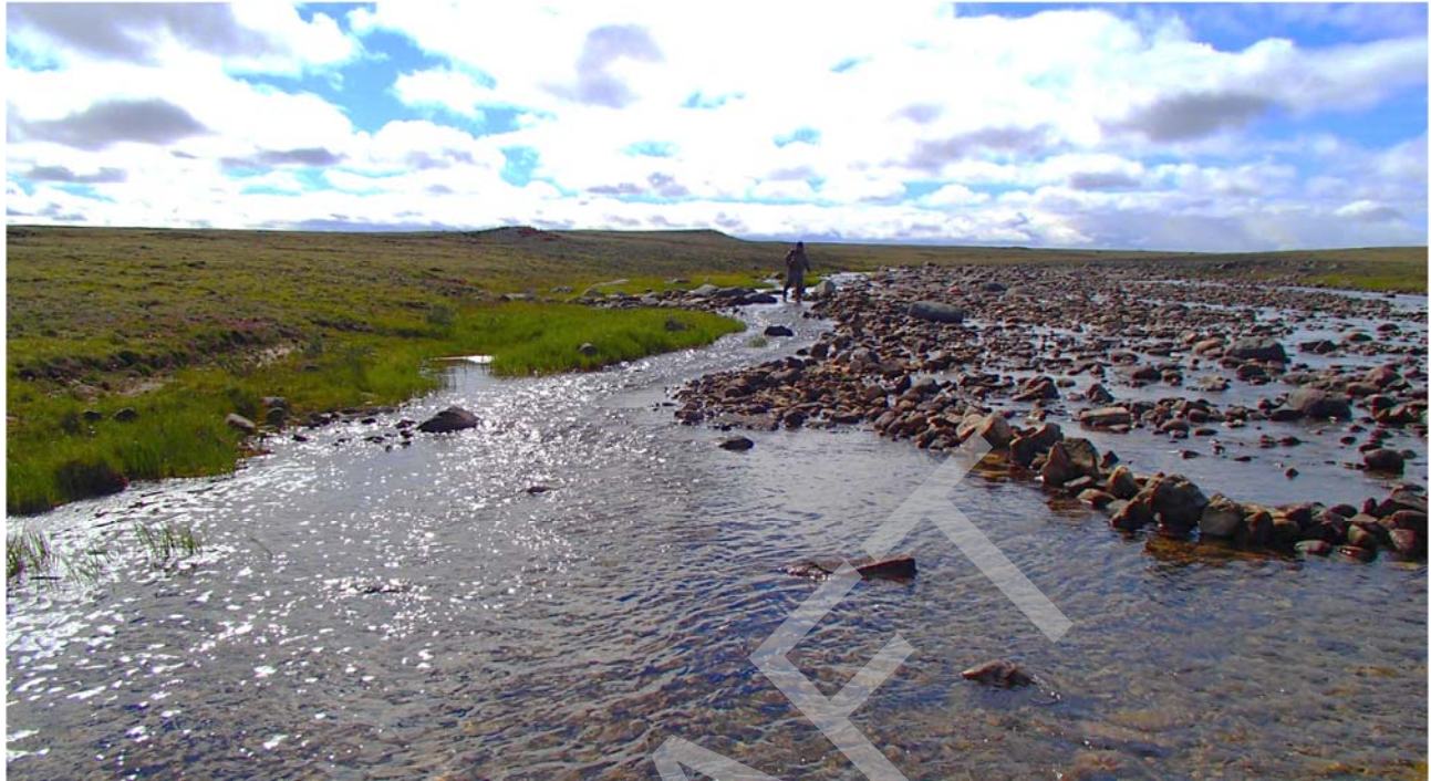
Photo 31: Upstream view of weir A constructed at Site 4 to direct fish passage towards low-flow channel A. 19 July 2016.
