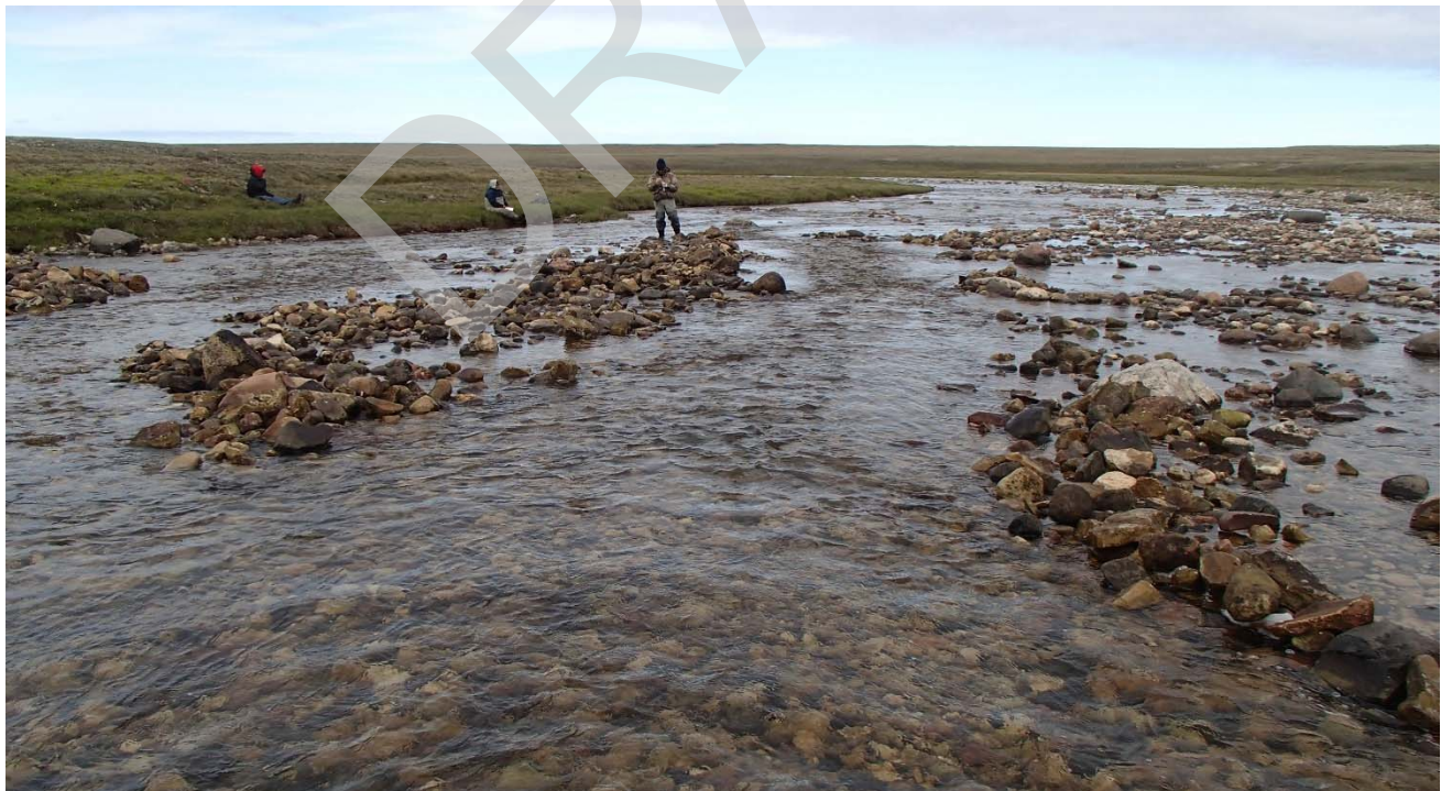
Photo 20: Downstream view of low-flow channels constructed at Site 2. Note the natural cobble bar which was utilized to separate the two channels. 18 July 2016
