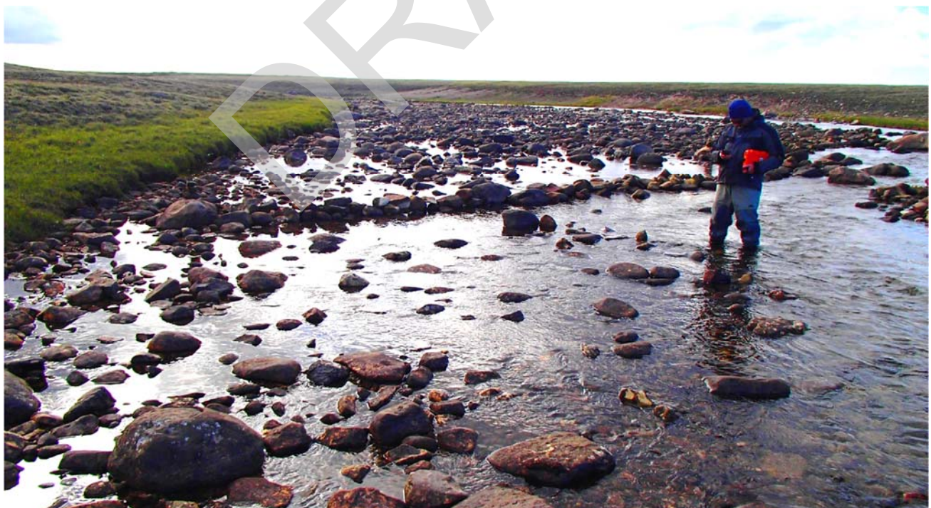
Photo 58: Upstream view of weir A constructed at Site 12 to direct fish towards the constructed low-flow channel and away from the dry streambed along the RDB. 21 July 2016.
