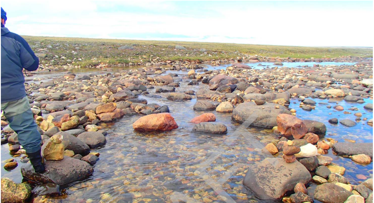
Photo 35: Downstream view of the low-flow channel at Site 5. Boulders too large to move by hand were left within channel to provide cover for migratory fish. 20 July 2016.
