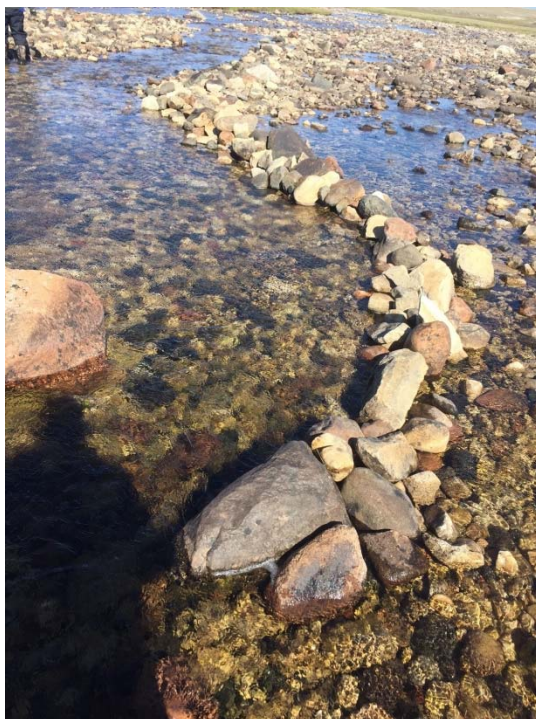
Photo 8: Downstream view of Augmentation Weir at Site 2. 26 July 2017.
