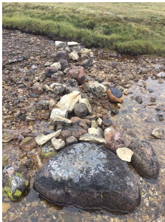
Photo 30: Upstream view of Directional Weir at Site 10. 25 July 2017.
