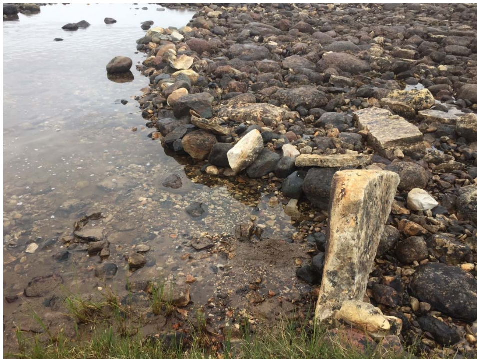
Photo 21: Upstream view of Directional Weir at Site 7. 25 July 2017.
