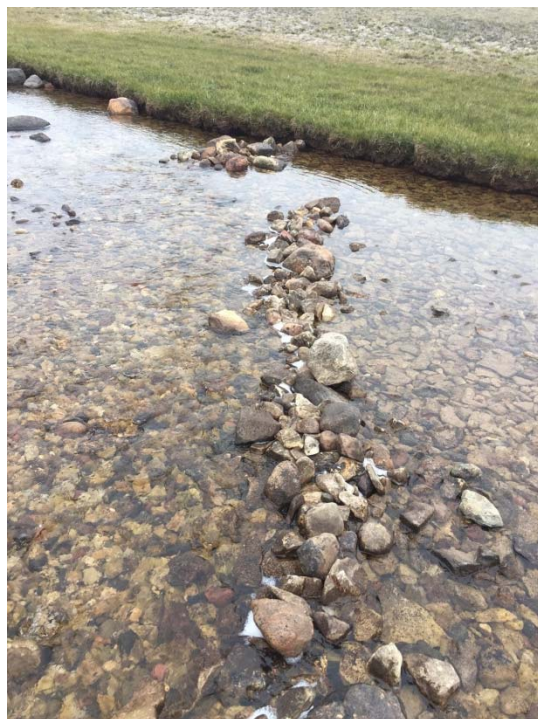
Photo 40: Downstream view of Directional Weir at 2012 Project 1. 27 July 2017.
