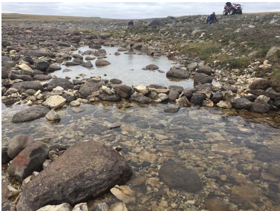
Photo 16: Upstream view of Directional Weir post-repair at Site 5. 26 July 2017.
