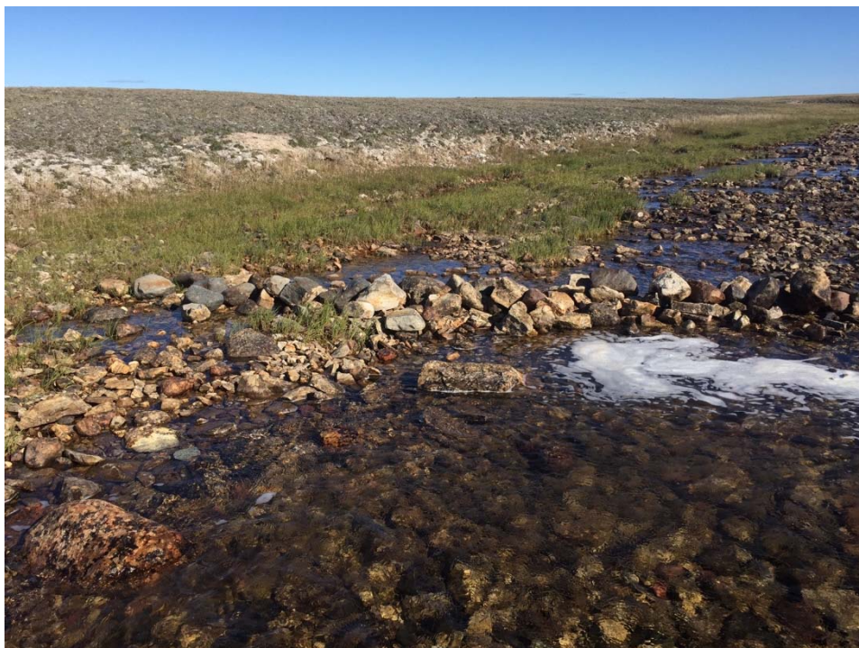
Photo 2: Upstream view of Directional Weir A post-repair at Site 1. 26 July 2017.
