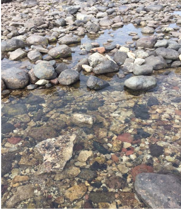
Photo 1: Upstream View of the Directional Weir at Site 12, Pre-Remediation, 26 July 2017
