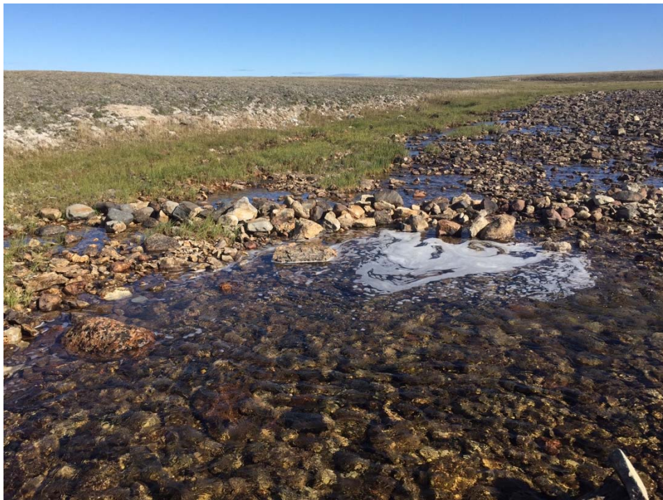
Photo 1: Upstream view of Directional Weir A pre-repair at Site 1. 26 July 2017.
