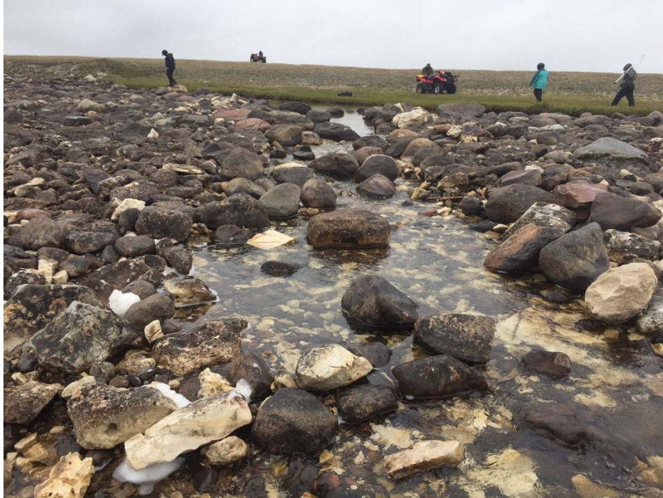
Photo 5: Low-flow Channel (Upstream View) at Site 8 Requires Removal of Displaced Boulders, 26 July 2017
