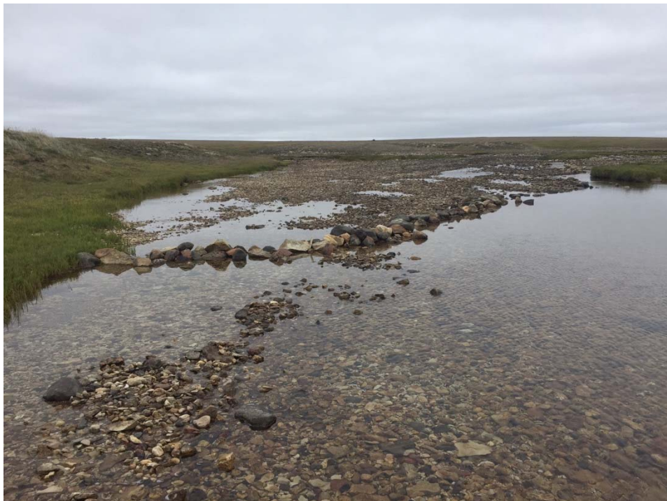
Photo 51: Upstream view of Directional Weir A at 1212 Project 5. 27 July 2017.
