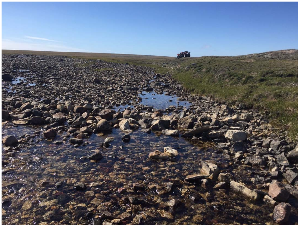
Photo 7: Upstream view of Directional Weir at Site 2. 26 July 2017.
