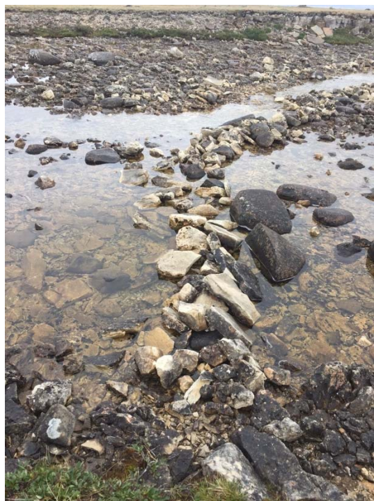
Photo 26: Upstream view of Directional Weir at Site 9. 25 July 2017.
