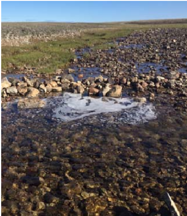
Photo 3: Upstream View of the Directional Weir A at Site 1, Pre-Remediation, 26 July 2017
