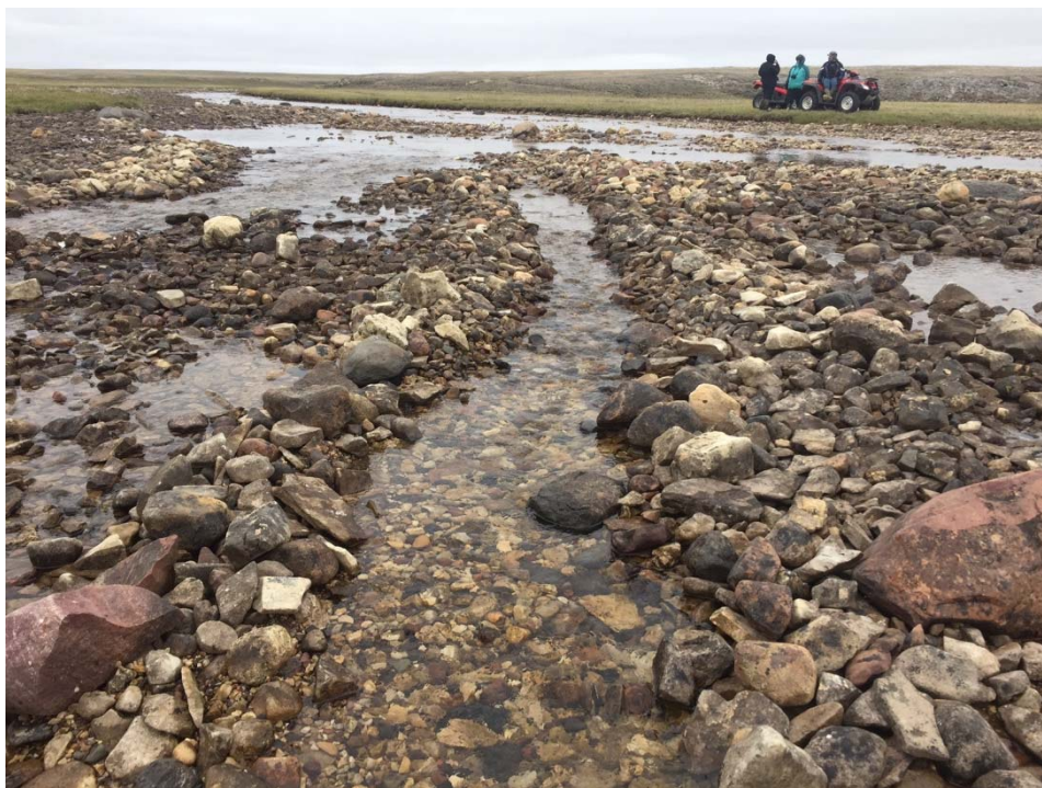
Photo 41: Upstream view of Low-flow Channel B pre-repair at 2012 Project 1. 27 July 2017.
