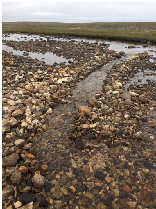
Photo 42: Downstream view of Low-flow Channel B post-repair at 2012 Project 1. 27 July 2017.
