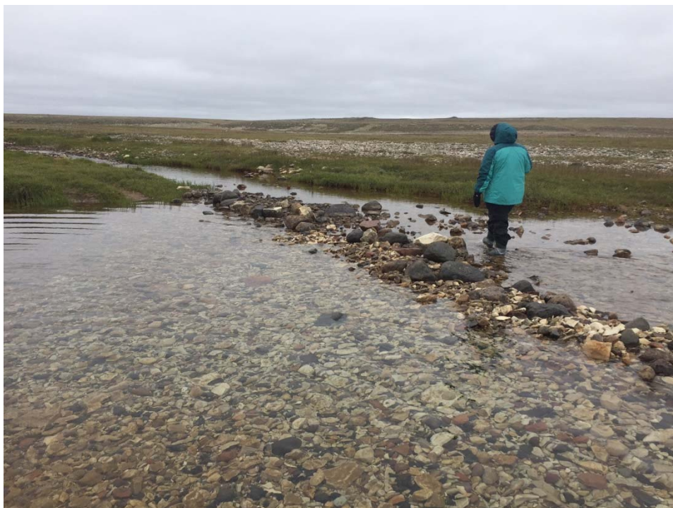
Photo 52: Upstream view of Directional Weir B at 1212 Project 5. 27 July 2017.
