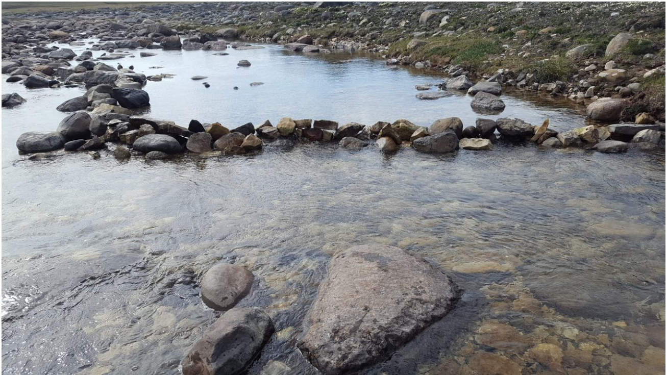
Photo A17: Upstream View of Directional Weir, Pre-Improvement, at Site 5 on 24 July 2018
