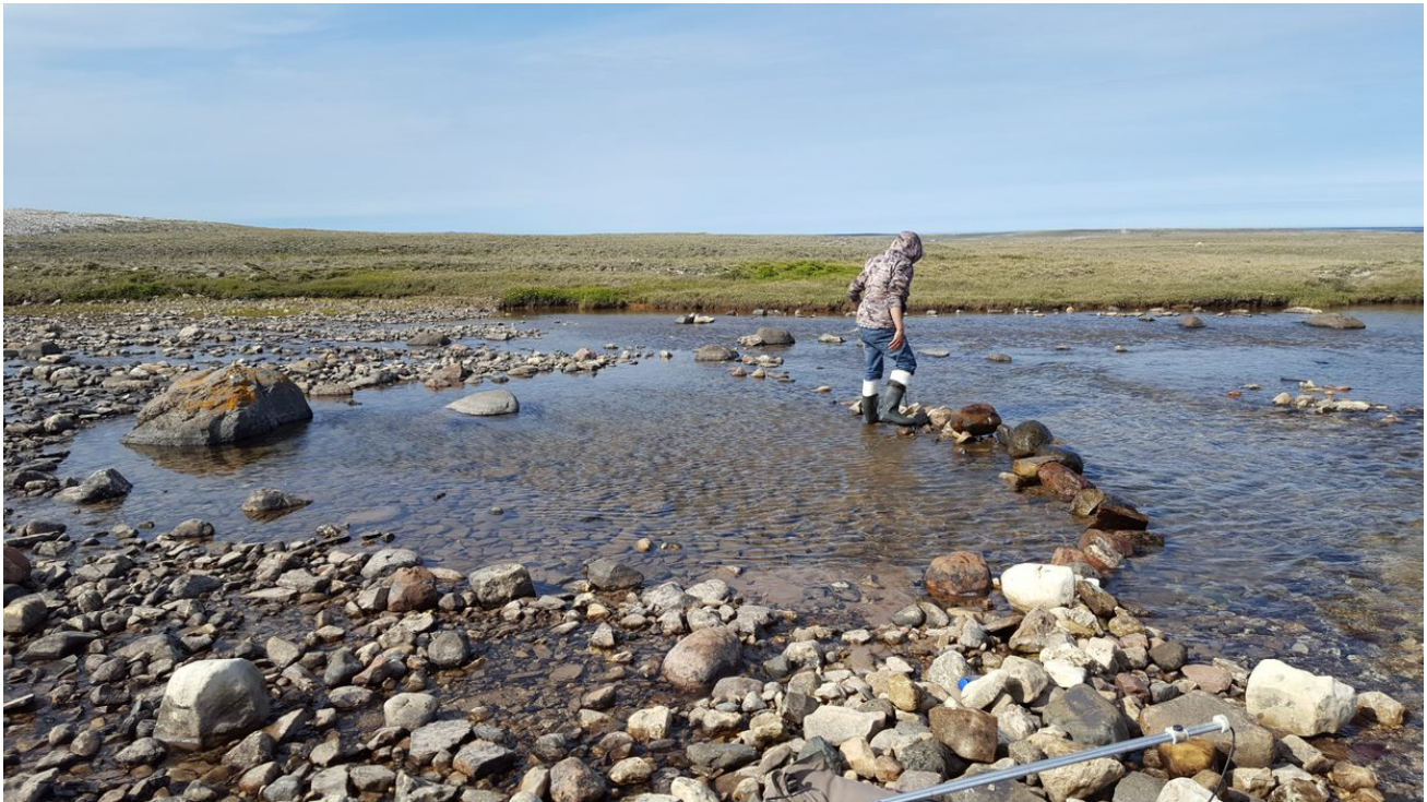
Photo A41: Downstream View of Directional Weir, Pre-Repair, at 2012 Project 2, 24 July 2018
