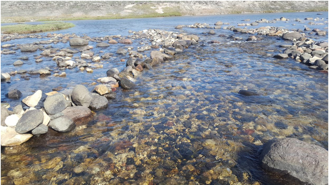
Photo A19: Downstream View of Low-flow Channel, Post-Repair, at Site 6 on 24 July 2018
