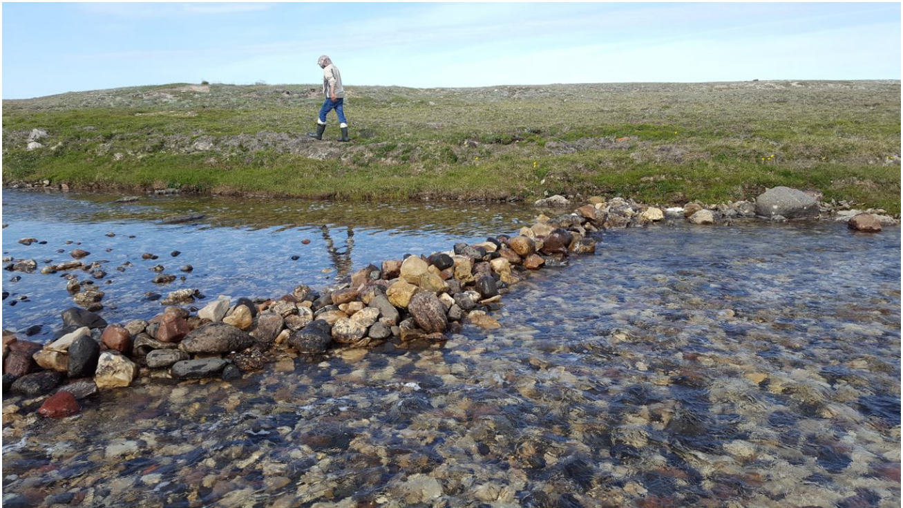
Photo A7: Downstream View of Augmentation Weir, Post-Repair, at Site 2 on 25 July 2018
