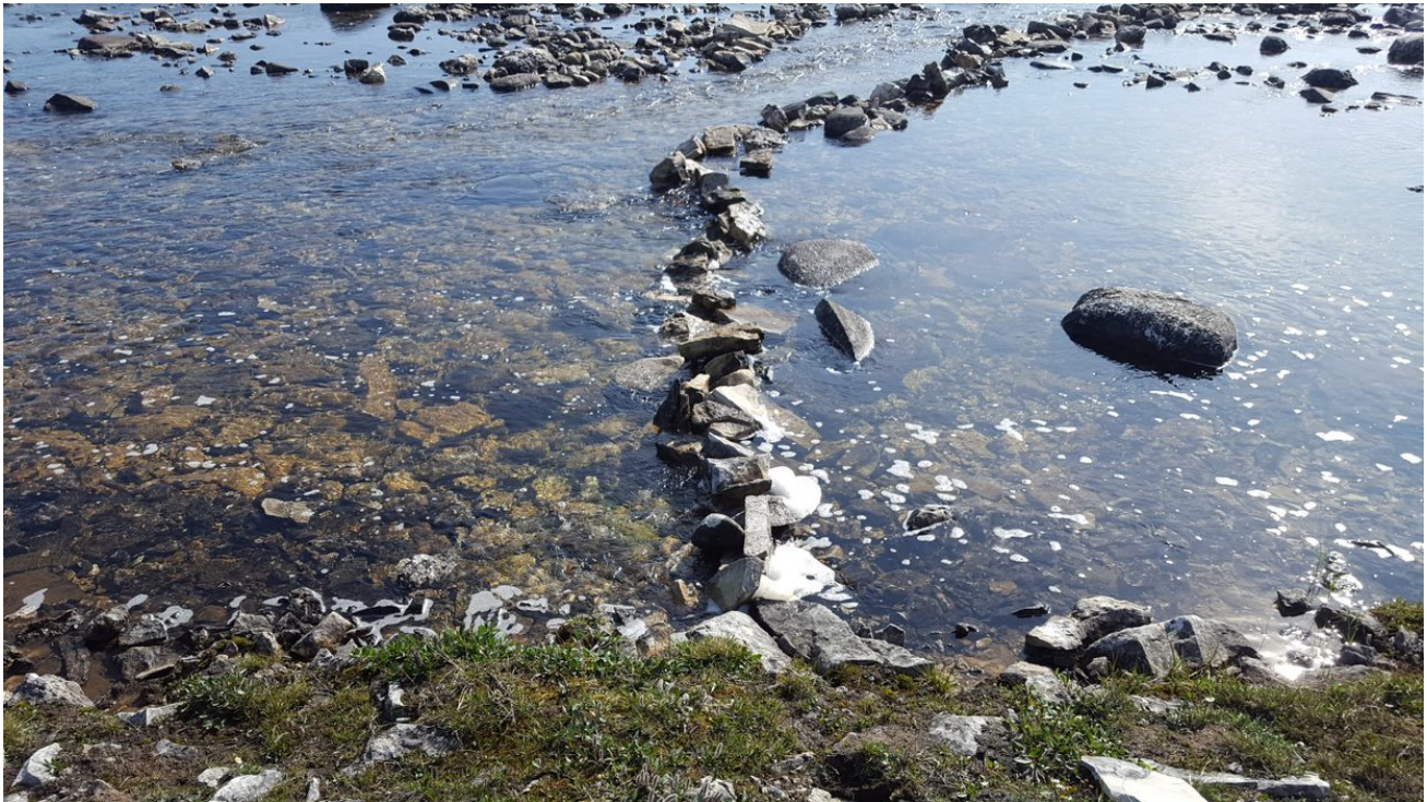
Photo A25: View from Left Downstream Bank of Directional Weir, Post-Improvement, at Site 9 on 25 July 2018
