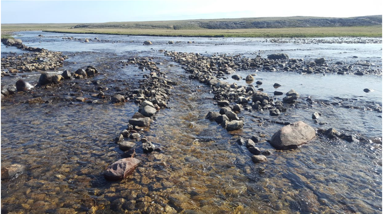
Photo A35: Upstream View of Low-flow Channel B at 2012 Project 1, Depths Allows for Fish Passage, 25 July 2018
