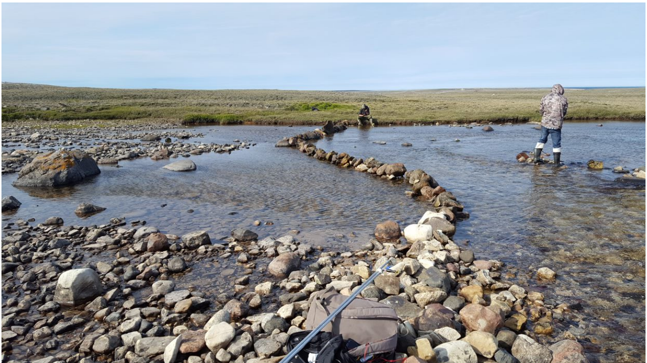
Photo A42: Downstream View of Directional Weir, Post-Repair, at 2012 Project 2, 24 July 2018
