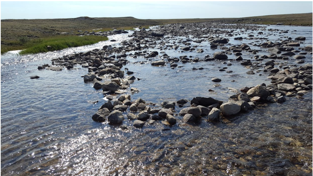
Photo A12: Upstream View of Directional Weir at the confluence of Low-flow Channel A and Low-flow Channel B, Pre-Repair, at Site 4 on 24 July 2018
