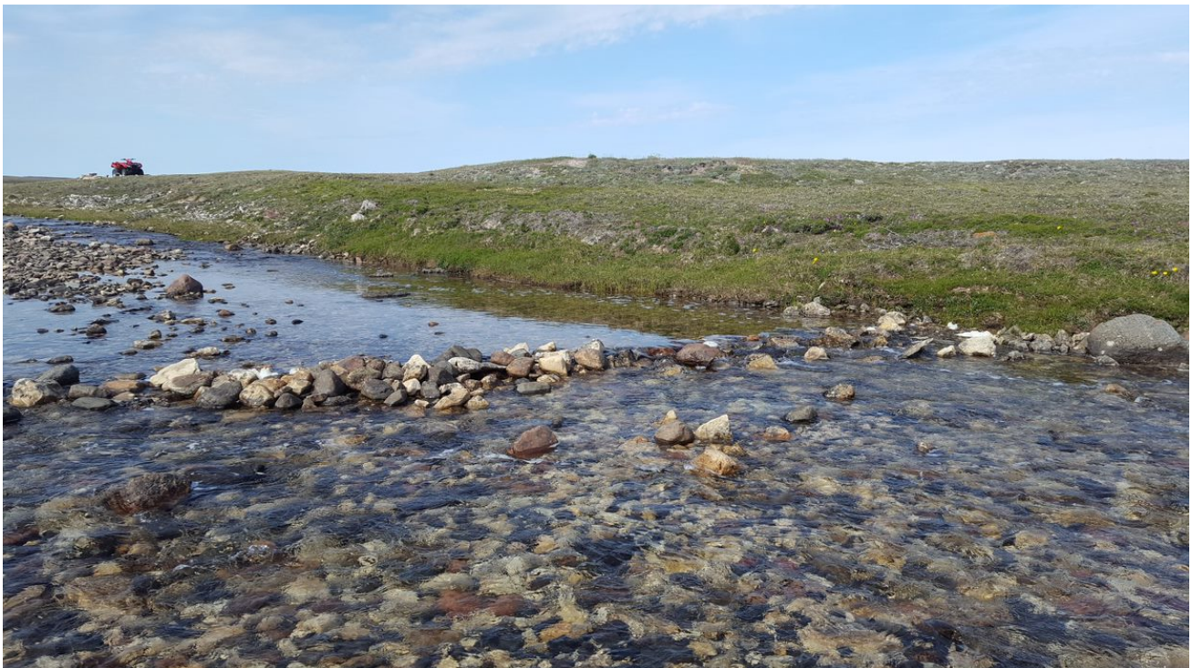
Photo A6: Downstream View of Augmentation Weir, Pre-Repair, at Site 2 on 25 July 2018
