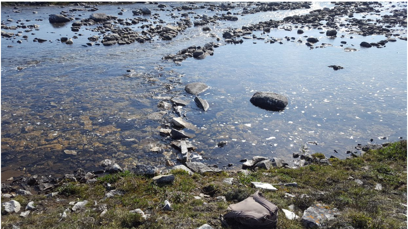
Photo A24: View from Left Downstream Bank of Directional Weir, Pre-Improvement, at Site 9 on 25 July 2018
