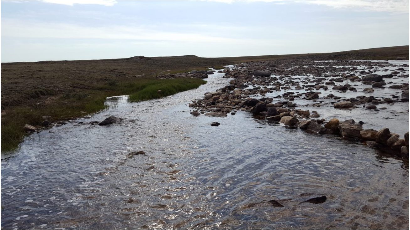
Photo A13: Upstream View of Low-flow Channel A and Directional Weir, Post-Repair, at Site 4 on 24 July 2018
