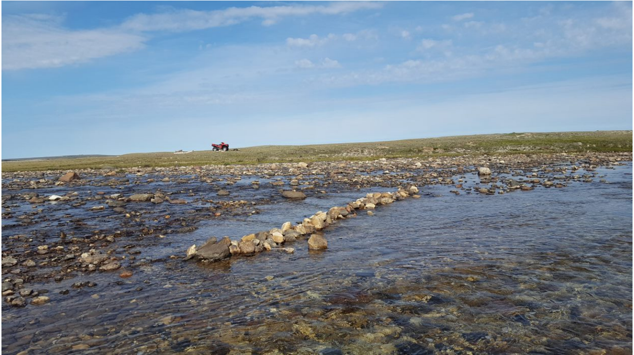
Photo A9: Downstream View of Directional Weir at Site 3 on 25 July 2018
