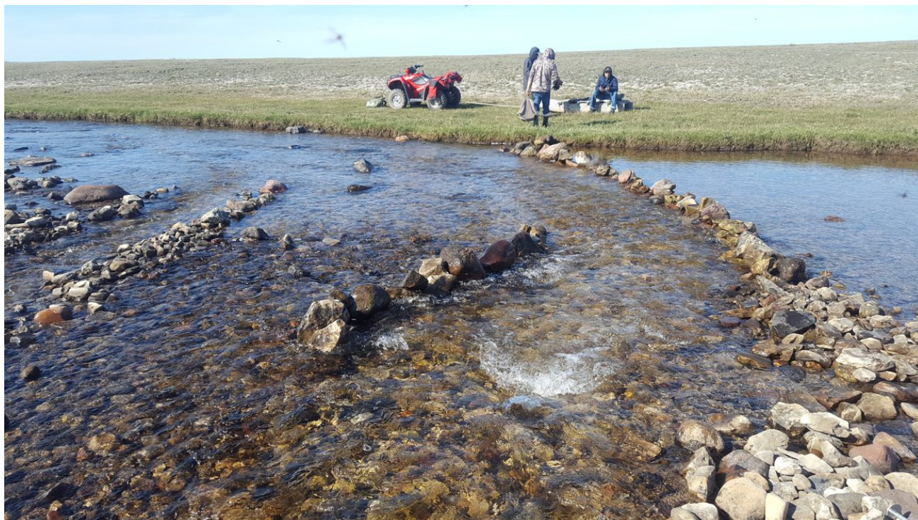
Photo A37: Downstream View of Low-flow Channel A, Post-Repair, at 2012 Project 1, 25 July 2018
