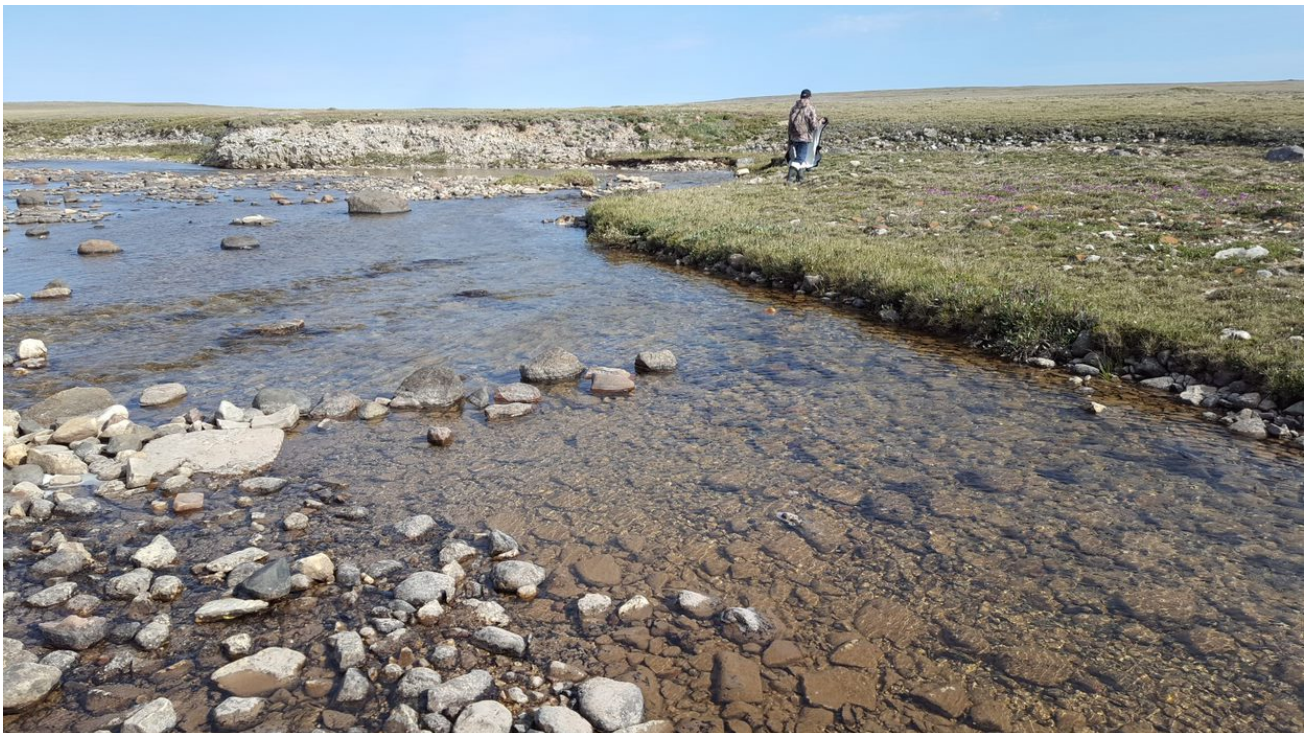
Photo A44: Downstream View of Directional Weir, Pre-Repair, at 2012 Project 3, 24 July 2018
