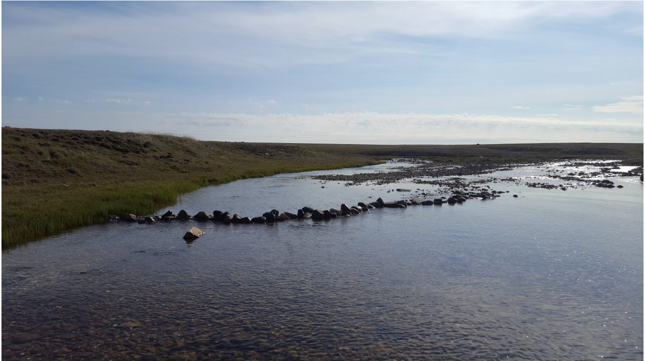
Photo A49: Upstream View of Directional Weir A at 2012 Project 5, 25 July 2018
