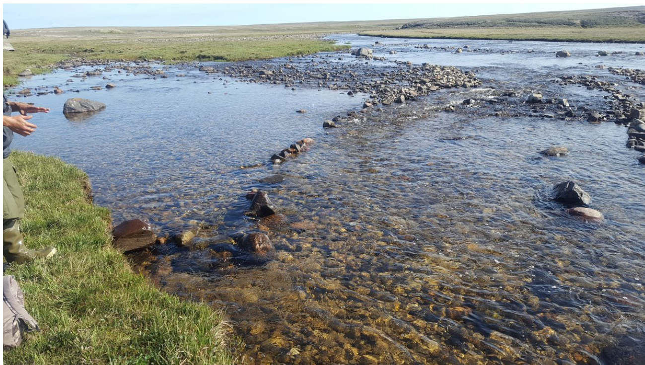
Photo A38: View from Right Downstream Bank of Directional Weir, Pre-Repair, at 2012 Project 1, 25 July 2018
