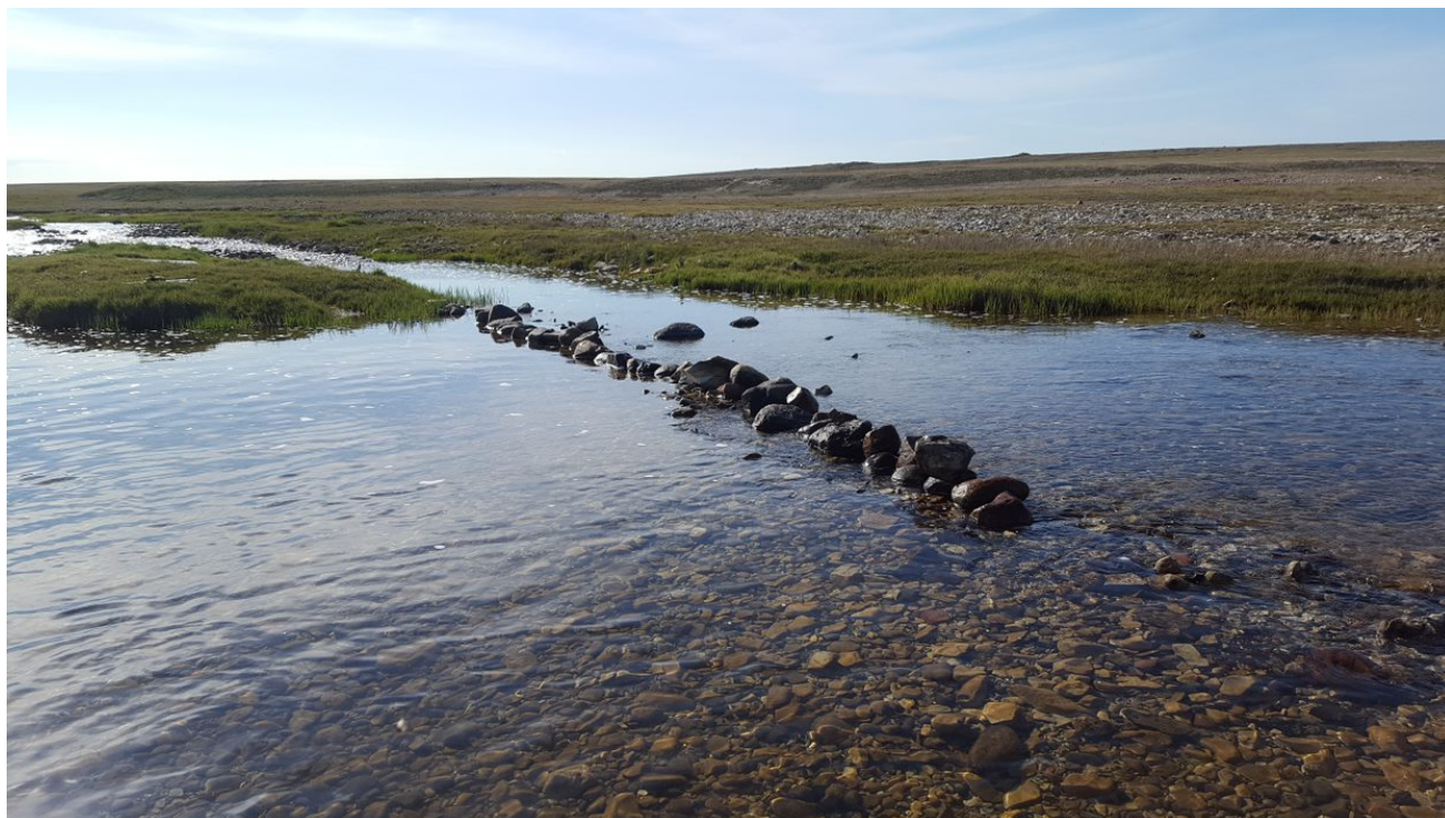
Photo A51: Upstream View of Directional Weir B, Pre-Repair, at 2012 Project 5, 25 July 2018
