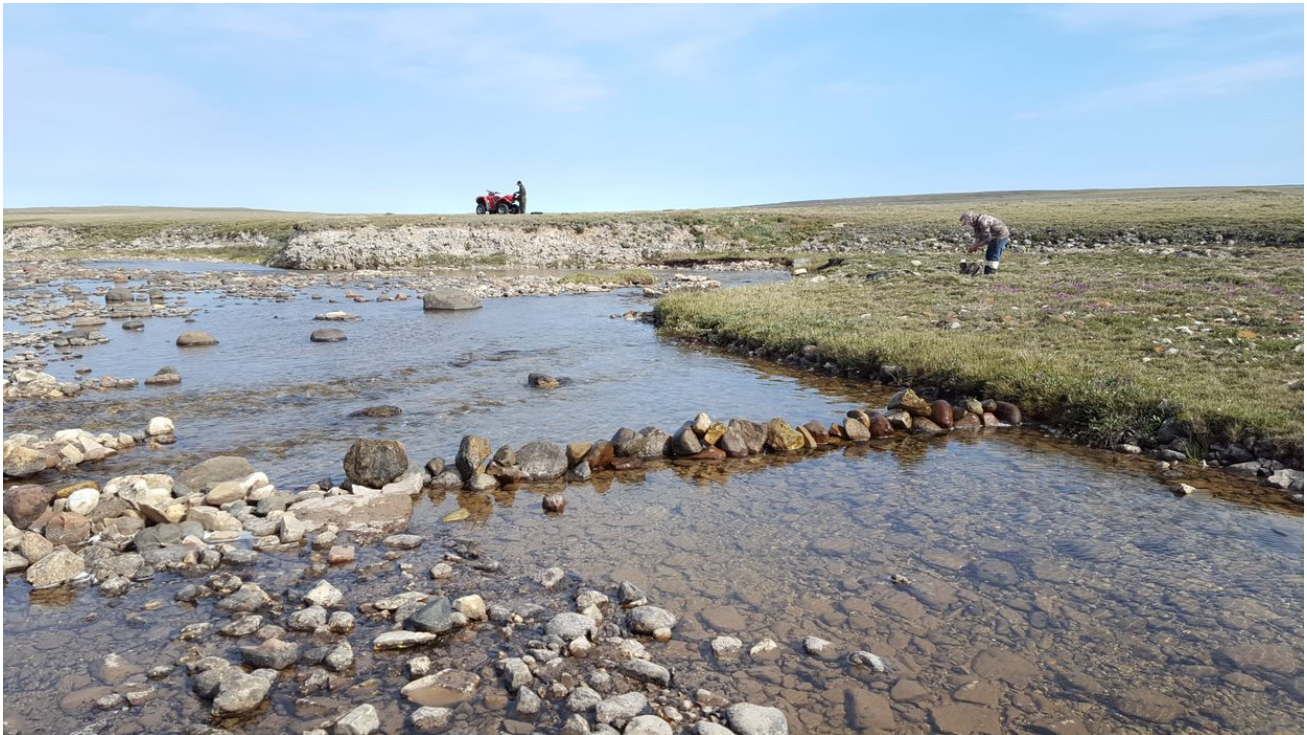
Photo A45: Downstream View of Directional Weir, Post-Repair, at 2012 Project 3, 24 July 2018
