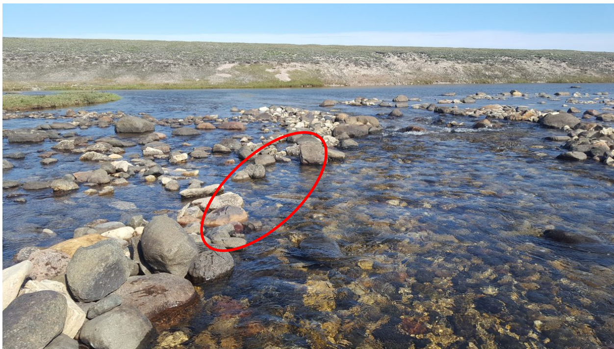
Photo 5: Downstream View of Low-flow Channel, Pre-Repair, at Site 6, 24 July 2018
