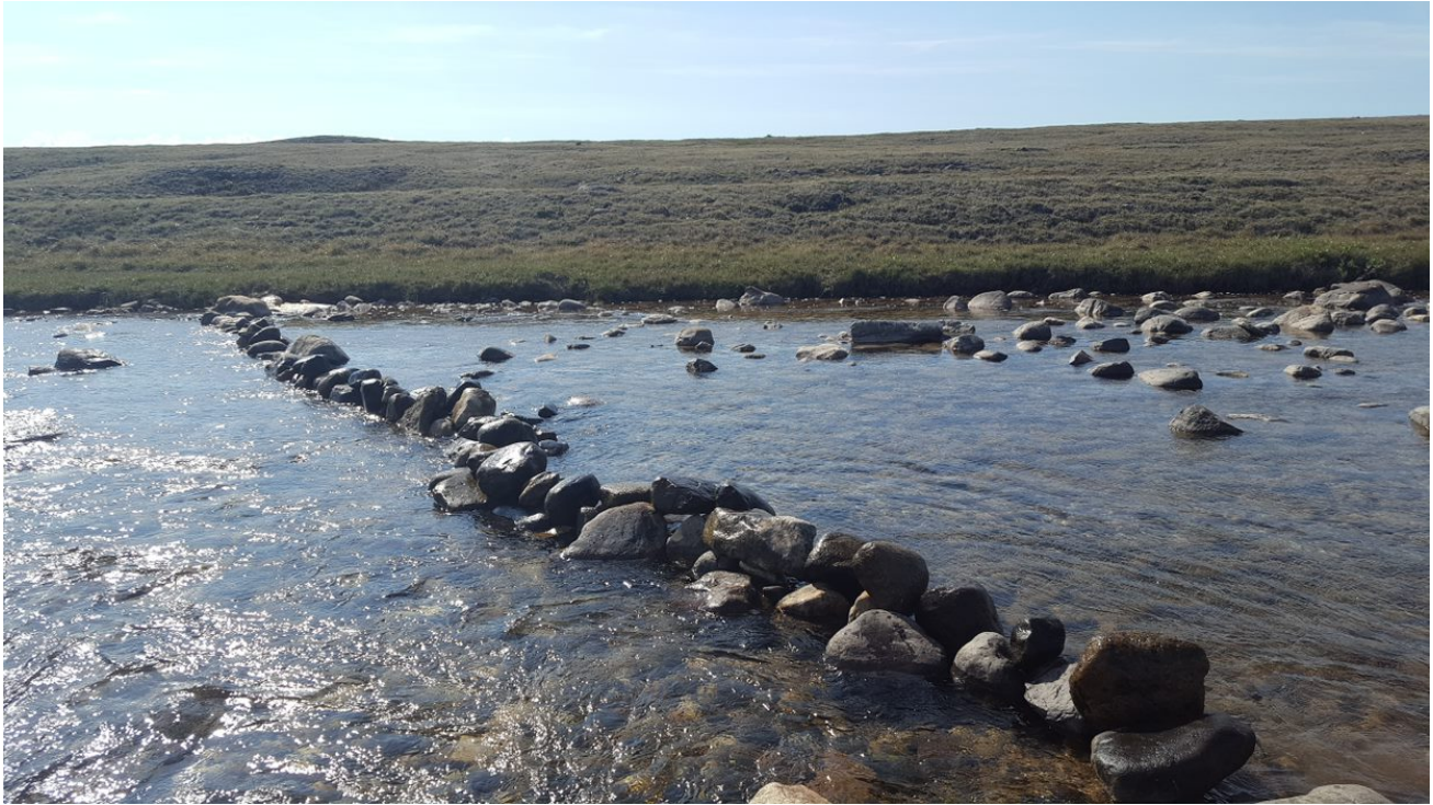
Photo A33: Downstream View of Directional Weir, Post-Repair/Improvement, at Site 12 on 24 July 2018
