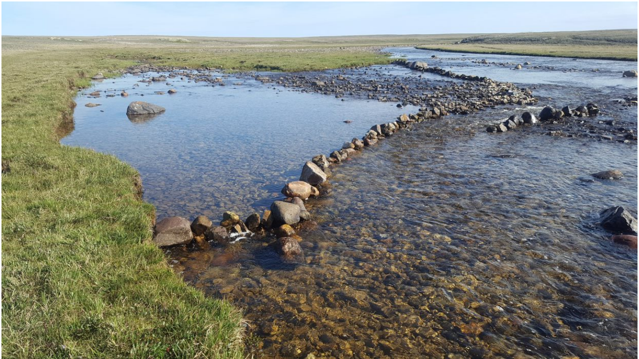
Photo A39: View from Right Downstream Bank of Directional Weir, Post-Repair, at 2012 Project 1, 25 July 2018
