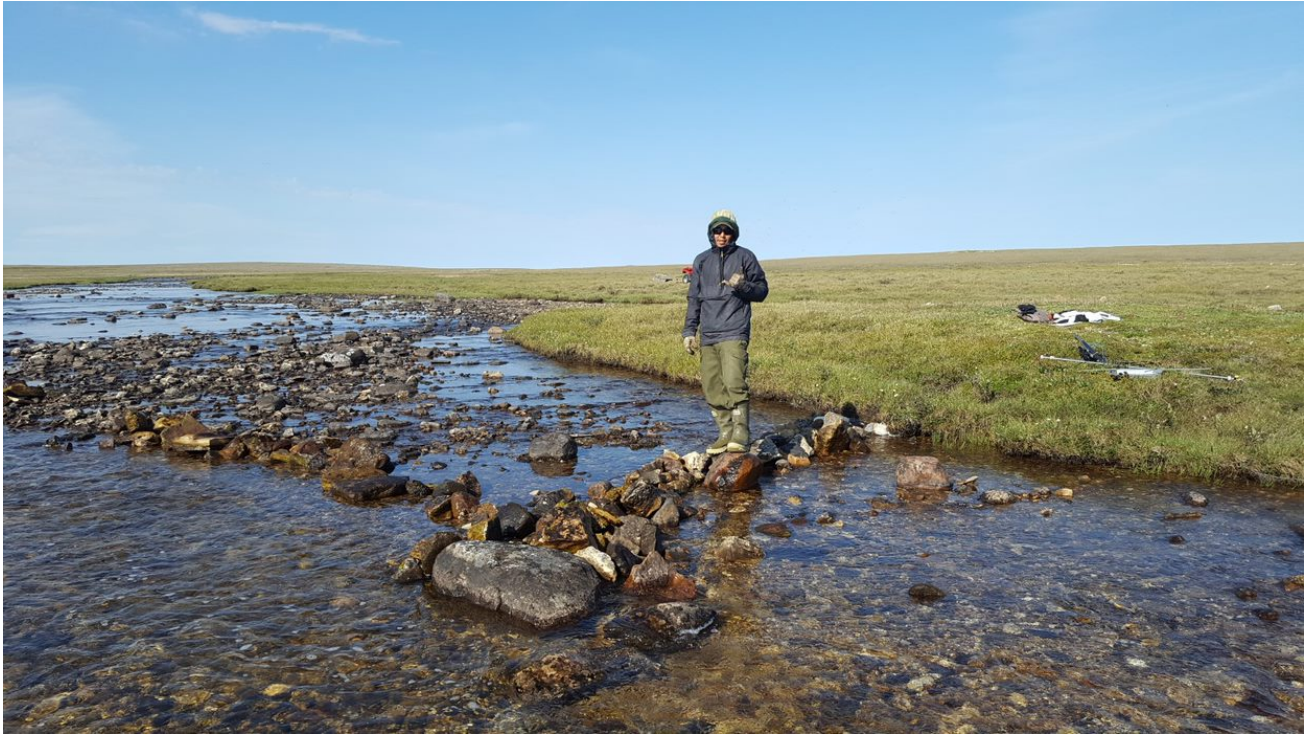
Photo A29: Upstream View of Directional Weir, Post-Repair, with assistant Adrian at Site 10 on 25 July 2018
