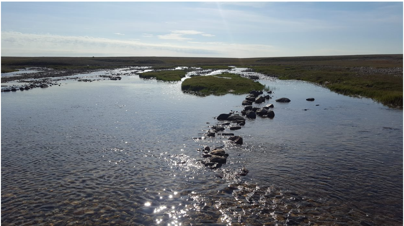
Photo A50: Upstream View of Directional Weir B, Pre-Repair, at 2012 Project 5, 25 July 2018
