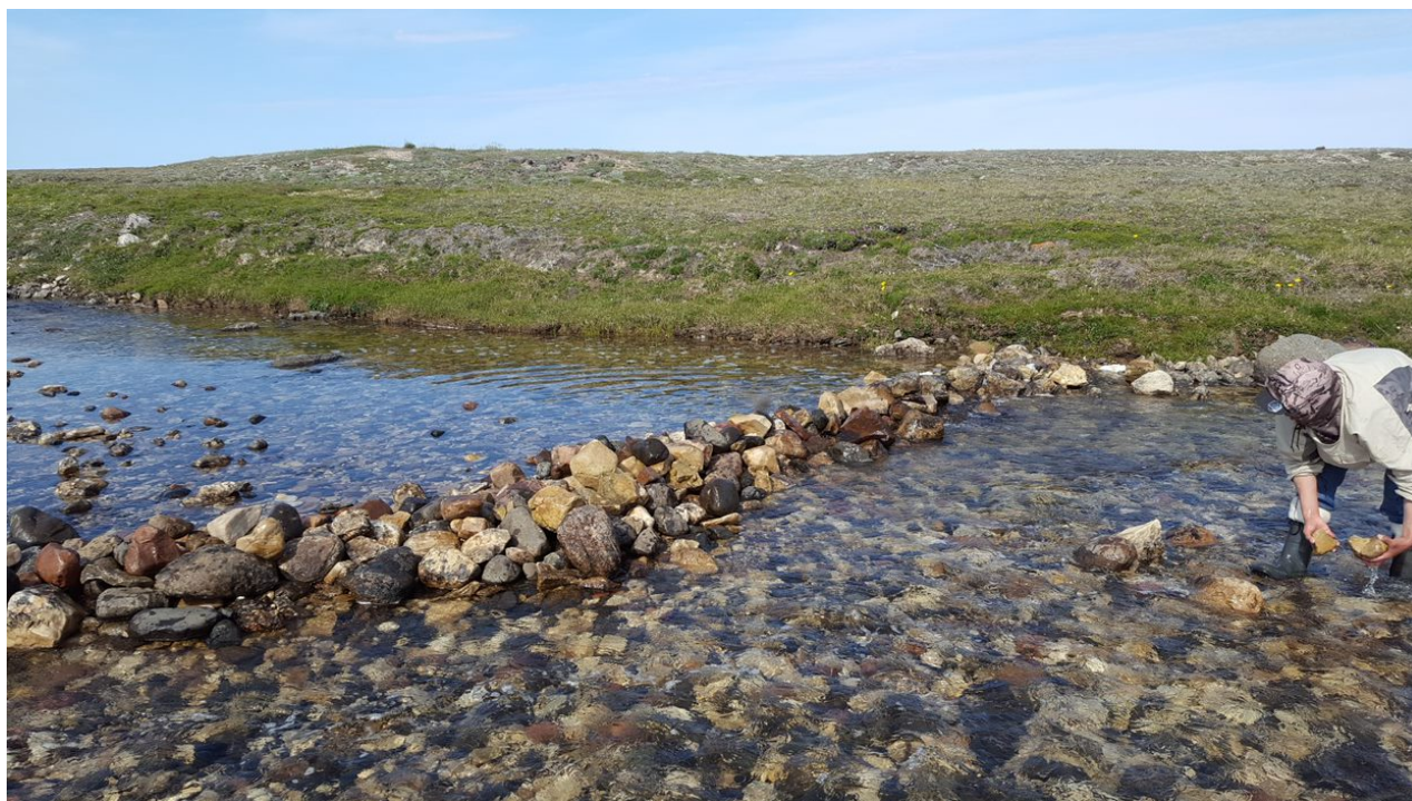
Photo 8: Local Participant Austin Manivogena Repairs a Weir, 25 July 2018
