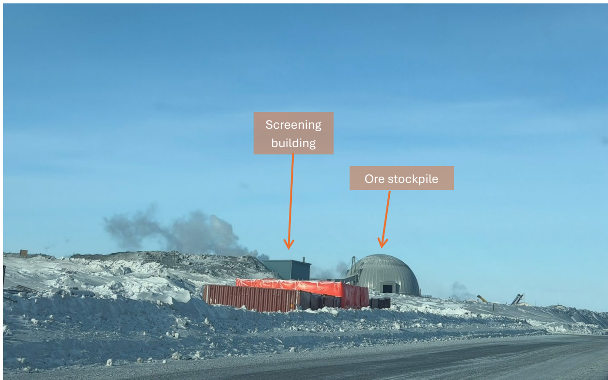
Photo 37: Screening building and ore stockpile dome facing west from Goose Lake
