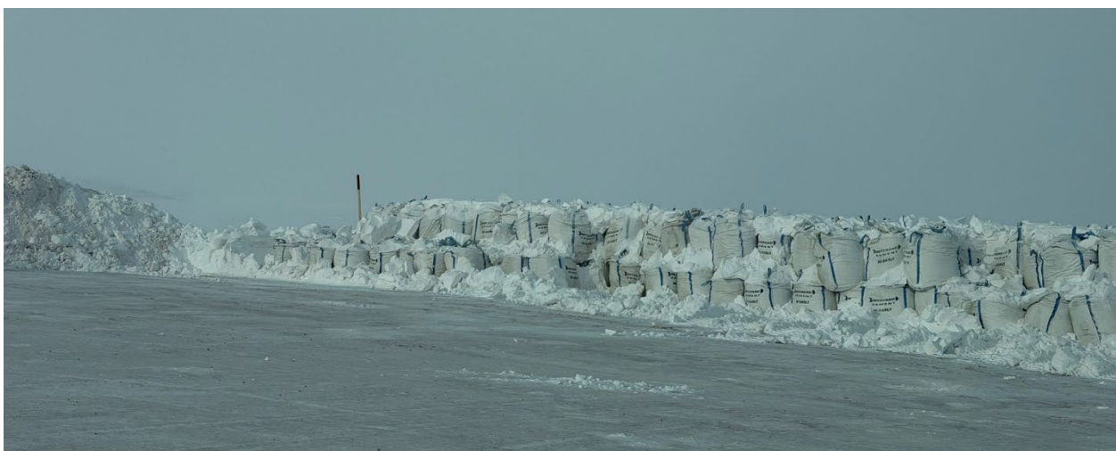
Photo 118: Concrete bulk bags
