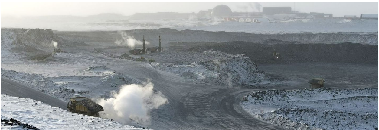
Photo 44: Close-up view of ongoing open-pit mining activities, looking southeast
