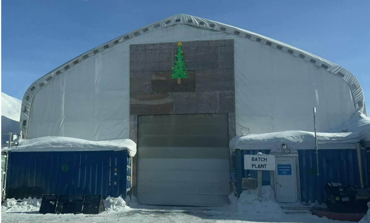
Photo 38: Batch plant located north of the ore stockpile dome
