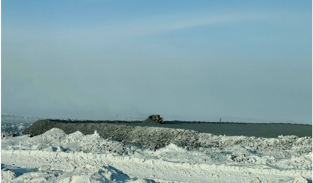
Photo 47: Umwelt WRSA facing west from the blasting area access road
