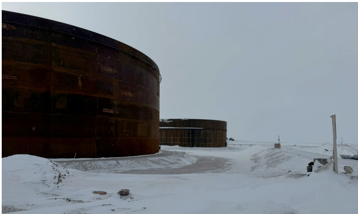
Photo 132: Fuel tanks within secondary containment, facing west
