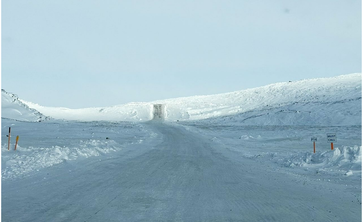
Photo 88: Portage 14, northbound to MLA
