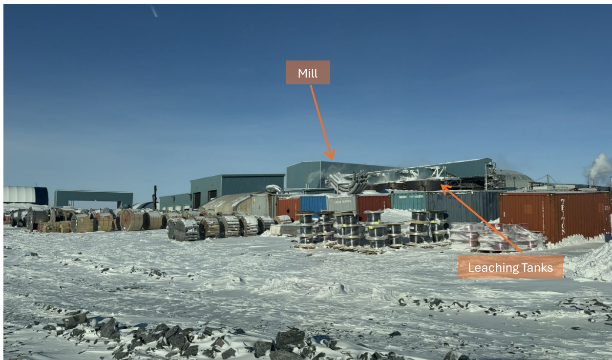
Photo 35: Leaching tanks, mill, and laydown area located north of the Tank farm
