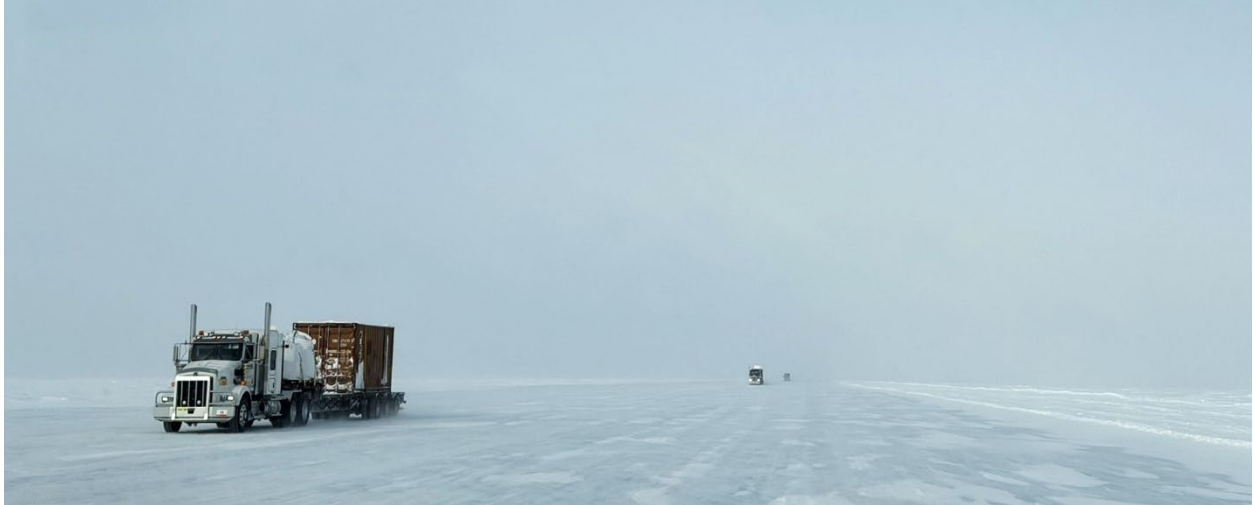
Photo 106: Truck traffic on sea ice section of the road, northbound view
