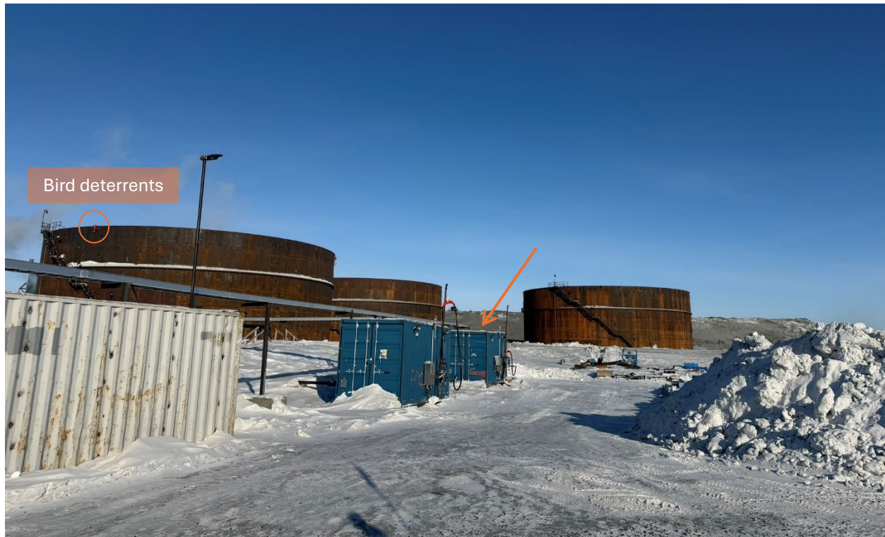
Photo 34: Fuel truck offloading area with spill containment catchments
