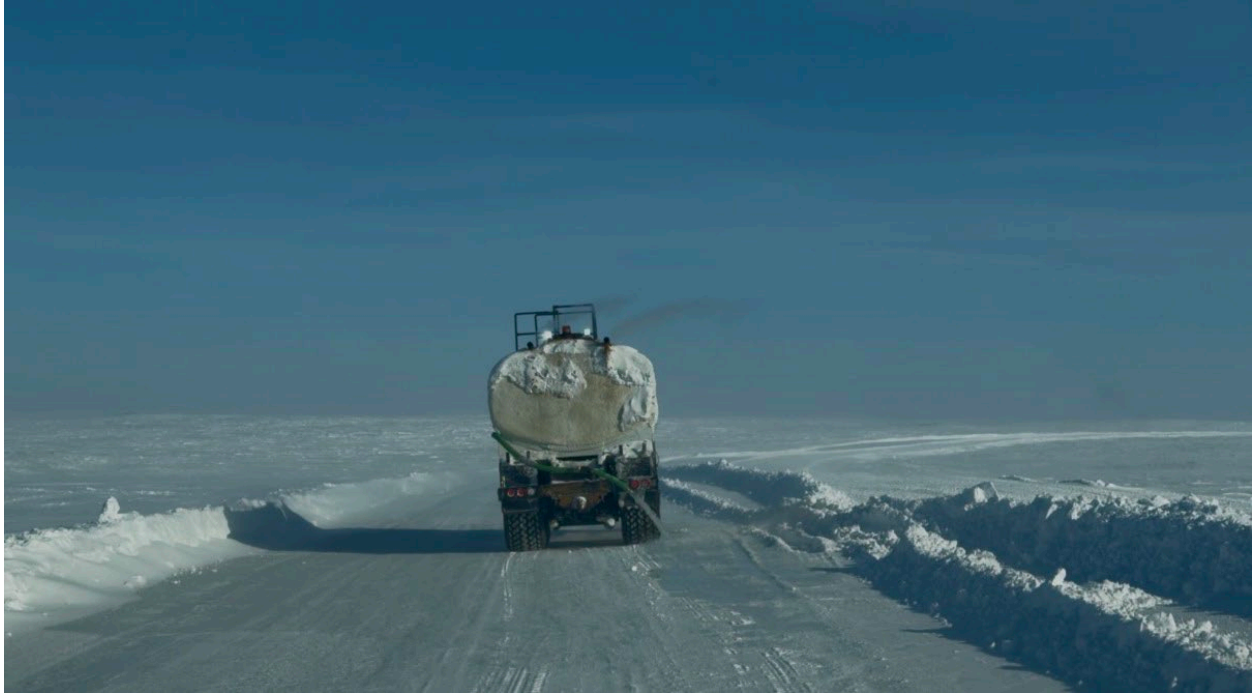
Photo 78: Water application on Portage P8 to strengthen the winter road surface
