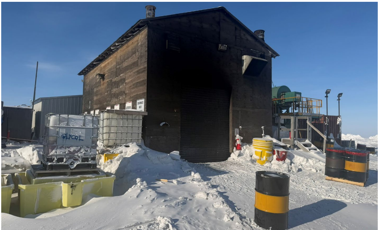
Photo 8: Incinerators and HAZMAT waste segregation (facing west)
