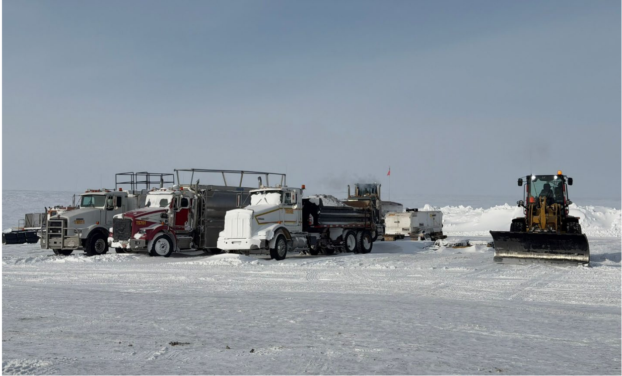
Photo 94: Equipment laydown area
