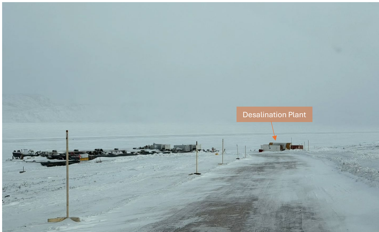
Photo 114: Cargo Offload Area and Desalination Plant
