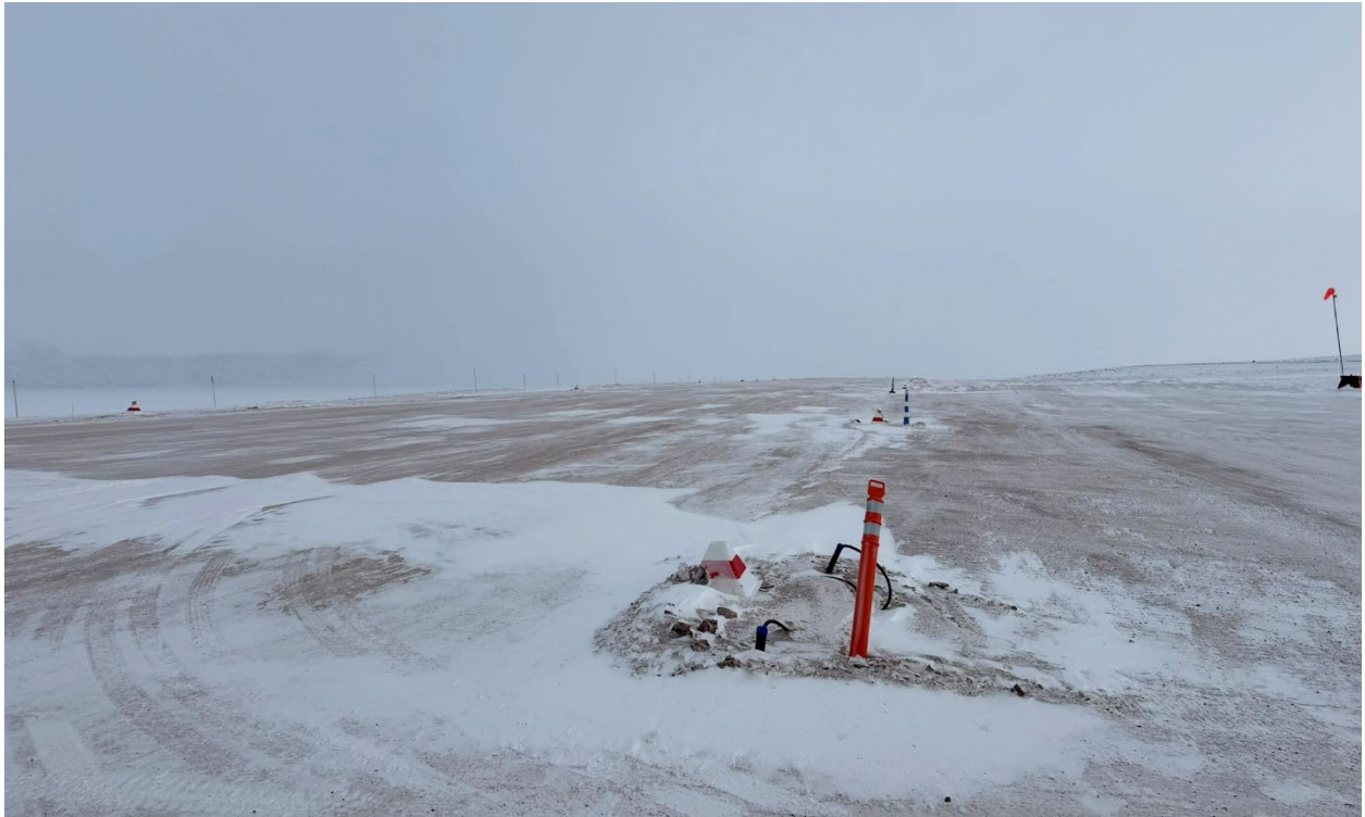
Photo 121: Airstrip, facing northwest
