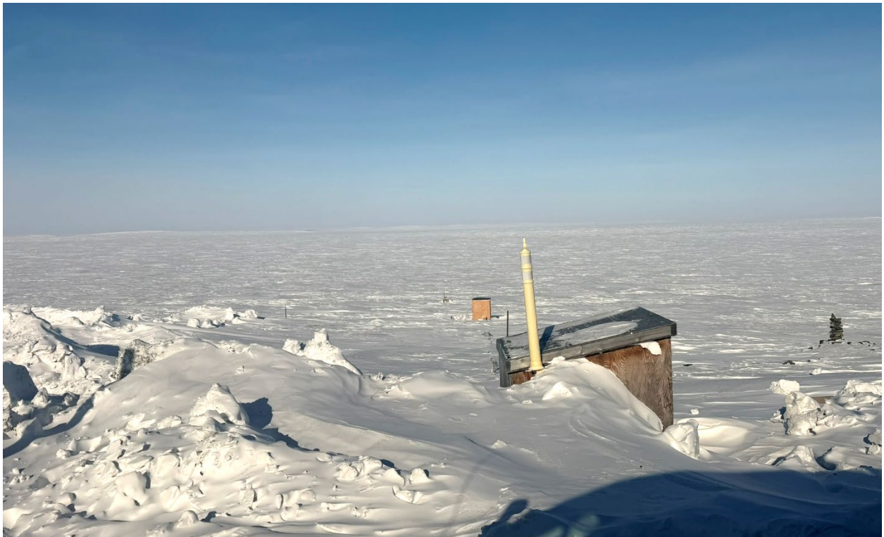
Photo 20: Water intake facility
