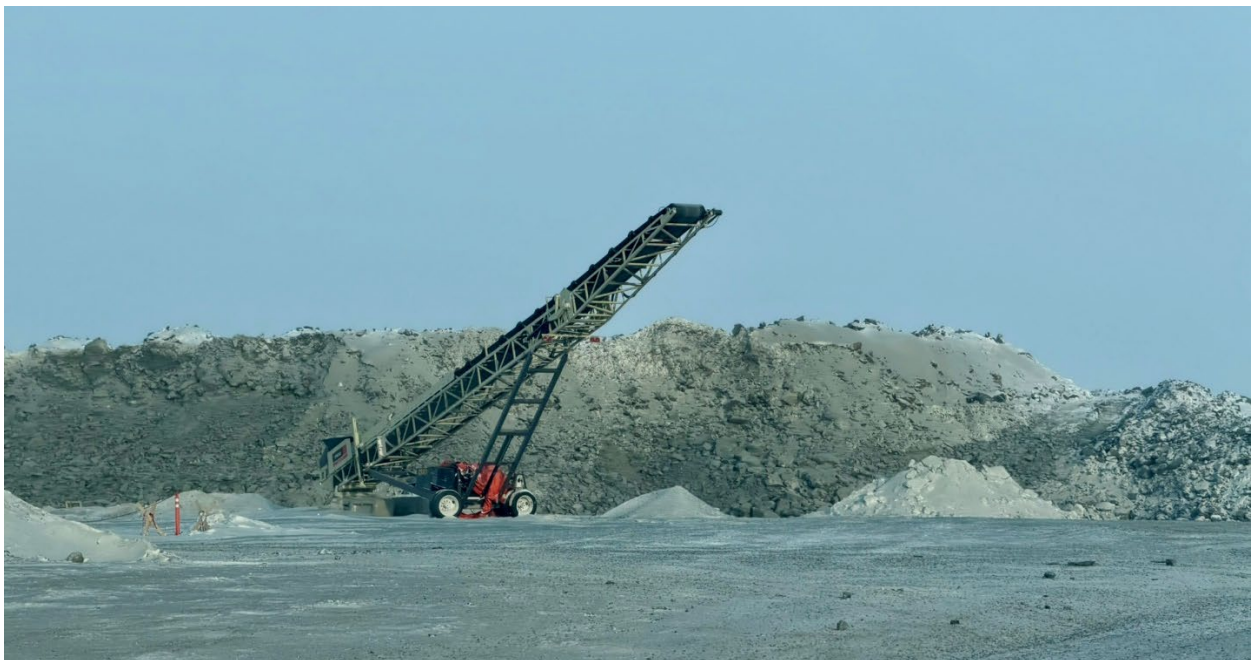
Photo 61: Crusher pad facing west from the access road
