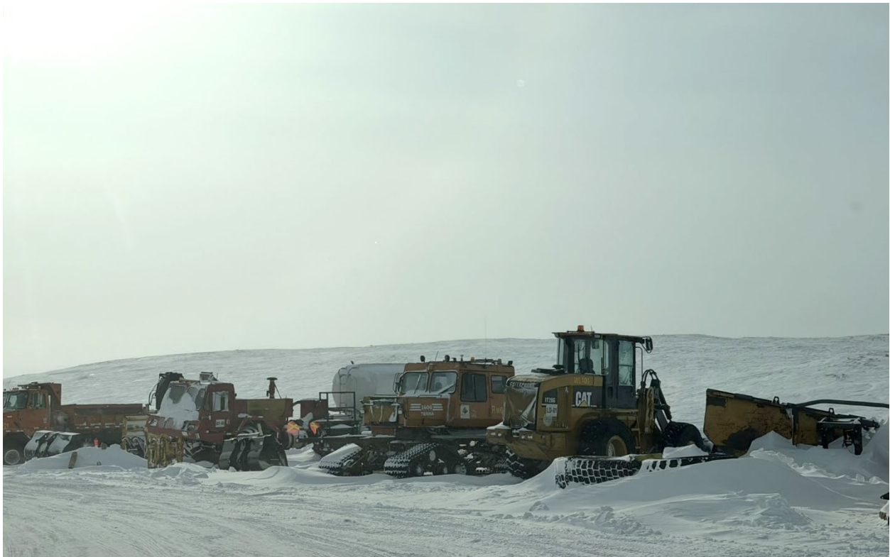
Photo 95: Equipment laydown area
