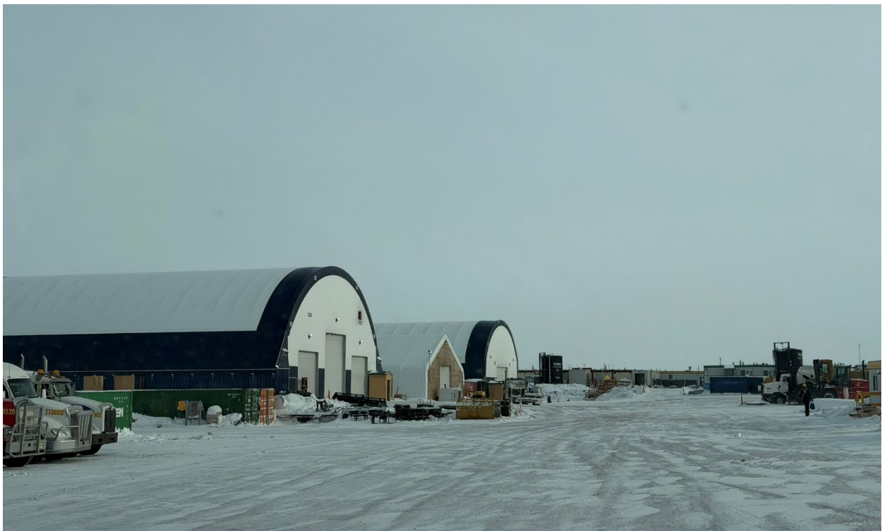
Photo 120: Maintenance shop and Warehouse, facing east
