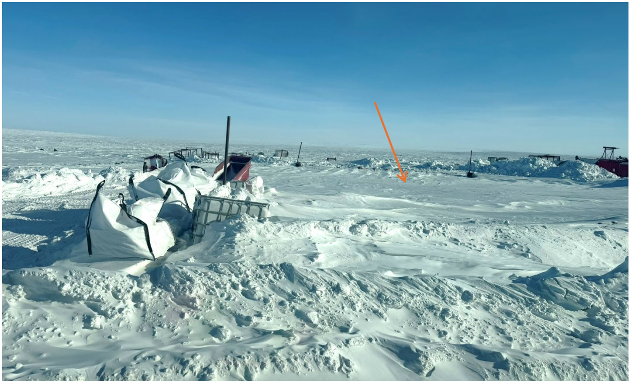
Photo 18: Settling pond area, currently frozen and snow-covered
