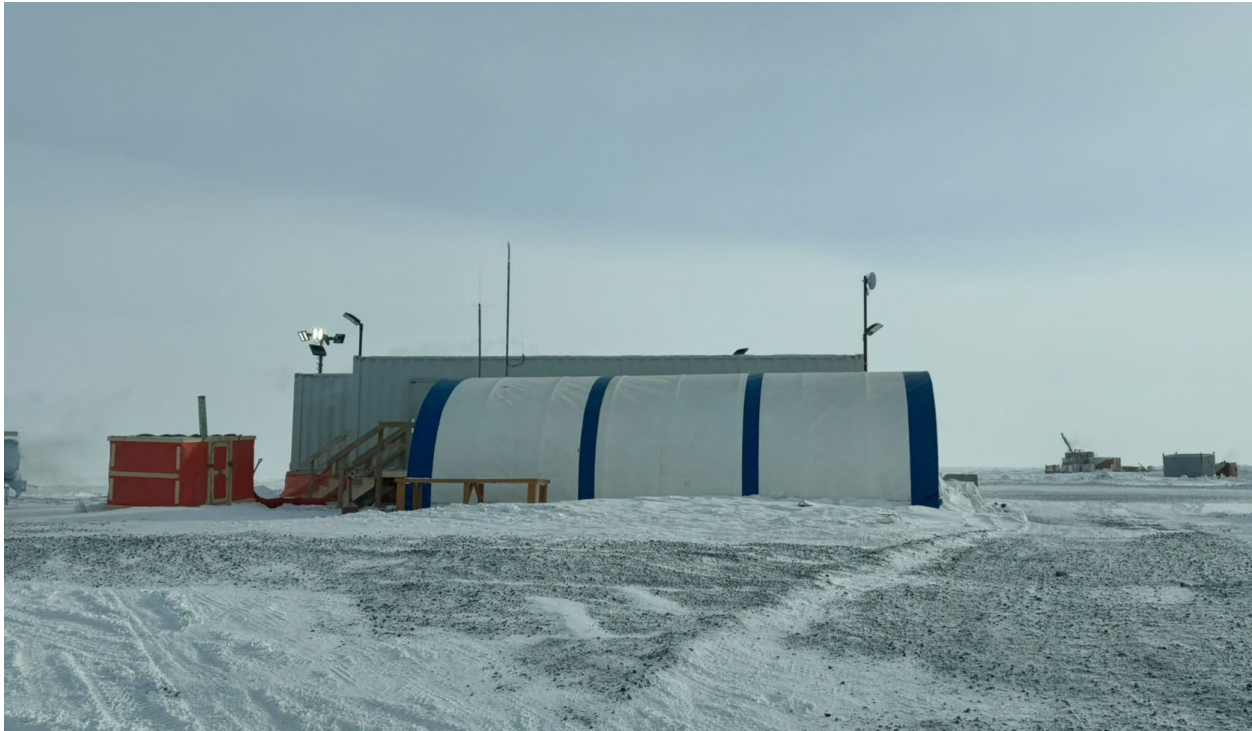
Photo 68: Dispatch building and staging area in the background
