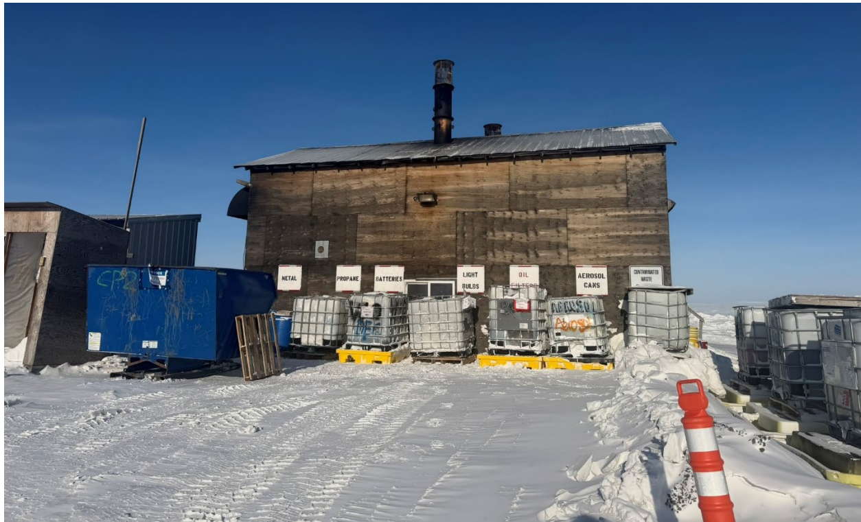
Photo 9: Incinerators and HAZMAT waste segregation (facing north)
