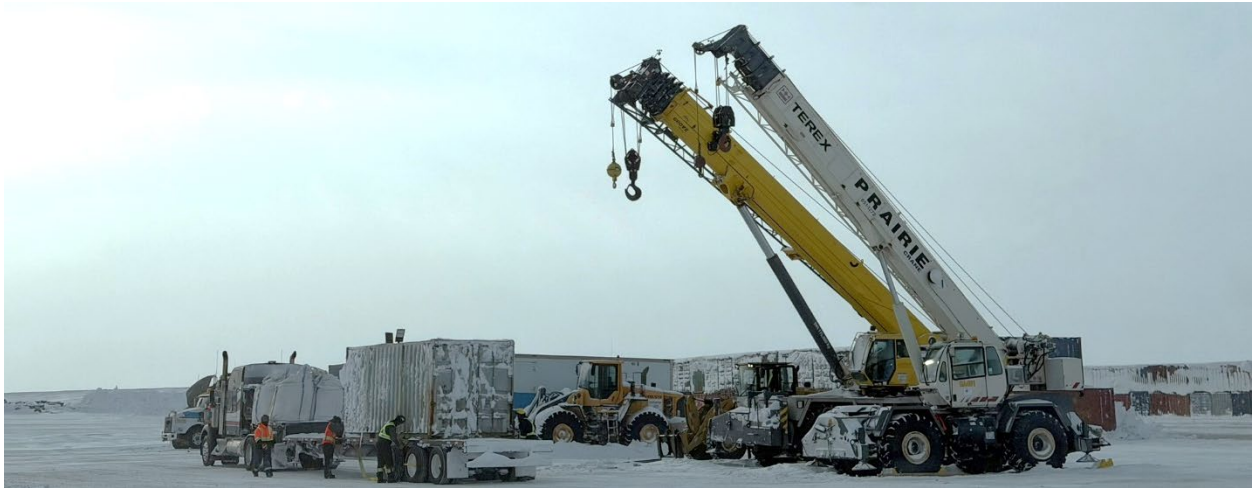
Photo 116: A truck being loaded at lower laydown
