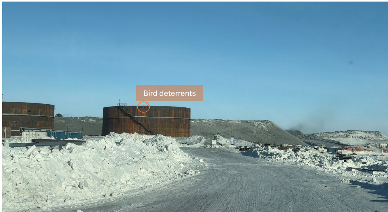
Photo 31: Tank farm access road, looking east, with laydown areas on the right
