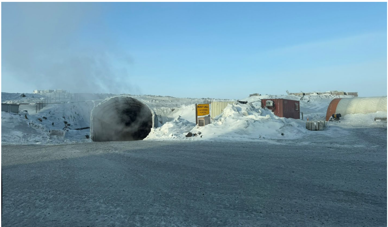
Photo 41: Underground portal facing southwest
