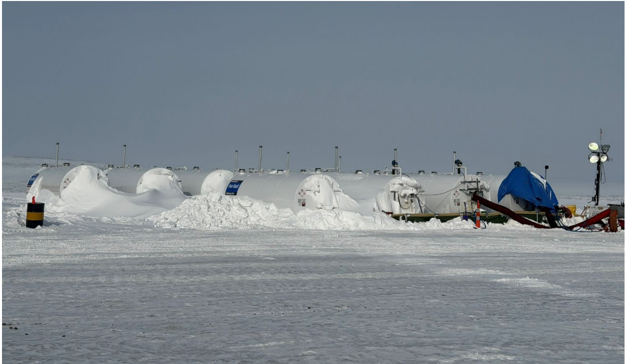
Photo 96: Fuel tanks in secondary containment
