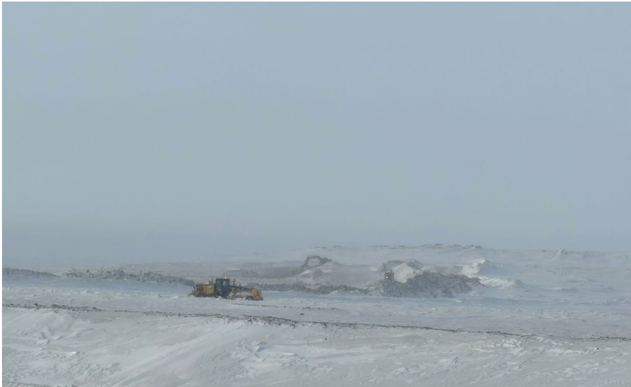
Photo 53: Saline Water Pond construction ongoing, facing southwest from the Umwelt pit
