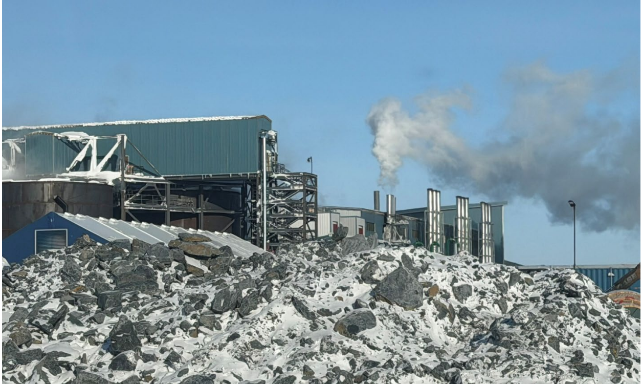
Photo 36: Powerhouse located north of the Tank farm
