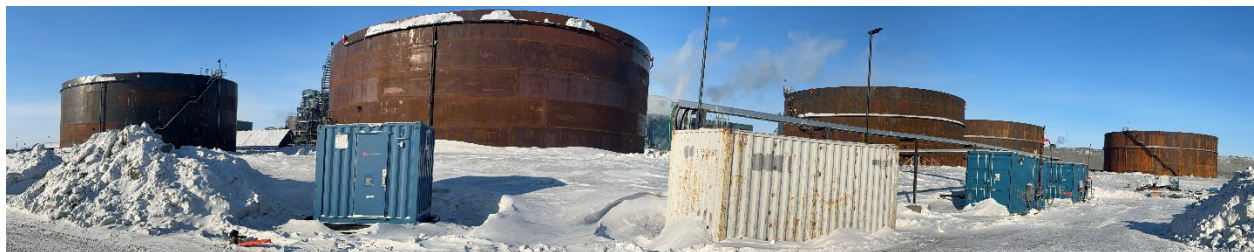
Photo 33: Panoramic view of the Tank farm
