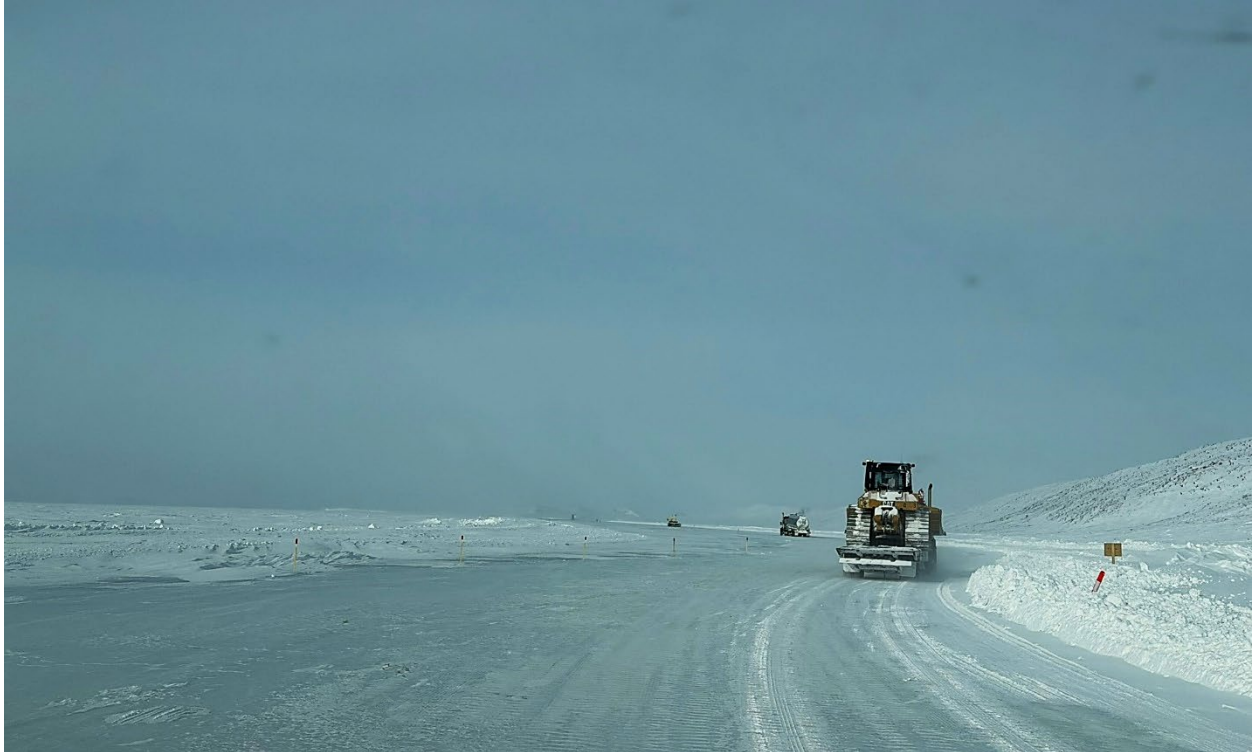
Photo 100: Road along the eastern edge of Bathurst Lake (~ Km 120) with traffic signage present and a 10 km/h speed restriction in effect
