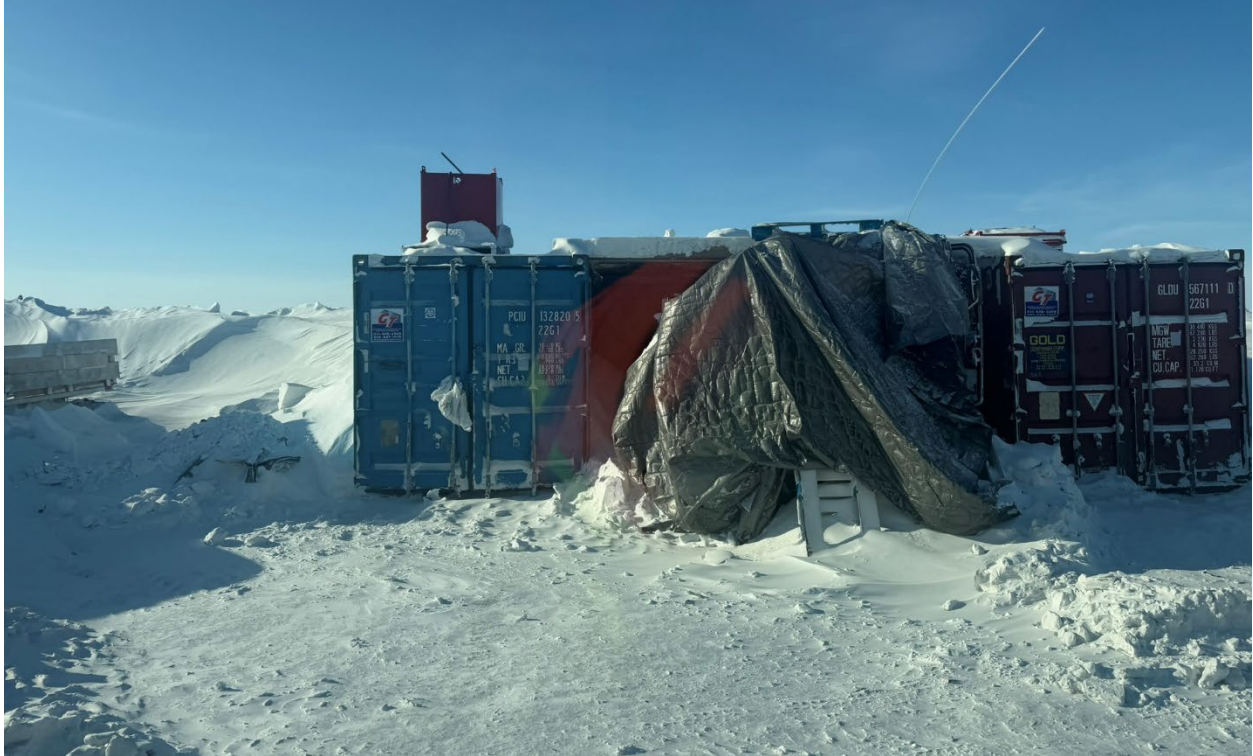
Photo 17: Improperly secured seacans east of the air traffic control unit
