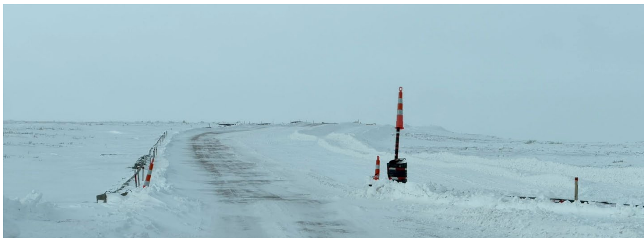
Photo 127: Fuel transfer line running along the fuel transfer road toward the tank farm, facing north
