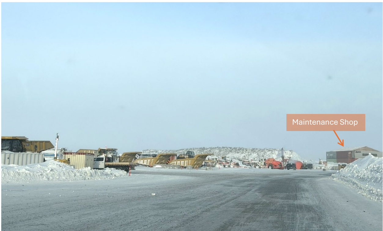
Photo 63: Equipment laydown area and maintenance shop located southwest of the Llama crushers
