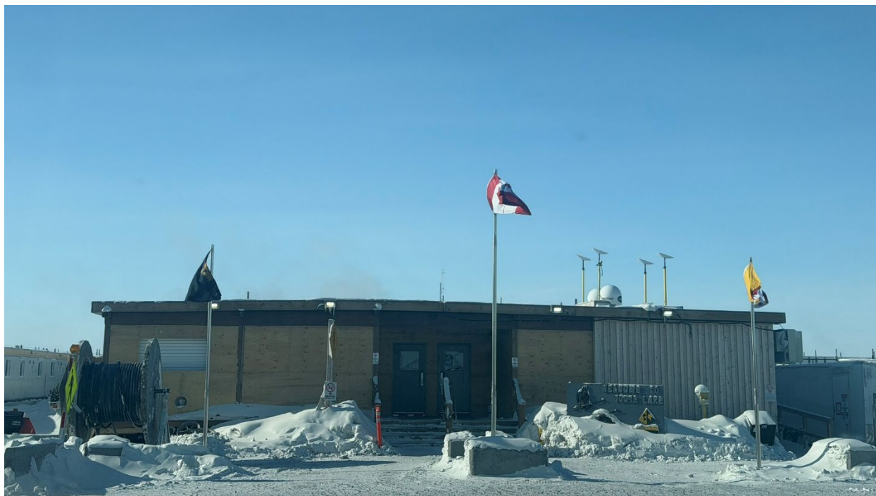
Photo 64: Goose camp main entrance
