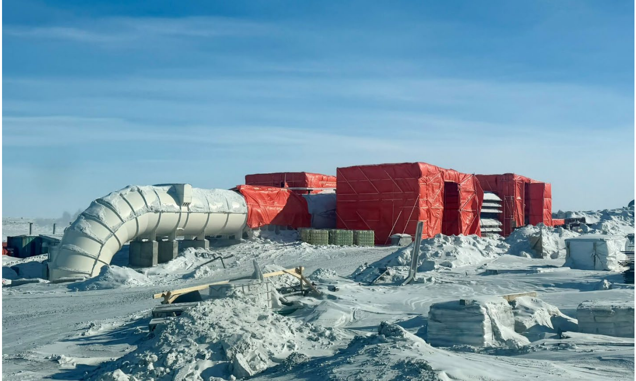
Photo 40: Fresh air intake 2 (construction ongoing)
