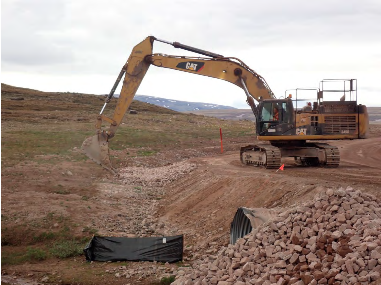
Excavator lining swale in the upstream south swale at BG-04 with rip-rap stone
