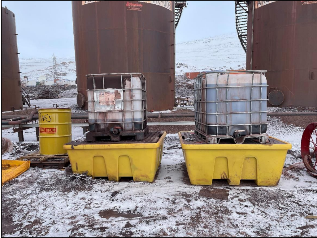
Photo 9: Mine Site Fuel Tank Farm and Secondary Containment for oil storage.
