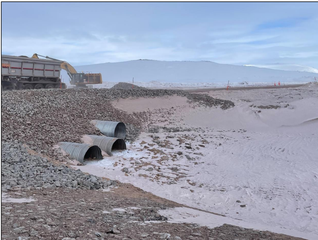
Photo 40: Completed Culvert Repair on the West side of the Tote Road.
