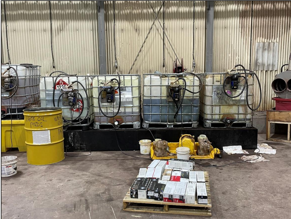
Photo 11: Secondary Containment for Fluid Dispensing Station inside the Incinerator Facility.
