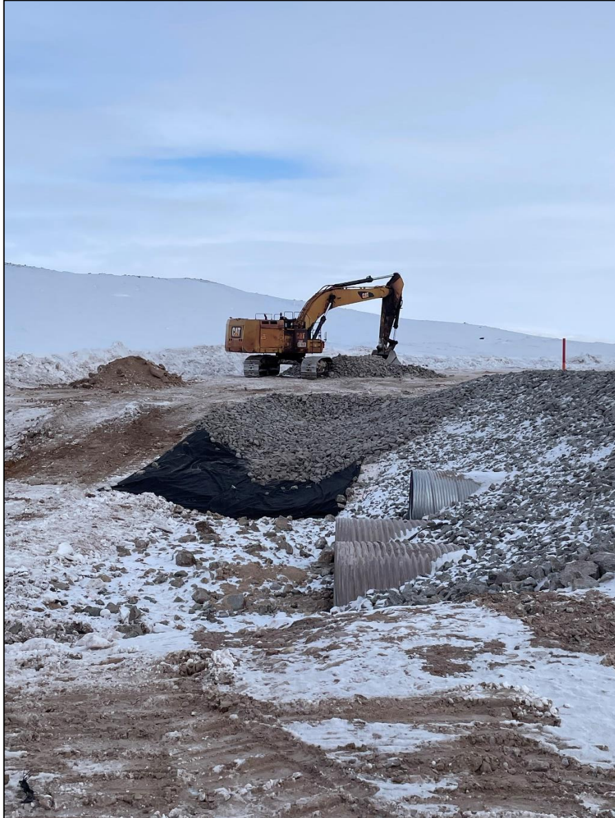
Photo 41: Installation of riprap in Completing Culvert Repair on the East Side of the Tote Road.
