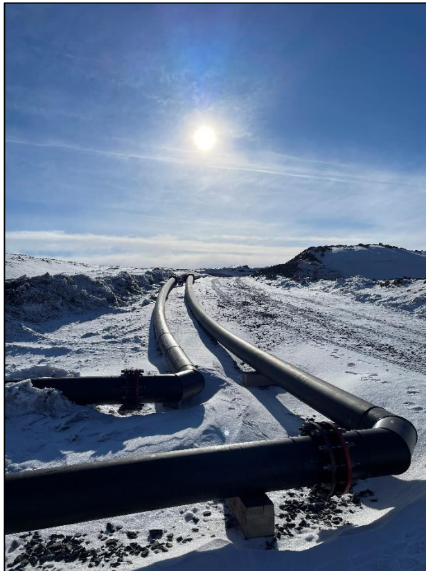
Photo 32: Recirculation piping for Effluent that doesn't Meet Discharge Criteria
