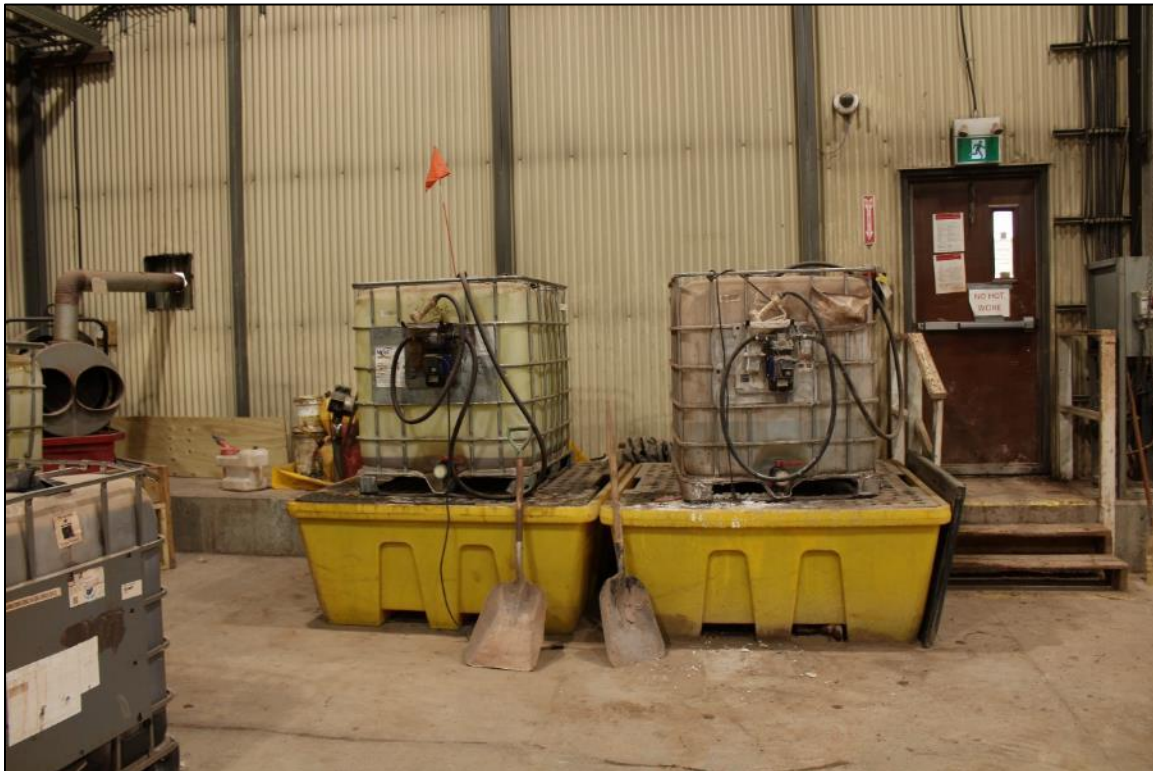
Photo 37: Secondary Containment for Fluid Dispensing Station inside the Incinerator Facility.
