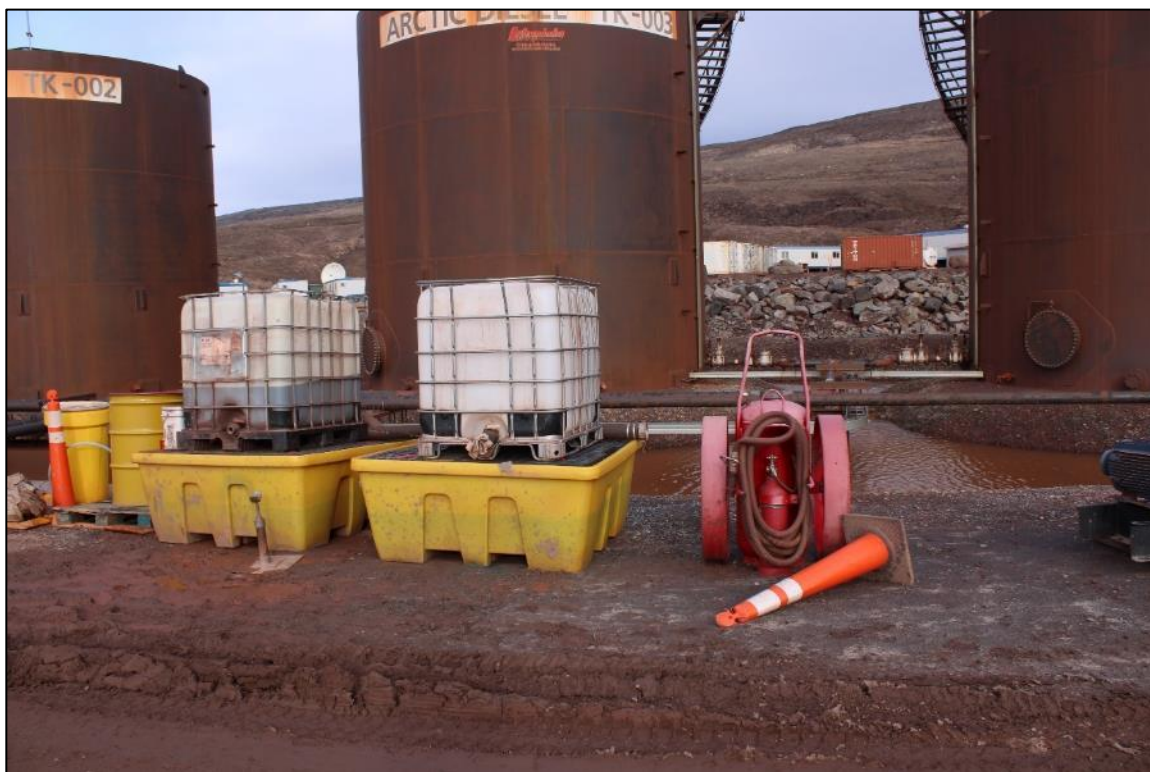
Photo 23: Mine Site Fuel Tank Farm and Secondary Containment for Windshield Wiper Fluid.
