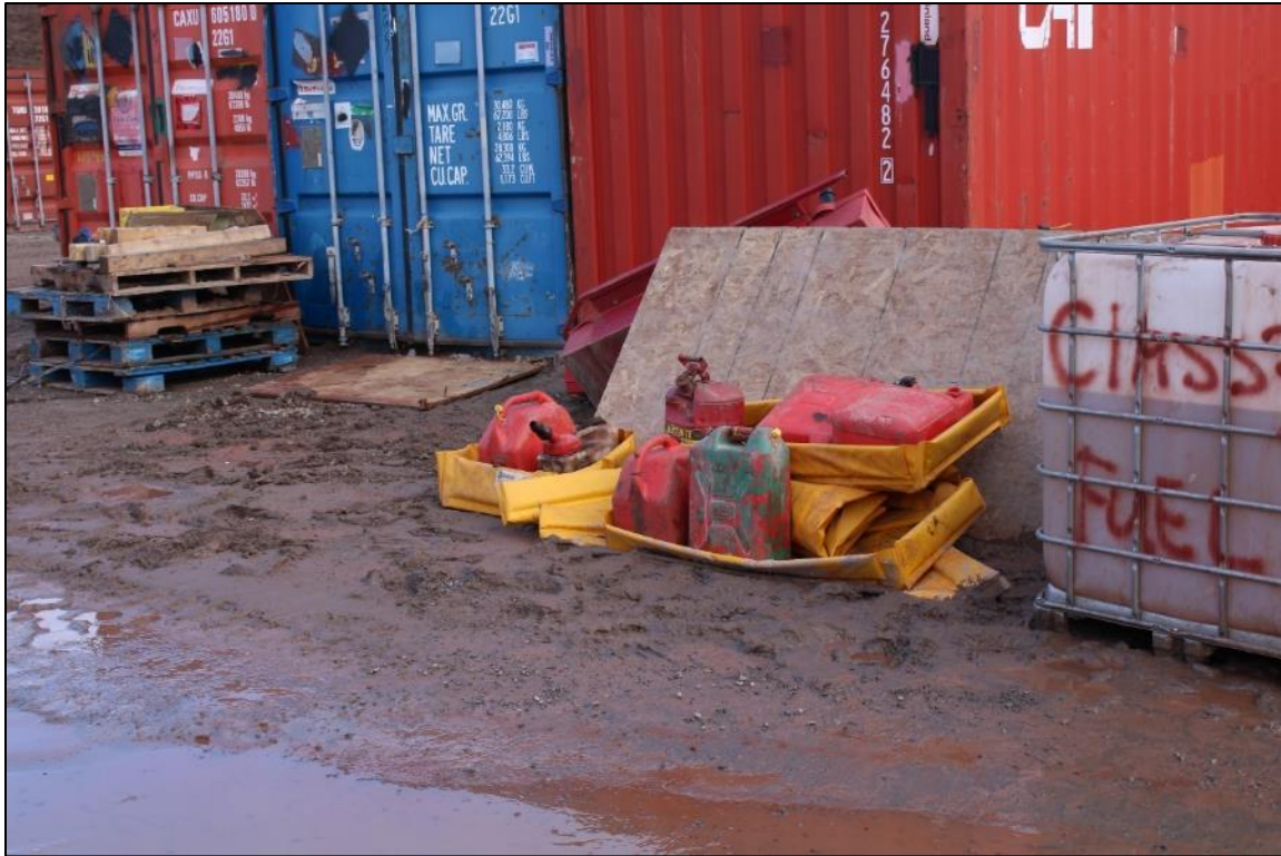
Photo 40: Hazardous Waste Storage Area with Secondary Containment Incorrectly Installed.
