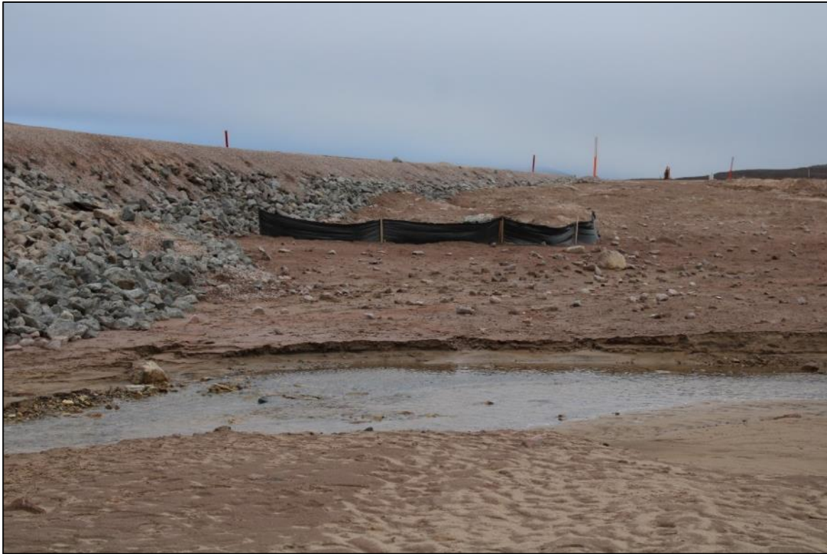
Photo 45: Silt Curtain Installed near the Culverts along the Tote Road.
