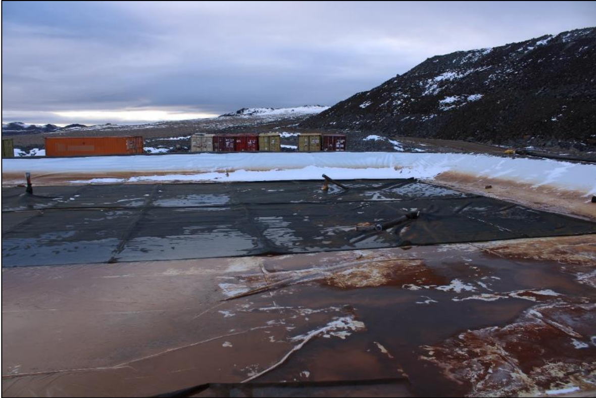
Photo 28: Decommissioned Sedimentation Pond and Geotube from Water Treatment Plant for Run off Water from the Waste Rock Facility.
