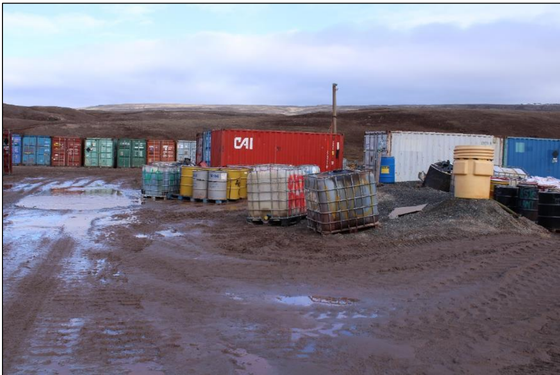
Photo 41: Hazardous Waste Storage Outside of the Lined Area
