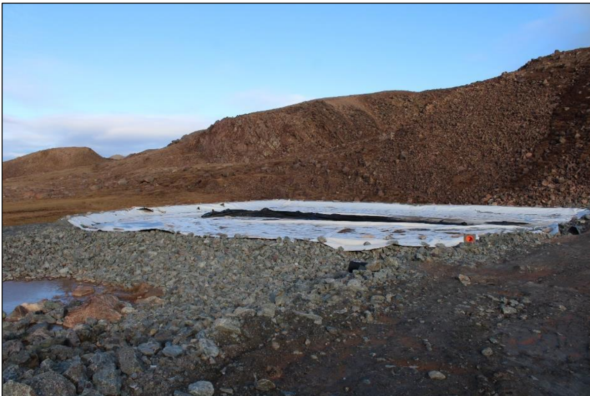
Photo 20: KM 105 Dam Downstream Geotube.
