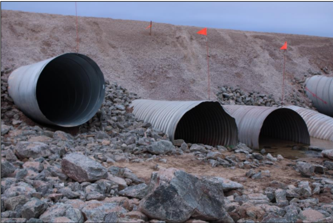
Photo 42: Culvert Repair at KM 80 that Failed.
