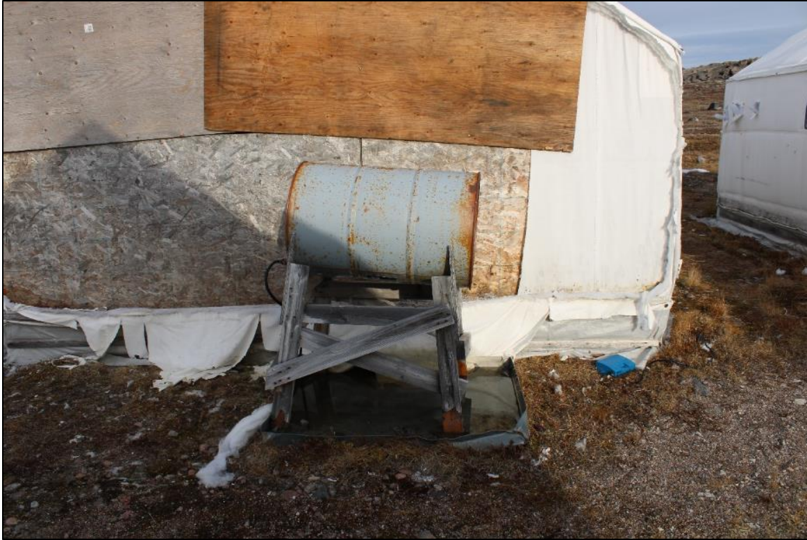
Photo 64: Damaged Secondary Containment on camp Fuel Barrel.
