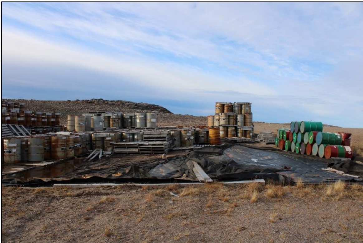
Photo 63: Fuel Storage and Damaged Secondary Containment.
