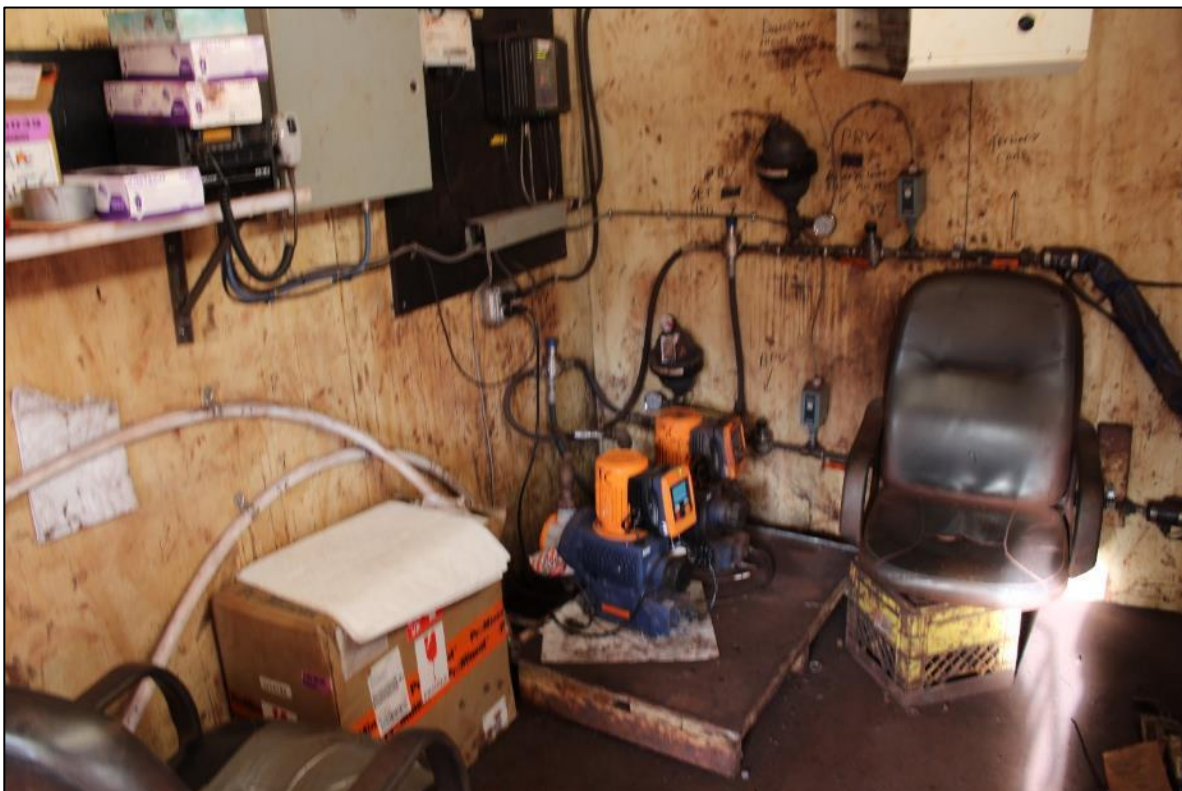
Photo 14: Pump System for Liquid Dust Suppressant.
