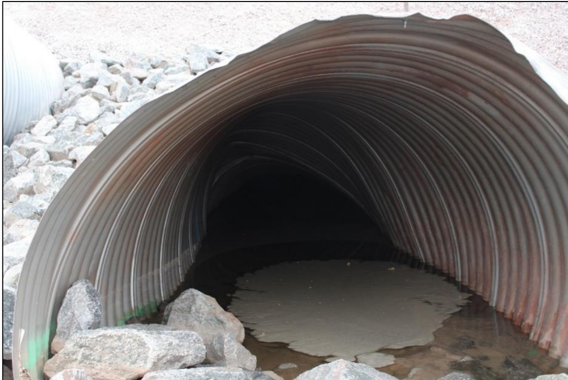
Photo 43: Blocked Culvert at KM 80.
