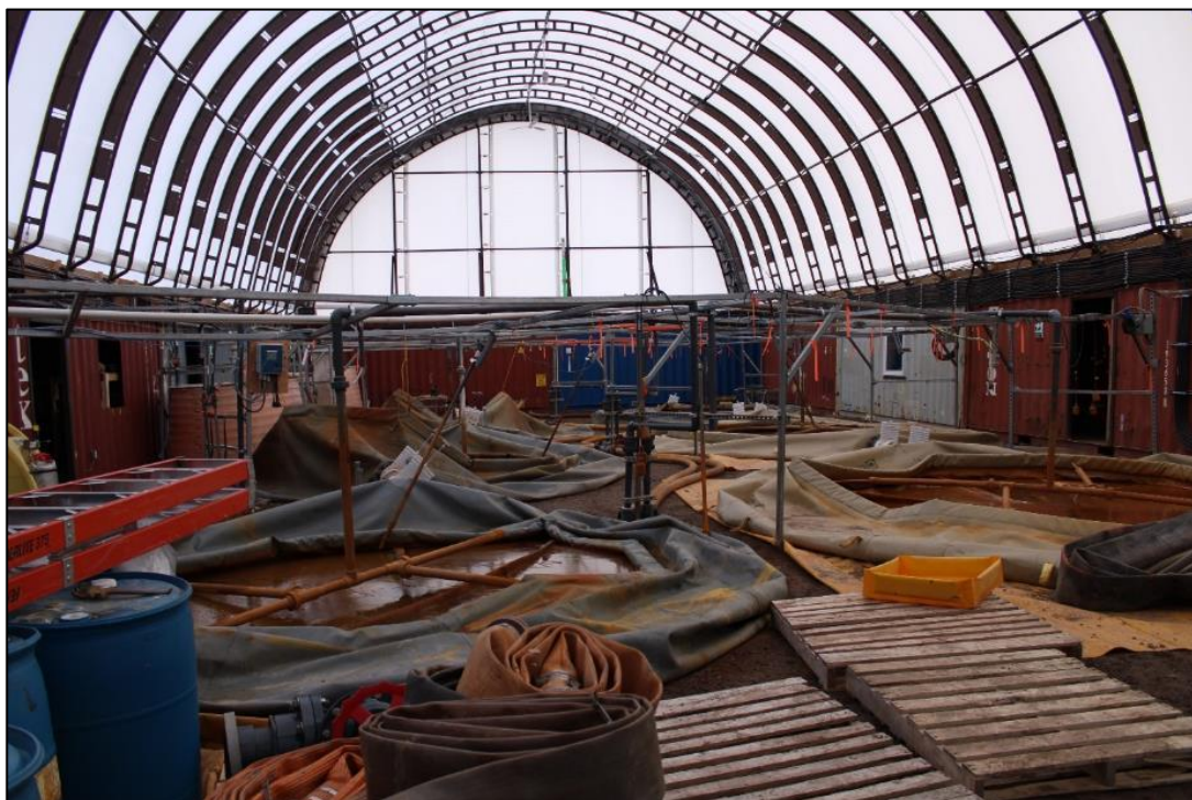
Photo 27: Decommissioned Water Treatment Plant for Run off Water from the Waste Rock Facility.
