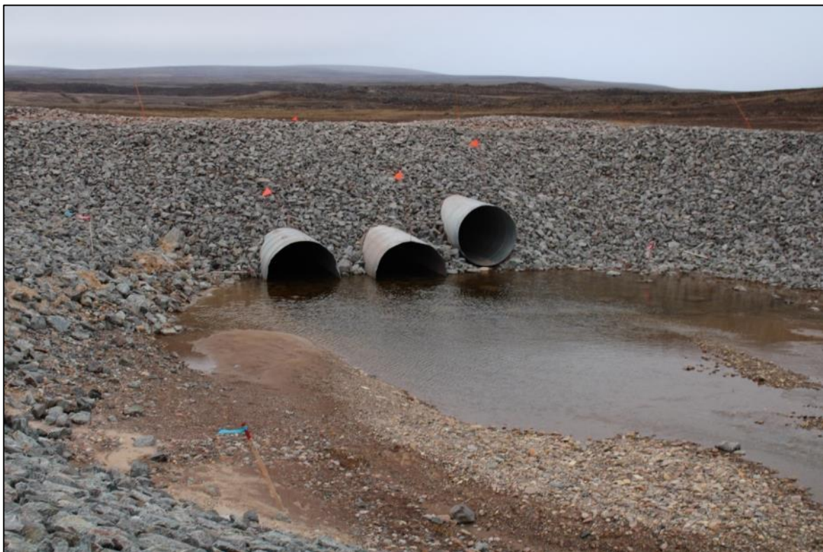
Photo 44: Culvert at KM 90 that was Successfully Replaced.
