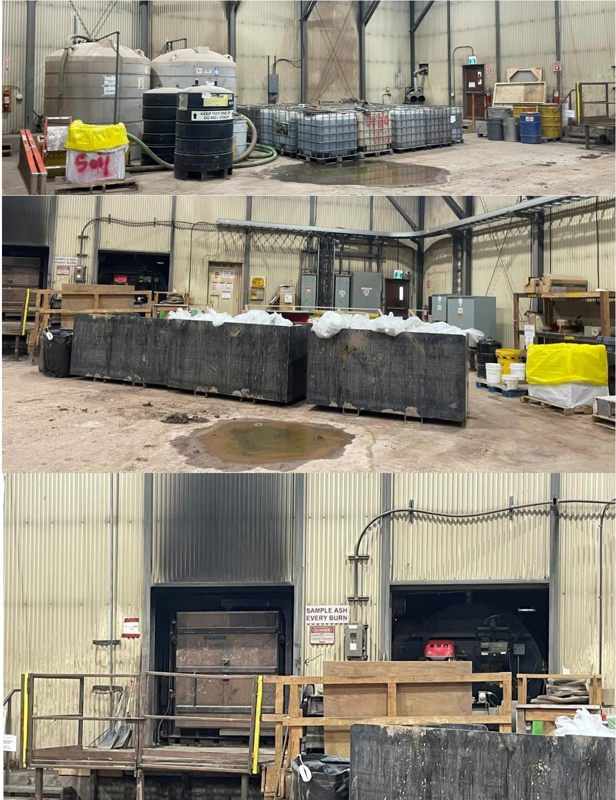
Photo 34: Mary River Incinerator Building
