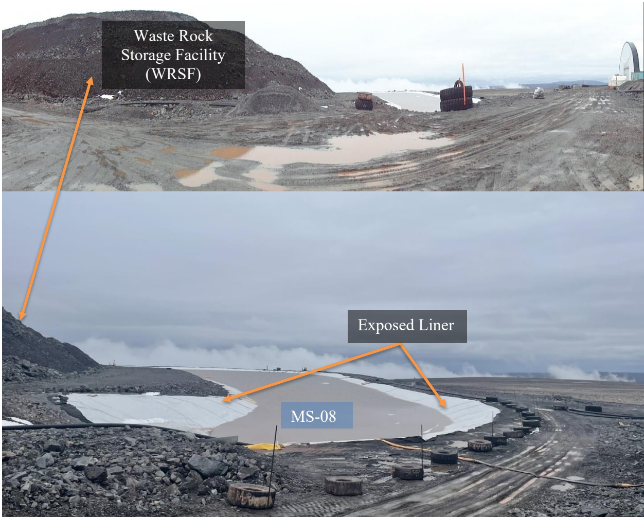
Photo 9: Lined Surface Water Management Pond (MS-08 Pond) next to Waste Rock Storage Facility
