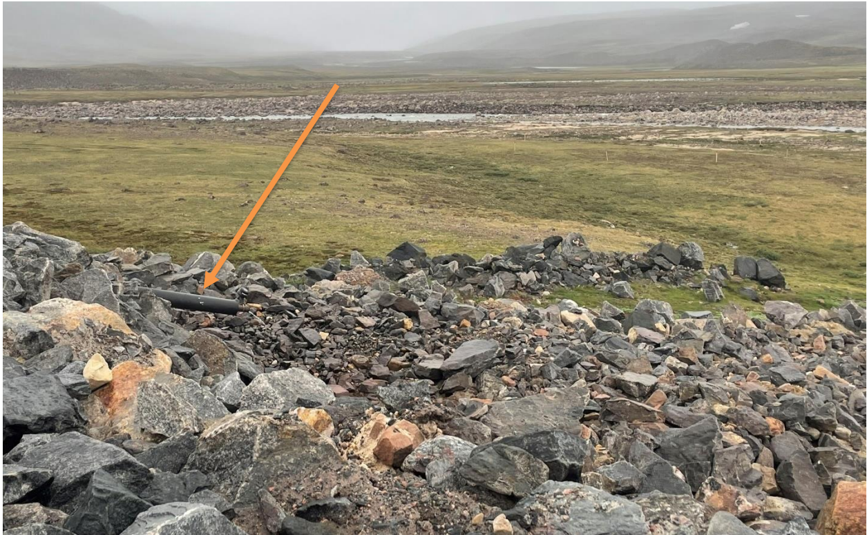
Photo 32: Treated water outlet with passive filtration at Water Discharge Area
