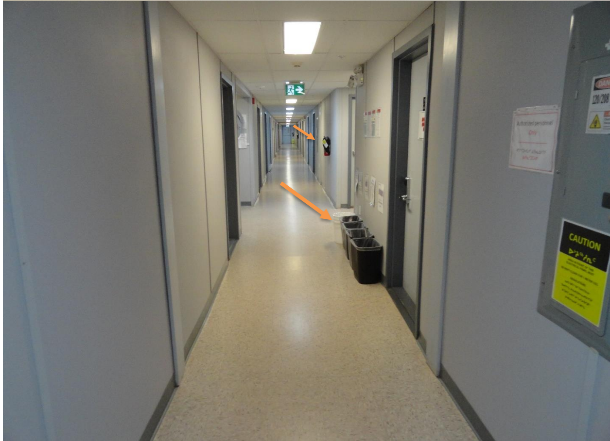
Photo 40: Waste sorting guidelines, bins, and fire extinguisher in Camp Hallway
