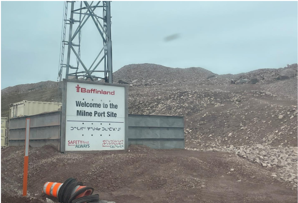
Photo 62: Communication Tower and Welcome Sign
