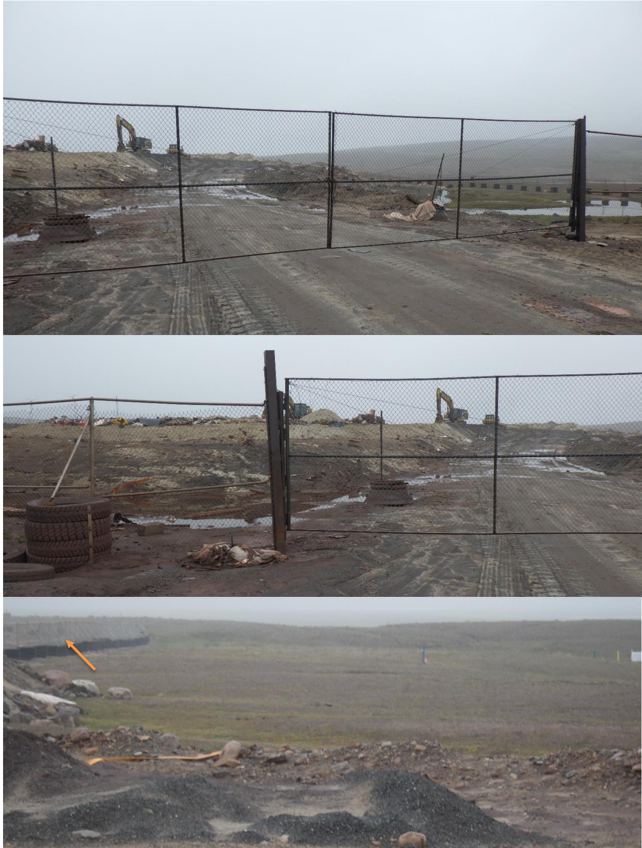
Photo 29: Main Landfill Facility
