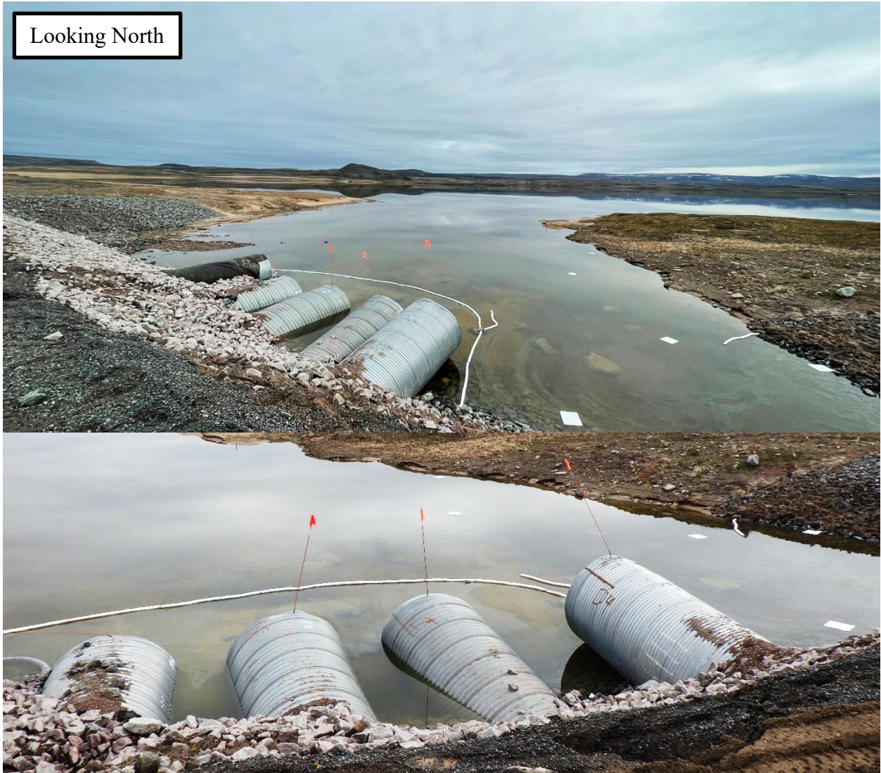
Photo 48: Culvert Inlet at KM80 (Looking South) requiring Replacement; hydraulic fluid spill observed.
