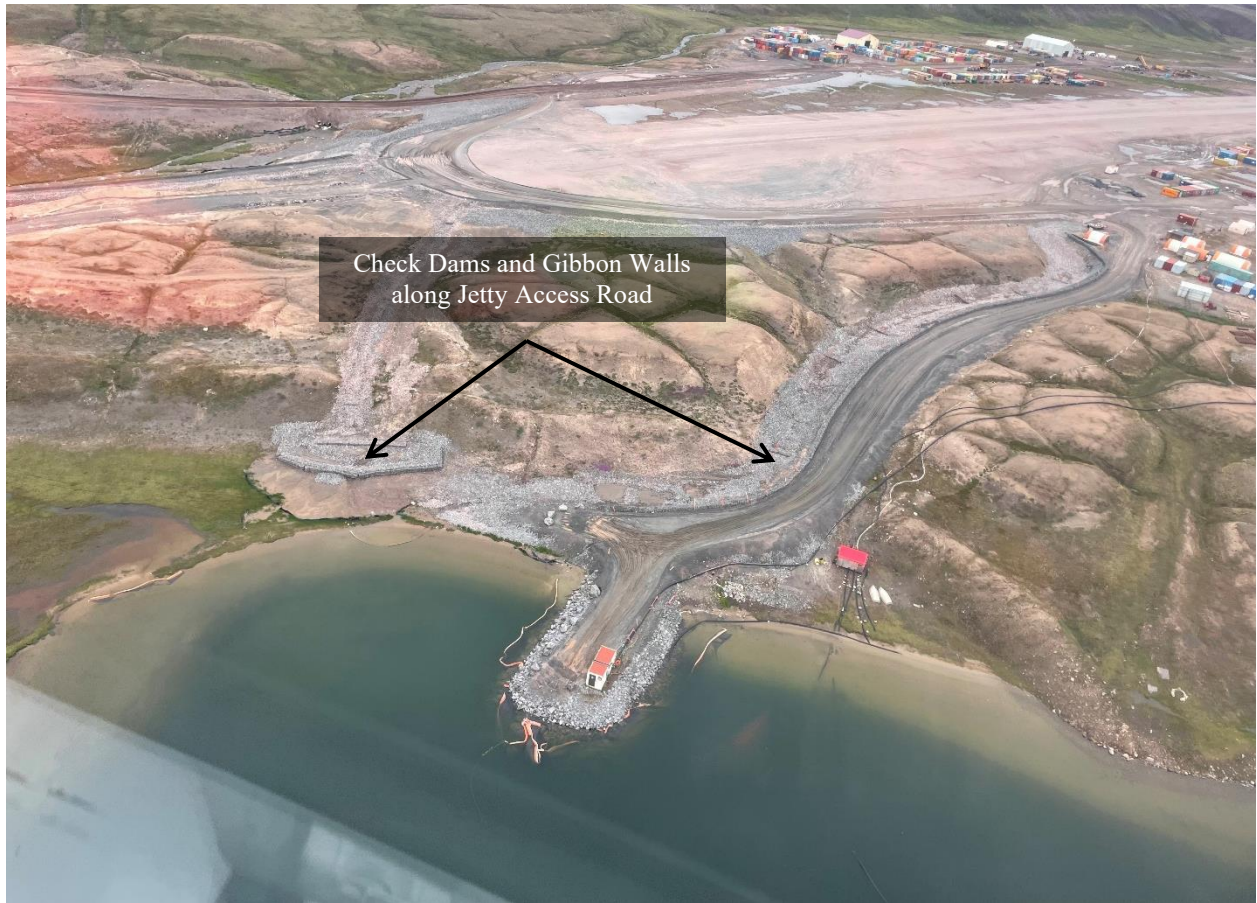
Photo 36: Aerial View of Camp Lake and Water Intake Jetty
