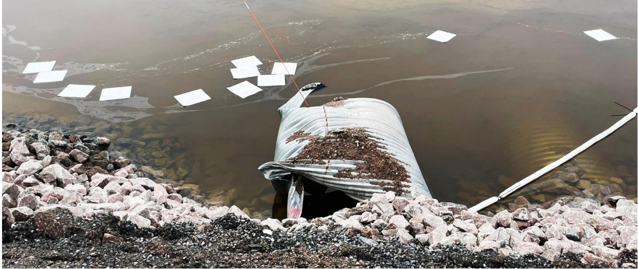
Photo 48: Culvert Inlet at KM80 (Looking South) requiring Replacement; hydraulic fluid spill observed.
