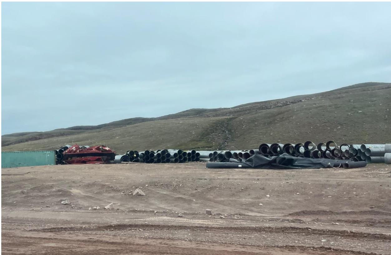
Photo 60: Culvert construction material laydown
