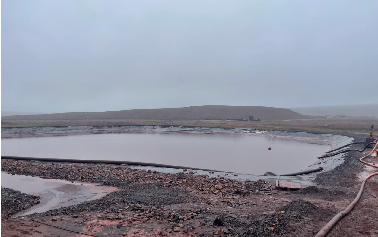
Photo 25: Surface Water Management Pond (SM-06) adjacent to the Crusher Pad
