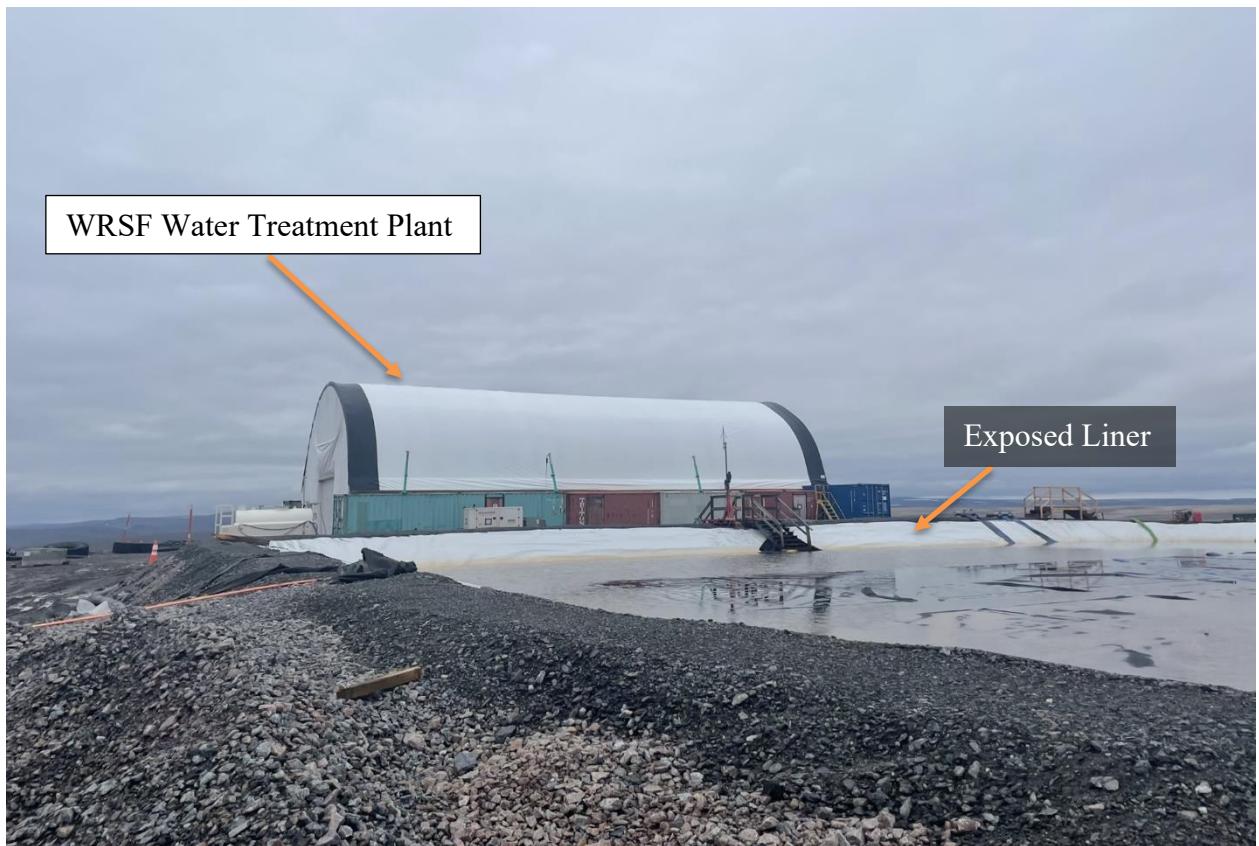
Photo 7: Lined Treatment Cell (Geotube Pond) next to the WRSF Water Treatment Plant
