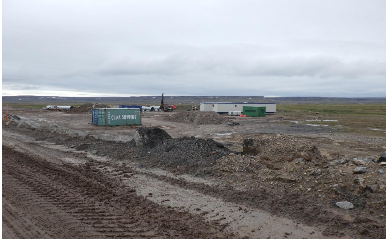
Photo 52: Ongoing culverts replacement work
