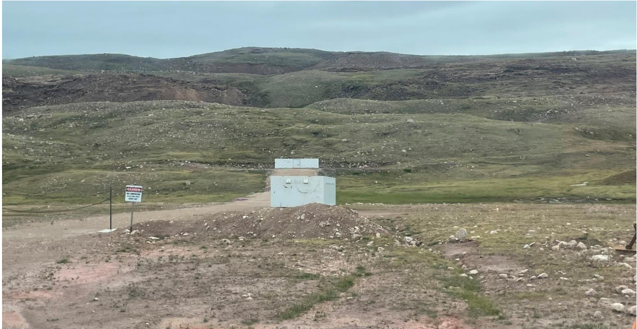
Photo 61: Explosives Magazines near Blasting Area KM 7
