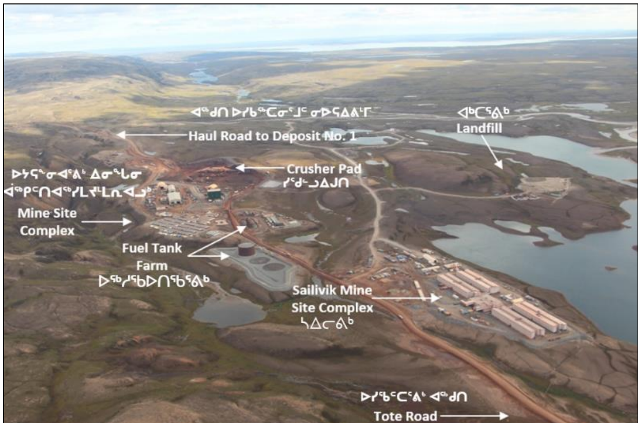
Photo 2: Aerial View of Mary River Site
