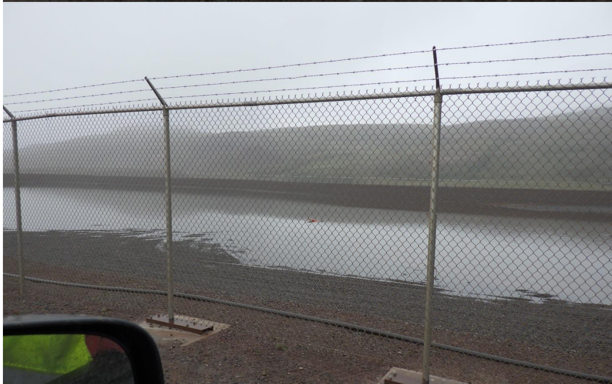
Photo 23: Chain link fence and secondary containment around Fuel tank at MS-03B
