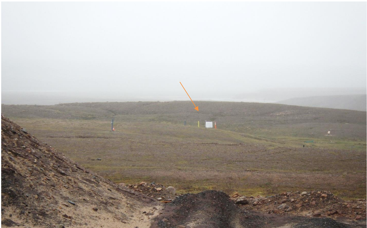
Photo 26: Water Monitoring Well (installed in April 2025)
