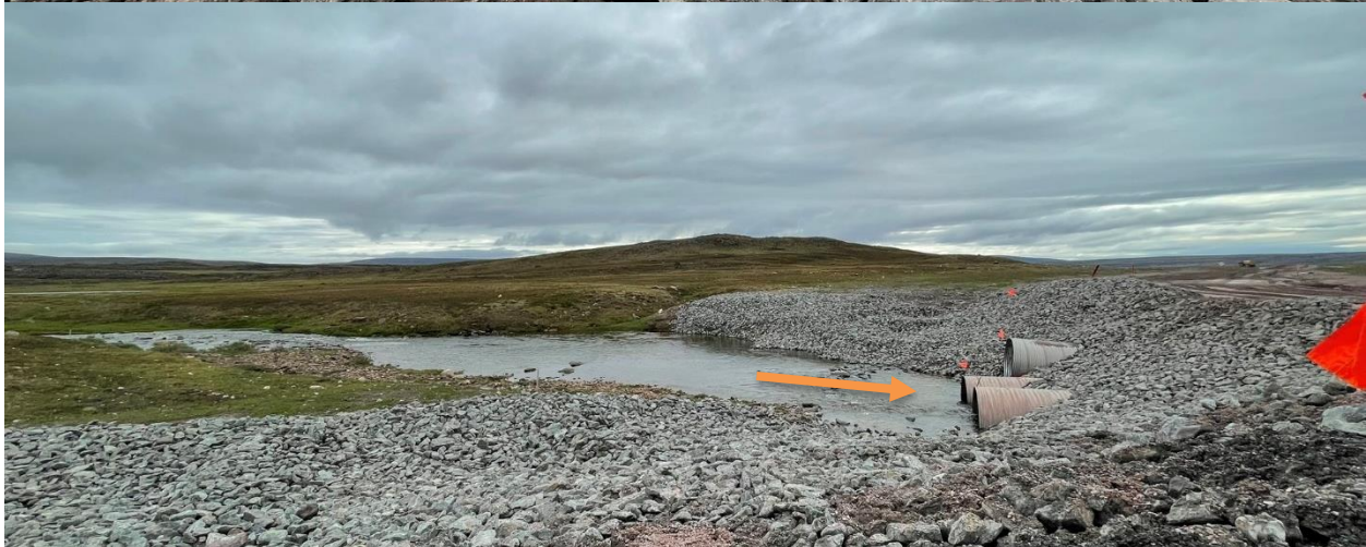
Photo 45: KM94 culverts observed to be clear and functional
