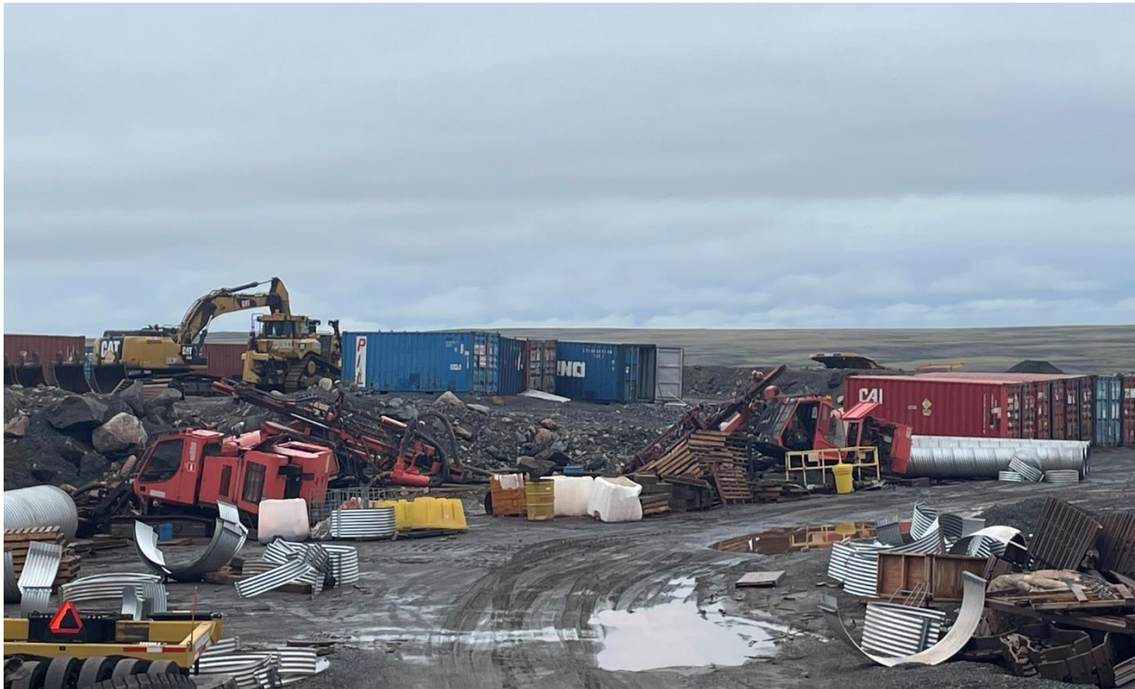
Photo 16: KM 105 Construction Materials Laydown Area
