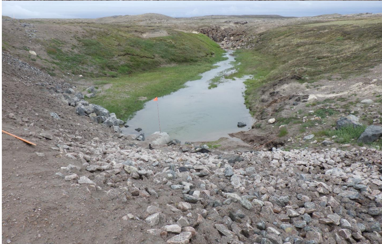
Photo 47: Culverts at KM 85
