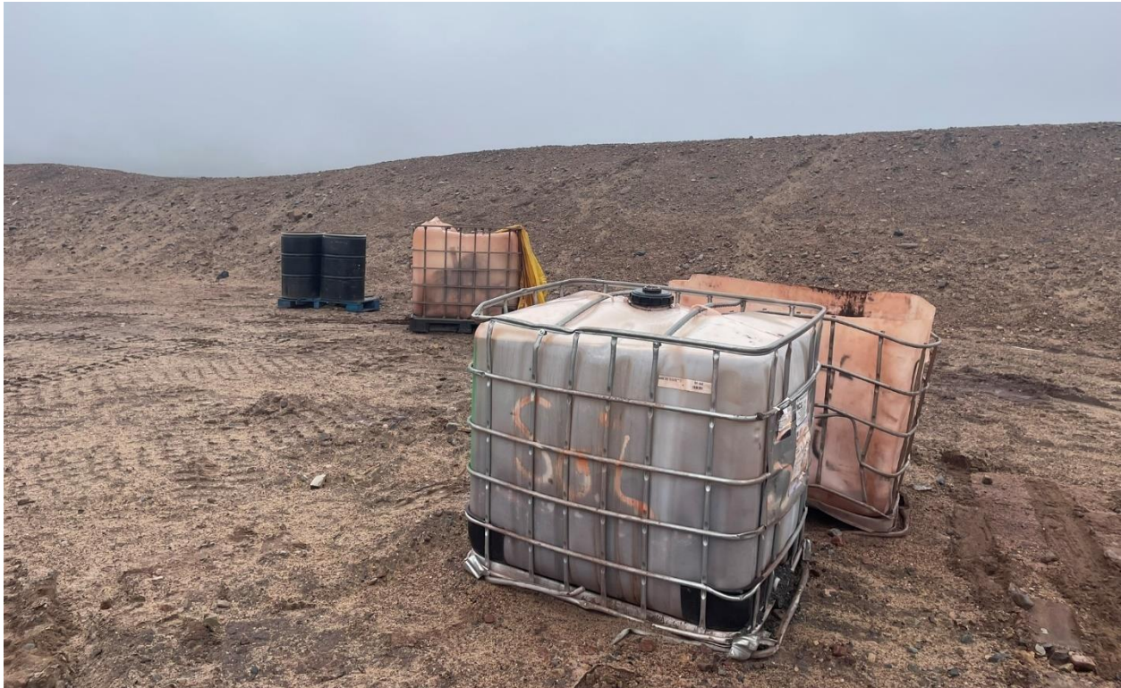
Photo 27: Uncontained Hazardous Material at New Monitoring Well Site
