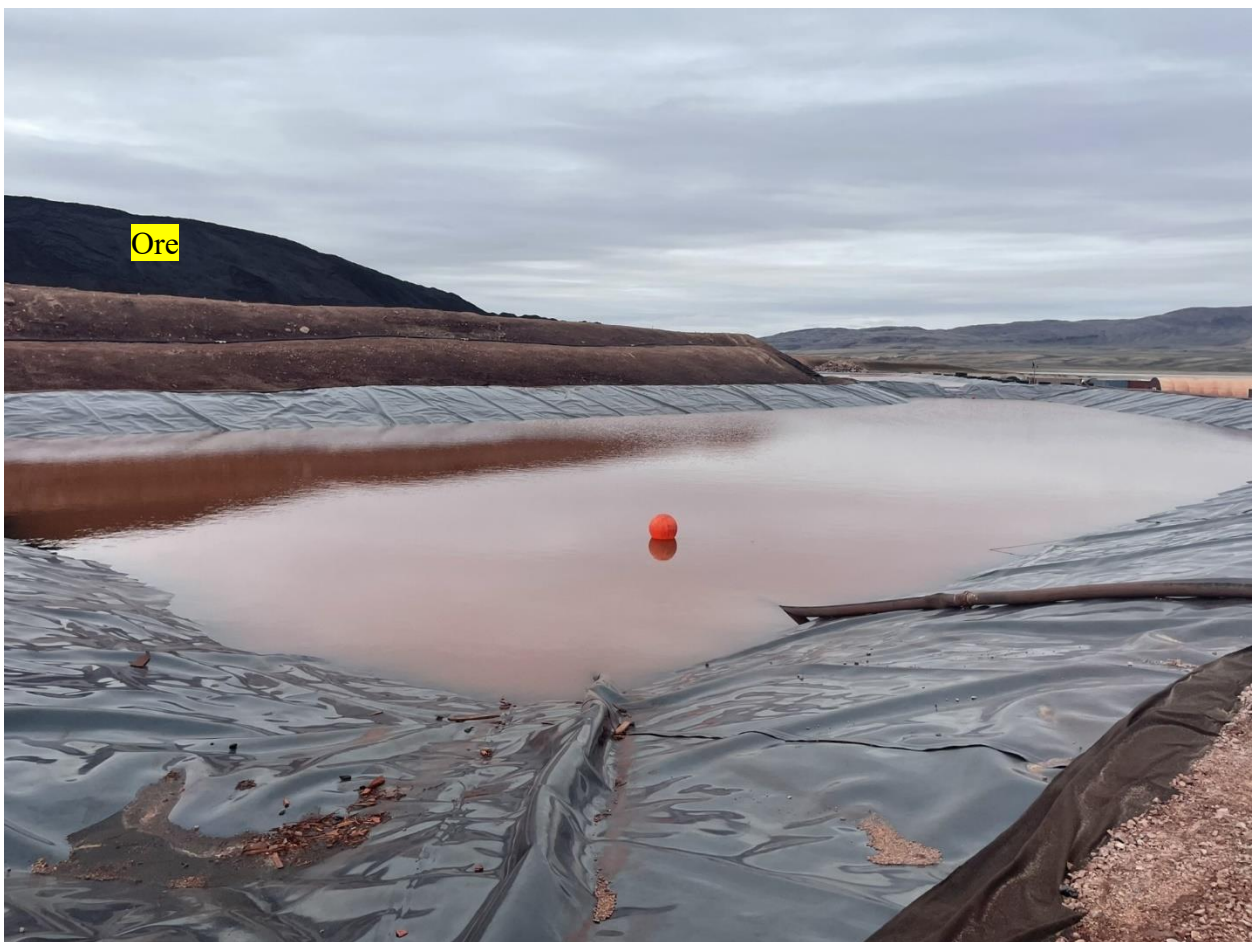
Photo 71: Ore Stockpile Sedimentation Pond West
