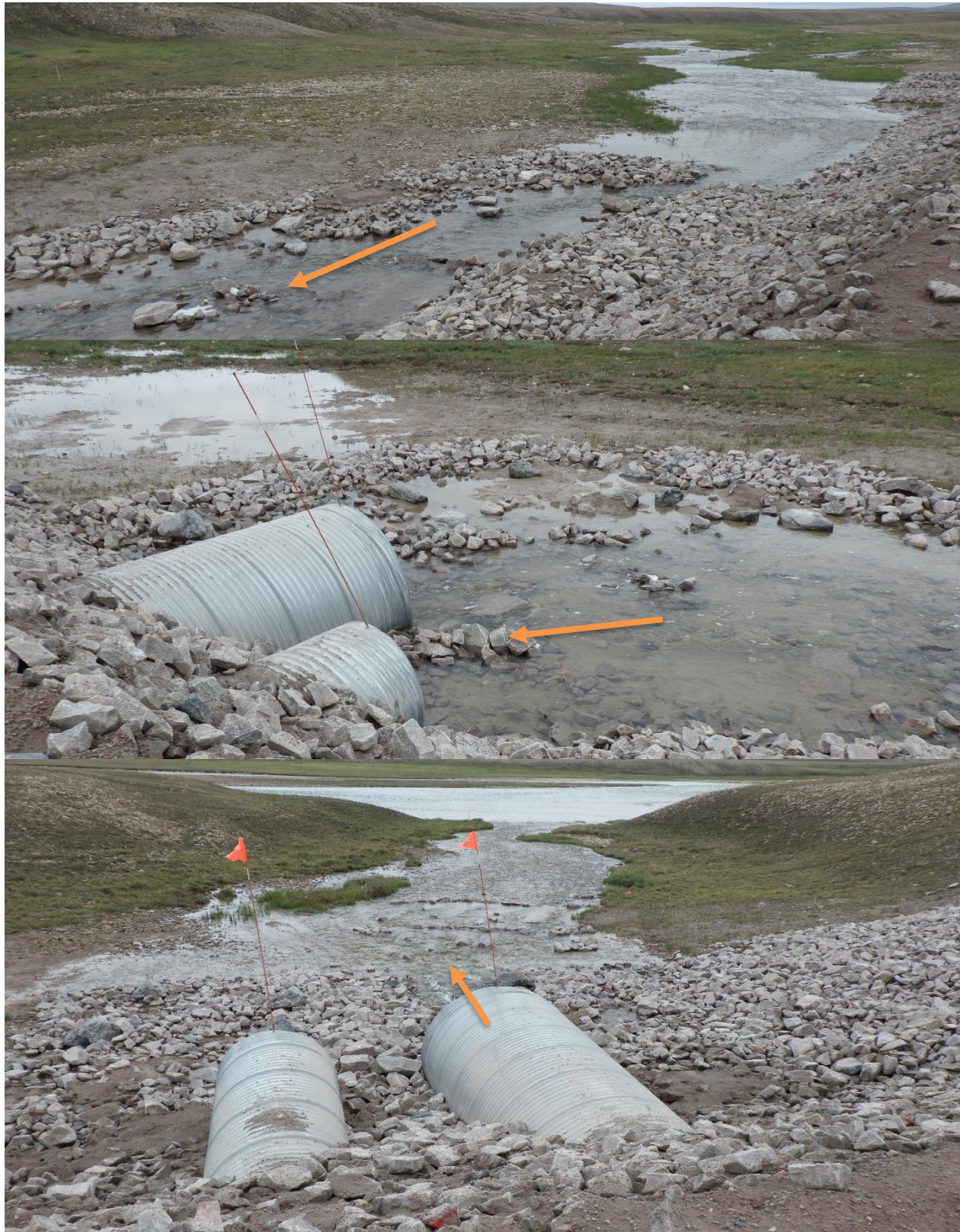
Photo 58: Culverts at KM 36 in good condition
