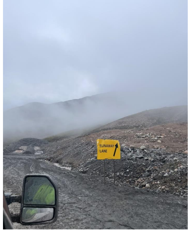
Photo 15: Runaway Lane on the Haul Road
