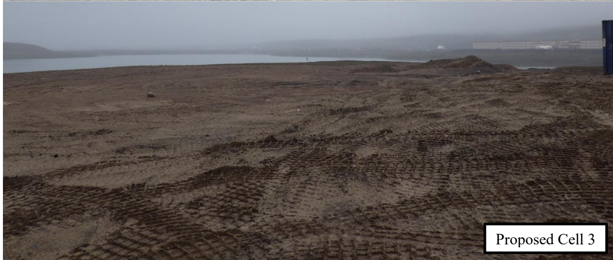
Photo 31: New landfarm cells constructed near the main Landfill Facility
