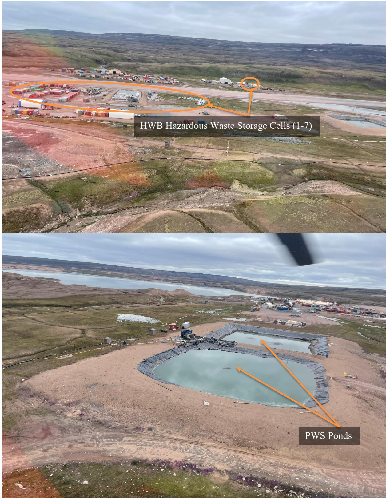
Photo 35: Aerial View of Mine Site Western Zone-Exploration Camp Polishing Waste Stabilization (PWS) Ponds, Hazardous Waste Berm (HWB) Storage Cells
