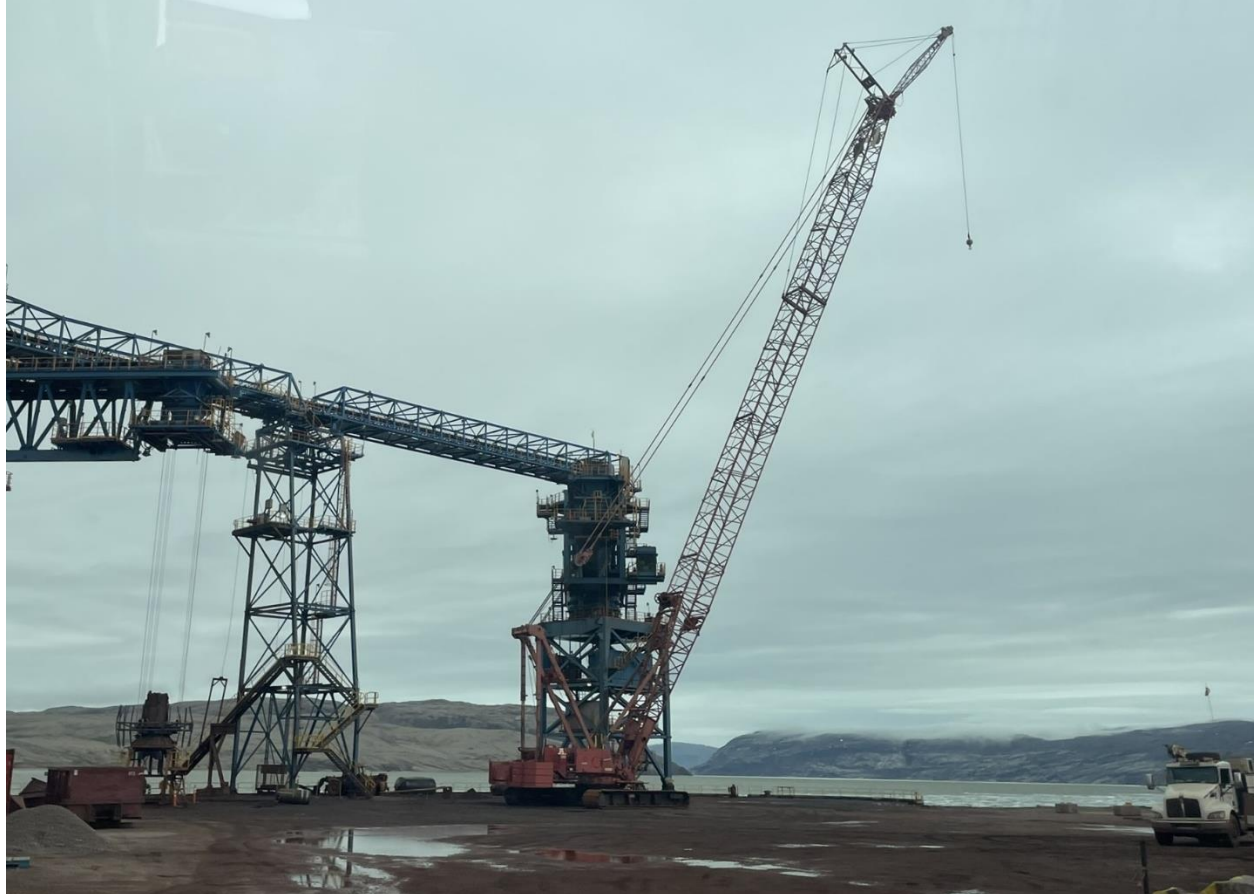
Photo 74: Ship Loader (One operational, second under construction)
