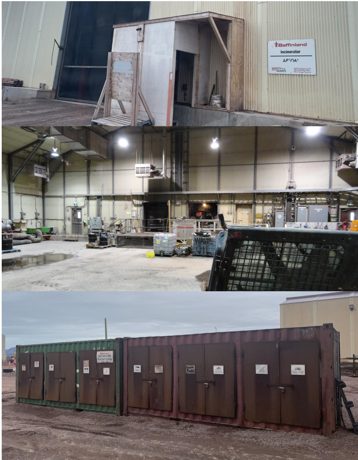
Photo 67: Incinerator Building and Hazardous Waste Storage outside Incinerator Building
