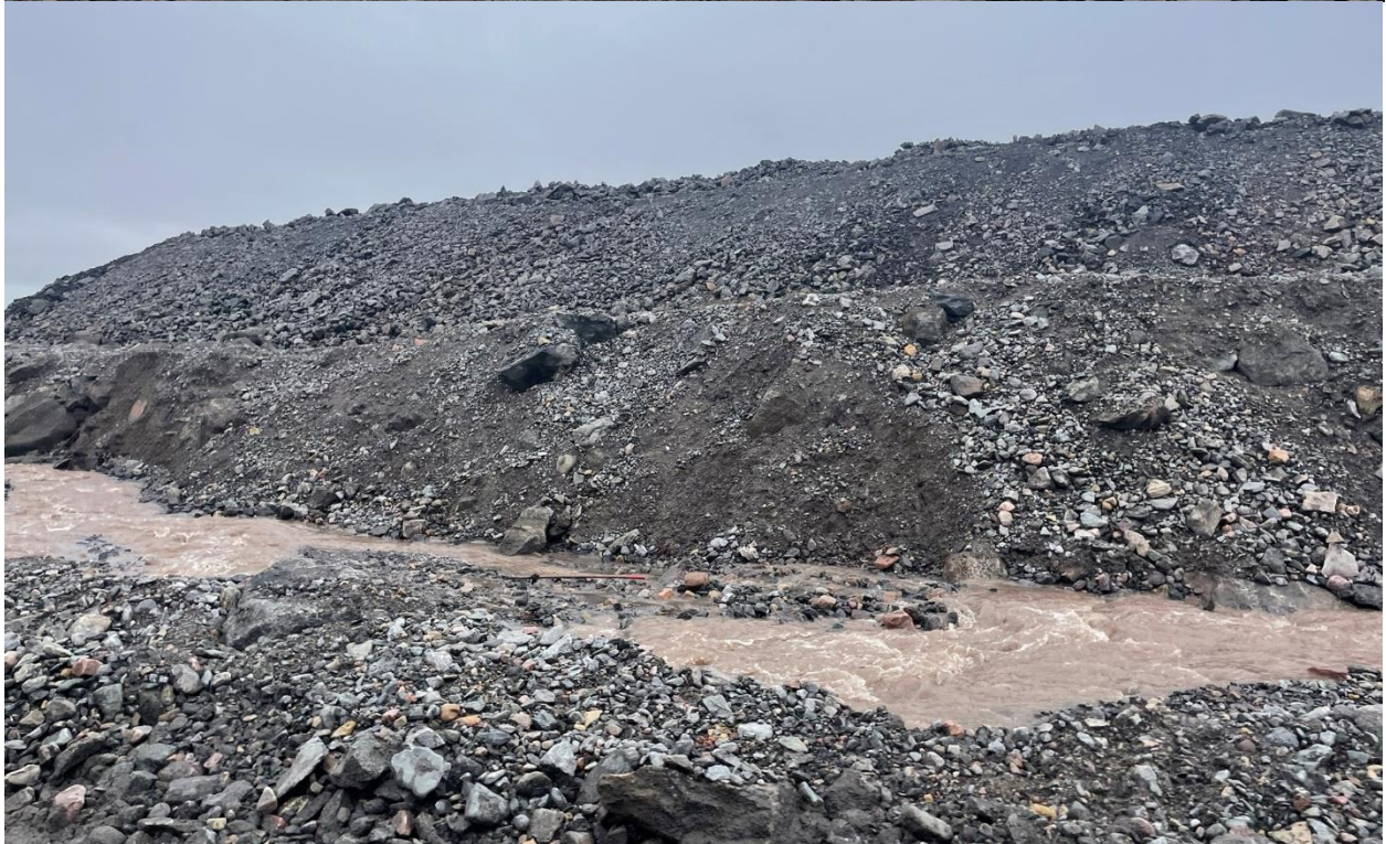
Photo 17: Drainage along the Haul Road
