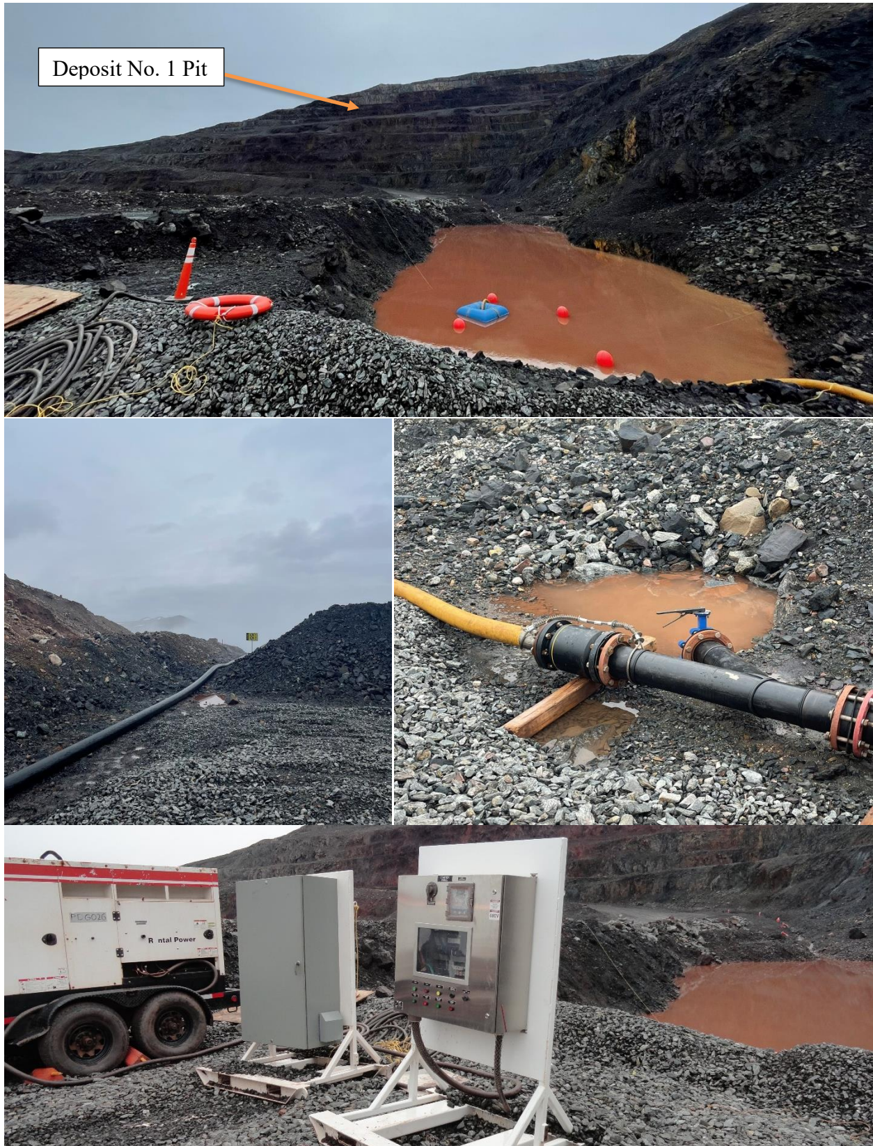
Photo 5: Pit Water Collection
