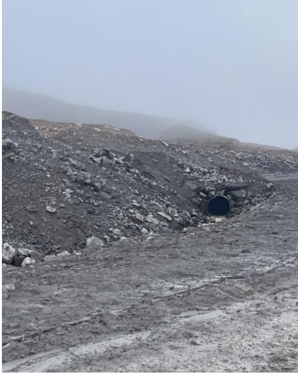
Photo 14: One (1) of the culverts along the Haul Road
