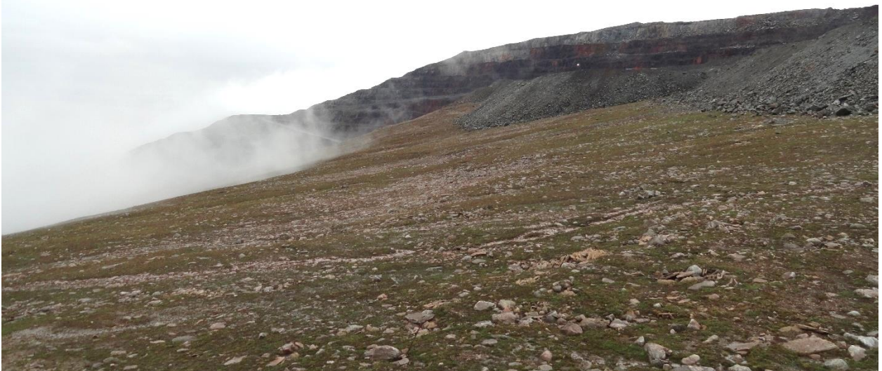
Photo 4: Westward View of Pit Benches for Deposit No. 1 from Communication Tower
