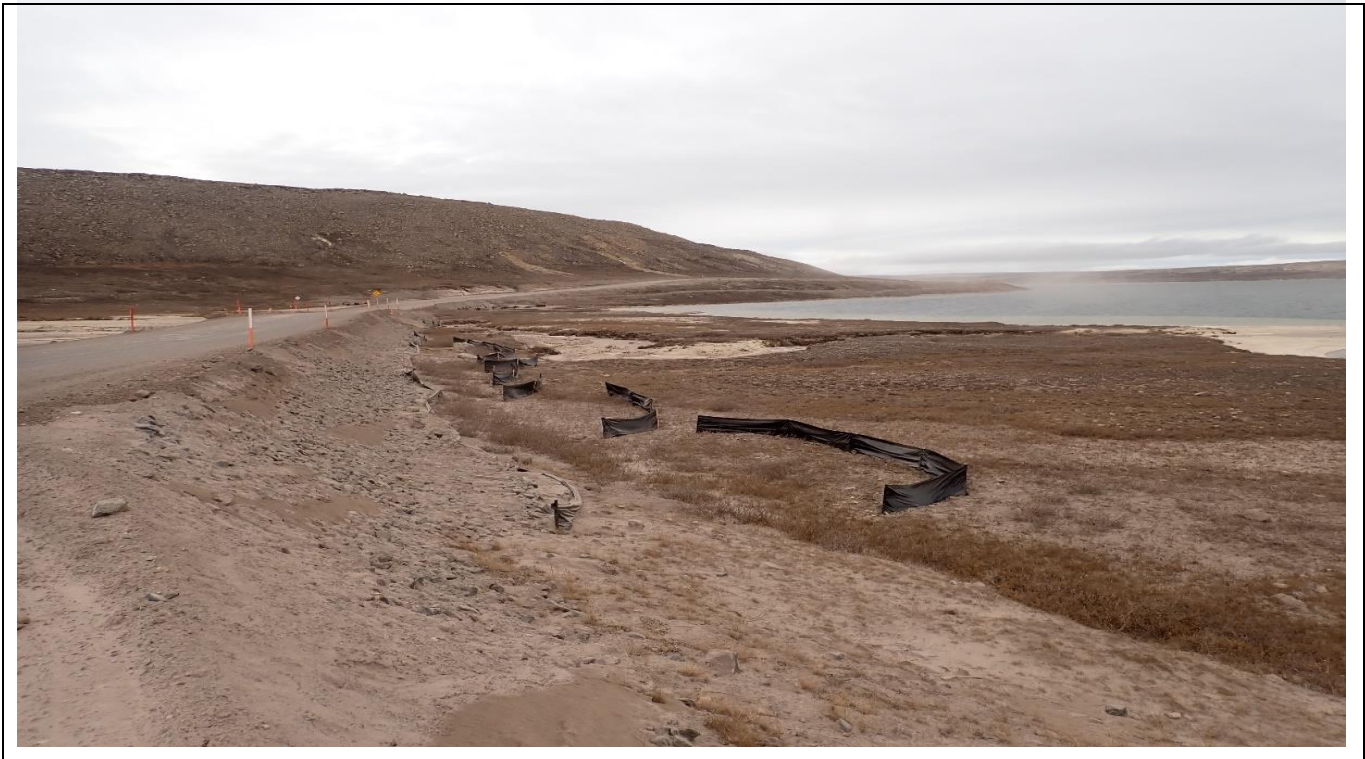
Photo 3. BG-24 (KM 87.5)- Follow up photo of new silt fences installed to mitigate erosion and sedimentation adjacent to the crossing.
