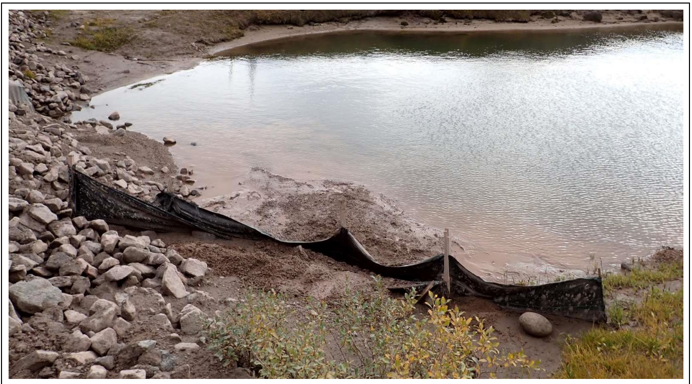
Photo 8. BG-30 (KM 85)- Re-secured and performed maintenance on silt fence
