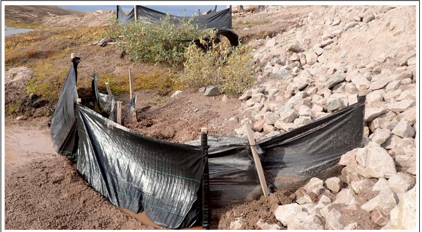
Photo 9. BG-30 (KM 85), Roadway bank erosion, additional silt fence installed upstream of culvert
