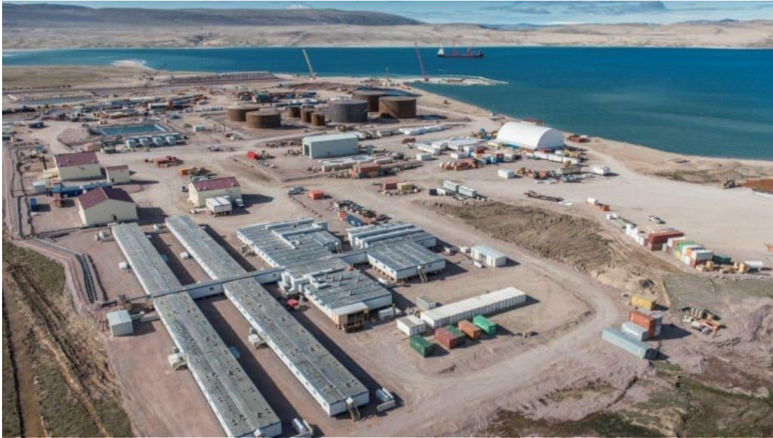
Baffinland Iron Mines Camp at Milne Inlet.
