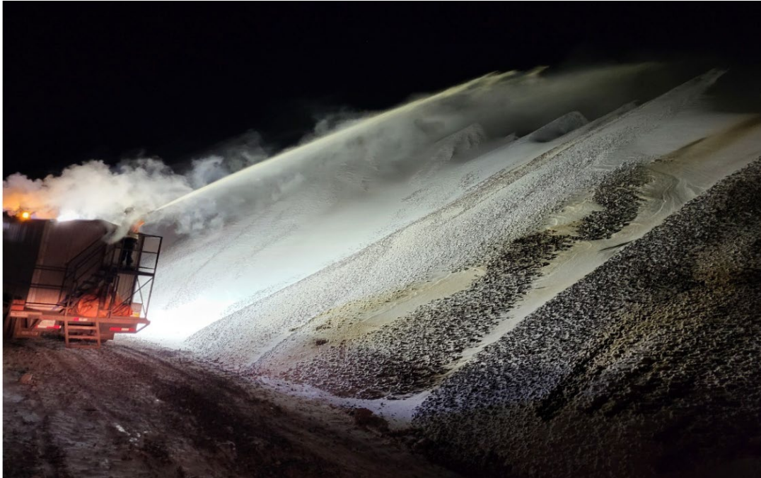
Photo 12: Dust Suppression at the Ore Pad Stockpile at Milne Port – January 2025
