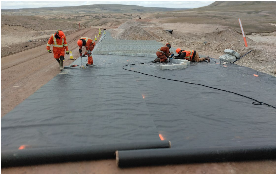
Photo 8: Installation of Geo Cell at KM 64 – July 2025
