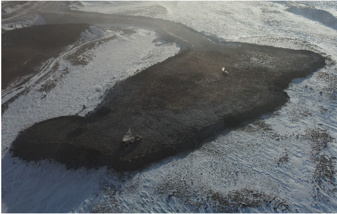
Photo 7: KM 105 Steensby Aggregate Pad Construction – April 2025
