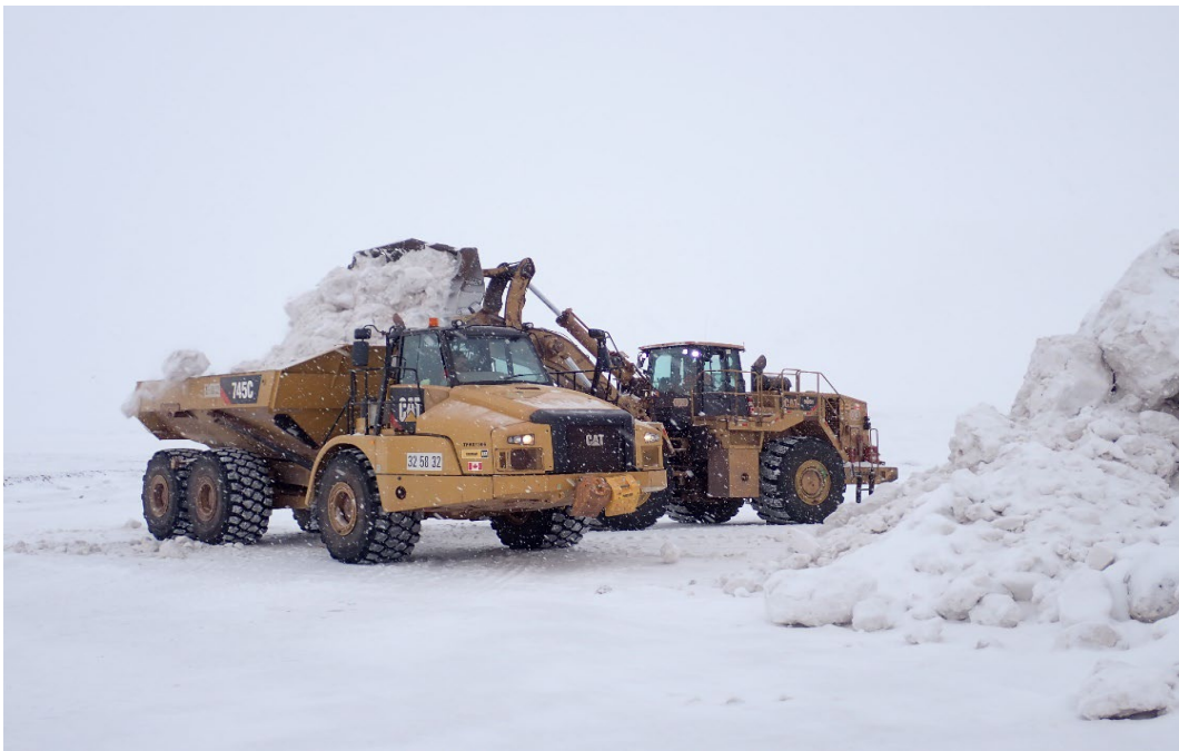
Photo 14: Snow Clearing for Freshet Preparation – April 2025
