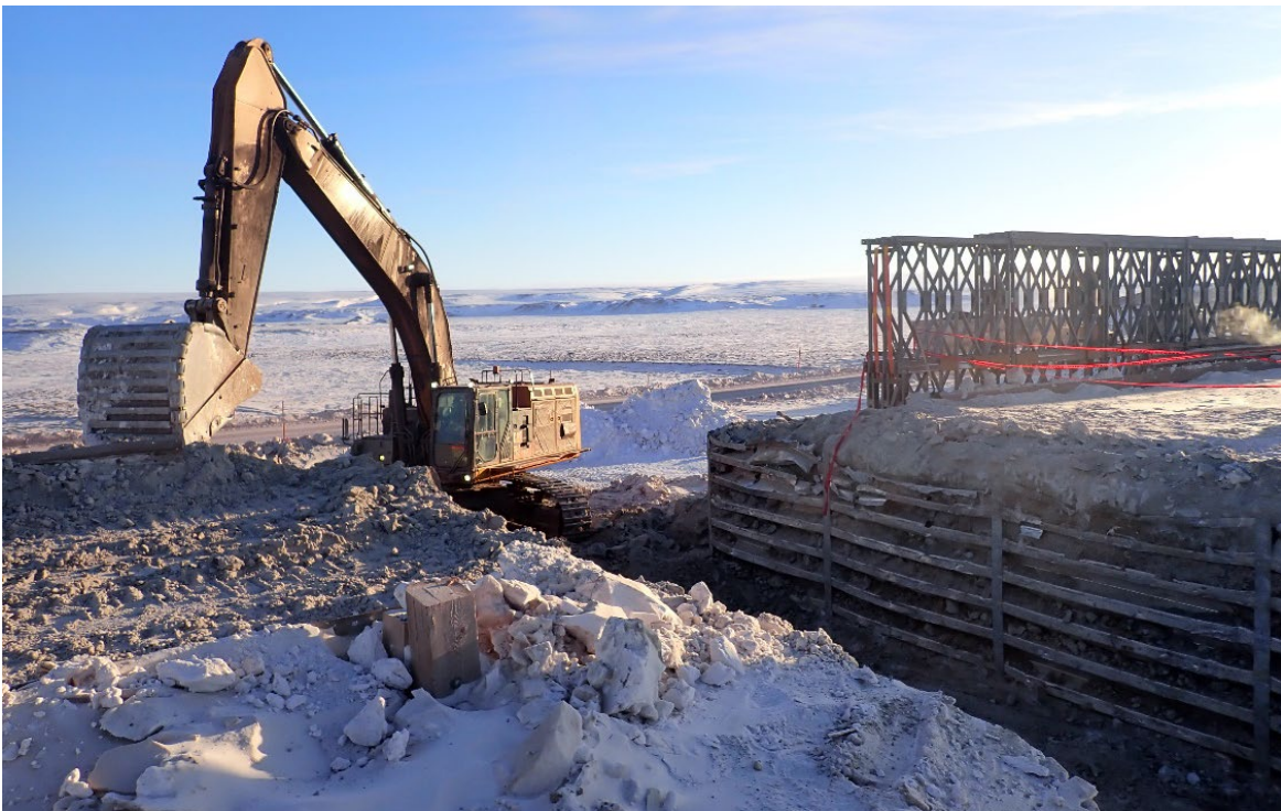
Photo 6: Removal of Southern Abutment of KM 97 Bridge – March 2025
