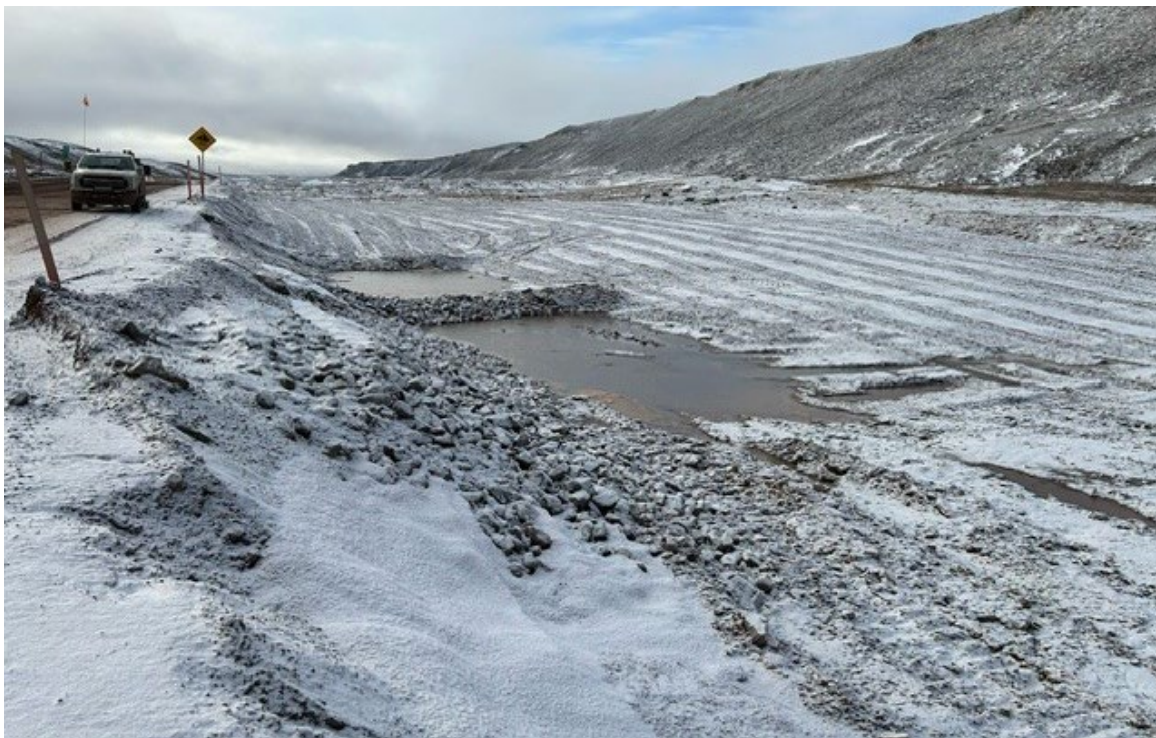
Photo 9: Borrow Pit 14A Remediation at KM 89 - September 2025
