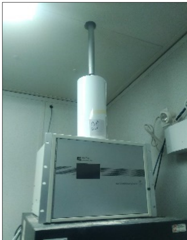
Photo 3.1-5 TSP BAM 1020 analyzer at the Port Site Complex ambient air quality station.
