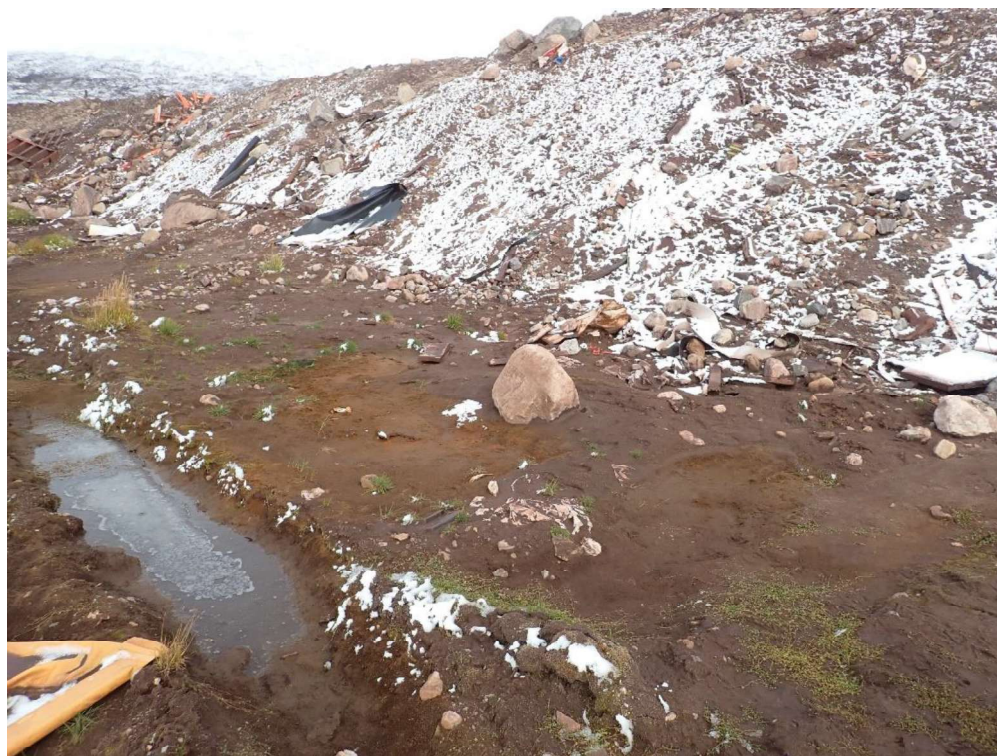
Photo A-40: Seep LF-DS-SEEP-02 (August 29, 2025) – Seep was dry. Some stagnant water observed 4 metres from the 2024 seep location.
