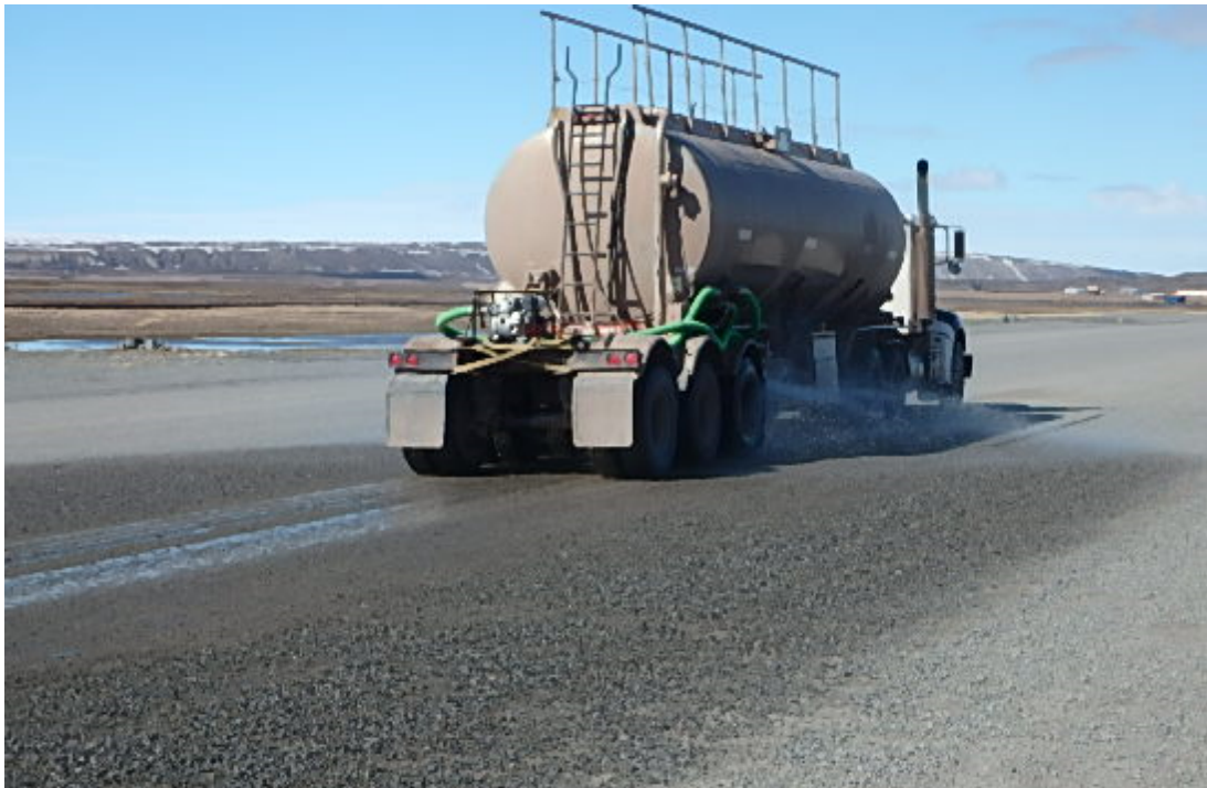
Figure 8 Application of water along the airstrip (provided by Baffinland, October 2025).
