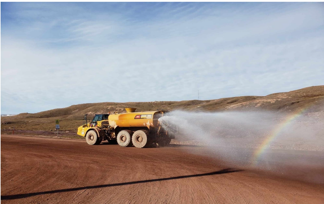
Figure 6 Application of water along the Tote Road to re-activate calcium chloride (provided by Baffinland, December 2025).
