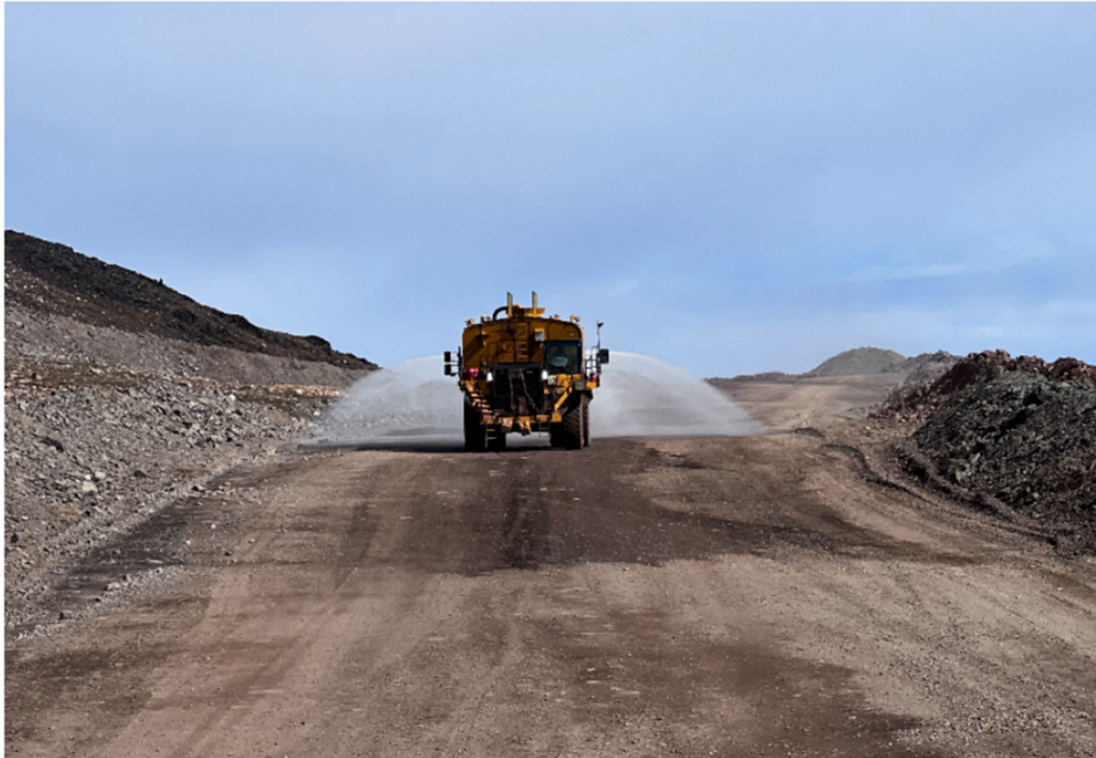
Figure 6 Application of water along the Tote Road to re-activate calcium chloride (provided by Baffinland, December 2025).
