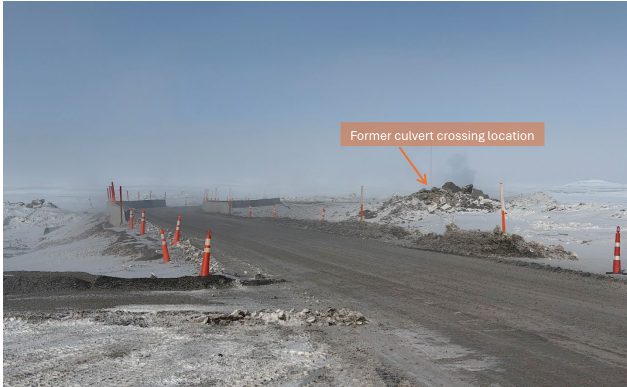
Photo 69: Newly constructed by-pass Road at KM 80 following culvert collapse in 2025
