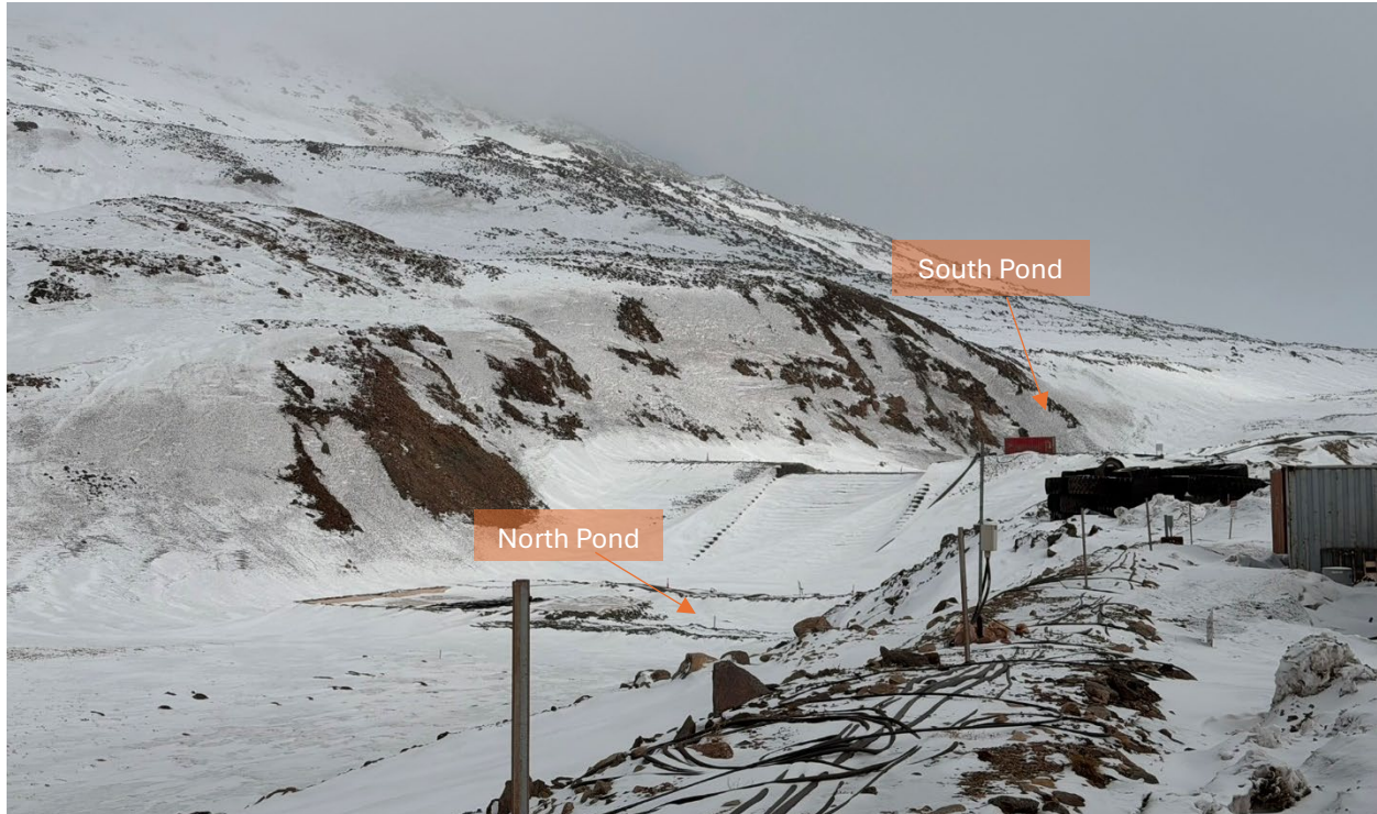
Photo 6: General overview of KM 105 Dam facing East
