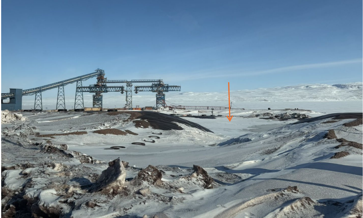
Photo 85: Ore stockpile sedimentation pond (North), frozen and snow covered, used for runoff treatment from the ore stockpile
