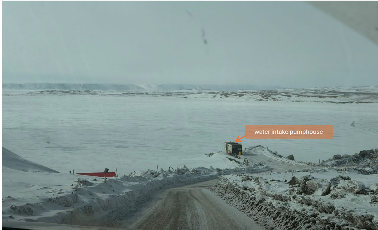
Photo 42: Camp Lake and water intake pumphouse, facing west
