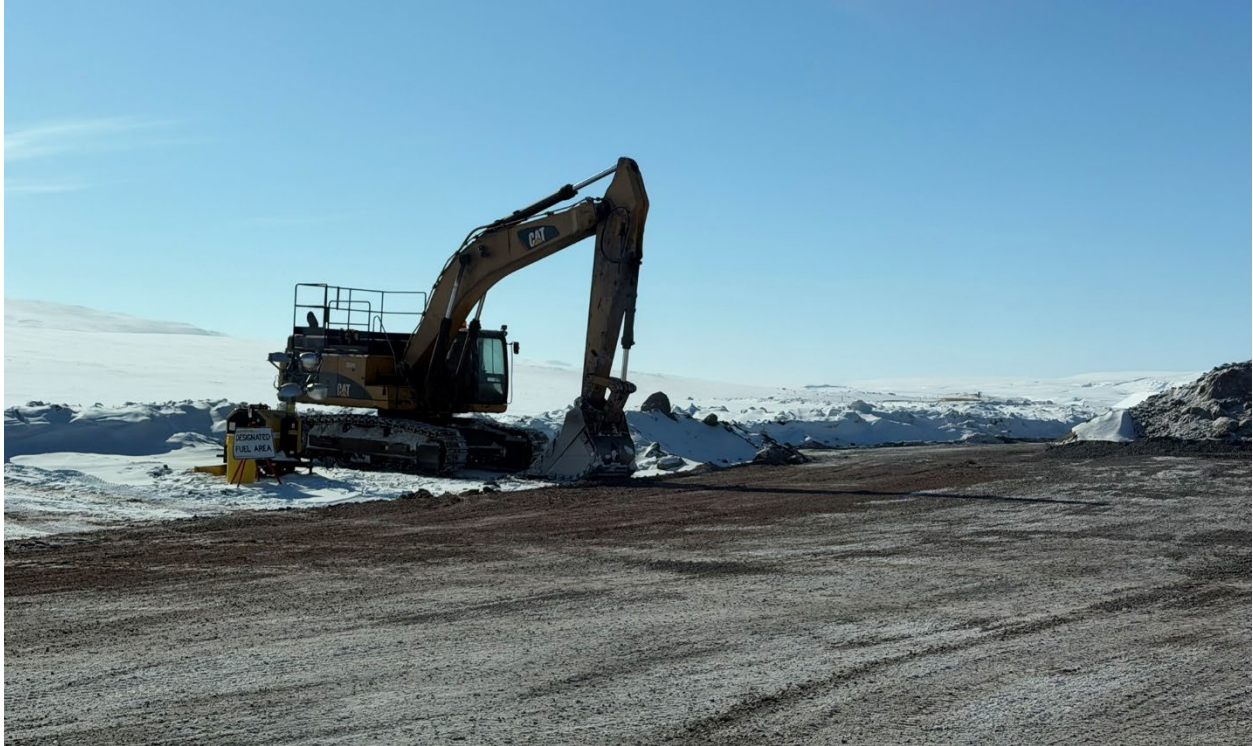
Photo 57: Designated fuel storage area with spill kit accessible nearby
