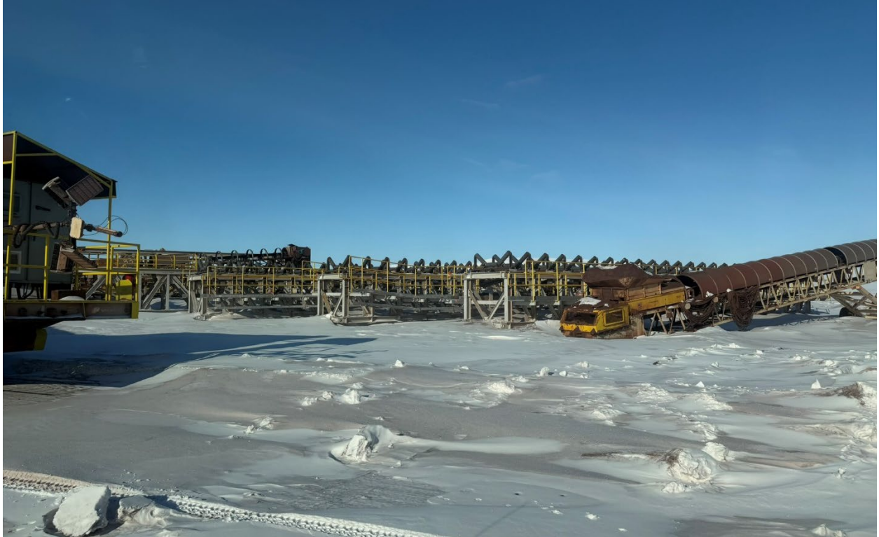
Photo 101: Phase 2 laydown area
