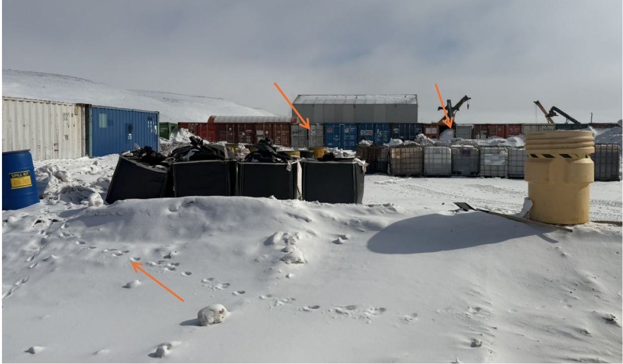
Photo 28: Hazardous waste berm with visible wildlife snow tracks; unsecured sea cans in background
