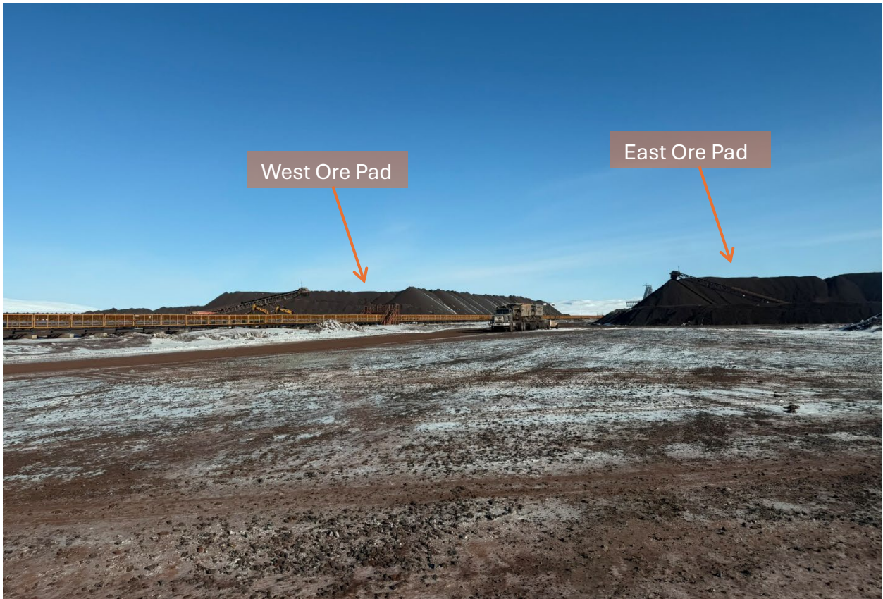
Photo 82: Distant view of Ore Pad
