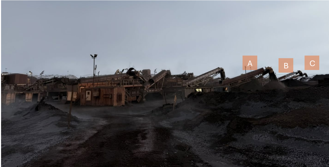
Photo 14: General overview of Crushers A, B, and C, facing south
