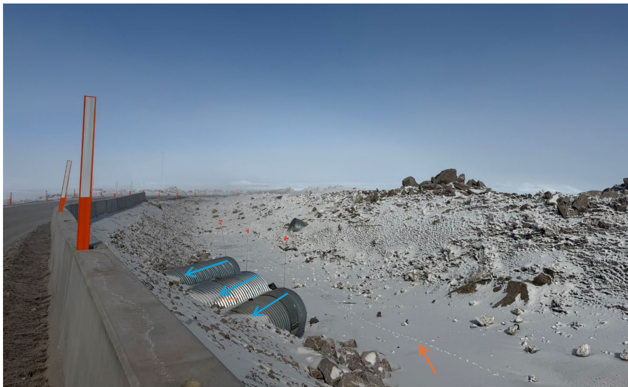
Photo 70: Newly installed three (3) culverts at KM 80
