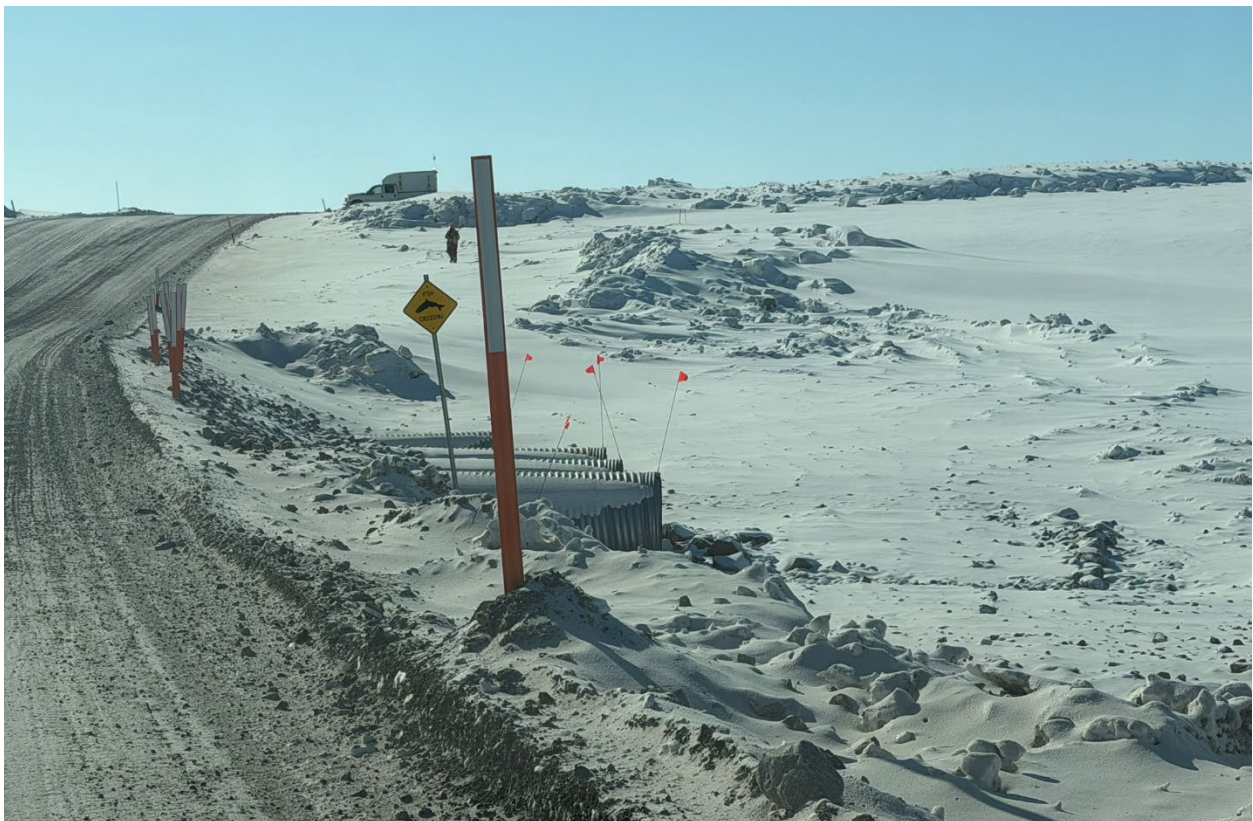
Photo 62: Fish passage culverts at KM 51
