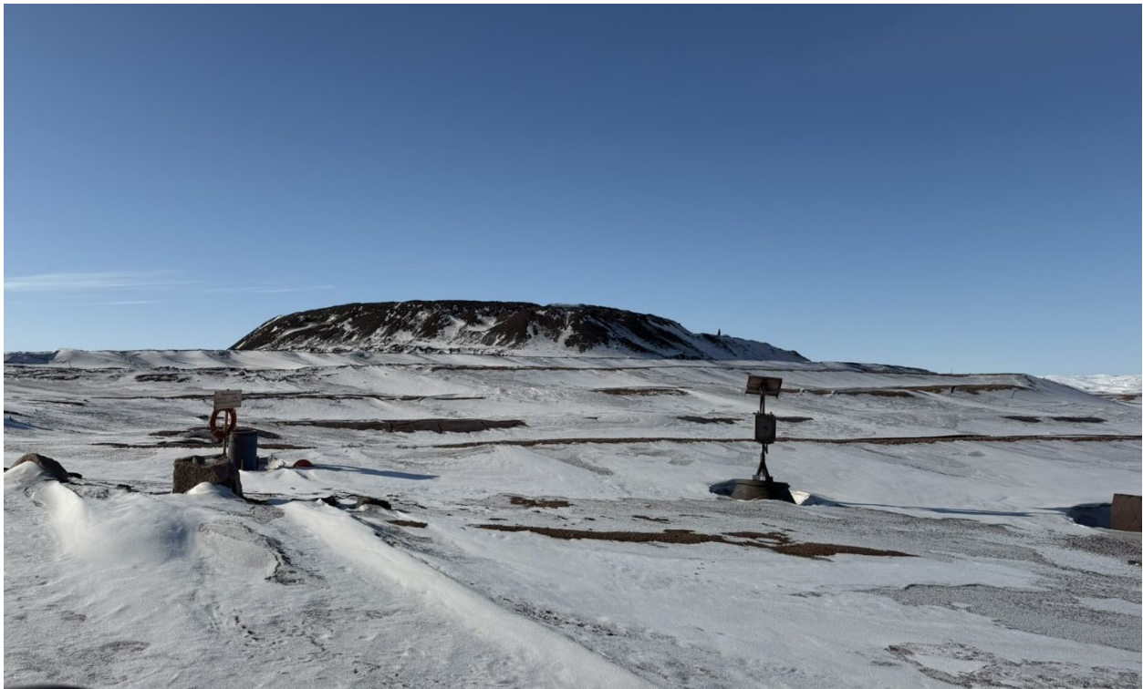
Photo 86: Ore stockpile sedimentation pond (East), frozen and snow covered, used for runoff treatment from the ore stockpile
