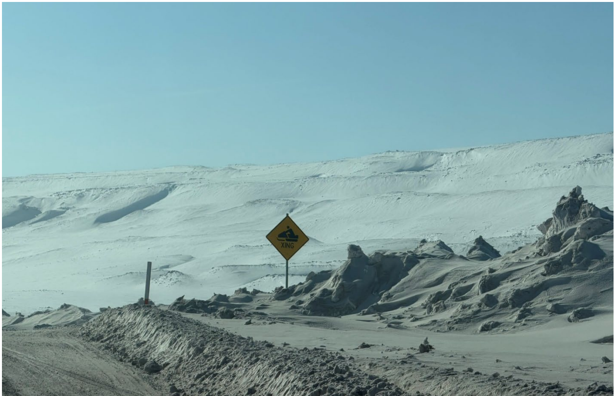
Photo 52: Close-up view of the crossing signage and adjacent steep, uneven berms blocking safe entry
