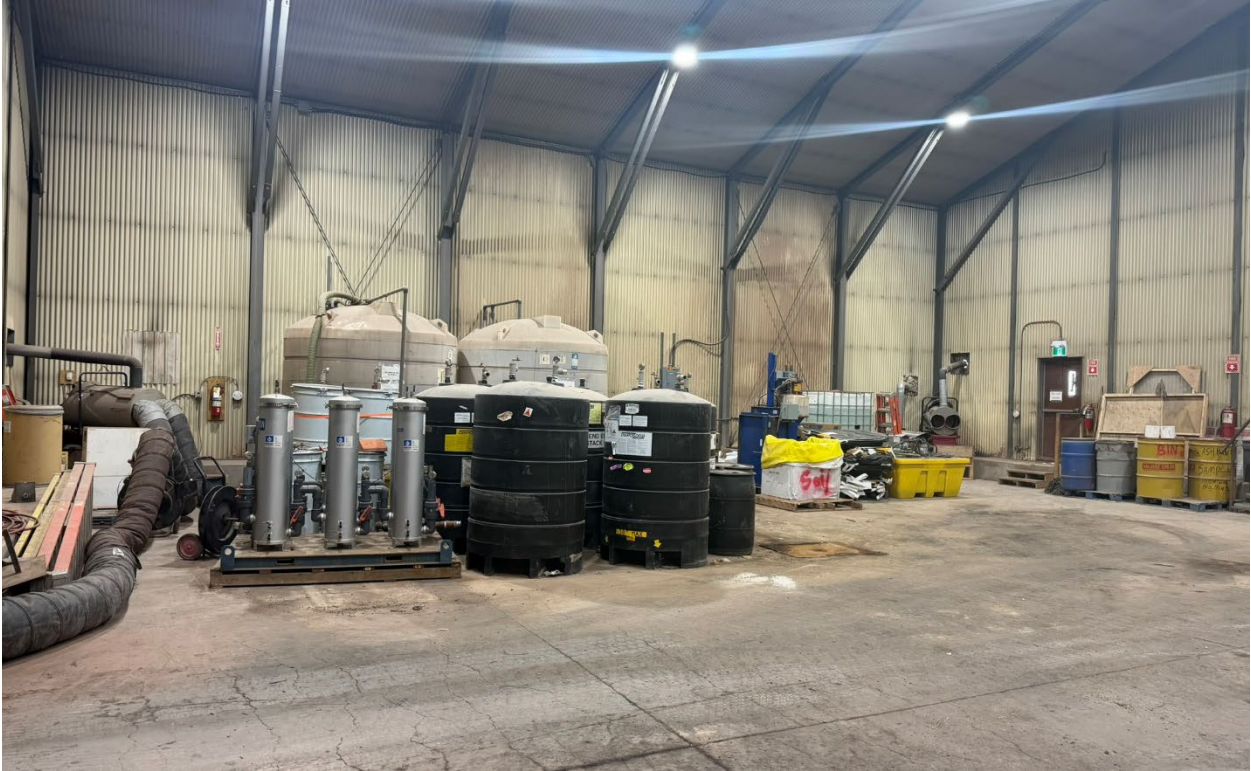
Photo 26: Incinerator building interior: well organized, with spill kits readily accessible
