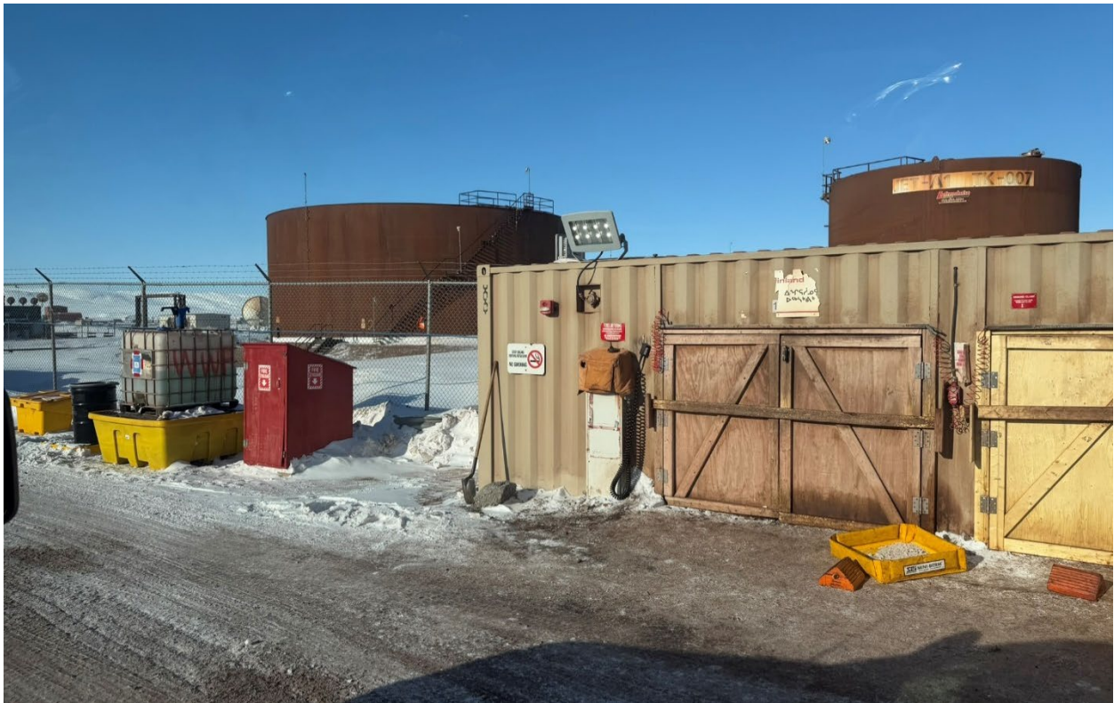
Photo 98: Vehicle fuel module and spill kits
