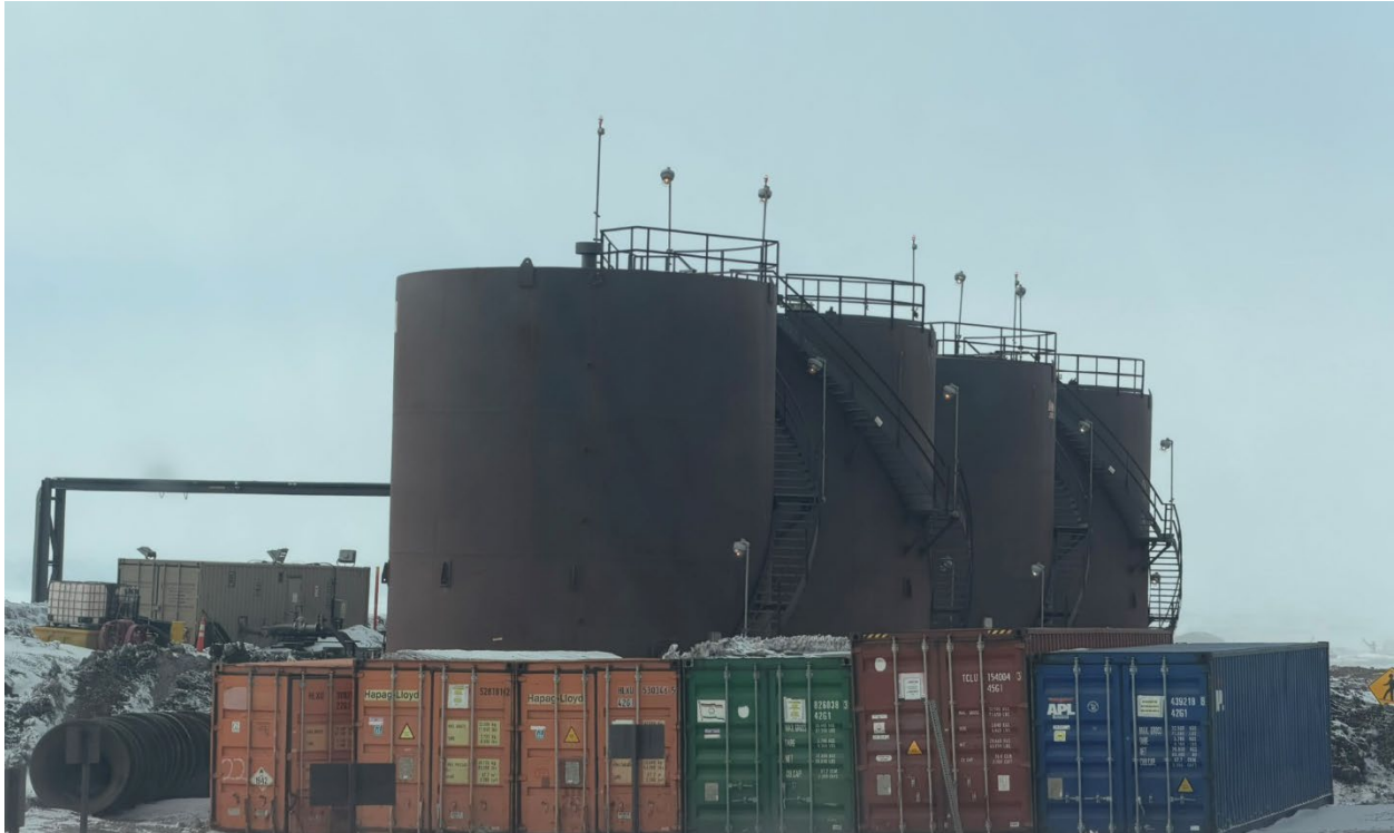
Photo 22: Mine site tank farm (MS-03)
