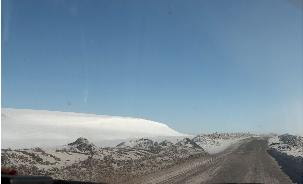
Photo 65: Dust conditions at KM 70, showing localized deposition
