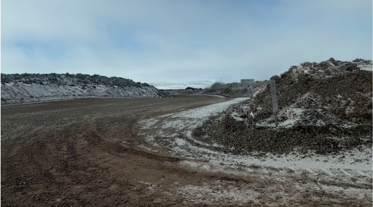
Photo 10: Haul Road, facing west at KM 105
