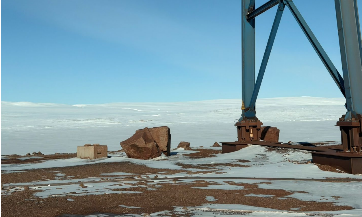
Photo 81: Base of the ore dock structure with sea ice conditions visible in the background
