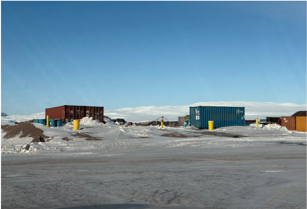
Photo 94: Hazardous Waste Berm located northeast of fuel tank farm
