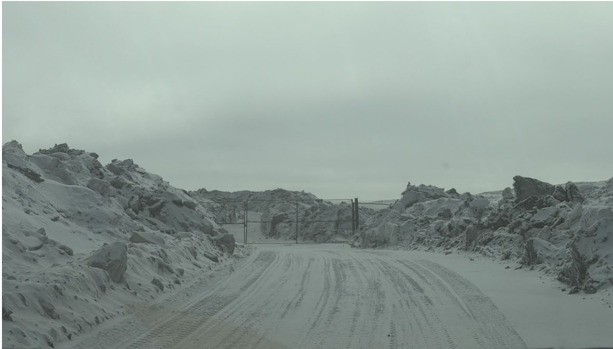
Photo 34: Fenced landfill with gated access
