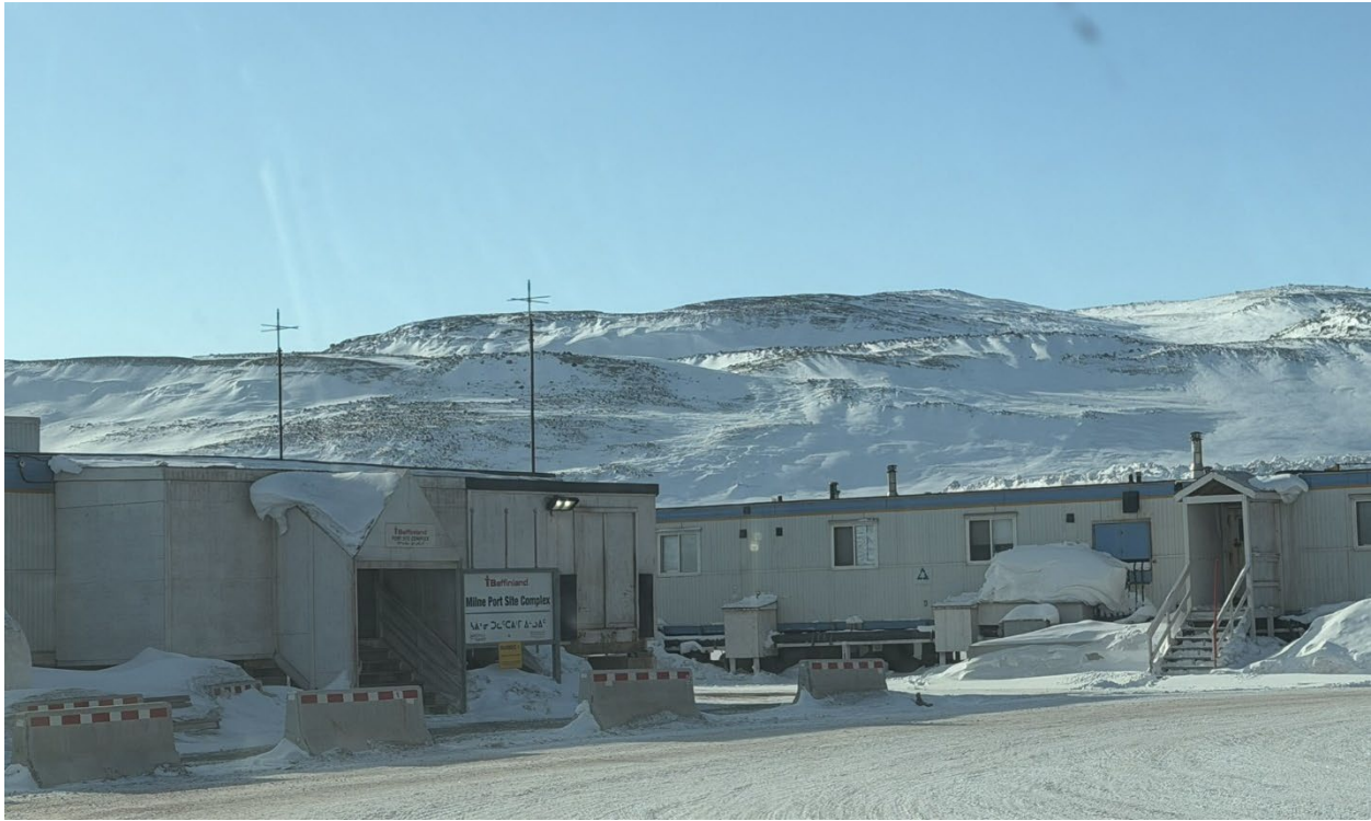
Photo 103: Milne Port Site Complex entrance
