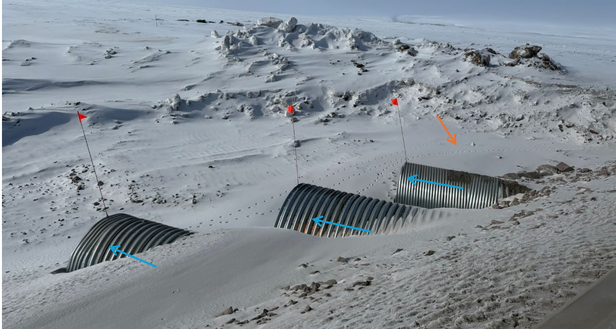
Photo 71: Newly installed three (3) culverts at KM 80
