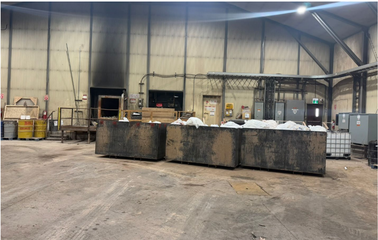
Photo 27: Incinerator building interior: well organized, with spill kits readily accessible
