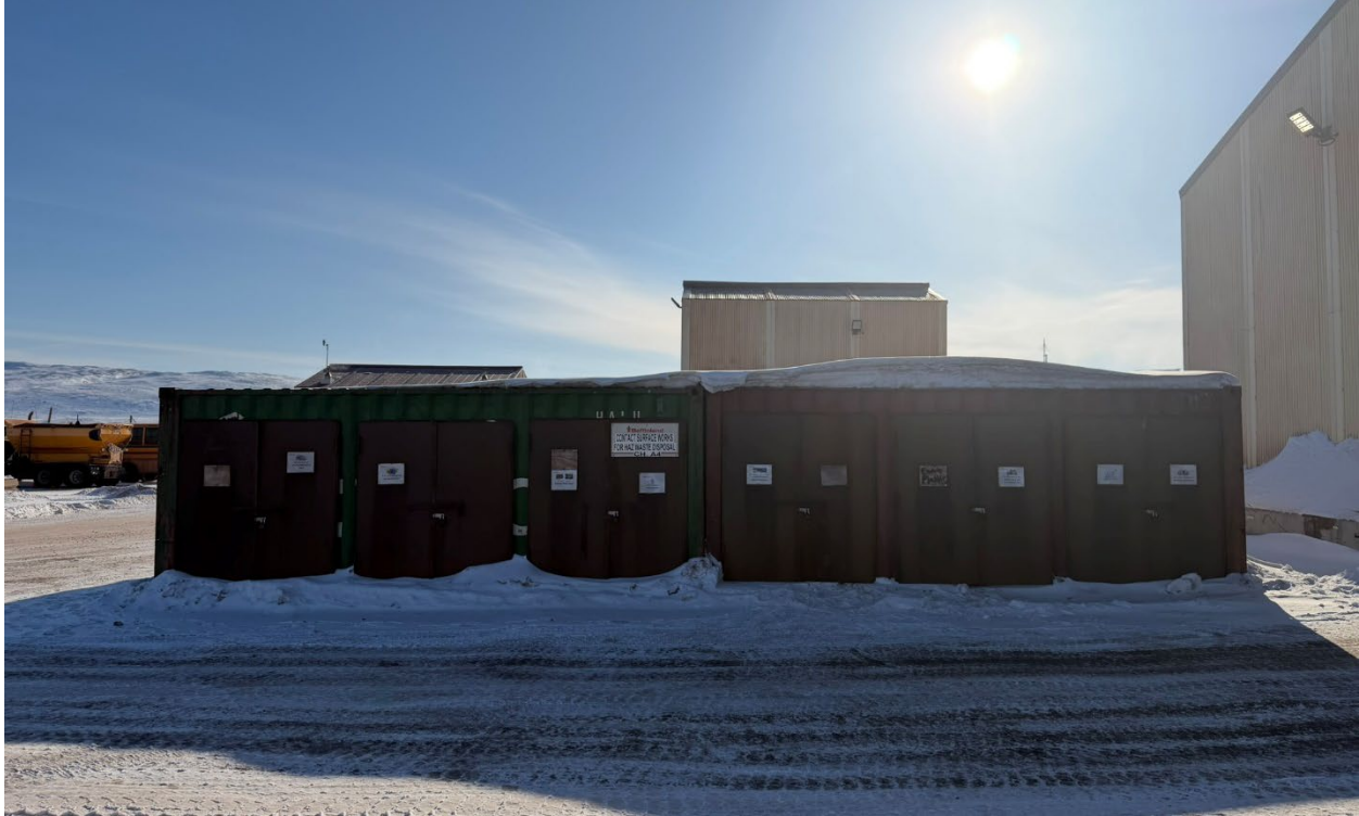
Photo 91: Secured HAZMAT storage units in front of incinerator building
