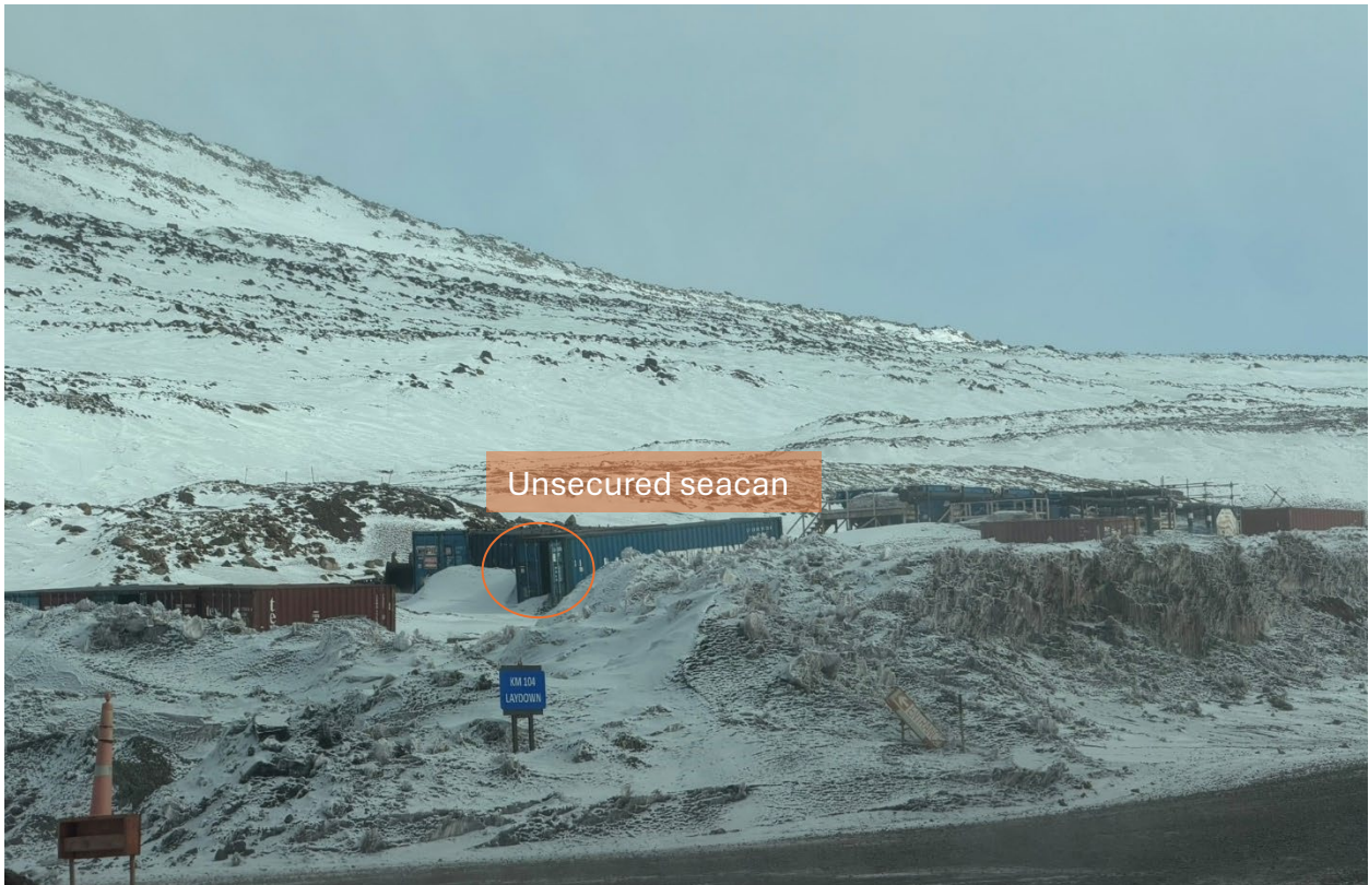
Photo 9: KM 104 Laydown, located west of KM 105 Dam
