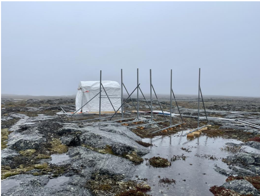
Figure 1. Setup of solar panel frame and started the installation of the white tent that will house the backup power and the “brains” of the equipment.
