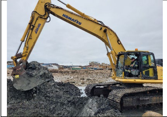
Photo 7: Geotechnical Test Pits
