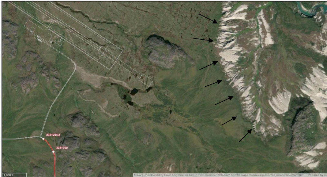
Figure 4.16 Gullies and landslides (indicated by the black arrows) in marine soils near the southern end of the aerodrome area (in white).
