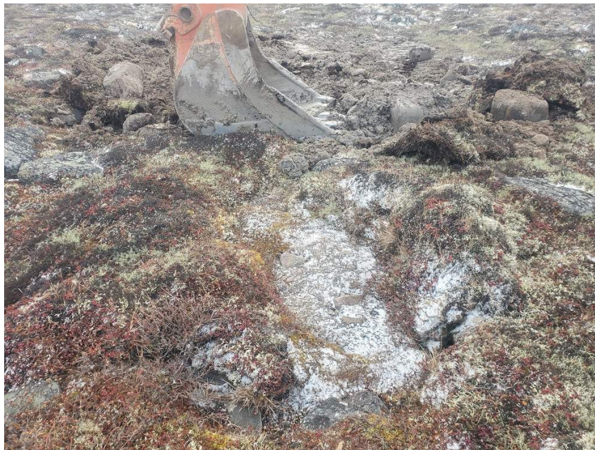
Photograph 20 - October 8, 2022 Backfilling TP-BS2-06.
