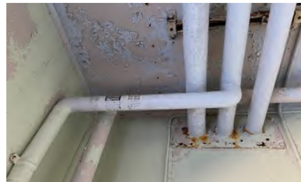
PCB painted walls and asbestos wrapped pipes.
