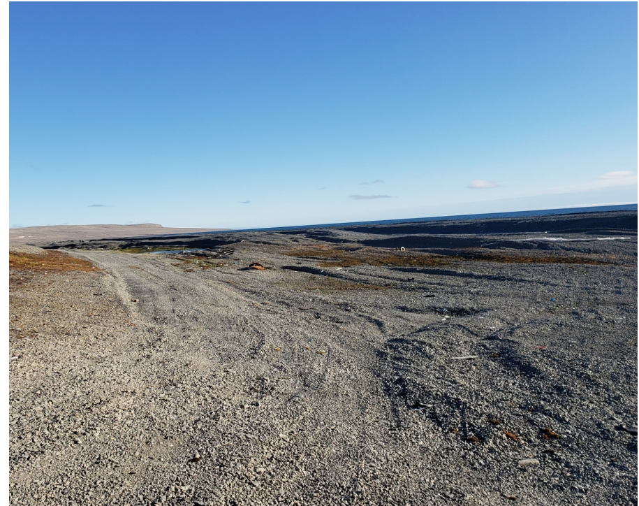
Inadequate ditching along access road
