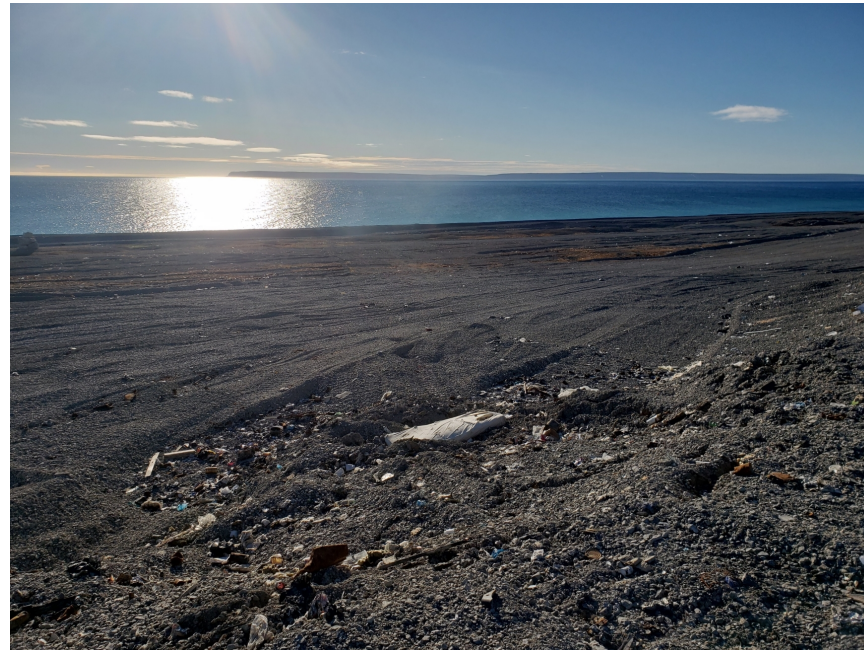
Municipal Waste Dump and Burning Site – no fencing
