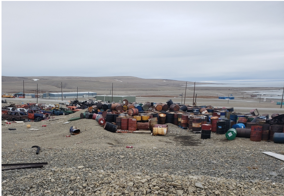
No containment of waste oil barrels – staining visible
