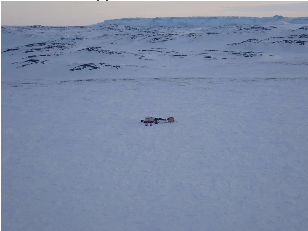
Photo 1. Drill set-up, prior to the start of drilling at the Proposed port site
