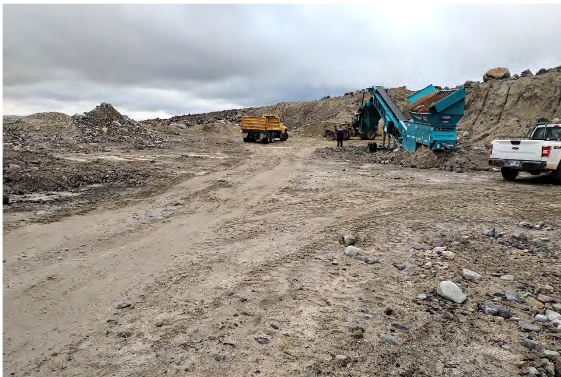
Photo 13: Site 5 Hamlet Borrow Pit- Water Plant Road Screening plant only with loader and truck- 6m Banks- in operation
