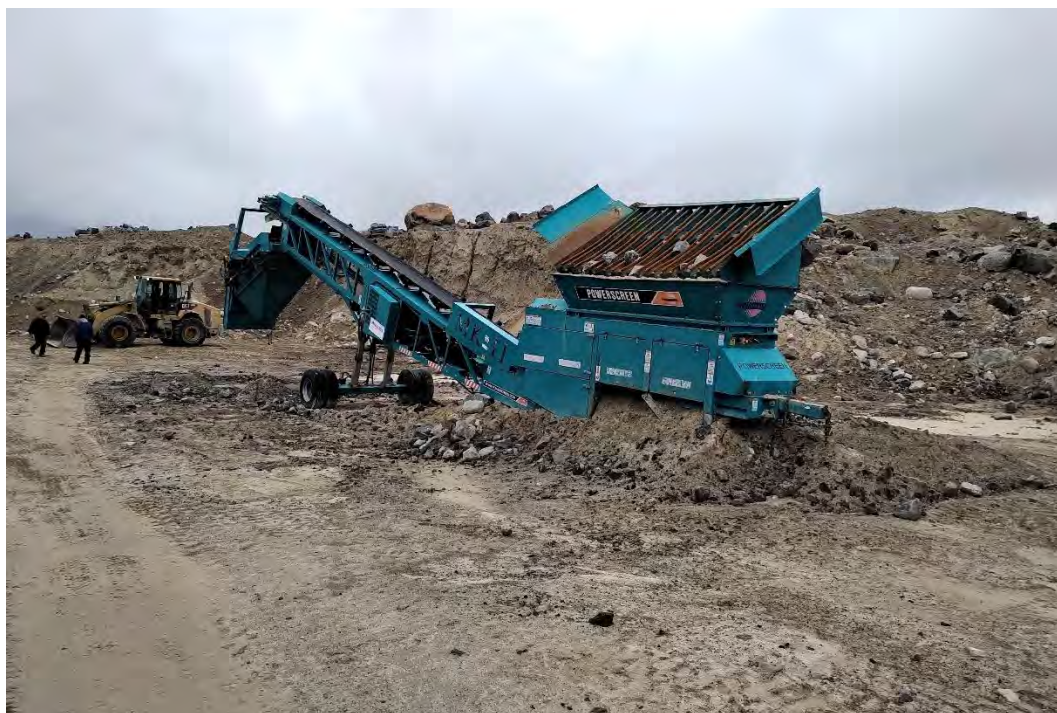
Photo 14: Site 5 Hamlet Borrow Pit- Water Plant Road -Screening Plant and Loader
