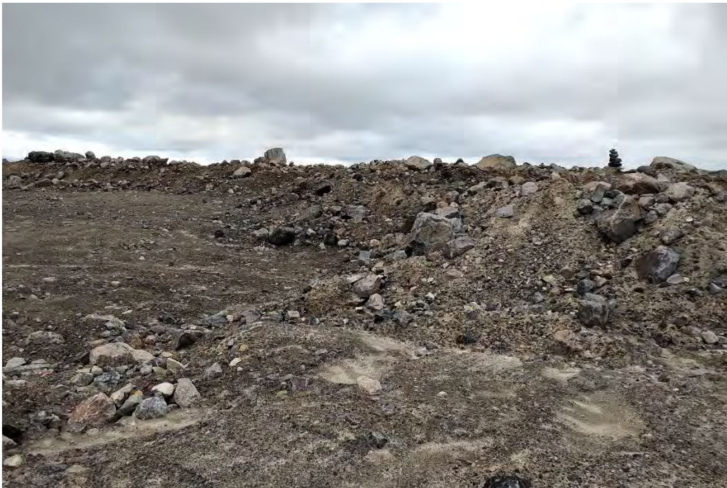
Photo 17: Site 6 Clay Pit – East of Hamlet Borrow Pit – Area on top of Borrow Pit Stripped to Surface of Clay
