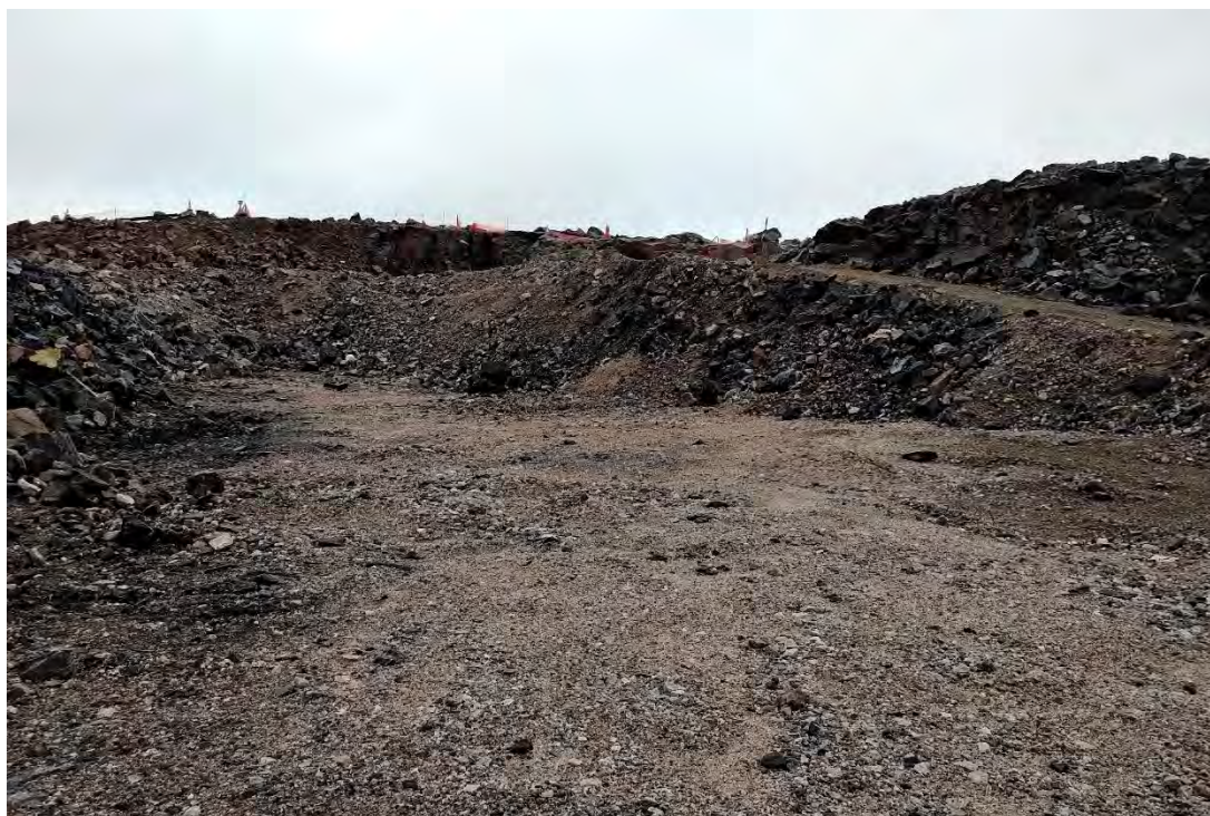
Photo 2: Site 1- Kudlik Quarry – Additional Blasted Rock Stockpiles for Crushing
