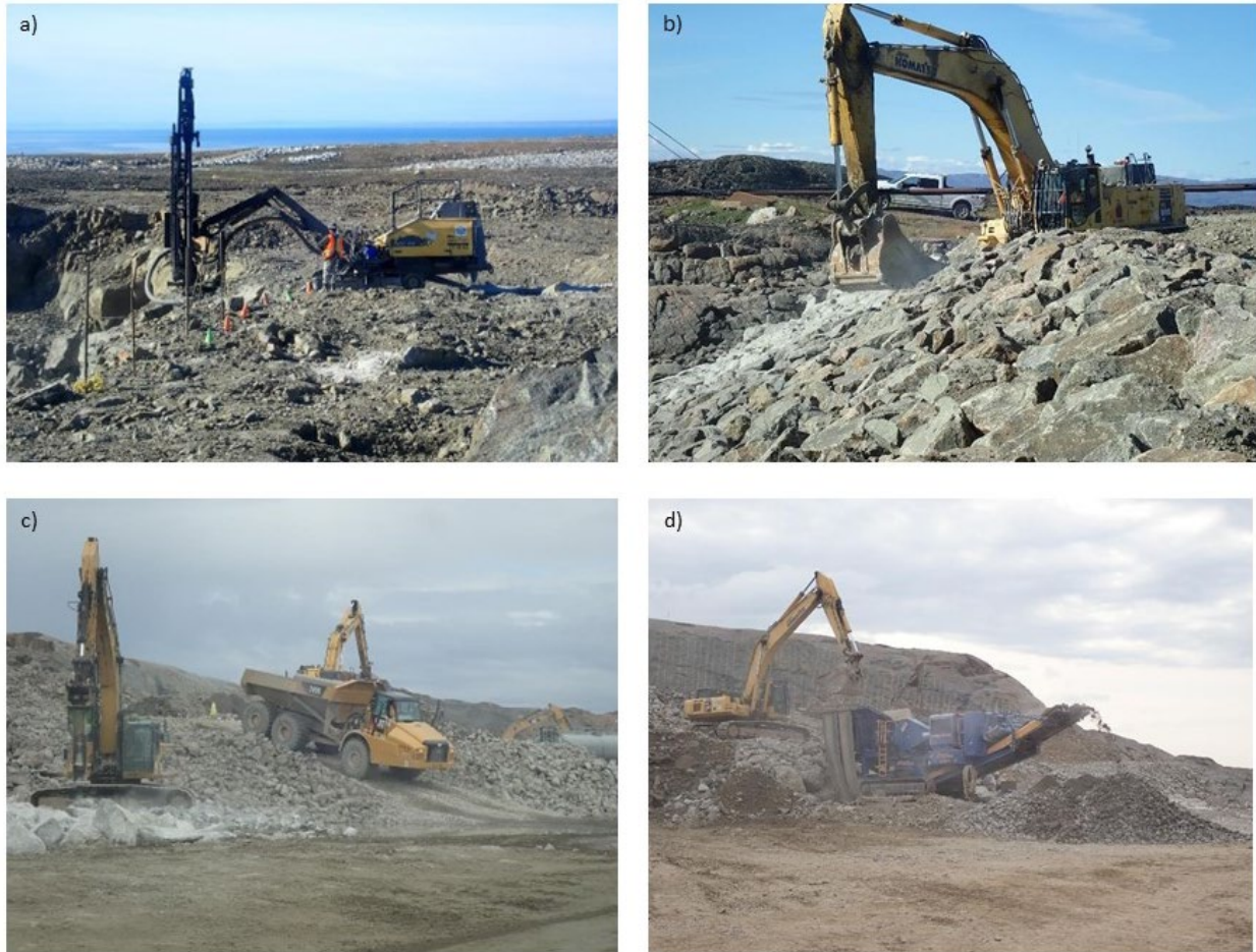
Photo 1-3: Representative Construction Equipment a) Drill Rig; b) Excavator; c) Rock Truck; d) Crusher
