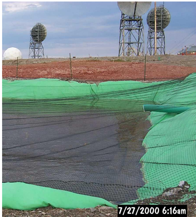
Lady Franklin DEW line contaminated water collection pond.
