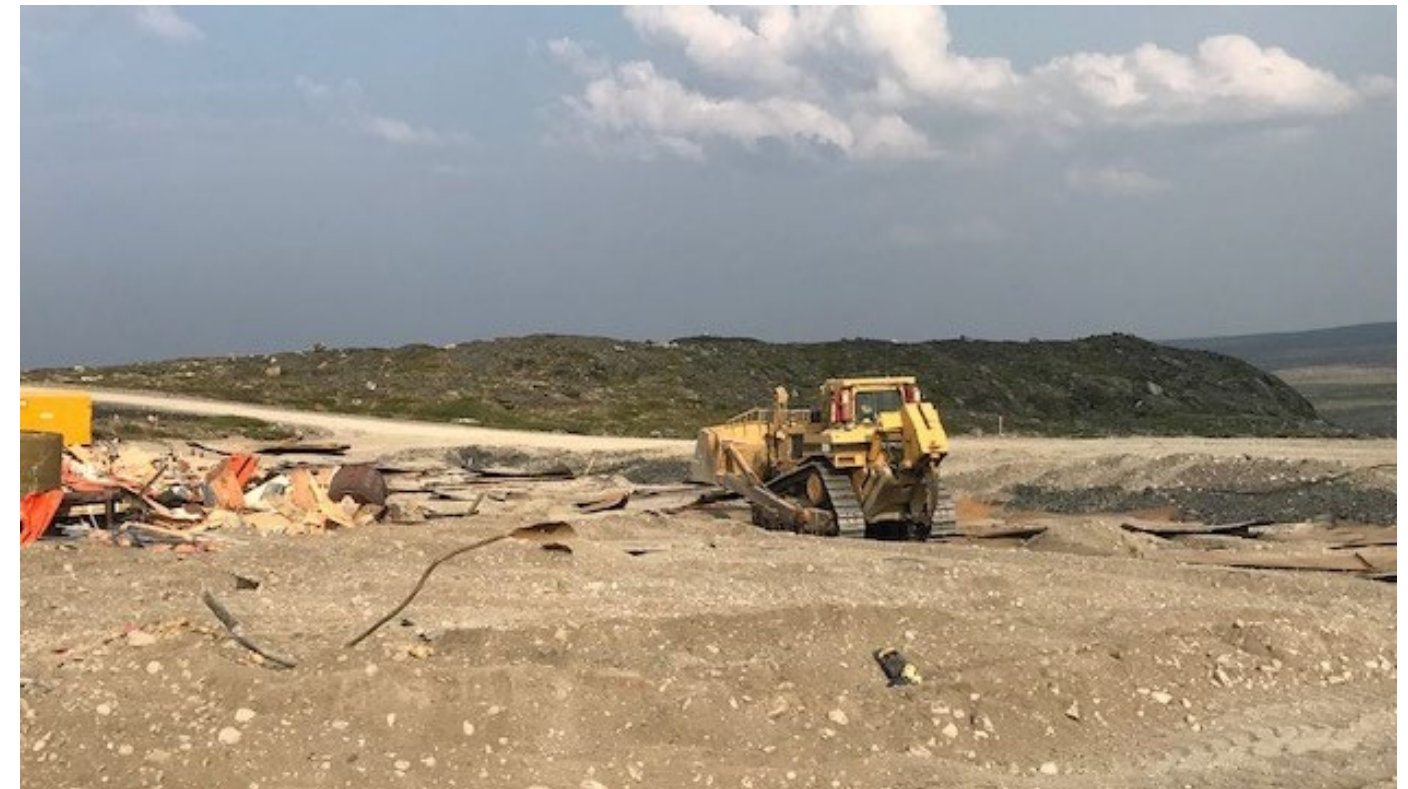
Bulldozer placing steel in the landfill. July 22, 2021
