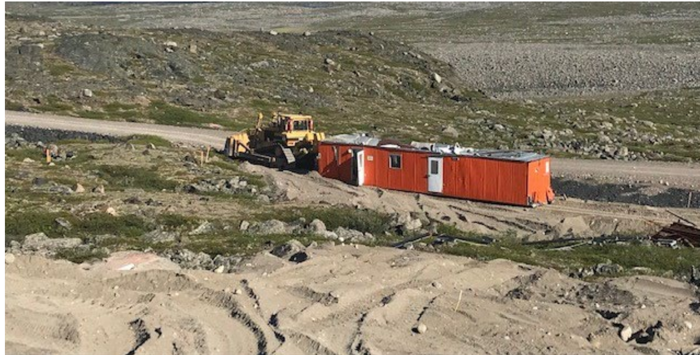
Disassembly of Bunkhouses on July 19, 2021
