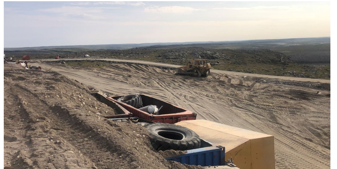
Esker sand placed over waste. August 13, 2021
