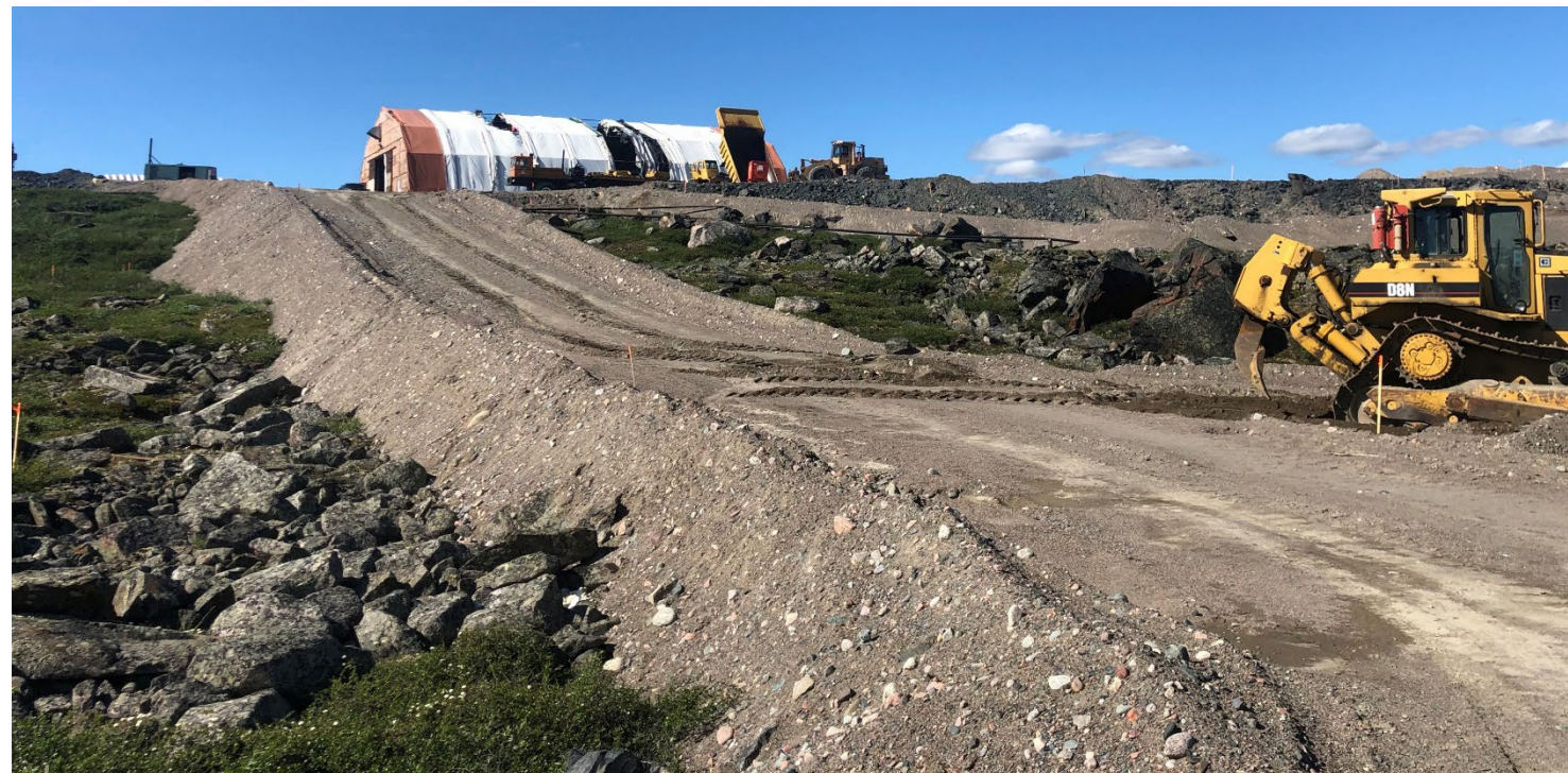
A new access road under construction on July 7, 2021
