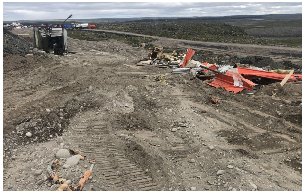
Debris placement and esker cover on July 16, 2021
