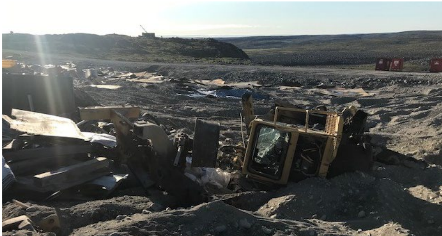
Surface haul truck placed. July 24, 2021
