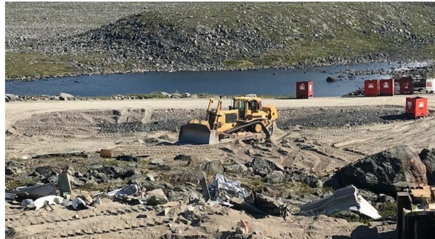
Esker sand placed over bunkhouses on July 21, 2021
