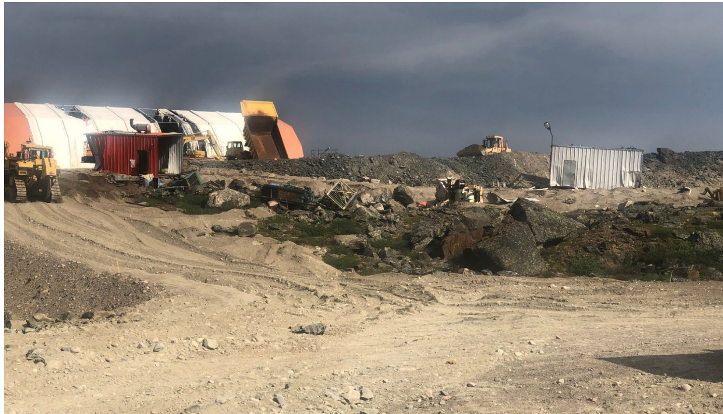
The south side of the site facing north on July 7, 2021
