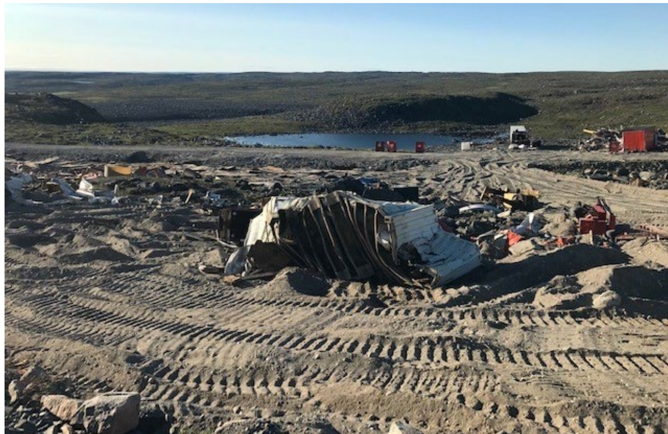
Seacan filled and compacted in landfill on July 24, 2021
