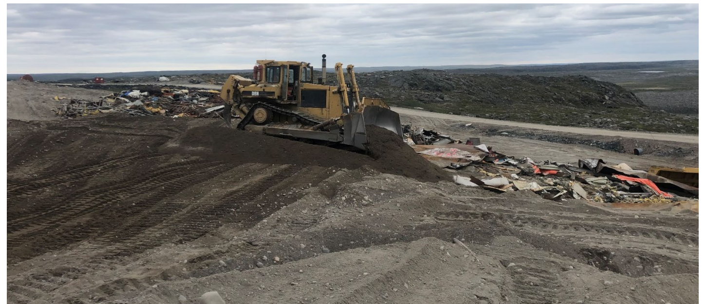
Placing esker sand on August 9, 2021
