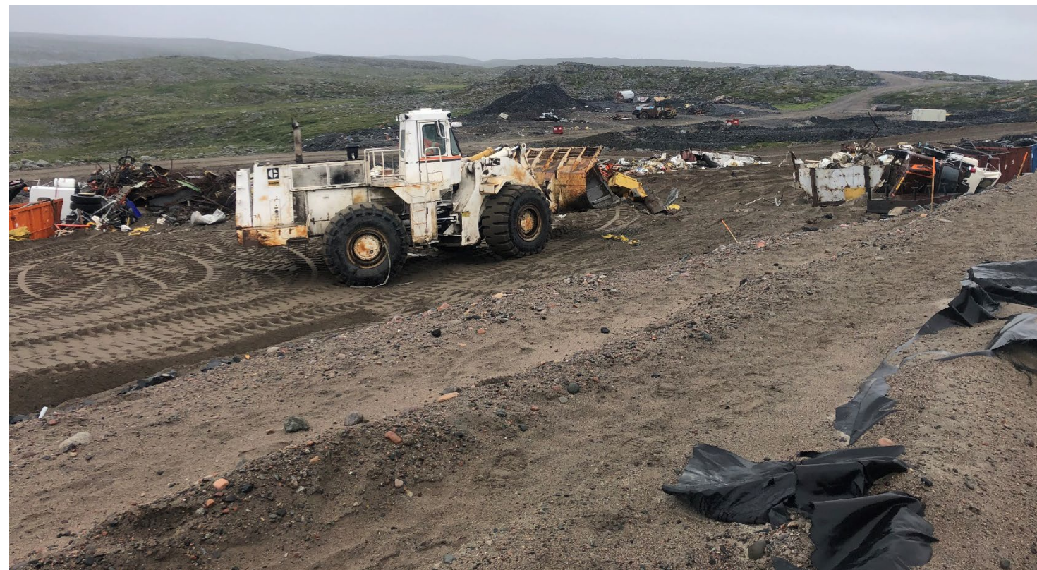
The northeast side of the site facing southwest on August 3, 2021
