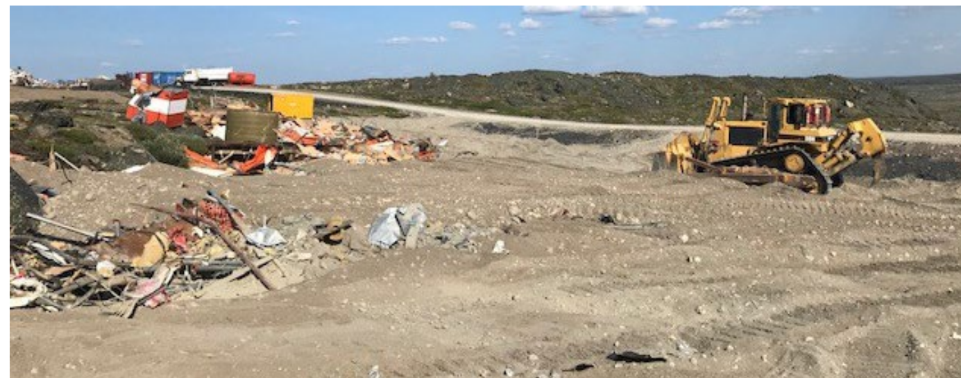
Esker sand placed over bunkhouses on July 21, 2021
