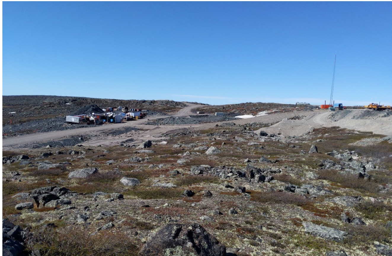
The east side of the site facing west as of June 25, 2021
