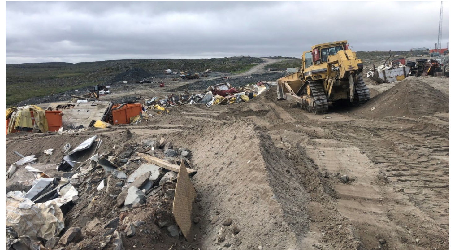
The east side of the site facing west, esker placement within voids and wind cover on August 3, 2021
