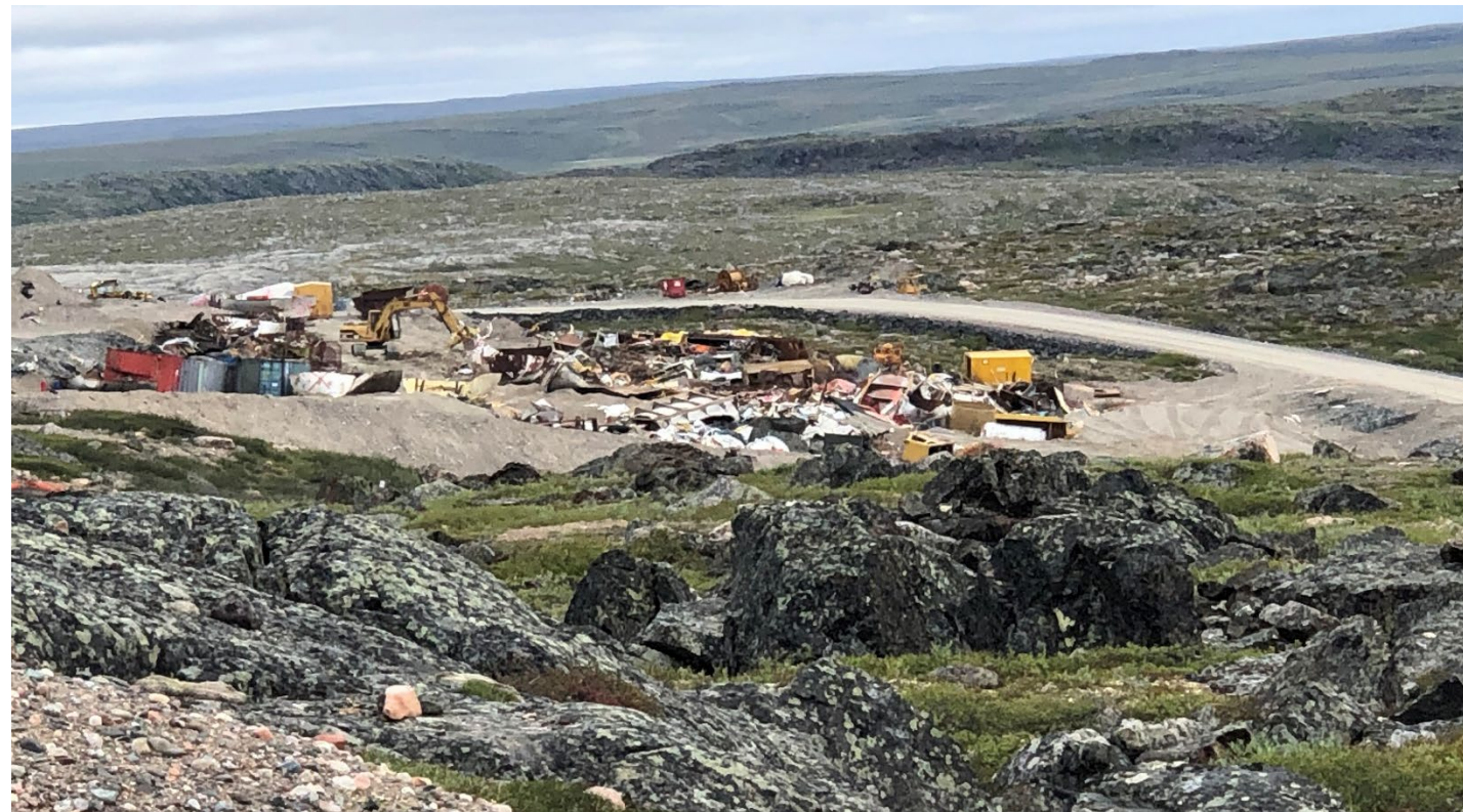
The west side of the site facing east with material placement on August 7, 2021
