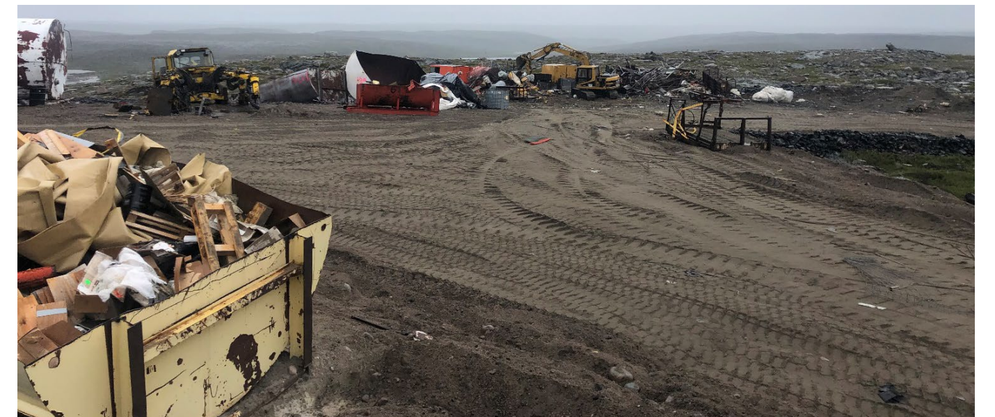
Loading waste in tanks on August 3, 2021
