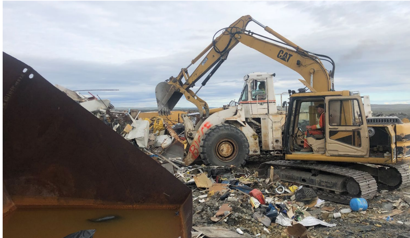
Waste placement and compaction on August 2, 2021
