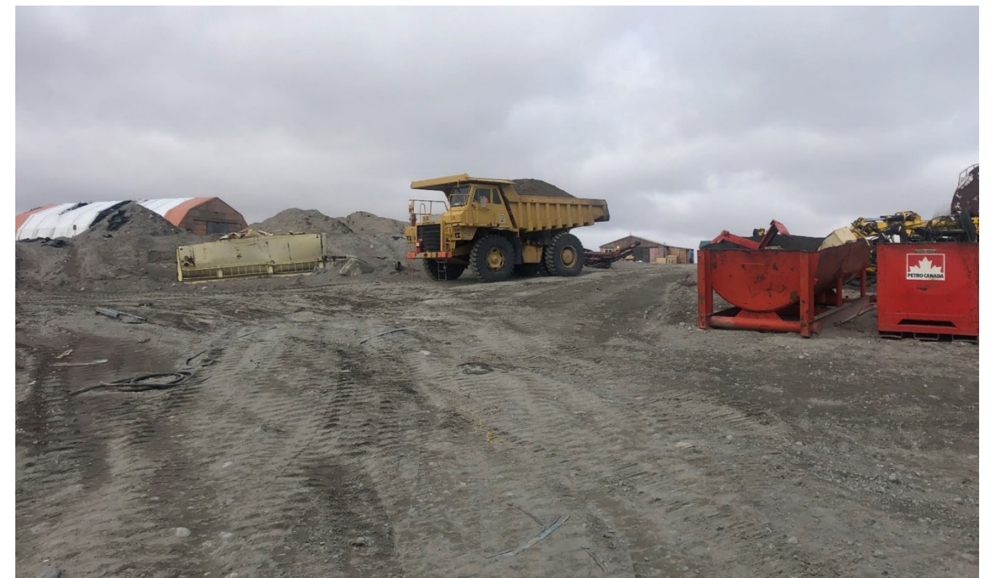
Unloading esker sand on August 3, 2021
