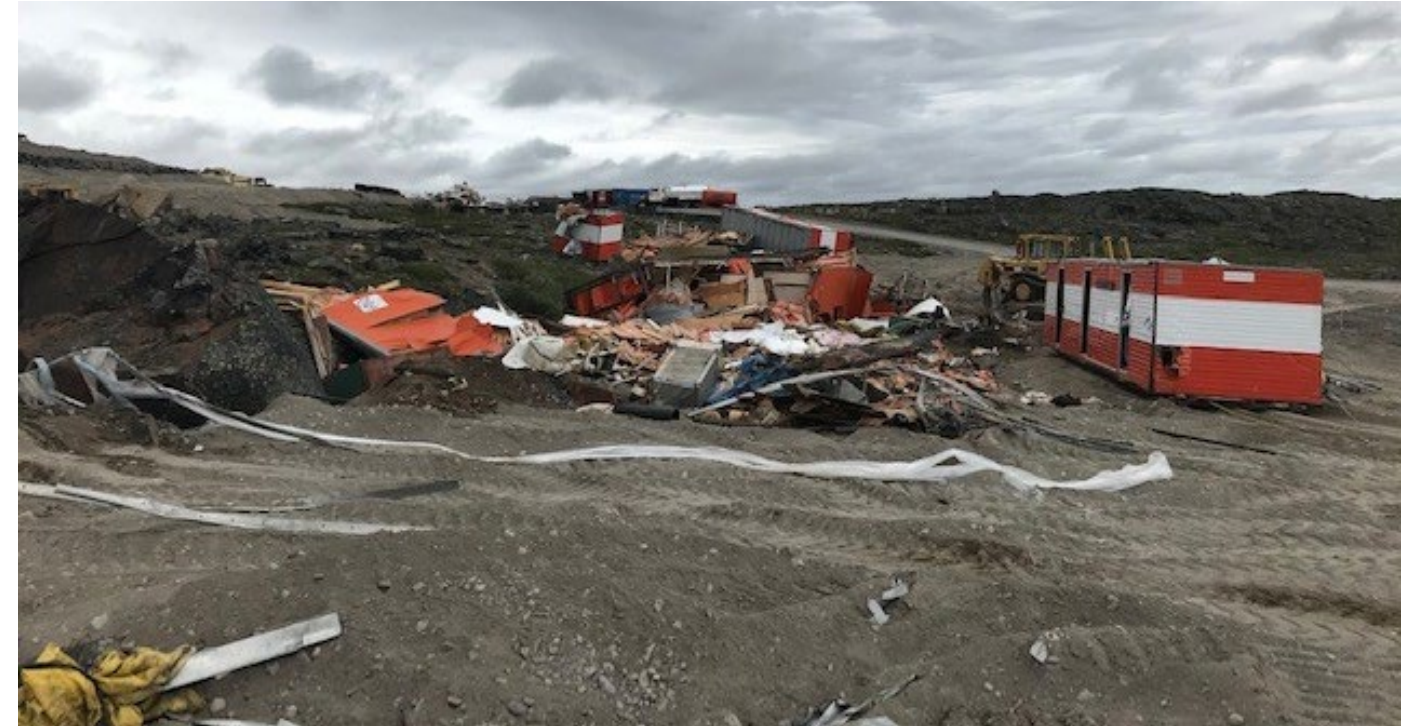
Continued bunkhouse placement and disassembly on July 19, 2021
