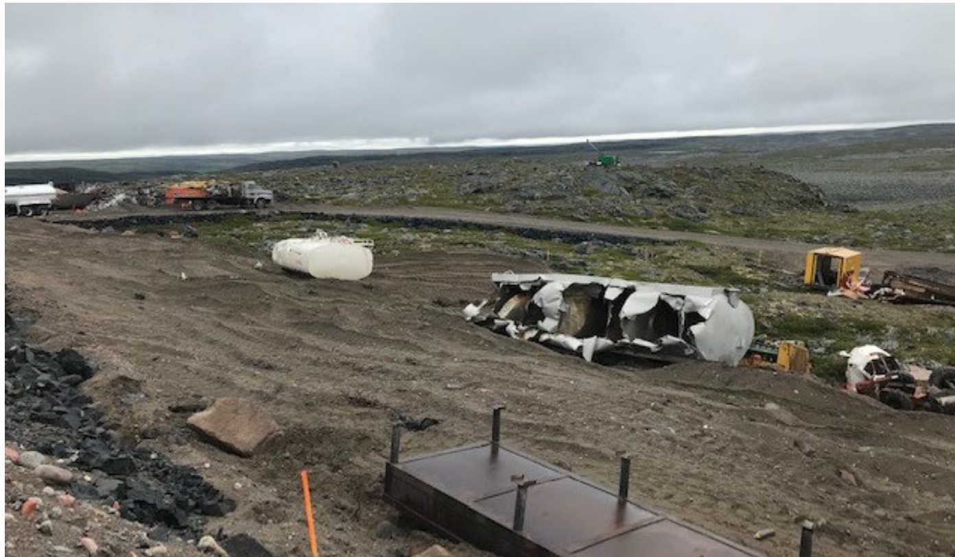
Clean tanks were staged in the landfill for cutting. July 25, 2021
