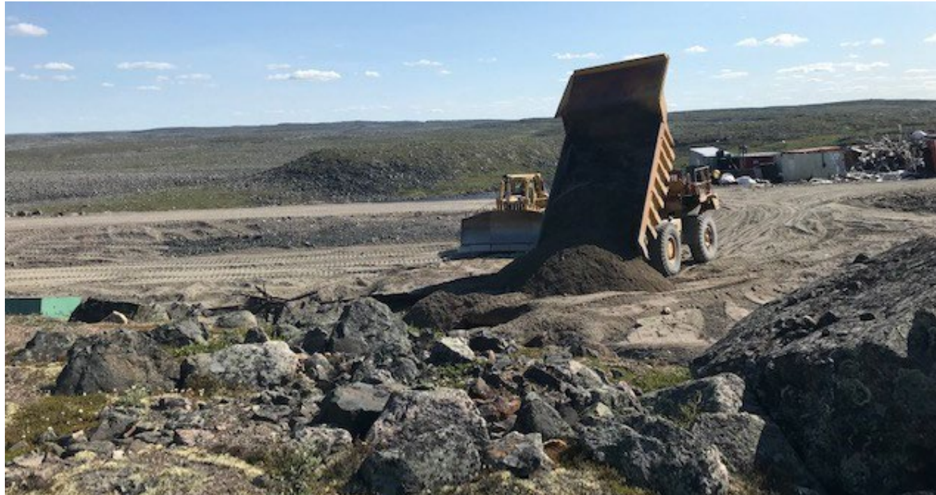
Esker sand used for access and foundation leveling on July 15, 2021
