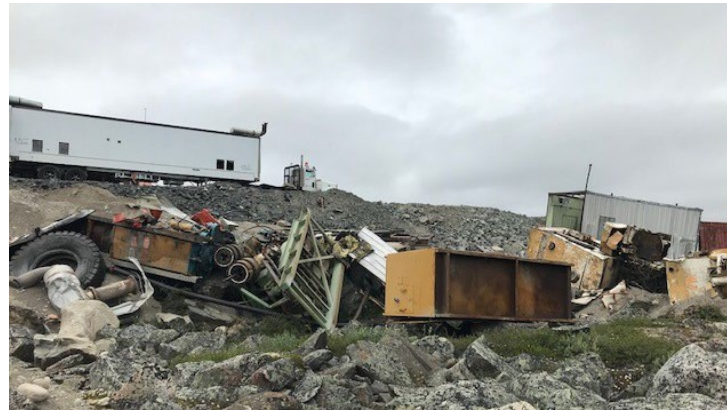
The south side of the site facing north on July 19, 2021
