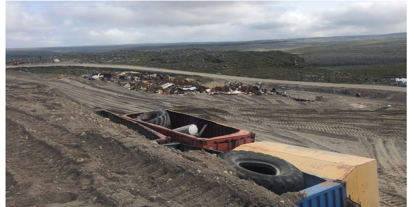
Esker sand placed over waste. August 10, 2021
