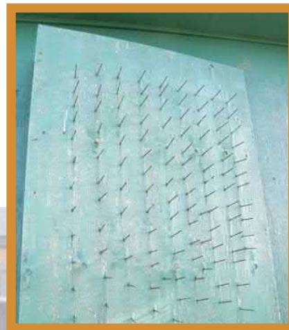
Properly-spaced nails on a bear board covering a cabin door
