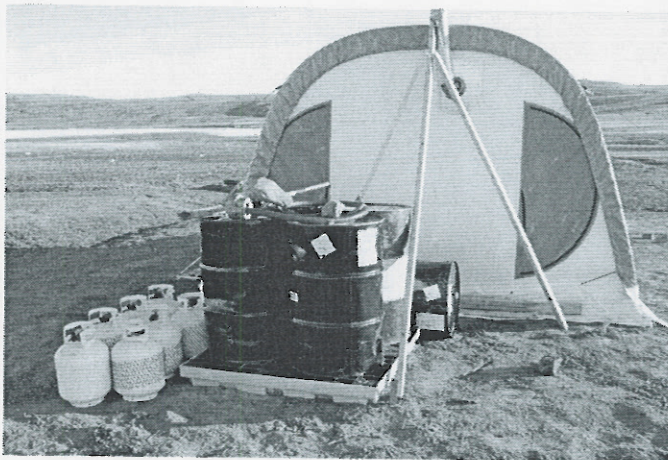
Fuel storage August 2014. 2.5 drums of diesel heating fuel are stored on a rigid pallet, and an empty drum (on side) for emergency use is available. Pump on drums is removed seasonally.
