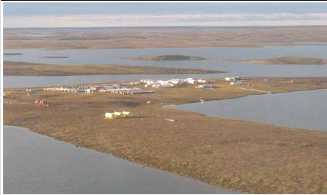
PHOTO 50. Meliadine West Gold Project, camp. Darker green near buildings is vegetation that has developed since the camp has been built.
