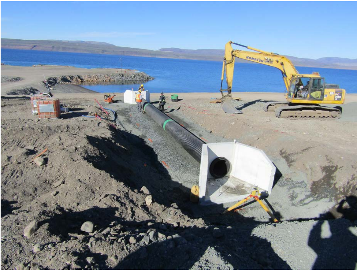
Figure 3. Installation of Culvert at Nanisivik 2015
