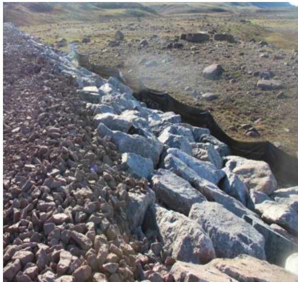
Picture 19: Silt fencing near crusher area
