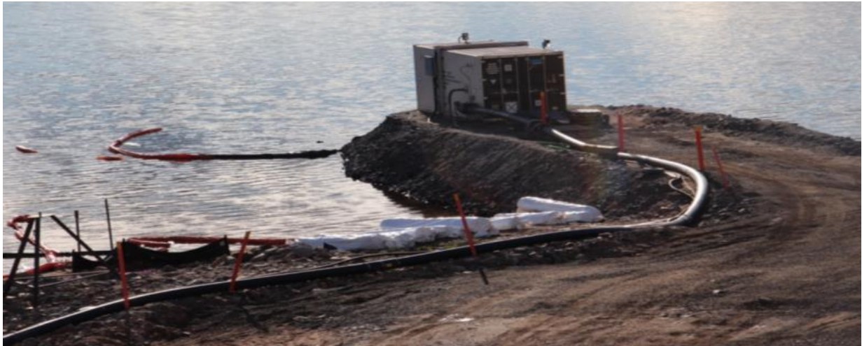
Picture 3: Jetty and freshwater intake area
