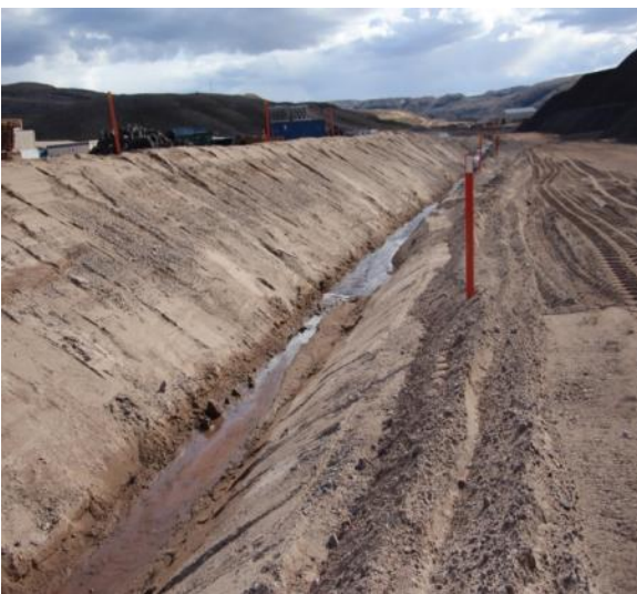
Picture 26: Ditching system around ore stockpile
