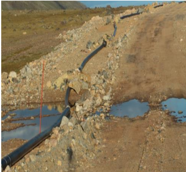
Picture 21: Sewage outfall pipeline
