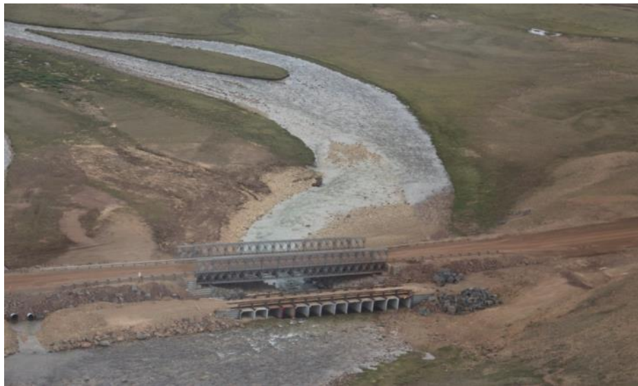
Picture 54: Bridge crossing along Tote Road
