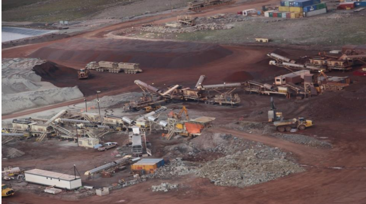
Picture 17: Crusher area
