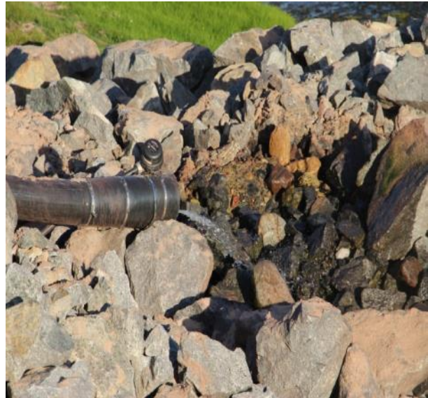
Picture 20: Sewage outfall area
