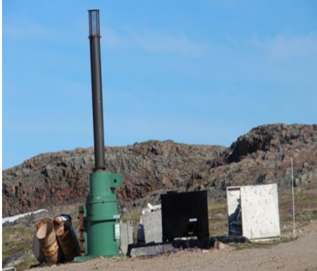
Picture 37: Unused incinerator stack and materials
