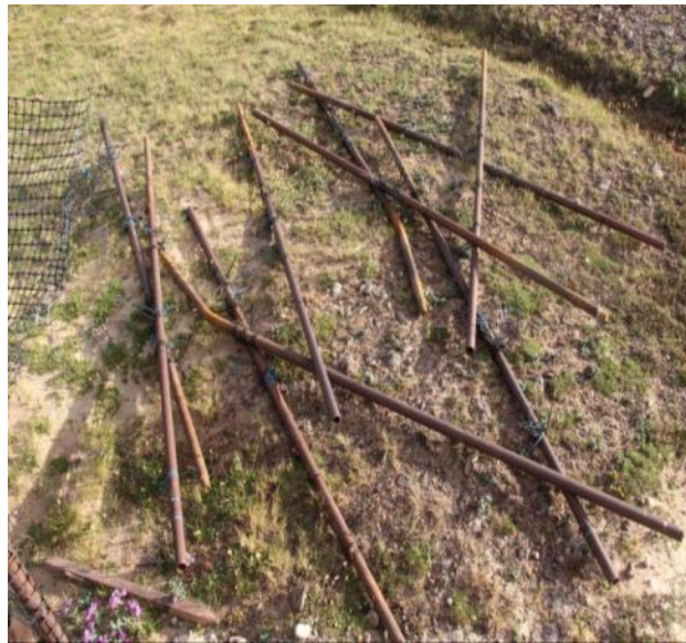
Picture 57: Damaged landfill fencing poles
