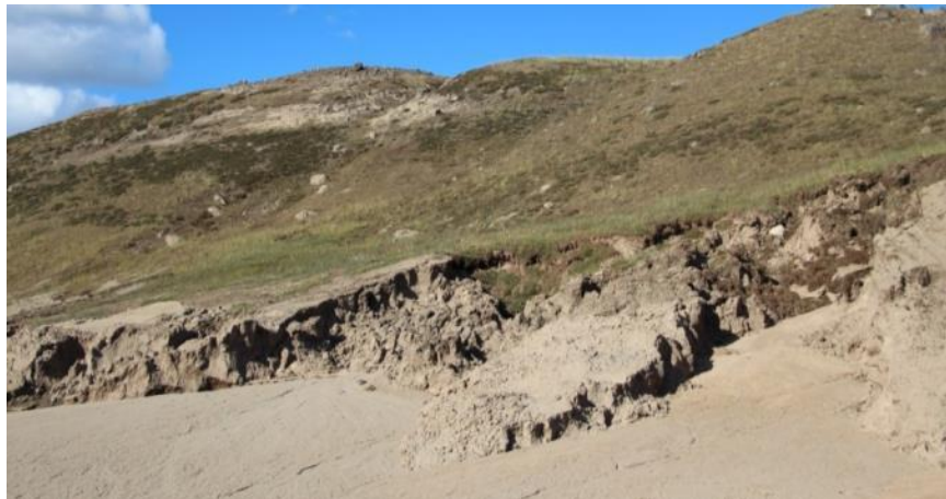
Picture 50: Embankment failures along Tote Road
