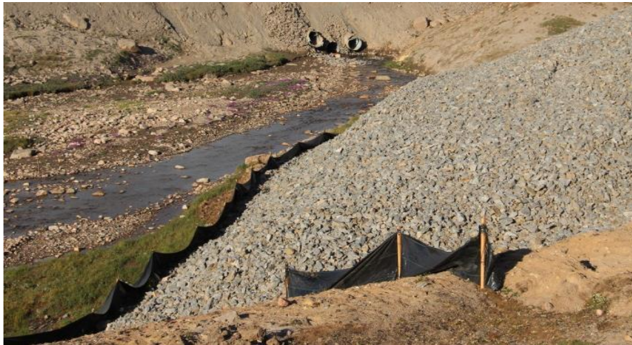
Picture 48: Embankment protection
