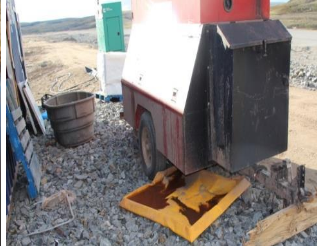
Picture 5: Use of spill pans at site
