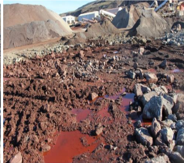
Picture 18: Soil sloughing around crusher area
