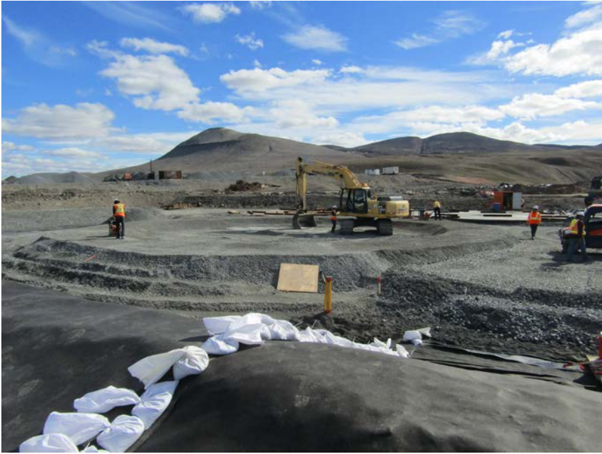
Figure 3. Diesel Tank Containment Construction
