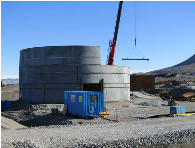
Figure 2. Naval Distillate Tank Construction
