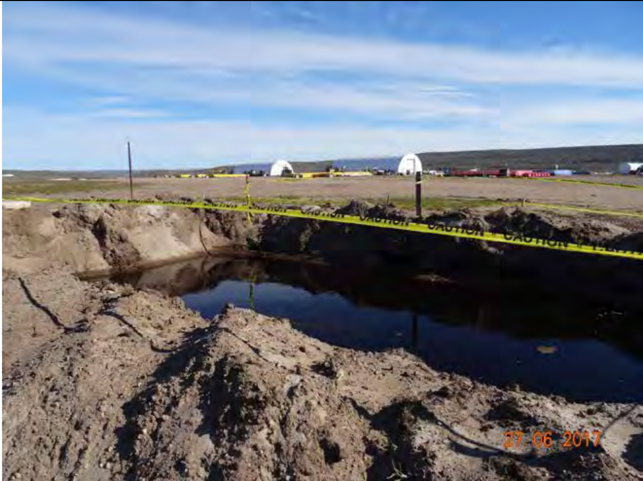
Description: Temporary holding pond for WWTP discharge. This is to be reclaimed as soon as possible to prevent impacts to the permafrost below.
