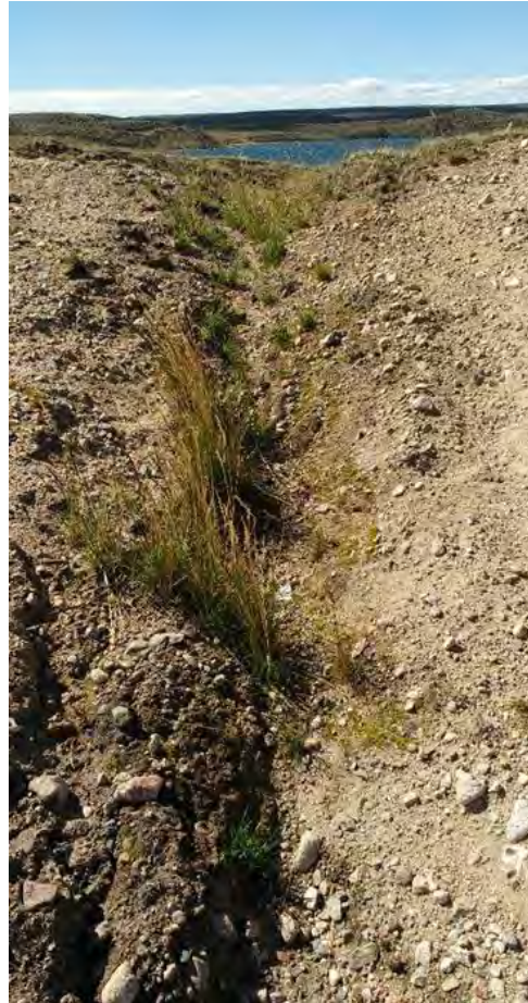
Figure 12: Close-up of grading causing slight blockage to natural drainage on western side of Burrow Area 1: July 8, 2017 (facing N)
