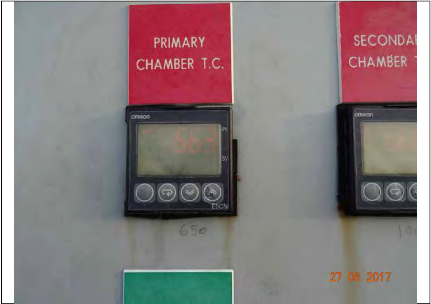
Description: Low temperature and sensor errors showing on incinerator.
