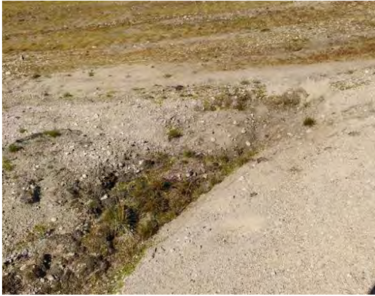
Figure 12: Close-up of grading causing slight blockage to natural drainage on western side of Burrow Area 1: July 8, 2017 (facing N)
