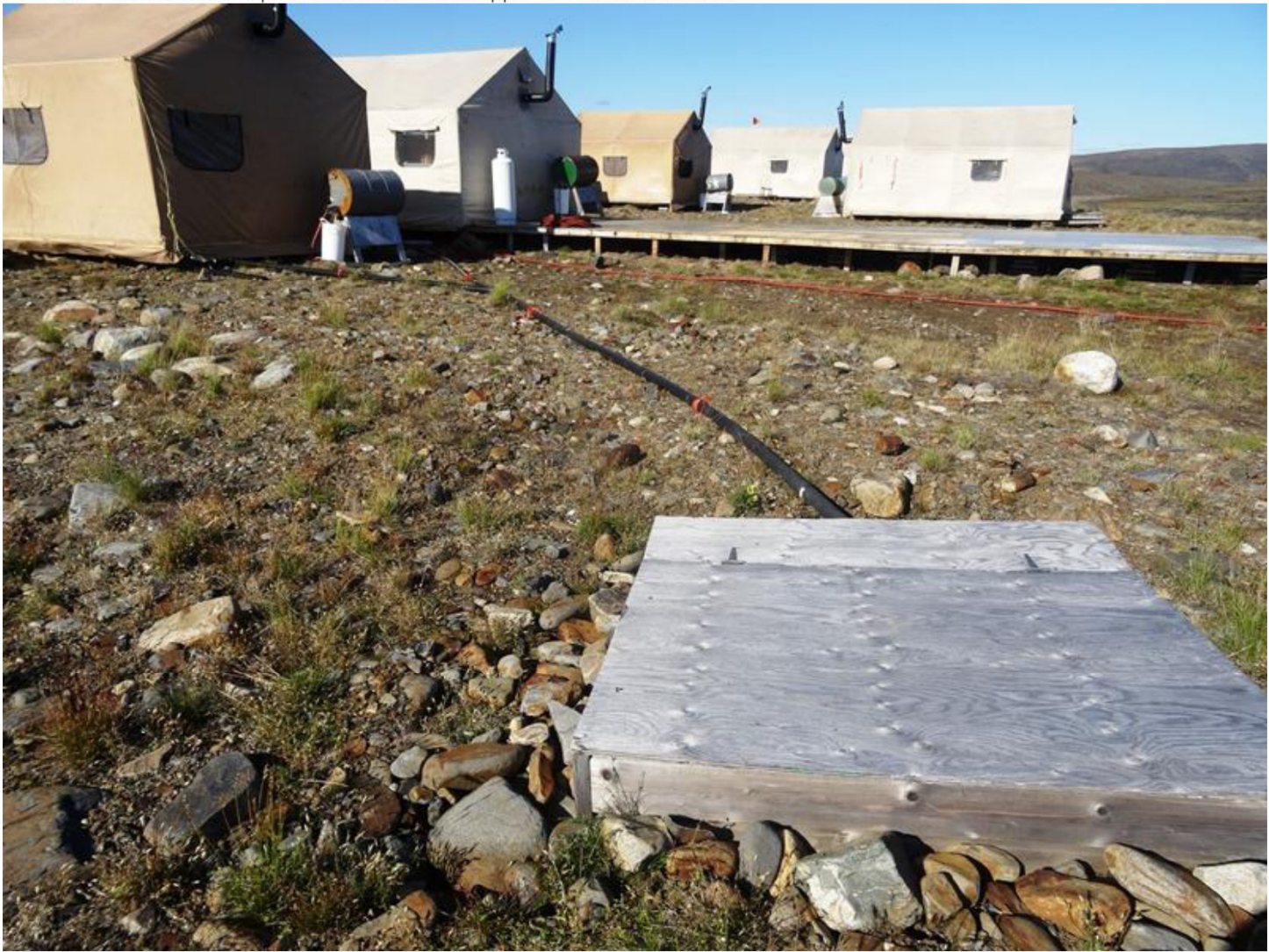
Photo 3: Sump where greywater is discharged.
