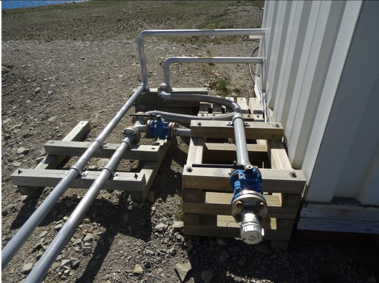
Description: 2 Unsecured Pipeline Valves beside Beach Tanks Pump House
