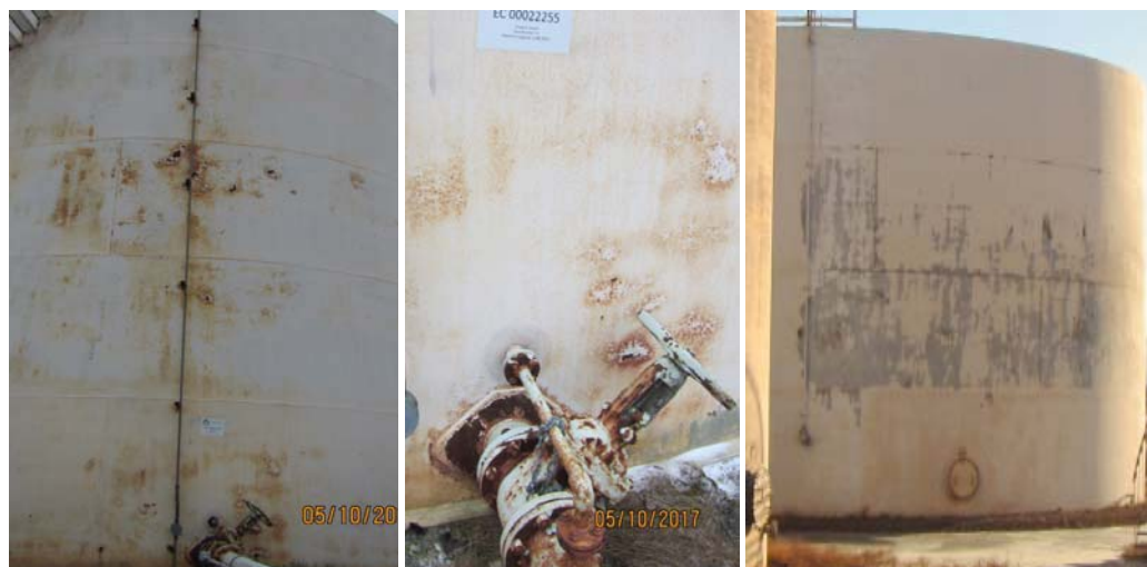
Figure 25: Tank #10 (left), Tank #11 (centre) and Tank #12 (right) exterior shell wall paint deficiencies.
