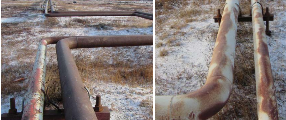
Figure 5: Aboveground pipeline expansion loops with incorrect pipe guide support practice.
