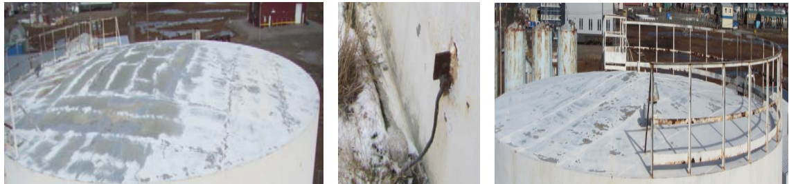
Figure 11: Rusty grounding lug and cable (centre). Tank # 11 (right) and Tank#12 (left) partial roof handrails.
