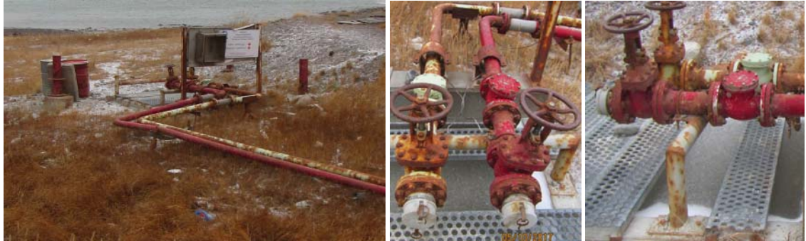
Figure 3: Shore manifold and marine spill basin. Shore manifold is lacking sea hose valve cover and chain lock on gate valves to prevent accidental spillage or vandalism.
