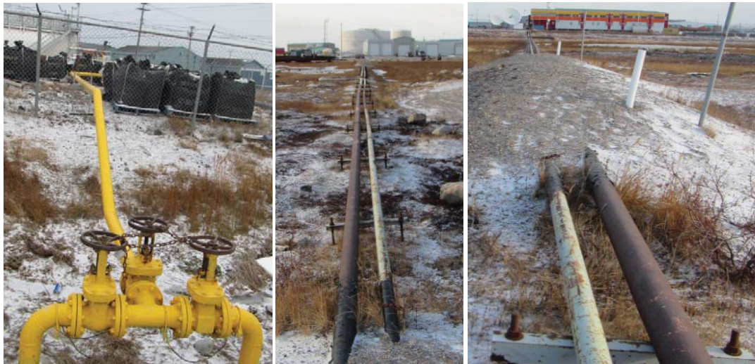
Figure 6: Resupply pipeline aboveground pipeline sections. ULSDL piping to QEC power plant (left). ULSDL and gasoline resupply pipe line aboveground section, downstream of 6th street road crossing (centre and right).
