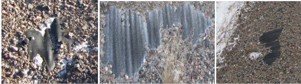
Figure 15: Exposed geomembrane that covers HDPE liner.
