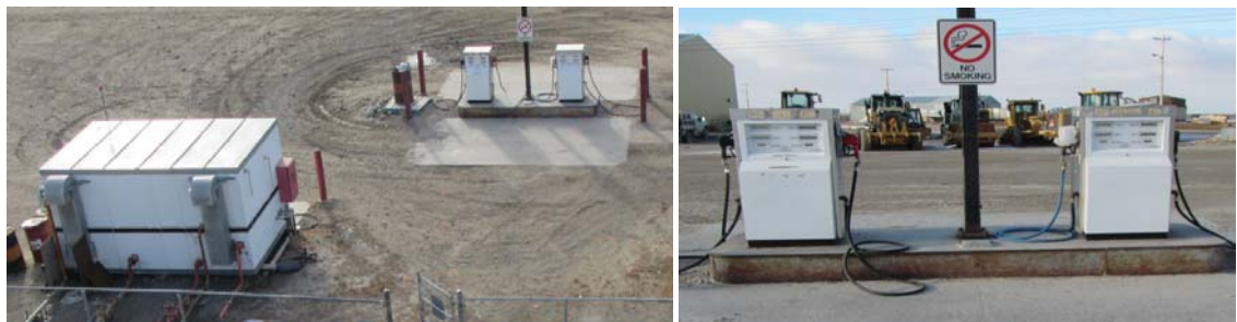
Figure 22: Remote Dispenser Island and dispenser building (left). Gasoline and ULSDL dispenser cabinets located in the remote dispenser island (right).
