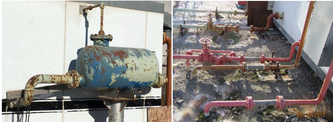
Figure 21: ULSDL relaxation chamber (left) and dispenser building inlet piping (right).
