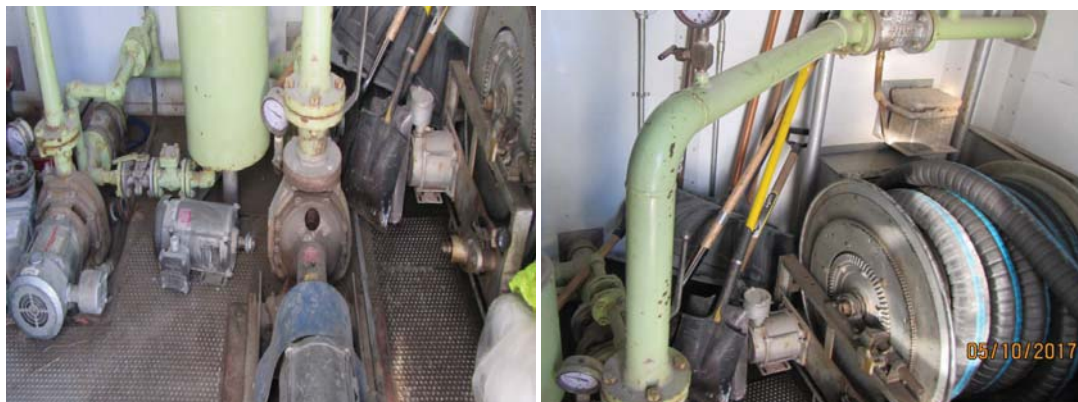
Figure 19: ULSDL truck loading pump (left) with hose reel assembly (right).
