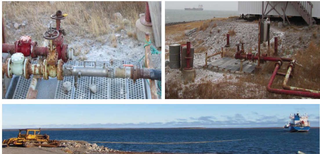
Figure 4: Resupply fuel tanker and shore manifold shown on top. Fuel floater hose approximate length is 700 meters from fuel tanker to the shore manifold. Fuel tanker anchored by a grader during resupply operation shown on bottom.
