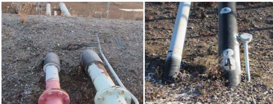
Figure 16: Berm penetration single wall resupply pipeline.
