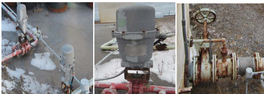
Figure 14: Existing non-functional motor operated valve (MOV) on gasoline and ULSDL lines (left and centre). Typical tank inlet & outlet piping nozzle layout (right).
