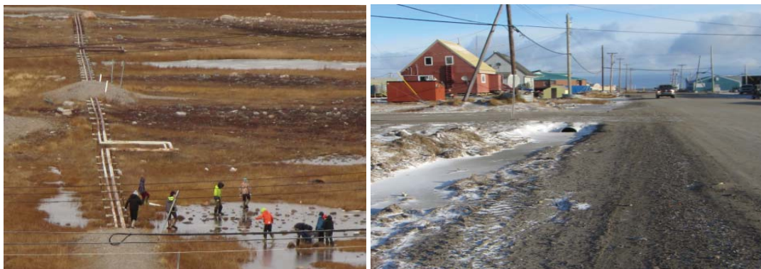
Figure 8: Aboveground resupply pipeline (left) and underground section (right) runs parallel to 6th street, centre of community.
