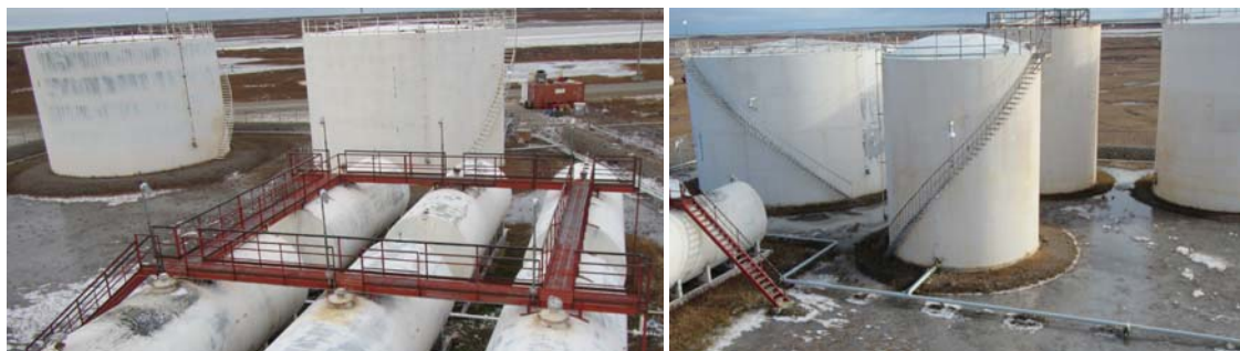
Figure 10: Tank #10 and Tank #11 (left). Tank #6(9), Tank#12, Tank#23 and Tank #24 (right). Water lying around tank foundations.
