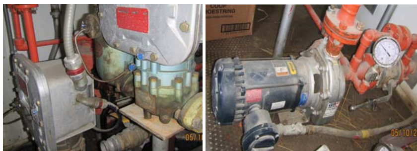
Figure 18: Gasoline and ULSDL meters inside the dispenser building (left). ¾ HP Gasoline light vehicle pump (right).
