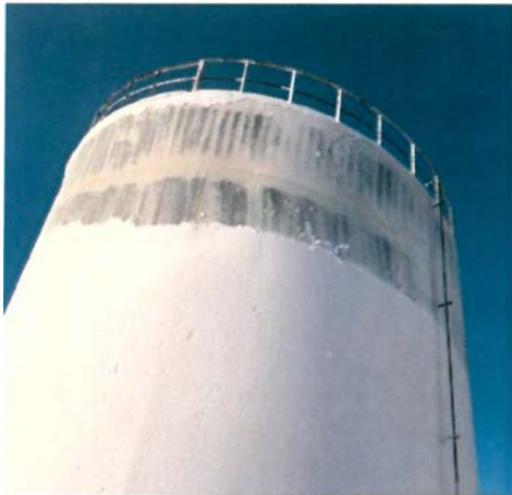
Figure1. Coating failure - gray primer.
