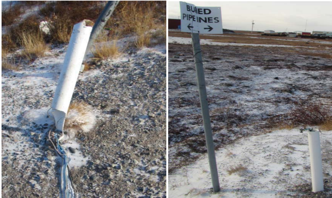
Figure 7: Damaged CP test stations along resupply pipeline.
