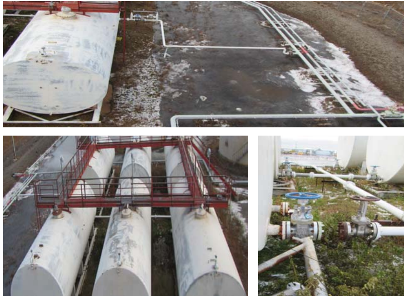
Figure 9: Horizontal tanks tied-in to ULSDL piping in 2017 summer (top). Overview of horizontal tanks (bottom left). Horizontal tank interconnecting piping (right). Grass and moss growing out from under the tanks.
