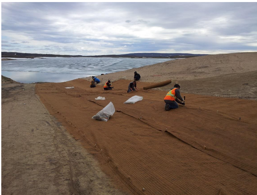
Figure 21: Additional coconut matting installation to the right, dark grey coconut matting installed during 2017 on the left (Facing: South).
