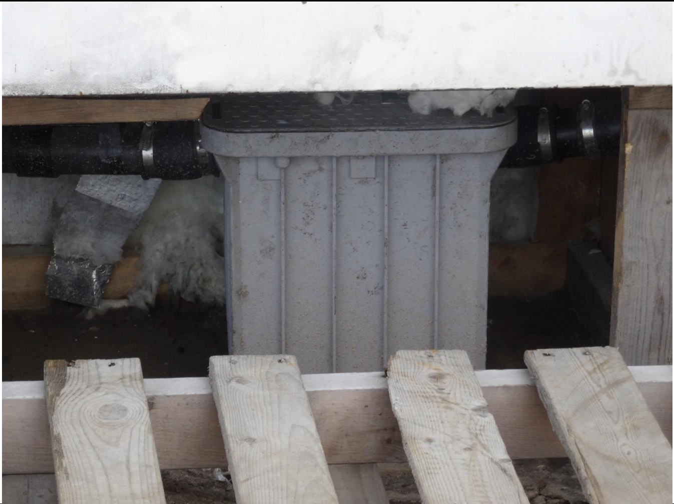
Description: Close-up of Kitchen Grease Trap installed as per Inspector Eva Paul’s direction from last Inspection – Thank You
