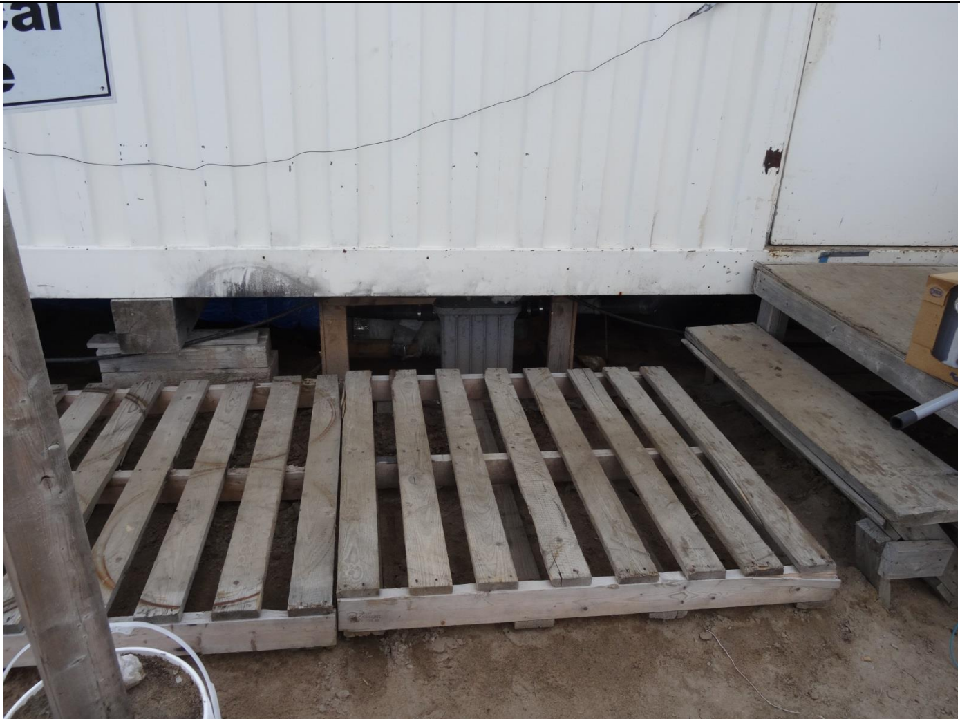
Description: Kitchen Grease Trap installed as per Inspector Eva Paul’s direction from last Inspection – Thank You
