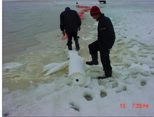
Figure 9.5: Absorbing pads being applied on spilled products
