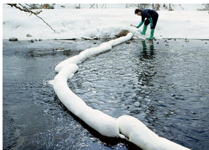
Figure 11.8 Boom Deployment
