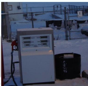
Figure 13.1: A modern RDR diesel dispenser
