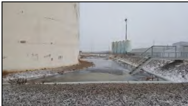
8 : Pooling water in area used to discharge standing water off site.
