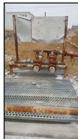
36 : Resupply manifold, spill basin and pipelines.
