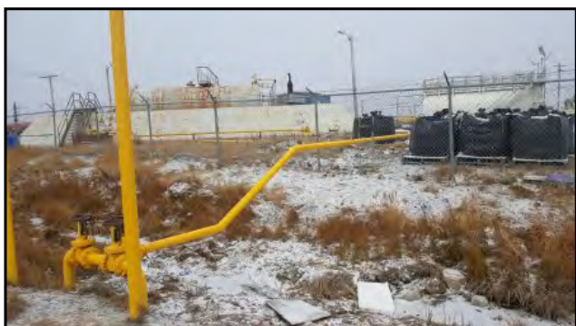
29 : Pipeline connection between Qulliq Energy Corp. facility and resupply pipelines.
