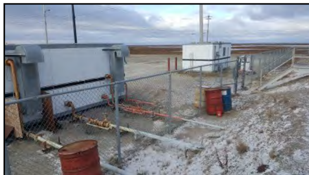
22 : Aboveground pipeline connection to dispenser building.
