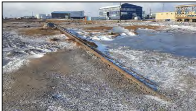
32 : Uncovered section of buried resupply pipelines.
