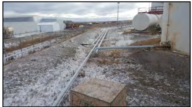
4 : Aboveground pipelines and berm in Arviat tank farm.
