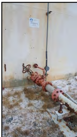
5 : Connection between aboveground tank and pipeline at Arviat tank farm.
