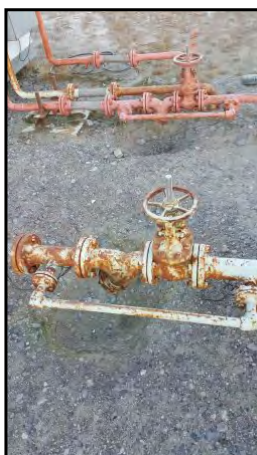
23 : Depressions below pipeline connections behind dispenser building.
