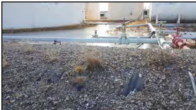
7 : Exposed liner beneath the tank farm berm.
