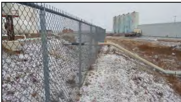
9 : Resupply pipelines entering tank farm.
