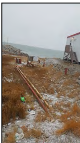
35 : Resupply manifold and pipelines.
