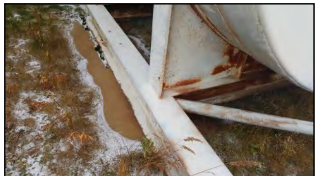
6 : Discoloration on tank and pooling surface water below horizontal emergency tanks.
