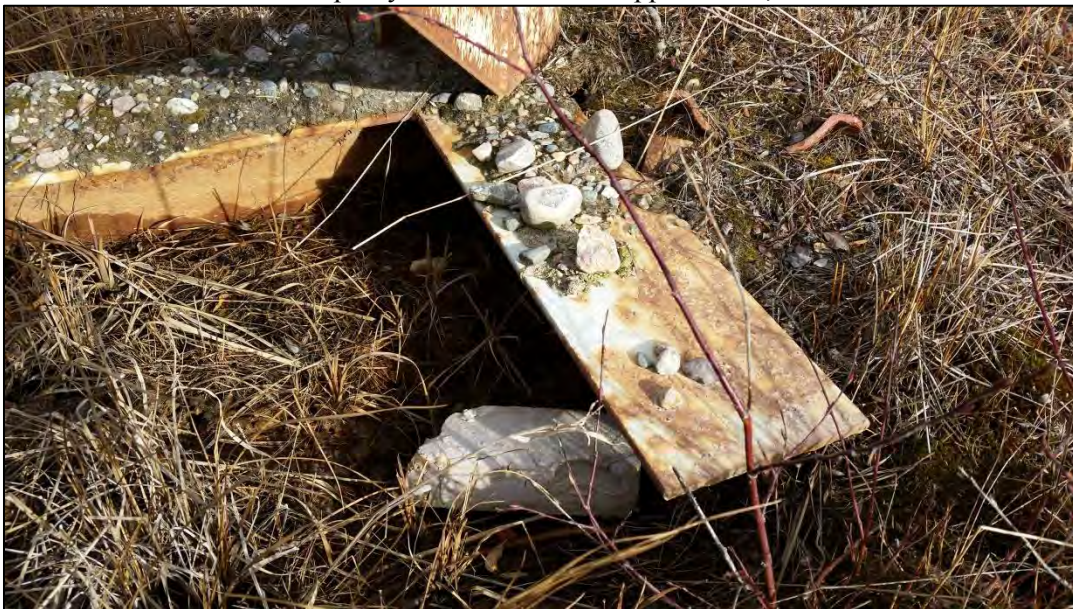
Photo 4 – View of partly unearthed EPLS support stand, October 5 2016.
